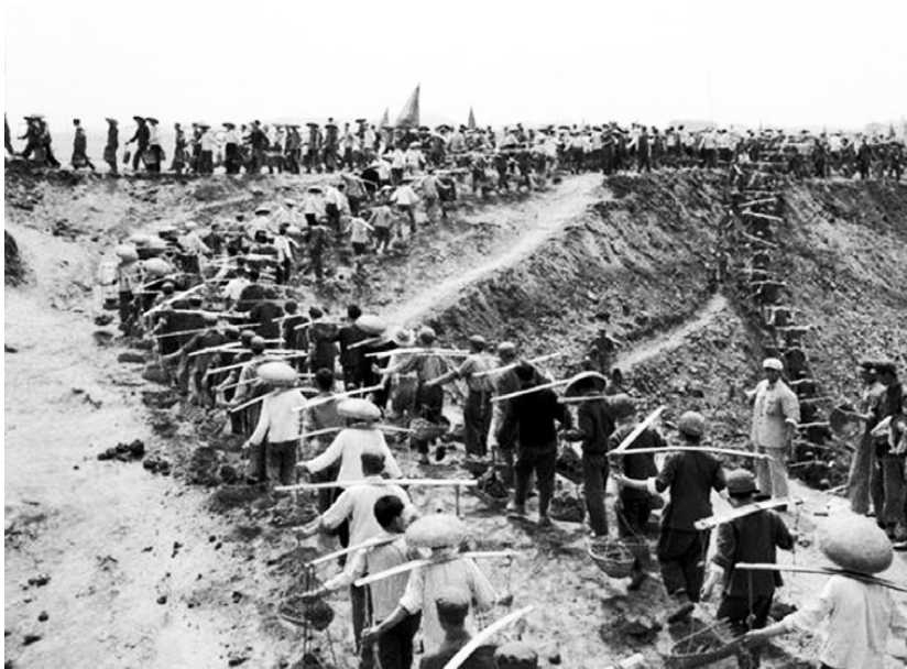
Figure 3.3 Building the Gezhouba Dam in 1970. Source: “Dujia Changjian le wanli changjiang di yi ba Gezhouba shuili shuniu gongcheng,” China Energy Engineering Group Co., Ltd, February 28, 2014, group.ceec.net.cn/art/2014/2/28/art_738_13.html
