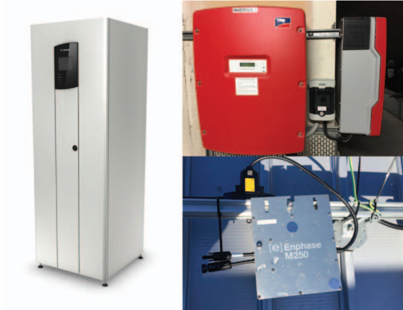
Hybrid inverter including battery storage (left) (Photo: Bosch Power Tec GmbH), 6 kW central inverter (top right) and a micro inverter located on the roof behind each panel (bottom right).
