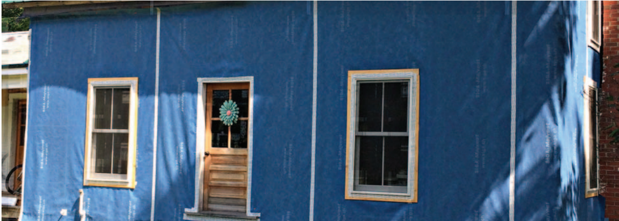
Photo of weathertightness layer. (Photo: Marc Coviello).
