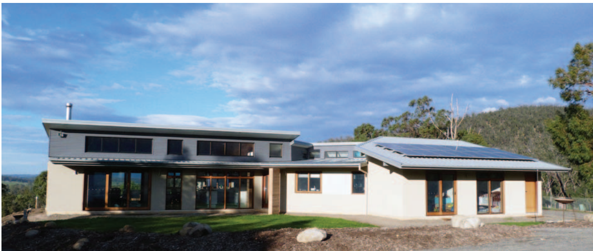
Home designed to optimise light harvesting, winter solar heat gain in the living area, summer solar control and solar electric harvesting (over the bedroom) (Photo: David Halford).
