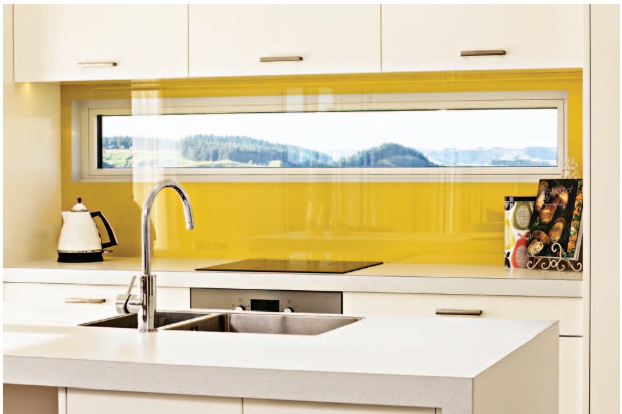
Outlook from the kitchen to the east. The window is fixed, and the splash back – left transparent over the window area – adds a third layer of glass (Photo: ecoBuild Developments Ltd).
