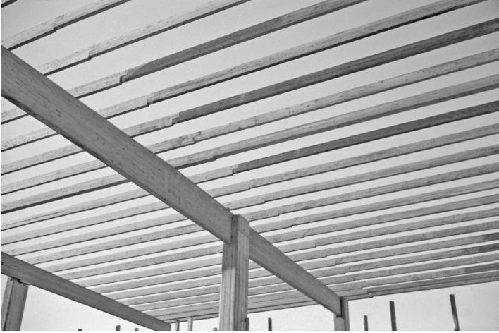
Fig. 3.1 Structural timber joists supported by glulam beams
