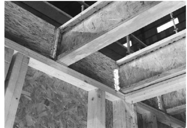
Fig. 2.23 Geometry of typical I-beams and metal web beams
