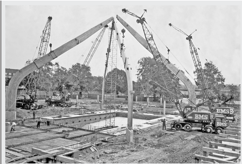
Erection of glulam portal frames
