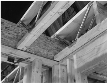
Fig. 2.23 Geometry of typical I-beams and metal web beams
