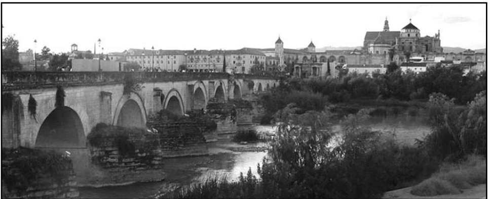
▲ The Córdoba Roman Bridge is still in use.
