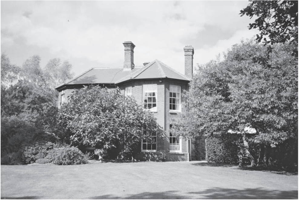
FIG. III.3. View of The Old Rectory from the garden, shortly before the house was sold (summer 2006). © Jo Catling
