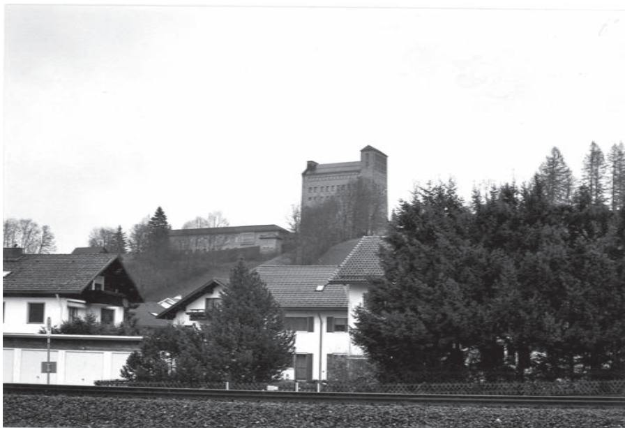
FIG. 2.44. The Ordensburg, Sonthofen (April 2005), one of three built by the Nazis as élite training schools 1934–37. The building, now the Generaloberst-Beck-Kaserne, dominates the hills to the east of Sonthofen and can be clearly seen in the centre/right of FIG. 1.12.
