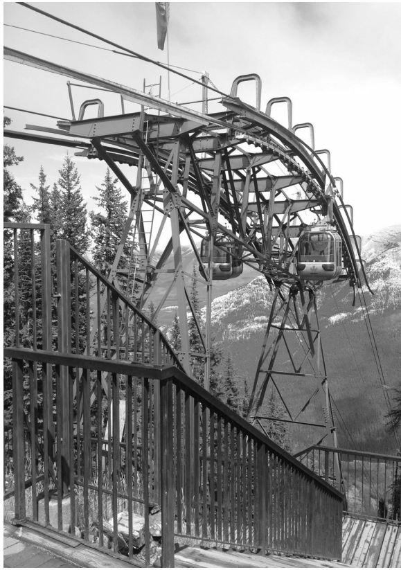
FIGURE 1-5a Aerial cable cars supported by steel space trusses at Banff National Park in Alberta, Canada (Photo by Abi Aghayere)
