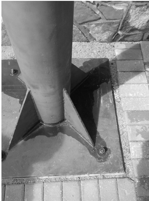
FIGURE 8-45b Base plate with stiffeners (Photo by Abi Aghayere)
