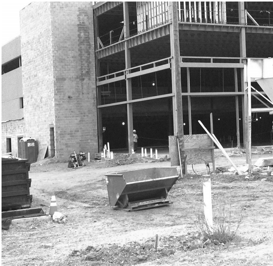
FIGURE 14-17c HSS girts and wind columns (photo by Abi Aghayere)
