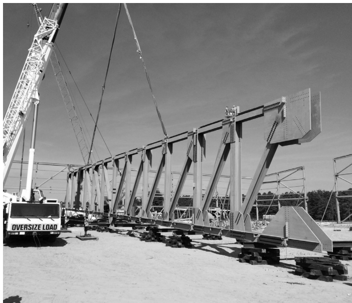
FIGURE 8-3b Bolted truss with continuous top and bottom chords (photo courtesy of Joe Messner, JGM Inc.)
