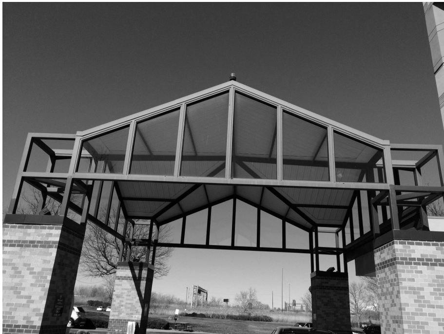
FIGURE 1-18g Vierendeel truss entrance canopy roof framing (Photo by Abi Aghayere)
