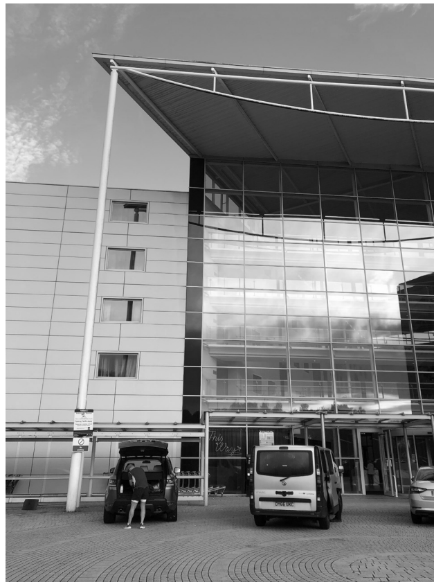
FIGURE 5-2c Slender column at an entrance canopy (Photo by Abi Aghayere)
