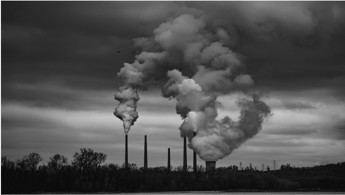
FIG. 7.1 Coal-fired power plant.
