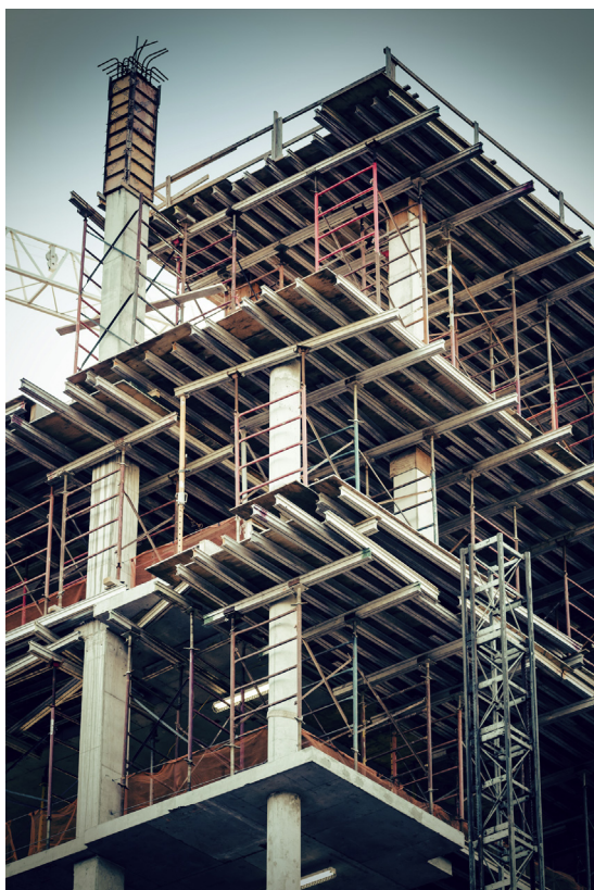
FIG. 7.2 Closed construction site.
