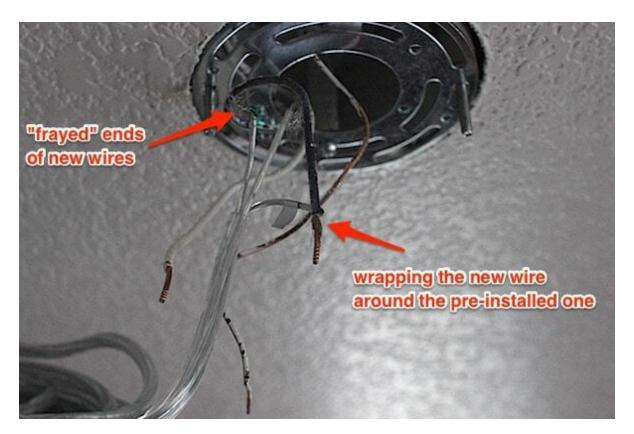
The wires descending from the ceiling will have bare ends, while the new wires will have what looks like frayed, silver ends. You can see that in the image above.
