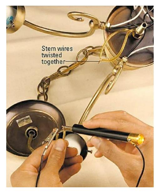
To test the stem wires, twist them together at the junction box. At the other end attach a continuity tester clip to one wire and touch the probe to the other wire. If the tester does not glow, replace the stem wires.
