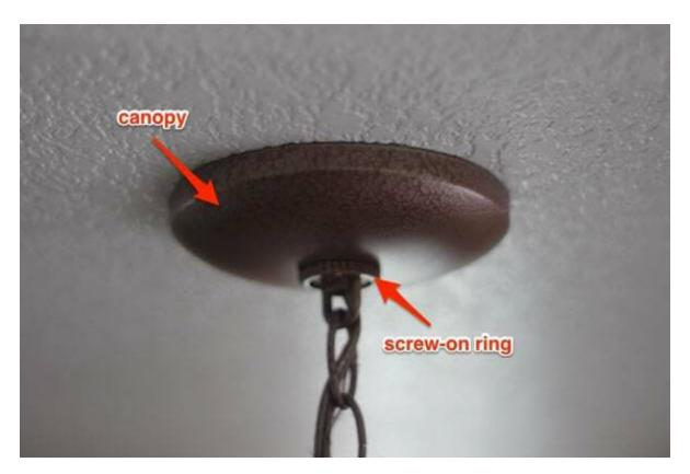
The fixture I was replacing used a simple screw-on ring to hold up the canopy (and fixture). Each fixture is different, but no matter what it is, it should be pretty easy to figure out.
