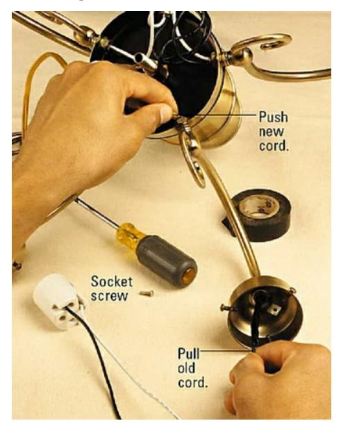
To replace a cord, separate, strip, and splice the old cord to the new. Pull the old wire through until the new wire appears. Attach the new cord to the socket.
