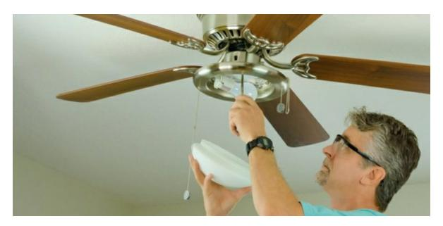
Once you discover that your switch is working, move to checking the ceiling fan wiring. Again, turn off the electricity to the room at the breaker box and, if you have someone to hold up the ceiling fan while you work, then just unscrew it from the ceiling. If you don't have an assistant, you will need to remove the fan blades and then unscrew the ceiling fan from its mounting bracket.
