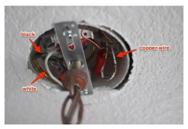
*Three sets of wires, each held together by a red wire connector.*
