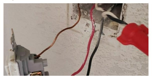
Gently remove the switch from the box and unscrew the two wires from their terminals. Then, use a small set of pliers to straighten out the ends of both wires. Twist the bare wires together and use a wire nut to hold them in place.
