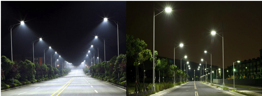
Figure 6.5 LED street lights. LED , light-emitting diode.
