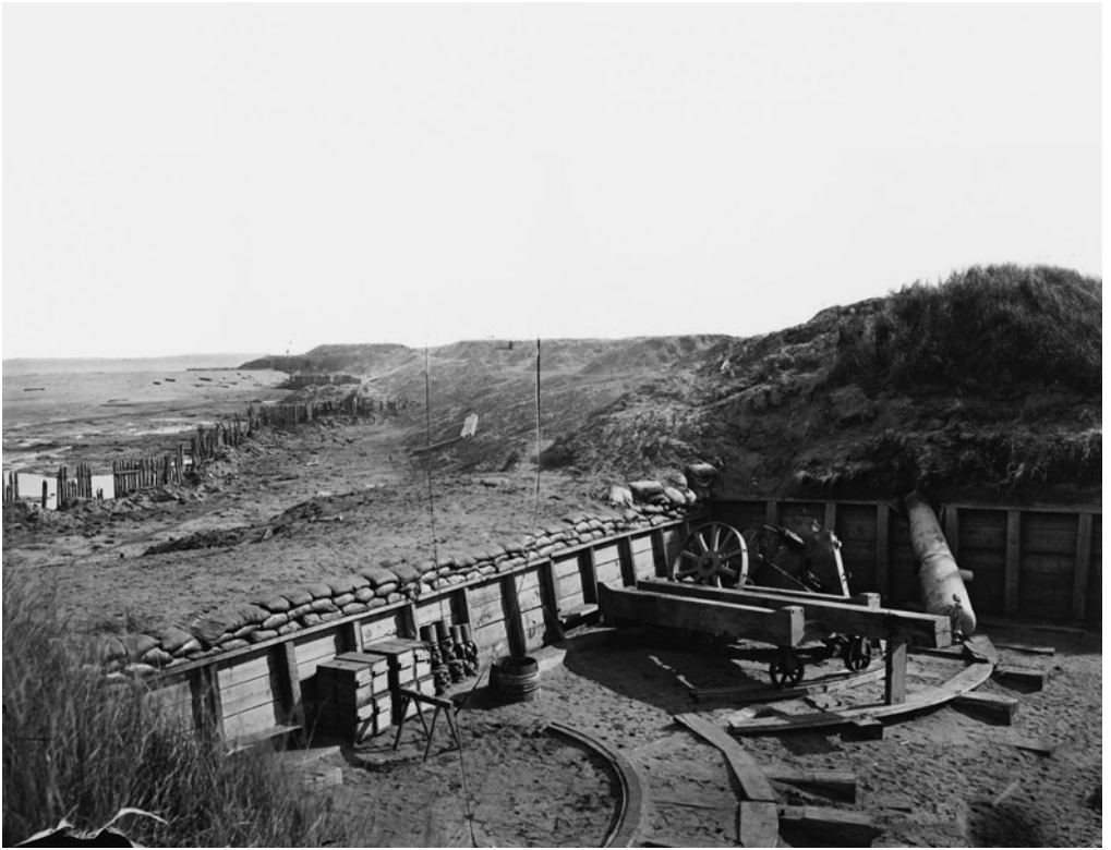
Part of the land face of Fort Fisher after the Union naval bombardment and army assault on January 15, 1865. Note the dismantled gun next to one of the traverses and the stockade splintered by Union shells.
