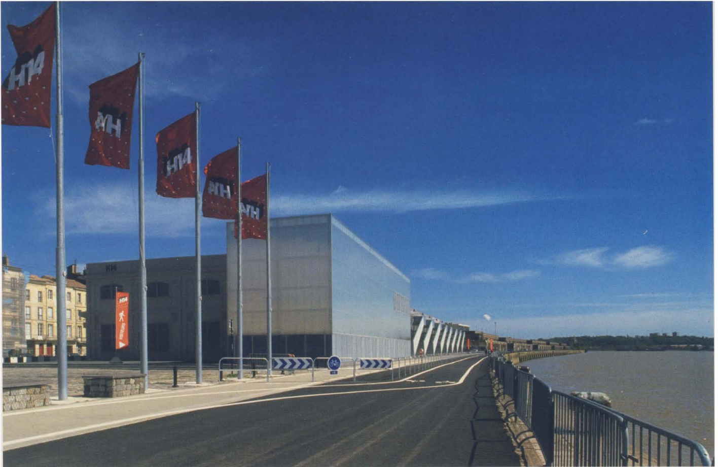
General view and detail of the external stairs
