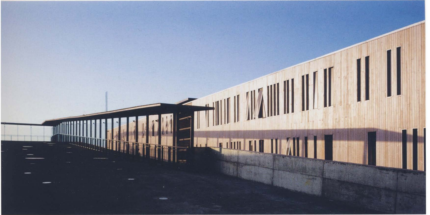
Detail of the portico
