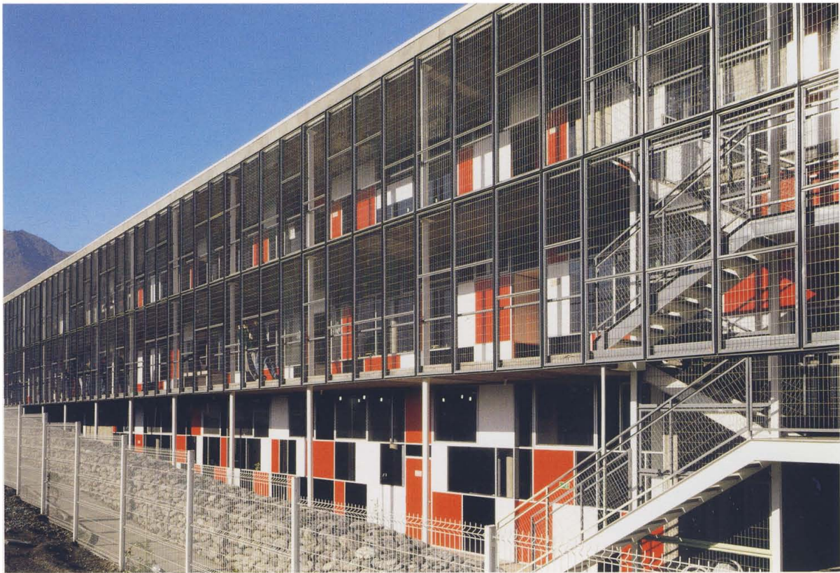
Detail of the external platform
