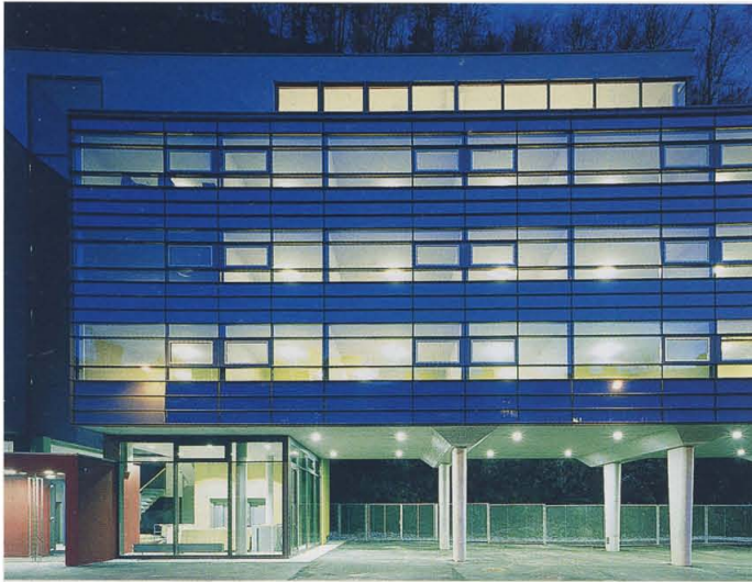
The main street facade
