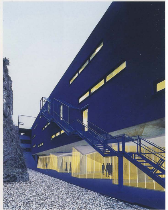
The fire stairs
