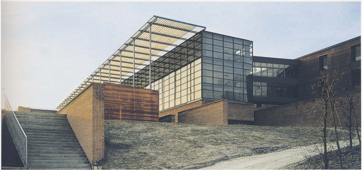
The portical and the waiting room
