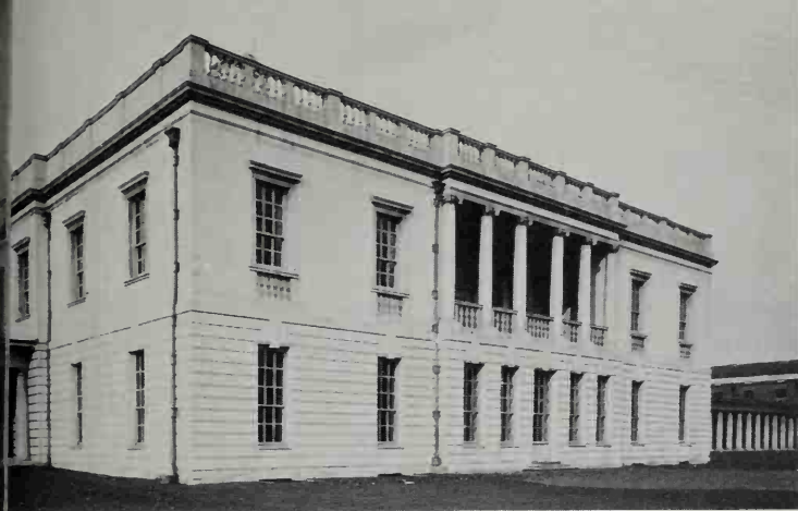
284 The Queen's House, Greenwich, by Inigo Jones (1616–35). Its elements – rusticated ground storey, plain wall, colonnade – all derive from Palladio; the skill with which they are handled is itself mature Palladian. Compare the scheme of the Palazzo Chiericati, Ill. 228
