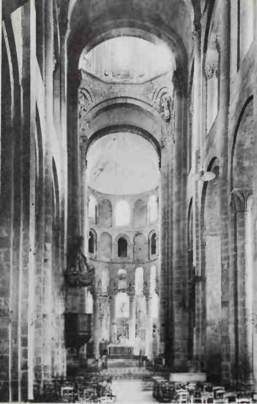
95, 96 Romanesque achievement and Gothic virtuosity: above, Ste-Foy at Conques (begun c.1050; see also p. 113) with high tunnel-vaulted nave, and crossing covered by a lantern on squinches; below, St Anne, Annaberg (begun 1499; see also p. 154) – the functional stone vault transformed into a fantastic pattern of ribs
