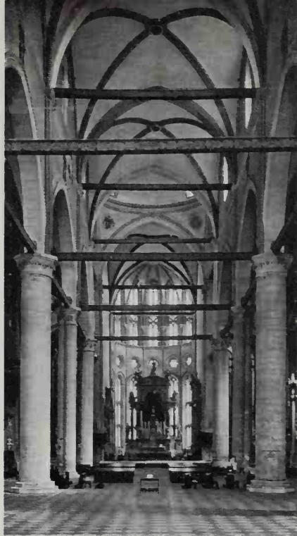
172 SS. Giovanni e Paolo, Venice (begun 1246). This vast church, impressive as it is, brings out the limitations of Italian Gothic. Widely spaced arches, circular piers and large areas of plain wall surface belong to a Romanesque, or even Roman, aesthetic, while the use of tie-beams shows a complete rejection of the Gothic system of abutment and of the effects which that system could achieve
