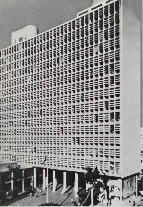
414 Ministry of Education, Rio de Janeiro (1937-43), designed by Costa and Niemeyer with Le Corbusier as consultant. This building, with its rich 'brise soleil' grid, shows how refinement can lift the standardized world office block to a new level
