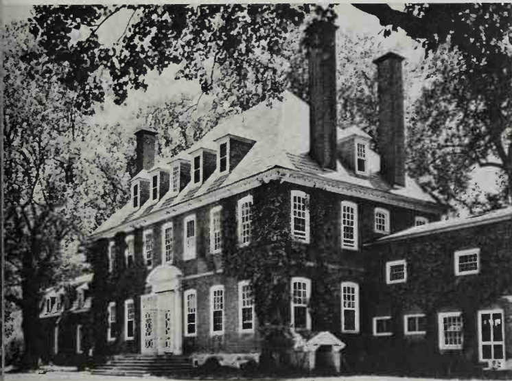
331 Westover (c.1730), by Richard Taliaferro, one of the first known American architects, shows how 'Georgian' was the best architecture of Virginia. The brickwork, the sashes, the dormers and the big chimney stacks are all very English, and of the highest quality. Only the plan – with the entrance hall running through from front to back – marked a new departure
