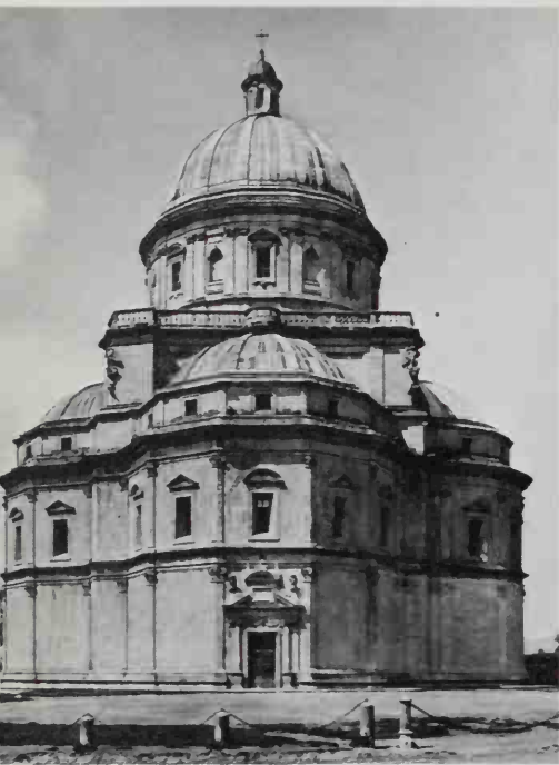
194 Sta Maria della Consolazione, Todi (begun 1508), by Cola da Caprarola: one of the few large central-space churches, built up within a pyramidal outline. Three of the four apses are polygonal; the sanctuary apse – right – is differentiated by being round
