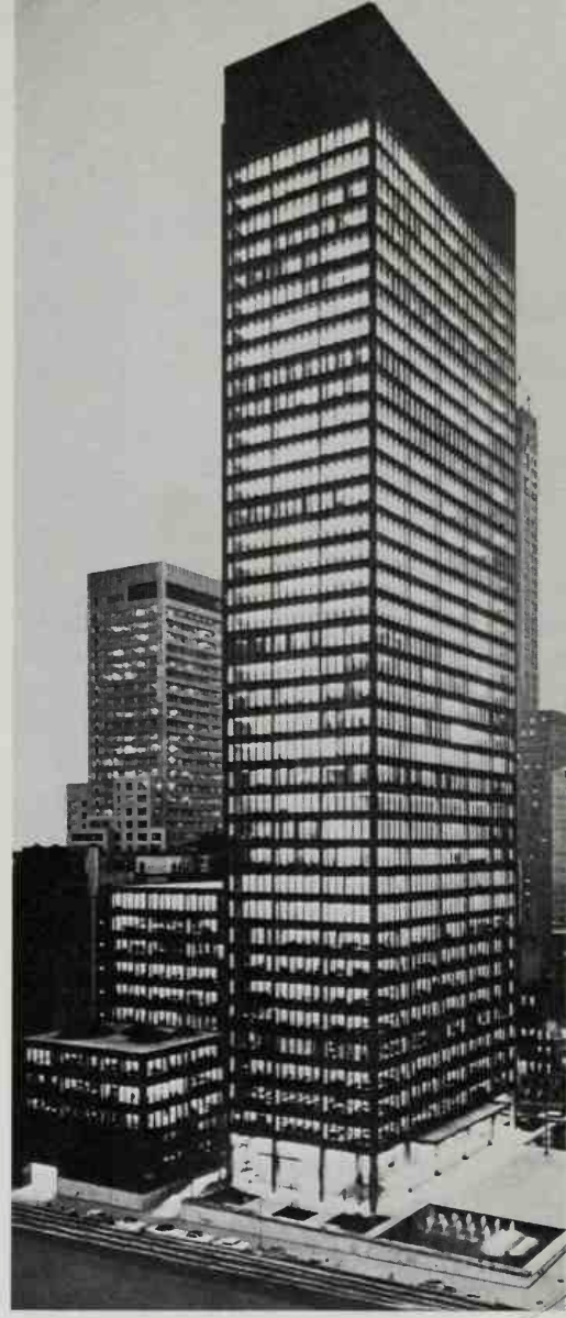
421, 422 Two of Mies van der Rohe's essays in the use of fine steelwork to enclose and outline carefully proportioned and related rectangles. Left, the Bacardi offices in Mexico City (1963): steel liberates interior space. Above, the Seagram Building in New York (designed with Philip Johnson, 1956–8): major and minor vertical divisions subtly articulate a vast surface; at ground level there is no podium, valuable ground being instead given over to an open plaza
