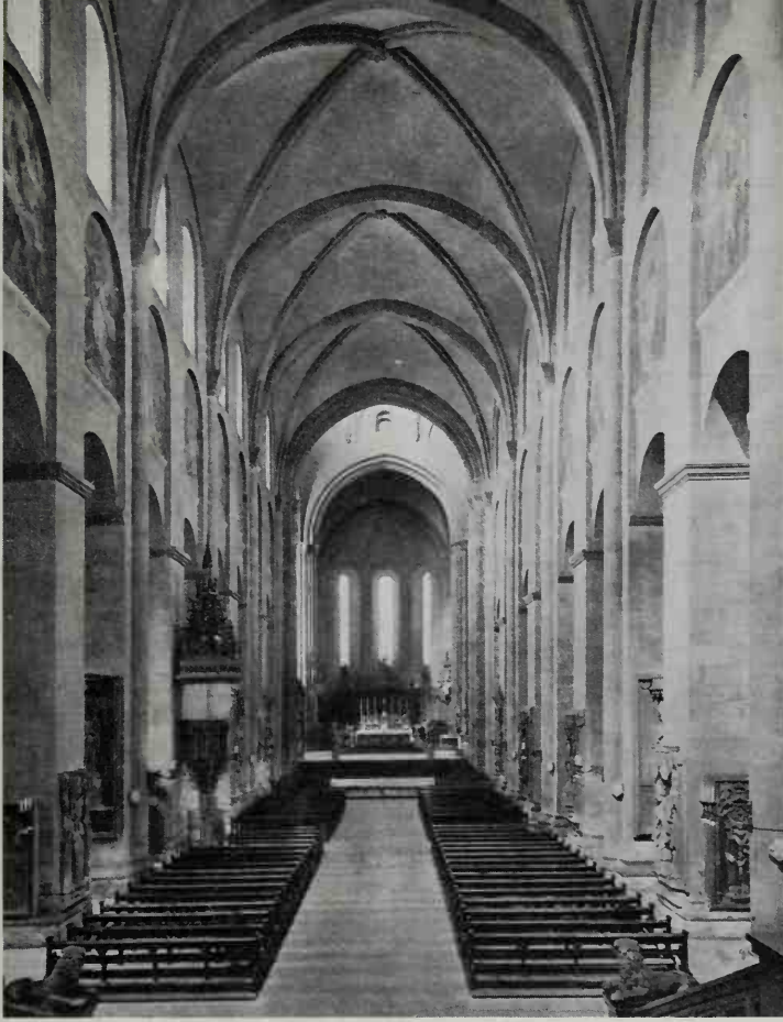
109 Mainz Cathedral (11th century and after 1181). Giant quadripartite vaults cover the nave in a double-bay system (see p. 118). Unlike the Auxerre crypt, there are simple diagonal ribs to mask the groins and to simplify construction
