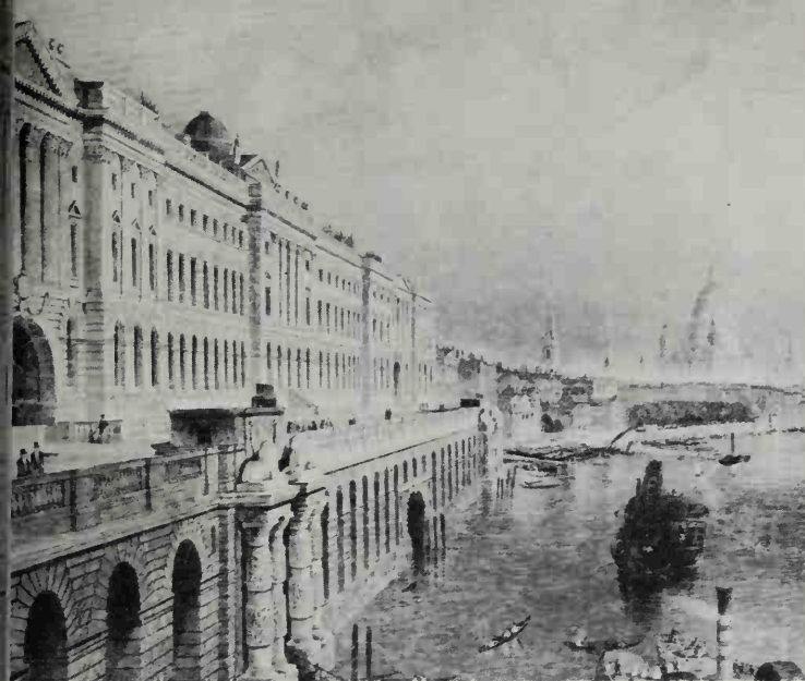
325 William Chambers's Somerset House, London (begun 1776), appears in this 19th-century view as it was originally – the heavily rusticated podium rising directly from the Thames. The long façade is given variety by giant columns and pilasters, and great arched openings in the rusticated ground storey
