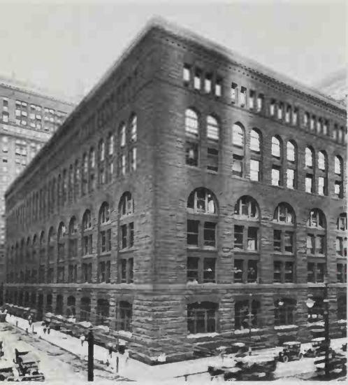
379 Marshall Field Wholesale Store, Chicago (1885–7), by H. H. Richardson: a lesson in grandeur, if not in technique
