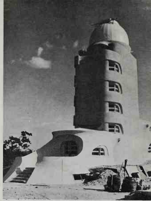
402 Einstein Observatory Tower, Neubabelsberg (1919–21), by Erich Mendelsohn: propaganda for new, mainly streamlined, forms in design rather than a technical achievement in itself
