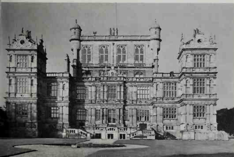
264 Wollaton Hall (finished 1588), by Robert Smythson. Its stylistic features come from an odd assortment of sources – Italian Renaissance, Flemish pattern-books, Gothic and even – in the tourelles – fantastic castle architecture. The plan is extremely novel (while based on Serlio): the hall rises through the centre, lit by a clerestory just above the roof, and is in turn surmounted by a 'great chamber'
