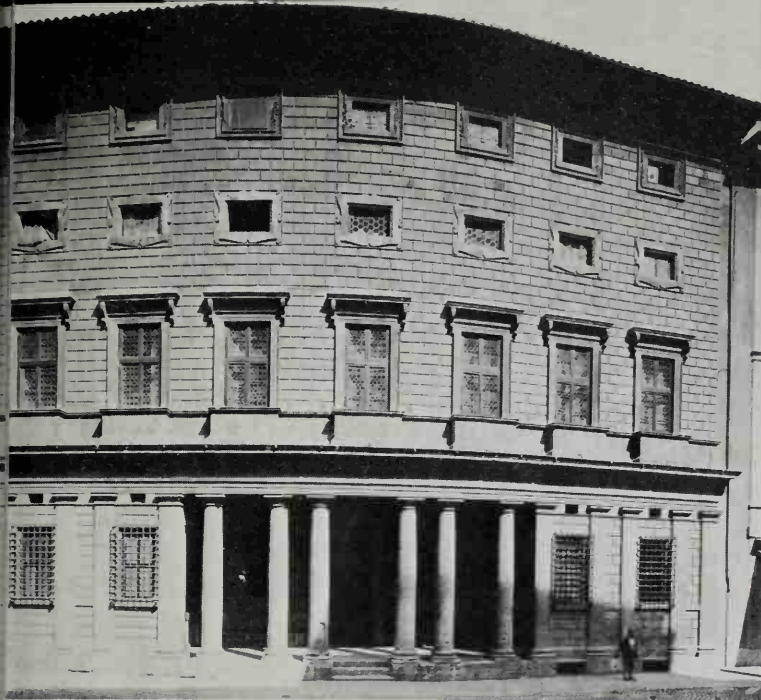
213 Palazzo Massimi alle Colonne, Rome (1535; at the right in Ill. 211), by Peruzzi. Note its individualism, even its eccentricity – e.g. windows framed like pictures, and the use of flat detail and flat rustication – compared with the masculine directness of the Palazzo Farnese, below
