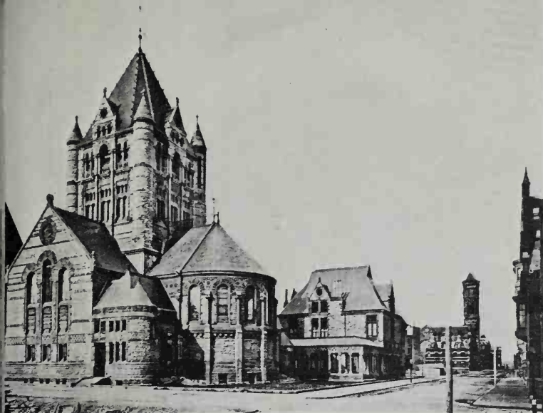
376 Trinity Church, Boston (1873–77), shows H.H. Richardson's rugged style of masonry – here pink granite trimmed with brownstone – and also his ability to control masses, the almost detached blocks building up to the climax of the tower. The inspiration is clearly Romanesque
