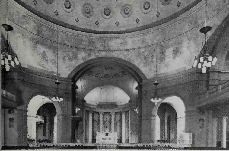
341 Catholic Cathedral, Baltimore (1805-18). Latrobe's grand design is a blend of European precedents: the plan, and perhaps the perspective of the arches, are derived from the Panthéon, while the segmental arches and the treatment of the pendentives come from Soane
