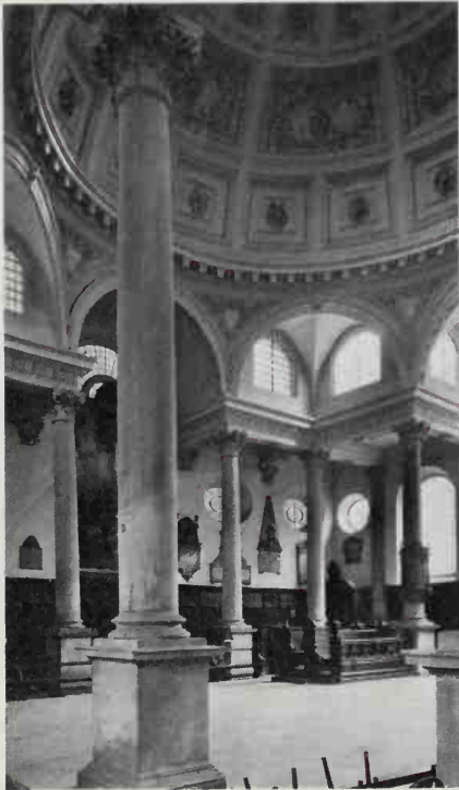
288, 289 St Stephen, Walbrook, London (1672-87), by Sir Christopher Wren, the most complex of the City churches. The plaster dome is carried over an octagon, with a circumambient aisle doubled at the west end, combining the merits of centralized and longitudinal plans. In the view below, we are looking diagonally across the octagon – from lower right to top left in the plan
