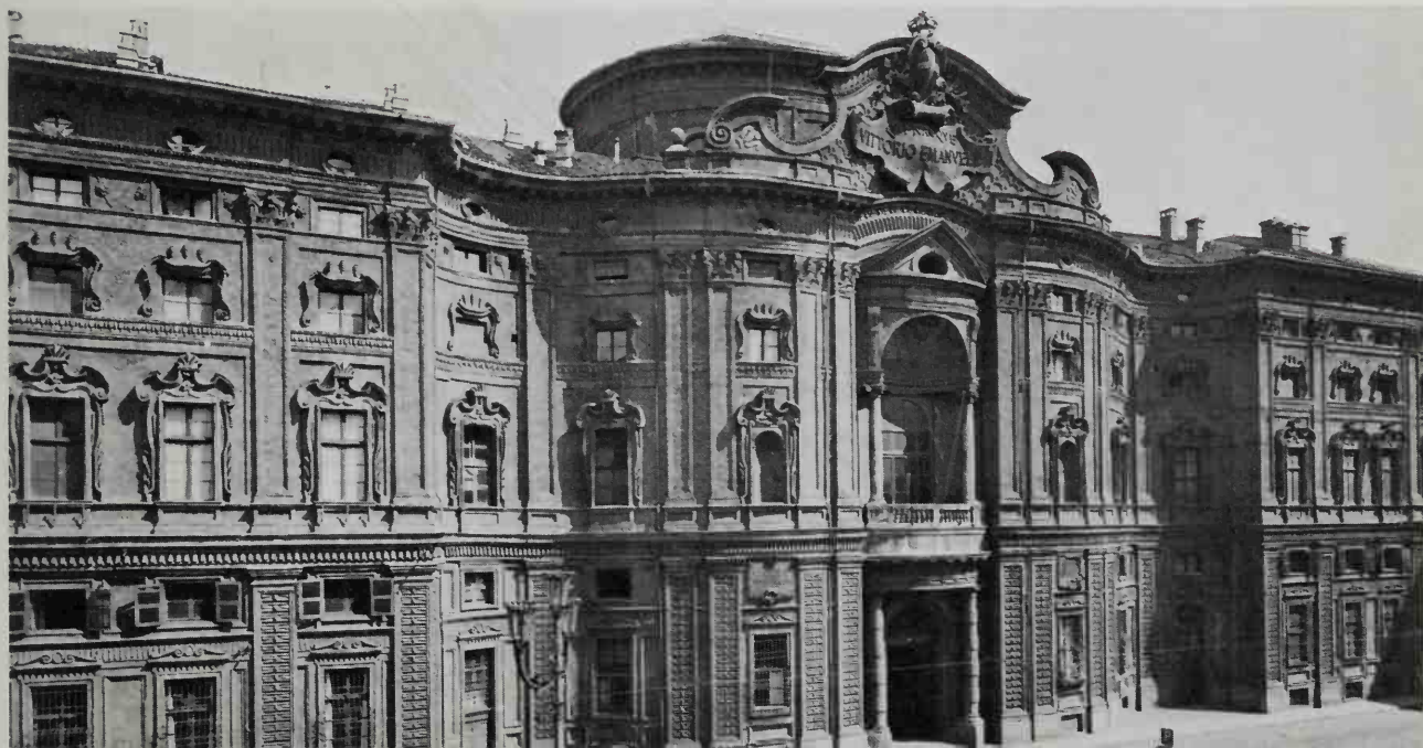
246 Palazzo Carignano, Turin (begun 1678). Guarini gives interest to the long façade by alternating concave and convex sections, in a way which seems to derive from Bernini. The texture and ornament, entirely of brick, is almost Arabic in character
