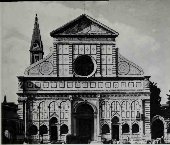
197 Sta Maria Novella, Florence. Alberti completed the façade – of which the lower part is medieval – in 1456. His work is based upon a module, represented by each of the dark squares below the round window. Volutes link nave and aisles (see Ills. 224, 233, 275). The marble veneer used throughout was one of ancient Rome's most persistent cultural legacies
