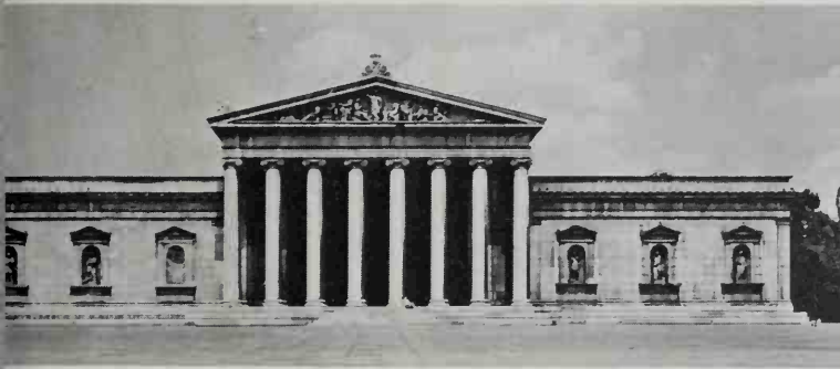
342 Glyptothek, Munich (1815-34). Leo von Klenze was, like Schinkel, an exponent of Romantic Classicism. This building, with central Grecian portico and side walls relieved by Renaissance aedicules – the three parts perhaps too nearly equal in width – was built to house the Duke of Bavaria's magnificent collection of antique sculpture
