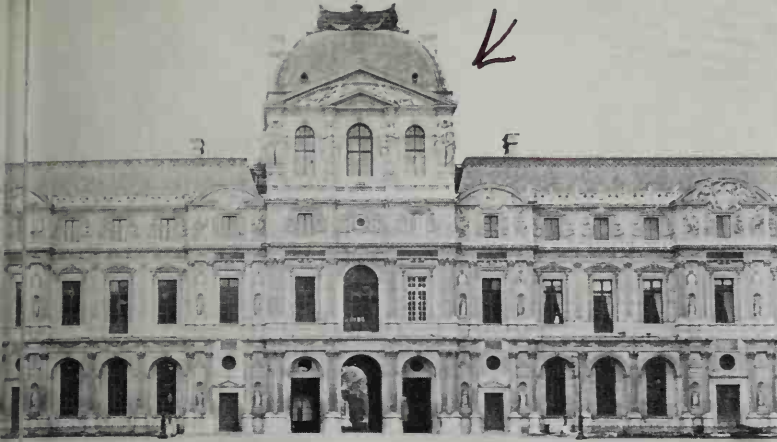
270 Pavillon de l'Horloge in the Louvre, Paris (begun 1624). Lemercier by this accent joined Lescot's wing, on the left (see Ill. 255), with his own replica of it on the right. In the upper part of the pavilion there is a new freedom: note the trebled pediment, 'caryatid order'; and domed pavilion roof
