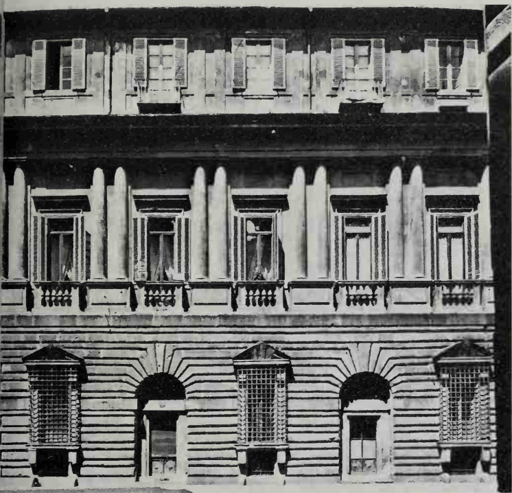
208, 209 The Palazzo Vidoni-Caffarelli in Rome (c.1515), by Raphael, shows the palace design invented by Bramante in the 'House of Raphael': a heavily rusticated ground storey, below a 'piano nobile' with windows set between paired columns. The High Renaissance achievement is clearly seen if one compares this richly sculptural façade with the first palace design to make use of the orders, Alberti's Palazzo Rucellai in Florence (below), of 1446-51
