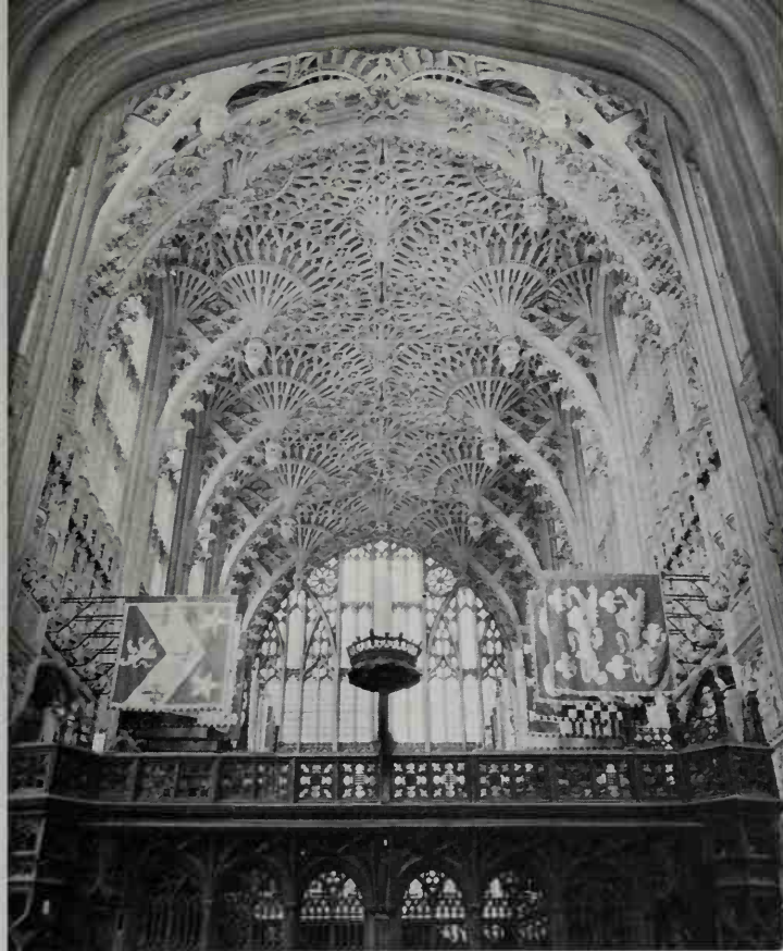
186 Henry VII's Chapel, Westminster Abbey, London (1503-19). This astonishing roof – with its stone pendants apparently hanging from a fan vault – is the last blaze of English Gothic. The handling of masonry could go no further, while the spirit of the building is royal and secular rather than ecclesiastical: it is the end in more senses than one
