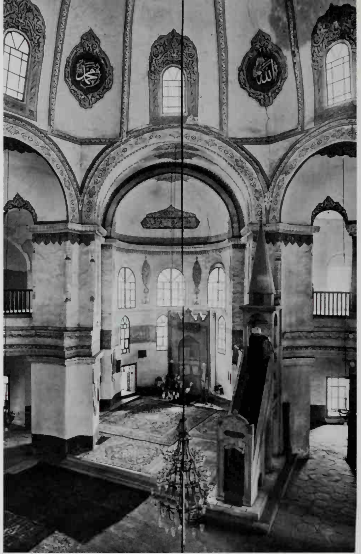
72, 73 Interior and plan of SS. Sergius and Bacchus, Istanbul. This church – slightly earlier than Hagia Sophia – is an octagon surrounded, except on the east side, by a roughly square aisle. The domed central area is only 52 feet across, so that the pendentives bridging the eight corners are quite small. They are true pendentives, nevertheless. The eight spaces between the piers are closed by triplets of arches alternately straight and curved
