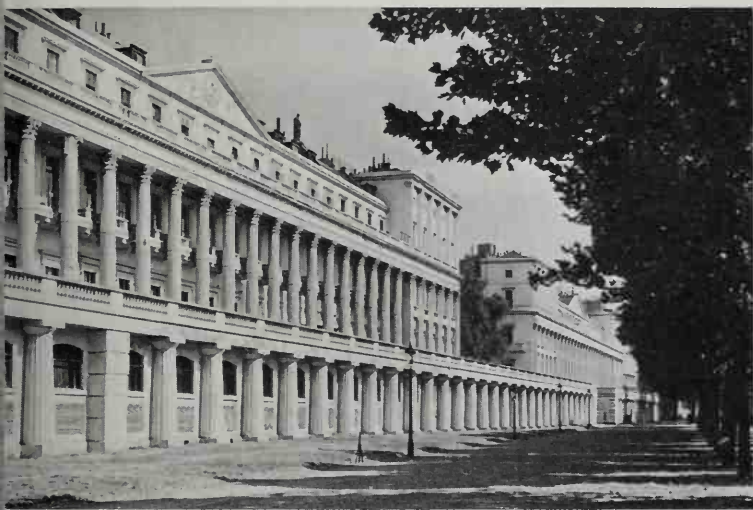
318 Carlton House Terrace, London (1827–33). The culmination of Nash's plan (see p. 269), these two stuccoed white ranges of houses are, like the Rue de Rivoli, a magnificent backcloth to a park. The podium, made necessary by a change in ground level, has Doric columns of cast iron
