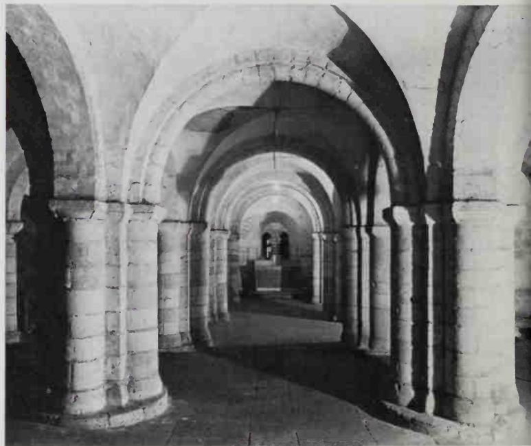
108 Auxerre Cathedral crypt (c.1030): the intersections of the cross vault are left as groins, but each bay is separated from the next by a heavy arch
