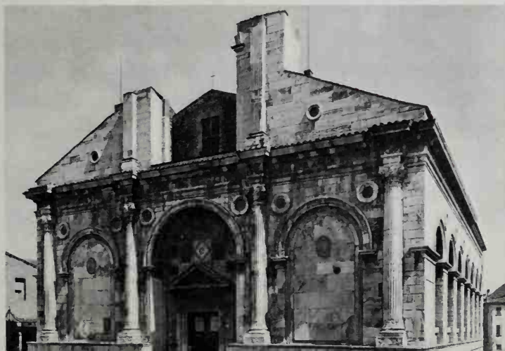
198 Tempio Malatestiano (S. Francesco), Rimini. Alberti began the remodelling – never finished – in 1447. The façade, with its half-columns and flanking arches, is derived from a Roman arch at Rimini. Note the row of deep niches along the side, in the thickness of the encasing stone wall, intended to hold tombs
