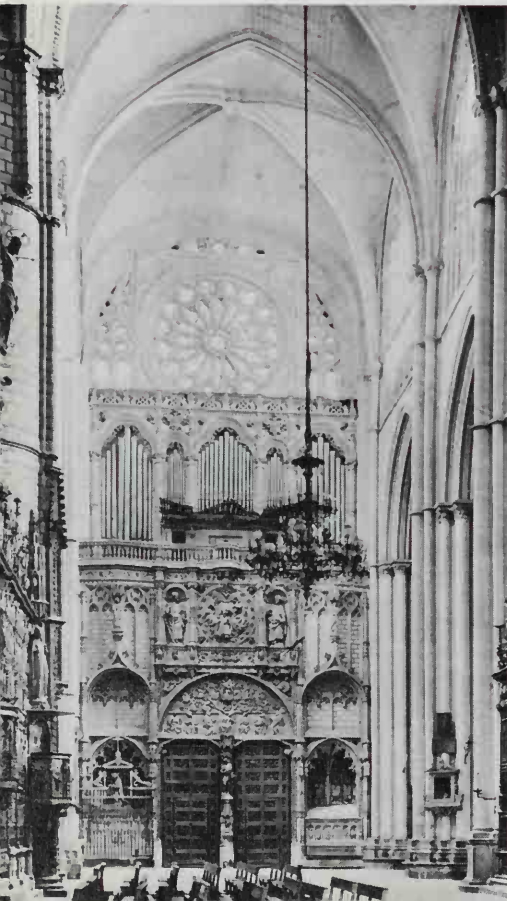
175 Toledo Cathedral (begun 1227), looking across the transept. The style is basically French, though it differs in having only two storeys - arcade and clerestory
