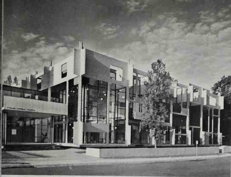
416 Tyrone Guthrie Theatre, Minneapolis (1961-3). Ralph Rapson here tackled the old problem of how, externally, to give unity to the awkward forms of auditorium and stage, solving it with a symphony of slender concrete planes and fins
