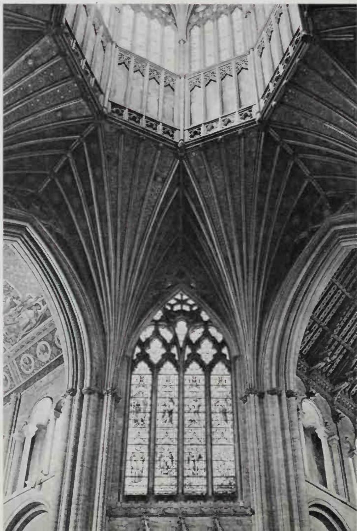
164 Ely Cathedral Octagon (1322-42). From each corner of the crossing – opened out into an octagon – ribs close in to support a central wooden lantern. The placing of windows at a diagonal to the nave-axis is another bold innovation
