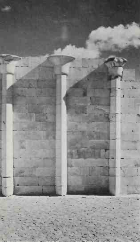
2 Sakkara. Columns in the shape of papyrus – with tulip-shaped flowers and ridged stem – in the north court (h, in Ill. 1); the builders did not yet trust stone enough to make them free-standing. Symbolic of Lower Egypt, the papyrus became a common decorative motif
