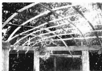
Lattice strips in position.
