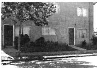
An abrupt entrance—no transition.
