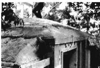
Lightweight concrete on.
