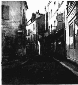
Slight angles in the building fronts.
