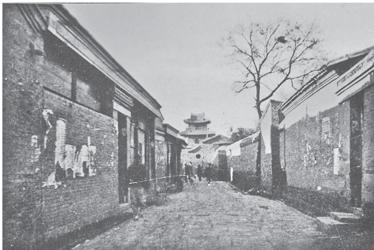
This photograph shows a street in Tianjin, with an old multi-story tower in the distance.
