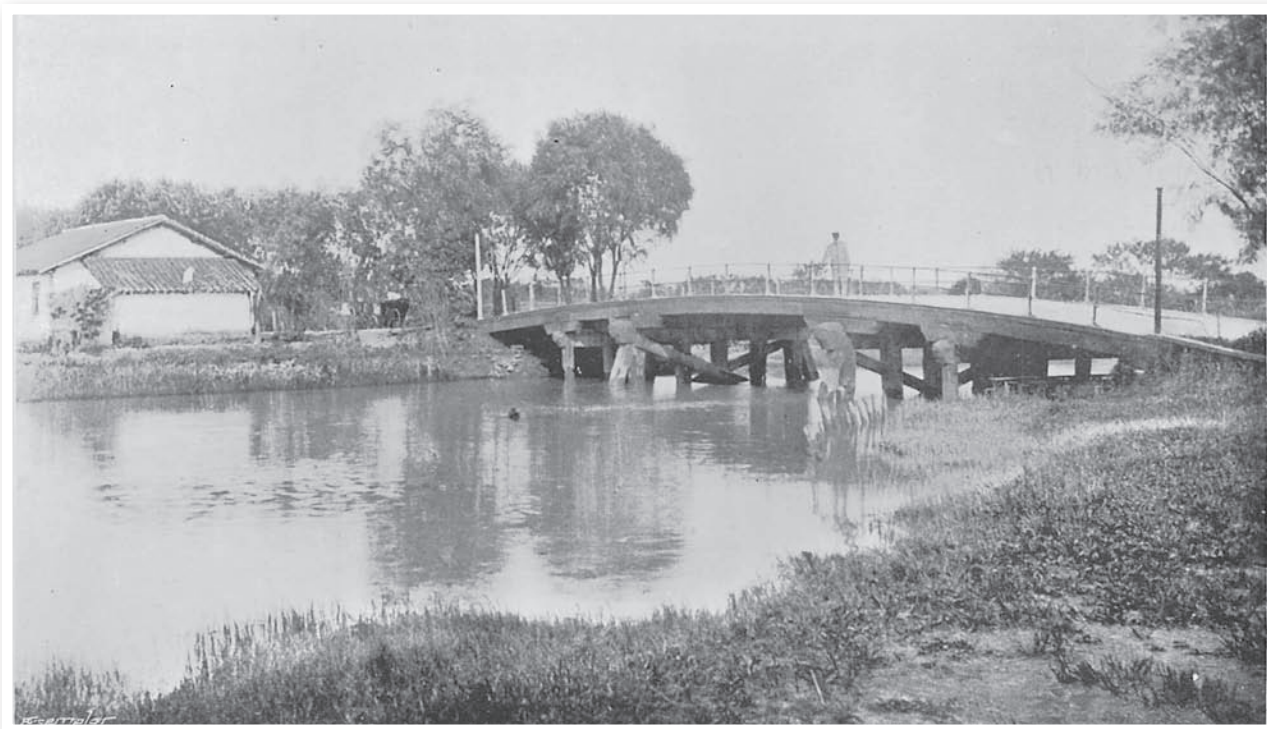
This photograph is a beam bridge of the late Qing Dynasty. It had timber bridge piers, a timber deck, and metal guardrails.
