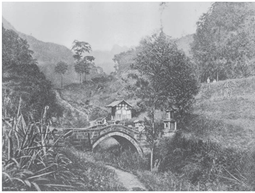
This bridge was built in a valley and was used when the river flooded.
