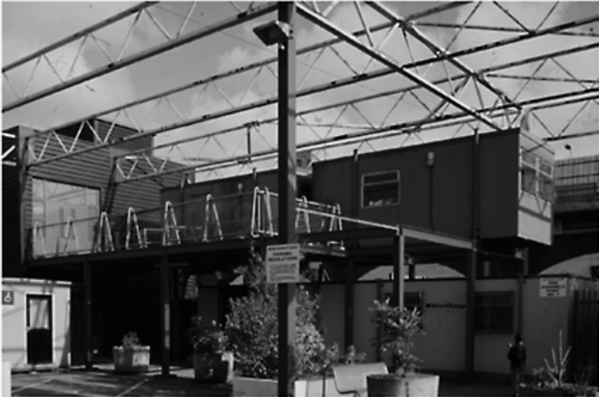
1.2.1 Cedric Price and Ed Berman, Interaction Centre, London, 1977, demolished 2000. Photograph, Adrian Forty.
