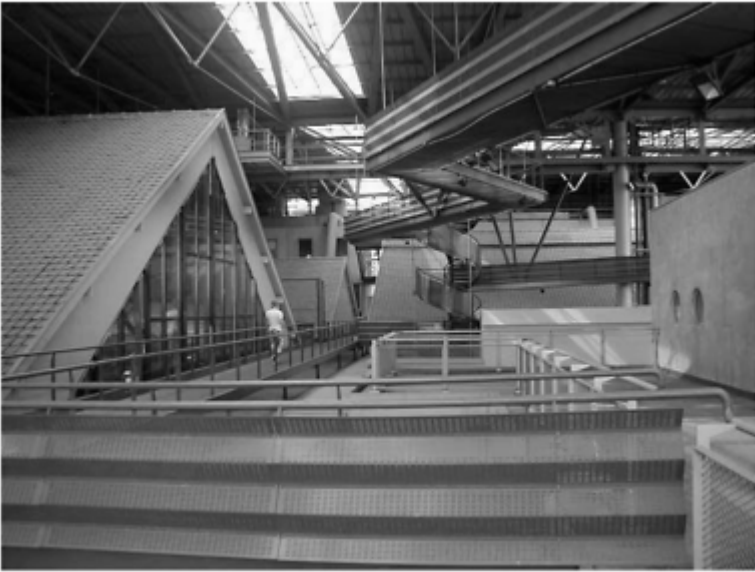
1.3.10 Bernard Tschumi, Le Fresnoy National Studio for Contemporary Arts, Tourcoing, 1997. The space between the new and old roofs. Photograph, Victoria Watson.
