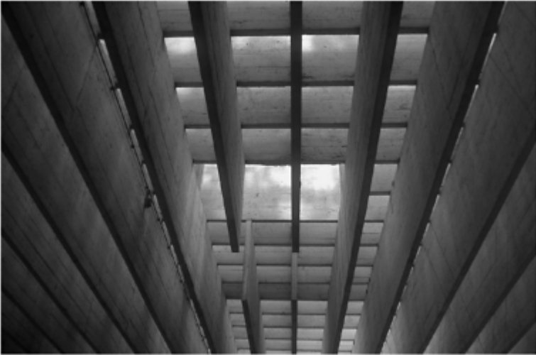
2.2.9 Sverre Fehn, Pavilion of the Nordic Nations, Venice Biennale, 1962. Roof detail. Photograph, Jonathan Hill.
