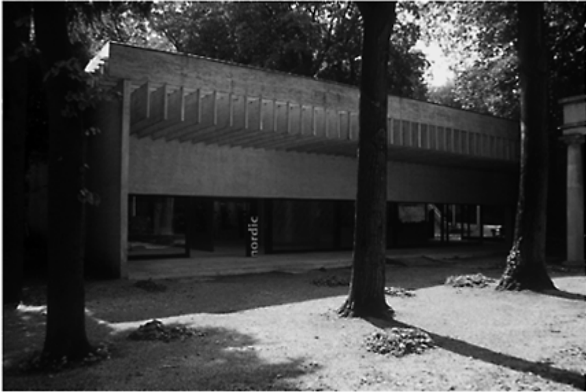
2.2.7 Sverre Fehn, Pavilion of the Nordic Nations, Venice Biennale, 1962. East elevation. Photograph, Jonathan Hill.
