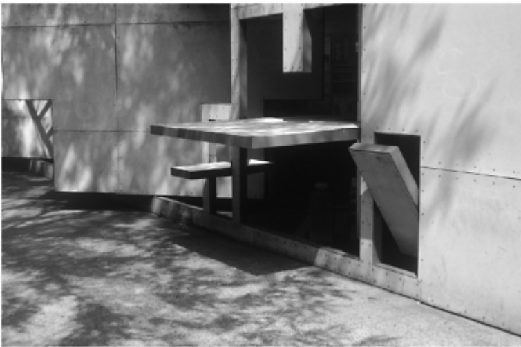
2.8.2 Steven Holl and Vito Acconci, Storefront for Art and Architecture, New York, 1993. Façade open. Photograph, Jonathan Hill.
