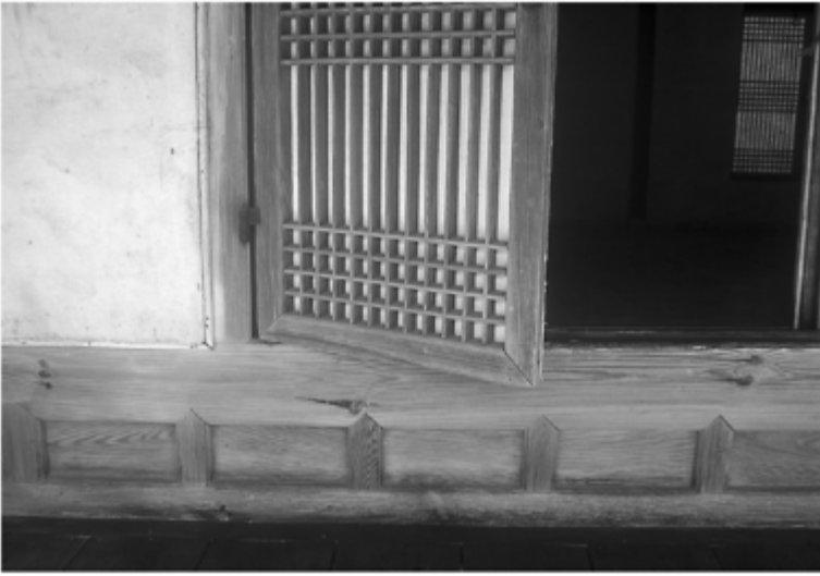
1.2.5 Yangban Class House constructed by King Sunjo, Changdeokgung Palace, Seoul, 1828. Window faced in rice paper. Photograph, Jonathan Hill.
