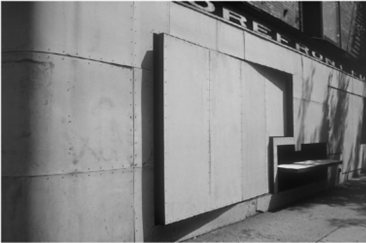
2.8.1 Steven Holl and Vito Acconci, Storefront for Art and Architecture, New York, 1993. Façade open. Photograph, Jonathan Hill.
