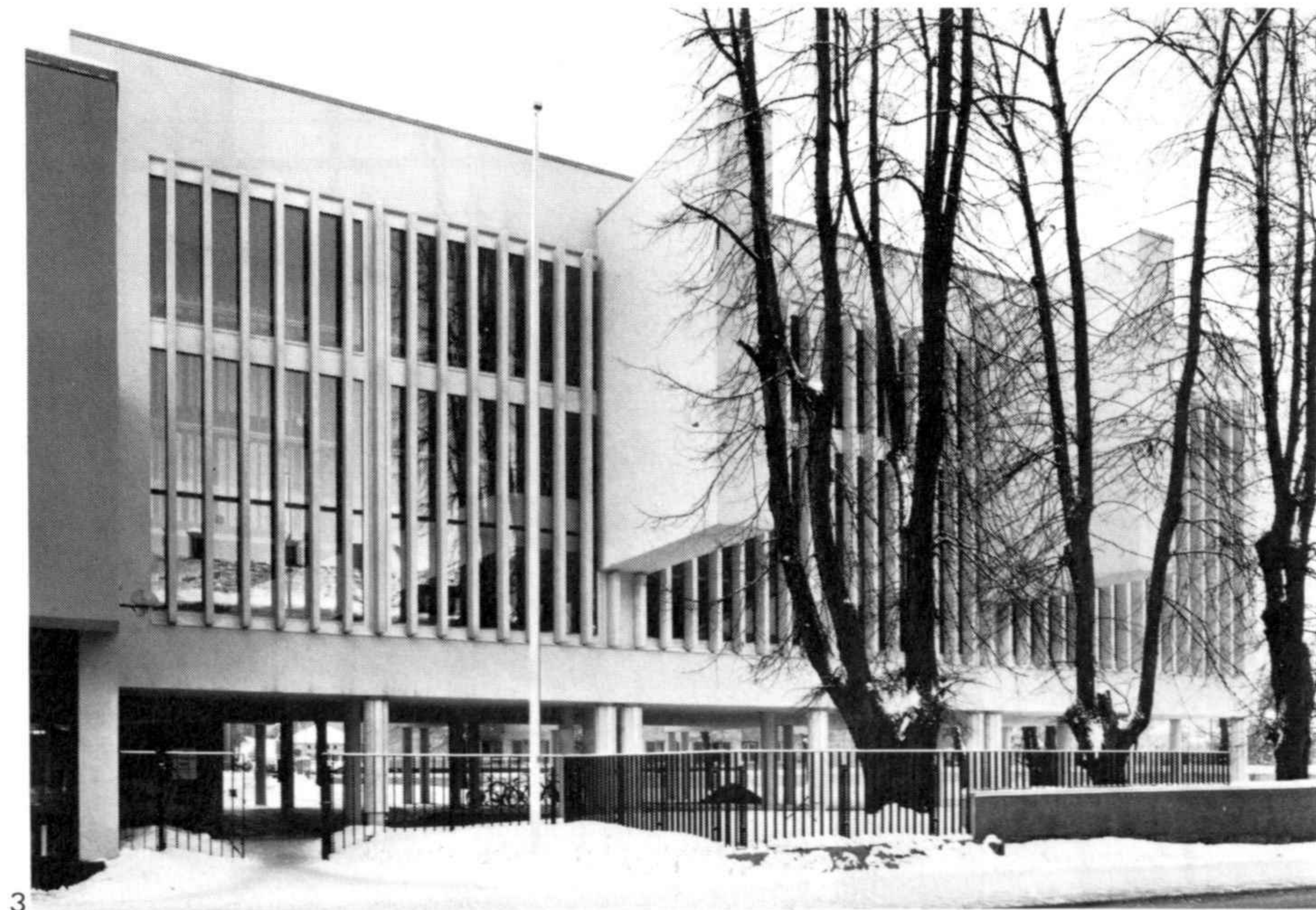
1-2 Exterior views 3 Facade from the street showing the projecting volumes which are used to store the partitions
