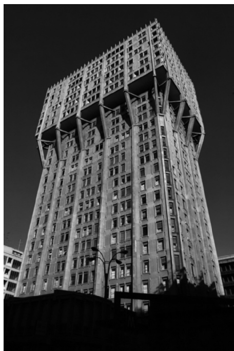
Figure P.1 BBPR, Torre Velasca, Milan (1950–1958). Image courtesy of Davide Secci.
