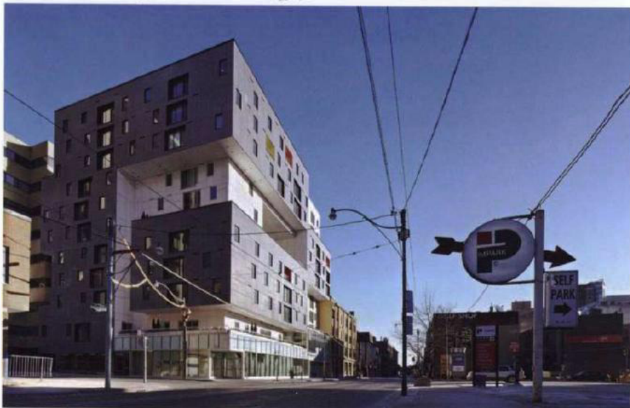
Unlike other residential building types, the entire structure is wrapped in a highly insulated cladding that eliminates all thermal bridging.
