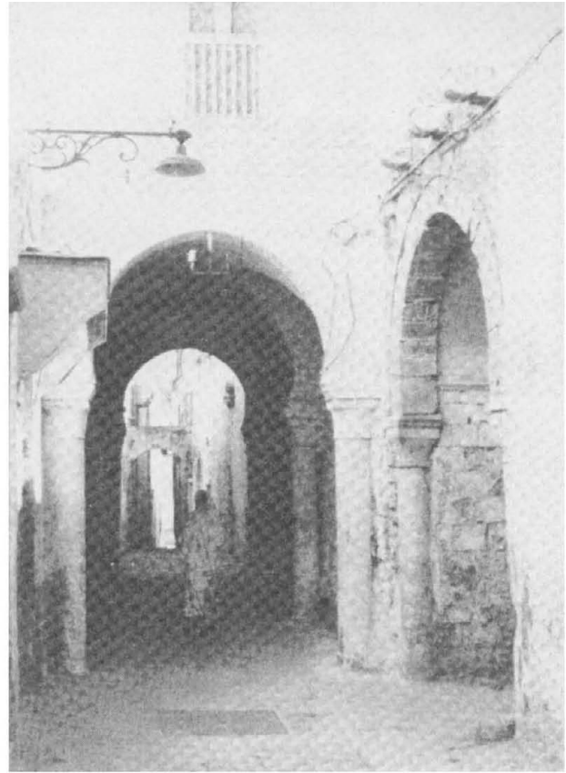
Figure 46 ( above left ) Example of Sabat supported on wall and columns. View in the Rue Tourbet el-Bey, Tunis looking south. Note the Sabat in the foreground and background are supported on the right by columns and on the left by the wall.
