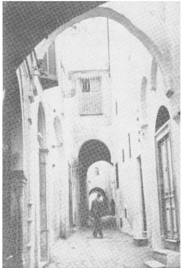
Plate 45 ( right ) Example of a Sabat supported on two walls. View in the Rue du Tresor, Tunis. Note window levels of the ground floor, and the locational relationship of doors on opposite sides of the street.
