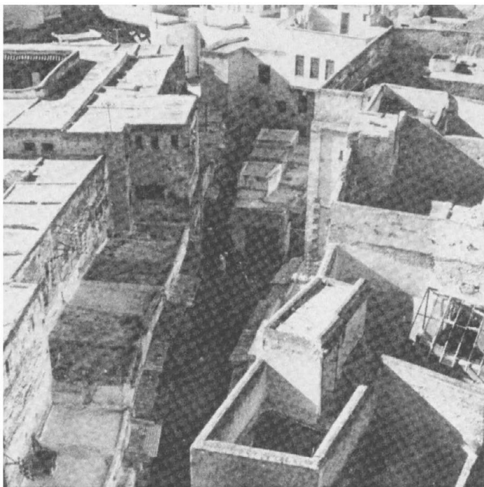
Plate 6 ( left ) Roofs of houses that are actively used must be screened with parapets to prevent overlooking the private domain of neighbours. The photo shows clustered houses on the right with adequately screened roofs. On the left the roofs of a row of shops which will not be used and therefore do not require screening. Location: Fez, Morocco. (Photo: Papini, M.H.A.T., Rabat)
