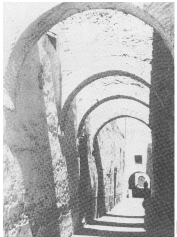
Plate 19 ( right ) Buttressing arches over Rue Ben Othman in Tunis. Note the shadows created, and the location of the Sabat in the background. (Photo from Revault, J., 1971, Palaise et Demeures de Tunis: XVII et XIX siècles , Centre National de la Recherche Scientifique, Paris)
