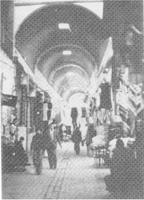
Plate 44 Example of Suq vaulting. (a) ( above left ) Suq et Trouk in Tunis, taken from near the base of the minaret of Zaytuna mosque. Note the brick vaulting system and the sequence of structural ribs. (b) ( above right ) View of the same Suq et Trouk sometime during the period 1881–1930. At that time the coverage system was of wood construction. (Photo provided by Paul Vaughan, Tunis)
