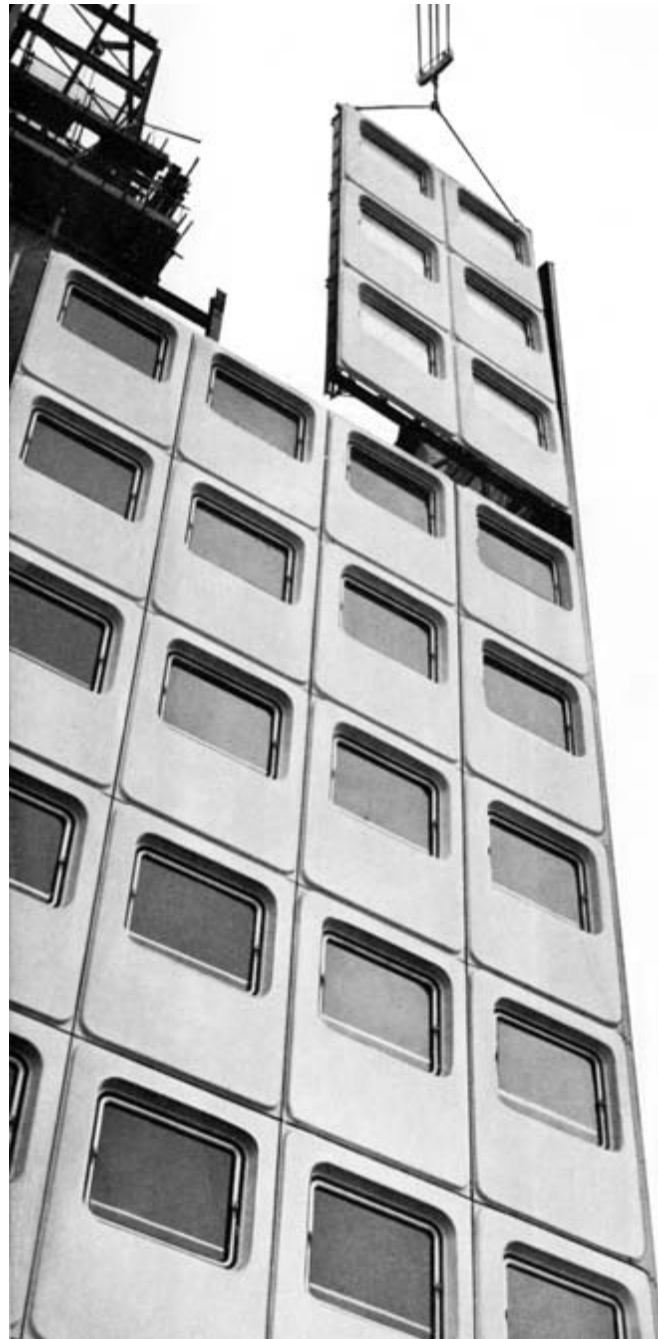
4.46 Greater London Council Architects' Department, section leader J. W. Davidson, SF1 Housing during construction, Elgin Estate, London, 1968: the GLC tried its hand at the "plug-in" plastic units and fiberglass cladding promoted through Archigram by some of its former employees four or five years earlier (and which more distantly recollected experiments such as Harrison and Abramovitz's Alcoa Headquarters, Pittsburgh, 1951–1953). But the techniques were similar to system building, which was quickly diminishing in reputation, and they received little further development within the public sector.
