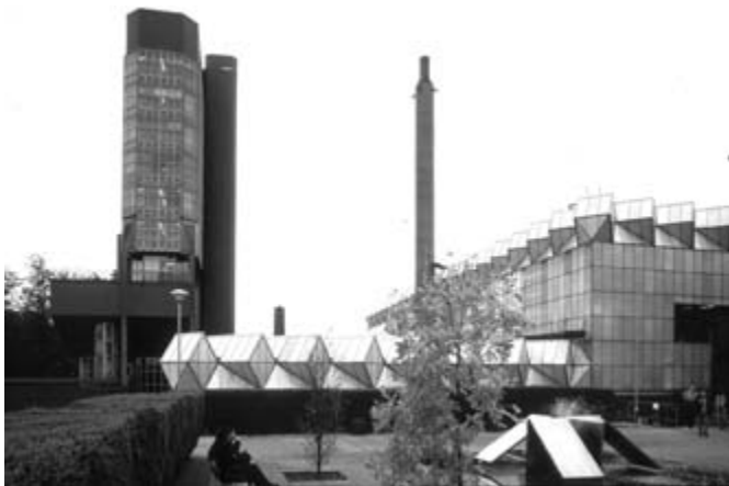
1.13 James Stirling and James Gowan, Engineering Building, Leicester University, 1959–1964 : perhaps the most avant-garde building actually constructed in Britain at the time Archigram was launched, it demonstrated the unabashed pleasures in form to be found in Corbusian, futurist, expressionist, and constructivist sources, ranging from the red-brick tower to the dramatically freestanding stack and the ridge-and-furrow glazing. The work of Stirling and Gowan was numbered among the inspirations for Archigram .
