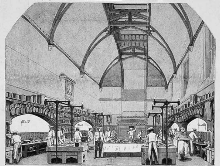
Great kitchen in the upper ward of Windsor Castle c. 1855. The kitchen has been modernised by bricking up the fireplaces at the side leaving only one oven at the far end wall. Gas lighting has been installed over the work stations
