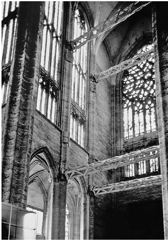
Figure 2-8 The builders of Beauvais Cathedral (a) reached the limits of building in stone in the thirteenth century. A repaired structural failure at the time of the cathedral's construction showed signs of movement in 1988 when structural shoring (b and c) was added to enable modern structural repairs.
