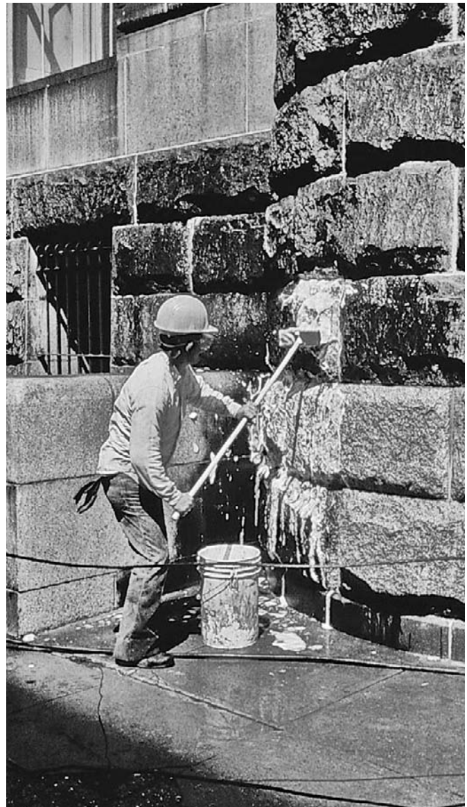
Figure 28-14 Architectural conservator Morgan Phillips repairing an historic window sash in the laboratory of the Northeast Regional Office of the U.S. National Park Service (a). The chemical cleaning of the granite base of the Post Office Building, Washington, DC (b). Images courtesy U.S. National Park Service, Washington, DC.
