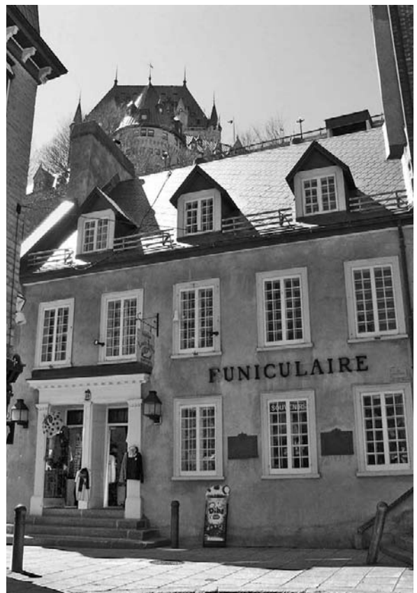
► Figure 29-9 Famed French Canadian explorer Louis Jolliet used this house in Vieux Quebec as a base of operations for exploration of lands to the west. It now serves as the base of the funicular of old Quebec.
