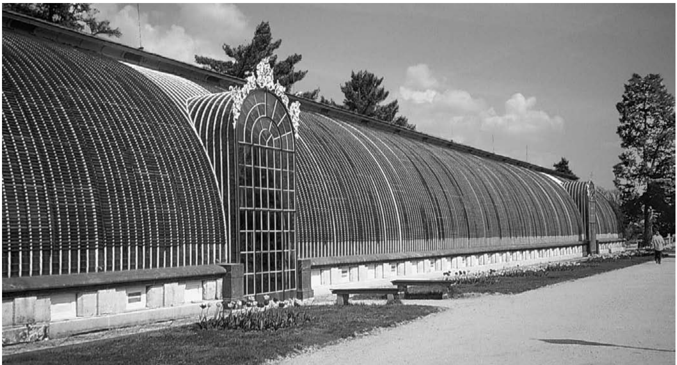
Figure 16-5 The distinctive glass conservatory built by Johannes Lichtenstein in 1850 as an adjoining structure to Lednice Zamek in southern Moravia was restored in 2002 under the direction of Památkový ústav of Brno through a funding partnership between the World Monuments Fund and one of the biggest Czech banks—Československá Obchodní Banka (ČSOB). This was one of several priority conservation projects since the early 1990s at the Lednice-Valtice cultural landscape that derived from two international charrettes (planning sessions) that addressed conservation issues and opportunities ranging in scale from conserving paintings in the baroque chapel at Valtice Zamek to development of the Czech Greenways system that connects this World Heritage List site to several neighboring countries through reactivation of historic road and trail systems.
