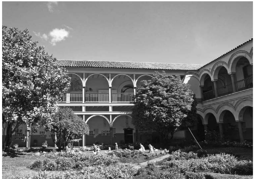
Figure 35-3 Before its replacement in 1997 by the Dirección de Patrimonio (Heritage Directorate) within a new Ministry of Culture, Colcultura played a key role in architectural heritage protection in Columbia for over two decades. The restoration of the Convento de San Agustín in Boyacá (a) was organized by Colcultura in collaboration with the Central Bank's Foundation for the Conservation and Restoration of Colombian Cultural Heritage. The restoration of the convent's courtyard facades includes abstract representations of missing masonry arches in new painted steel (b). Images courtesy Rodolfo Vallin and Jairo H. Mora
