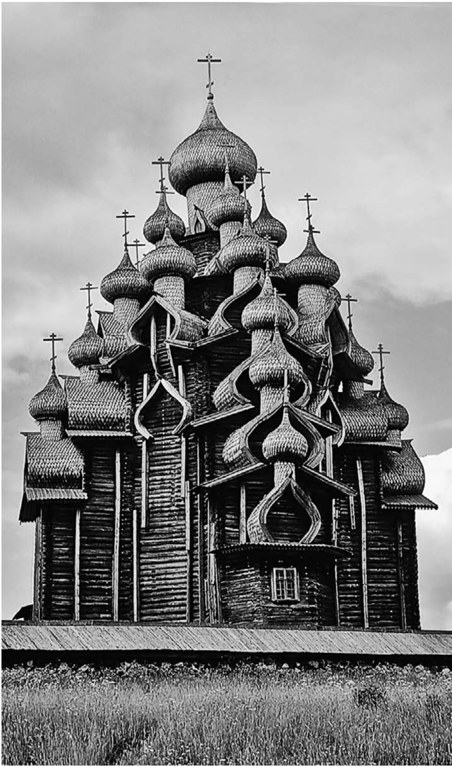
Figure 18-11 After much research and expert consultation, the ingenious solution devised for the restoration of the wooden Church of the Transfiguration at Kizhi Pogost (a) involves the suspension of the church from a metal scaffolding and consolidation of its wooden members from the bottom up. The process requires the installation of temporary structural shoring and new wooden members (b, c, d).
