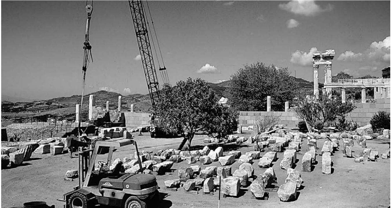
Figure 22-5 Partial reconstruction using the anastylosis method was conducted in 1996 at the Temple of Trajan at Pergamum by the German Archaeological Institute. In 2009 similar stabilization and partial reconstruction of the southern round tower of the Red Hall at Pergamum was completed.
