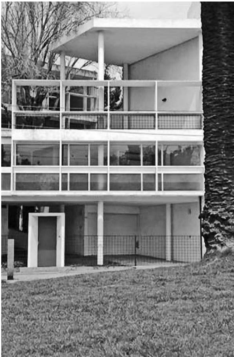
Figure 36-9 Dating from the mid-1950s, the Curutchet House in La Plata, Buenos Aires, was designed by Le Corbusier and is a protected national landmark. It now serves as the headquarters of the Colegio de Arquitectos de la Provincia de Buenos Aires (Architects Association of Buenos Aires Province).
