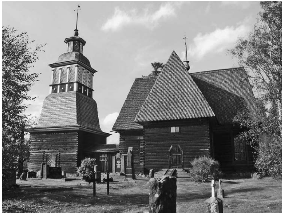
Figure 9-2 The late-eighteenth-century Petäjävesi wooden church in the Finnish lake district, a World Heritage Site since 1994, is a well-preserved example of Lutheran log architecture in Scandinavia. Restoration and conservation of the church has been ongoing since the 1920s and has influenced conservation practice in Finland.
