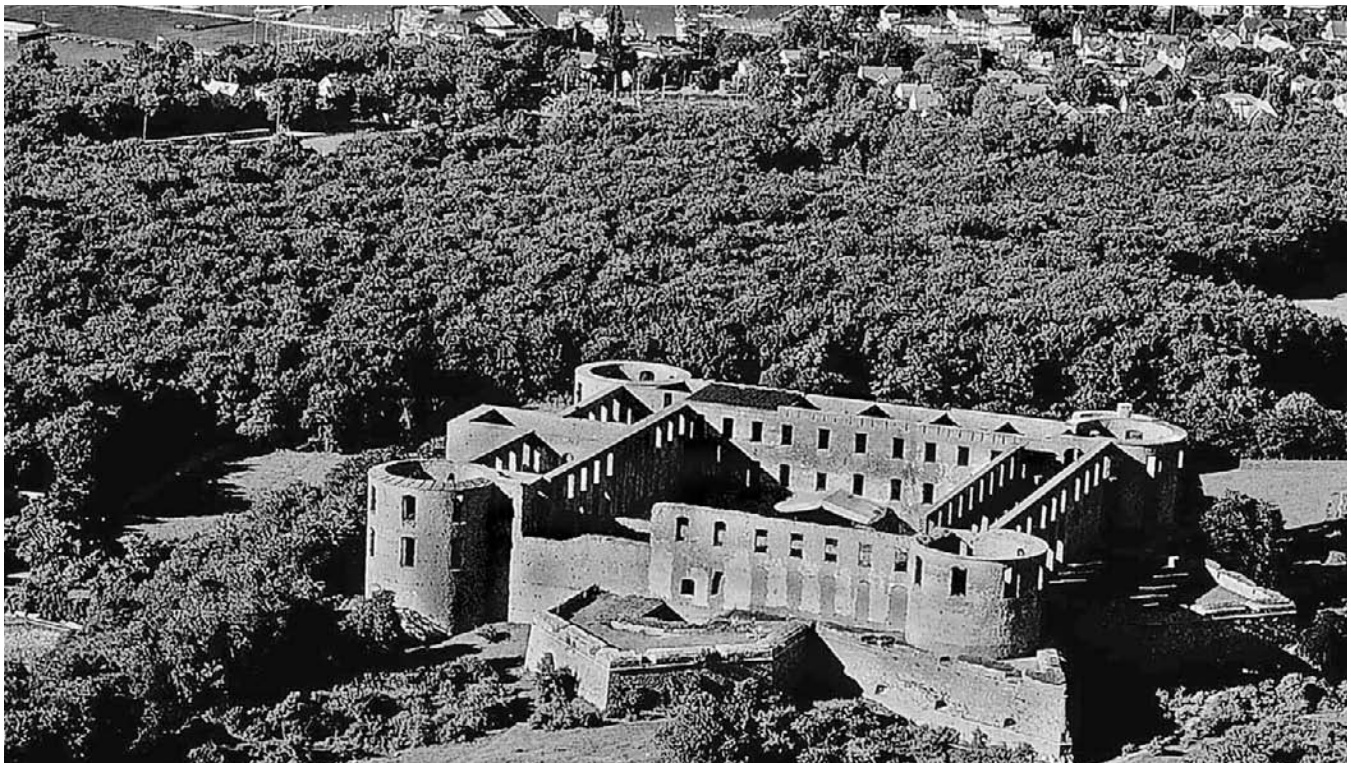
Figure 8-7 Under the direction of the Statens Fastighetsverk (National Property Board), structural stabilization work at the ruin of the baroque Borgholm Castle (a, b, and c) in 1996 included re-creation of a lime production process similar to the originally used process. The hydraulic lime that was produced enabled modern restorers to correct damage done by earlier restoration work, which used cement mortar. A traditional lime kiln (d and e) was specially constructed and limestone pieces were transformed into powder form. High-quality hydraulic lime was a key constituent in formation of structurally and visually compatible repair mortars used in masonry conservation at the site. Images courtesy of Mark Weber.
