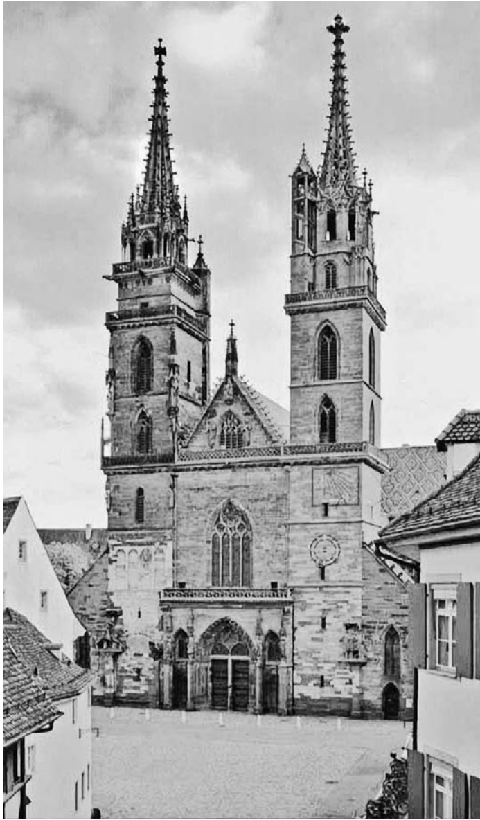
Figure 7-1 Conservation of the deteriorated sandstone facades of the Basel Münster (a and b) has been a multiyear project conducted by the Institut für Denkmalpflege (Institute of Monument Conservation) of the Swiss Federal Institute for Technology in Zurich. Conservation work has entailed a range of interventions from cleaning and in situ consolidation, as required, to replicating (c) severely deteriorated or missing elements with physically and visually compatible new composite stone. Figure 7-1a courtesy of Basler Denkmalpflege, © 2006 Erik Schmidt. Figures 7-1b and 7-1c courtesy and copyright of Basel Münster construction hut 2009.
