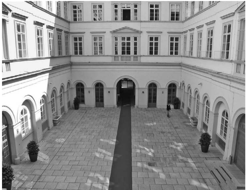
Figure 14-5 Various historic interiors in the former Niederösterreichisches Landhaus (State House of the Federal Province of Lower Austria), with elements dating to 1513, were sensitively restored by architect Gerhard Lindner for use by the Governor of Vienna and the Federal Minister of European and International Affairs. Other parts of the complex became conference facilities. Completed in 2005, the work was supervised by the Bundesdenkmalamt assisted by specialty conservation consultants.
