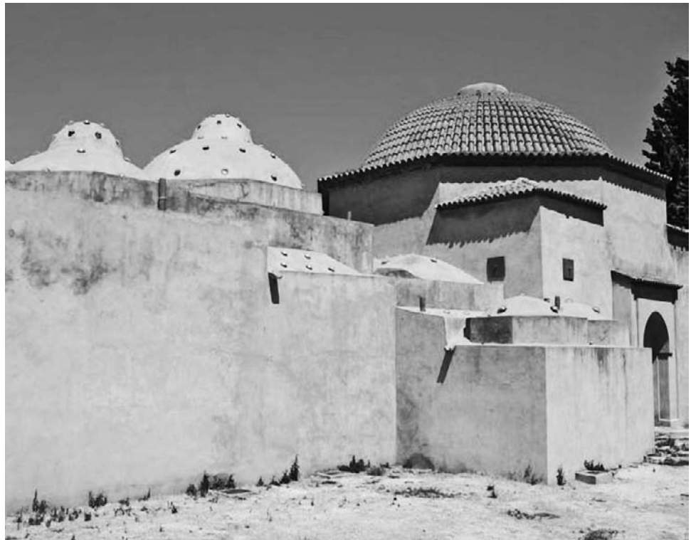
Figure 21-5 The Turkish hammam in Mytilene, Lesvos, was restored in 2004–5 by the 14th Ephorate of Byzantine and Post Byzantine Antiquities (a Greek government official) and was converted into a gallery for art exhibits. The mottled look of the facade comes from the use in the restoration of a lime wash instead of paint. In the past two decades, there has been an increase in the number restorations of such buildings representing the heritage of former foreign rulers and current minority ethnic groups in modern Greece. Courtesy Pamela Jerome.
