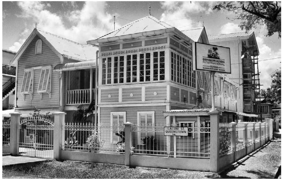
Figure 33-3 Urban conservation in Georgetown, Guyana, has entailed the full range of interventions from rehabilitations and adaptive use—such as a former residence restored and transformed into an office for an international NGO (a)—to complete restoration and reconstruction of key structures, such as the completely rebuilt neo-Renaissance Church of the Sacred Heart (b), which had been destroyed by a fire in 2004.
