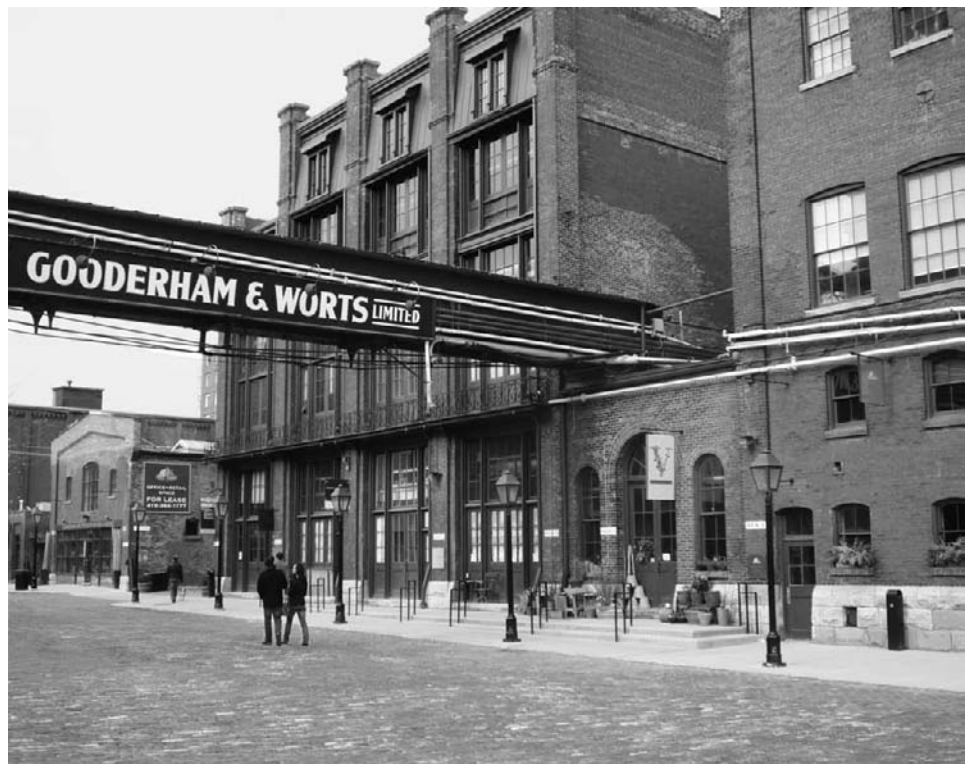
Figure 29-17 The Distillery District in Toronto, once the largest whiskey producing site in the British empire, is now the largest collection of preserved Victorian-era industrial buildings in North America, accommodating artists' studios, theatres, new housing, and public activities to suit tourists and local inhabitants alike.
