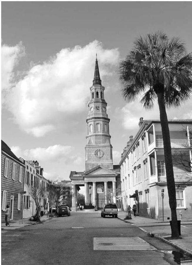
Figure 28-7 Enhancements of an existing city ordinance in 1931 in Charleston, South Carolina, to protect a twenty-three block area known as the Old and Historic Charleston district, entailed the creation of America's first official historic district. Some of the city ordinance's provisions, such as the creation of an architectural board of review, likely represent "firsts" in architectural conservation practice in the world.
