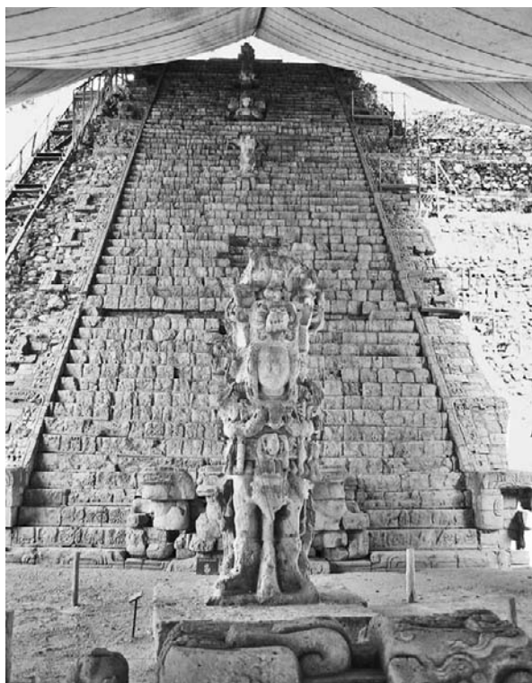
Figure 32–12 Development of a new conservation plan in 2001 for the conservation and presentation of Copán, Honduras, was a process that involved national and foreign experts and local stakeholders and resulted in the present effective program to preserve and display the Copán historic site in a sustainable way.
