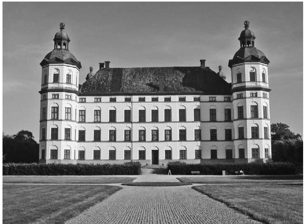
Figure 8-4 Restoration of Skokloster Castle in the region north of Stockholm using traditional materials in the 1970s marked a turning point in the country's approach to the restoration of significant historic buildings. The techniques used by the chief architect, Ove Hidemark, including employing traditional materials and restoration methods, are considered a best practice in Sweden today.
