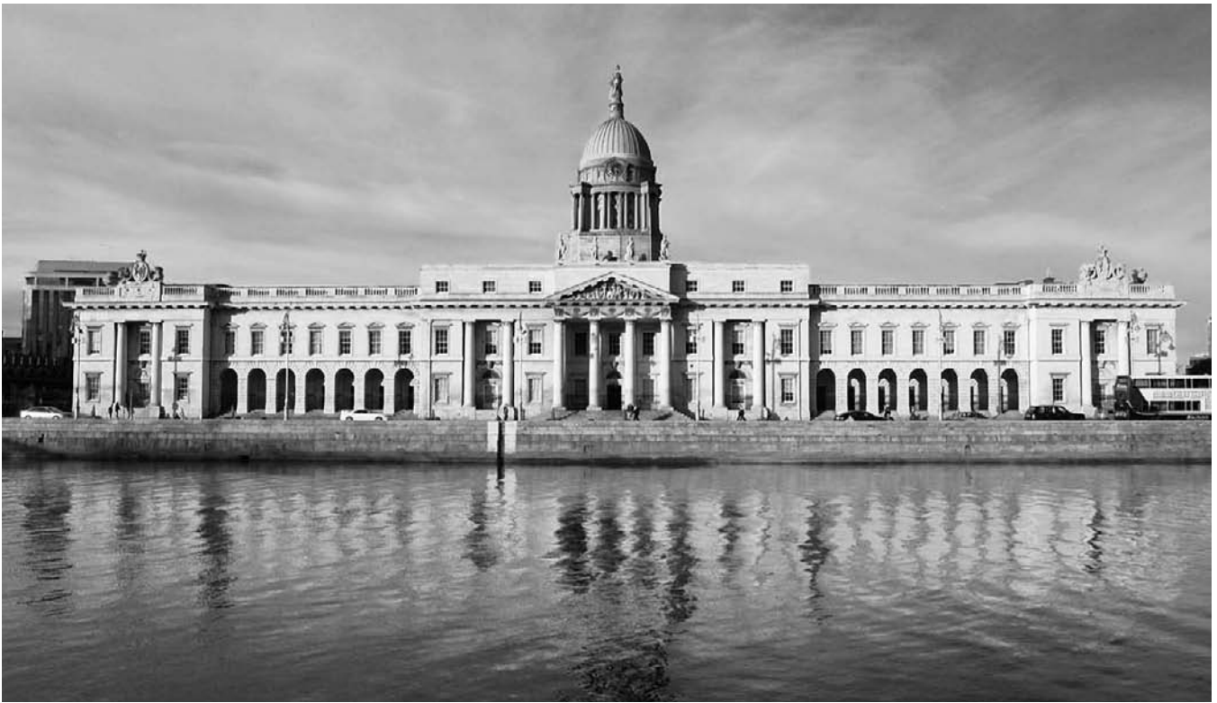
Figure 4-4 The neoclassical Custom House (James Gandon, 1791) situated on the River Liffey in Dublin was extensively damaged by fire in 1921 but restored under the direction of the Office of Public Works in the 1980s. The restoration entailed complete reconstruction of the interiors, including its collapsed dome, and two campaigns of exterior stone restoration work. The building that currently houses the Department of the Environment, Heritage and Local Government, exemplifies Irish government support for architectural conservation from the 1980s forward.
