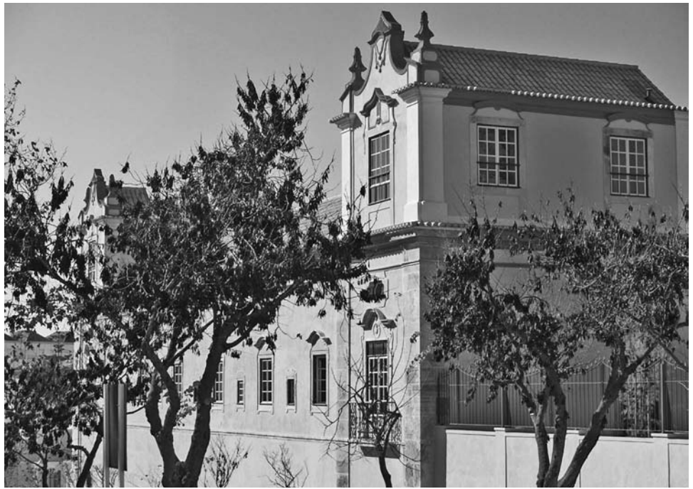
Figure 5-2 The Pousada Tavira Convento de Senora Graça in Portugal is representative of one of the Iberian Peninsula's major contributions to architectural conservation and the history of tourism: reuse of redundant castles, monasteries, and palaces through their conversion to hotels and guest facilities. The creation of paradores in Spain since the 1930s derived from the country's needs for a national quality hotel system.
