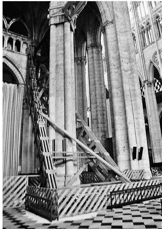
Figure 2-8 The builders of Beauvais Cathedral (a) reached the limits of building in stone in the thirteenth century. A repaired structural failure at the time of the cathedral's construction showed signs of movement in 1988 when structural shoring (b and c) was added to enable modern structural repairs.
