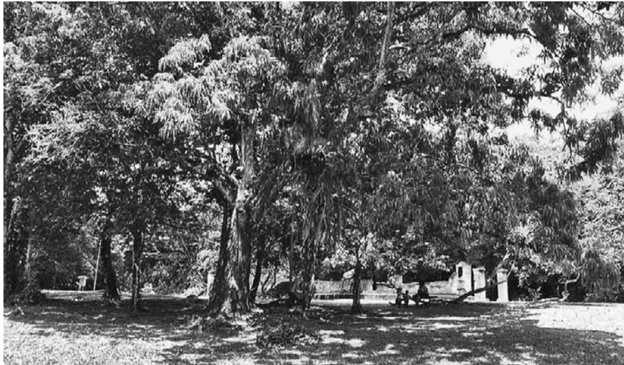
Figure 33-6 Conservation of the seventeenth-century brick remains of the Beracha Ve Shalom synagogue in Jodensavanne (a), Suriname, founded by Sephardic Jews, has garnered interest and support from international organizations including the World Monuments Fund. Since 2008 the Jodensavanne synagogue remains and landscape features of the site have been maintained (b) and aided by an interpretive program (c). Images courtesy WMF and Rachel Frankel, Architect, on behalf of Jodensavanne Foundation.
