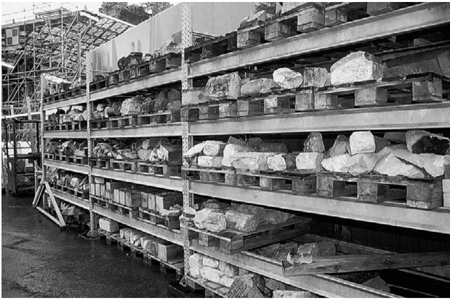
Figure 13-9 Salvaged, catalogued, and temporarily stored original stone (a) from the destroyed Frauenkirche in Dresden in November 1996 awaiting reinstatement in their original positions in the reconstructed building. A new cross and orb (b) designed by English sculptor Alan Smith, son of one of the British aerial bombers of Dresden, symbolizes reconciliation and was displayed on site before its erection as the pinnacle of the reconstructed dome of the Frauenkirche.
