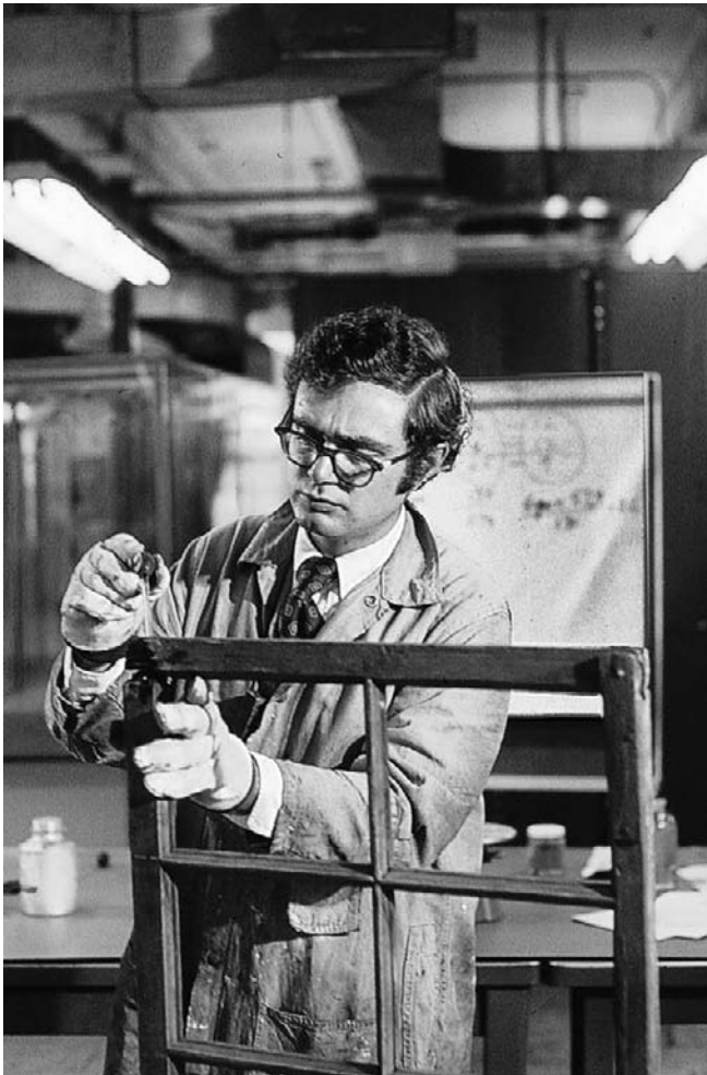
Figure 28-14 Architectural conservator Morgan Phillips repairing an historic window sash in the laboratory of the Northeast Regional Office of the U.S. National Park Service (a). The chemical cleaning of the granite base of the Post Office Building, Washington, DC (b). Images courtesy U.S. National Park Service, Washington, DC.
