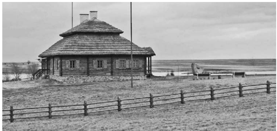
Figure 19-5 The boyhood home of Thaddeus Kosciuszko, a Belarusian native who fought in the American Revolution, was restored with aid from the U.S. Ambassador's Fund, showing the reach of innovative funding in international architectural conservation.
