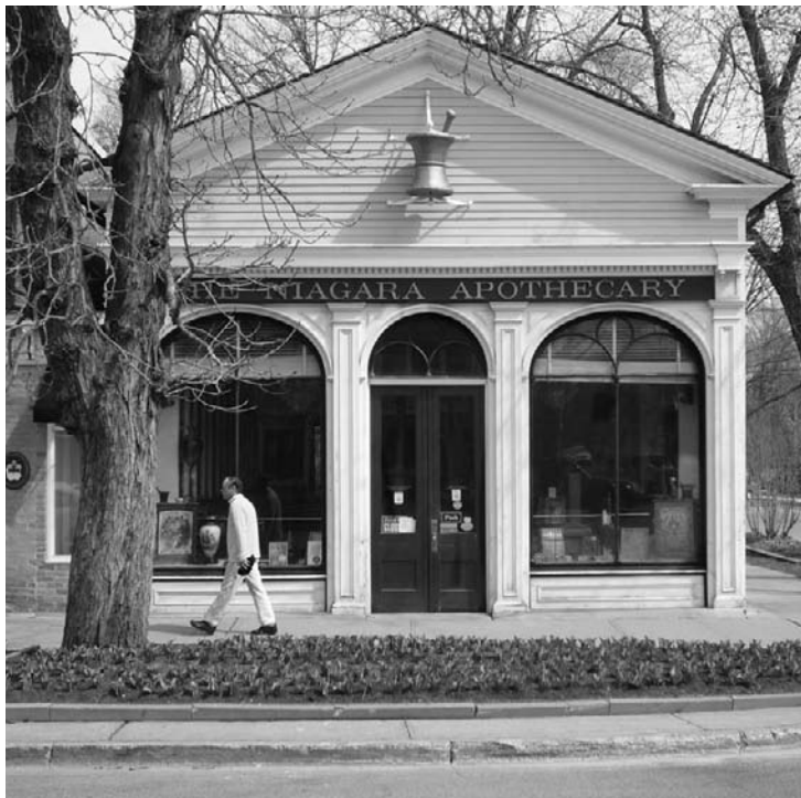
◄ Figure 29-10 The Apothecary at Niagara-on-the-Lake, circa 1820, was exactly restored to its 1869 appearance, with advice from local architect P. J. Stokes and support from the Ontario Heritage Foundation. The restoration, begun as a Centennial Project in 1967, involved approaches that set a new model for conservation practitioners in Canada. Photo Barbara Ross.
