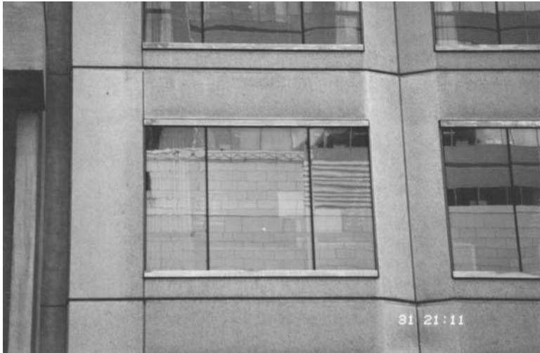
2.5 Typical punched window glazing system.
