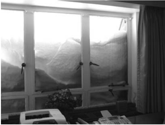
4.1 Avoid locating glazing assemblies in areas subject to sliding snow and ice.
