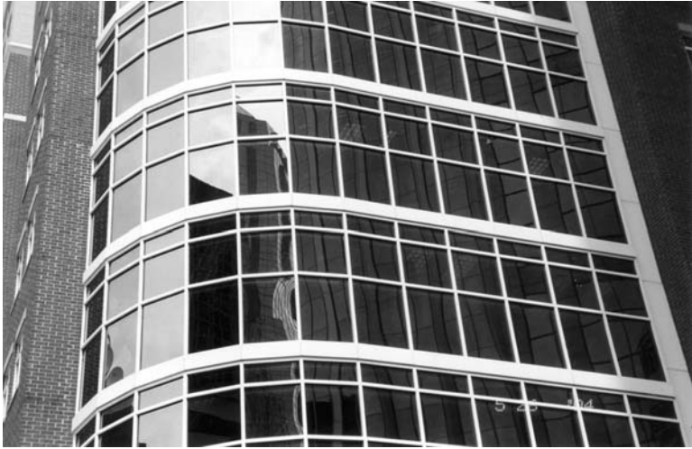
2.3 Typical dry-glazed curtain wall system.
