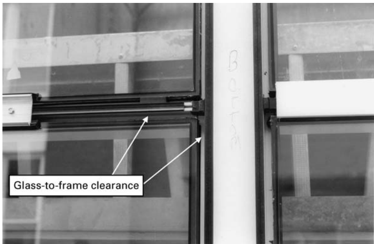
2.8 Typical glass-to-frame clearance.
