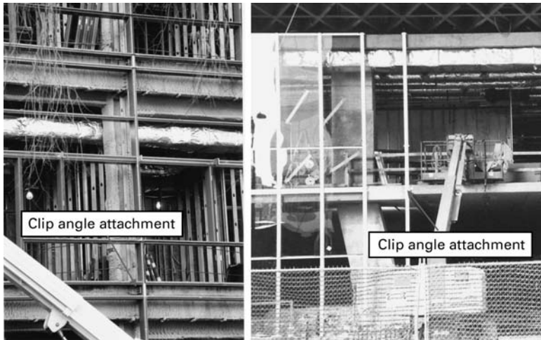
2.7 Typical attachment through clip angles of mullions to steel frame and concrete floor over two adjacent stories.
