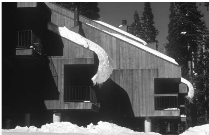
3.18 Snow/ice curl at eaves of sloped metal standing seam warm roof (Matrix IMA Archive photograph).
