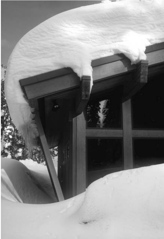
3.19 Snow/ice curl effects mitigated with sufficient cold roof overhang and bracing (Matrix IMA Archive photograph).
