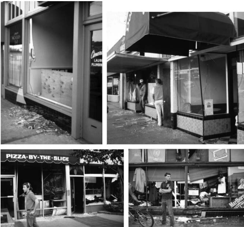
2.12 Glass breakage in several storefronts during Loma Prieta (magnitude 6.9) Earthquake of October 17, 1989 ( armory.com/~images/?s=quake89 ).
