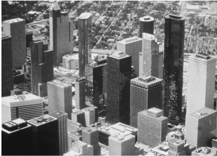
5.1 Damage to glass windows in Houston, Texas, resulting from Hurricane Alicia in 1983 (courtesy of WISE, Texas Tech University).
