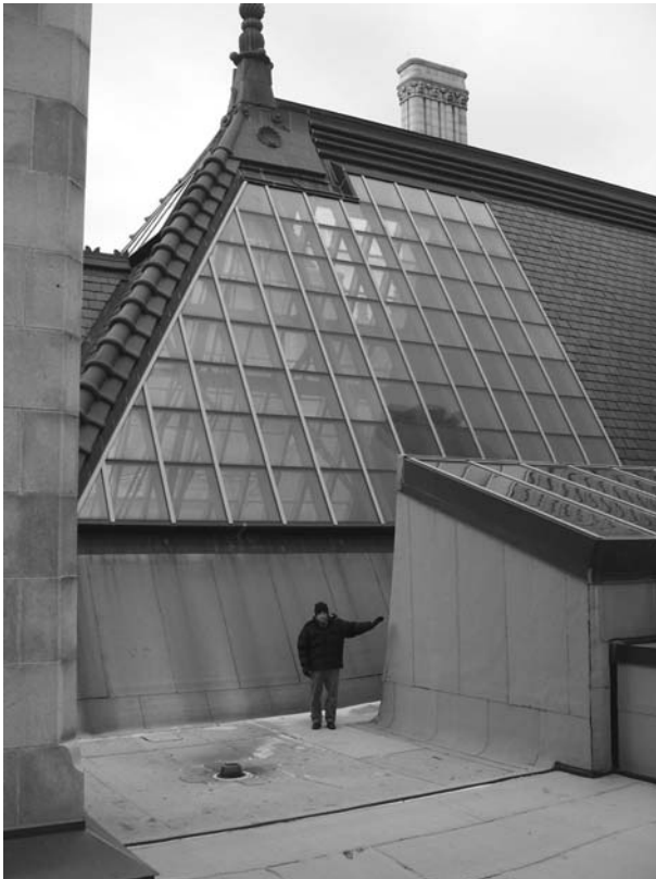
4.3 Rainfall on a snow blanket may cause water to pond against glazing unless waterproofing height is sufficiently high.
