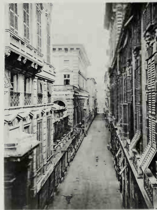
Above: The balanced ensemble of palaces reflects Renaissance love of symmetry.
