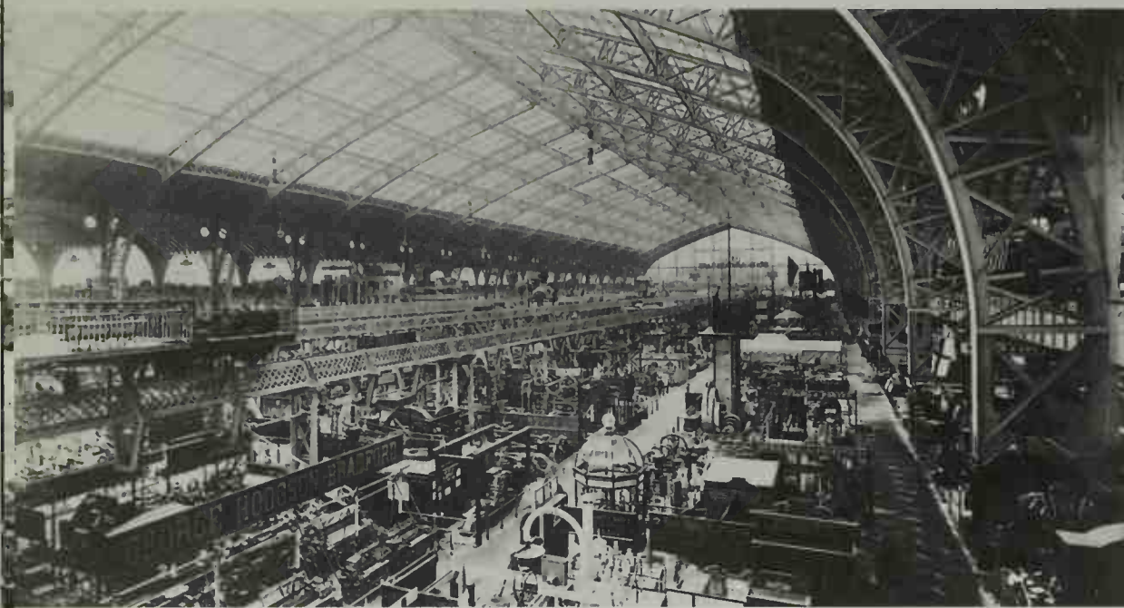
Left: The Galerie des Machines, by Contamin, Pierron and Charton. Like the Eiffel Tower, it was a metal structure of breathtaking size, built for the Paris exhibition of 1889.
