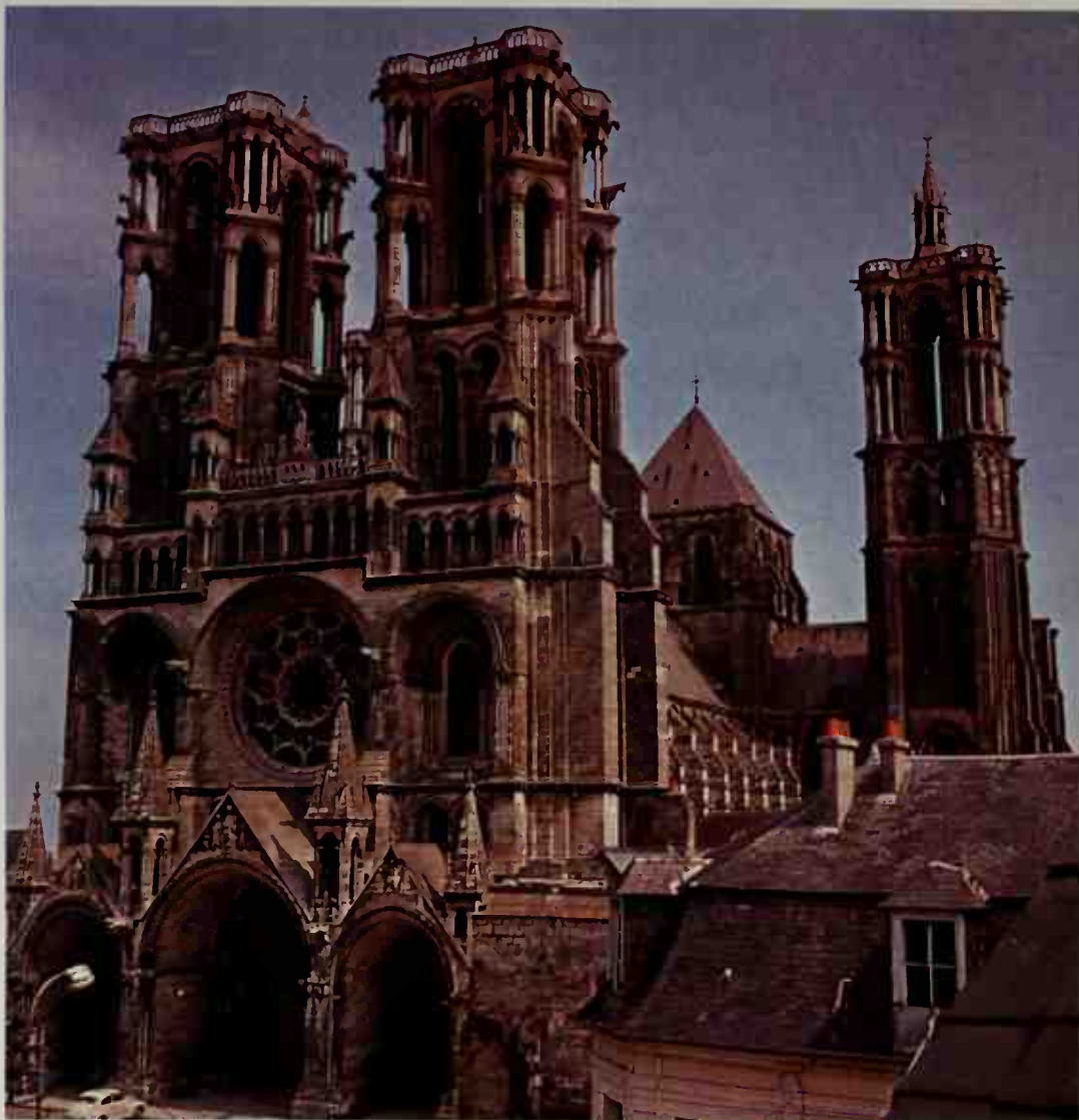
Above: The west front of Laon Cathedral, France, c.1190. Early Gothic façades were divided into three with two towers above. Here the sculptured doorways are under deep gabled porches. The upper parts of the towers are polygonal with added turrets from which peer figures of oxen said to represent those which hauled the carts of stone to the cathedral site.
