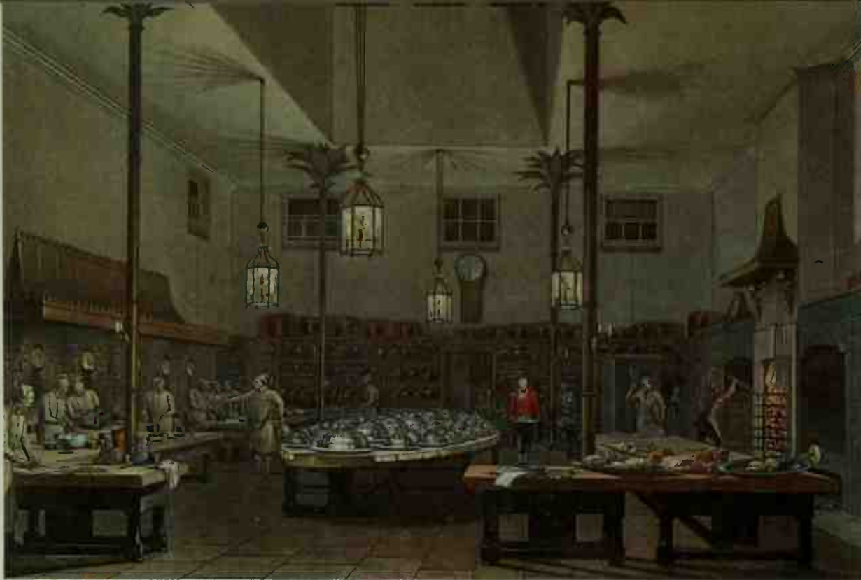
Left: The kitchen of John Nash's Royal Pavilion, Brighton, England, 1816–20. The trunks of the palms are cast iron tubes and the fronds are of copper. Iron was still an exotic material at that time.
