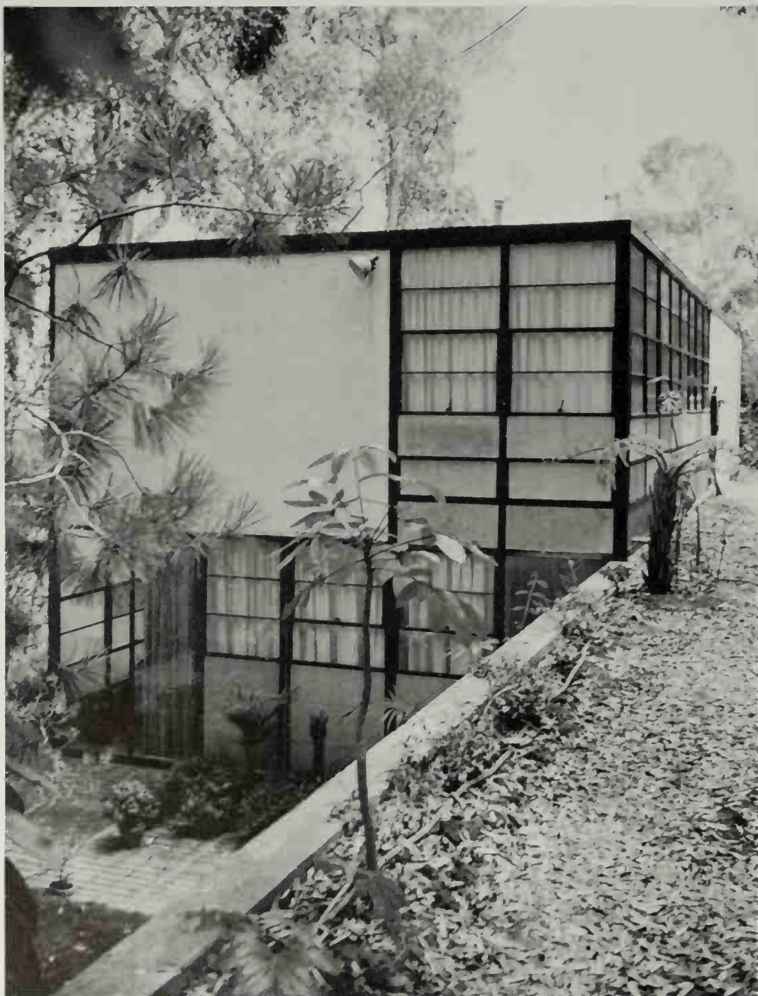
Right: Eames's house and studio, Santa Monica, California, USA, 1949: a creative use of out-of-the-catalogue components.
