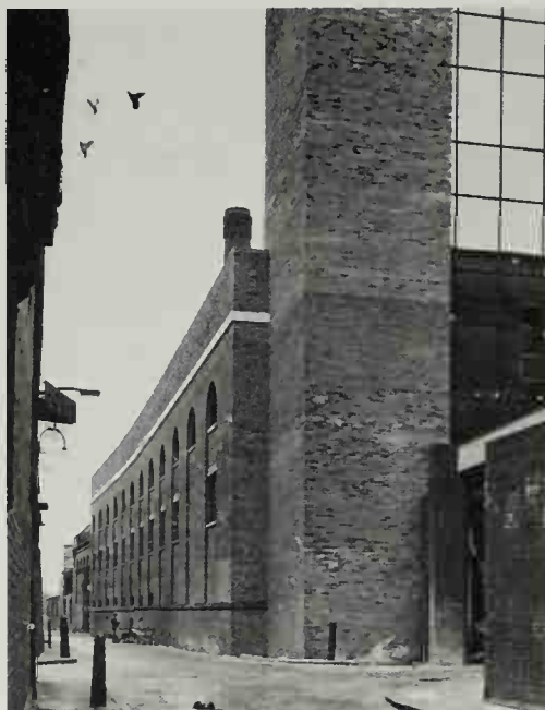
Left: The Quaker Street façade is slightly curved, following existing street lines, its blind arcades of brick reminiscent of late Georgian industrial architecture. The rear curtain wall shows on the right, indicating the location of floors of administrative offices above the rear, double-height servicing and loading yard and workshops.
