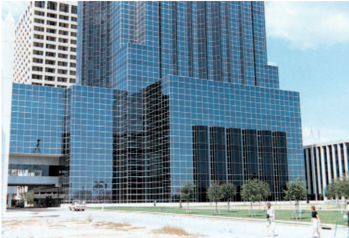
▲ Houston, USA: Transio Tower, early 1980s: Acres of glass curtainwalling typifying the commercial solution and image of corporate capitalism
