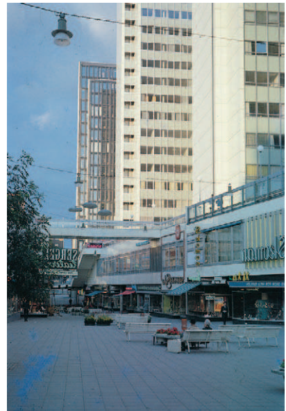
▼ Stockholm, Sweden, 1950s: A universal downtown solution to a business/retail precinct - clinical and presenting an uninviting face to the public space
