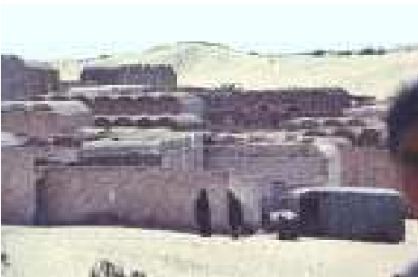
◀ Ouarghla near El Oued, S. Algeria: Single storey with efficient barrel roof vaulting in response to the absence of timber supplies
