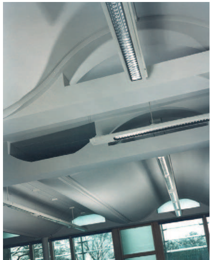
▶ ▲ Garston, Watford, UK: The BRE Building: The design reflects the challenge of integrating structure and services to inform the aesthetic
