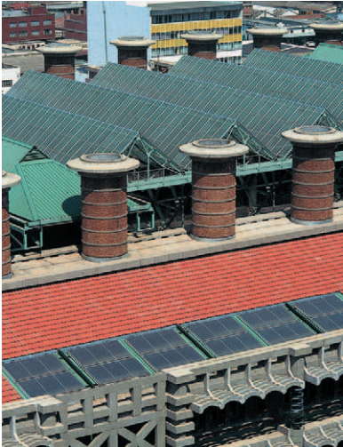
▼ ▼ Harare, Zimbabwe: Eastgate: Novel forms of aesthetic are derived from passive energy-reducing design measures
