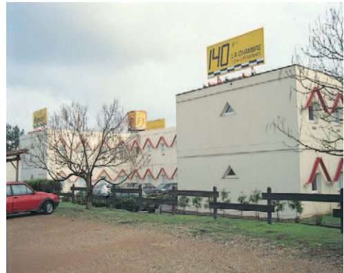
▲ St Etienne, France: Formula One Hotel of prefabricated concrete room cells, assembled on site. Architecturally precasting can deliver efficiency but usually at the expense of design sensitivity
