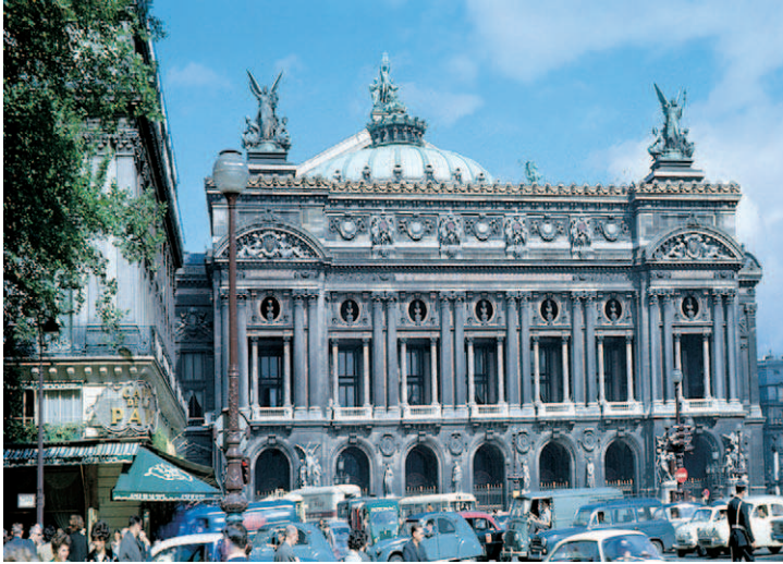
► The Opera House, Paris, France, by Charles Garnier, a Beaux Arts paragon, with its sculptures, gargoyles, its quoins and jamb stones, its cartouches decorated with scrollwork, its cornices topped with cheneaux and lined with dentils. In keeping with his fractal philosophy, Mandelbrot states that 'art that satisfies lacks scale' and the Paris Opera House has no scale because it has every scale
