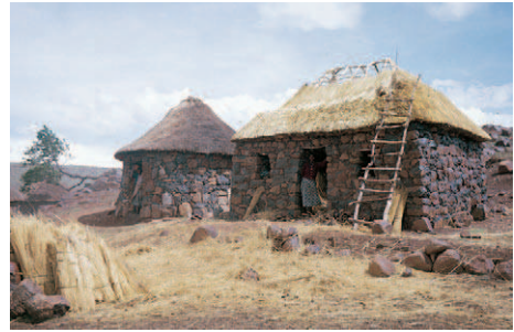
▲ Lesotho, southern Africa: The African hut: High altitude conditions requiring careful orientation, building mass and insulative performance. Materials are derived from immediate regenerative local resources
