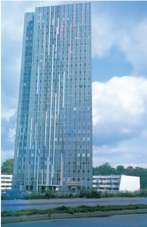
◀ Stockholm, Sweden: A tower block of the 1950s with a fully glazed external skin necessitating total dependence on mechanical airconditioning
