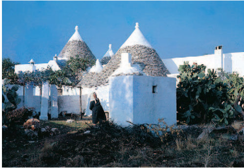
▲ Alberobello, Apulia, Italy: The trulli, with domical corbelled roofs of local stone
