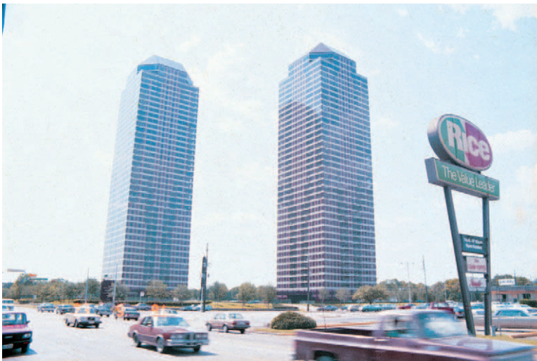
◀ Houston, Texas, USA, 1970s: Four Leaf towerblock condominiums, a refuge for the affluent from noise and air pollution in the public space. Such urban solutions afford little opportunity for community development
