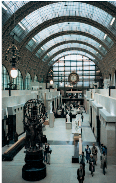
◀ Paris, France: The D'Orsy Museum, originally a railway station, 'recycled' to become an exhibition gallery for the work of famous sculptors, such as Balzac, Rodin et al. In the developed world the reuse of original fine historical structures for contemporary functions has become a trend and is to be welcomed
