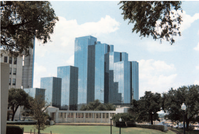
▲ Dallas, Texas, USA: Hyatt Regency Hotel (1970s): Clad with 7.85 acres of reflective glass that requires conditioned air to offset heat loss and gain daily and seasonally
