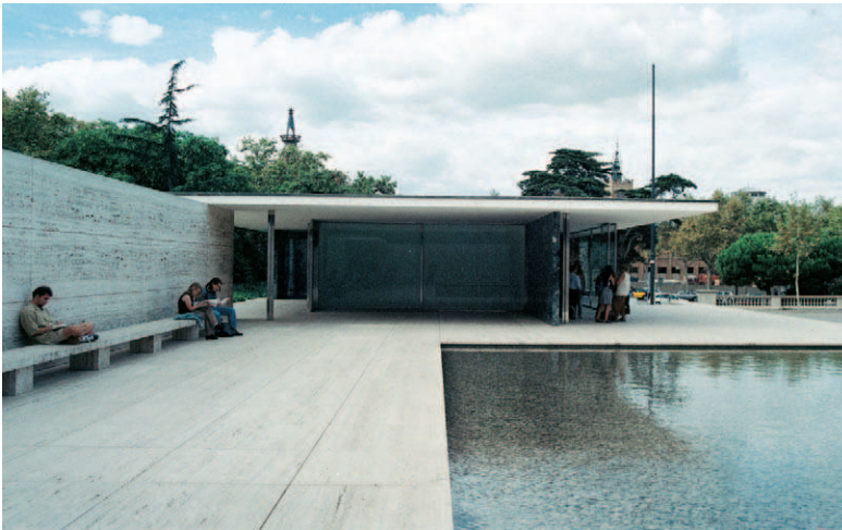
◀ Barcelona, Spain: The Barcelona Pavilion, 1928-29, by Modernist Mies van der Rohe: Demolished in 1930 and rebuilt to the original design in 1959, it epitomised the new order of Modernism. Sometimes the model has been described as being without practical purpose, and on the other hand as an 'icon of the Modern Movement' due to its freeing of the plan of structural considerations. Apart from structural considerations, through dogmatic functionalism the Modernists set out to liberate architecture from the pseudo-Classical chains of the past
