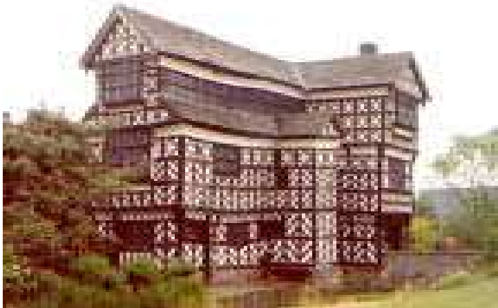
▶ Cheshire, UK: Little Moreton Hall, the Tudor approach to climate, affording maximum solar benefit during a moderate summer and cold winter months with extensive fenestration. A feature is the linear ambulatory in the upper storey enabling indoor exercise amongst other activities during long winters
