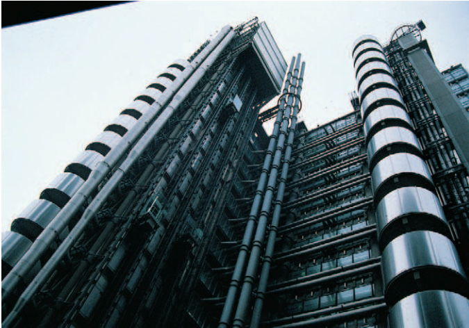
▲ Lloyd's of London, UK: The capital intensive route to sustainability, based on the 'pay back principle' with a longer term approach to resource efficiency and financial return on capital invested through energy-conserving measures
