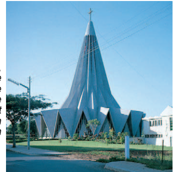
▶ Church, Maputo, LM: Folded concrete construction can be efficient in materials use due to the inherent strength of the folds in the shell construction
