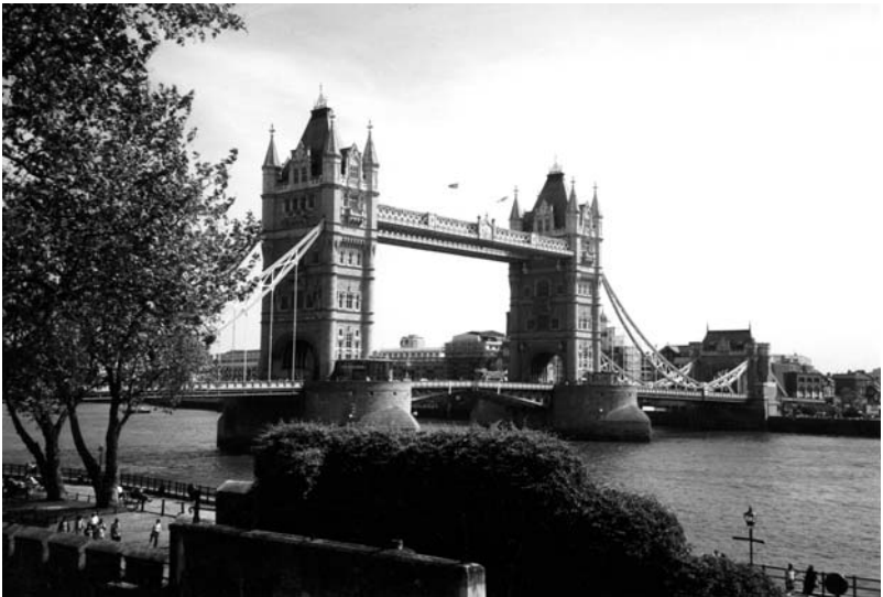
John Barry and Horace Jones, Tower Bridge, London, 1886–1894 (Photo: Allison Lee Palmer)
