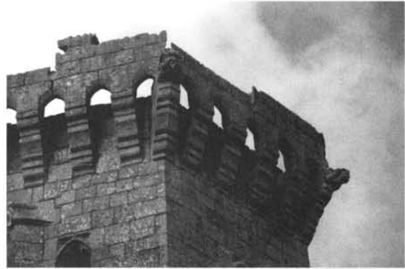
MACHICOLATIONS. The great gatehouse at Raglan Castle, Monmouthshire, features an impressive set of machicolations, carved openings at roof level that functioned like "murder holes" and were reputedly used to pour liquids or drop missiles down on an unsuspecting enemy.
