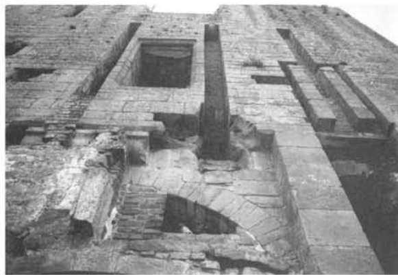
LIFTING GAFFS. Paired grooves for the lifting gaffs used to raise and lower the drawbridges into Raglan Castle's Yellow Tower of Gwent provide insight into how the mechanisms were used.
