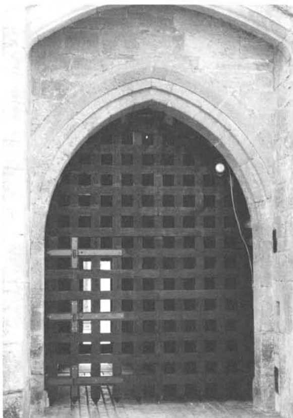
PORTCULLIS. A fine example of a typical portcullis, complete with a wicket, adorns the main gateway at Caldicot Castle in Monmouthshire.
