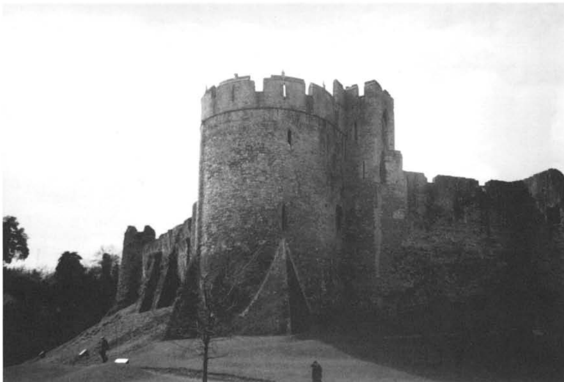
MARTEN'S TOWER, Chepstow Castle. Probably constructed to provide Roger Bigod III, the lord of Chepstow Castle, with well-defended private accommodation, the battlemented Marten's Tower retains substantial spurred buttresses, which helped prevent collapse and thwarted undermining.
