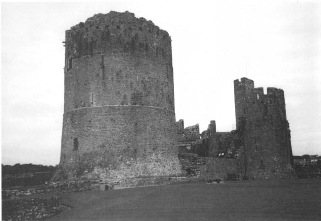
GREAT KEEP, Pembroke Castle. Erected in the early thirteenth-century, William Marshal's cylindrical keep completely dominates the inner bailey at Pembroke Castle. The dungeon tower added later in the century by William de Valence stands nearby.
