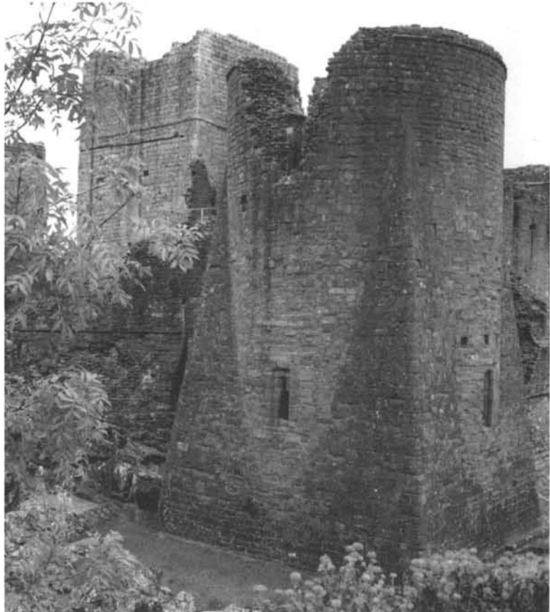
GOODRICH CASTLE, corner tower. Huge pyramidal spurs climb the walls of the southeastern tower at Goodrich Castle to bolster the tower and thwart the advances of sappers mining underneath the foundations.
