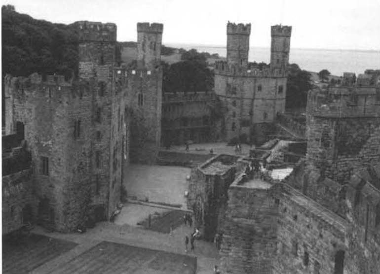
LOOKING TOWARD the upper bailey at Caernarfon Castle. Powerful polygonal towers dominate Edward I's imperial castle at Caernarfon, in Caernarfonshire, which he designed to resemble the great circuit of walls at Constantinople, now in modern Turkey.
