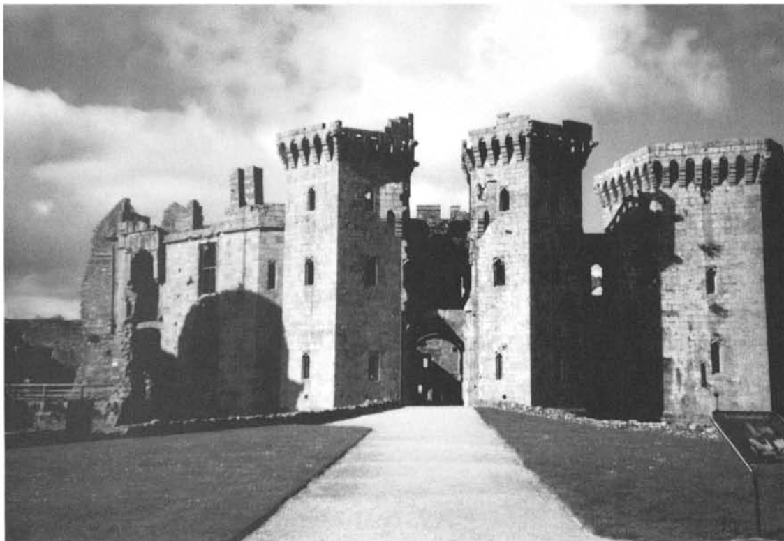
RAGLAN CASTLE, GATEHOUSE. The machicolated twin-towered main gatehouse and adjoining hexagonal closet tower built by William Herbert in the late fifteenth century still command attention at Raglan Castle, Wales' finest late medieval properly fortified military residence.
