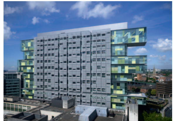
Photo: Tim Griffith
