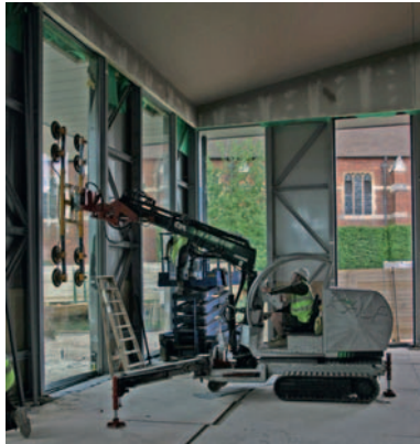
Photo: Eric Parry Architects
