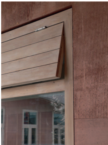
Ruthin Craft Centre – detail of concrete Photo: Ioana Marinescu
