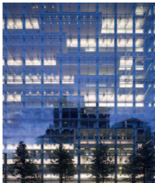
Manchester Civil Justice Centre Photo: Tim Griffith
