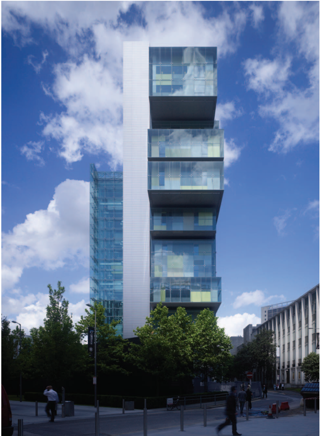
Photo: Tim Griffith
