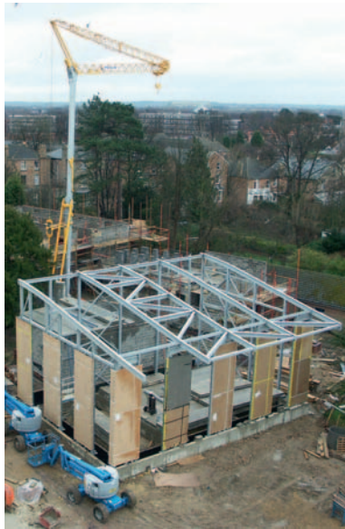
Photo: Eric Parry Architects
