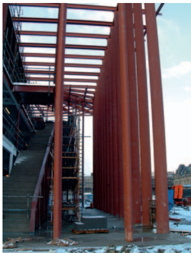
Photo: Designed by Erick van Egeraat
