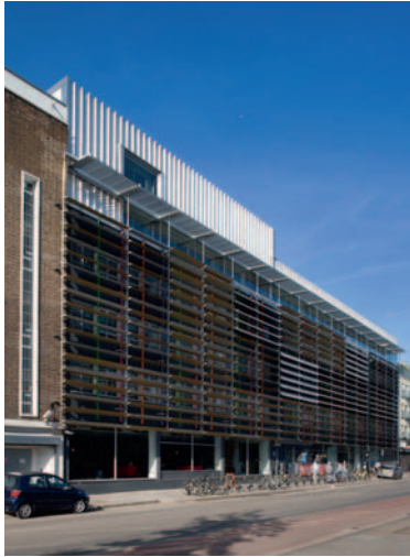
Rich Mix – new louvres on south façade Photo: Morley von Sternberg
