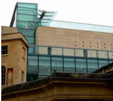
Thermae Bath Spa – stone cladding
