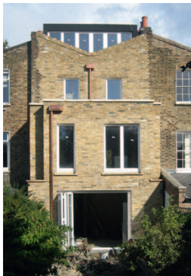
80% House – rear elevation
