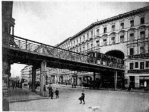
The Berlin Elevated Railway entering a building (c. 1900)
