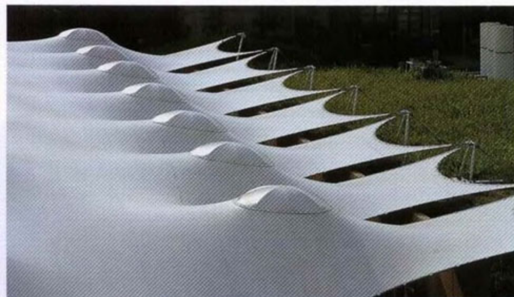
(Left) The translucent fibreglass membrane coated with teflon, seen from above and below
