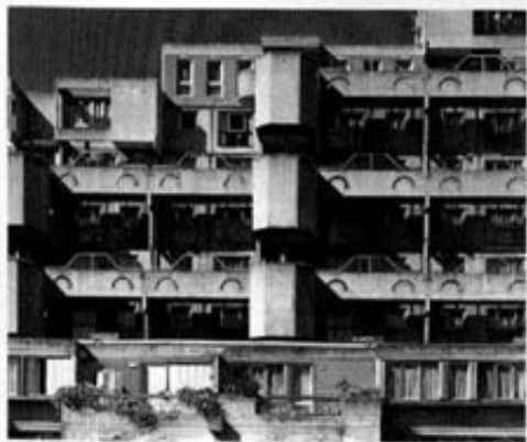
Paul Chemetov, block of flats, Saint-Ouen (1980)
