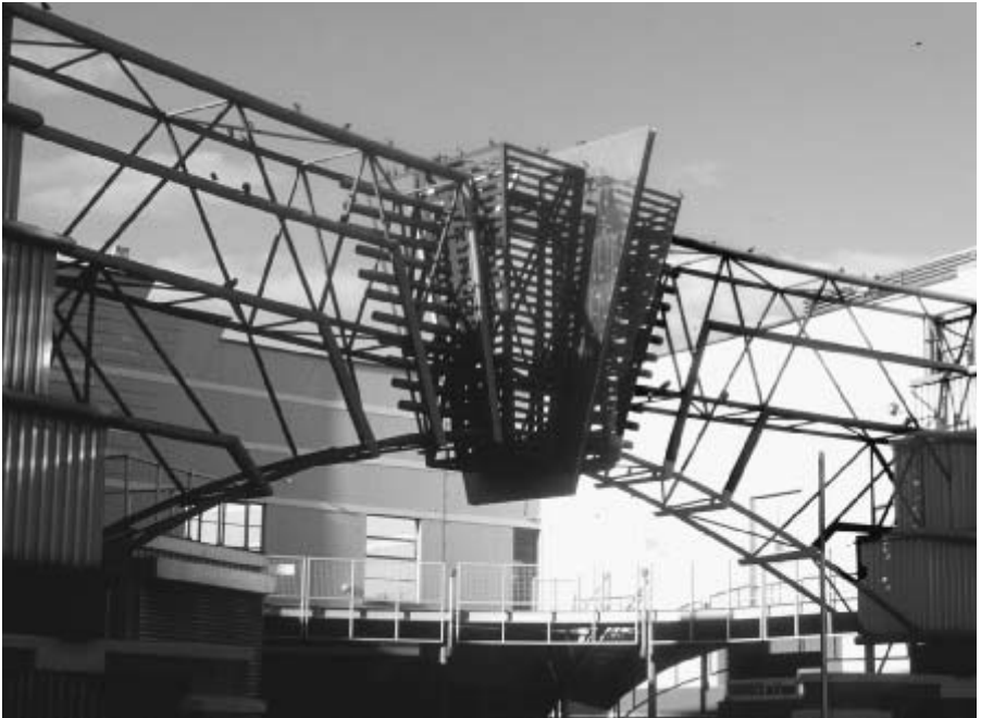
5.22. Terry Farrell, television studios, Camden Town, London, entry courtyard.
