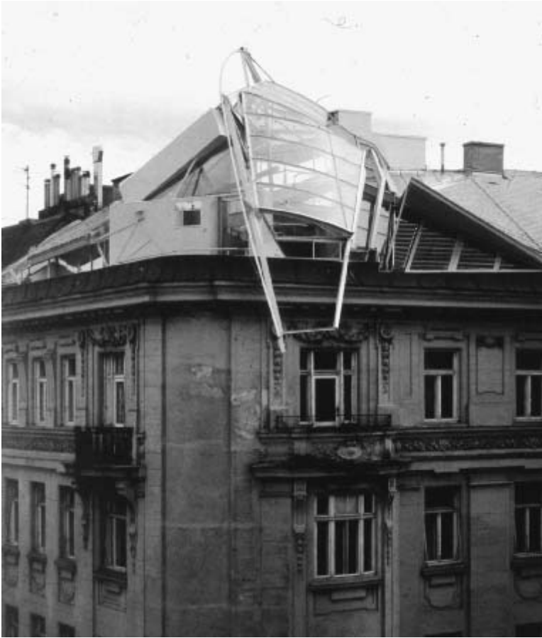
1.14. Coop Himmelblau, conversion of the attic space, Flakestrasse, Vienna (1989).
