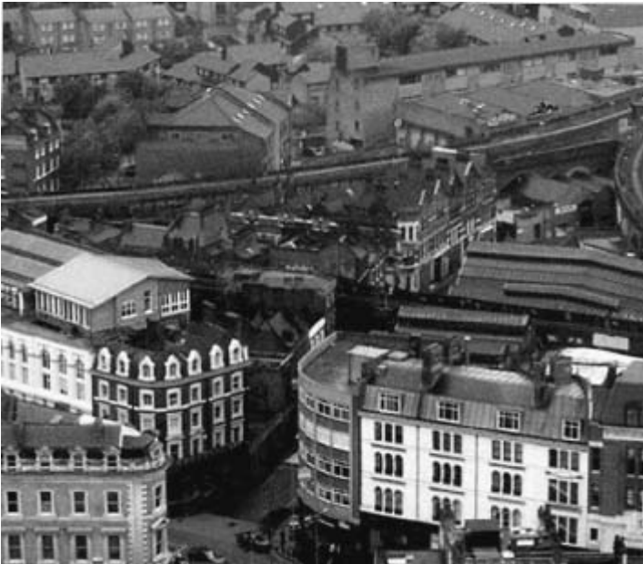
6.8. Railway viaducts in Southwark, London, aerial view.
