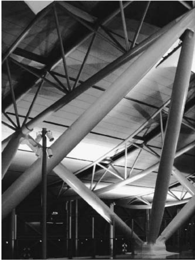
1.1. Renzo Piano, Kansai International Airport, passenger terminal.
