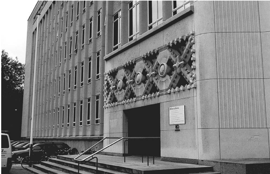
Figure 2.30 Former headquarters for Shell, The Hague. Design by J.J. Oud (1942). This design was characterised by a combination of strict symmetry and ornamentation in stone and coloured majolica. Oud had previously taken a very negative view of the application of ornament. For example, in 1921 he wrote, 'Ornament is the universal cure for architectural impotence'. Not surprisingly, he was much criticised for his Shell building design by those involved in modern building. His about-turn was seen as a betrayal of Het Nieuwe Bouwen [New Building].
