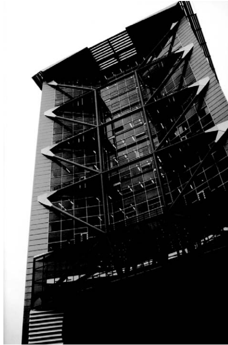
Figure 2.5 Malietoren, The Hague. Design by Bentheim Crowel Architects (1996). Because of its special situation – over a tunnel – this high-rise office block was constructed in the form of a steel and concrete bridge. The wind bracing on three levels shows how forces are offloaded on to the two side elevations.
