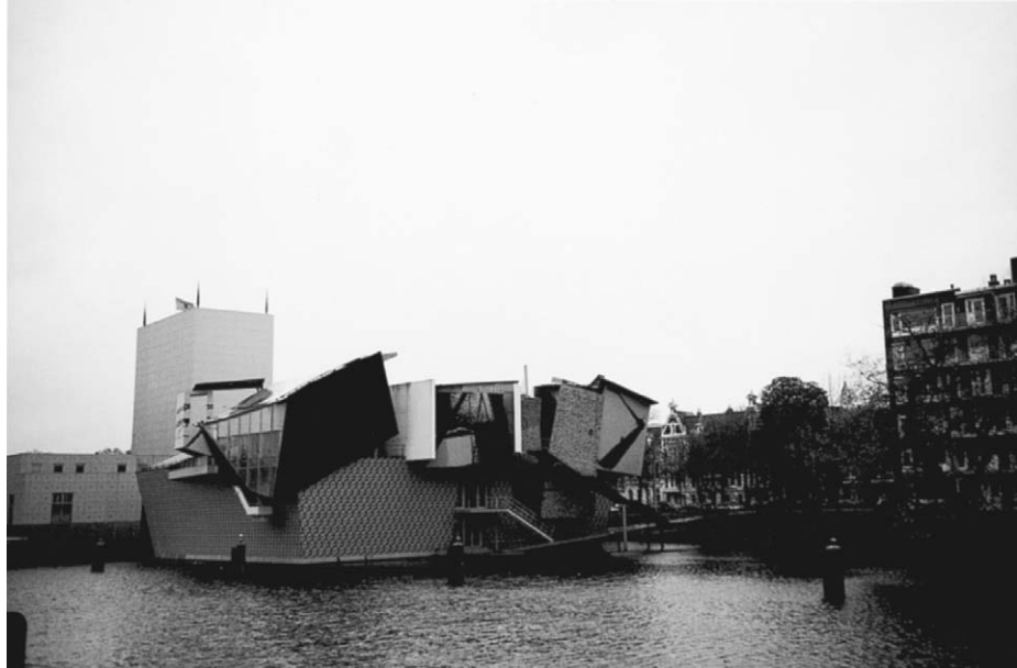
Figure 2.34 The Groningen Museum. Design by Alessandro Mendini, Philippe Stark, Coop Himmelblau and Michelle de Luchi (1994). The pavilion designed by Coop Himmelblau is a typical piece of deconstructivism. The roof, with its steel plates laid out at random, symbolises the breakthrough of fossilised systems.
