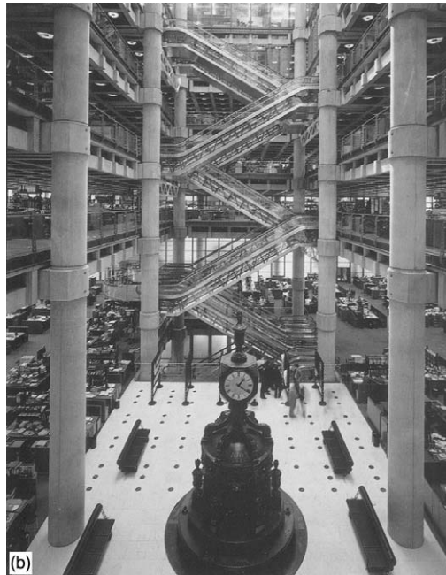
Figure 2.7 (a) Exterior and (b) interior views of, the Lloyd's of London, London. Design by Richard Rogers (1978–1986). All normal fixed obstructions, i.e. toilets, stairs, entrances, lifts and columns, are placed outside the building in six vertical towers clad in stainless steel. Another important aspect is the building's flexibility.
