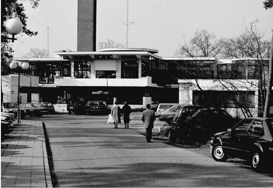
Figure 2.2 De Zonnestraal, Hilversum. Design by Duiker and Bijvoet (1926–1931). Jan Duiker was a member of De 8, a group of architects opposed to the excessively emphatic concern with design typical of, for example, the expressionism of the Amsterdam School and the architecture of De Stijl. The group's main concern was with functional and constructional efficiency.
