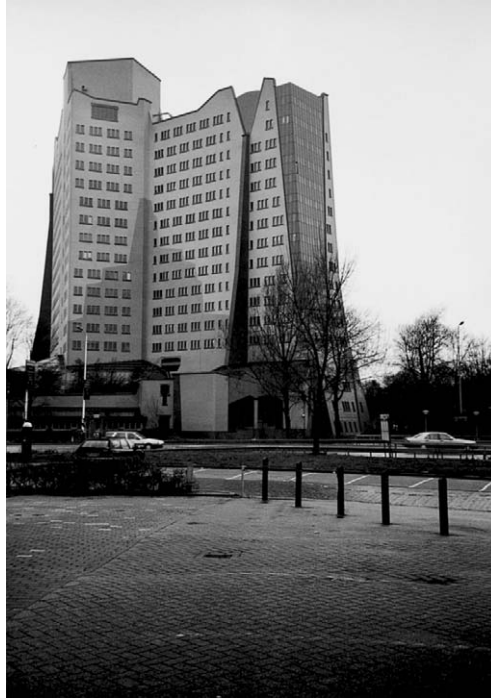
Figure 2.27 Headquarters building for Gasunie, Groningen. Design by Ton Alberts and Max van Huut. An example of (neo)-organic architecture, incorporating free expressive spatial forms. The design was strongly influenced by the desire to achieve a particular visual and spatial effect. For example, the rhythm of the windows is completely independent of specific inside rooms. The office space behind the windows is standard.
