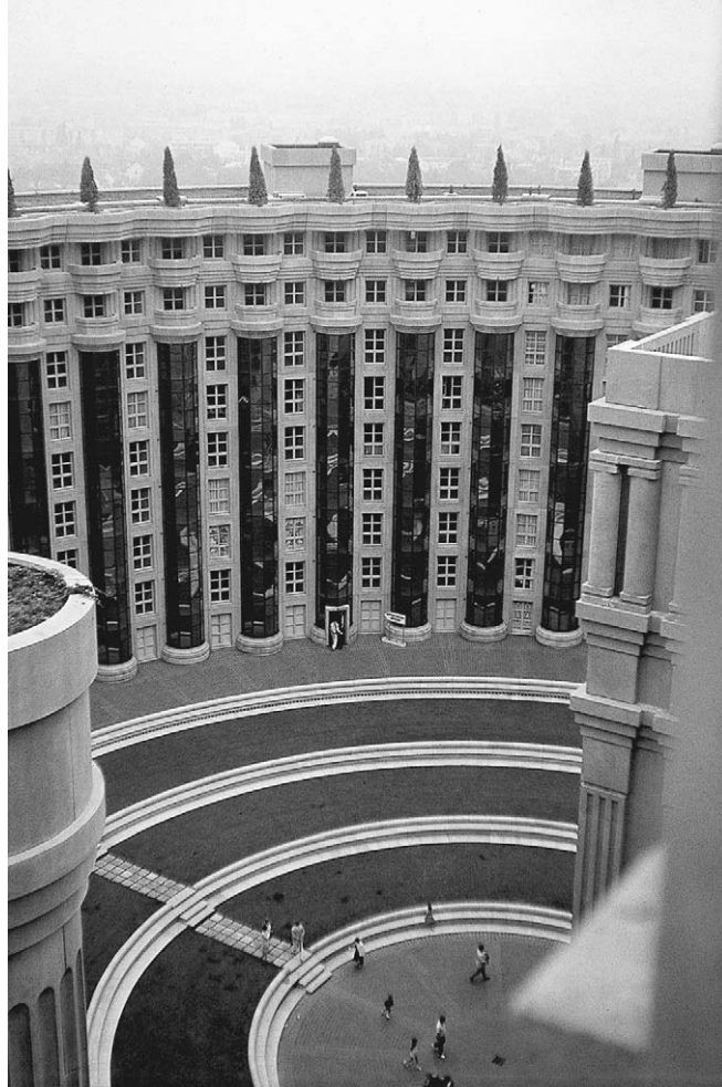
Figure 2.24 Le Théâtre, Paris. Design by Ricardo Bofill (1980). In the 1970s and 1980s Bofill and his Barcelona-based firm Taller de Arquitectura designed various large housing complexes in and around Paris, characterised by classical pilasters and arcades. The concrete elements used in the elevations incorporated coloured additives. In fact, the arrangement of the houses was subordinated to the historic décor.
