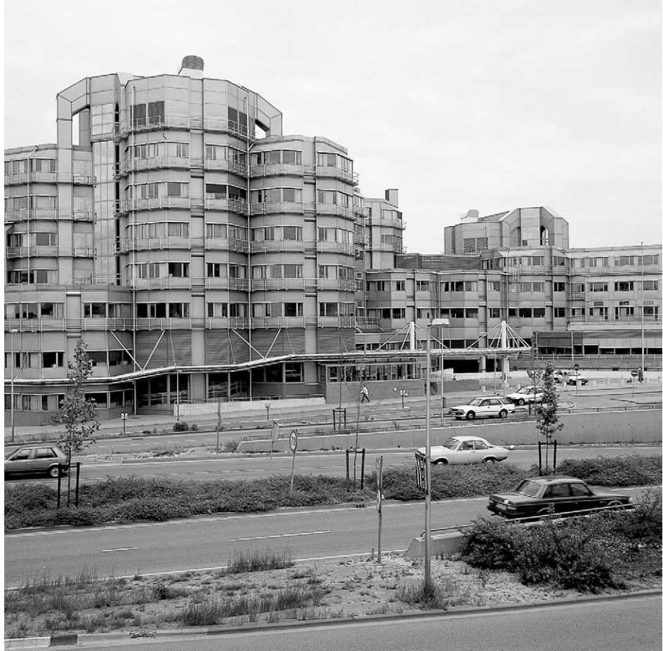
Figure 2.16 Ministry of Education and Sciences, Zoetermeer. Design by Philip Rosdorff (1976–1985). The way the rooms are arranged was determined by the wish to create individually recognisable units for different parts of the organisation, with short lines of communication between functions needing much contact with one another. The constructional plan was based on the metaphor of the city and contains a city centre (ministers and secretaries, senior civil servants, large conference rooms, etc.), a district community centre (directorates, small conference rooms, etc.), local community centres (lifts, toilet facilities, coffee machines) and housing (workrooms for staff). The original idea of an inward-looking building form comprising nine identical quadrangles was abandoned in favour of L-shaped blocks so that everyone would have an outside view. Differences in colour and material reinforce the recognisability of separate components.
