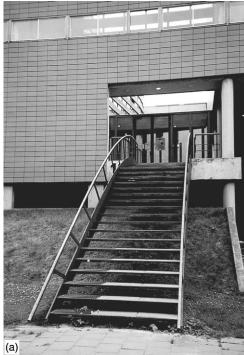
Figure 6.3 (a and b) A building with poor accessibility. Neither the cultural centre (a) nor the new NEN building (b), both in Delft, honour the principle 'building for everyone'. It is true that someone had the idea of putting special parking places right by the entrance and that wheelchair users can get to the main entrance of the NEN building by means of a lifting platform, but it would have been preferable to provide simple access for everyone, without the need for additional arrangements for special categories.
