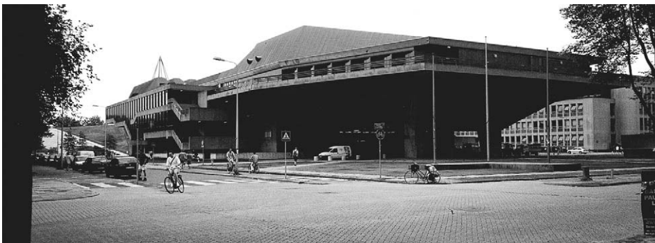
Figure 2.10 The Great Hall, Delft University of Technology. Design by Van den Broek and Bakema (1962–1965). The main outlines of the auditorium are clearly recognisable in the exterior. The fact that the ground floor is kept open on the side containing the entrance means that the main entrance stands on the same building line as the adjoining buildings. The huge cantilevers, the expressive stairways and the split-level floors all contribute to the building's fascinating visual quality.
