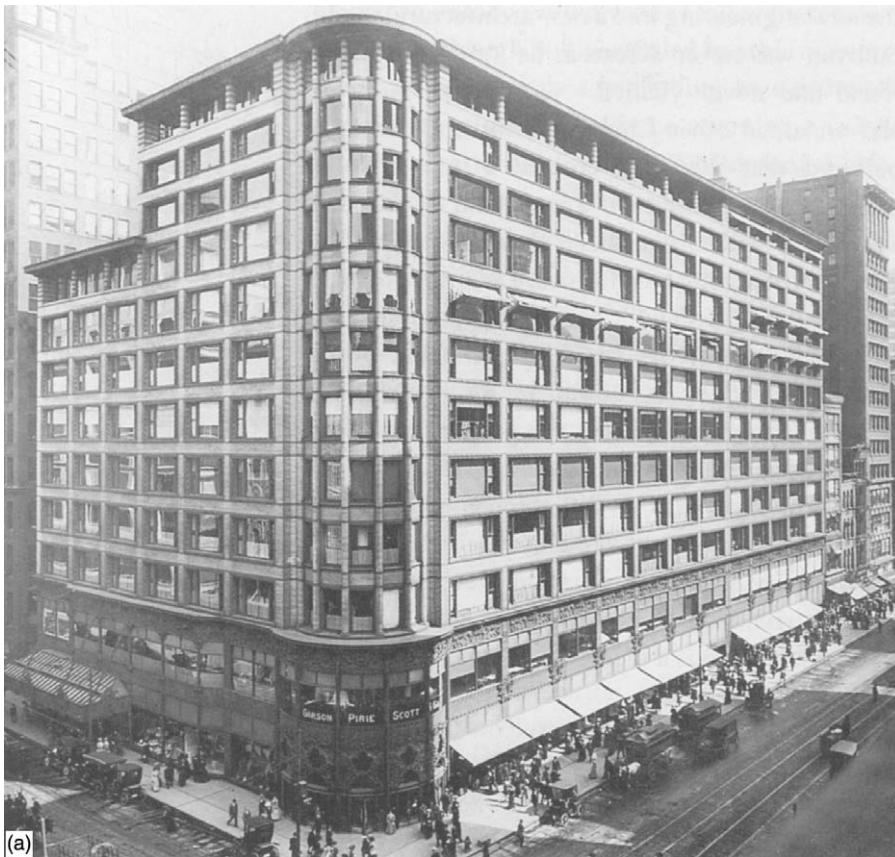
Figure 2.1 (a) The overall view and (b) the façade of the Carson Pirie Scott Department Store, Chicago. Design by Louis Sullivan (1899–1906). This building marked the high point of the functional tradition in the Chicago School and is a striking example of the transformation of utility and structure into powerful architecture. The great cellular screens along the streets are derived directly from the steel cage behind them.
