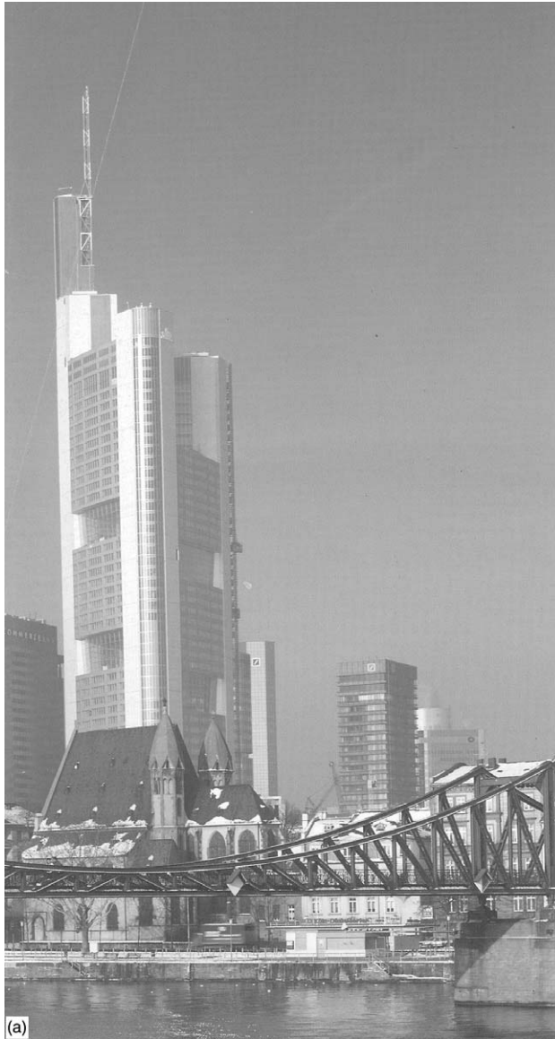
Figure 6.11 Commerzbank, Frankfurt, Germany. Design by Norman Foster (1991–1997). (a–c) Norman Foster’s Commerzbank is an example of a sustainable, energy conscious design on the scale of a skyscraper. At different levels of the buildings, winter gardens are situated, which allow vast amounts of light to enter deep into the building and also provide pleasant views to those working deeper within the building. These gardens have different functions that contribute to the well-being of the users. Operable facades create natural ventilation throughout the entire structure.
