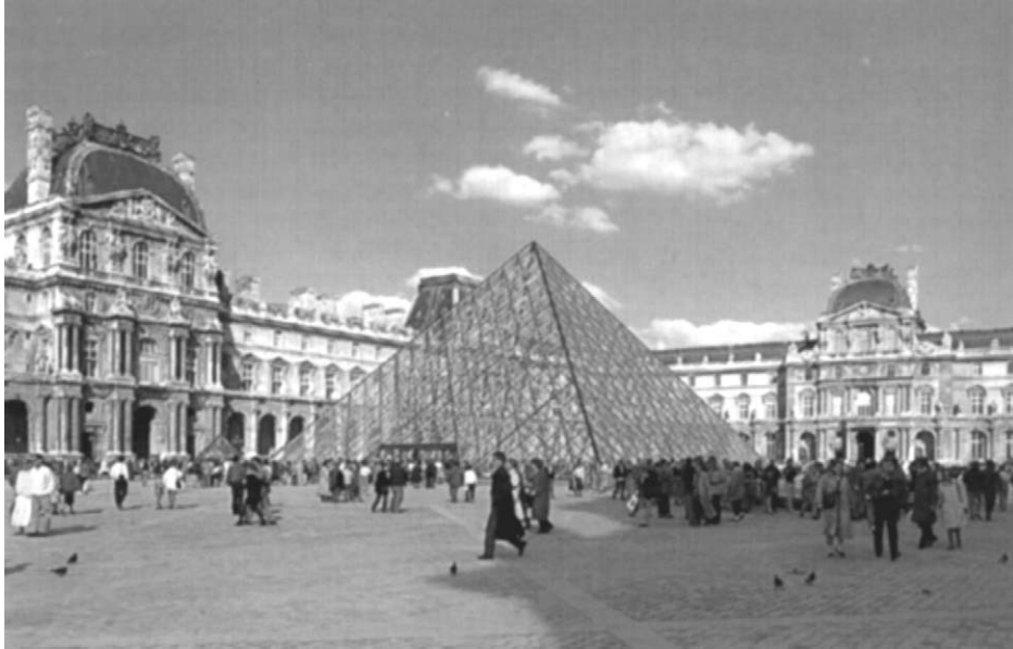
Figure 2.33 Louvre pyramid, Paris. Design by Ieoh Ming Pei (1989). I.M. Pei's proposal was to create the desired extension to the Louvre below the Cour Napoleon. The decision to create a monumental entrance in the form of a glass pyramid arose from the need to create a pure architectural form. The decision to use glass was inspired by a wish to provide ample daylight and to preserve the view of the historic Louvre. The pyramid is a lightweight construction and was one of former President Mitterrand's Grands Projects.
