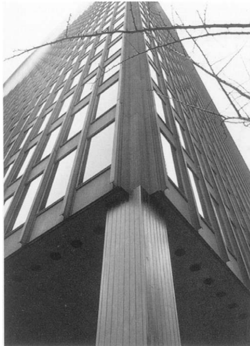
Figure 2.9 Seagram Building, New York. Design by Mies van der Rohe (1954–1958). This building has been regarded as the ultimate expression of the International Style. The design is based on the production of components and, as such, is anchored to the industrial process. I-beams were used in different kinds of length and function, load bearing and representative as well. The beams formed the skeleton of the building but also articulated the façade in segments.
