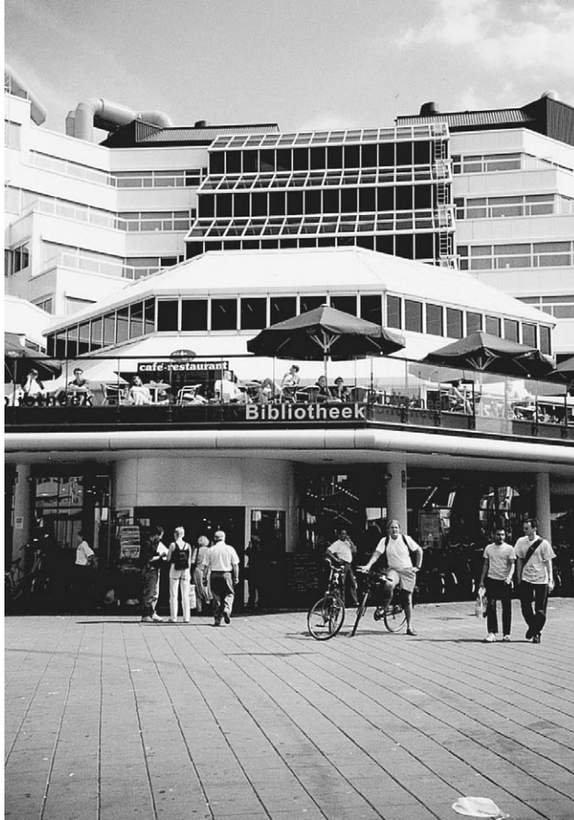
Figure 6.2 A building with good accessibility. In 1999 the Social Affairs and Employment Department of the city of Rotterdam published the report Over de drempel [Over the threshold]. This investigation into Rotterdammers' experiences with accessibility in their city showed that the city library scored high for accessibility. The wide revolving doors provide good accessibility for everyone, including wheelchair users and people with pushchairs. Within the building, good accessibility is ensured by lifts and escalators.
