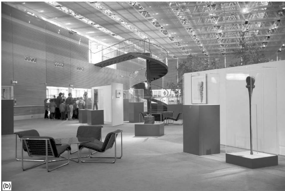
Figure 2.6 (a) Exterior and (b) interior views of, the Sainsbury Centre for Visual Arts, Norwich. Design by Norman Foster (1974–1978). The different functions are grouped within a single, clear-span structure, glazed at both ends, and lit from above. The internal space is covered by a double layer of the walls and roof, which houses service and ancillaries and also provides access for lighting and installations.
