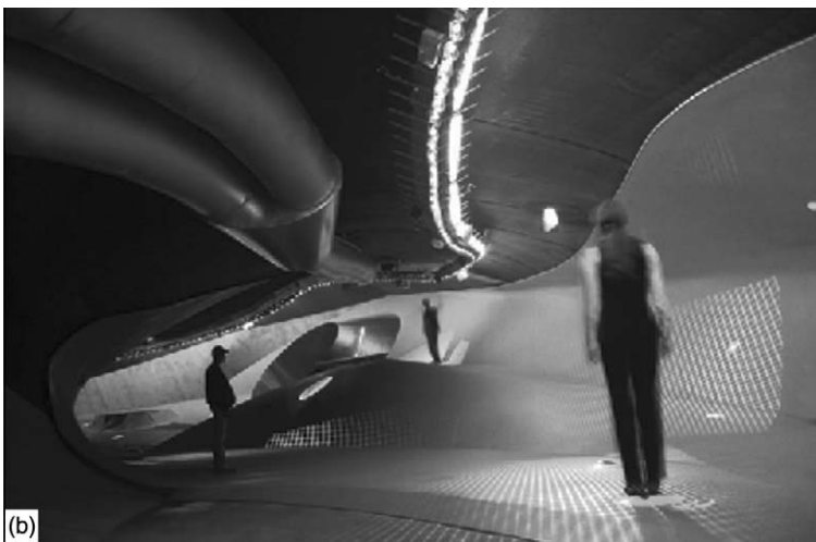
Figure 2.37 (a–c) Fresh Water Pavilion Neeltje Jans, Vrouwenpolder, Holland. Design by Lars Spuybroek (1993–1997). In this pavilion people can interact with light, sound, freezing of a wall, the spraying of mist, etc. The blob is made of 14 elliptical frames that vary in dimension, over which splines of stainless steel are braided.
