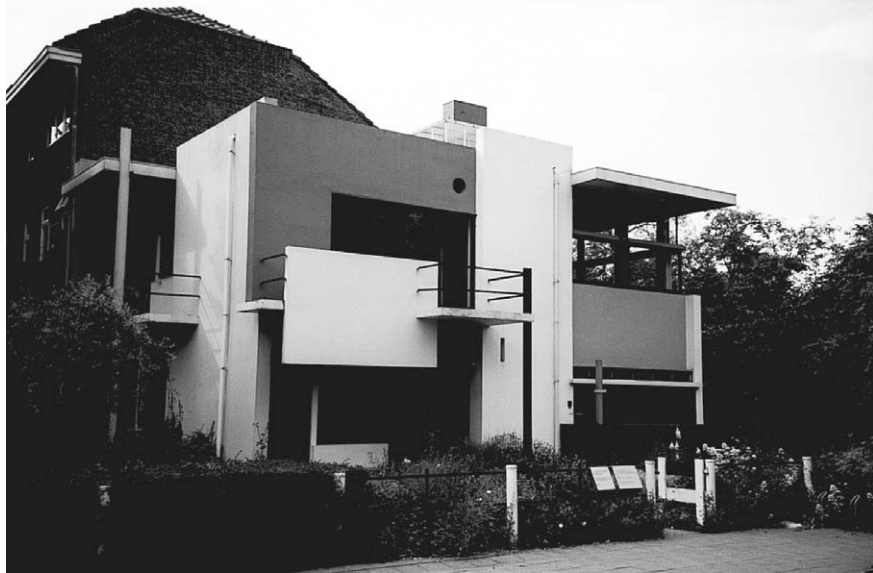
Figure 2.29 Rietveld-Schröder house, Utrecht. Design by Gerrit Rietveld (1924). The surfaces of the elevations are finished in white, broken white and four shades of grey. Window frames and pillars are painted red, yellow, blue and black.
