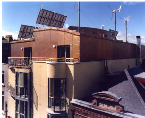
Figure 2-5: Three 1.5 kW Turbines on Green Building, Dublin developed by Murray O'Laoire Associates.
