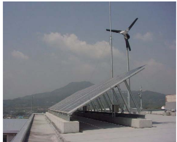
Figure 2-24: Five Proven WT600 (600 W) turbines on roof, Daito Bunka University, Japan (left) and WT2500 (2.5 kW) on a 6.5m tower on roof, Taku High School, Japan (right)
