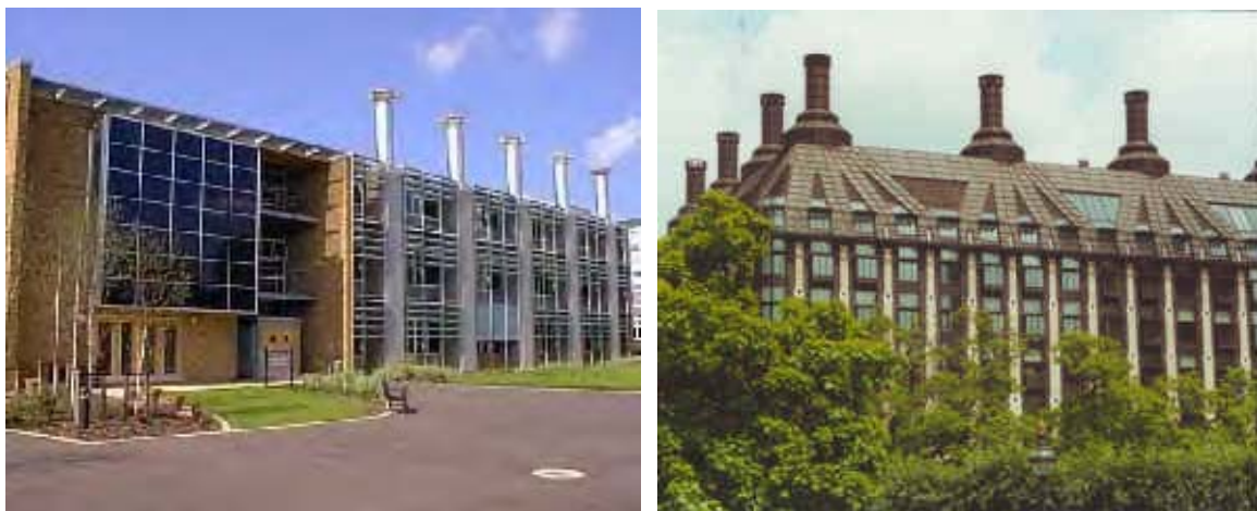
Figure 2-1: BRE's environmental buildings at Garston, NE London (left) and Portcullis House in Central London (right) which both incorporate passive stack ventilation towers
