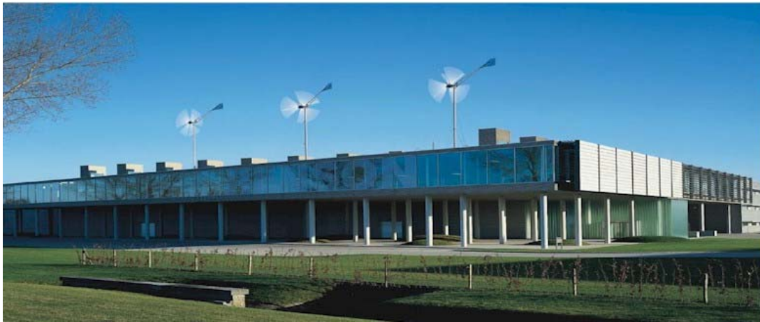
Figure 2-6: 3 x Fortis Montana wind turbines fitted to a factory/office
