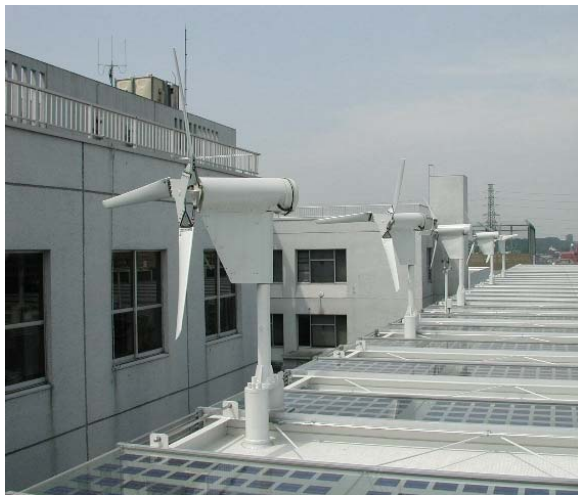
Figure 2-24: Five Proven WT600 (600 W) turbines on roof, Daito Bunka University, Japan (left) and WT2500 (2.5 kW) on a 6.5m tower on roof, Taku High School, Japan (right)
