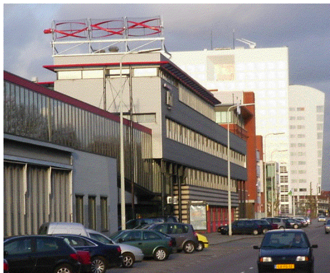
Figure 2-28: NGUp’s WindWall turbine installed on 15th January 2004 on the roof of the head office of the light rail company in the Hague in the Netherlands 85
