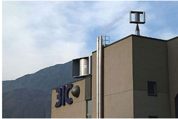
Figure 2-21: A WRE.005 0.5 kW and WRE.030 3 kW installed on the BIC (Business Innovation Centre), Bolzano in February 2003
