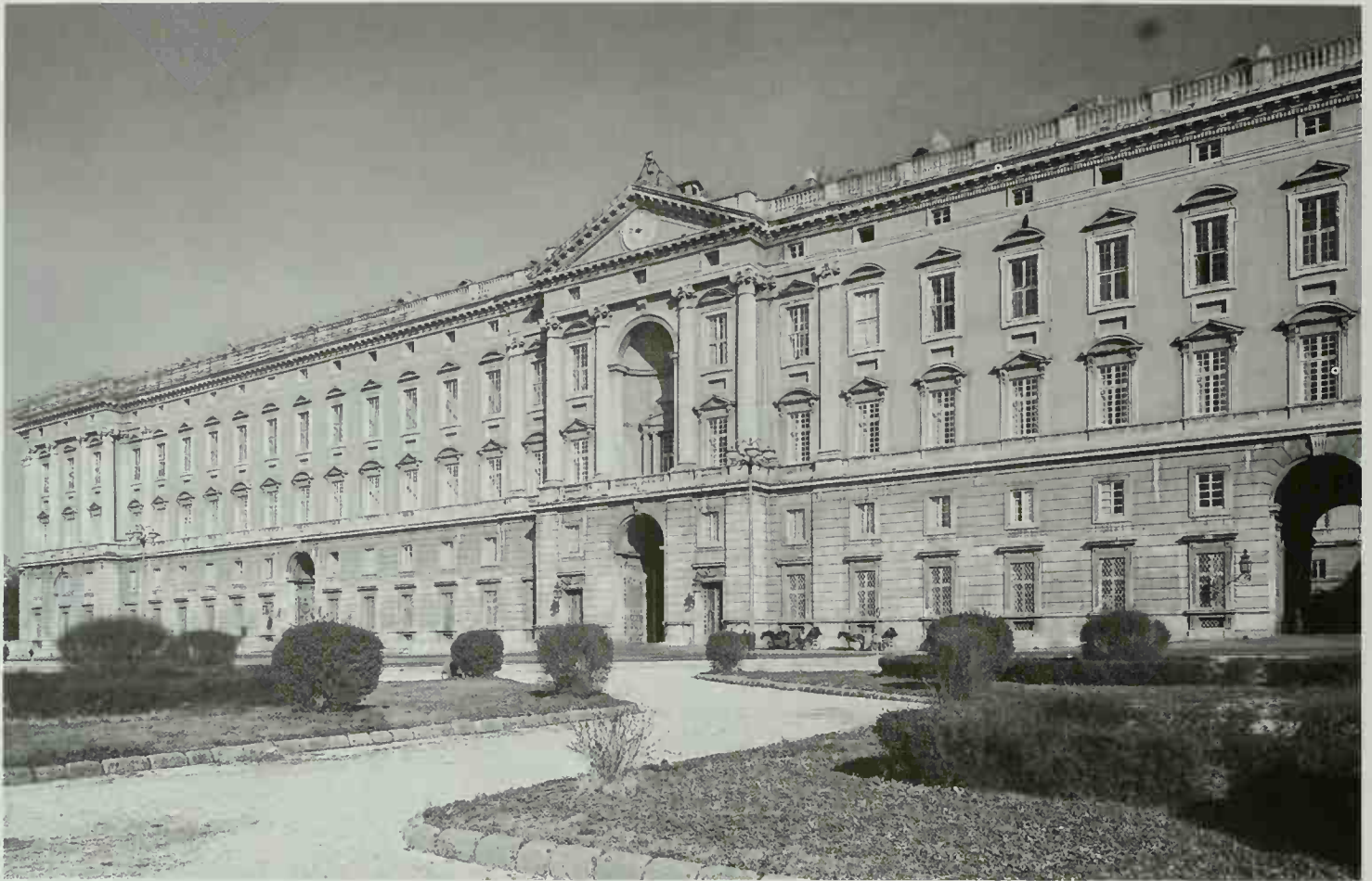
126 Above Caserta, Royal Palace by Luigi Vanvitelli, entrance front designed 1751
