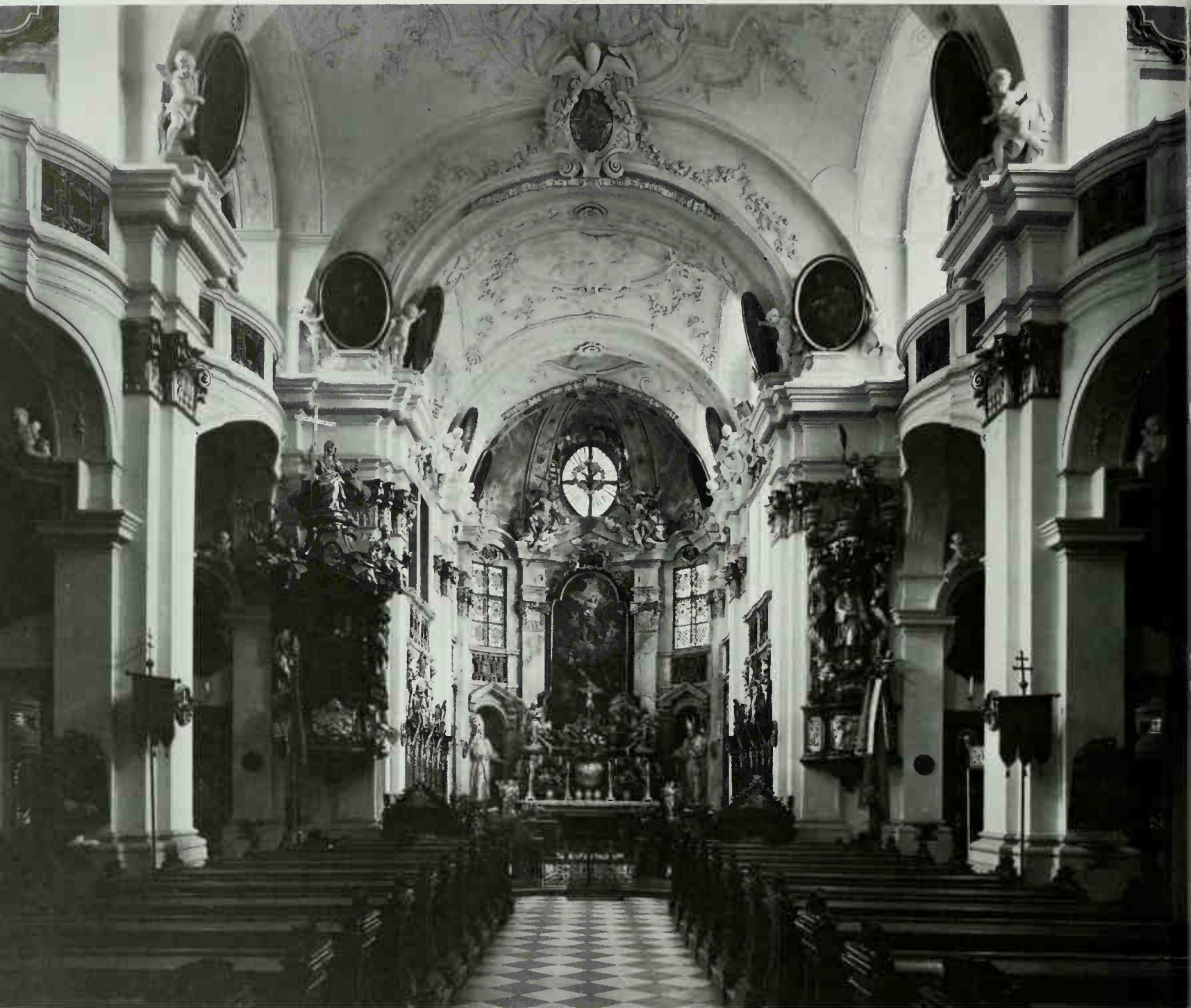
281 Duřín, interior of the church 1721–23, stucco by Santino Bussi
