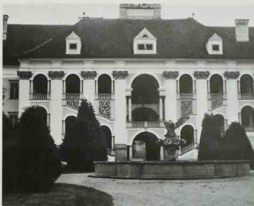
275 Opposite St Florian Abbey, upper flight of the staircase designed by Carlo Antonio Carlone and built (with alterations) by Prandtauer, 1706–14
