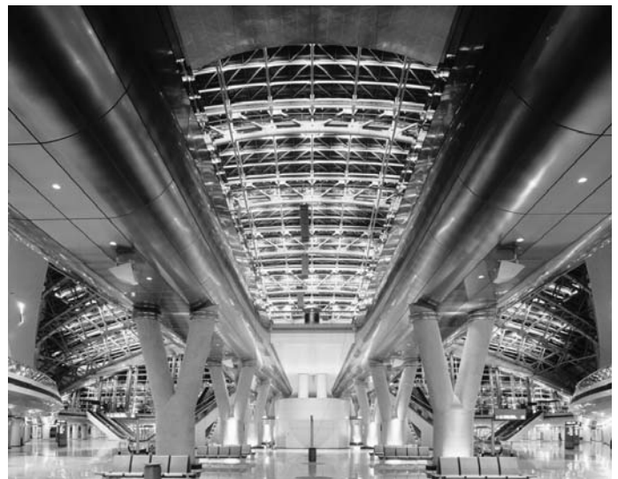
18.2 Incheon Transportation Centre, Seoul Airport. Architects: Terry Farrell and Partners.
