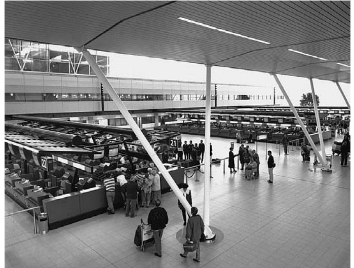
8.16 Structural separation used to define functional zones at Schiphol Airport, Amsterdam, the Netherlands. Architects: Bentham Crouwel.
