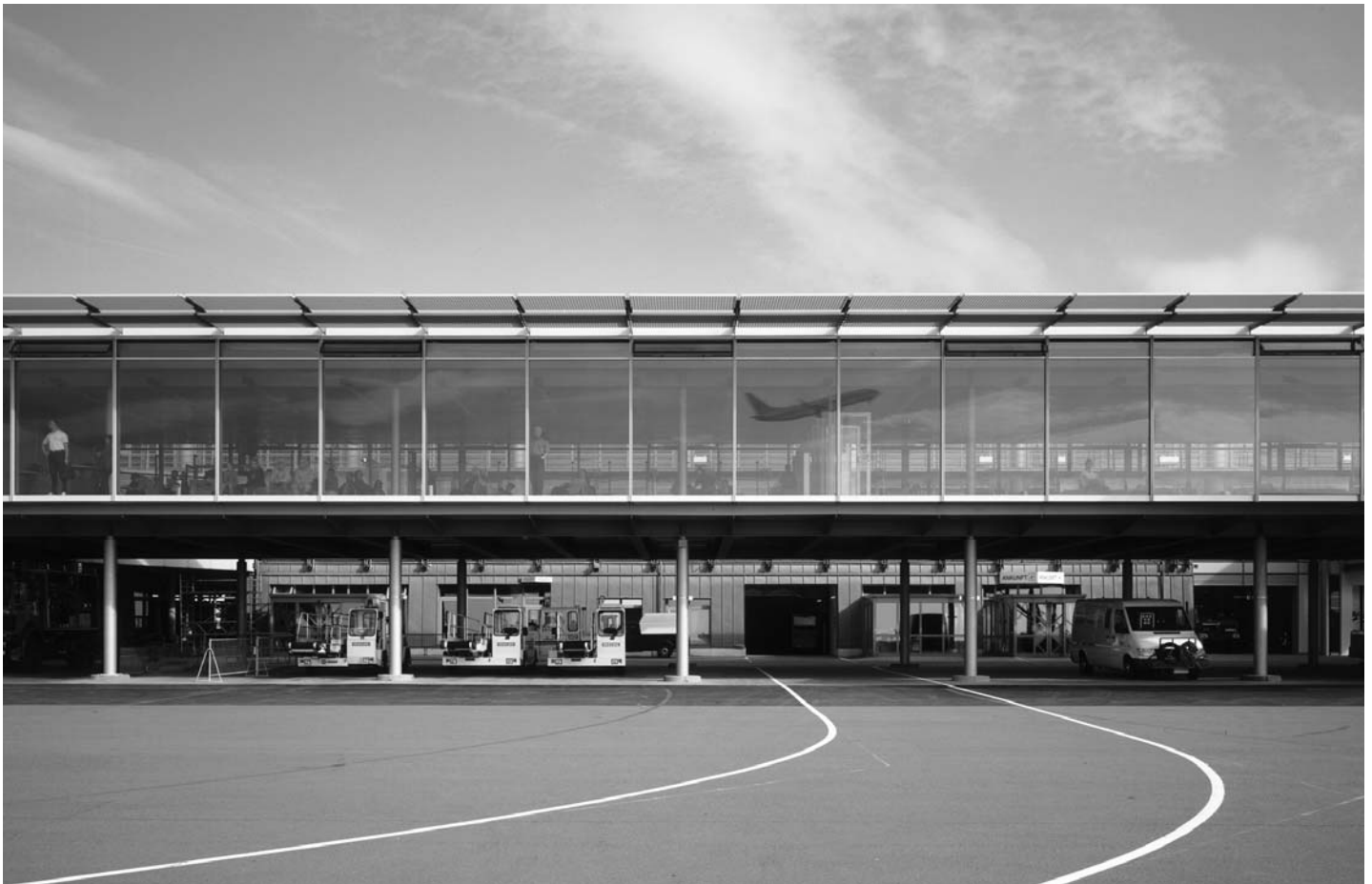
10.3 Airside view of passenger handling at rear of terminal. Paderborn-Lippstadt Airport, Germany. Architects: Von Gerkan, Marg & Partner.
