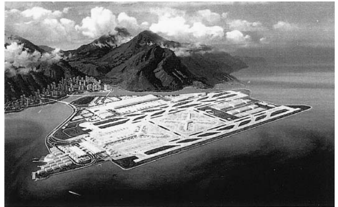
1.17 Off-shore islands can be created for the construction of new airports but for the economic benefits to flow to local communities, cheap surface transport is essential. Chek Lap Kok Airport, Hong Kong.
