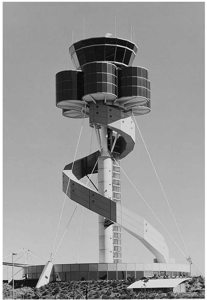
18.7 Control tower at Sydney Airport, Australia. Architects: Ancher/Mortlock/Wooley.
