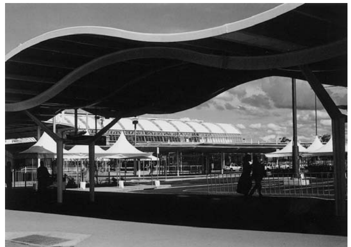
13.15 Shaded walkways reduce exposure to sunlight and glare which can impair vision. Sydney International Airport.
