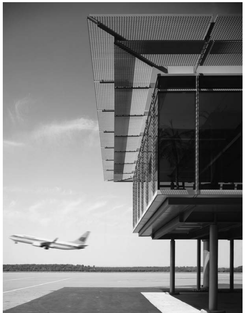
2.8 Tectonic construction is a feature of recent terminal design. Paderborn-Lippstadt Airport, Germany. Architects: Von Gerkan, Marg & Partner.
