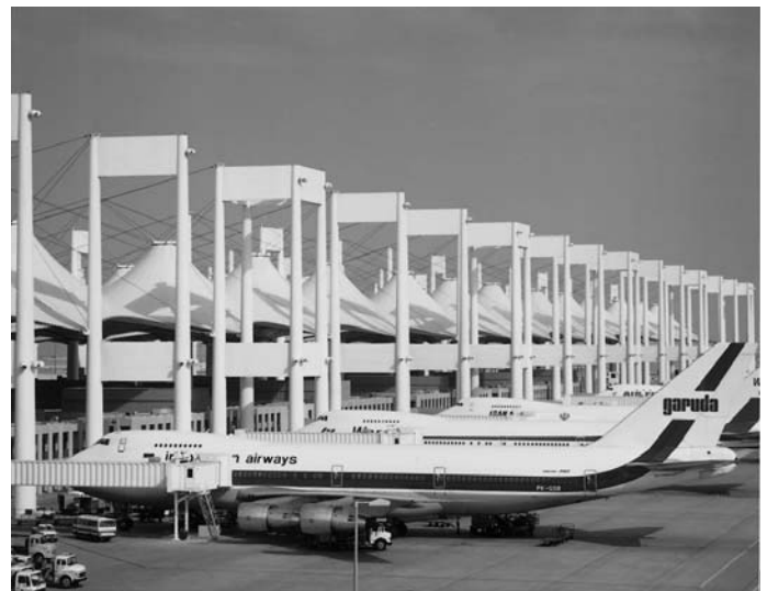
16.25 Haj Terminal, King Abdul Aziz Airport, Jeddah. Architects: Skidmore Owings and Merrill.
