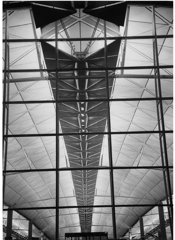
15.12 Detail of terminal ceiling at Chek Lap Kok Airport. Architects: Foster and Partners.
