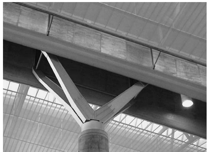
19.5 Detail of timber roof at Oslo Airport. Architects: Aviaplan AS.
