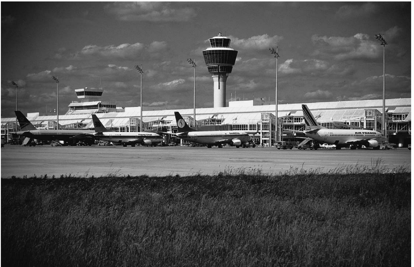
8.4 Changes in aircraft design trigger alterations to gate design. Munich Airport, Germany. Architects: Prof. von Busse, Blees, Kampmann & Buch.
