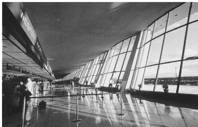
13.12 The check-in concourse at Dulles International Airport designed by Eero Saarinen and refurbished in 2000 by Skidmore Owings and Merrill benefits from high levels of natural light and clear company signage.
