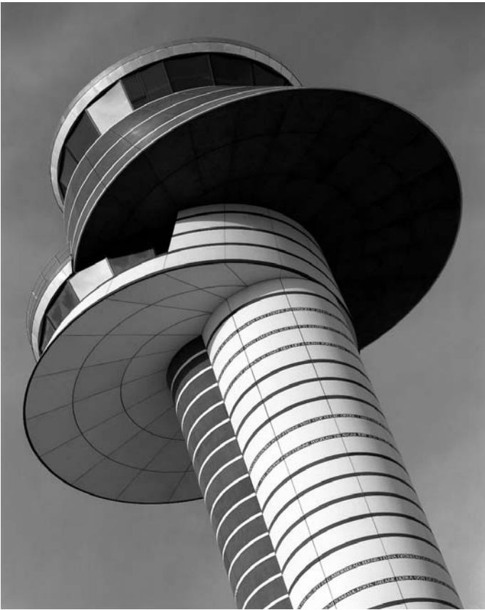
18.9 View of air-traffic control tower at Stockholm-Arlanda Airport.
