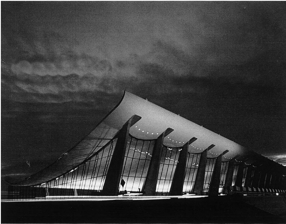
15.35 Dulles International Airport, Washington, designed in 1957 by Eero Saarinen and extended in 1999 by Skidmore Owings and Merrill.
