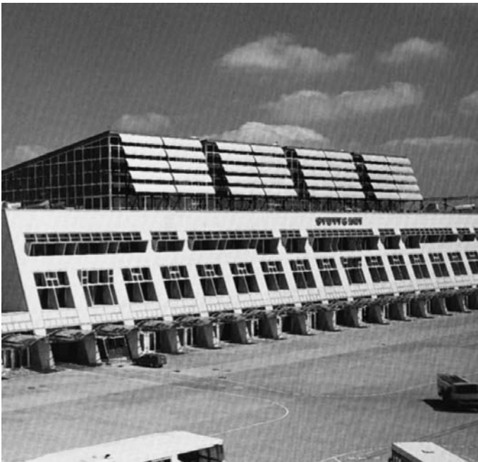
16.12 Acoustic and solar shading at Stuttgart Airport, Germany. The walls are angled to deflect sound. Architects: Von Gerkan, Marg & Partner.
