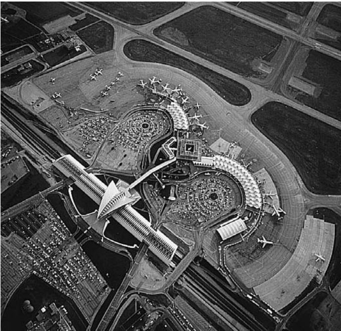
4.1 The classification of airports reflects passenger movements and architectural ambition. Lyon-Satolas Airport, France. Architects: Curtelin Ricard Bergeret/Scott Brownrigg and Turner/Santiago Calatrava.
