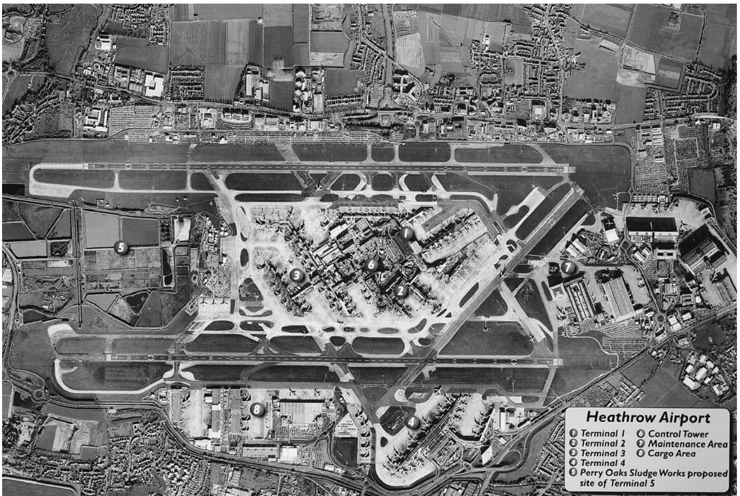
2.1 Heathrow from the air. Heathrow employs more people than the city of Oxford and contributes £1 billion to the UK economy.
