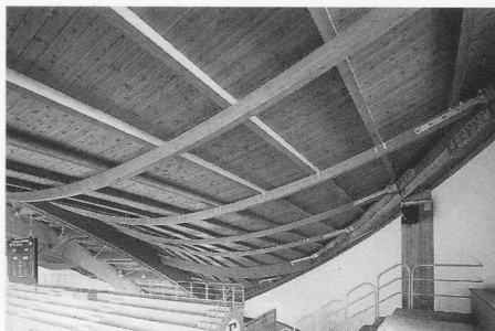
5 | Interior showing main beams and suspended shells.
