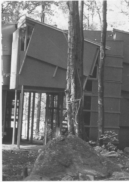
4 | The lookout tower seen from the lake side.
