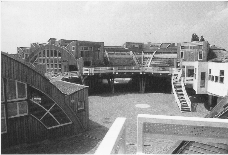
3 | View of courtyard. In the background the public gallery in front of the classrooms.
