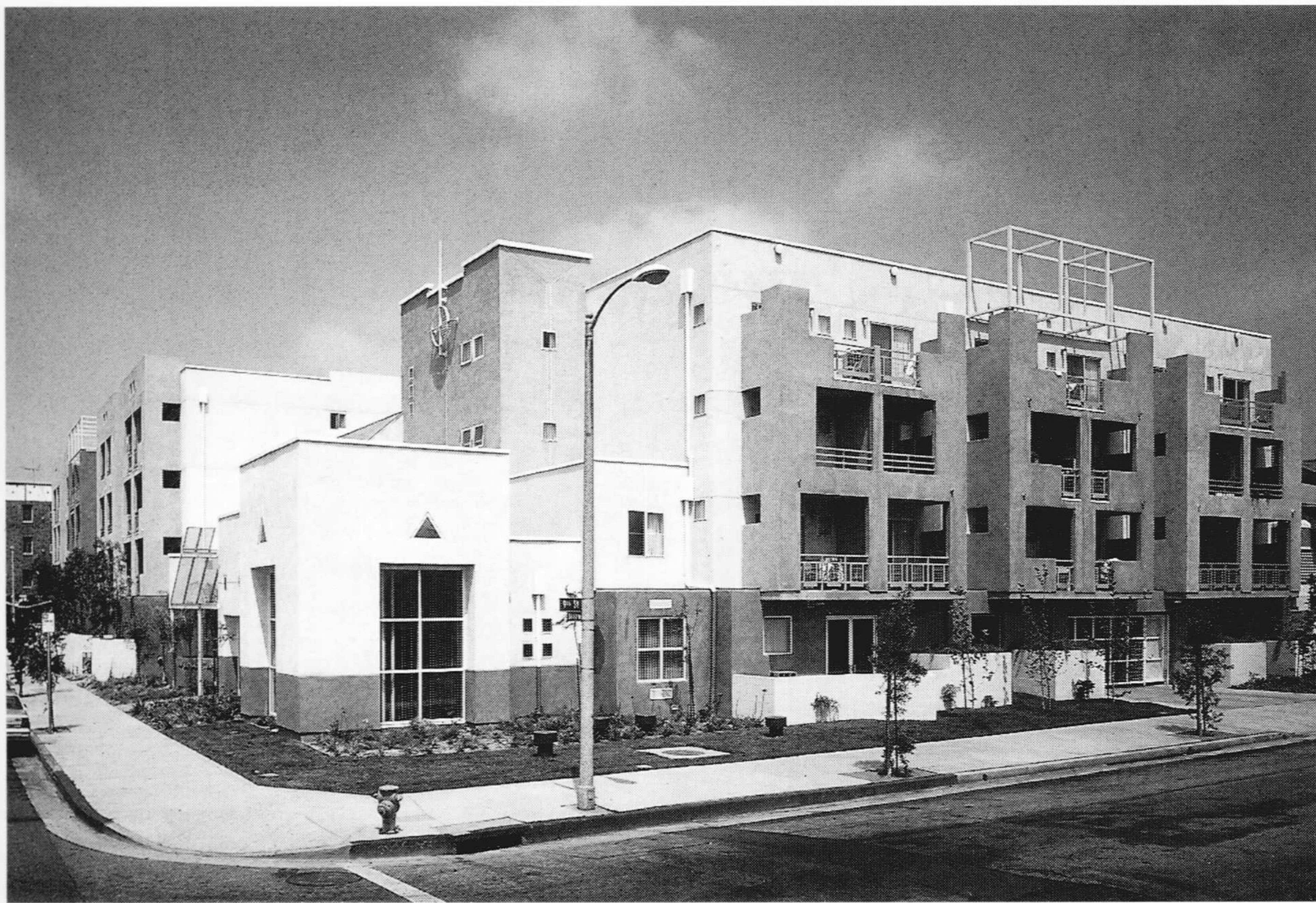
5 | View of the whole building from the south-east.
