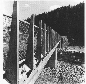
6 | The balustrading during construction.
