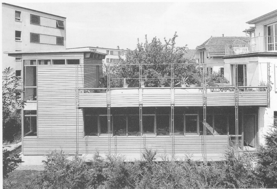
5 | South-east elevation of extension. Above, the private rooftop patio, below, the office, on the left, the pavilion, right, the old house.
