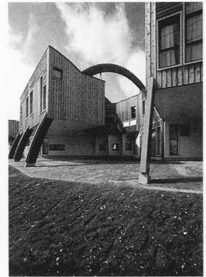
8 | Entrance and administration area.
