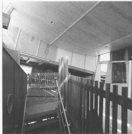
7 | Entrance hall during the construction stage. Same view as illustration 6.
