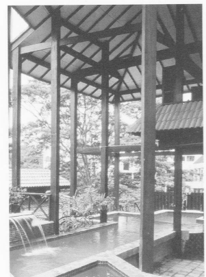
10 | View from patio level through the timber framework of the open roof towards the guest-house and the balcony to the living room, whose open timber balustrading is clad with a strip of roofing.
