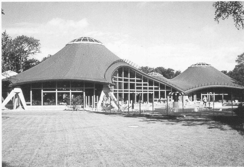
3 | View from sunbathing area. The three-legged reinforced concrete roof supports are clearly visible.
