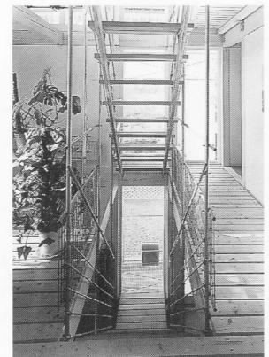
11 | Staircase at first floor level. Beechwood treads on steel stringers. The entire gallery is made from beechwood planking with open joints and no insulation or ceiling underneath. Also visible are the exposed solid timber joists which emphasize the construction.
