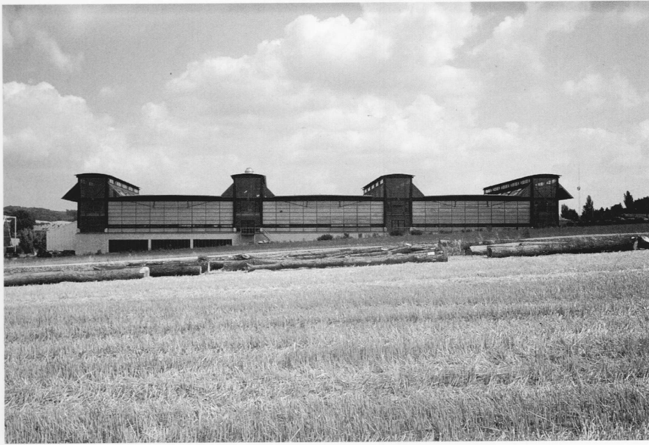
6 | View of production building from the west.
