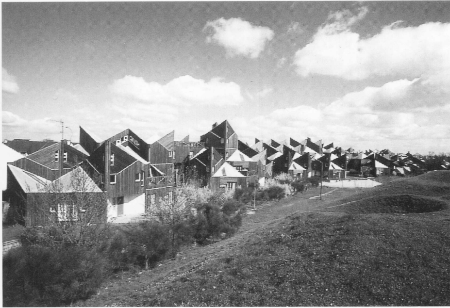
3 | View of the development from the screening embankment.
