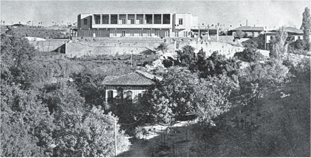
FIGURE 1.14. ATATÜRK'S RESIDENCE IN ÇANKAYA, DESIGNED BY CLEMENS HOLZMEISTER, WAS THE NEW TERMINUS OF ANKARA'S NORTH-SOUTH AXIS. IN THE FOREGROUND, THE VINEYARD HOUSE, THE INITIAL PROPERTY TO WHICH HE MOVED SHORTLY AFTER HIS ARRIVAL IN ANKARA. COURTESY OF THE TURKISH HISTORICAL SOCIETY LIBRARY.
