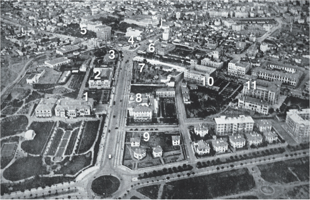
FIGURE 1.2. AERIAL VIEW OF ULUŞ FEATURING THE CITY'S GROWTH CIRCA 1930 (1—GRAND NATIONAL ASSEMBLY, 2—COURT OF FINANCIAL APPEALS, 3—MAKESHIFT FIRST BUILDING OF THE GRAND NATIONAL ASSEMBLY, ORIGINALLY, UNION AND PROGRESS PARTY CLUB, 4—ULUŞ ATATÜRK MONUMENT, 5— MINISTRY OF FINANCE AND TREASURY, 6—MINISTRY OF EDUCATION, 7—PARK (MILLET BAĖESİ), 8—ANKARA PALAS HOTEL, 9—THREE CITY BLOCKS OF HOUSING CONSTRUCTED BY THE PIOUS FOUNDATIONS ADMINISTRATION, INCLUDING A MULTISTORY PERIPHERY BLOCK CONTAINING A THEATER, 10—CENTRAL BANK, 11—BANK OF AGRICULTURE). COURTESY OF THE LIBRARY AT THE MINISTRY OF PUBLIC WORKS.
