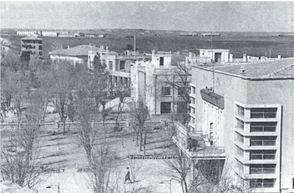
FIGURE 6.11. DIYARBAKIR HALKEVI UNDER CONSTRUCTION (TOP) AND FINISHED (BOTTOM) WITH OTHER INSTITUTIONAL STRUCTURES OF THE NEW STATE—INCLUDING THE TEACHERS’ AND OFFICERS’ CLUBS, GOVERNOR’S MANSION, AND A GIRLS’ INSTITUTE—THAT WERE BEING SITED IN THE SAME AREA. SOME OF THESE APPEAR IN THE BACKGROUND. COURTESY OF THE TURKISH HISTORICAL SOCIETY LIBRARY.
