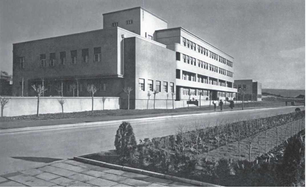
FIGURE 6.6. ANKARA İNÖNÜ GIRLS' INSTITUTE BUILDING BY SWISS ARCHITECT ERNST EGLI. COURTESY OF THE TURKISH HISTORICAL SOCIETY LIBRARY.
