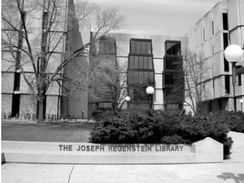
The Regenstein Library at the University of Chicago, our first Construction Management project involving federal government funds.
