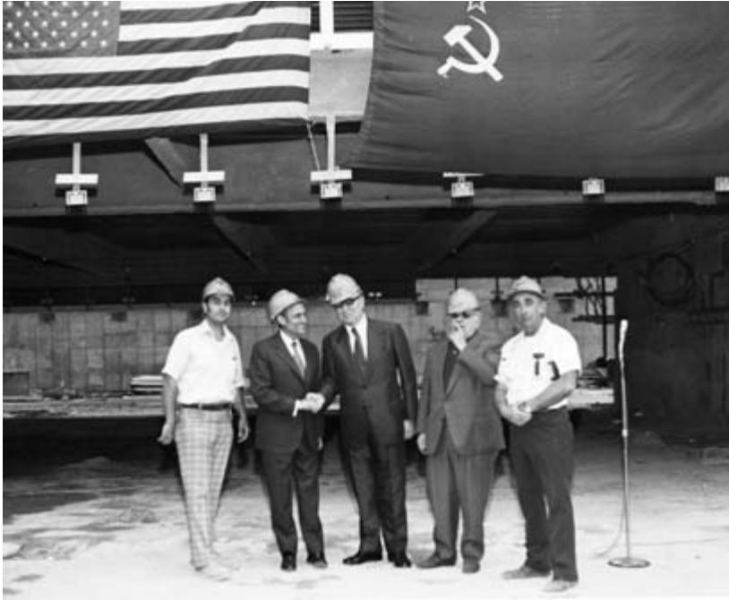
A topping-off ceremony for the Russian consulate in the Riverdale section of the Bronx.
