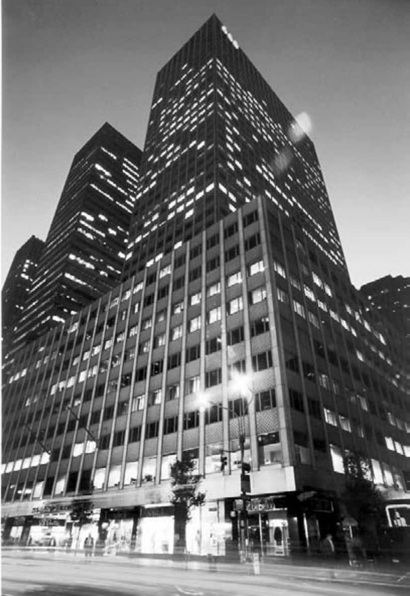
The Tishman Building, 666 Fifth Avenue, with its distinctive aluminum façade.
