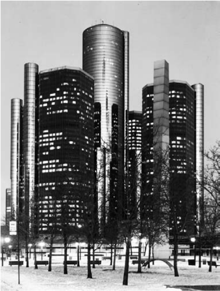
Renaissance Center in Detroit, on which we worked with Henry Ford, Jr. and architect John Portman.
