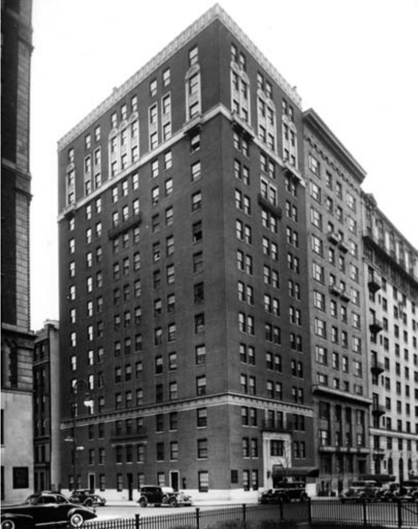
One of the early buildings constructed by Tishman Real Estate, 935 Park Avenue, in 1923.
