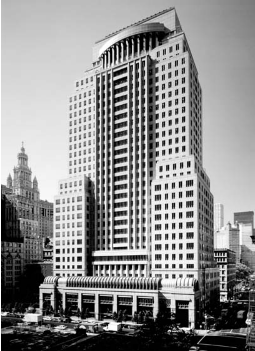
The Jacob Javits Federal Building in Foley Square, Manhattan, one of our many public-sector projects after we convinced the Public Buildings Service of the CM approach.
