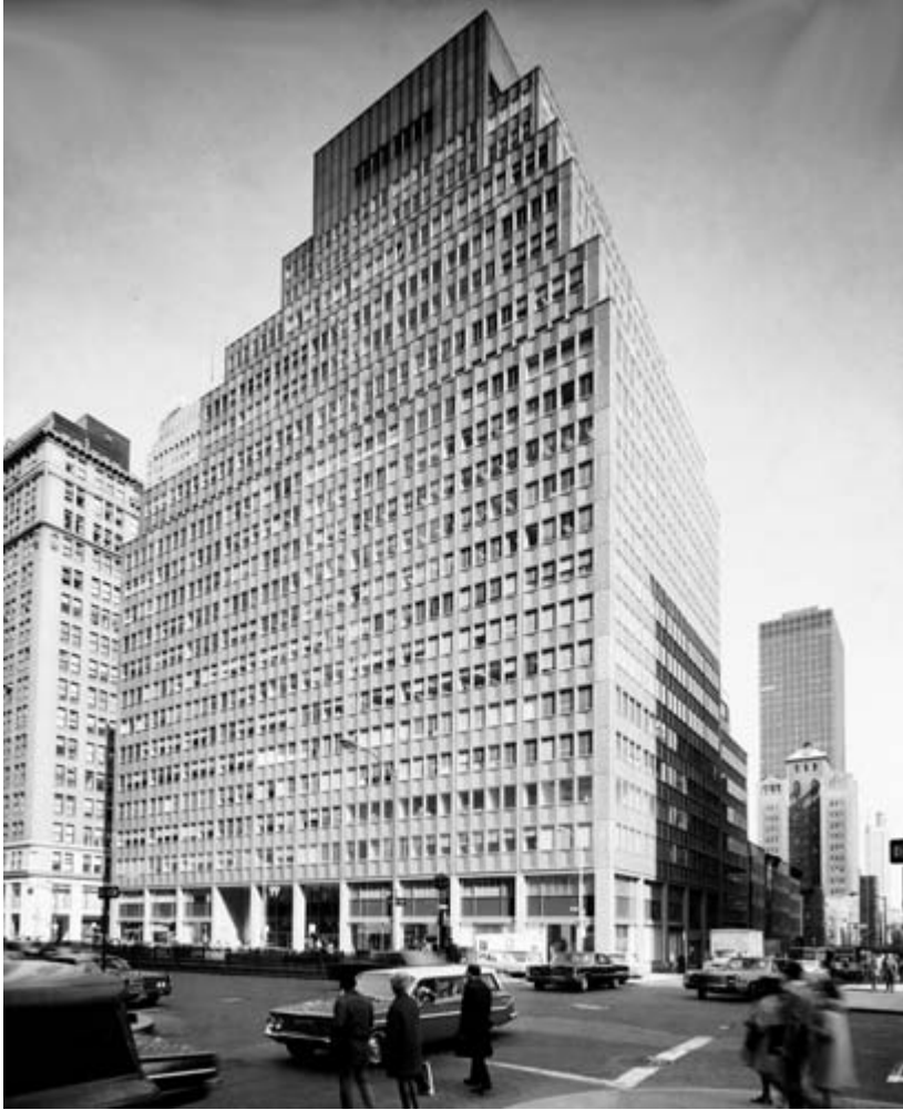
99 Park Avenue. Its all-aluminum façade was erected in just six days.
