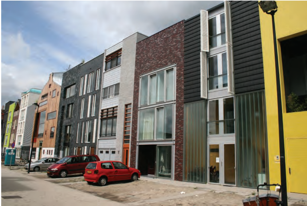
Colourful and diverse individual four-storey housing in IJburg.
