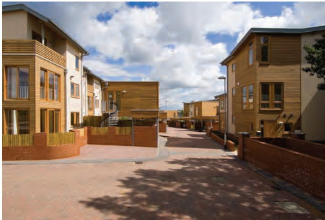
↑ The Summit House as new housing at Allerton Bywater, Leeds.
