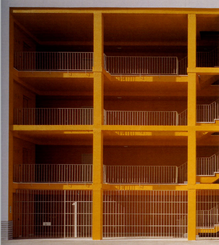
The eight portals are accessed from the patio, compulsory transitional space to and from the dwellings.
