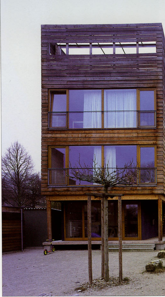
The housing blocks and community center (above) have been built with prefabricated wooden panels, a material chosen because it is inexpensive, energy efficient and sustainable.
