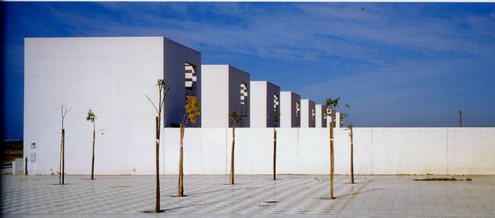
The living room and main bedroom open towards the street and the southeast, towards the plot's best views. The service area, kitchen and bathrooms are oriented toward the interior.
