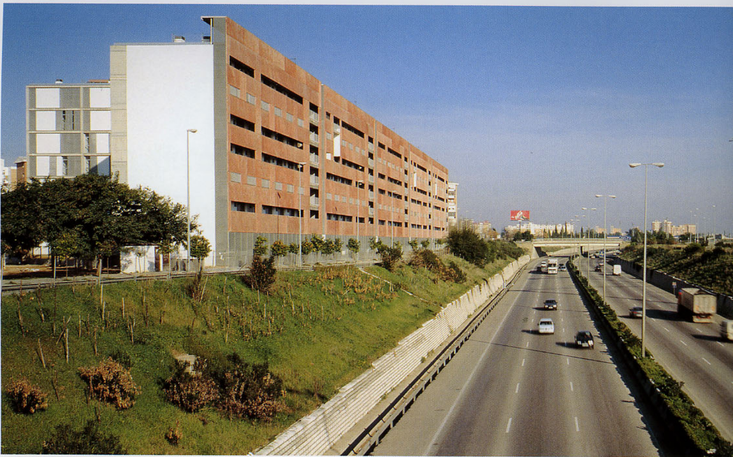
The new building has been conceived with a series of barriers facing the highway. A repetitive pattern perceived only at great speed due to small but continuous variations. The dwellings are shielded from the highway by five large volumes that act as acoustic barriers.
