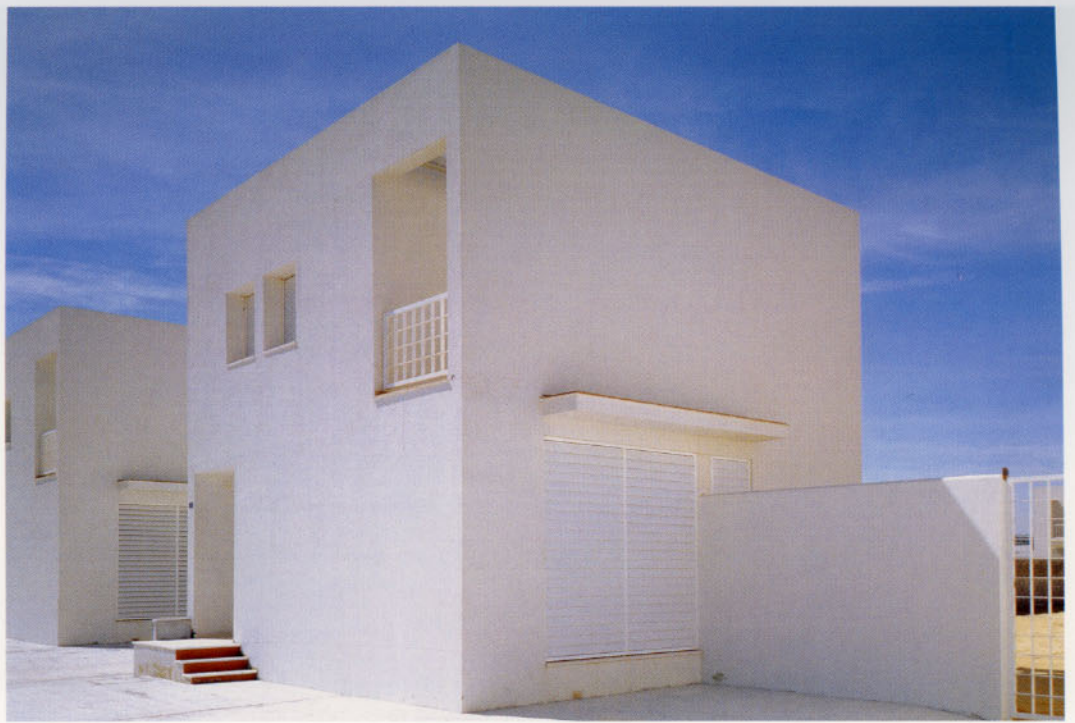
House is enclosed within a cube measuring 7.8 m on the sides.
