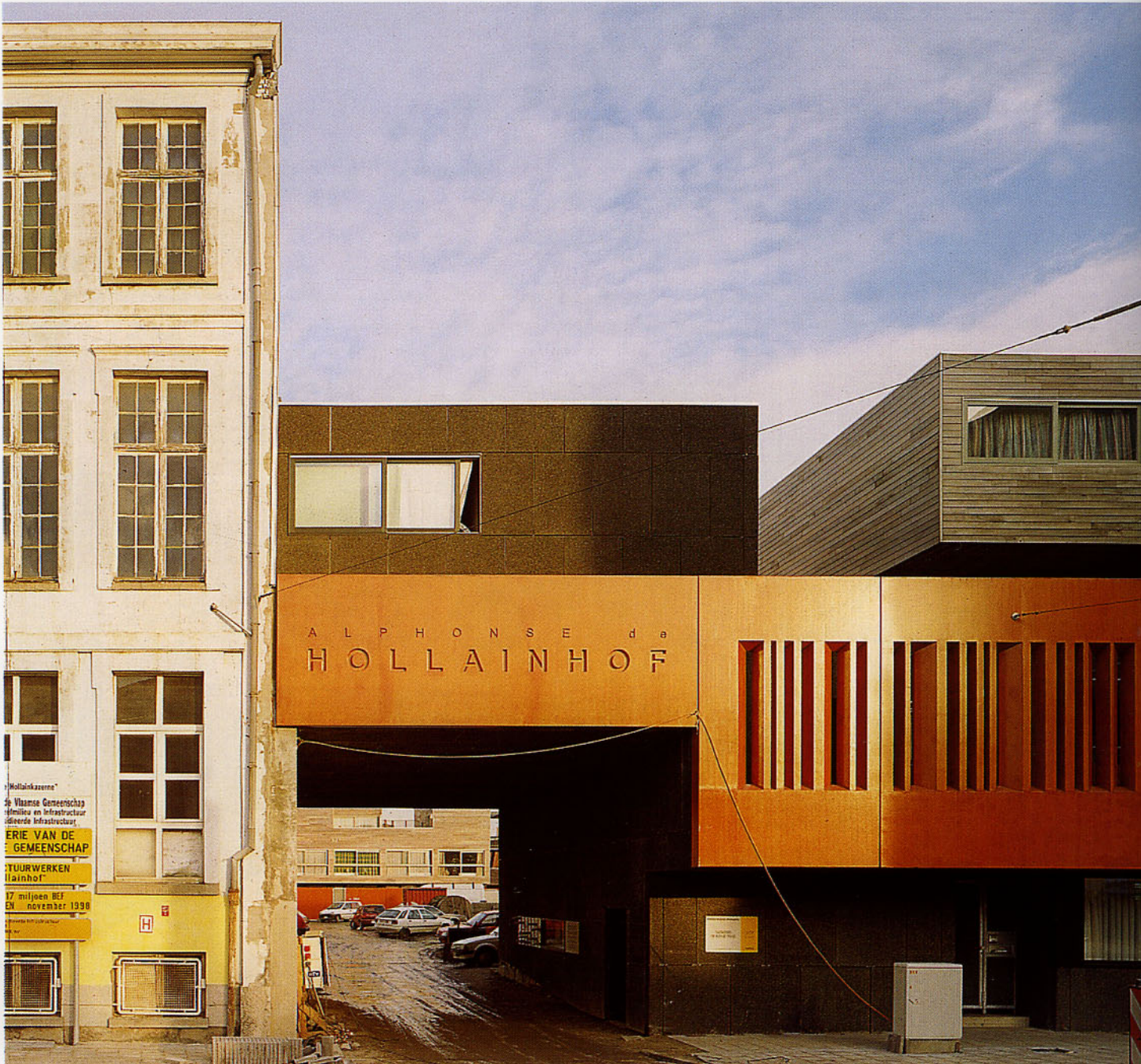
A large accessway at one end of the complex provides vehicular entry into the inner courtyard for the dwellings located alongside the river.
