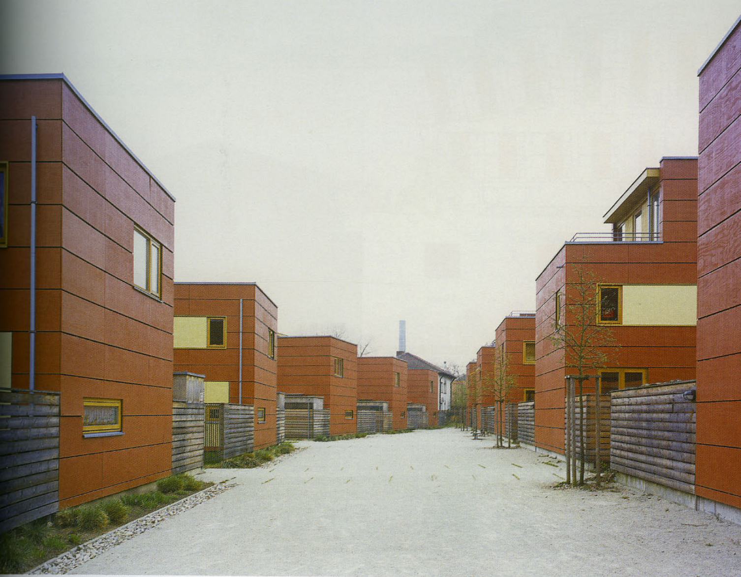
The search for privacy is reflected in the private patios and terraces as well as in the interstitial exterior spaces that create small squares and open-air leisure areas.
