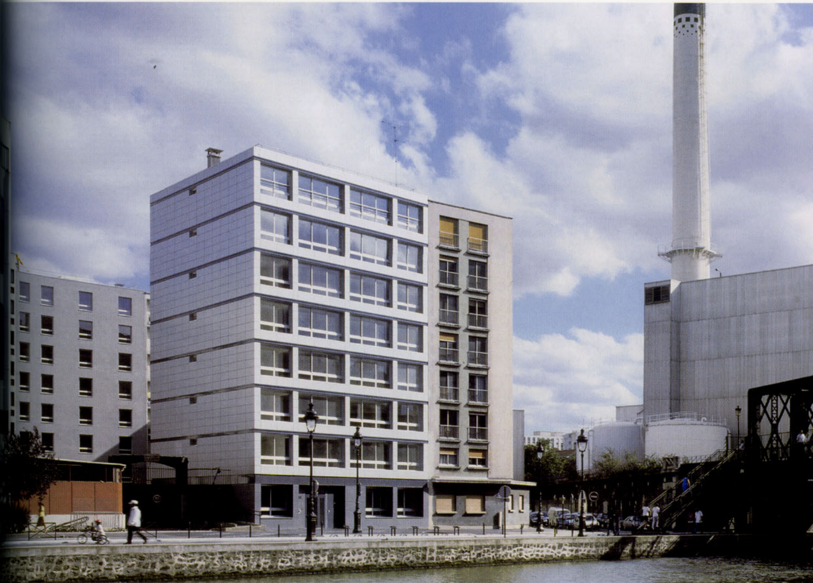
The narrow lot, measuring 13 by 68 meters, inspired the arrangement of two blocks and a spacious central garden courtyard. The double block visually distances itself from the traditional social housing image via large openings facing the canal.
