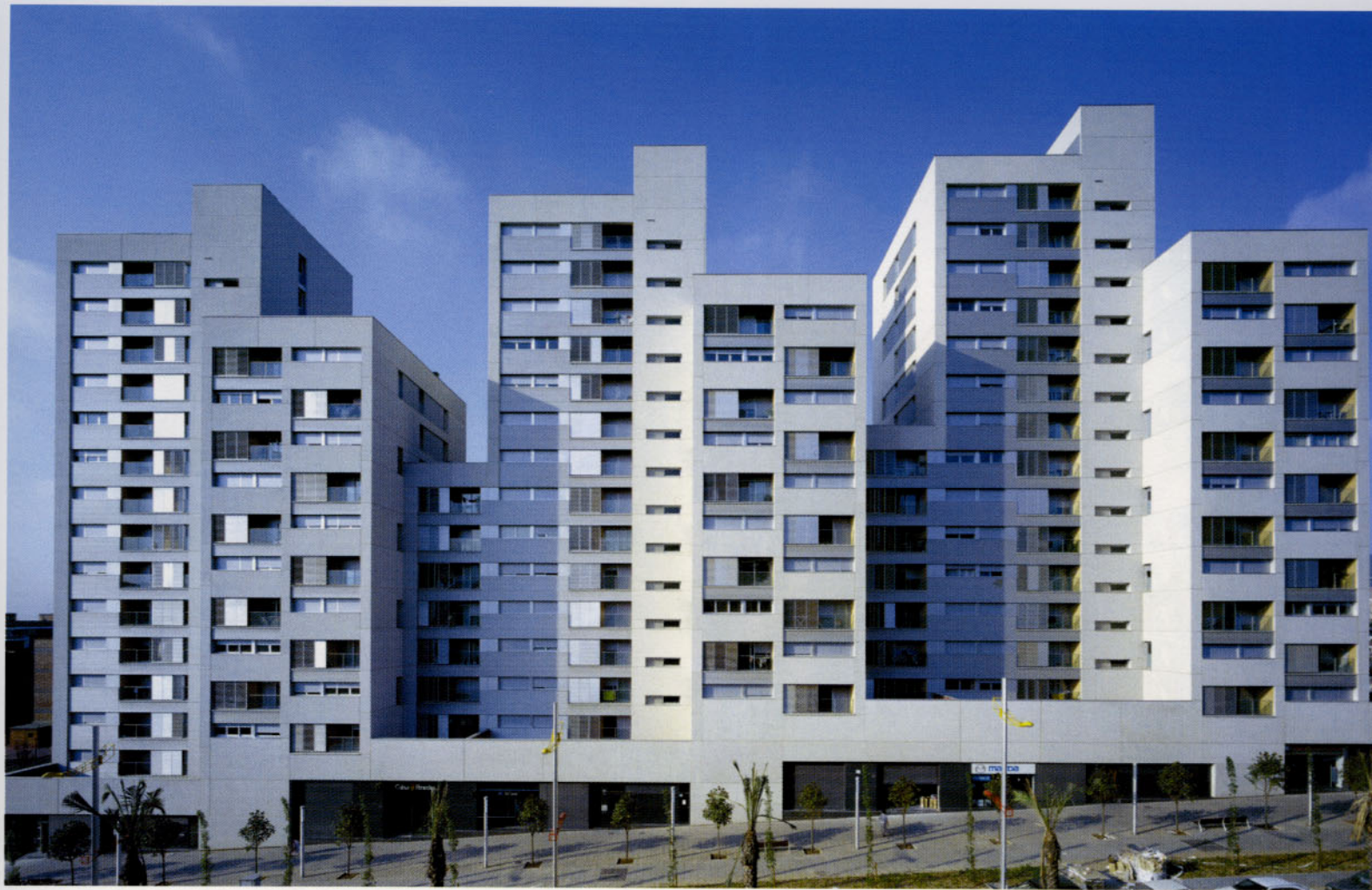
The complex forms a double relief in plan and volume rising from a continuous plinth intended for commercial activities. The building's relief is emphasized on the façade with the contrast between the GRC panels and corrugated aluminum panels of the cladding and the terrace's wide openings.
