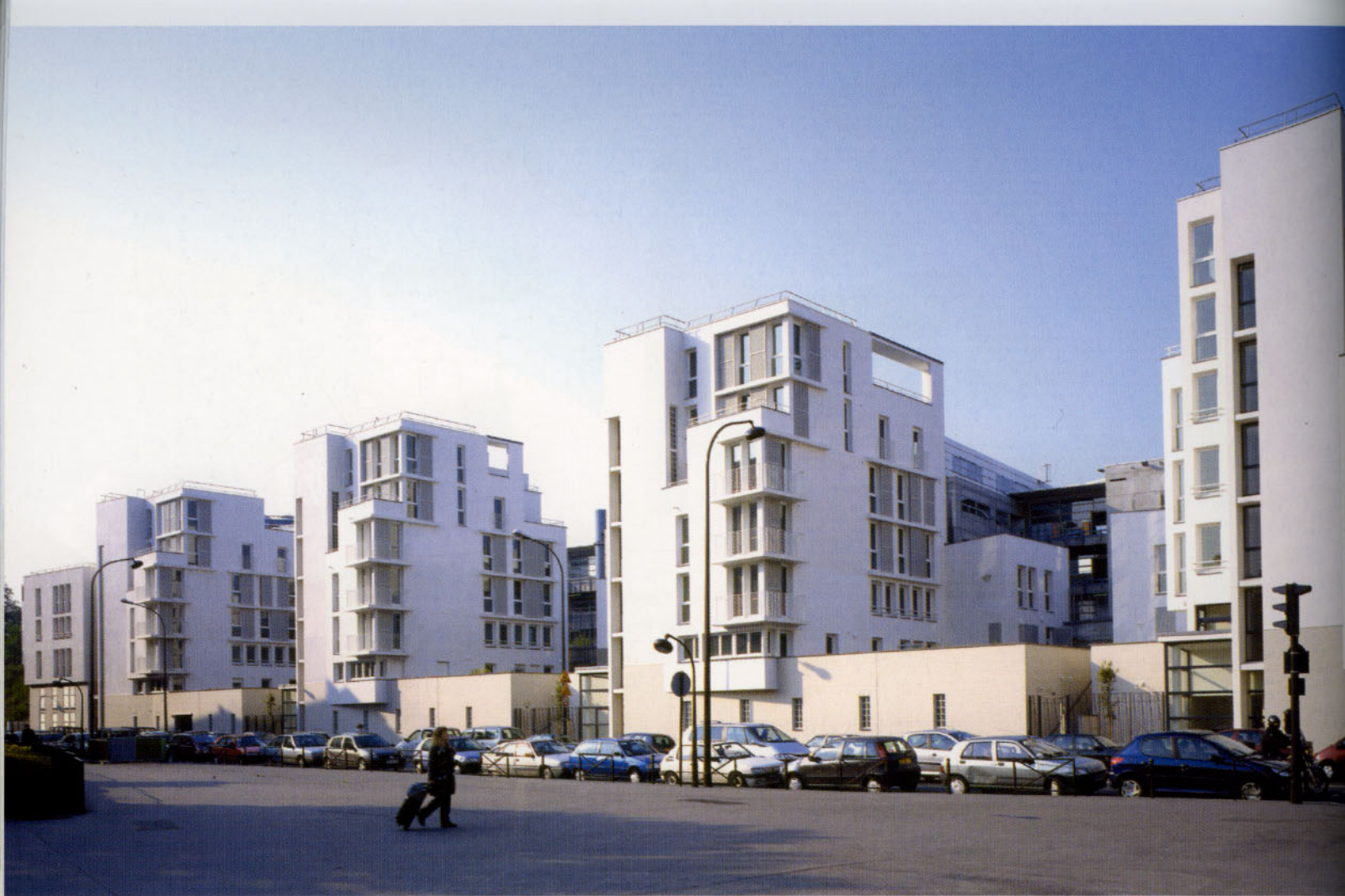
The project is composed of four housing blocks united on the ground floor by a continuous plinth that holds the parking space. The building is situated against a retaining wall that separates it from the railroad tracks.
