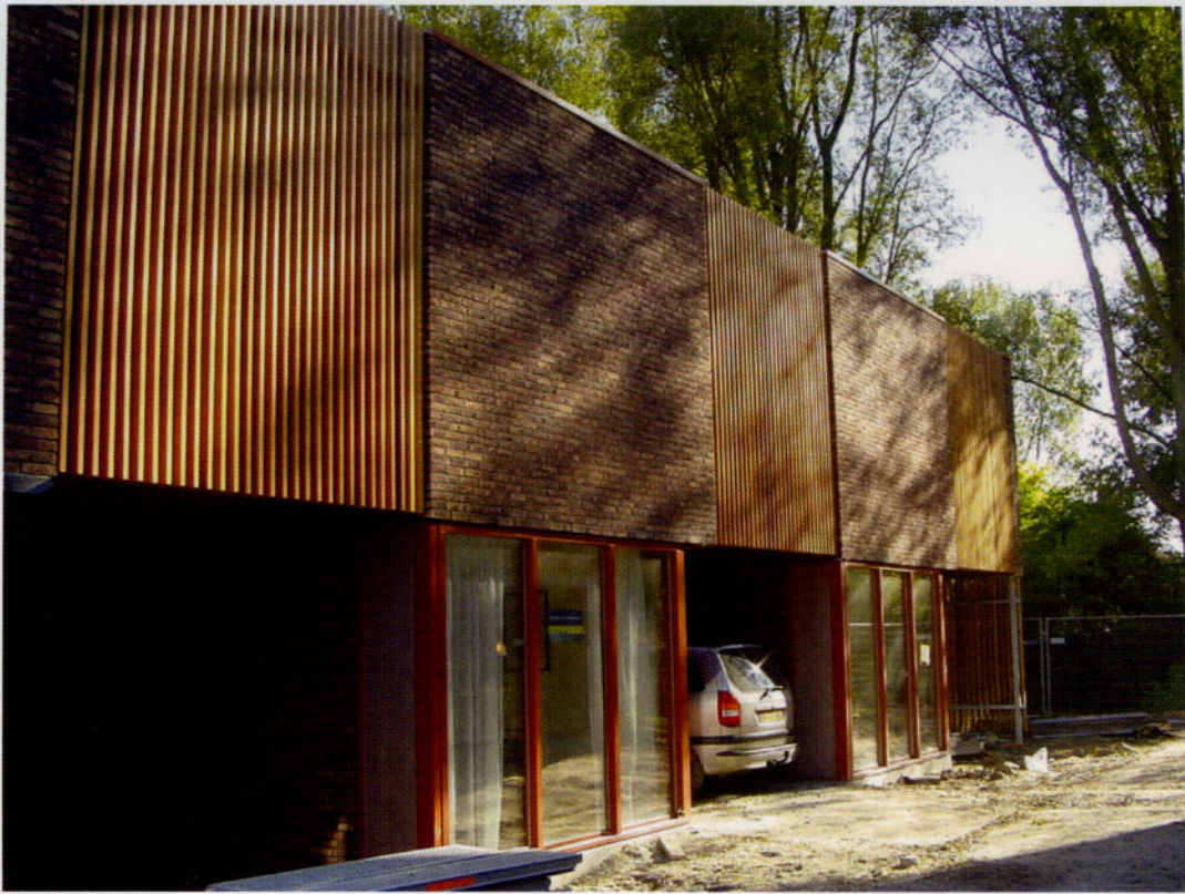
The single-family houses and the towers, independent at first sight, share the same façade materials and a common garage.
