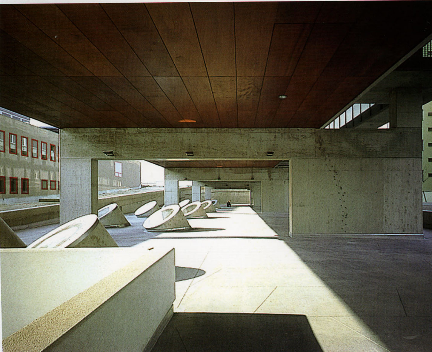
A series of skylights direct natural light to the underground floors.
