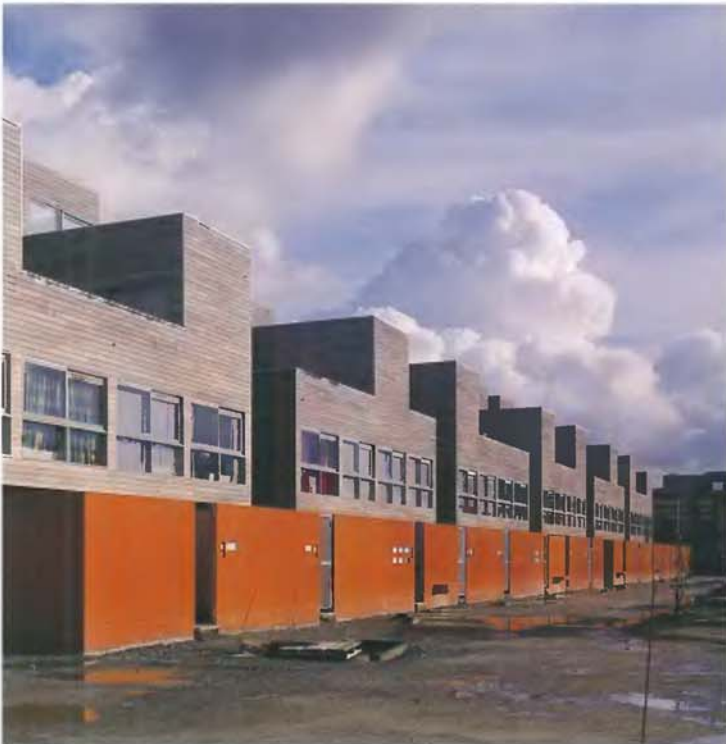
The cedar wood used in the upper part will gradually turn grey, contrasting with the terracotta colour of the prefabricated concrete walls that close the private courtyards.
