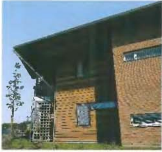
The buildings that form the housing complex were built using large structures of red sequoia wood treated with special oils for weather-resistance.
