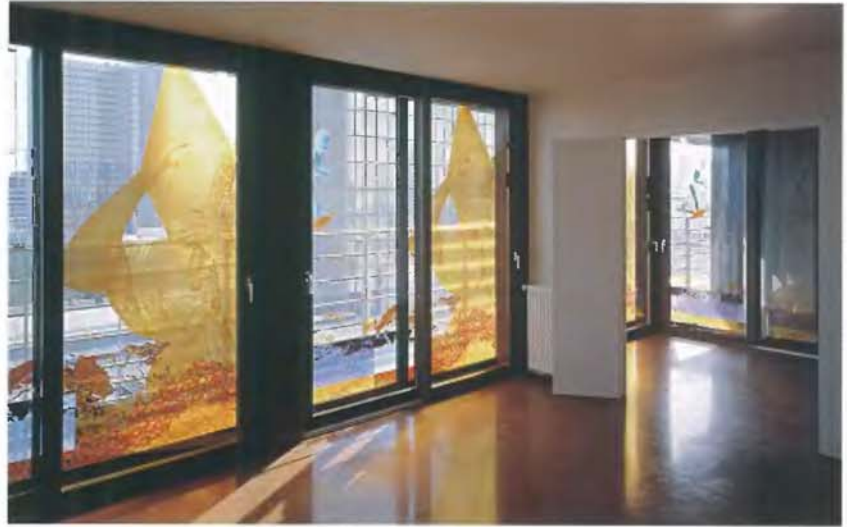
The accumulation of frescos allows the incoming natural light to be filtered, creating an appropriate atmosphere of intimacy in the interior spaces without the need for other types of filters.
