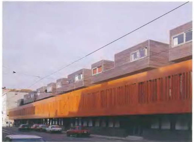
The cedar wood used in the upper part will gradually turn grey, contrasting with the terracotta colour of the prefabricated concrete walls that close the private courtyards.
