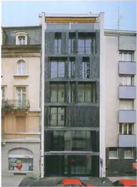
Front view of the main facade, characterised by the unusual cast iron curtain, which as it sways endows the whole scene with fluidity and dynamism. The detail below shows how the individual links of the curtain are joined together.
