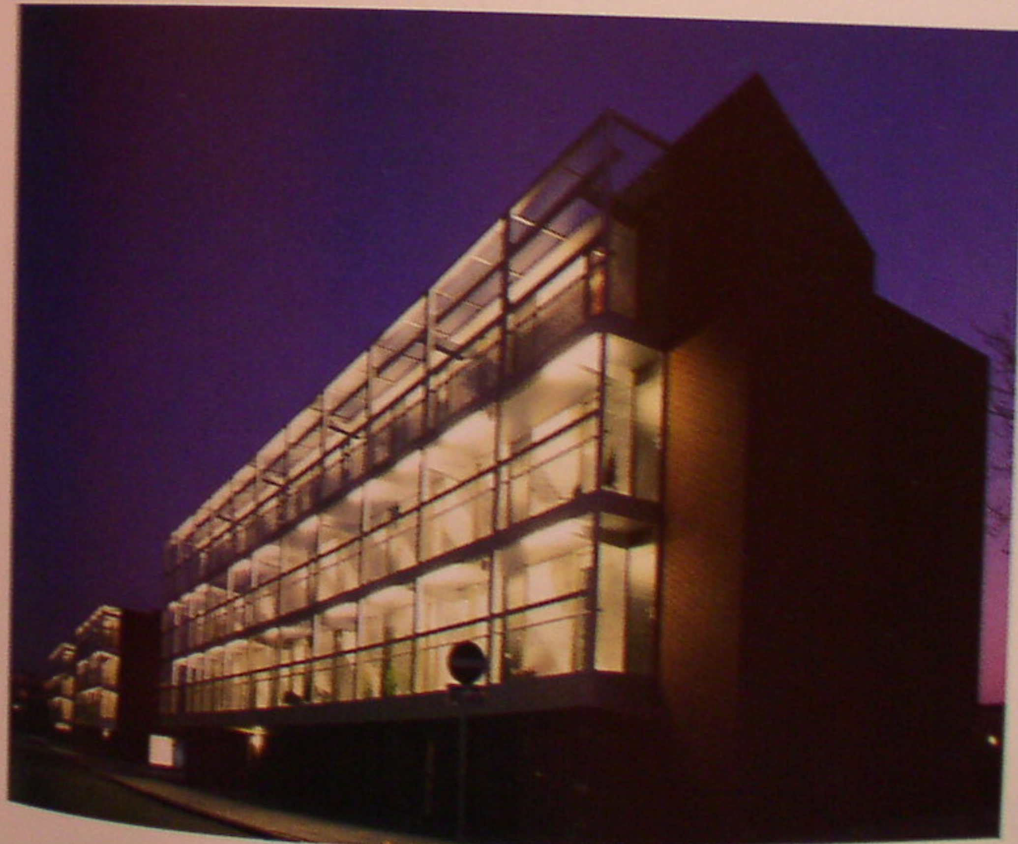
The glass galleries that give access to the dwellings facilitate and temper the transition between public and private spaces.
