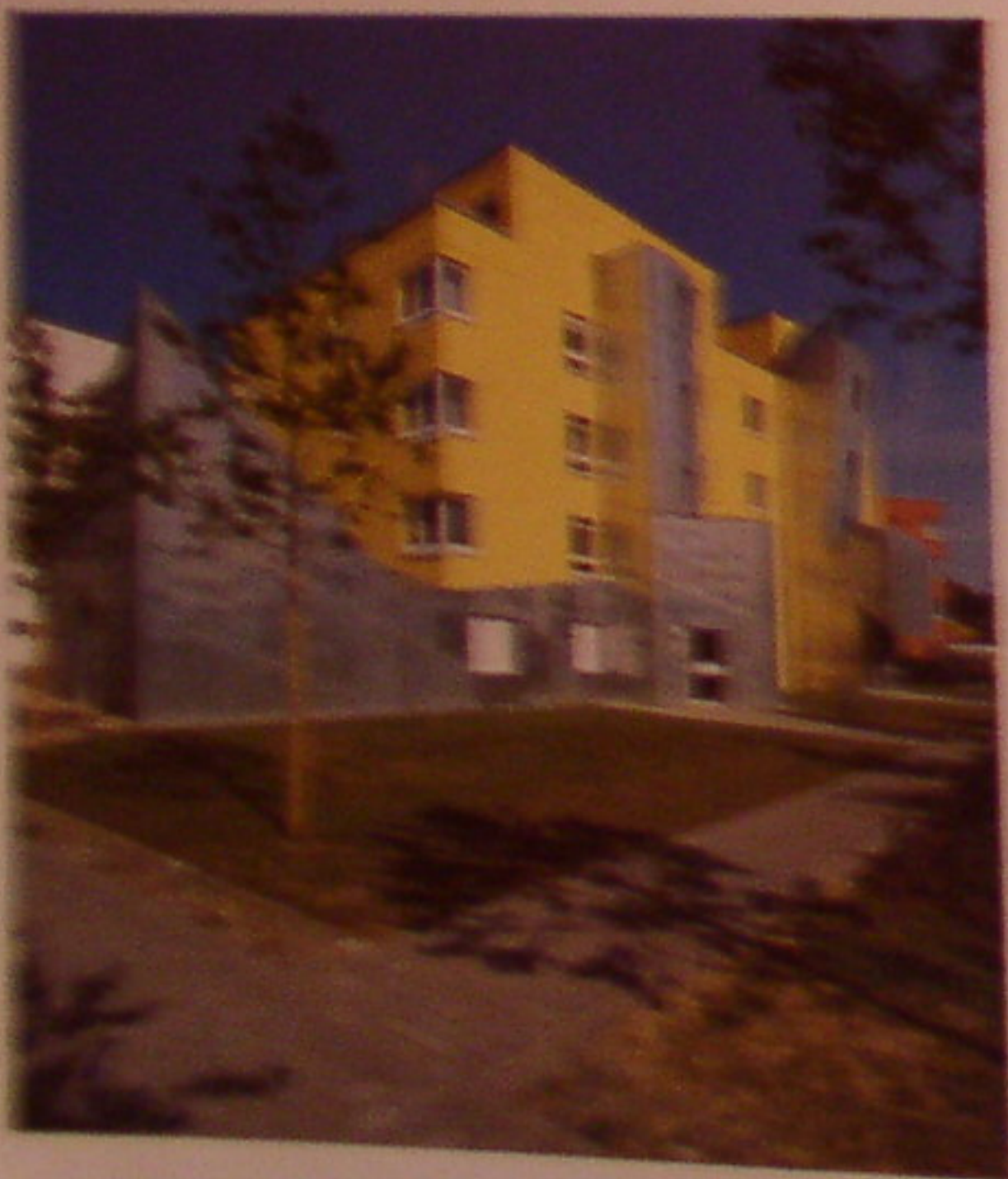
The building aesthetic is derived through the building forms that emphasize volume, mass, porches and balconies. These forms are emphasized with arc panels while boldly coloured plaster facades comprise the major surface material.
