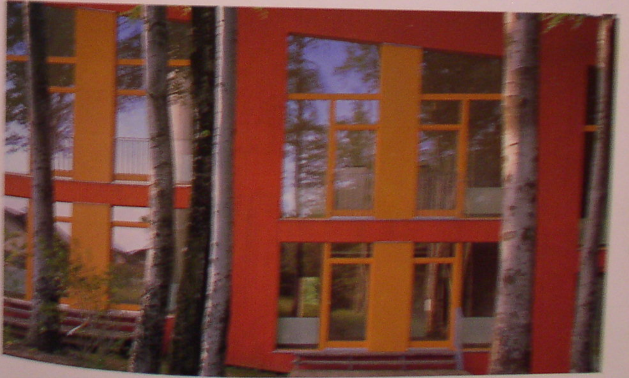
Both the position of the building and the layout of the exterior walls to make the most of the natural sunlight, wind energy. The living areas and bedrooms receive sunlight from their elevation along the southern slope of the elongated volume. On the northern side are the kitchen, bedrooms and smaller facilities, and the rear side of a long communal space which serves as a thermal curtain for the apartments.
