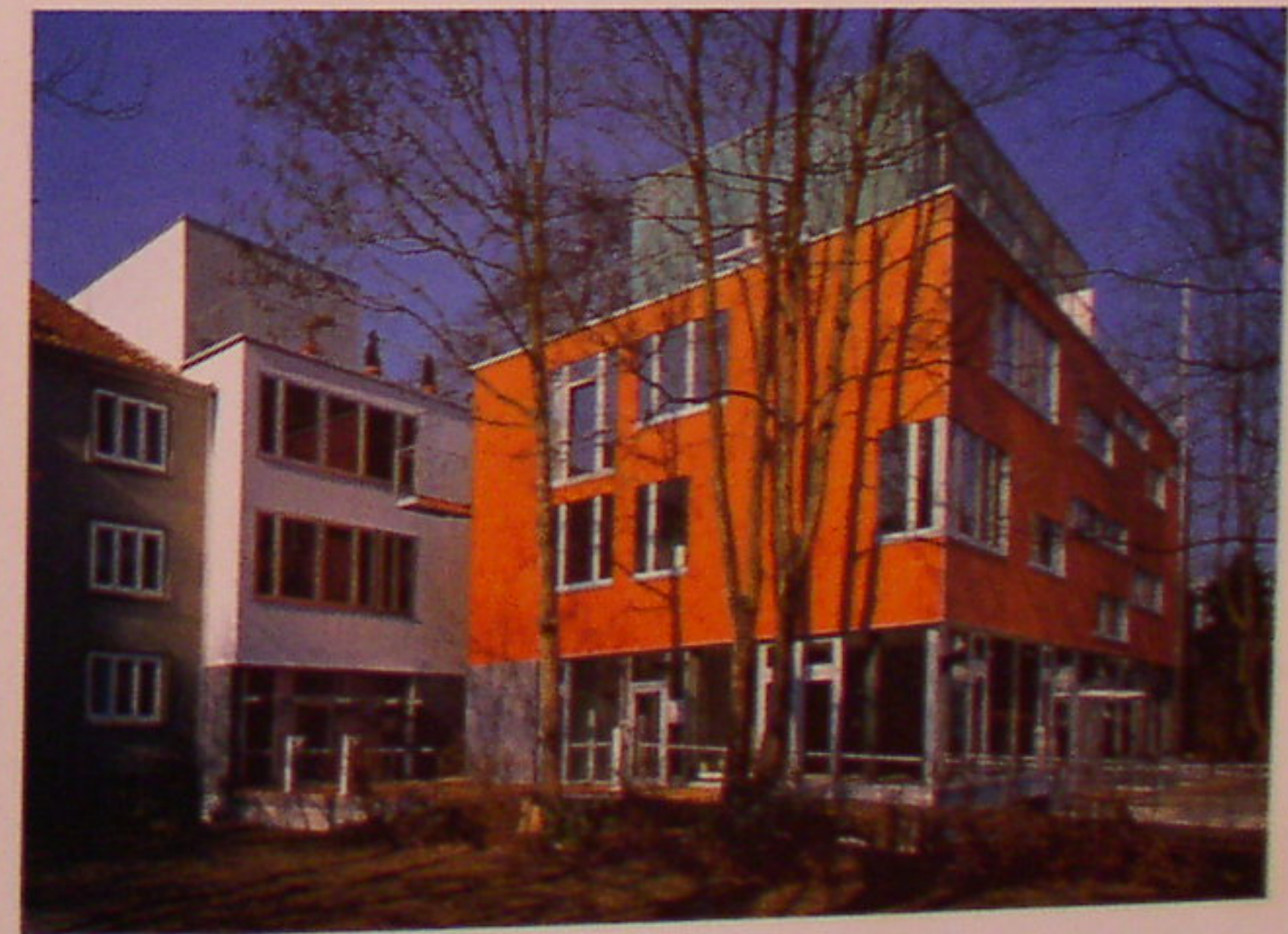
The front volume, with its completely glazed ground floor, was clad with red spruce boards in vertical strips. The absence of horizontal joints avoids deterioration due to damp.
