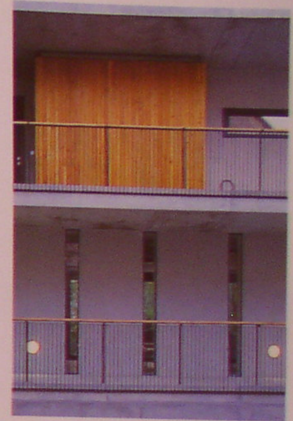
As can be seen in the photograph on the left, the west facade filters the incoming light by means of a system of sliding panels of perforated metal.
