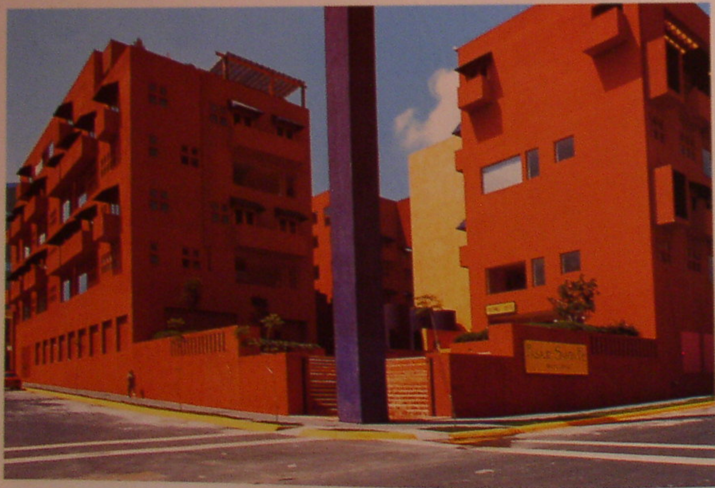
The buildings are developed around interior atriums with small gardens. The apartments have two levels with spaces of double height.
