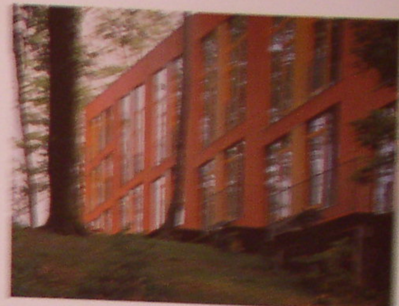
Both the position of the building and the layout of the exterior walls to make the most of the natural sunlight, wind energy. The living areas and bedrooms receive sunlight from their elevation along the southern slope of the elongated volume. On the northern side are the kitchen, bedrooms and smaller facilities, and the rear side of a long communal space which serves as a thermal curtain for the apartments.
