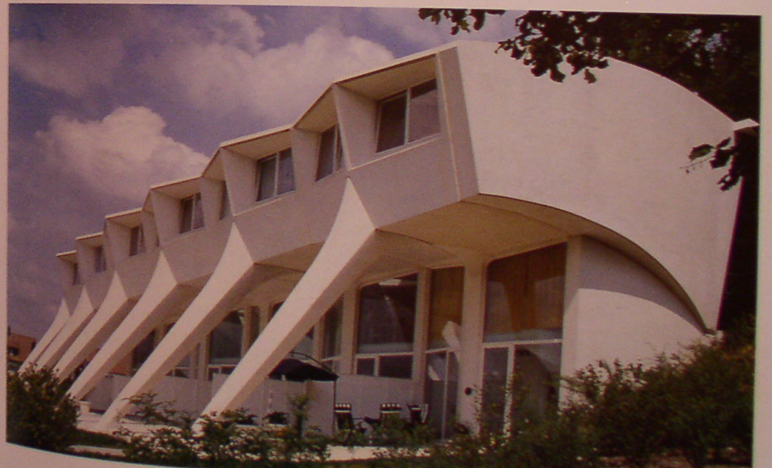
The complex, built mainly in concrete, runs parallel to the main road. The outer walls are made of prefabricated concrete elements.
