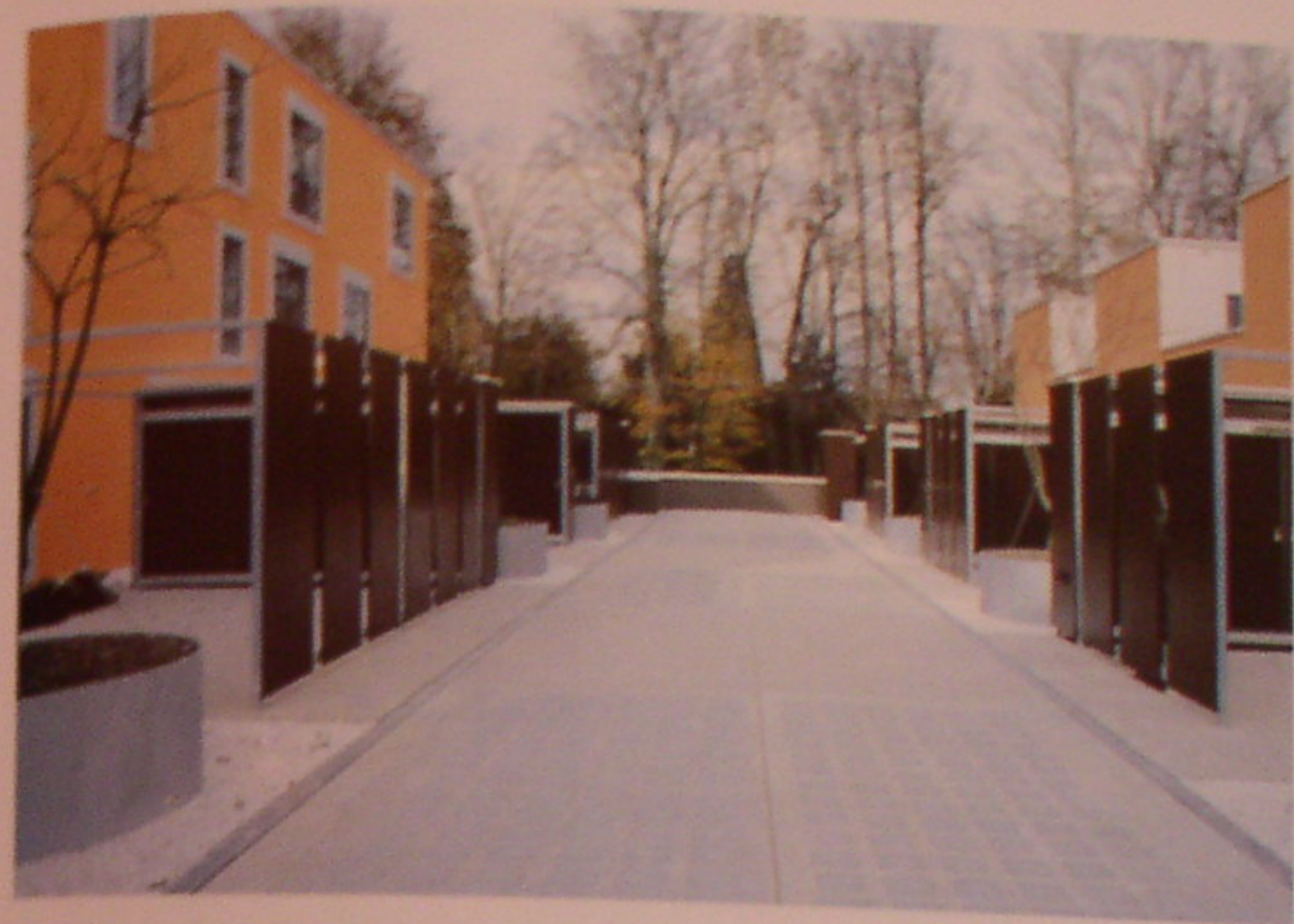
The inner courtyard is organized by means of semi-public spaces in front of the dwellings built with a metal frame and plywood boards. In the photographs below we can see the strong contrast between the dark brown colour of the metal facade and the orange colour of the facades that look onto the inner courtyard.
