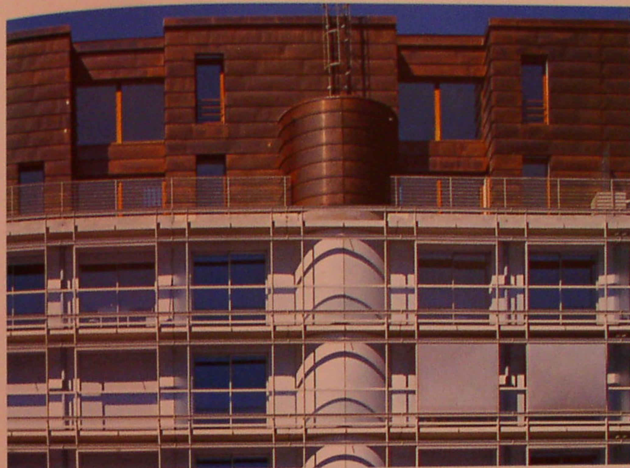
The facing page shows a front view of the facade of the complex facing the River Vilaine, with the small existing building between the two new volumes. The new volumes have six levels of single-floor dwellings and a double height area at the top housing twelve small duplex apartments that are expressed on the exterior in geometric elements clad with copper plate surrounded by balconies.
