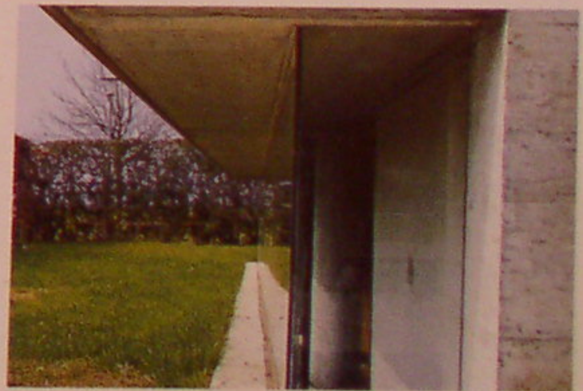
On both the outside and inside of the building there is a predominant use of exposed reinforced concrete and metal frames. These materials seem to glow thanks to the light flowing in from the skylight at the top of the staircase.
