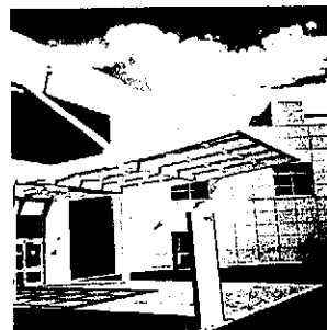
Figure 4.5 For maximum visibility and minimal confusion, modern hospitals often make the entrance an important landmark with elements such as a canopy
