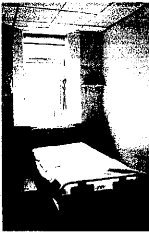
Figure 3.7 Splayed reveals surrounding windows can control sky glare by reducing the contrast between window and wall
