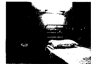
Figure 4.63 The bedhead luminaire can give combined uplighting and downlighting
