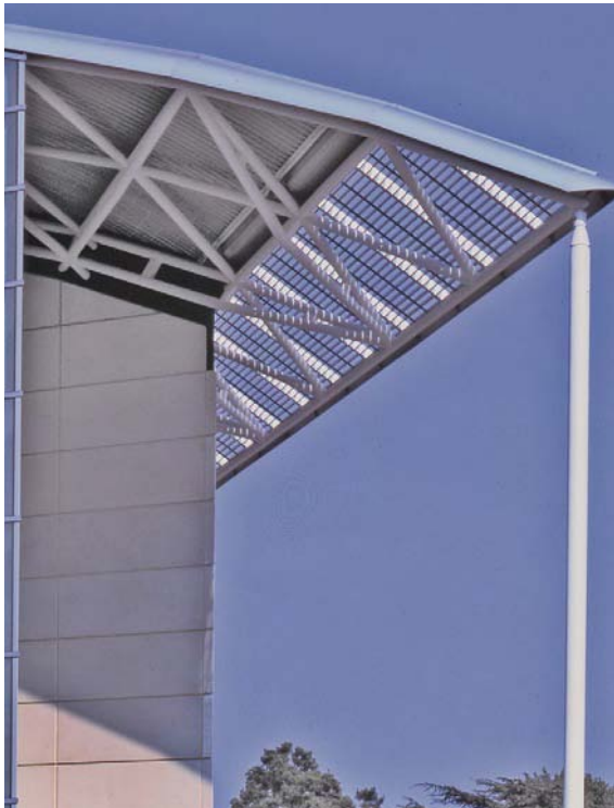
Combined daylight canopy and shading screen used at the Law Library, University of Cambridge. Designed by Foster and Partners. (Dennis Gilbert/View)
