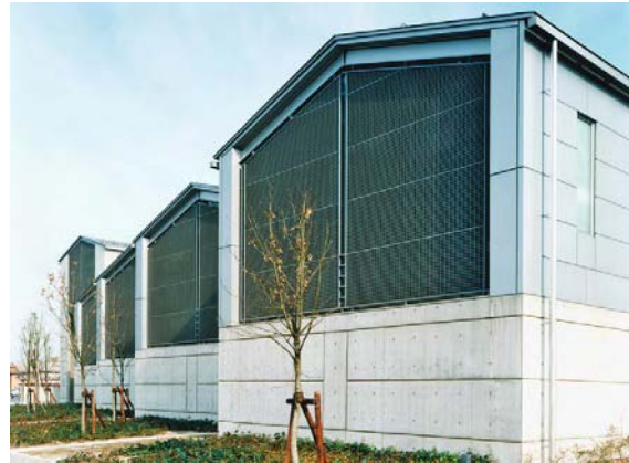
Daylight and security screens used at Hirata Public Library, Japan. Note the use of trees to provide further solar shading. (Teramoto Architects)
