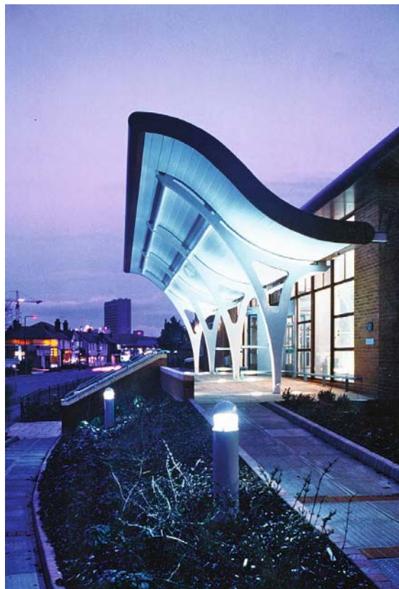
Distinctive entrance canopy at the Surrey History Centre Library, Woking. (W S Atkins)
