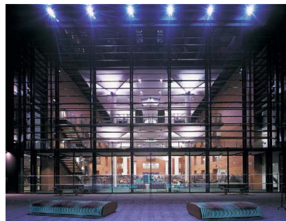
Night-time view of Brighton Public Library. The building glows at night like the adjoining retail development. (Bennetts Associates)
