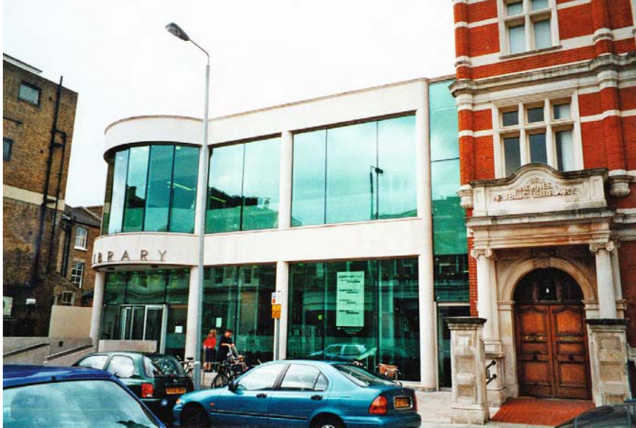
A modern wing attached to Putney Public Library to accommodate IT. (Biddy Fisher)
