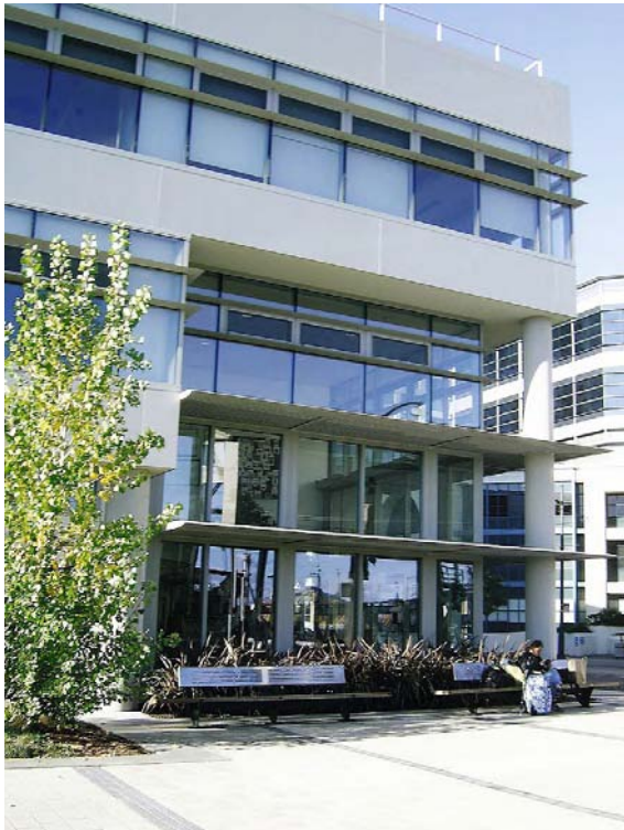
External seating at San Francisco Public Library. (Brian Edwards)
