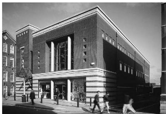
St George's Library in Sheffield, designed by Building Design Partnership, is a useful symbol of regeneration. (Roy Wooding/ICS)
