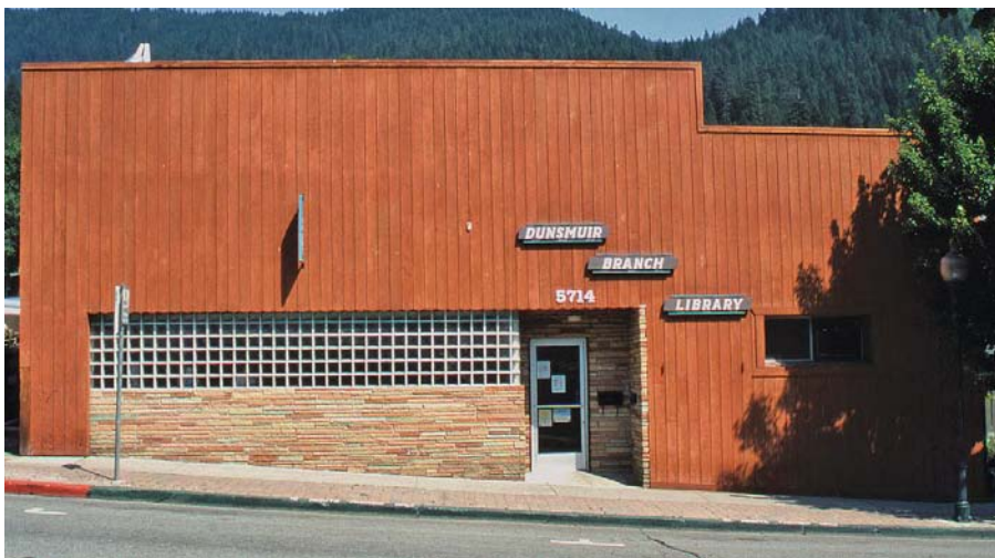
The branch library in the small town of Dunsmuir in California, built in 1964, uses materials from nearby forests in its construction, controls glare without loss of daylight levels, has its own bus stop and set down area for staff and users, and a simple library name sign. (Brian Edwards)
