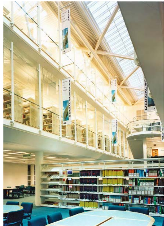
Low-energy library which maximizes daylight and natural ventilation. University of Hertfordshire Library, designed by Architects Co. Partnership. (Forster Ecospace)
