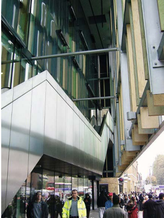
The Idea Store in Whitechapel, London is designed to be part of local street culture. (Brian Edwards)
