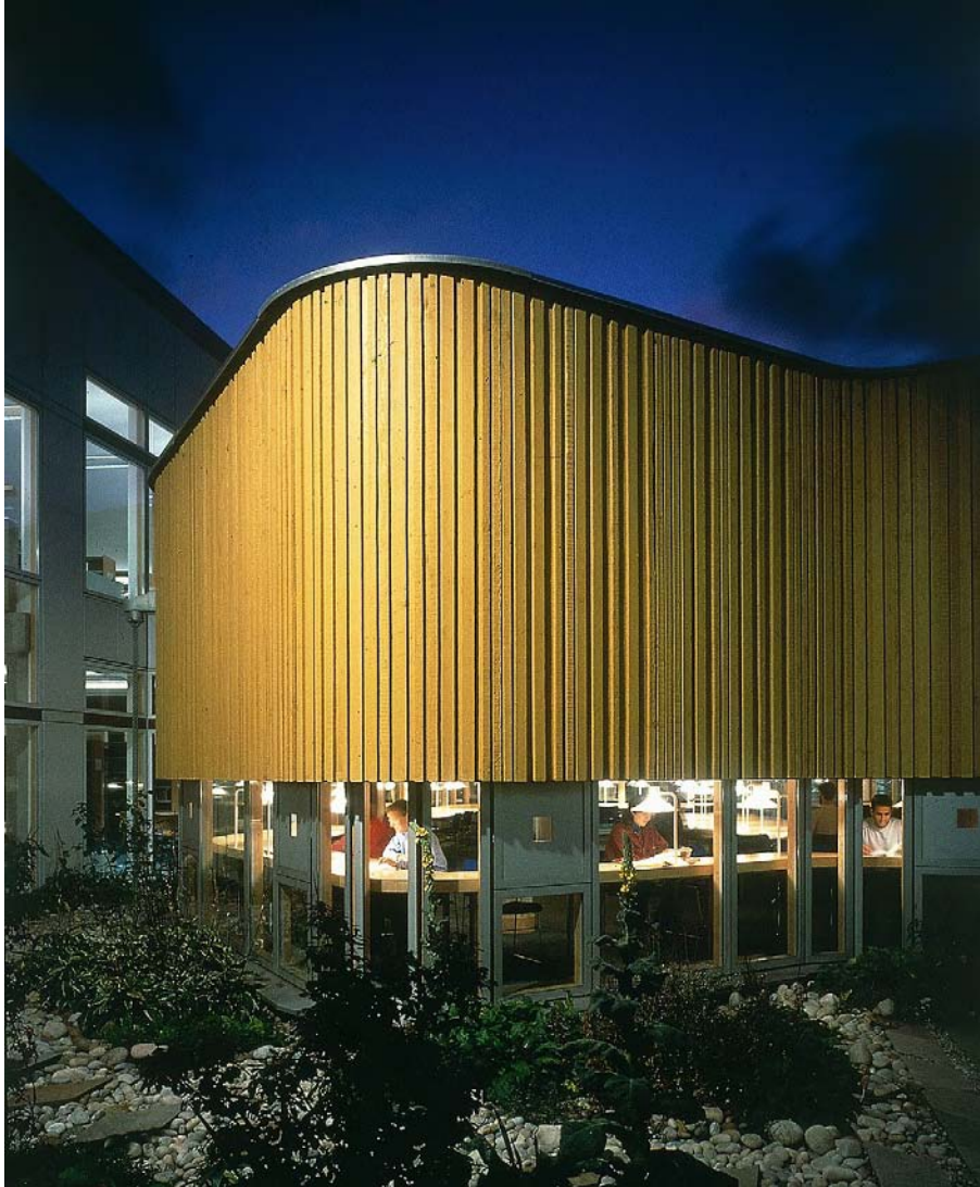
Catherine Cookson Reading Room, University of Sunderland, designed by Building Design Partnership. (M Hamilton-Knight)
