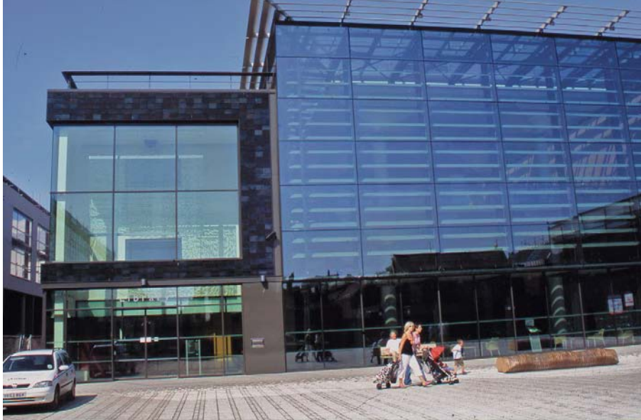
Brighton Public Library signals the importance of the library as an expression of democratic space – a place for people to meet as well as read. (Bennetts Associates, Brian Edwards)
