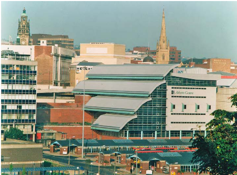
New typological adjustment for the library. Adsetts Centre, Sheffield Hallam University, Designed by Faulkner Brown Architects. (Sheffield Hallam University)
