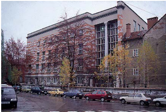
National and University Library of Slovenia built in Ljubljana in 1936 to designs by Joze Plecnik. (Anon)
