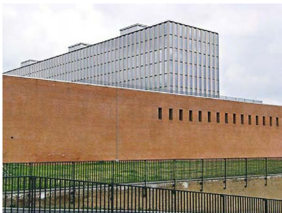
Extensions to the National Library of Italy showing the recent book deposit and administration/research tower. (Brian Edwards)
