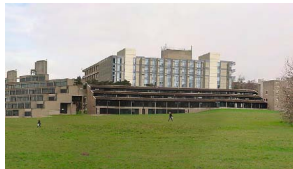
Future phase in context, University of East Anglia: CAD modelling of the extensions to the library at the University of East Anglia. (Shepherd Epstein Hunter)
