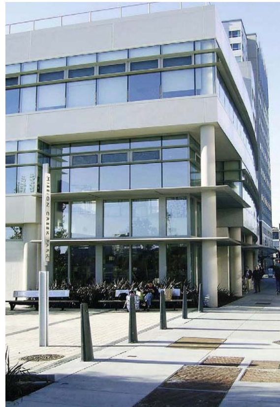
Mission Bay Public Library, San Francisco. Notice the small square and seats provided at the library entrance. (Brian Edwards)
