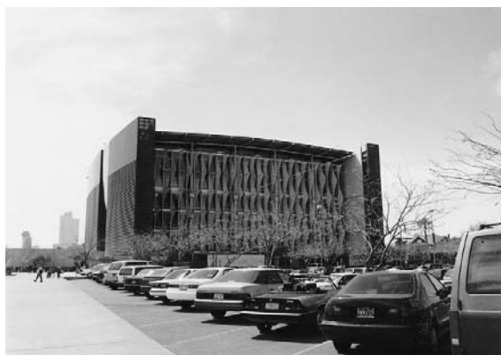
In hot climates, air-conditioning is often unavoidable but libraries can incorporate external shading to reduce energy loads. Phoenix Public Library designed by Will Bruder. (Andrew North)
