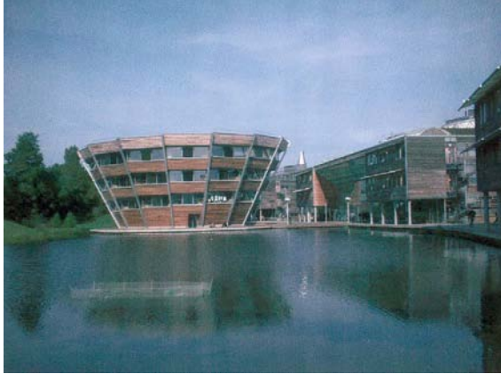
The library at the Jubilee campus, University of Nottingham, is a building to visit in its own right. Architect Michael Hopkins and Partners. (M Hamilton-Knight)
