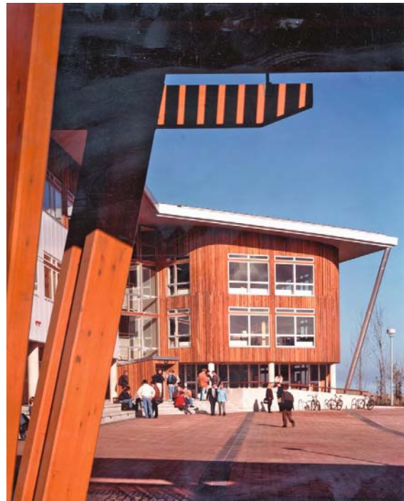
'Green' Library and Learning Resource Centre at Sunderland University. Designed by Building Design Partnership. (M Hamilton-Knight)
