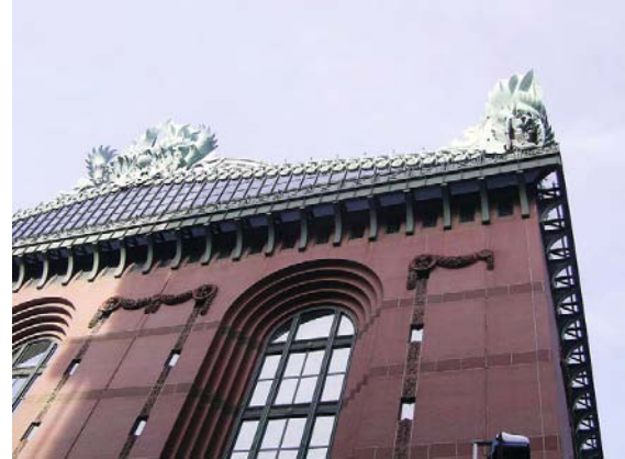
Detail of façade sculpture at Chicago Public Library. (Brian Edwards)
