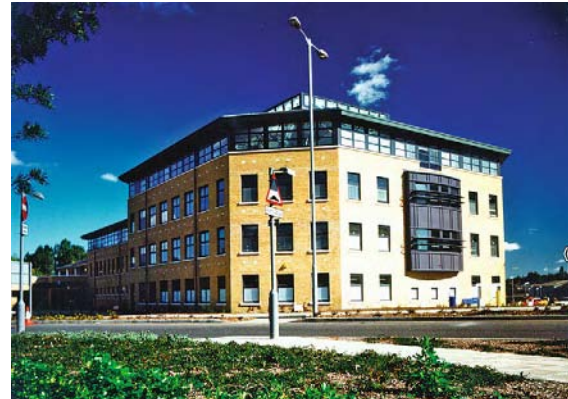
Learning Resource Centre, Anglia Ruskin University, designed by ECD Architects. (Anglia Ruskin University)
