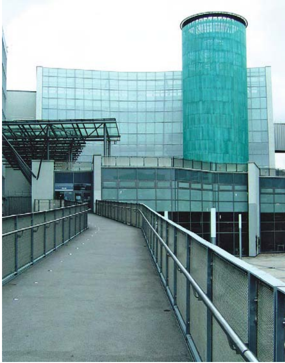
The elevated student entrance to the Saltire Centre at Glasgow Caledonia University signals the distinction between public and private access to the library. (Brian Edwards)
