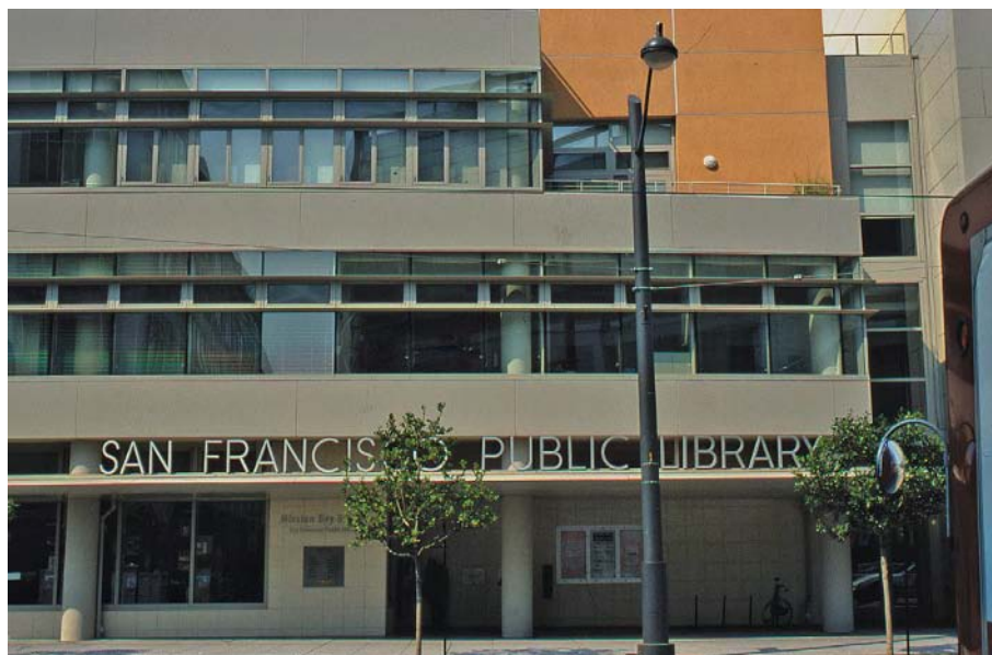
A strong street presence is needed for today's libraries as here at San Francisco Public Library. (Brian Edwards)
