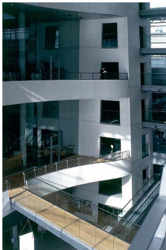
Atrium in the new wing of the Royal Library of Denmark, designed by Schmidt, Hammer and Lassen. (Fotografisk Atelier, Det Kongelige Bibliotek)
