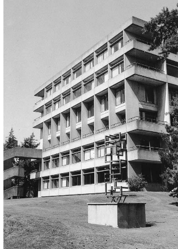
The modernist library designed by Denys Lasdun at the University of East Anglia expresses ‘libraryness’ through measured monumentality. (Brian Edwards)
