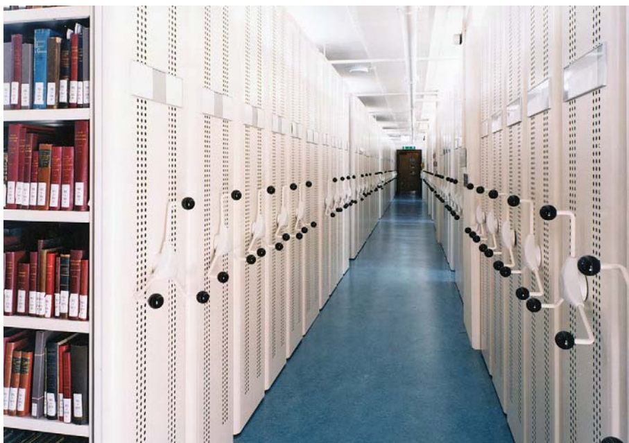
Compact mobile storage at Cambridge University Library. Note the perforations for ventilation. (Forster Ecospace)
