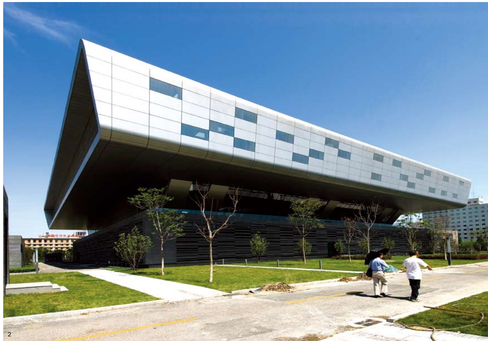
1. Aerial view 2. Back view 3. Façade detail
