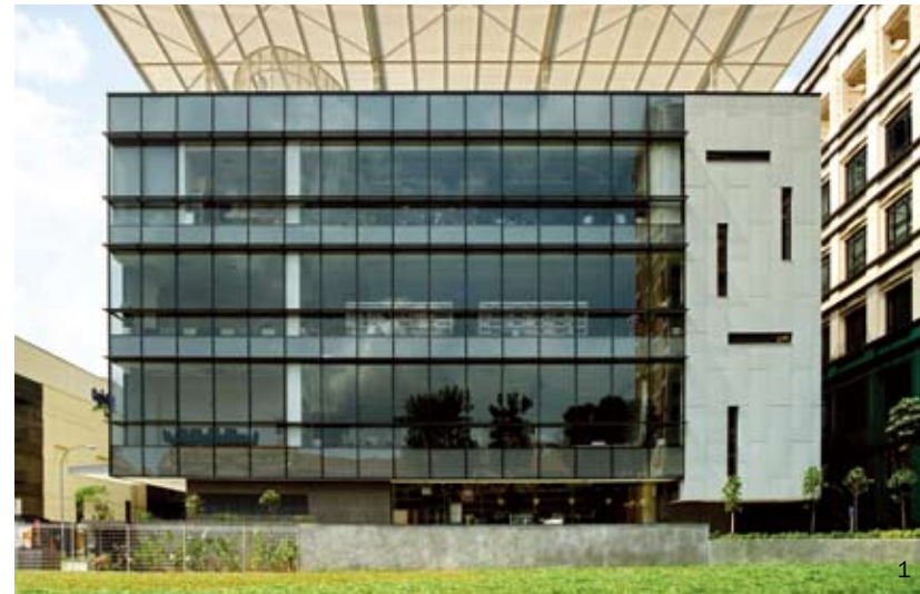
1. Side view 2. "Pods" cantilevered off the main building façade 3. Front view
