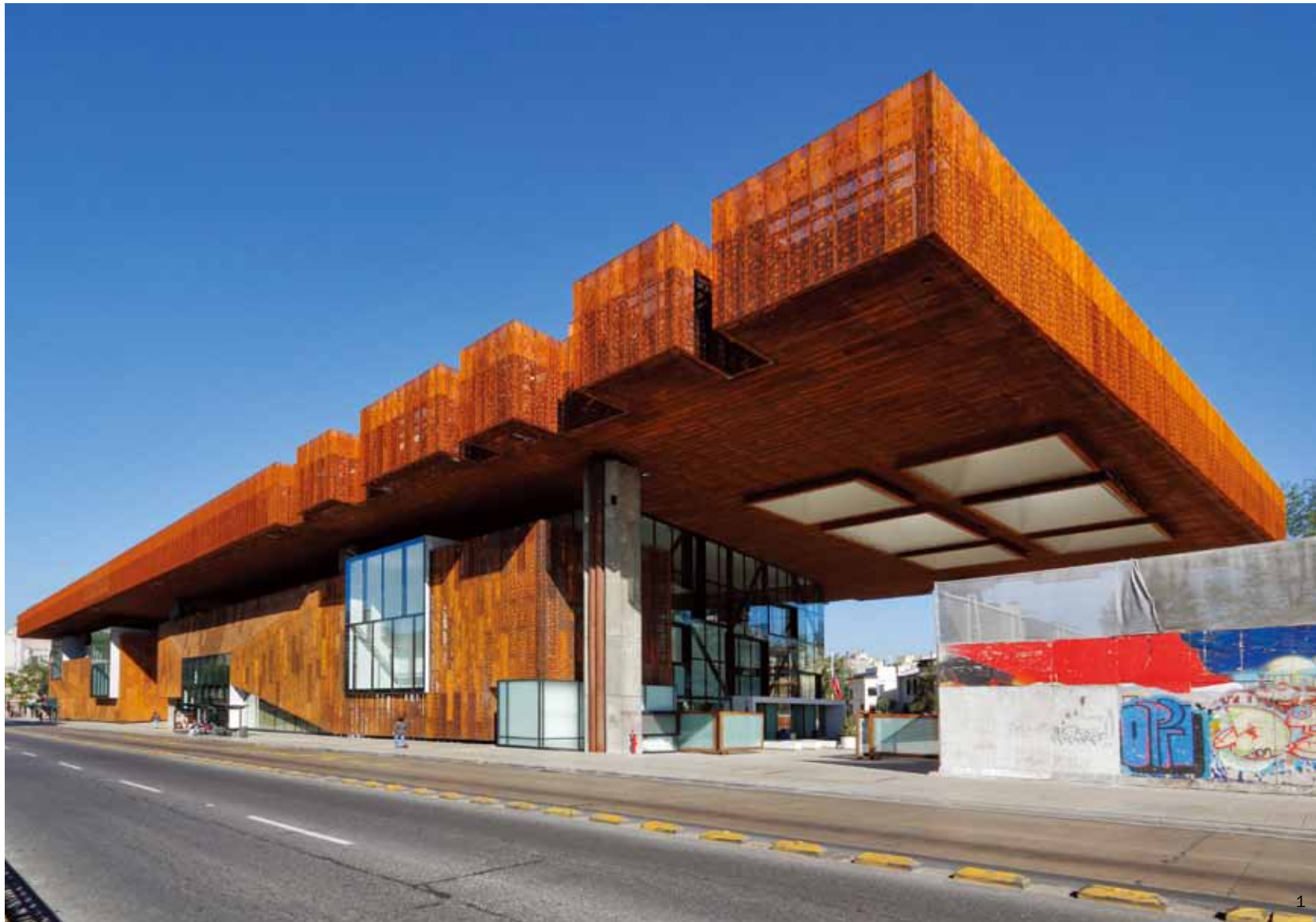
1. Weathering steel (with holes) creates special façade for the cultural centre 2. Lounge behind weathering steel (with holes) façade
