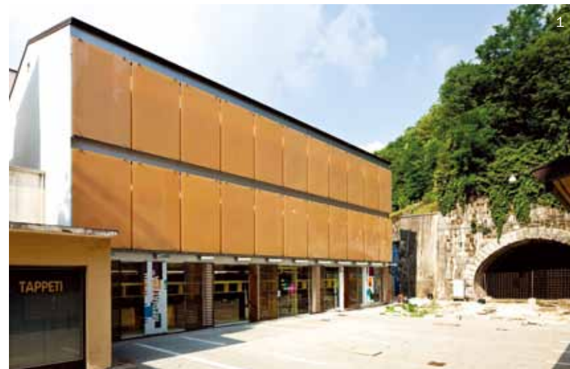
1.3. Side view of the building 2. Front view
