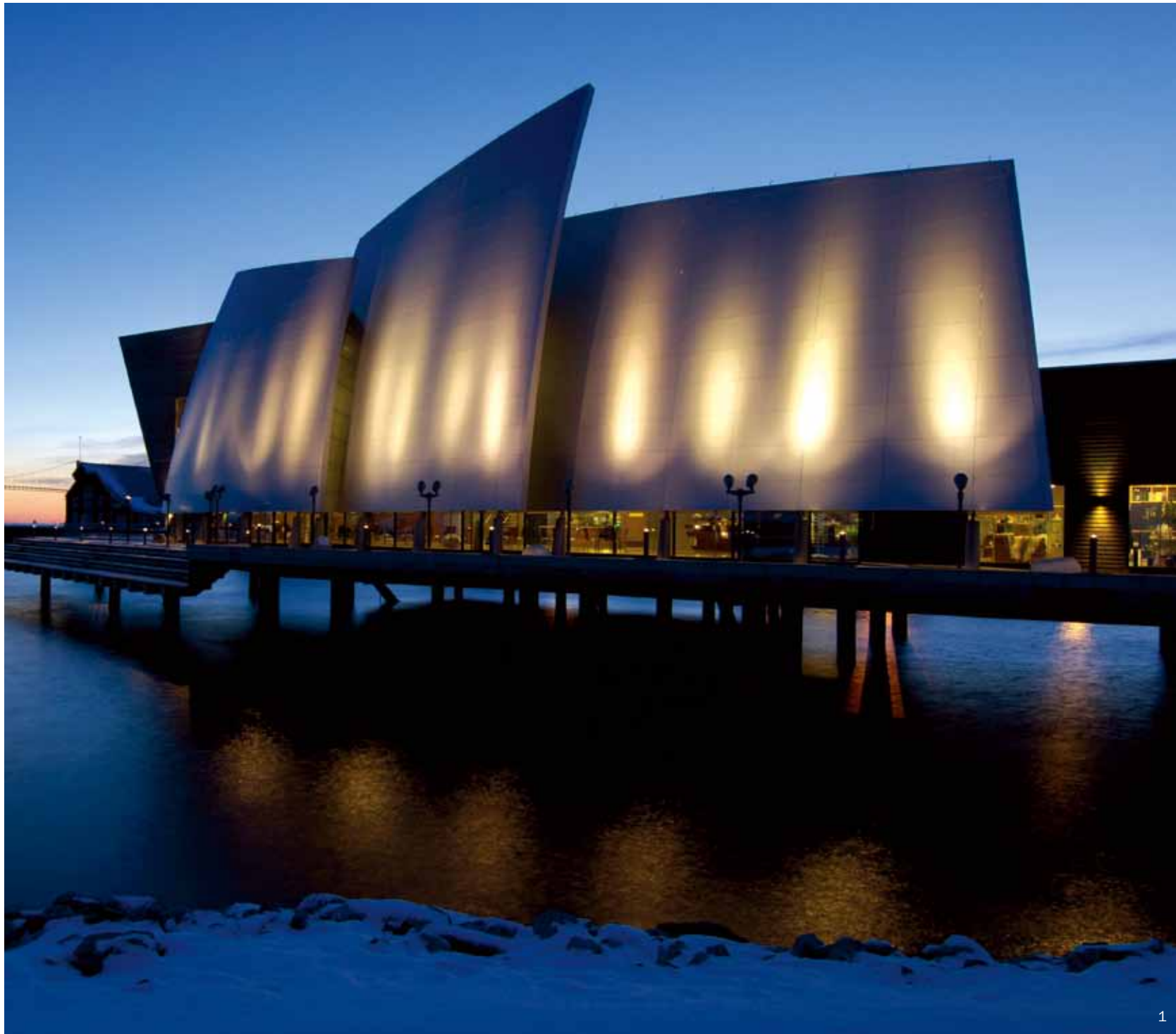
1. View of front façade 2. Main entrance at winter night
