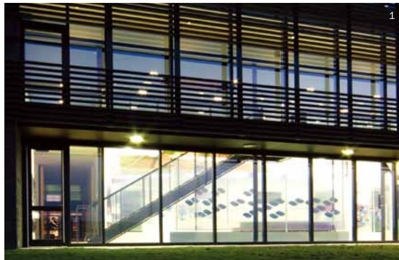
1, 2. Façade detail 3. Terrace
