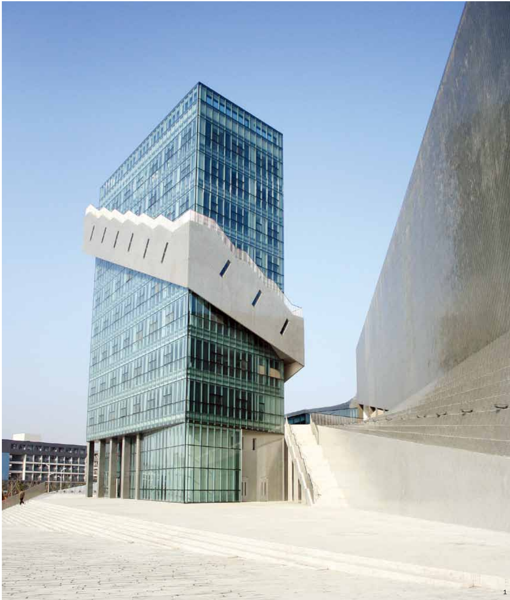
1. Tower and east façade 2. Hall
