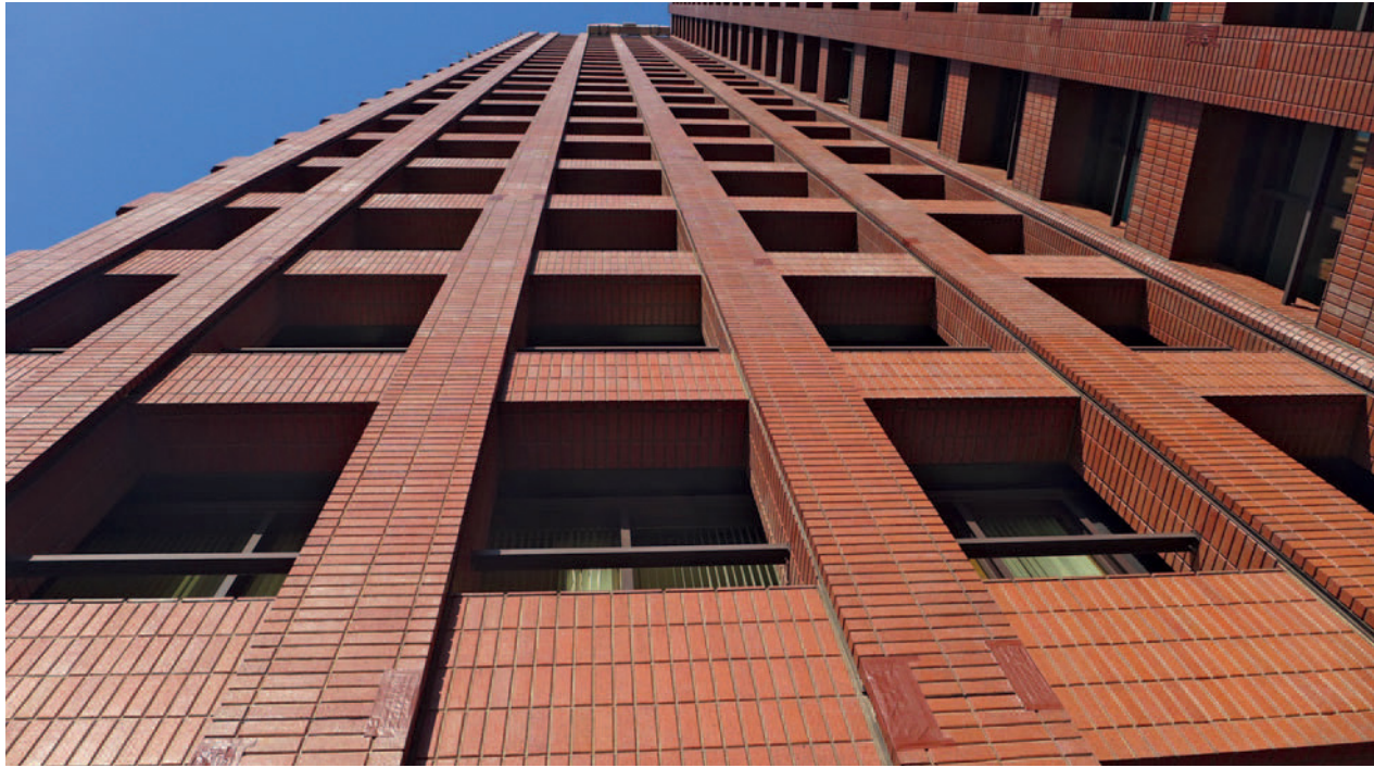
Figure 7.7 Tokyo Marine Holdings Tower
