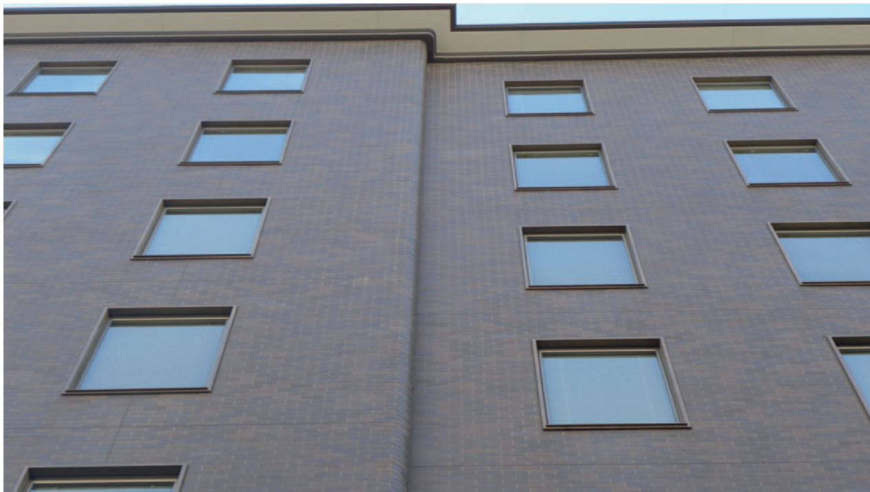
Figure 5.7 Morigo Office Building
