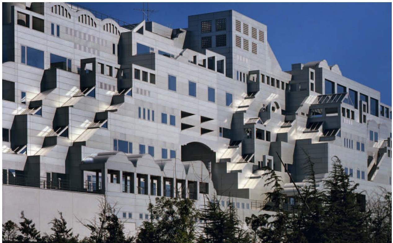
Figure 12.5 Yamoto International Office Building
