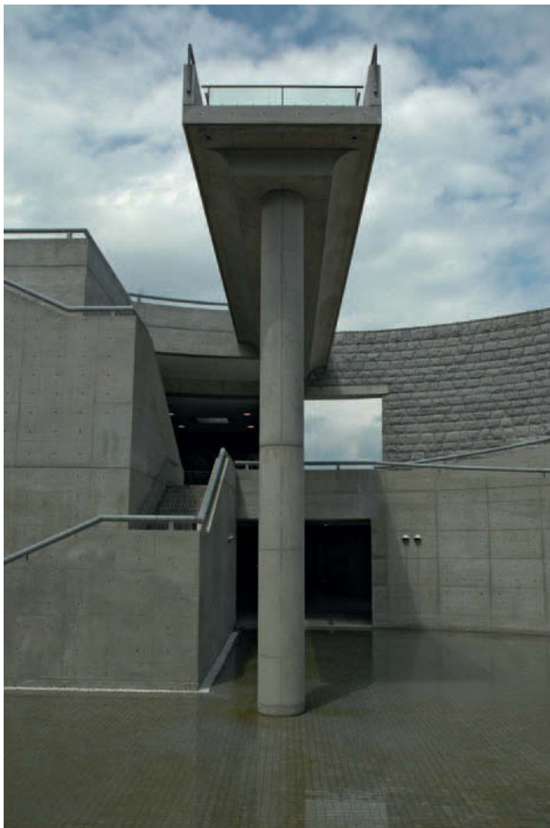
Figure 14.8 Awaji Yumebutai International Conference Center Source: James Steele
