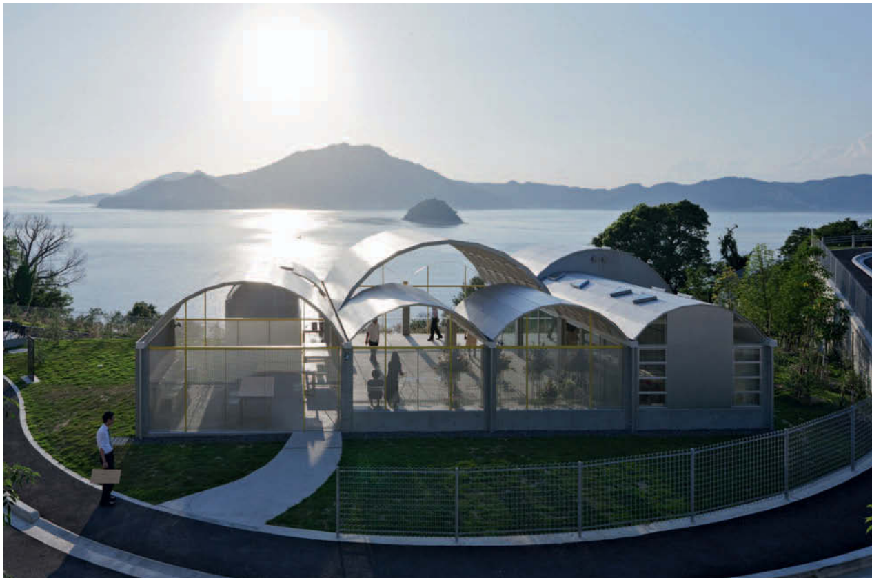
Figure 14.10 Steel Hut, Museum of Architecture on Omishima Island
