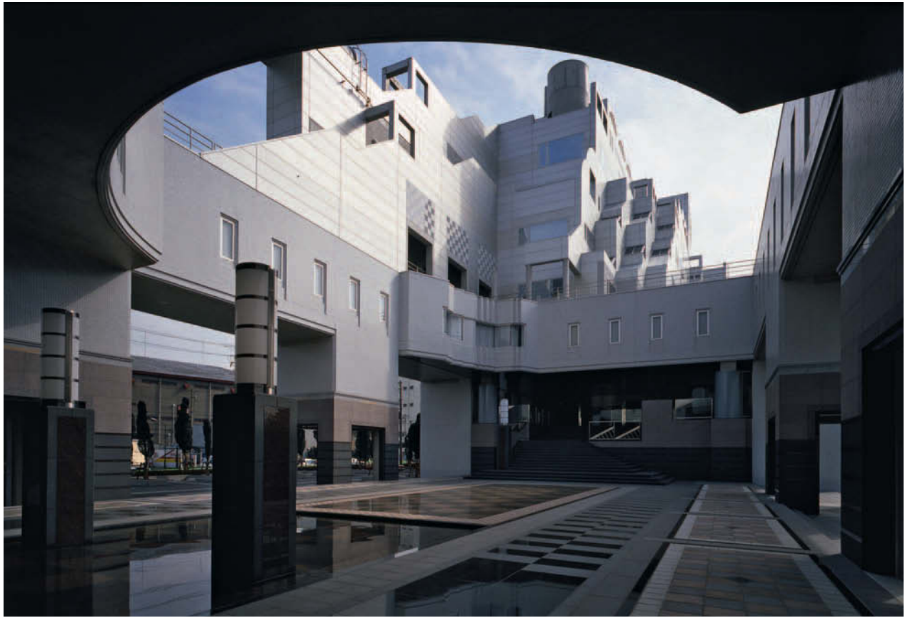
Figure 12.4 Yamoto International Office Building
