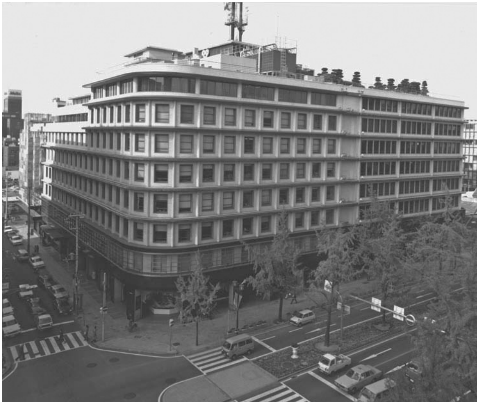
Figure 5.6 T. Yasui Gas Company Headquarters Building in Osaka
