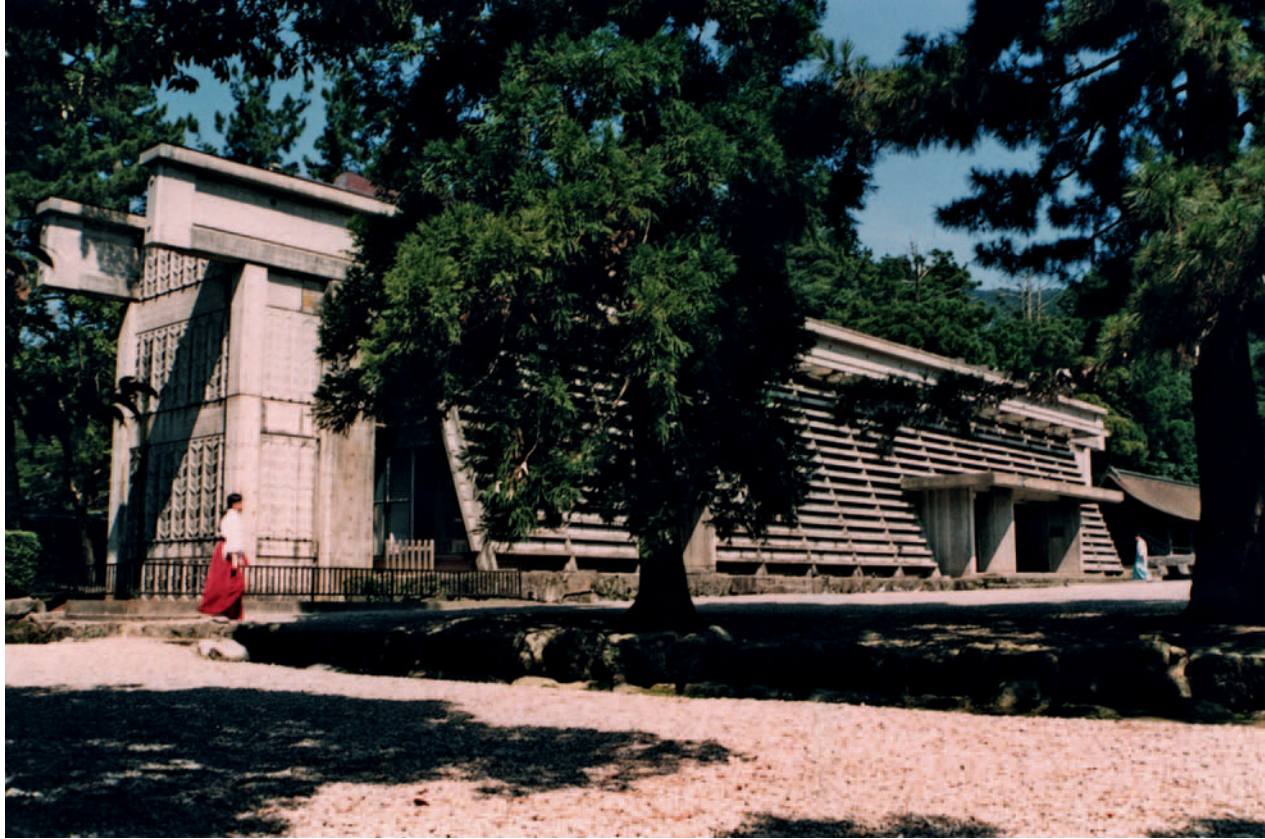
Figure 8.2 Izumo Shrine Administrative Building
