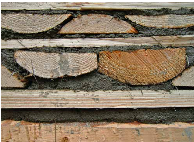
P.5. Cob masonry with waste wood from sawmills. Credit: Olle Hagman.
