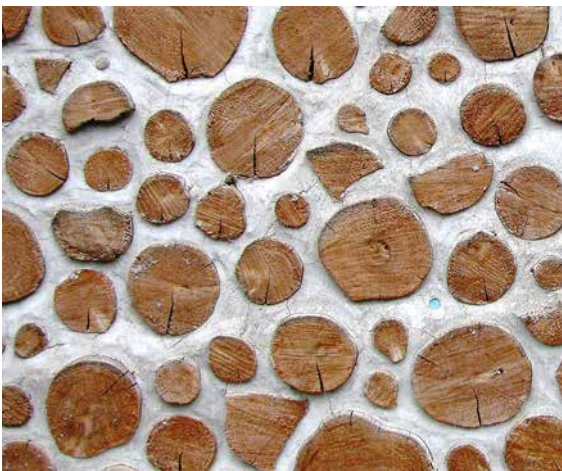
10.1. Cordwood masonry with lime putty mortar, made by Nancy Dow.
