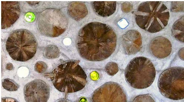
20.5. Ben would carefully cut through the long logs where 5 or 6 small branches came together to make beautiful end-grain designs in his Cook pine. Credit: Ben Oliveros.
