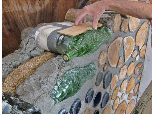
8.13. The fish bottle is supported by the inner mortar joint. A wooden shingle stops mortar or sawdust from falling between the fish and the clear cylinders.
