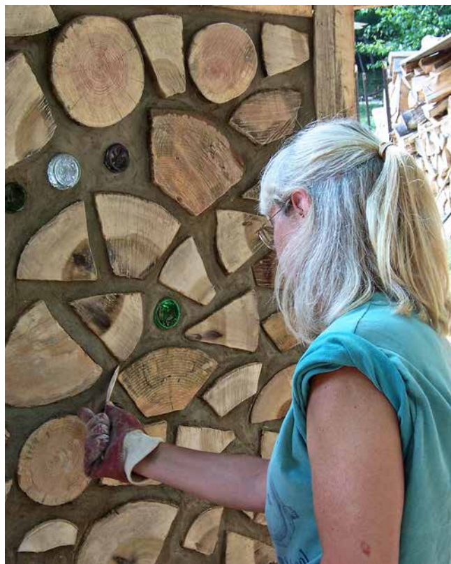
3.10. Jaki finishes the pointing on a mostly split-log wall.
