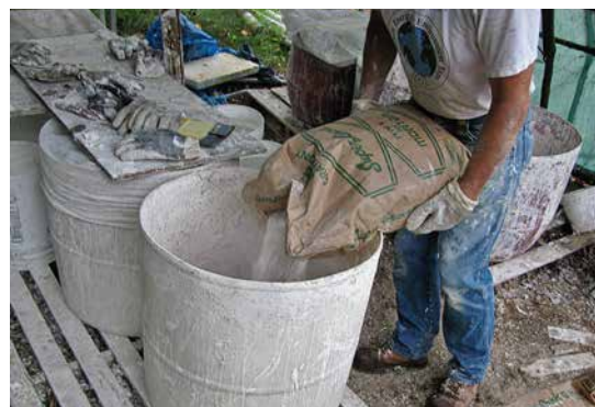
10.2. Bruce carefully measures water and Type S hydrated lime into a vessel made from half of a 55-gallon plastic drum.
