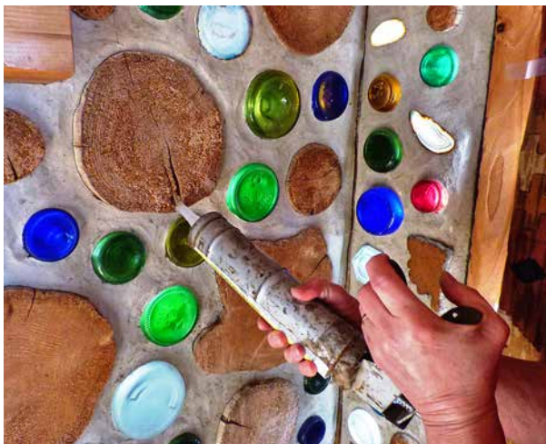
4.4. Caulk with clear siliconized caulking.
