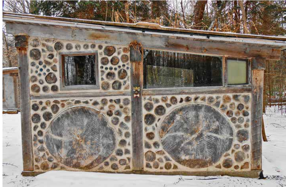
14.1. La Casita guest house at Earthwood. The 52-inch-diameter Balm of Gilead log-ends make up half the area of these panels. The other 60-plus log-ends—and all the mortar between them—make up the other half.
