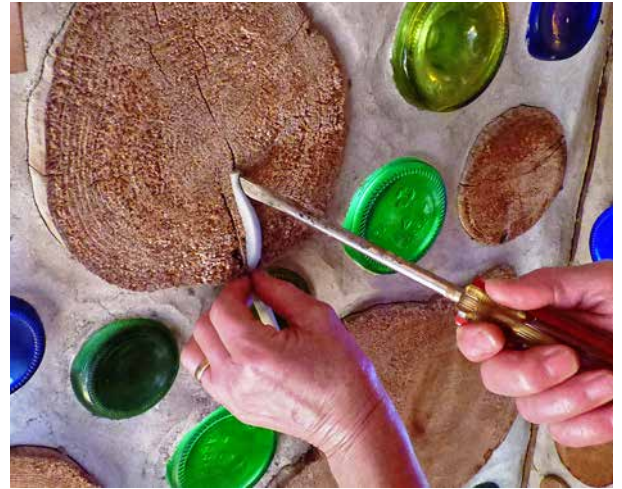
4.3. Push backer rod into the check with a flathead screwdriver.
