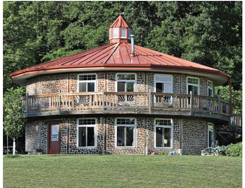
Below: Alan Stankevitz's home in La Crescent, Minnesota, features paper-enhanced mortar and spray-in foam insulation.
