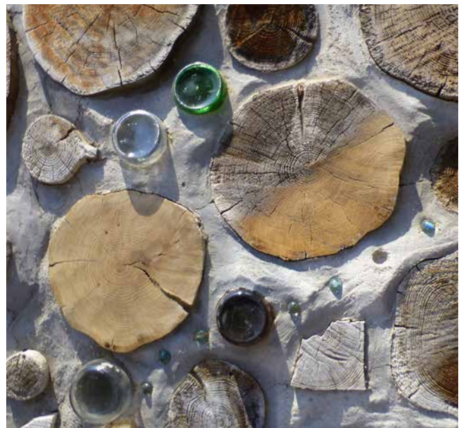
21.7. The right-hand log-end is half sanded, to show contrast. Sealer is applied with a brush.
