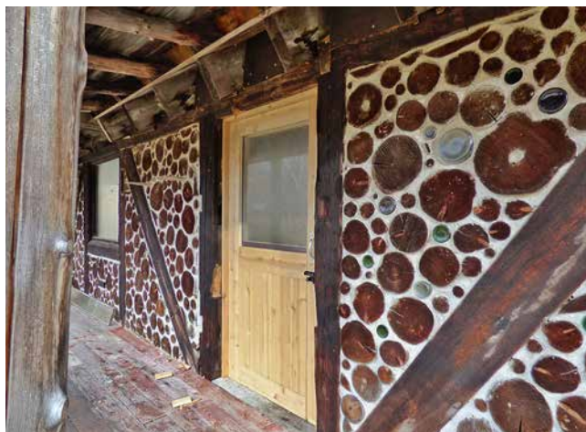
1.13. Log End Cottage, built in 1975. Doors and windows are enclosed by the timber frame itself, mostly 8-inch by 8-inch recycled barn beams.
