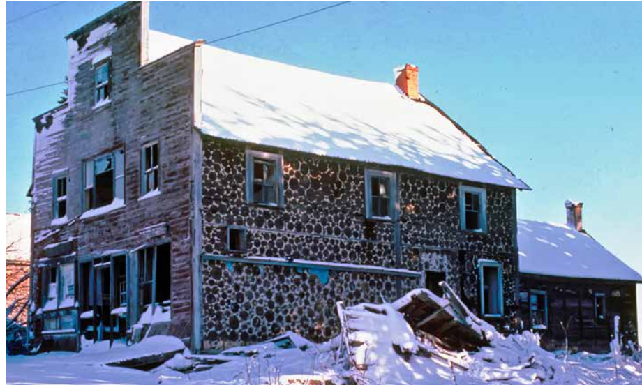
P.1. The Mecikalski General Store about 1983, before restoration.
