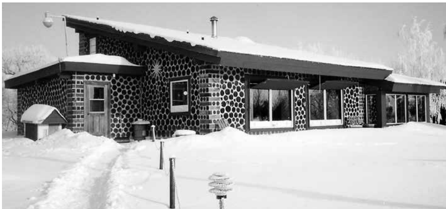
6.6. Cliff's main house, where he now lives, built 1978–80. Credit: Cliff Shockey.
