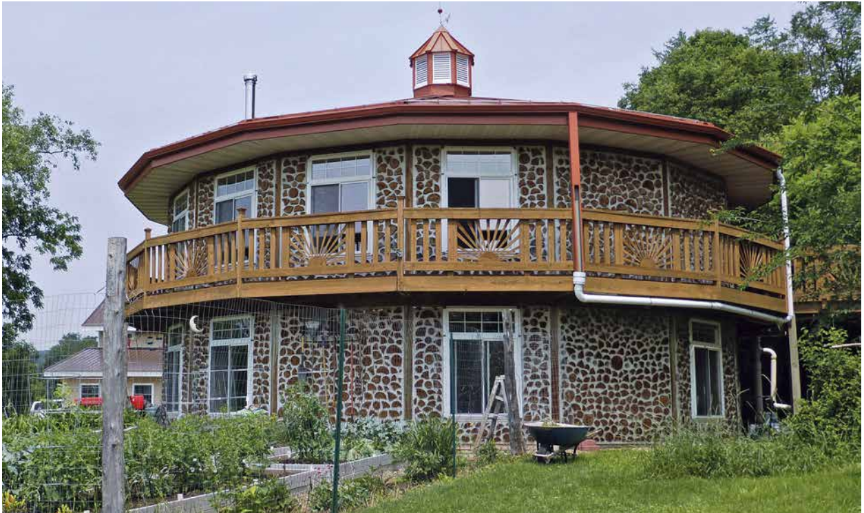
6.7. Alan Stankevitz built this beautiful 16-sided double-wall cordwood home near La Crescent, Minnesota.
