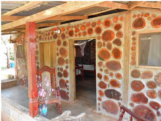
22.9. Nice log placement and pointing on the long entrance side.
