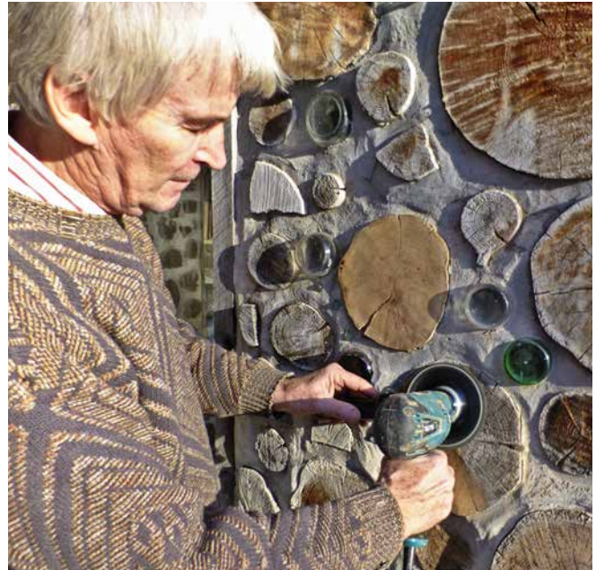
21.6. Rob sands log-ends with his favorite power tool, a Makita 4500-rpm circular sander.
