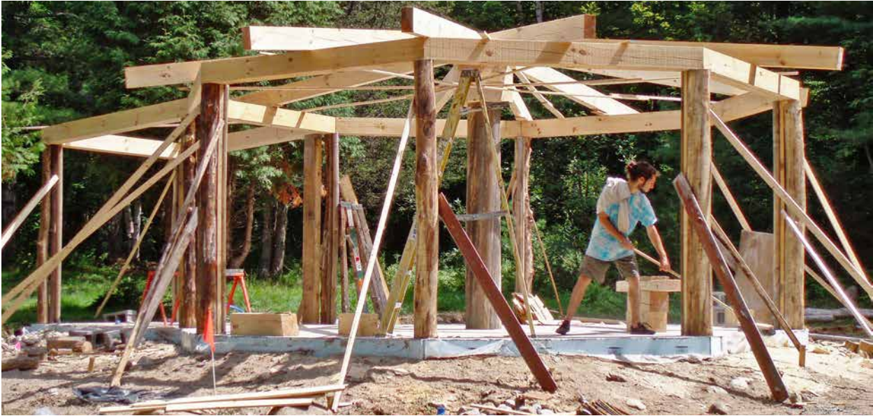
18.4. The timber frame. Credit: Rarilee Conway.
