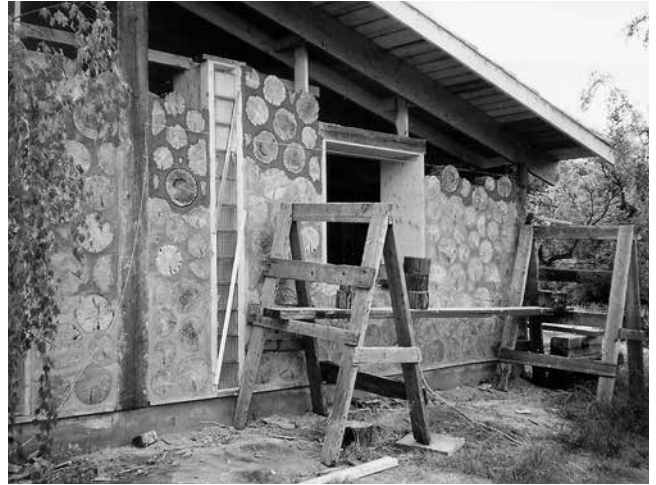
6.5. Cliff's addition, shown under construction, was built in 1990. Credit: Cliff Shockey.
