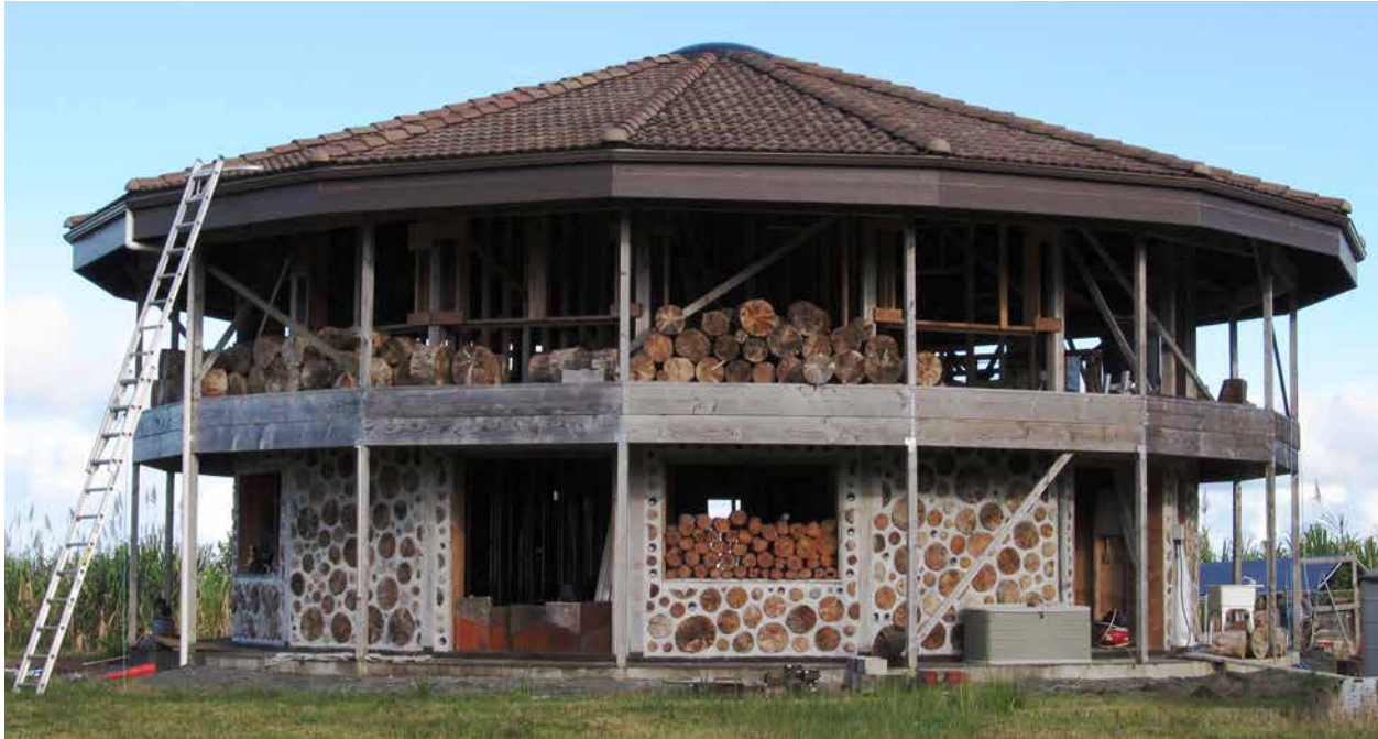
20.1. Ben and Mirtha’s house in 2008, just before we started helping Ben with the second story cordwood.
