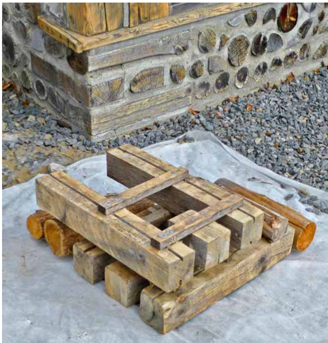
1.8. Two Lomax corner units, made from 4-inch-square timber stock, are stacked one upon the other. Note the tie pieces and chainsaw grooves for better friction bond to the mortar, not shown in this model. The short block is simply a decorative filler piece and helps retain the sawdust insulation which will be placed in the continuous inner cavity of the corner. In the background is a stackwall corner at Earthwood, made from 4-inch by 8-inch quoins for this 16-inch cordwood wall. The wall continues above with the cordwood supported by a “double-wide” pair of adjacent 8-inch-square posts.
