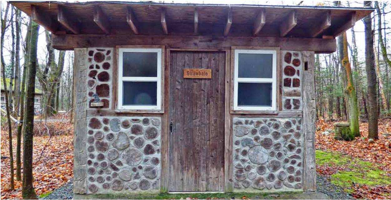
1.14. Strawbale (and cordwood) guest house at Earthwood. The door is exactly framed by the 4-inch by 8-inch jambs which extend from the foundation to the 8-inch by 8-inch girt.
