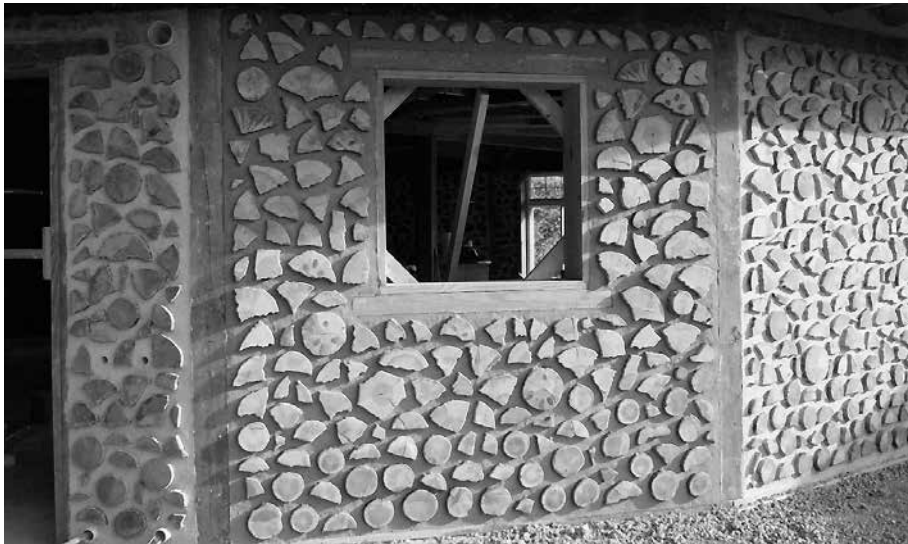
12.2. There are 16 panels on each of the two stories at the Stankevitz home. Credit: Alan Stankevitz.
