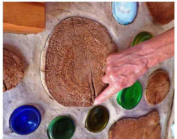
4.5. Jaki seals the caulk with her finger. The end result looks very much like a round log with a check in it. In fact, it looks exactly like Figure 4.2.
