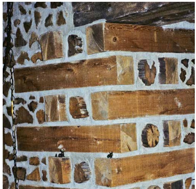
1.10. An internal stackwall corner on a house in Thornton, Ontario.
