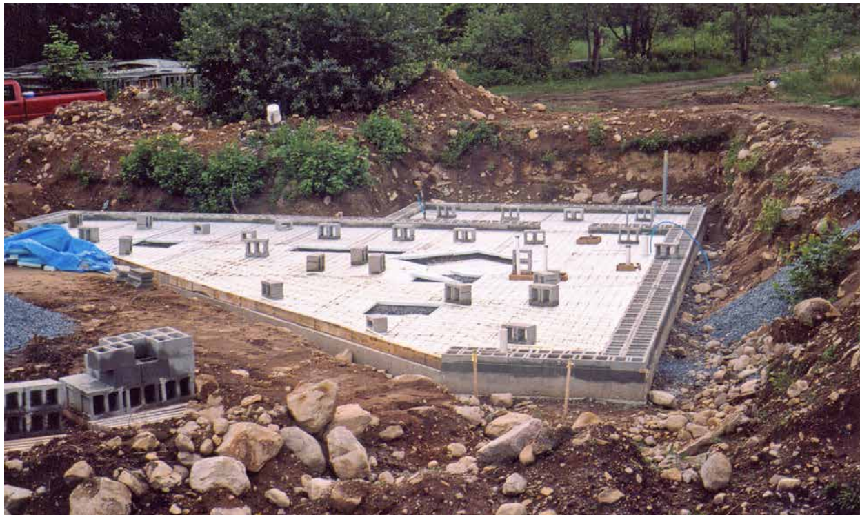
19.2. Our triangular Trisol foundation in place. Credit: Bruce Kilgore.
