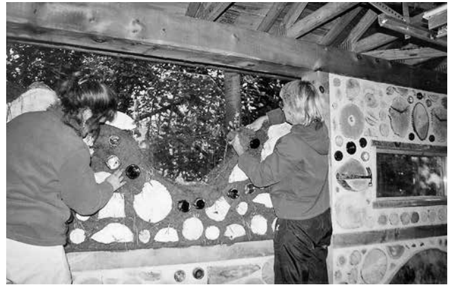
11.4. Linda Smiley (left) and Jaki Roy lay up cob in preparation for log-ends. Note that rubber gloves are not necessary for playing with “mud pies.” The panel at right is cordwood with mortar.
