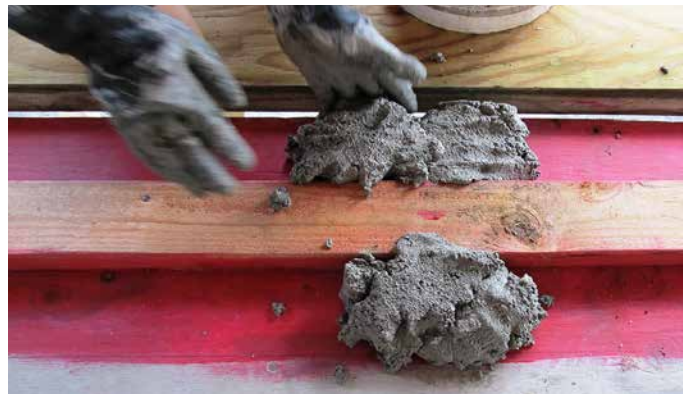
20.4. To do cordwood on plywood for the second floor, we first applied bonding agent and a wooden key piece.
