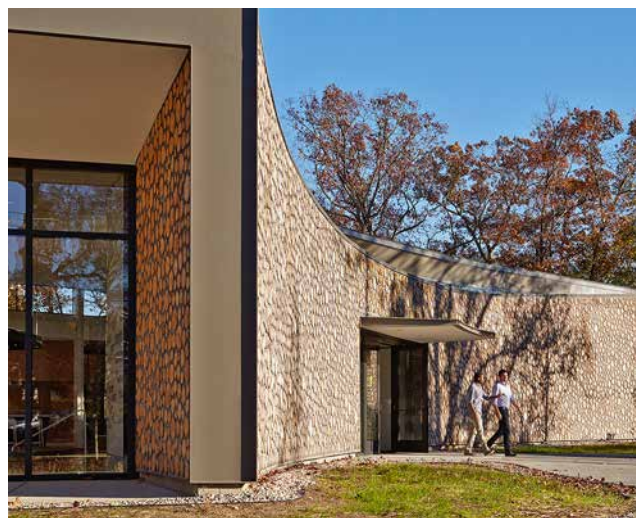
16.11. The three entrances are framed by wood masonry through walls, beginning two feet wide at the steel-framed ends and increasing in depth up to six feet further in; possibly the longest log-ends ever used in a cordwood wall. Photo by Steve Hall, © Hedrich Blessing.
