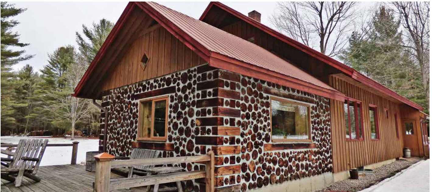
Below: Stackwall-cornered addition in Peru, New York, by Bruce and JoAnne Kennedy.
