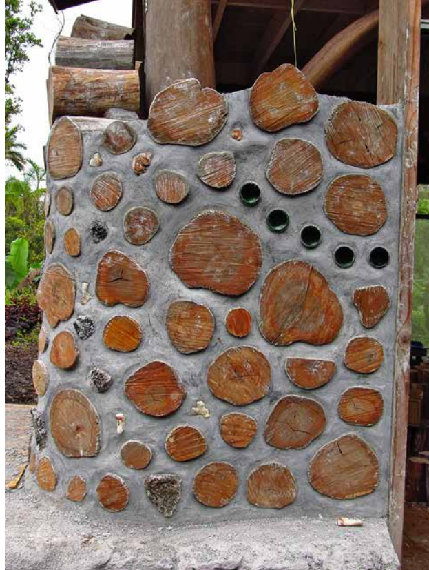
1.20. Exterior view of a “mini” bull-nose corner, wrapping around an ohia post in a timber-framed home in Hawaii. Small log-ends and chunks of lava helped fill large mortar joints.
