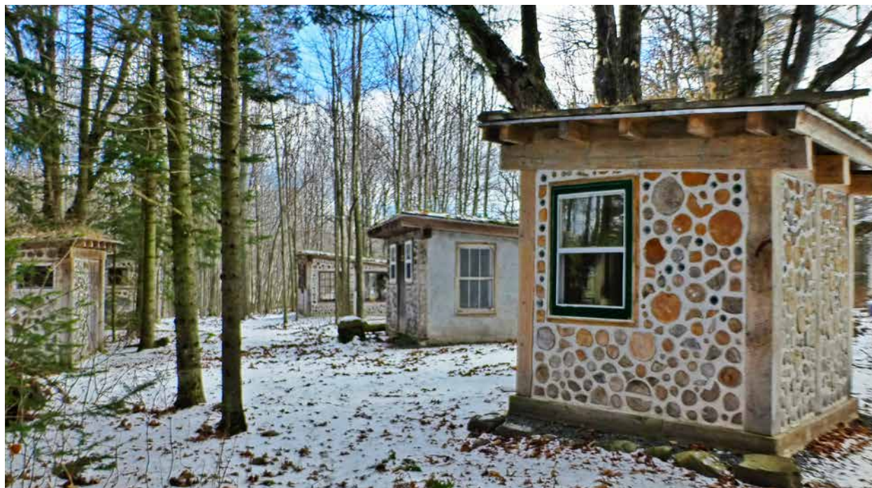
21.5. The north and west sides of the Hermit’s Hut, treated with siliconized sealer. The little building looks down over the avenue of the Cordwood Village at Earthwood.
