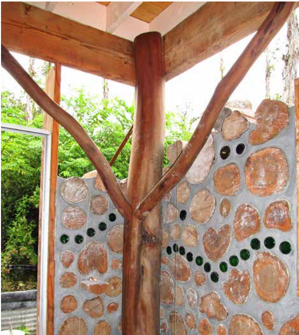
1.19. Tapered logs at the corner, with barbed wire reinforcing in the mortar joint for extra strength. Credit: Lonnie Sobeck.
