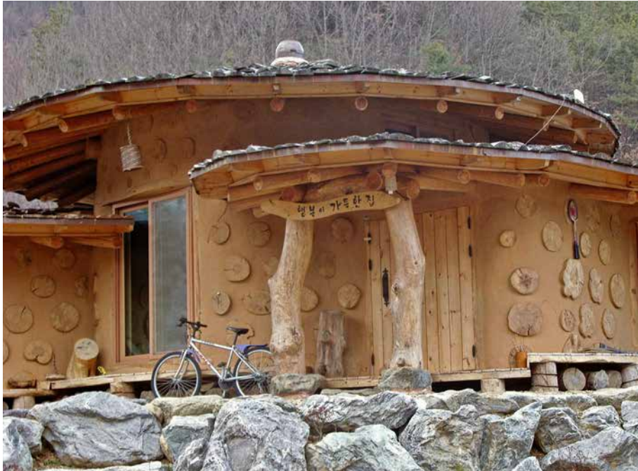
11.6. A typical Korean soil house with large log-ends as structural and decorative members.
