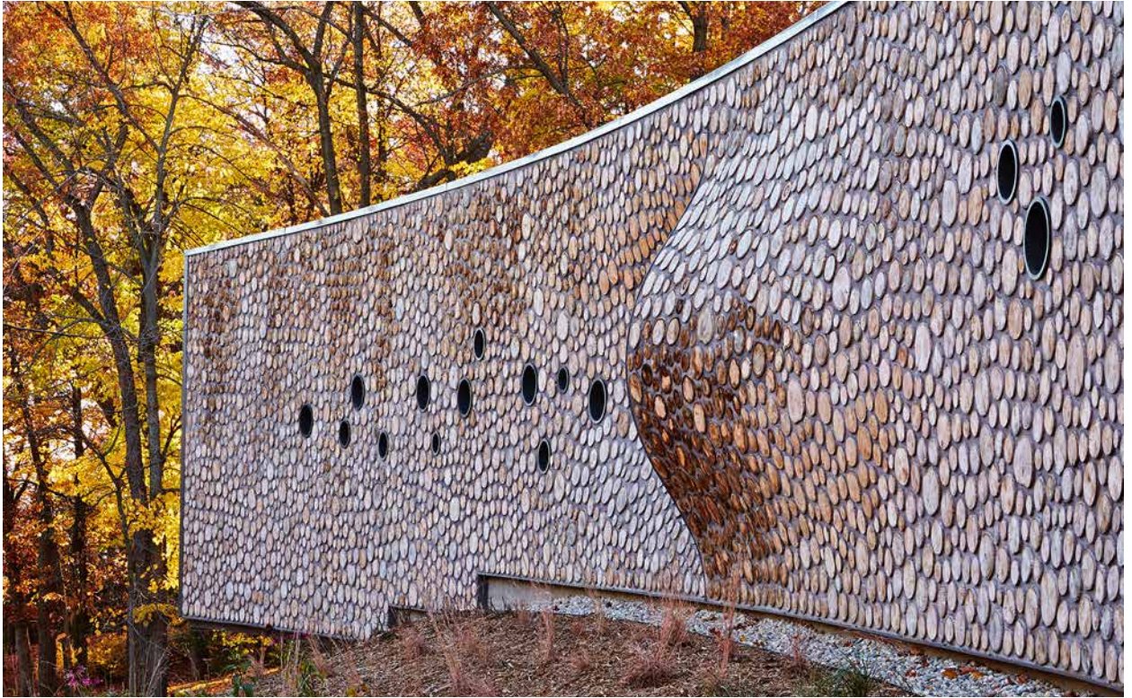
16.13. The warped wall in its completed state. Credit: Studio Gang Architects.
