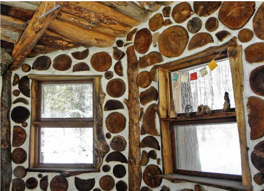
17.11. Slab-wood window frames. Credit: Geoff Huggins.
