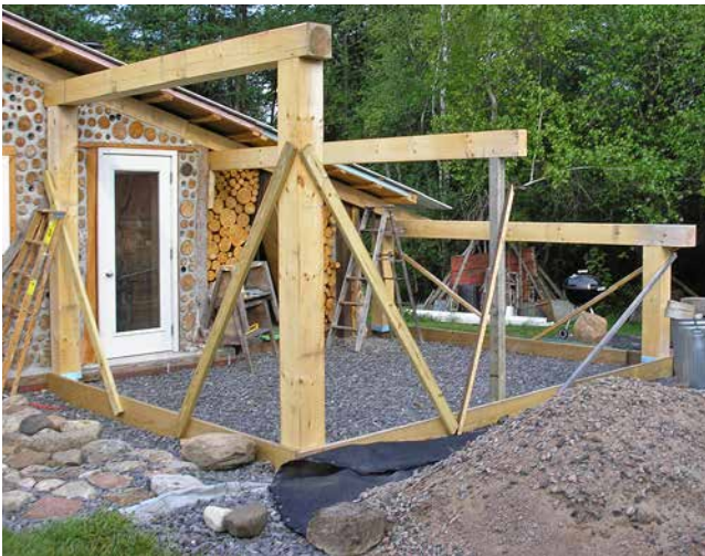
13.1. Foundation and timber frame for the east addition.
