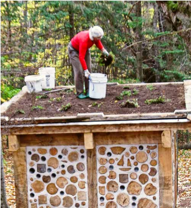
21.2. Jaki plants the lightweight living roof (three inches of topsoil) to sedum, dead nettle and other ground cover plants.
