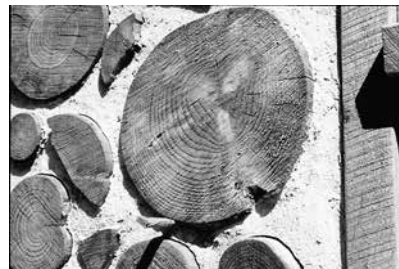
4.8. Presto Farino! When dry, it is not easy to see the patch, particularly when the little wedge is removed. Credit: Geoff Huggins
