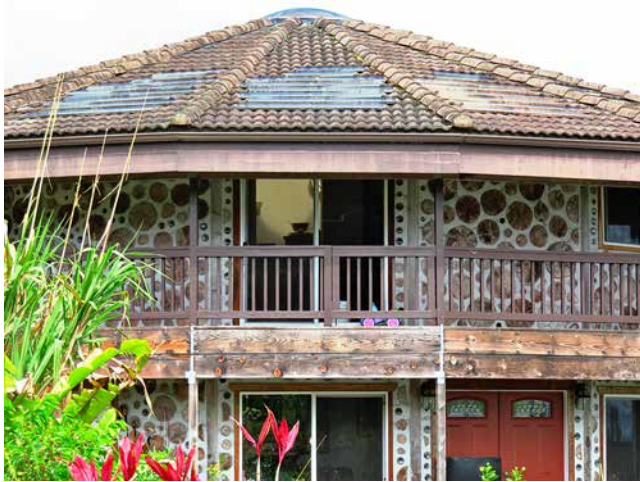
20.7. Solar shingles integrate with brown concrete tiles on the Oliveros roof. Credit: Ben Oliveros.
