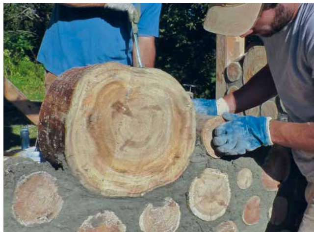
3.7. This student kept turning the large log-end until the right curvature matched the shallow cradle below. Now, he supports it with a small log-end in its own cradle.
