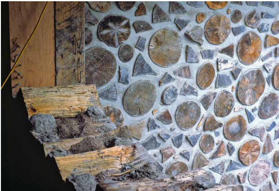
2.5. Former students built this beautiful cordwood wall of mixed splits and rounds in central Pennsylvania. Note how the rounds are featured, each surrounded by a variety of splits.
