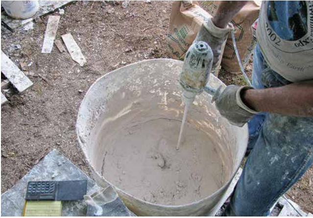
10.3. Mixing the lime putty with a paddle drill.
