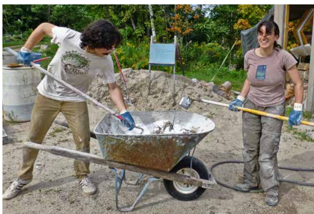
3.1. Cordwood students learn to mix mortar in a wheelbarrow, using ordinary garden hoes and, importantly, cloth-lined rubber gloves.
