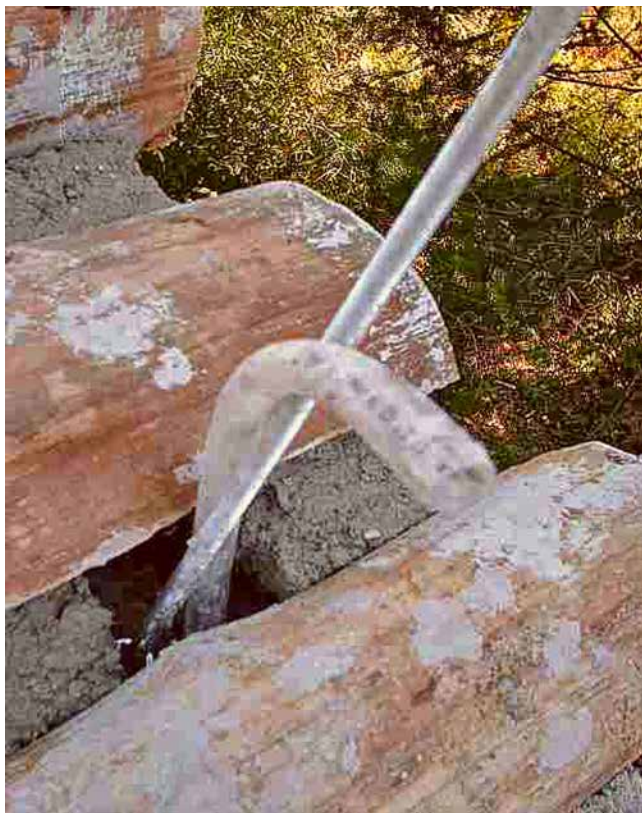
7.4. Place the nozzle into the installation pipe, insure a tight fit, and start injecting by pulling on the trigger gradually.
