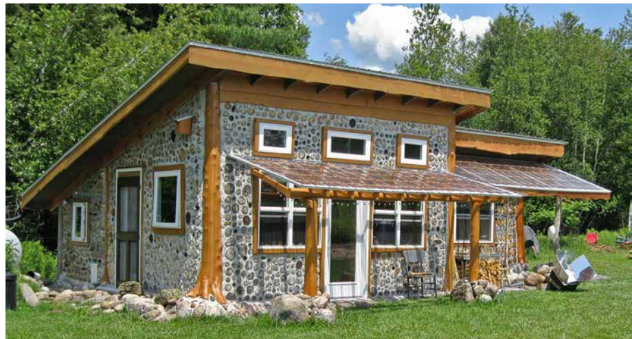
13.5. Cordwood cabin with additions at Cedar Eden (Potsdam, New York). Credit: Tom Huber.
