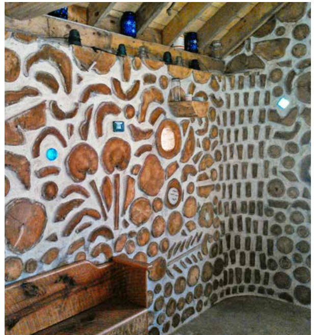
1.18. Interior of Bull Nose Cabin. Note that the corner logs have all been tapered. Credit: Lonnie Sobeck.
