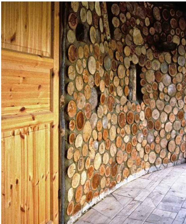
11.2. Detail of Steen Moller's cobwood wall in Denmark. Credit: Catherine Wanek.
