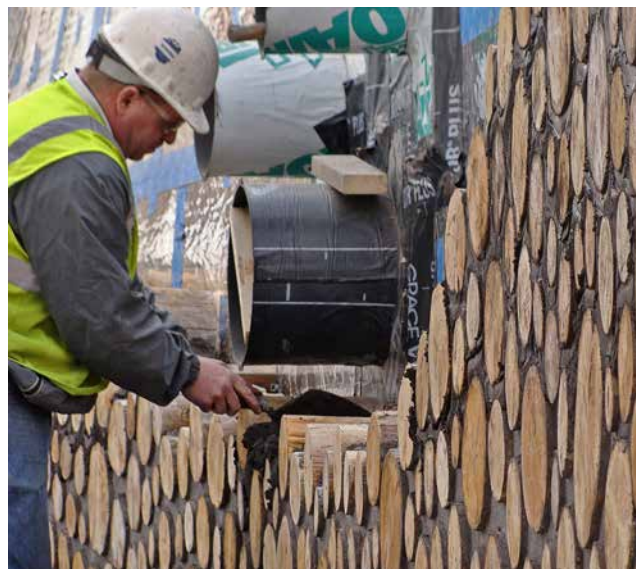
16.10. The wood masonry exterior is built around 46 prefabricated insulated window units of varying sizes, integrated into the log pattern. See also Figures 16.1 and 16.9 ( right ). Credit: Studio Gang Architects.
