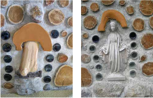
13.4. Two sides of a cordwood wall: “stoned on mushrooms” and a “blessed virgin.” Credit: Tom Huber.
