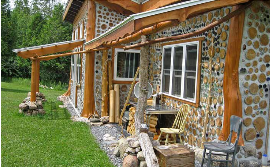
13.3. The east addition is completed, with a sheltered area for taking refreshment breaks. Credit: Tom Huber.
