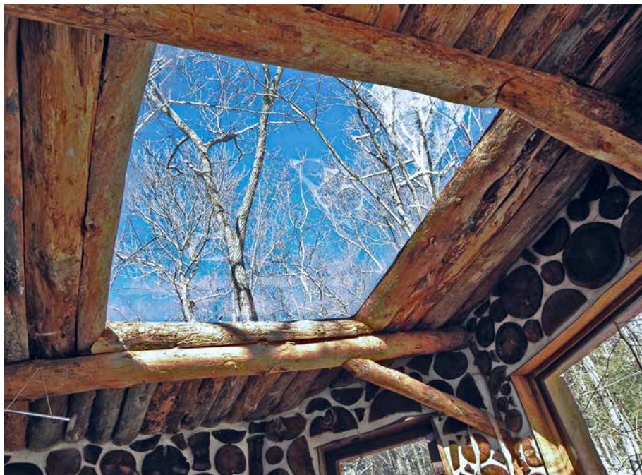
17.12. Kuti skylight. Credit: Geoff Huggins.
