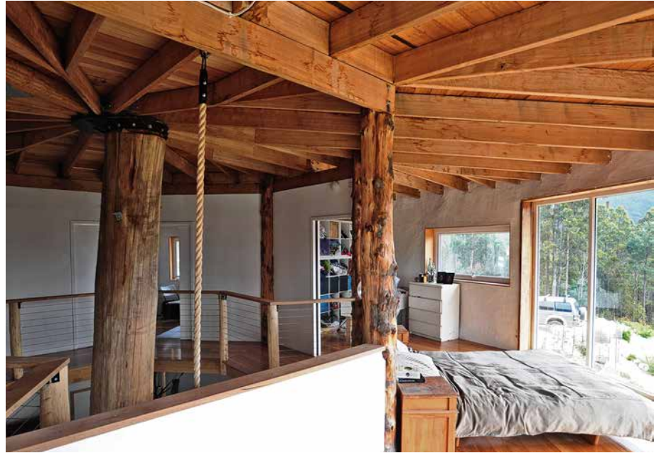
20.10. The interior of the house is open to the upstairs. The cordwood masonry is covered with plaster rendering. Credit: Peter Robey.
