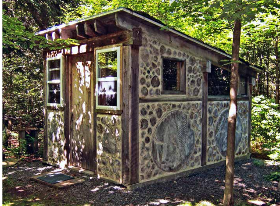
23.1. La Casita, a guesthouse at Earthwood, would make a good TS for a single person, while providing a lesson in simple post and beam framing.
