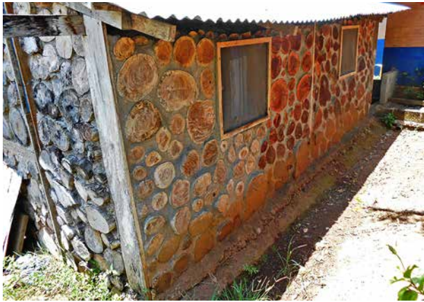
22.7. It is easy to see which panel was built first.
