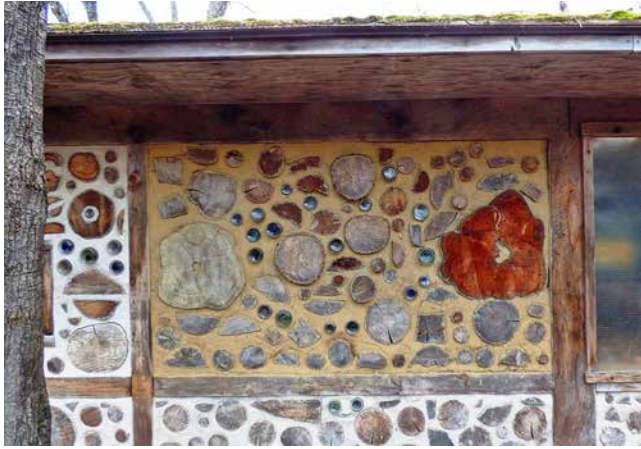
11.5. Our cobwood panel in the garage, well protected by overhang, still looks good after 15 years.
