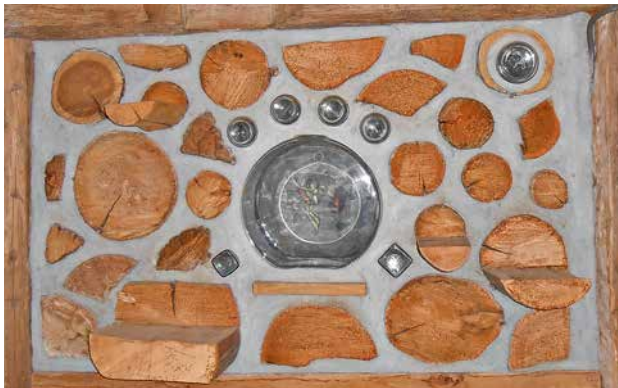
14.2. This panel is 60 percent wood and 40 percent mortar.
