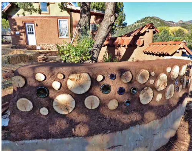
11.8. Our cobwood wall demo in New Mexico, completed.
