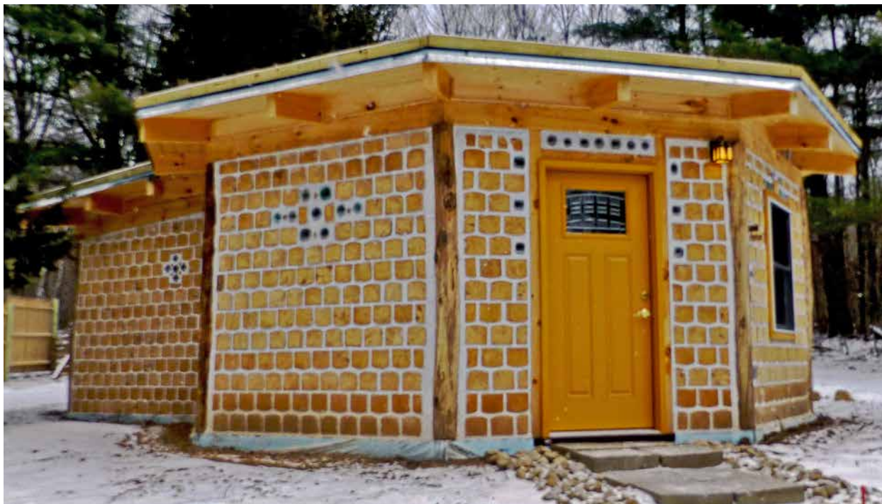
18.1. Our Adirondack Cordwood Cabin is a 22-foot-diameter octagon. Credit: Rarilee Conway.
