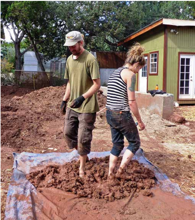
11.3. The cobber's dance. These young experienced helpers made our cob for us at our cobwood wall demo at the 2015 Natural Building Colloquium, Kingston, New Mexico.
