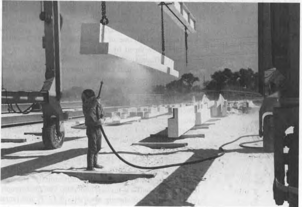
FIGURE 18.20 Sand-blasted architectural finish applied to a precast L beam.
