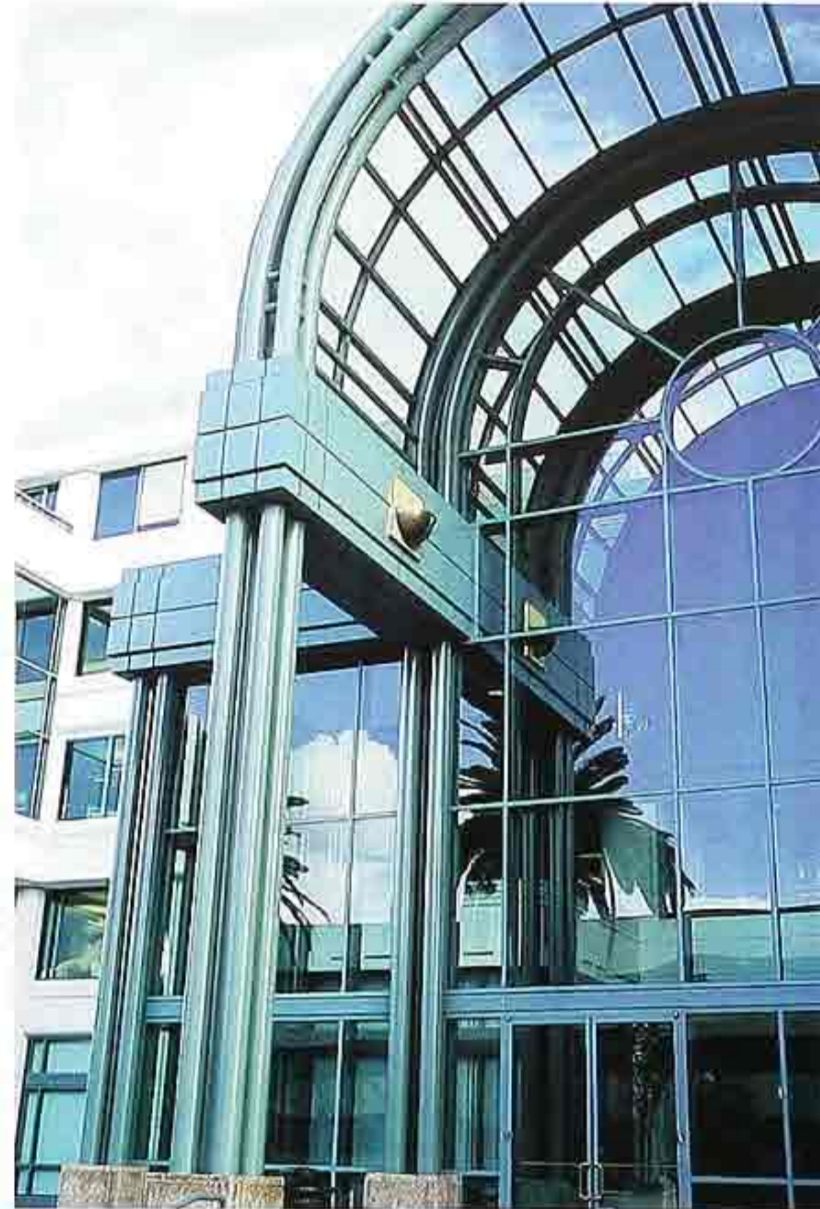
CP-177 Barrel-vaulted tubular-steel-frame-and-glass entry, modern commercial building
