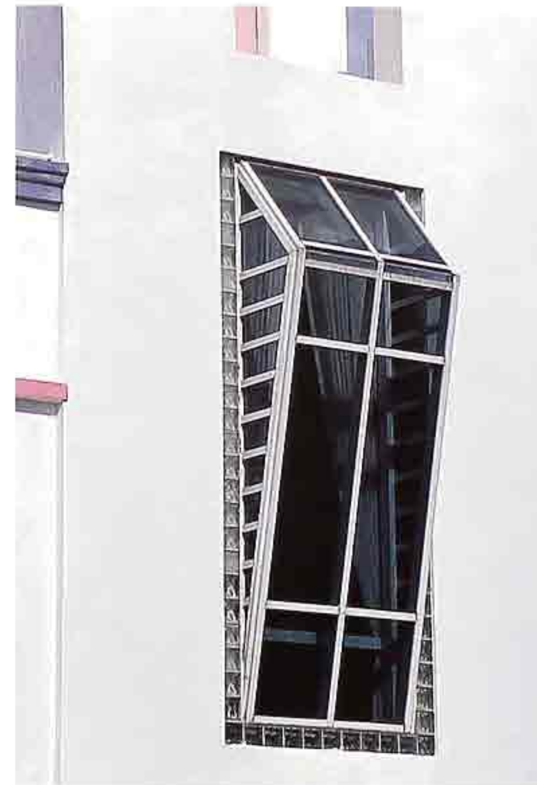
WI-90 Idiosyncratic bay with fixed lights, modern commercial building
