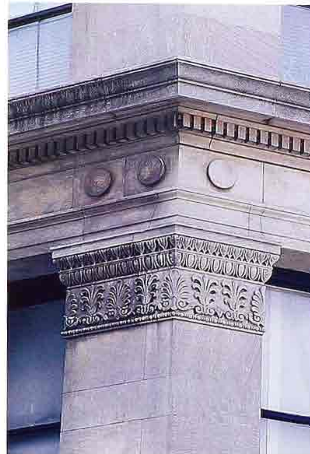
CP-21 Capital with profile derivative of Doric capital; necking ornamented with anthemion on a square corner pier with dentilated molding
