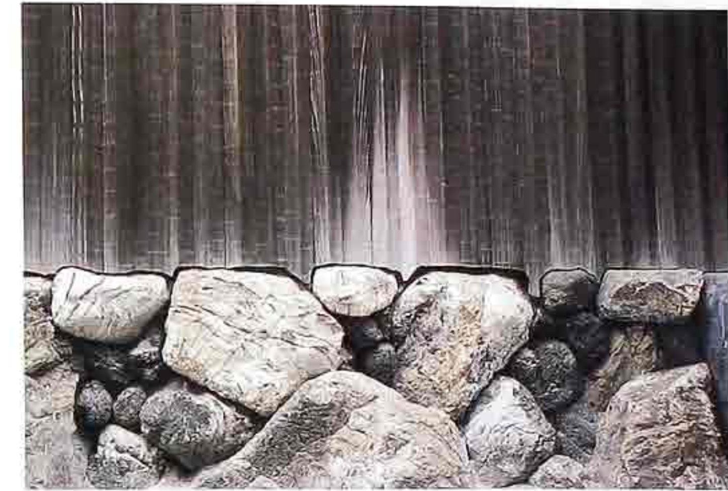
WA-270 Vertical planks of weathered cedar shaped to fit profile of fieldstone base
