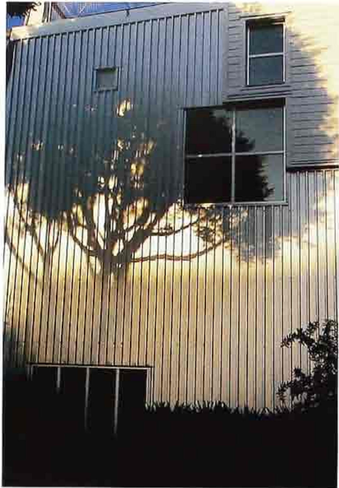
FA-19 Possibly galvanized steel, batten-seam vertical panels
