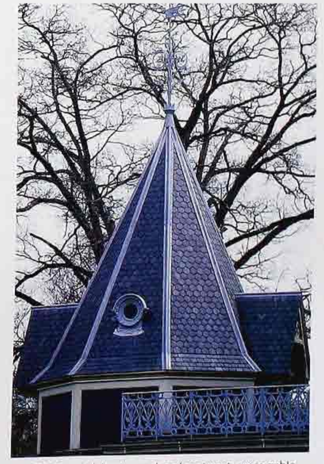
CR-133 Pyramidal octagonal roof on turret, cross-gable dormers
