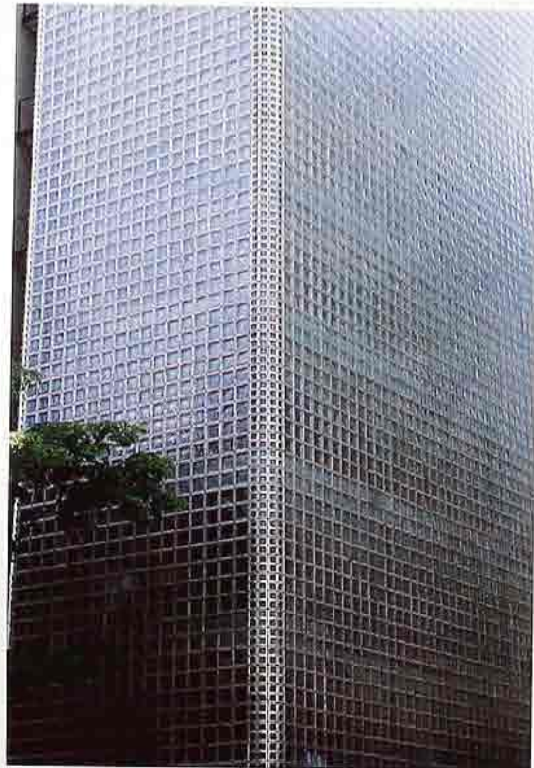
FA-35 Glass-block curtain wall with rounded corner
