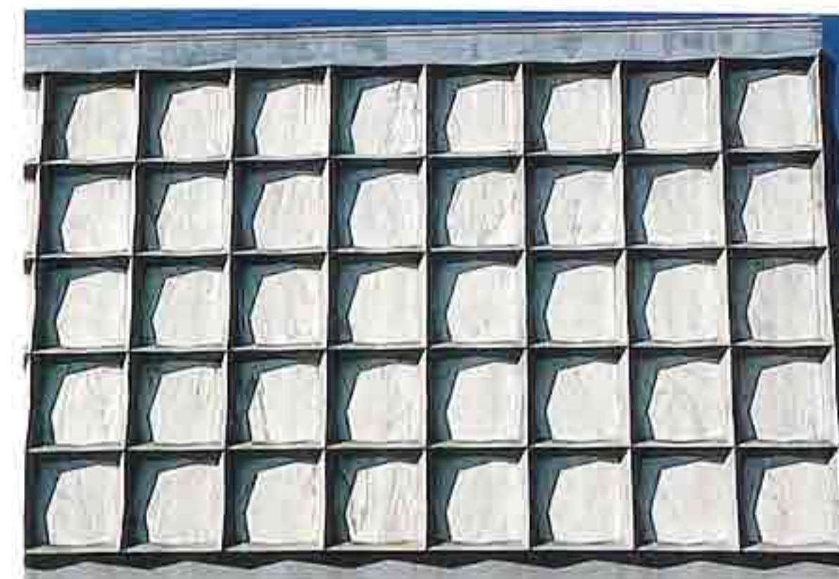
WA-66 Granite veneer on concrete frame with Vermont marble infill, modern commercial building
