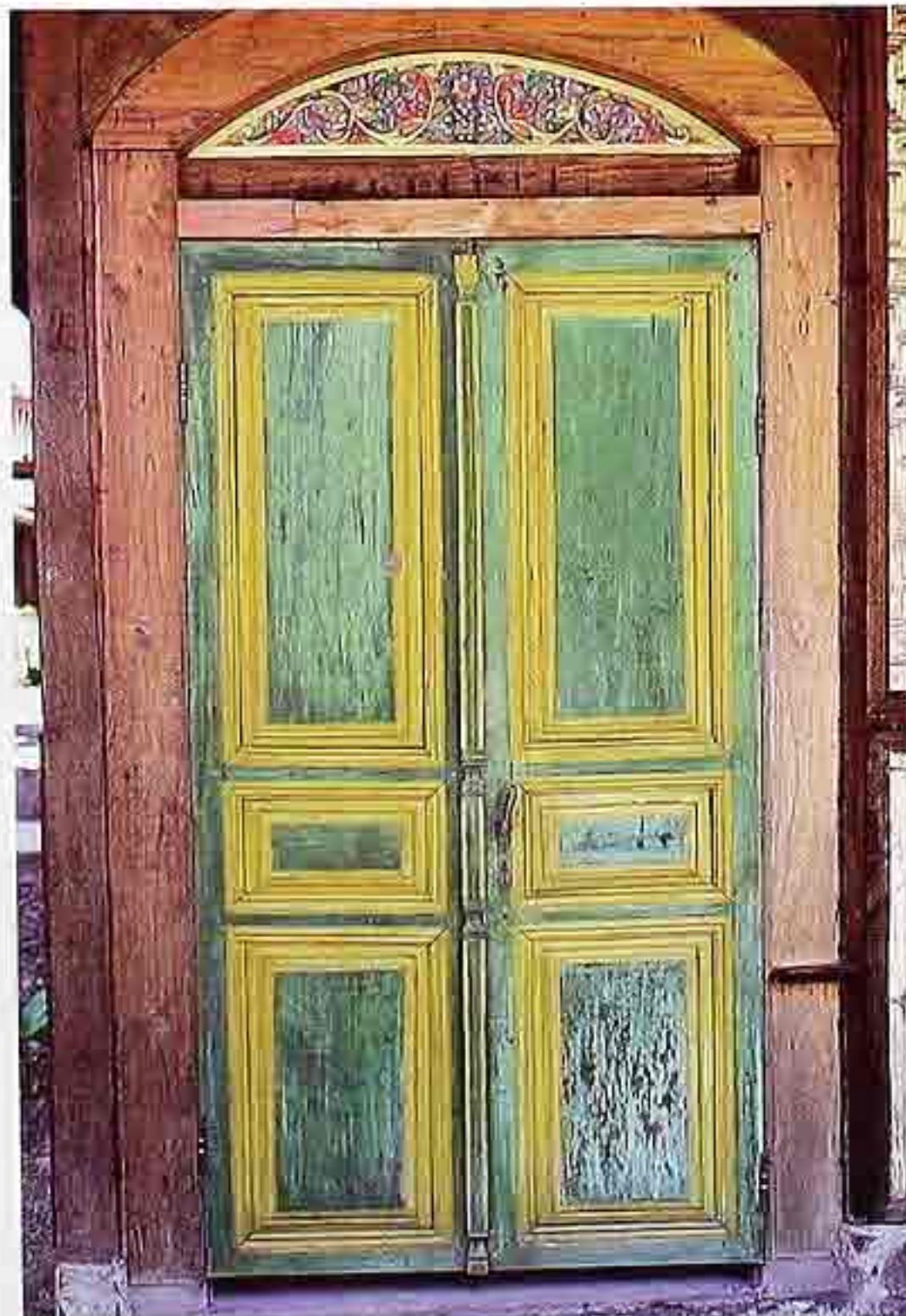
DW-39 Three-panel double doors with painted panels and painted carved ornament; segmental arch transom, Bali
