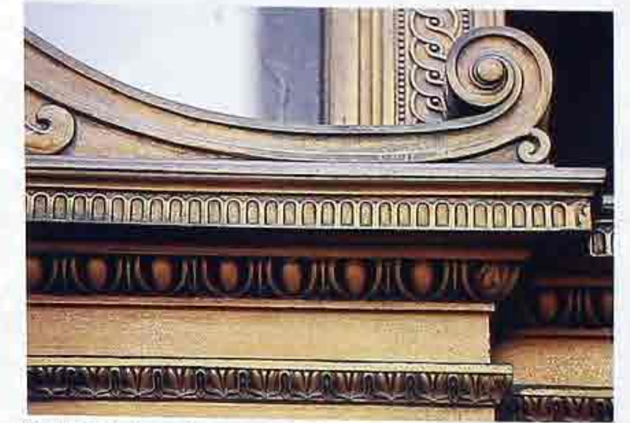
OM-5 Volute on bronze scrolled pediment. Molding, top to bottom: corona with band ornament; egg-and-dart ovolo; tongue-and-dart cyma reversa
