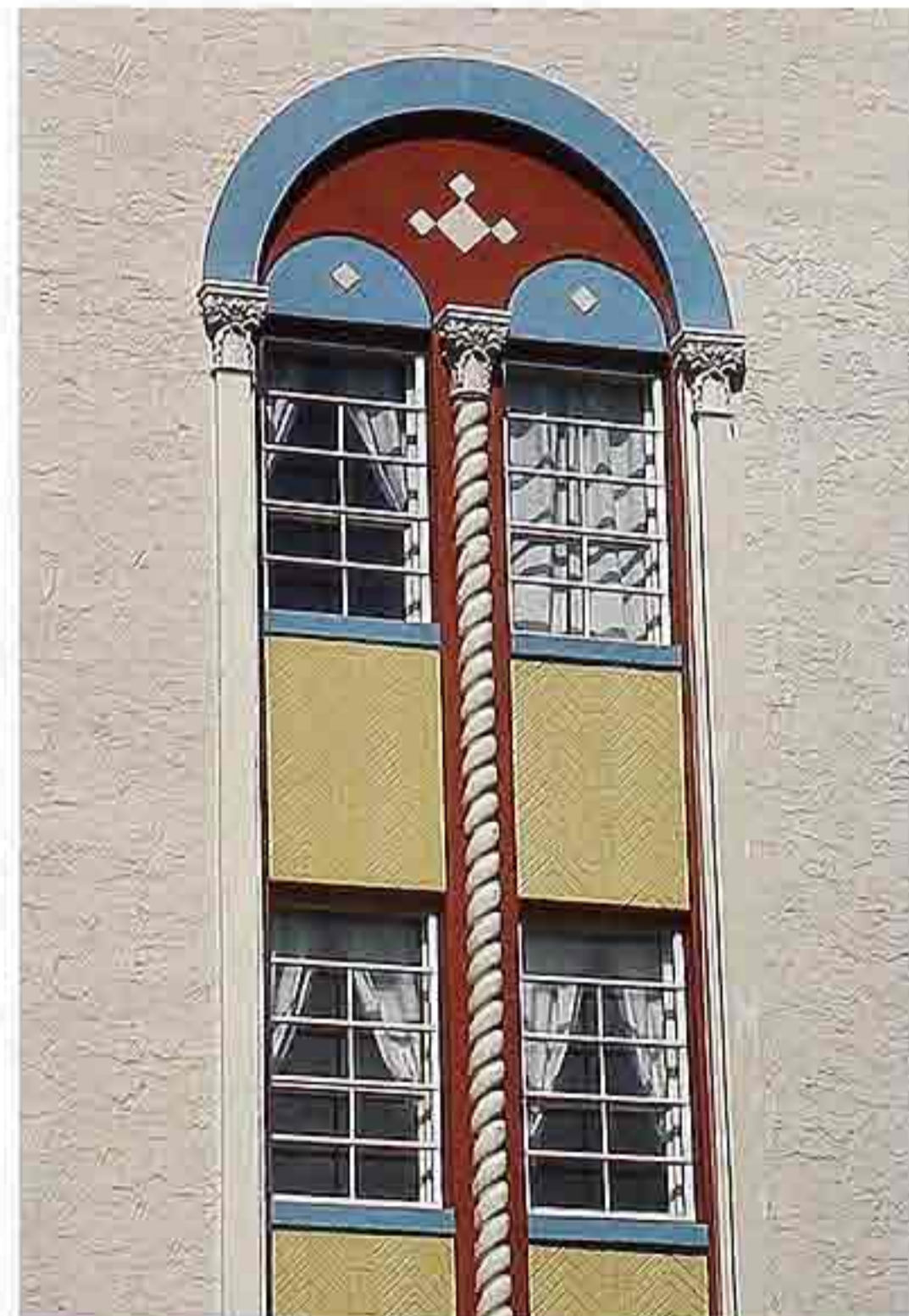
WI-153 Two-story variation of Venetian-style window; painted stucco and cast-concrete ornament, Art Deco hotel
