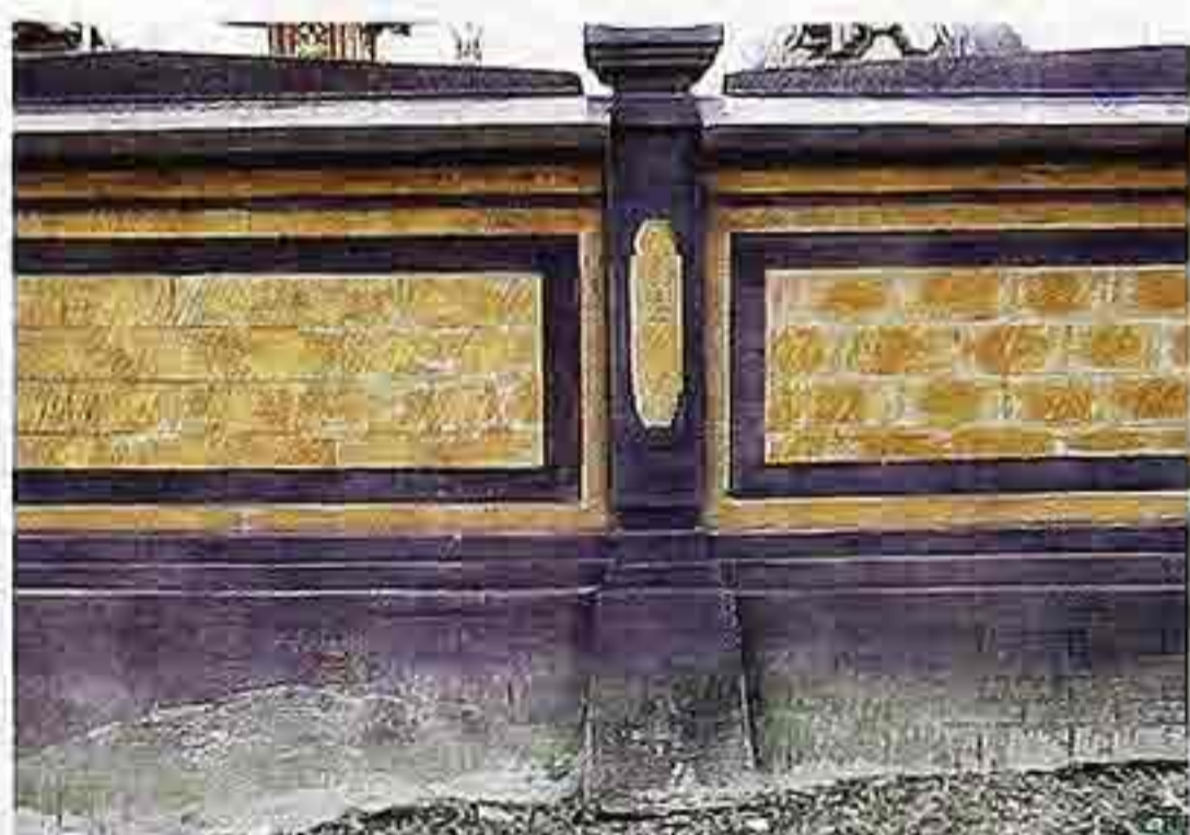
FA-84 Courtyard wall of painted stone and concrete block with scribed lines simulating masonry, Indonesia
