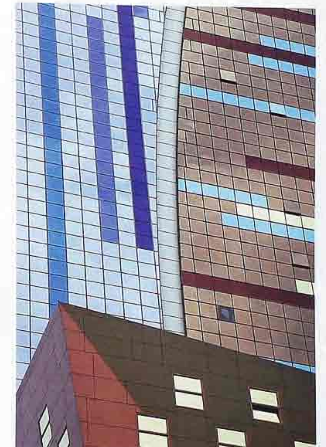
FA-125 Curtain-wall system of multicolored panels, supergraphic, modern commercial building
