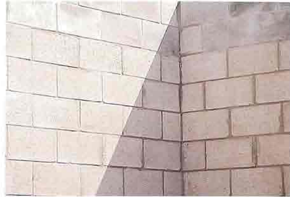
WA-222 Inside corner of mortared structural-block walls in running bond
