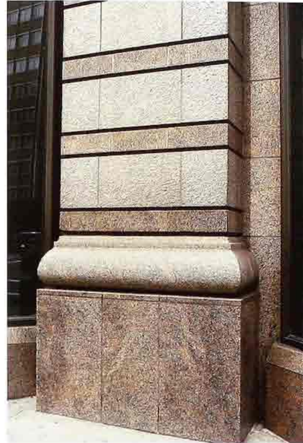
CP-45 Banded granite veneer pilaster on Tuscan-style base, entry of modern commercial building
