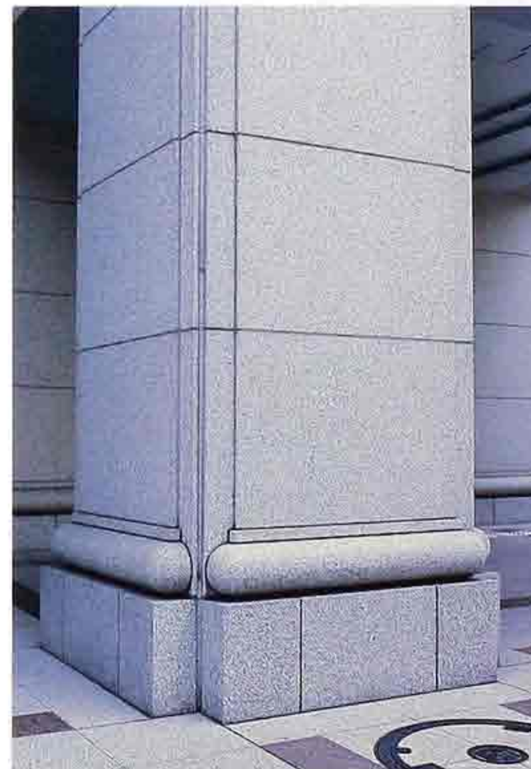
CP-47 Pier of granite veneer on Tuscan-style base, entry of modern commercial building
