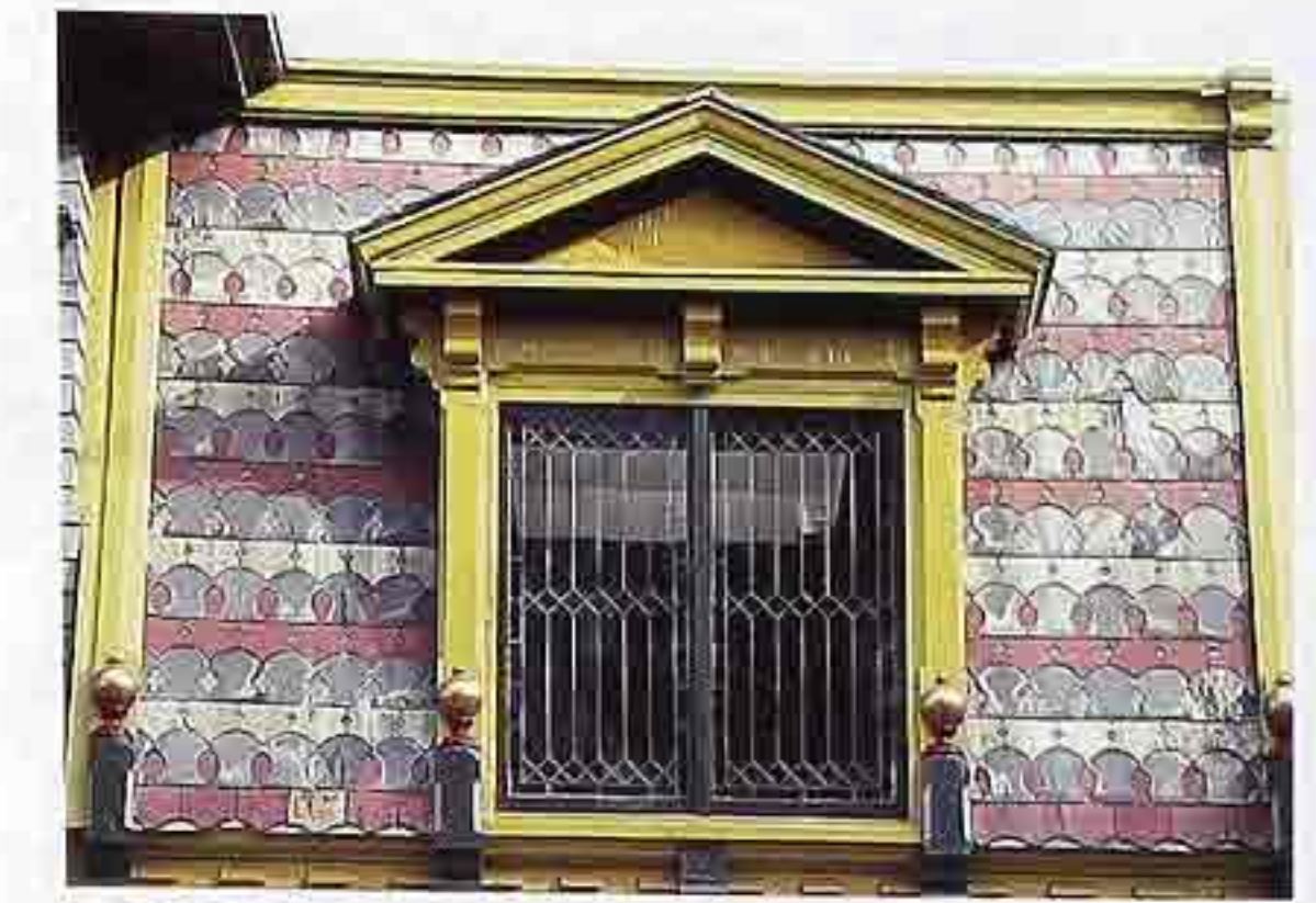
CR-59 Scalloped slate roofing in banded polychrome patterns around pedimented dormer
