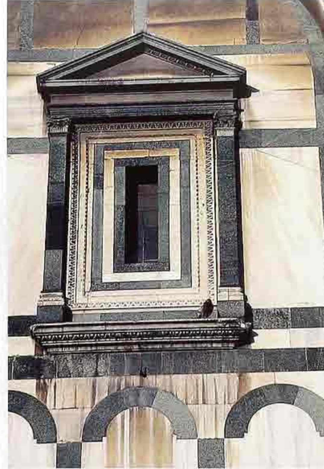
WI-133 Marble pediment and pilasters framing carved marble casing with polychrome marble bands, 12th-c. Italian church
