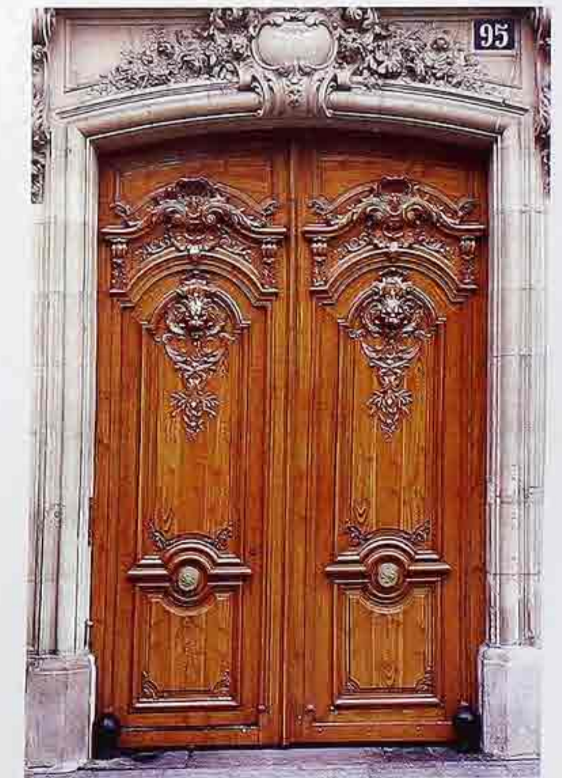
DW-8 Two panels, double doors with carved bas-relief ornament and trompe l'oeil wood finish. Cambered stone arch doorway with cartouche keystone
