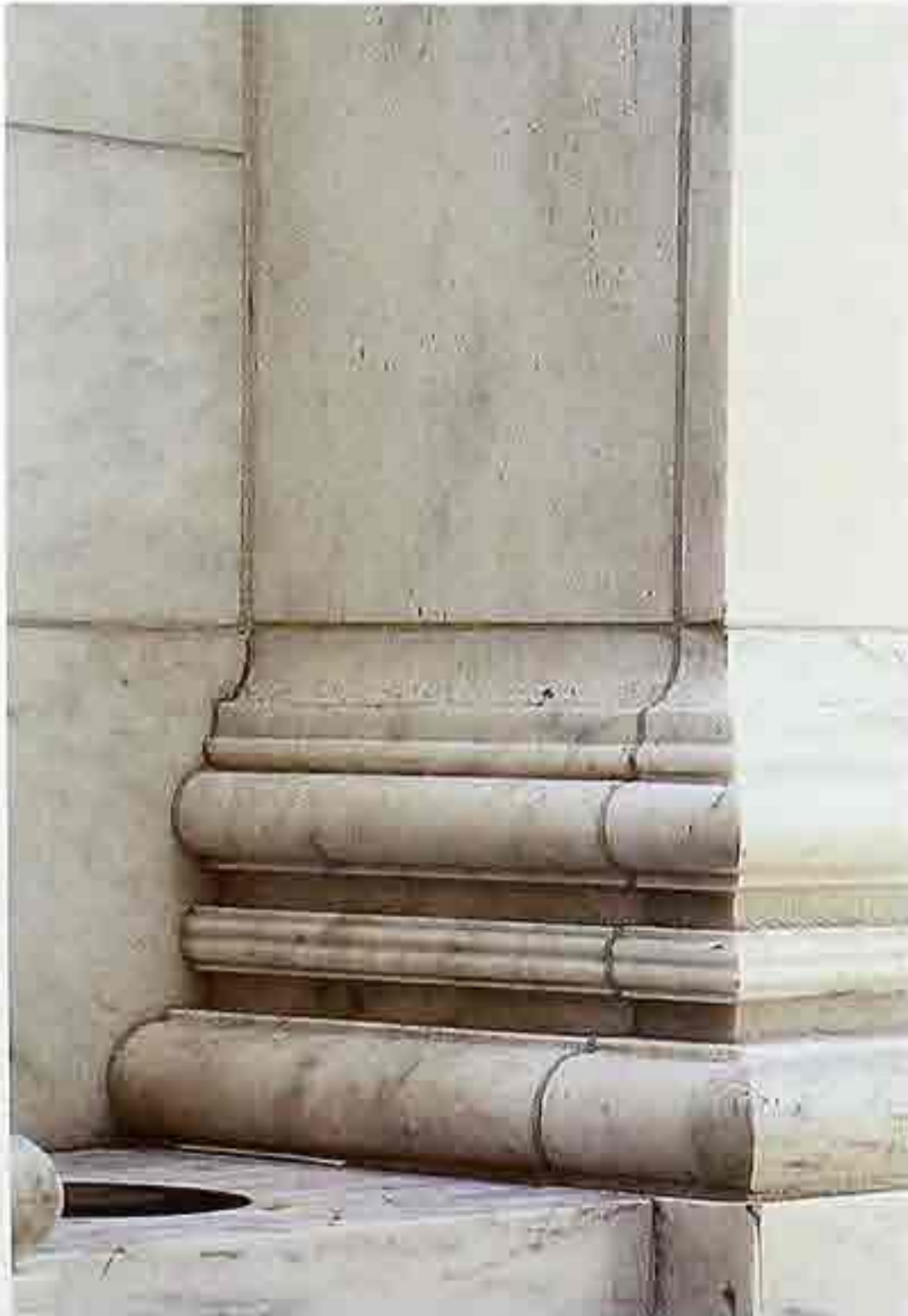
CP-43 Square pilaster with typical Roman Corinthian Ionic base; mason's miter on outside corner
