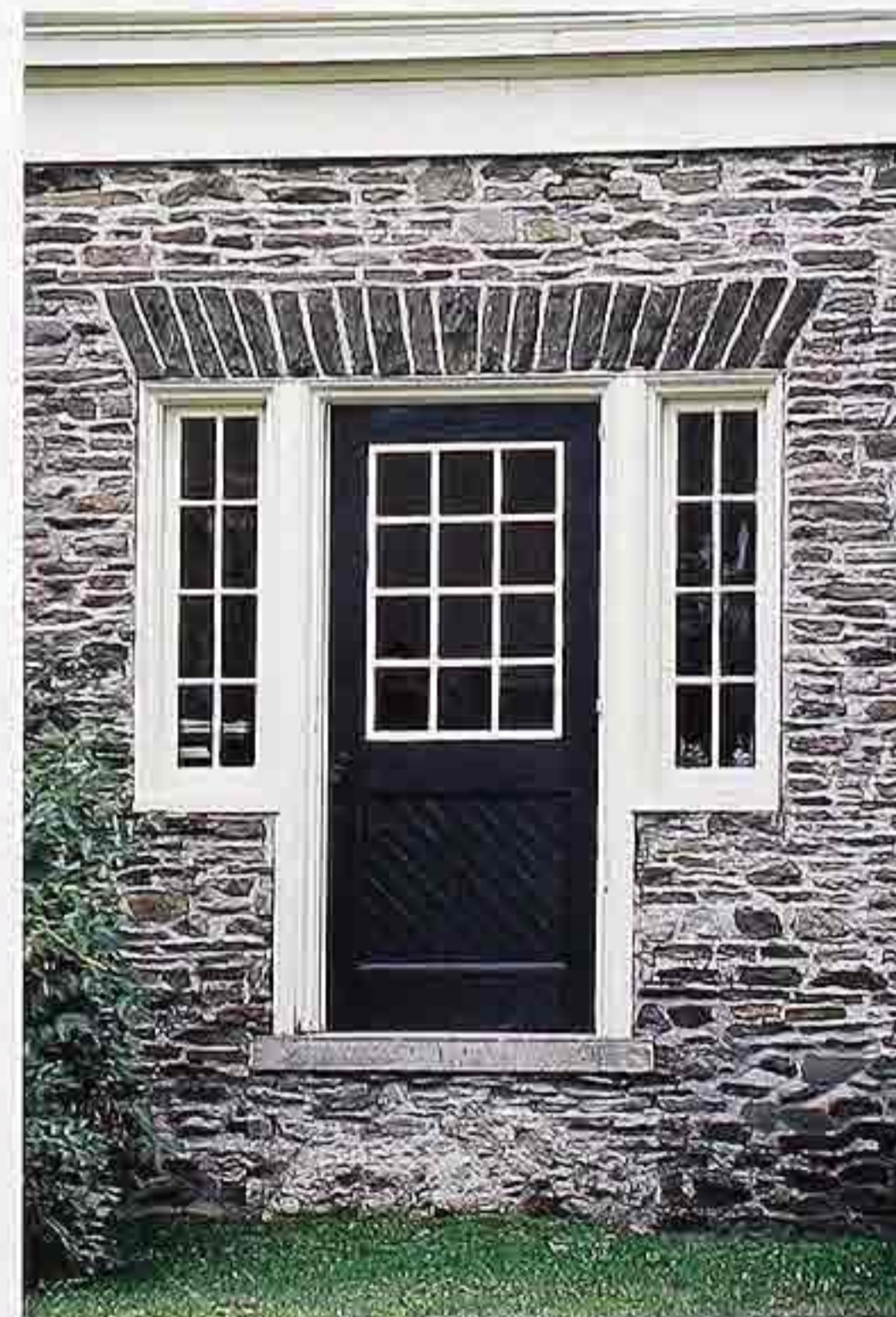
DW-64 Side lights flanking twelve-light painted wood paneled door; gauged-brick jack arch in fieldstone wall; American colonial village building
