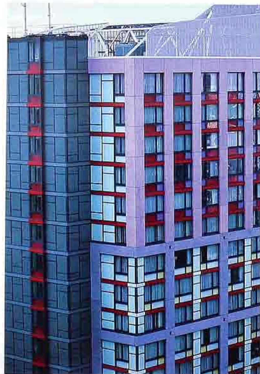
FA-131 Trabeated facade with multicolored infill and spandrel panels, modern commercial building
