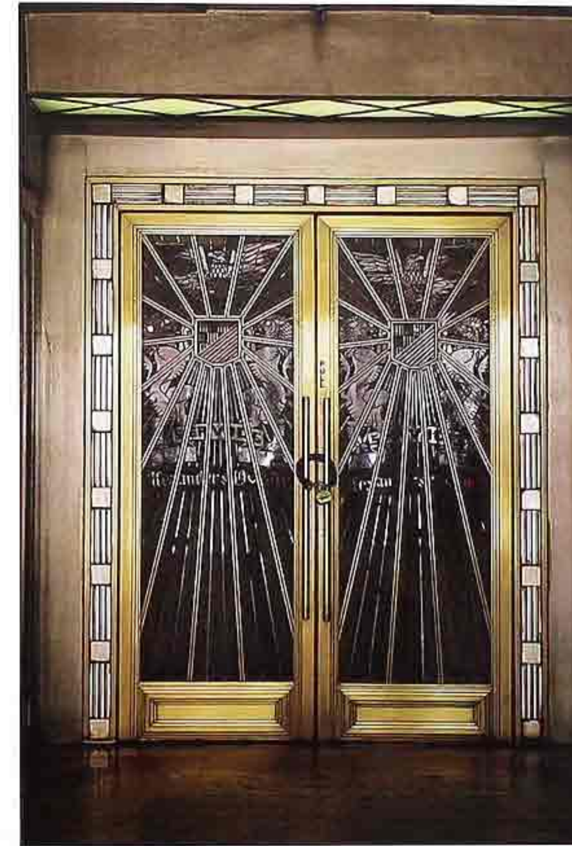
DW-49 Brass double doors; full glass with radial muntins or grille; brass doorframe; Art Deco commercial building
