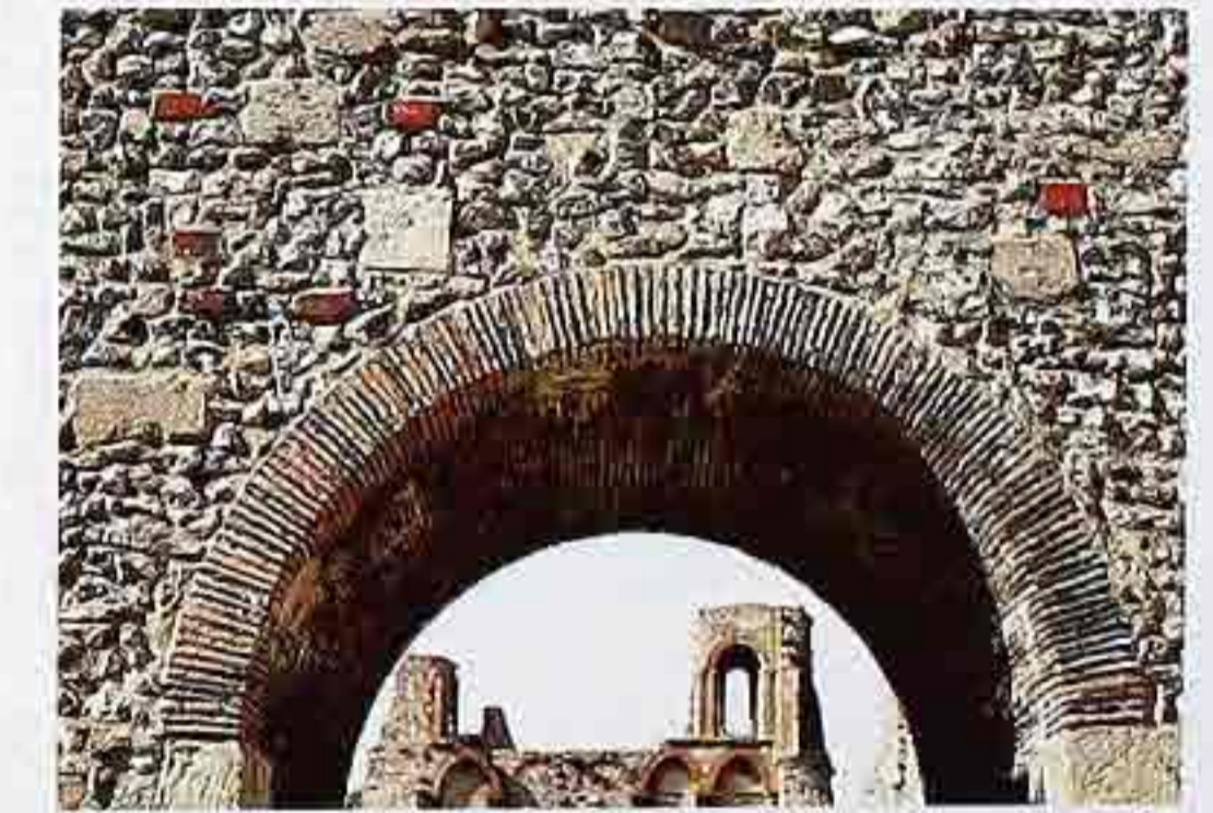
CP-153 Semicircular Roman brick arch in random rubble wall
