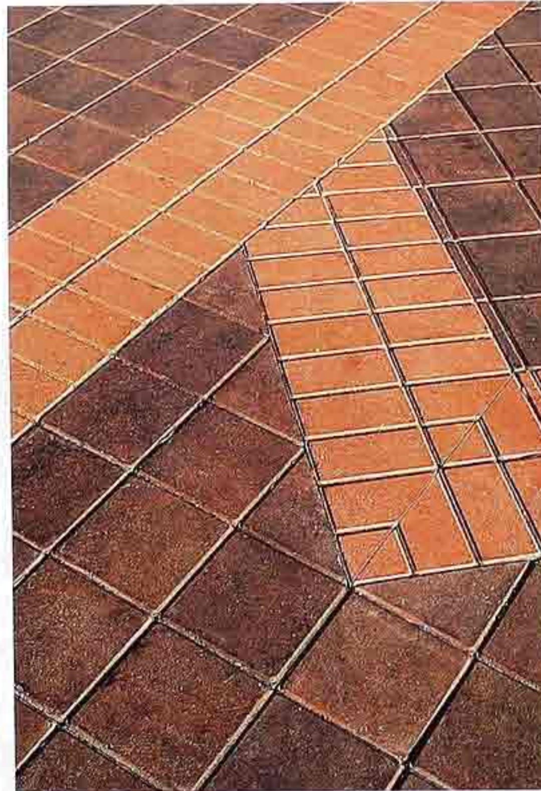
FP-82 Pre-cast concrete pavers; double soldier course in straight-joint-course field; flexible paving, urban public space
