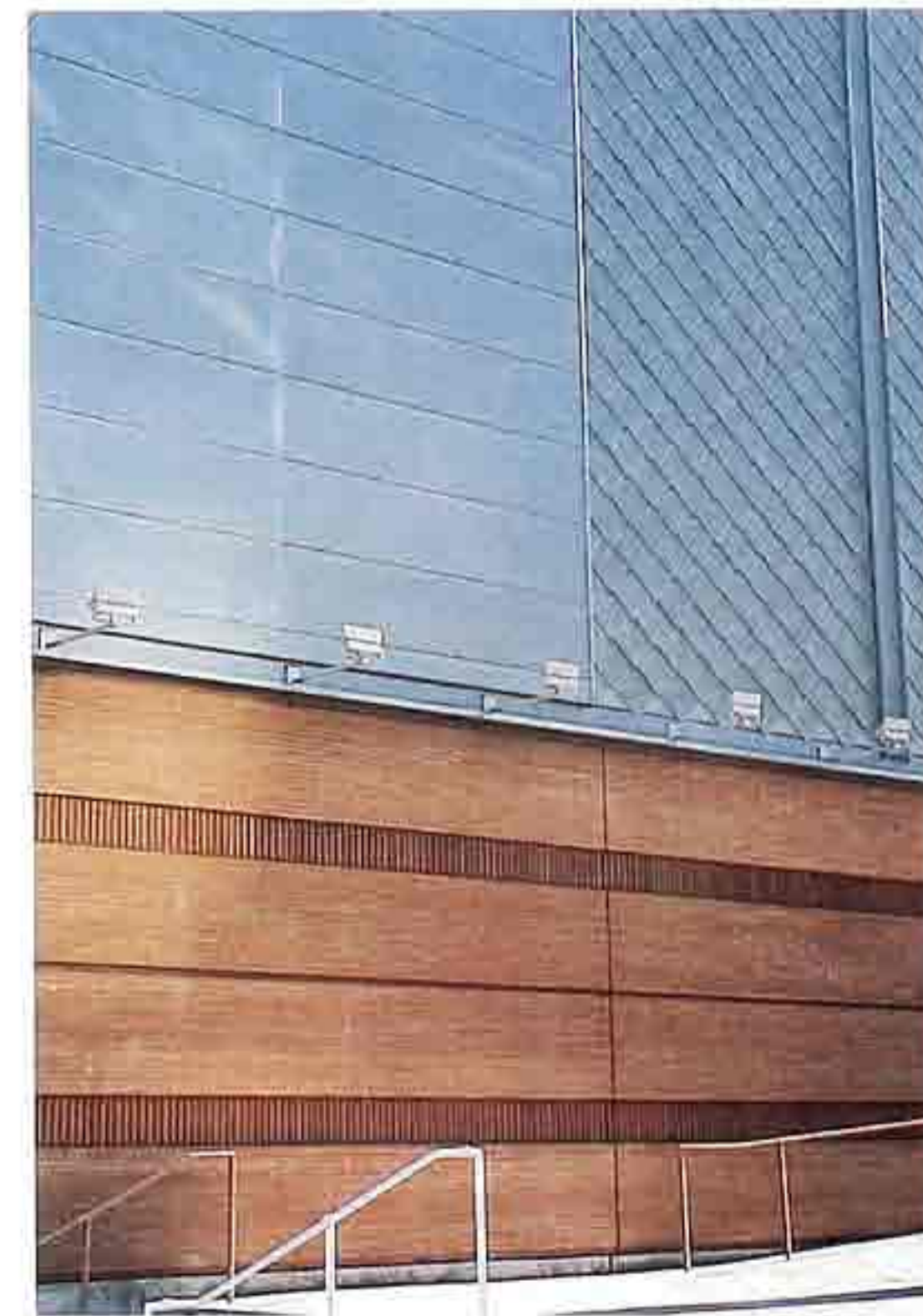
WA-309 Interior metal cladding with banded brick below, modern industrial building
