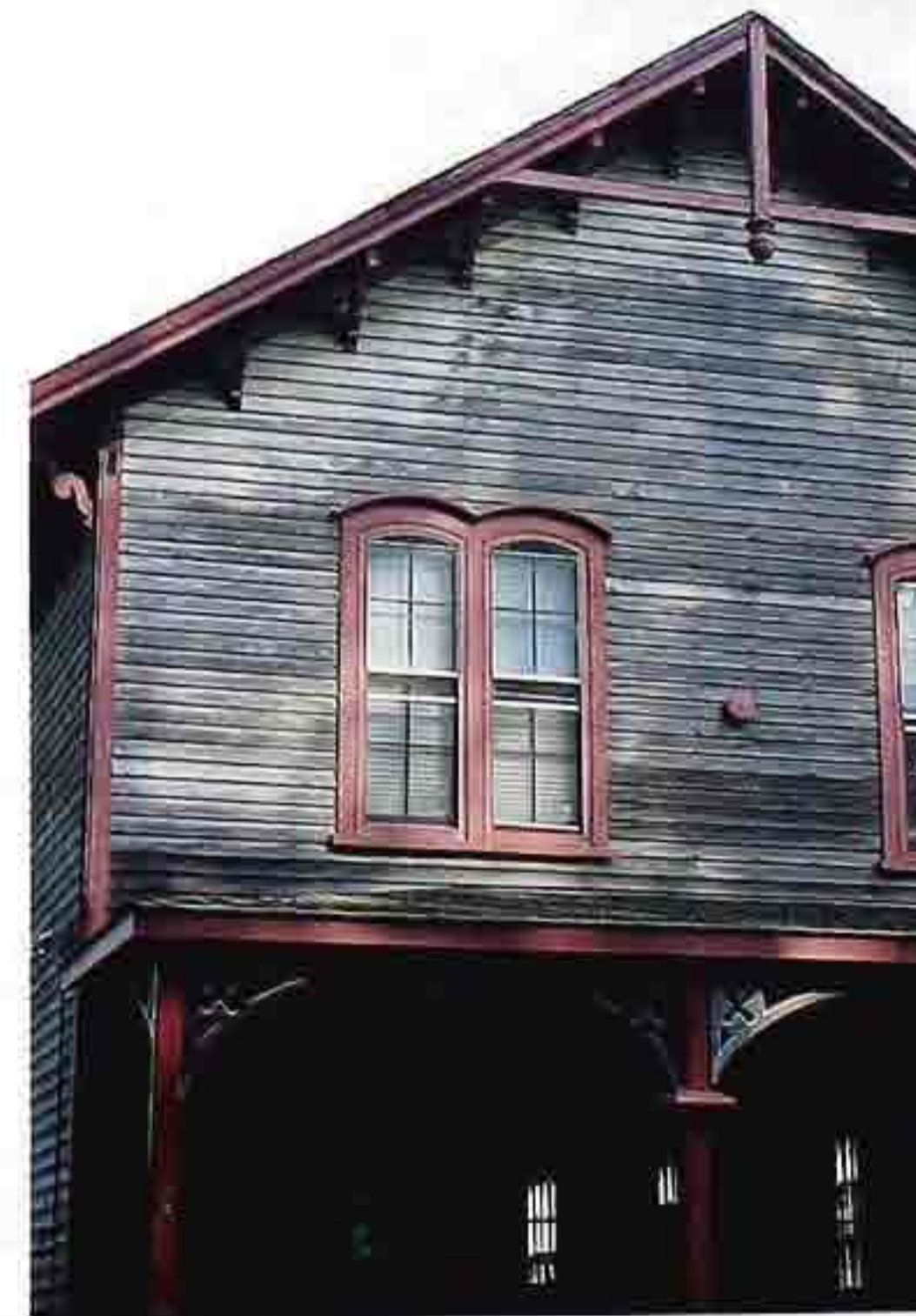
WI-53 Four-over-four double-hung windows with wood frames and modern storm windows, 19th-c. clapboard house
