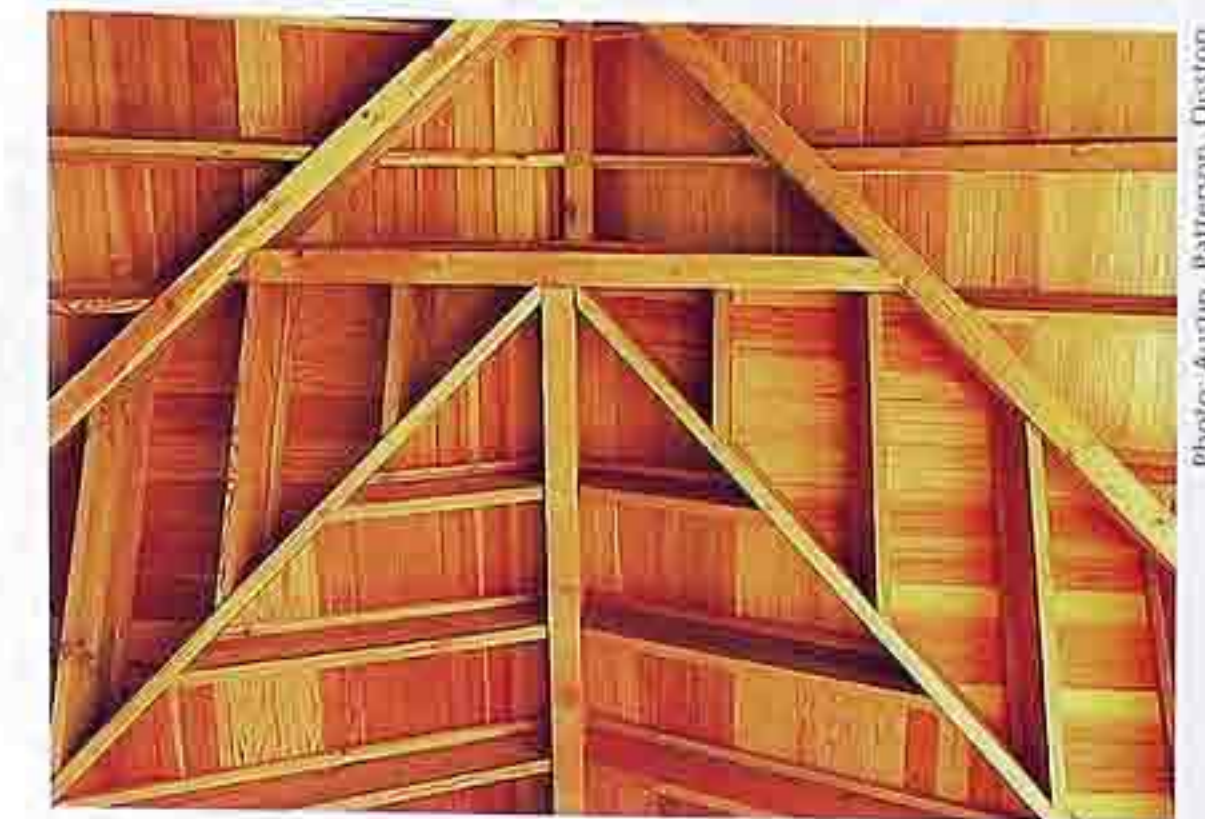
CR-6 Exposed select-fir framing in residential common room
