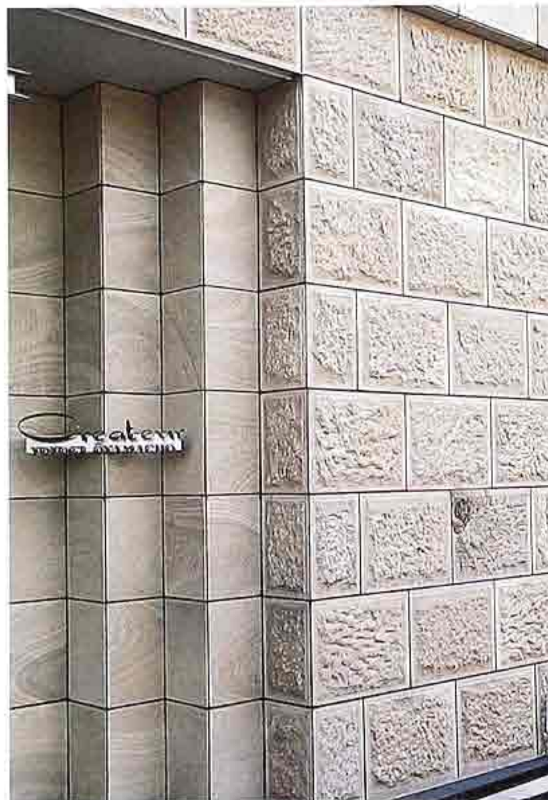
WA-132 Corner of rusticated running bond with reveal; sand-finish pilaster strips in stack bond on entry, modern commercial building
