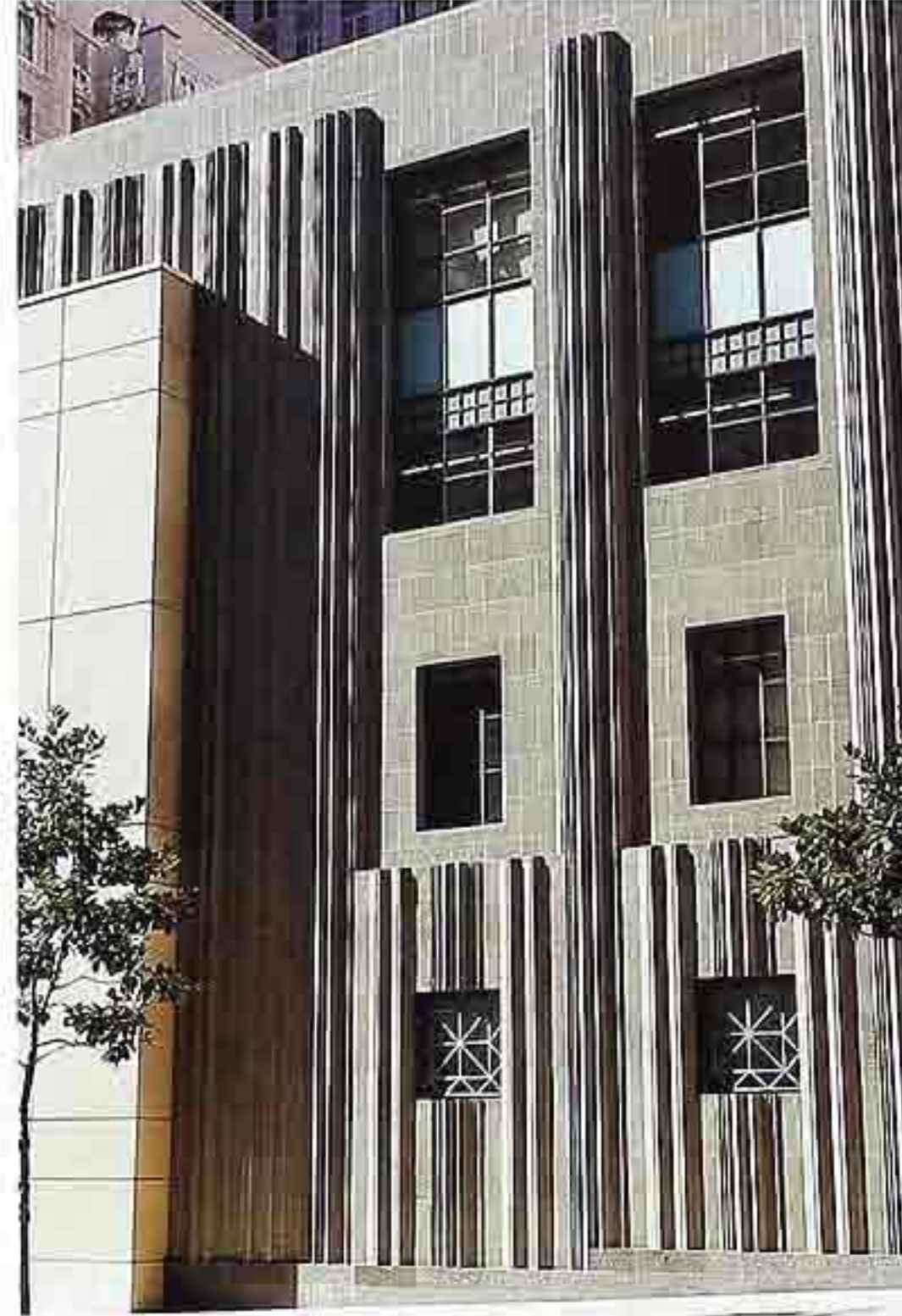
CP-97 Fluted and reeded pilasters on Art Deco facade
