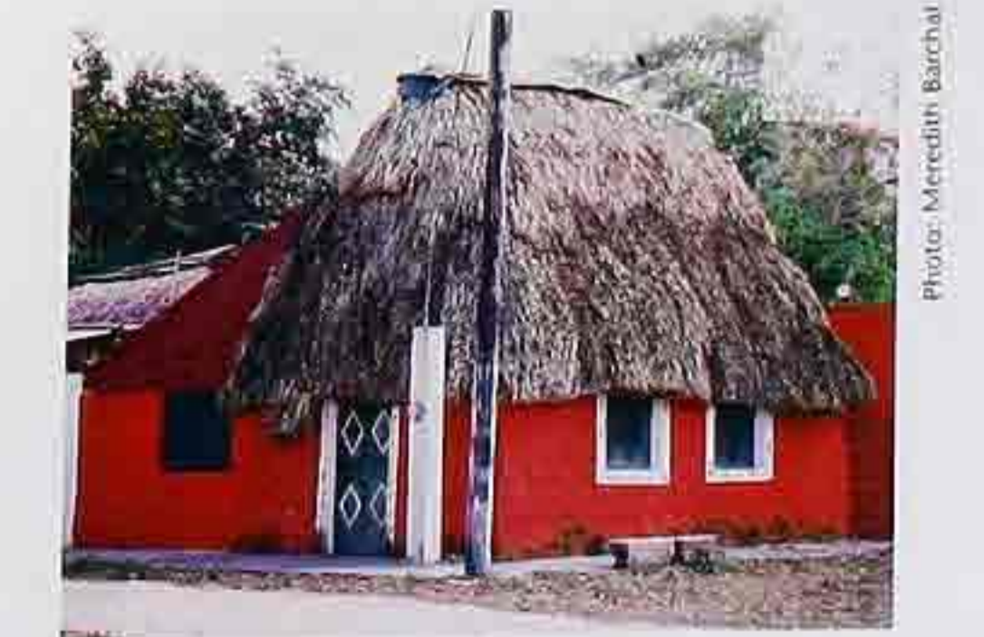
CR-75 Thatched roof on house, Latin-America
