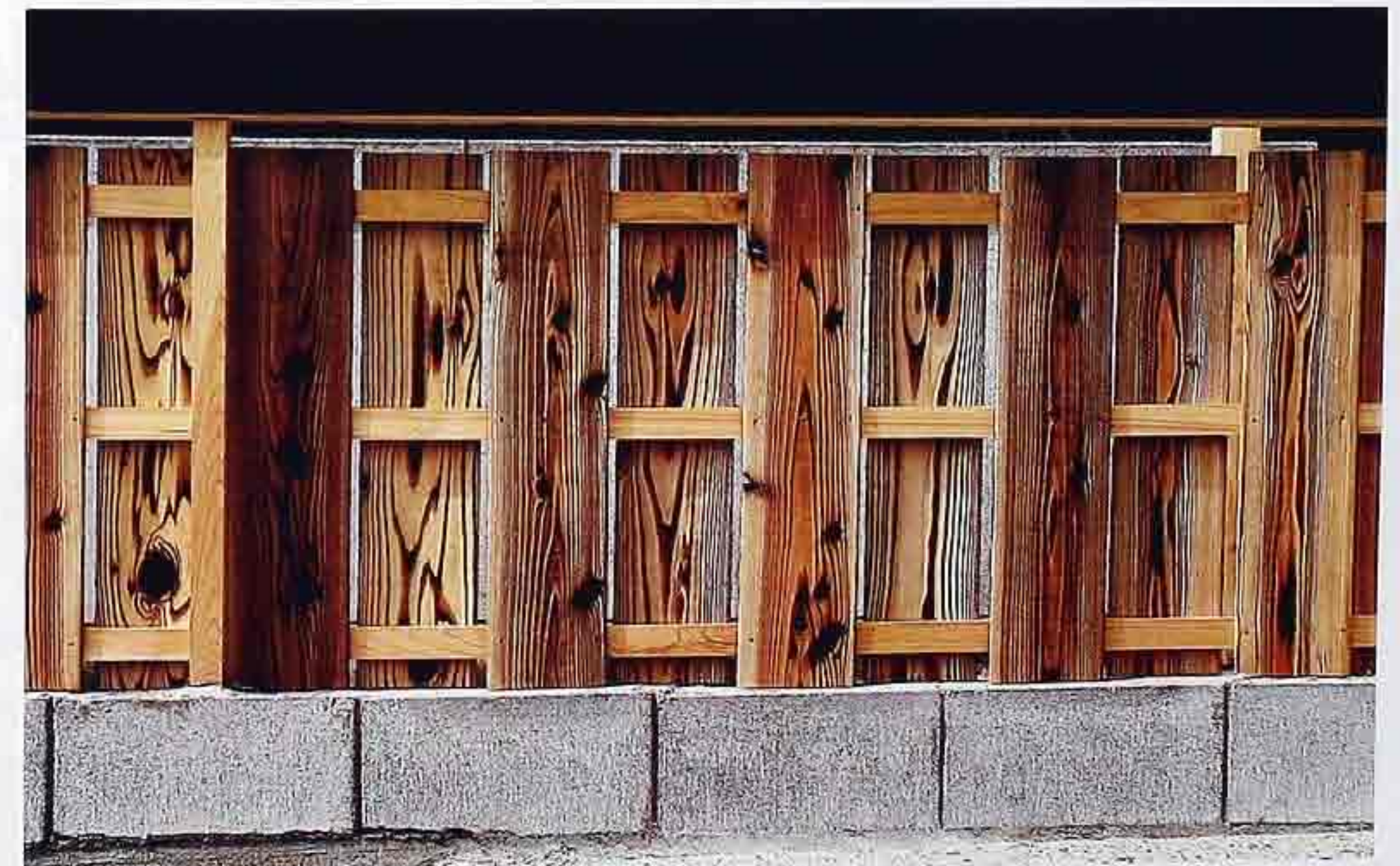
WA-17 Low entry wall of boxed plain-sawn planks on stone base
