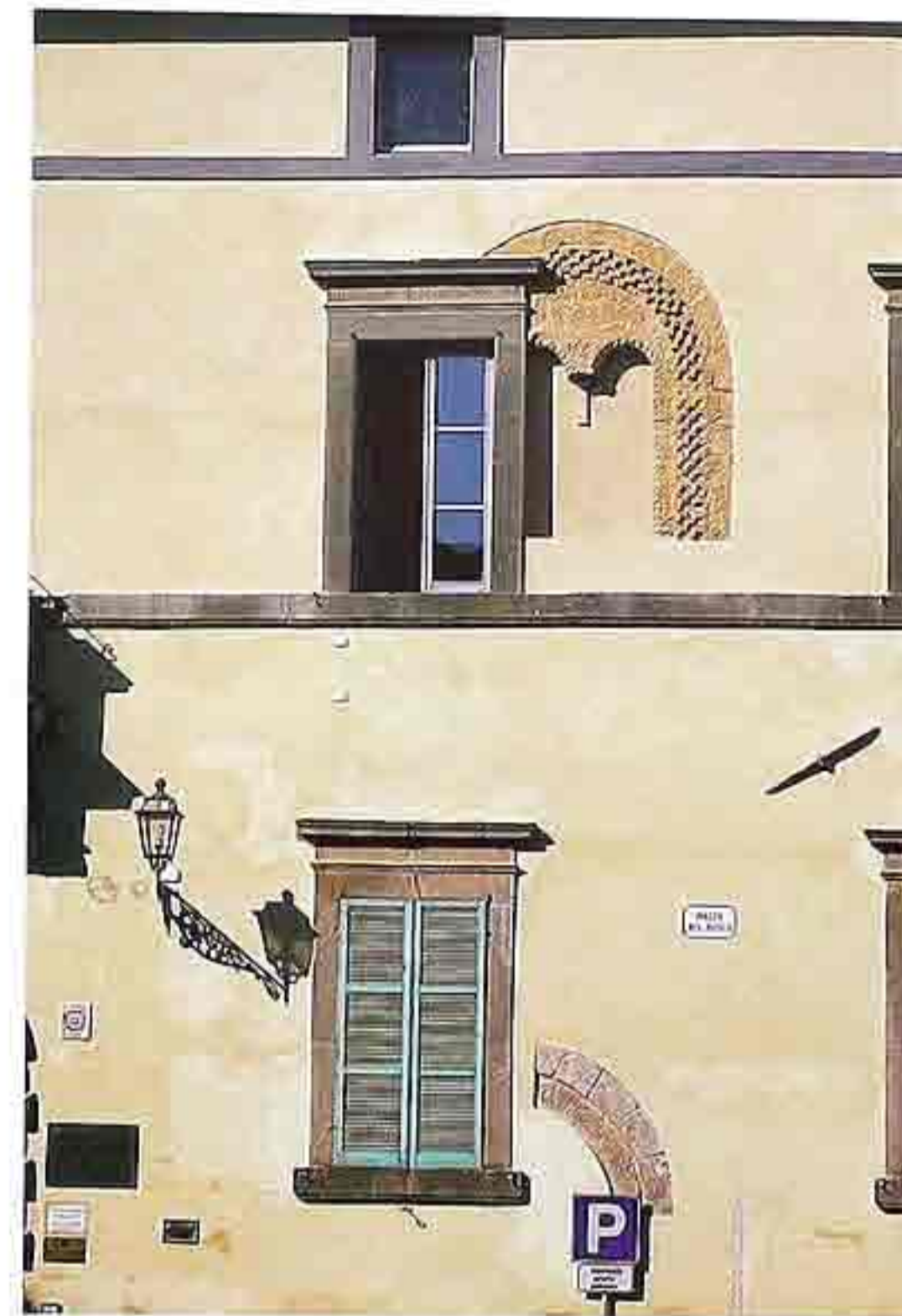
FA-115 Stucco facade with older arches embedded in the wall adjacent to modern windows
