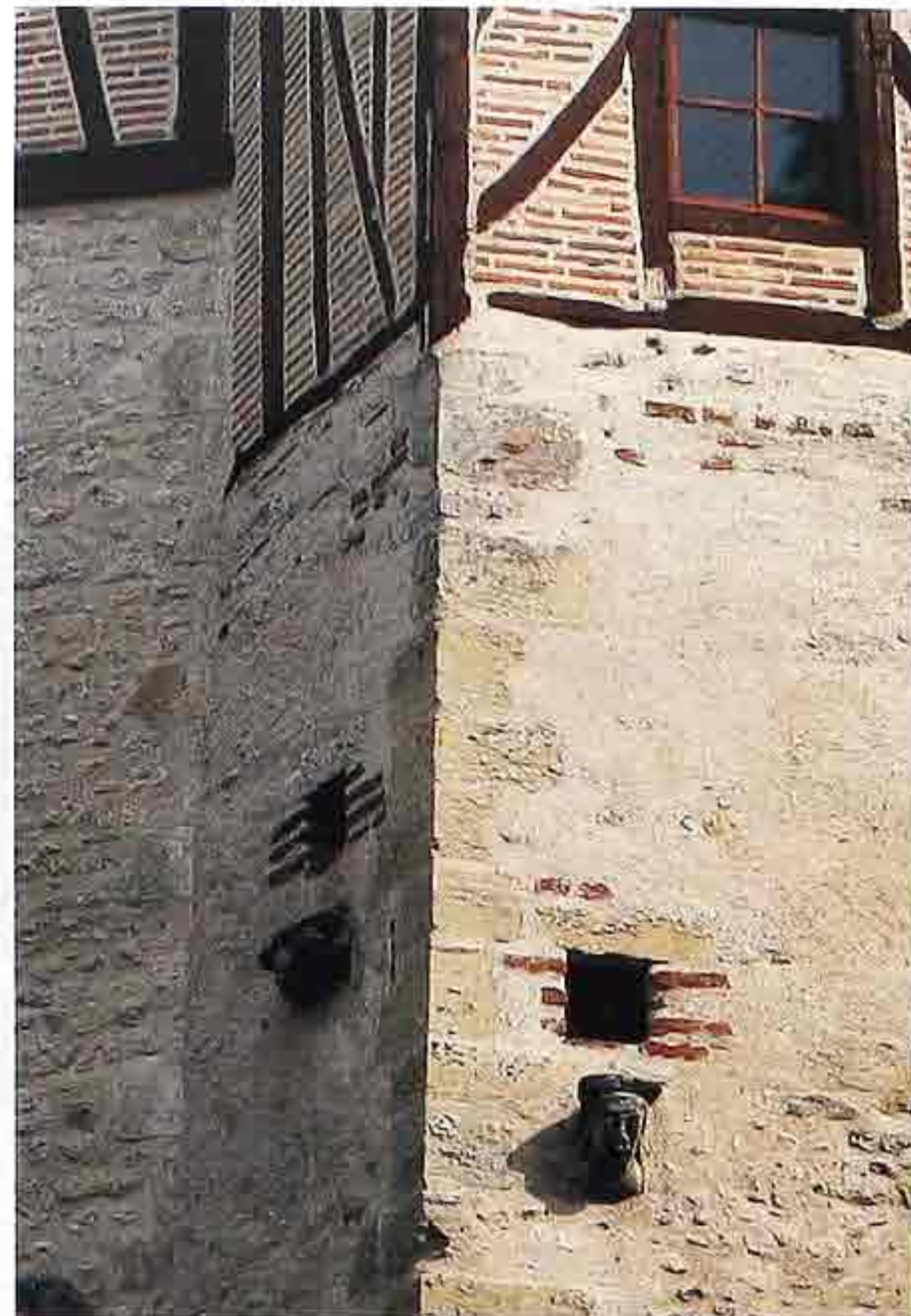
WA-291 Half-timber upper story with brick infill and stucco lower story with stone quoins
