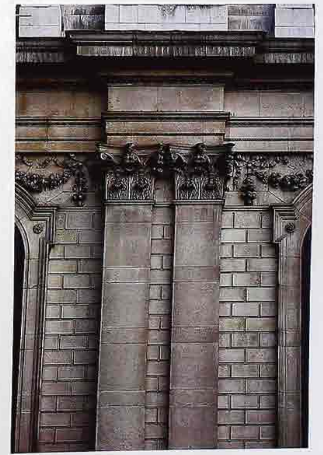
OM-104 Two-banded architrave, festooned frieze flanking Corinthian pilasters
