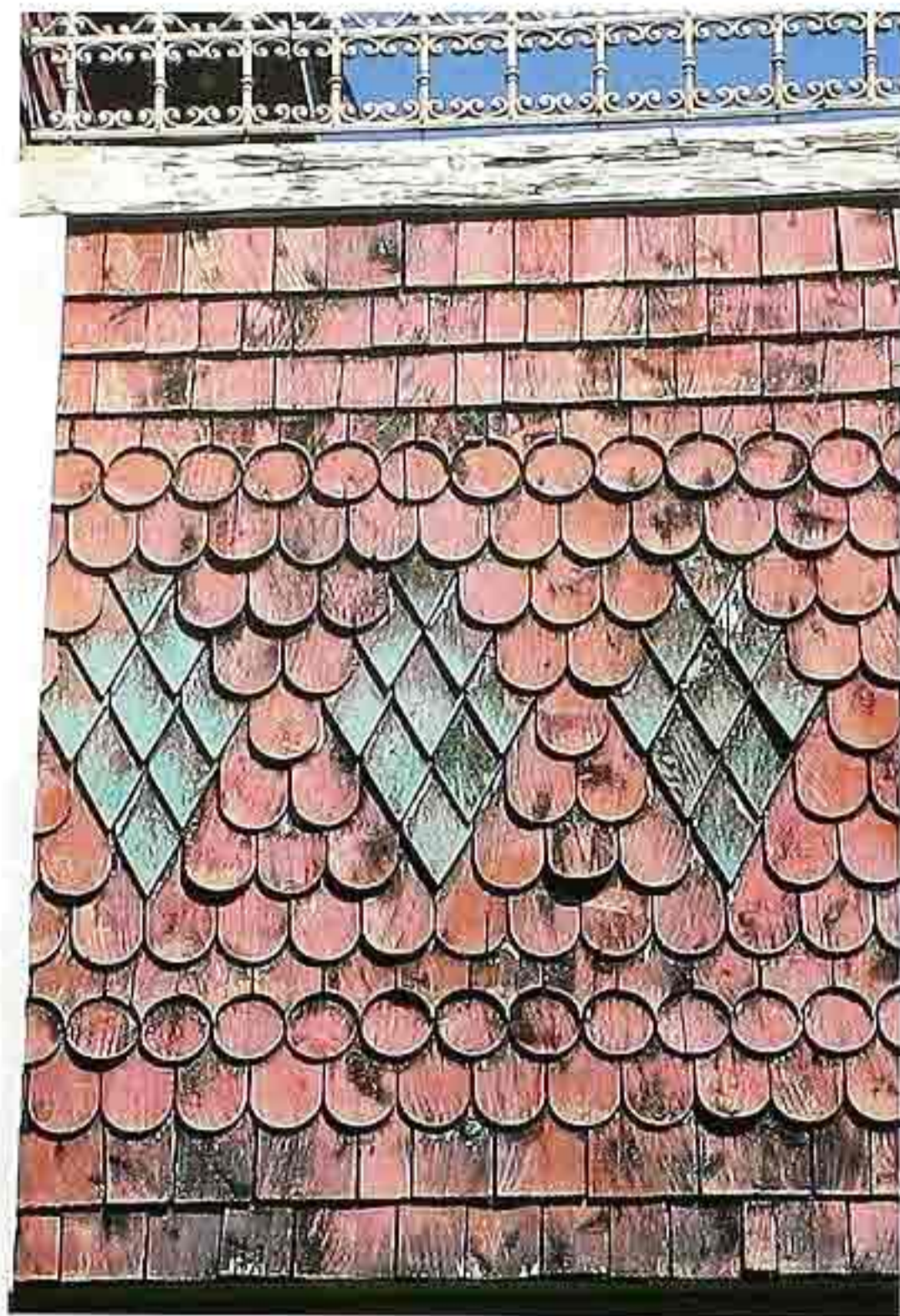
CR-64 Scalloped and diamond-shaped painted wood shingles
