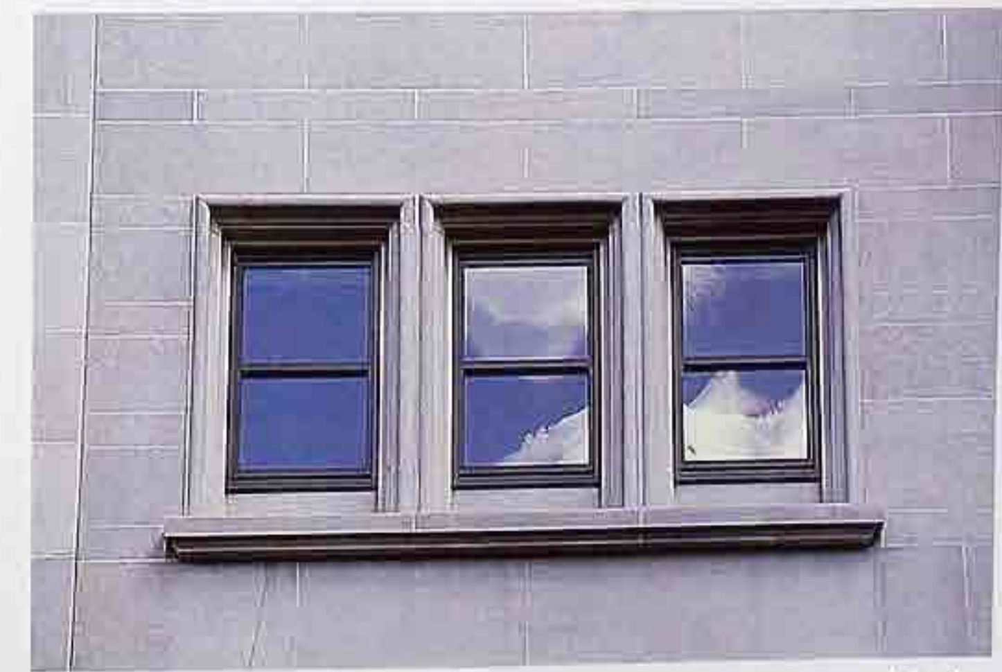
WI-131 Set of three recessed windows with stone molded casings and single molded sill, early 20th-c. commercial building
