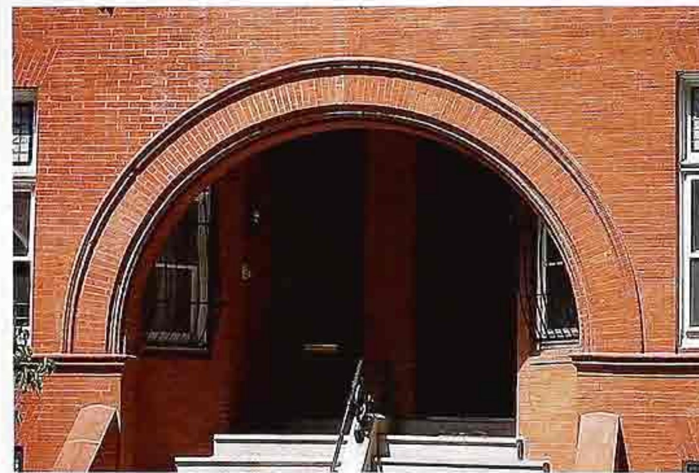
CP-157 Semicircular gauged-brick arch over entryway
