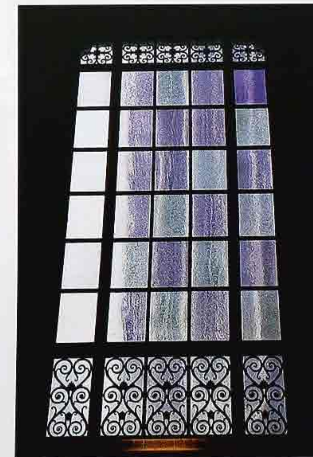
WI-18 Antique colored glass, lobby of 19th-c. mixed-use building
