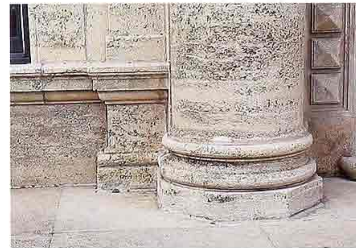
CP-37 Attic base of travertine engaged column on octagonal plinth
