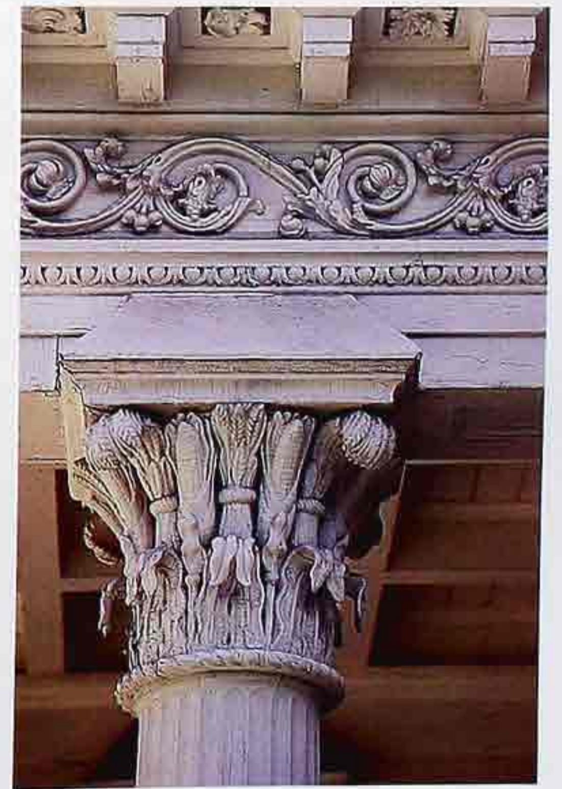
CP-24 American-order capital and entablature with egg-and-dart molding, arabesque frieze, and block modillions
