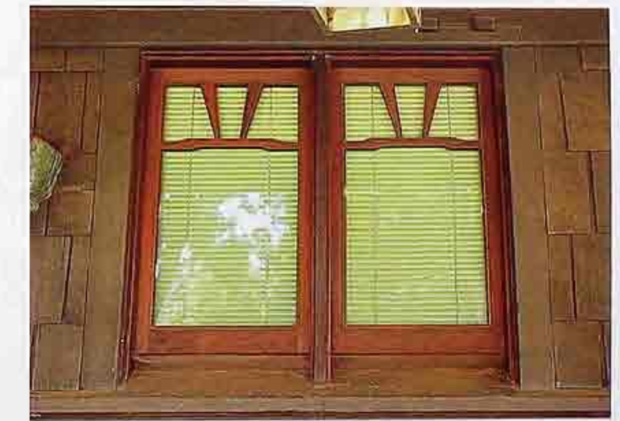
WI-28 Wood-framed awning windows with shaped wood muntins, Arts and Crafts house
