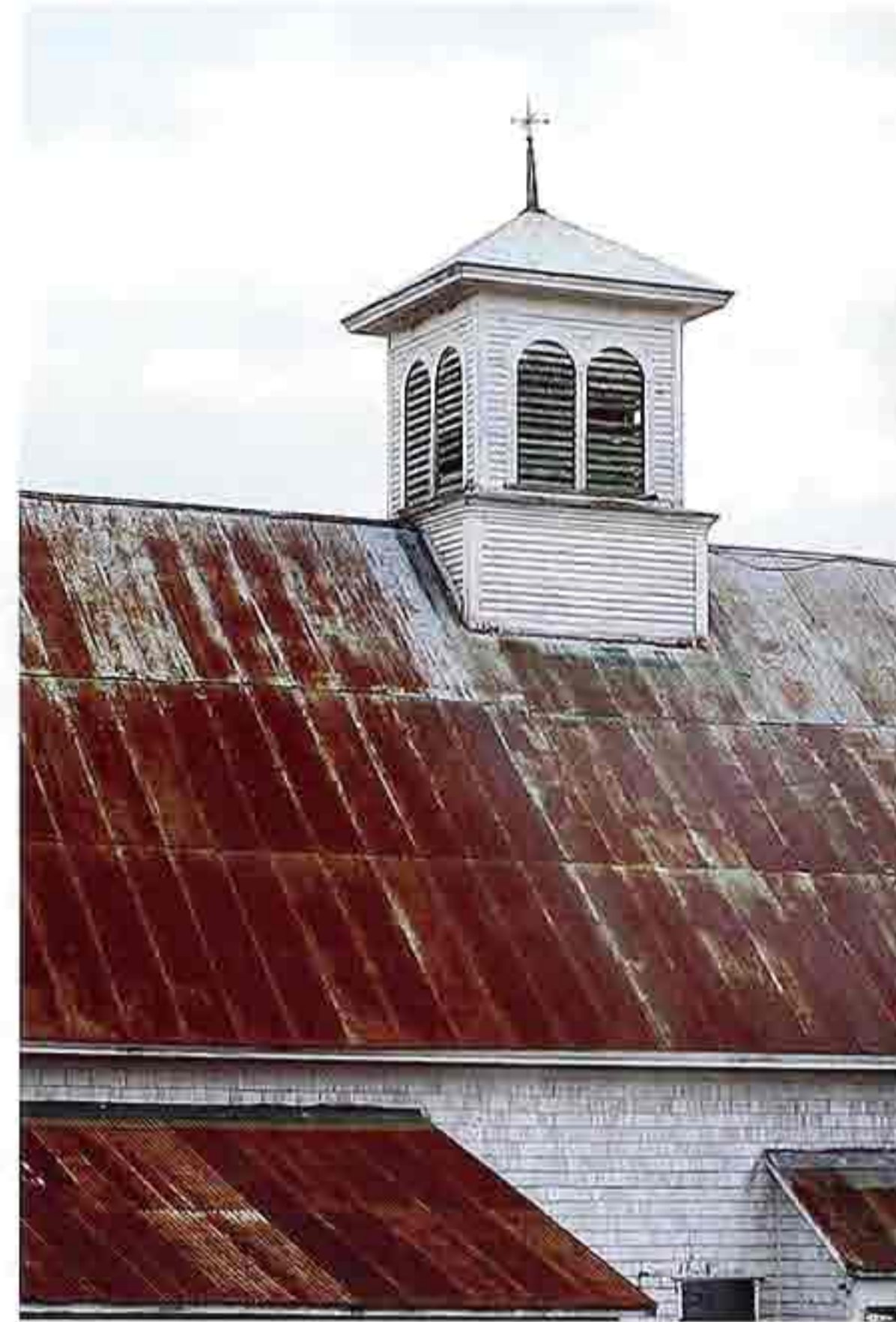
CR-38 Weathered corrugated metal barn roof with pyramidal roof on monitor
