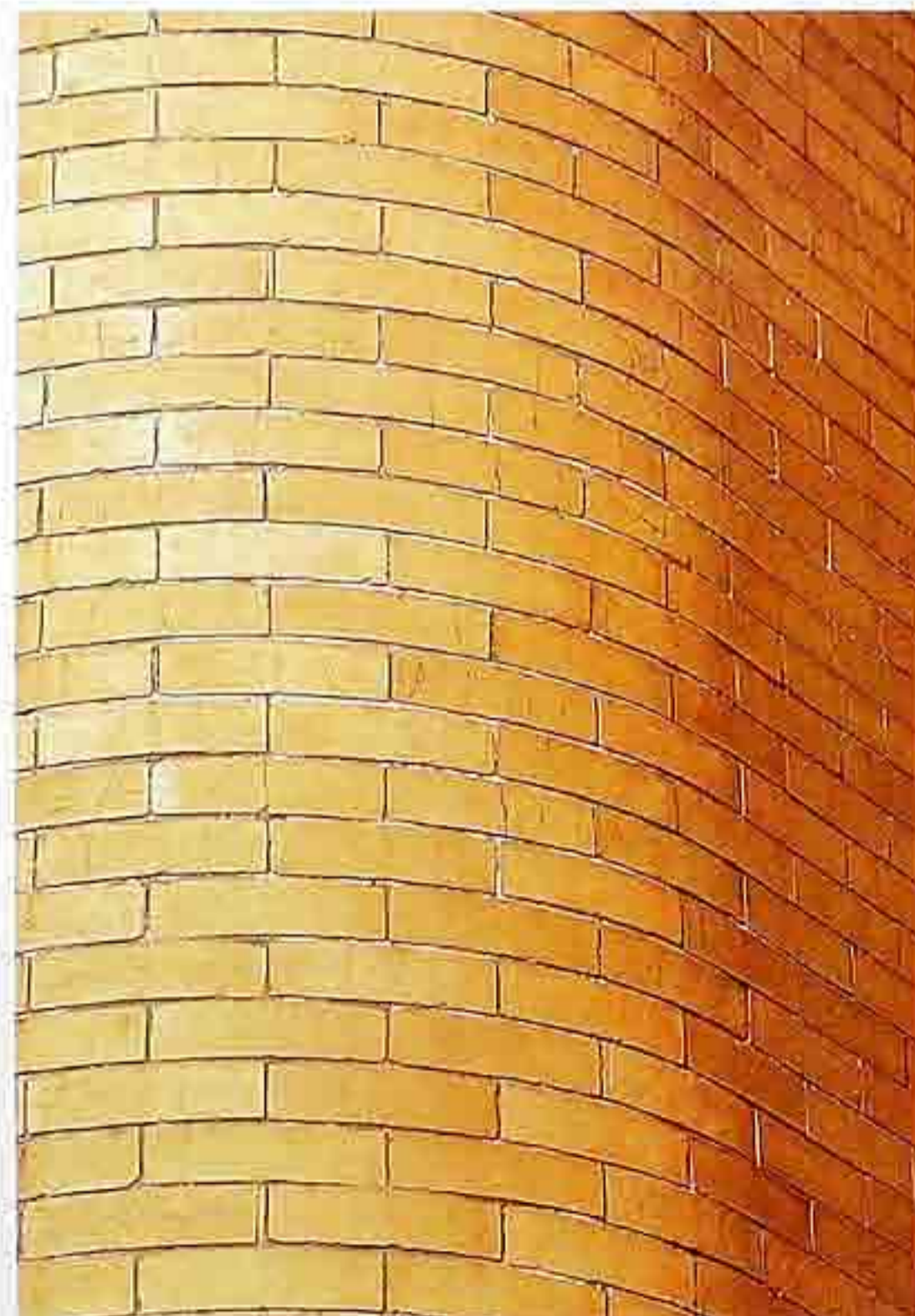
WA-168 Radial brick in running bond on curved wall
