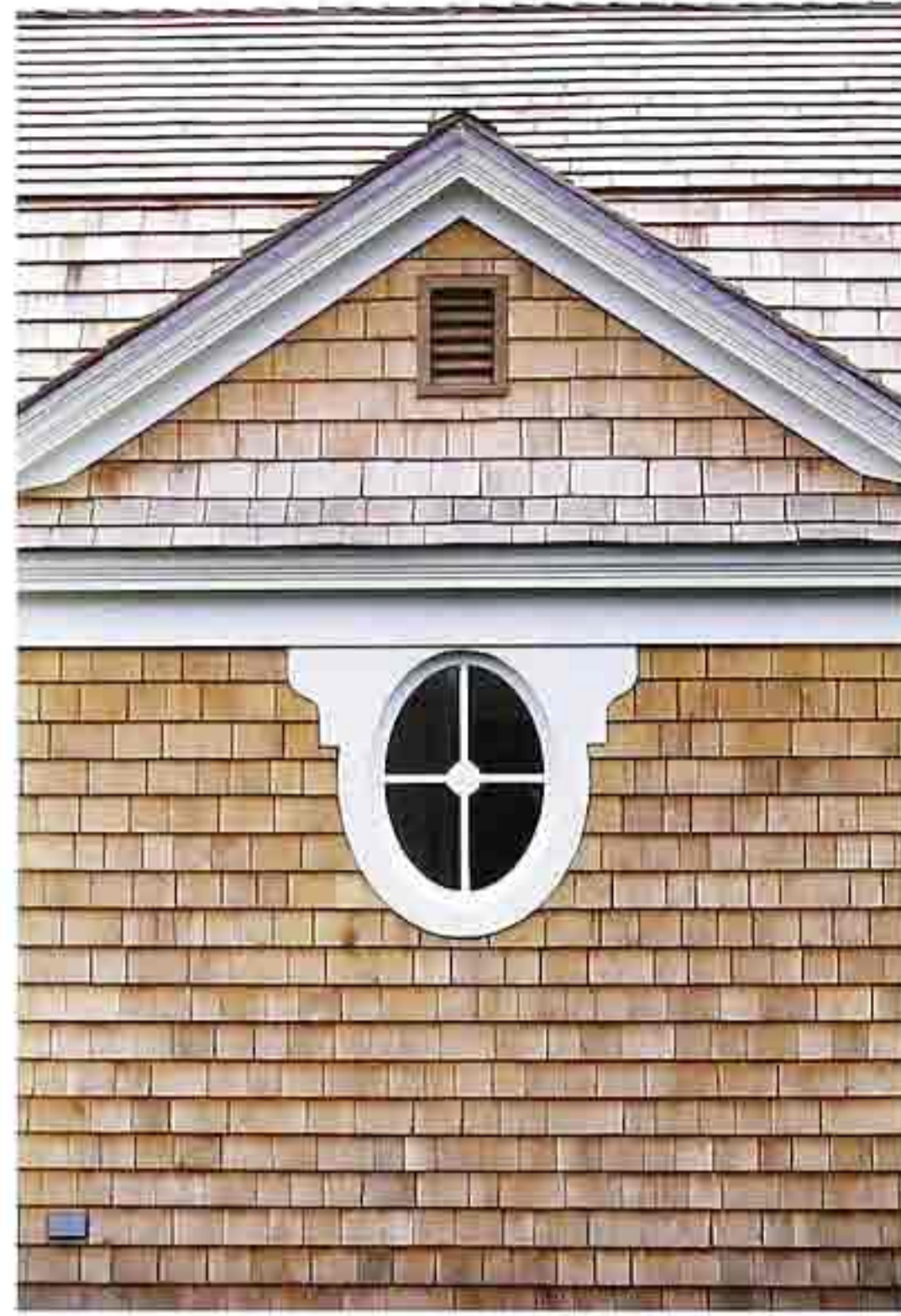
WI-66 Oval window divided by muntins, with flat wood casing in white cedar-shingle gable wall
