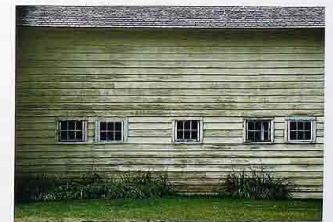
WA-25 Weathered painted clapboard wall with windows
