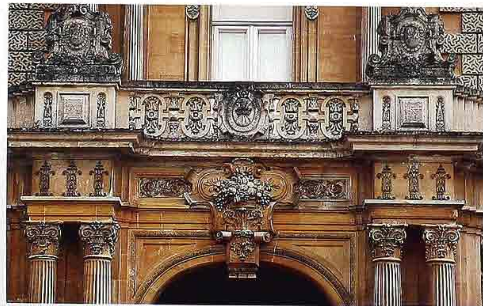
FA-123 Portal with coupled engaged columns and balcony heavily ornamented and embellished with cartouches, 18th-c. English country house
