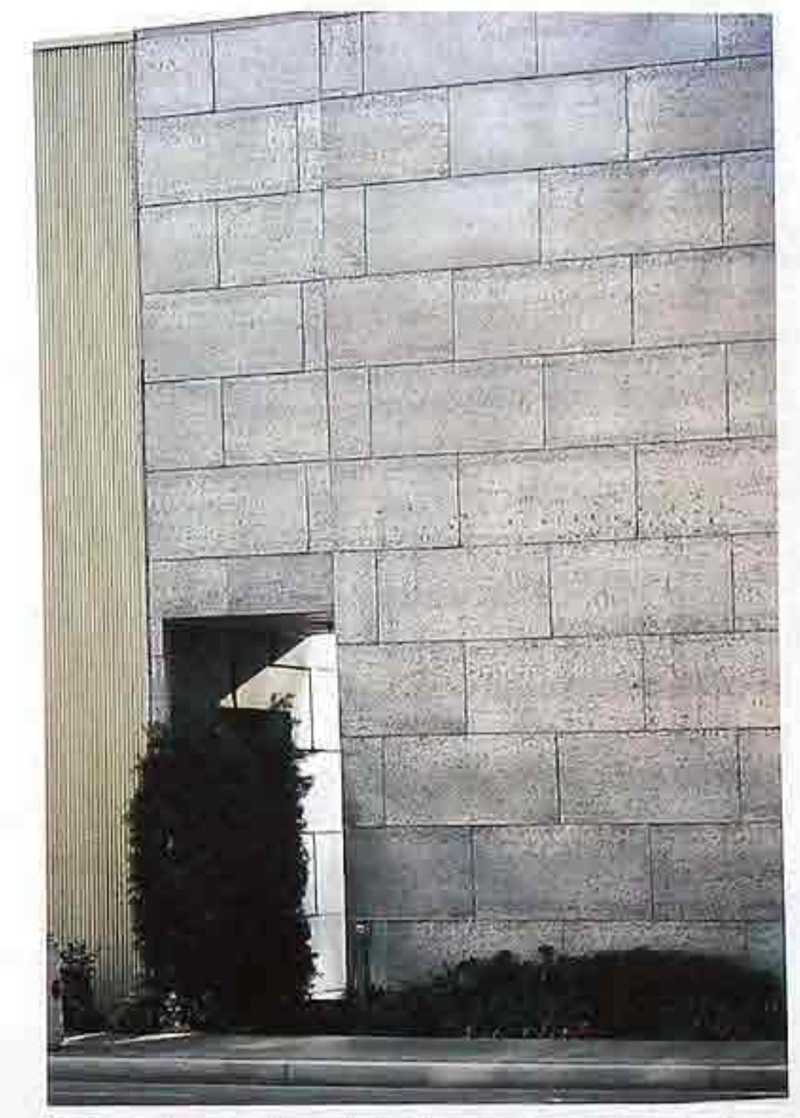
FA-16 Galvanized metal cladding in running-bond pattern
