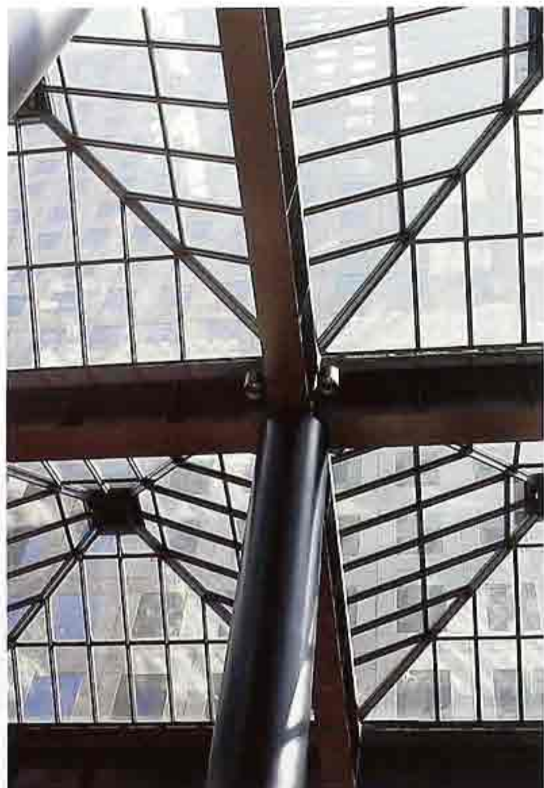
CP-112 Steel frame and tubular column; wide-flange beams supporting framed glass ceiling of modern commercial building
