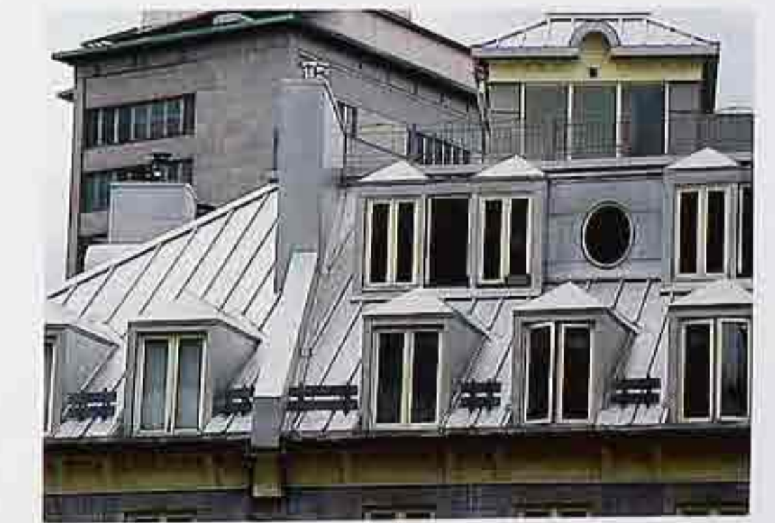
CR-102 Hipped-roof dormers on metal hipped roof with pipe snow guards, modern apartment house
