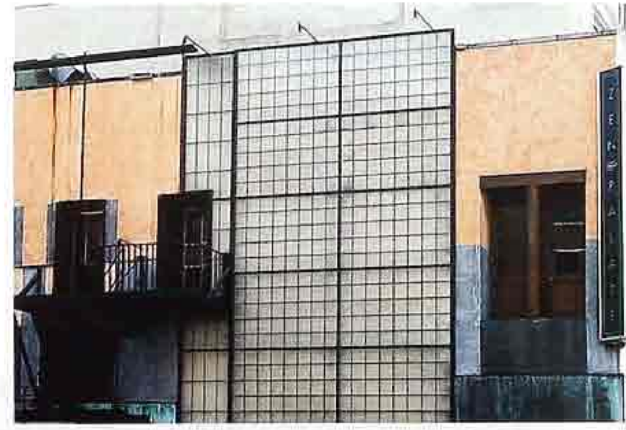
WA-298 Metal-framed glass panels with colored and patinated metal, modern commercial building
