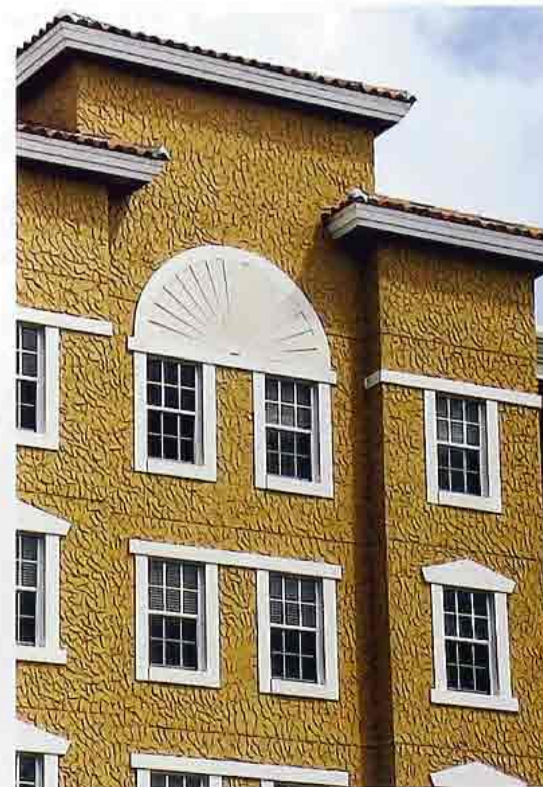
WA-246 Colored stucco with knocked-down skip-trowel finish on wall; double hung windows, Italian-villa-style modern apartment house
