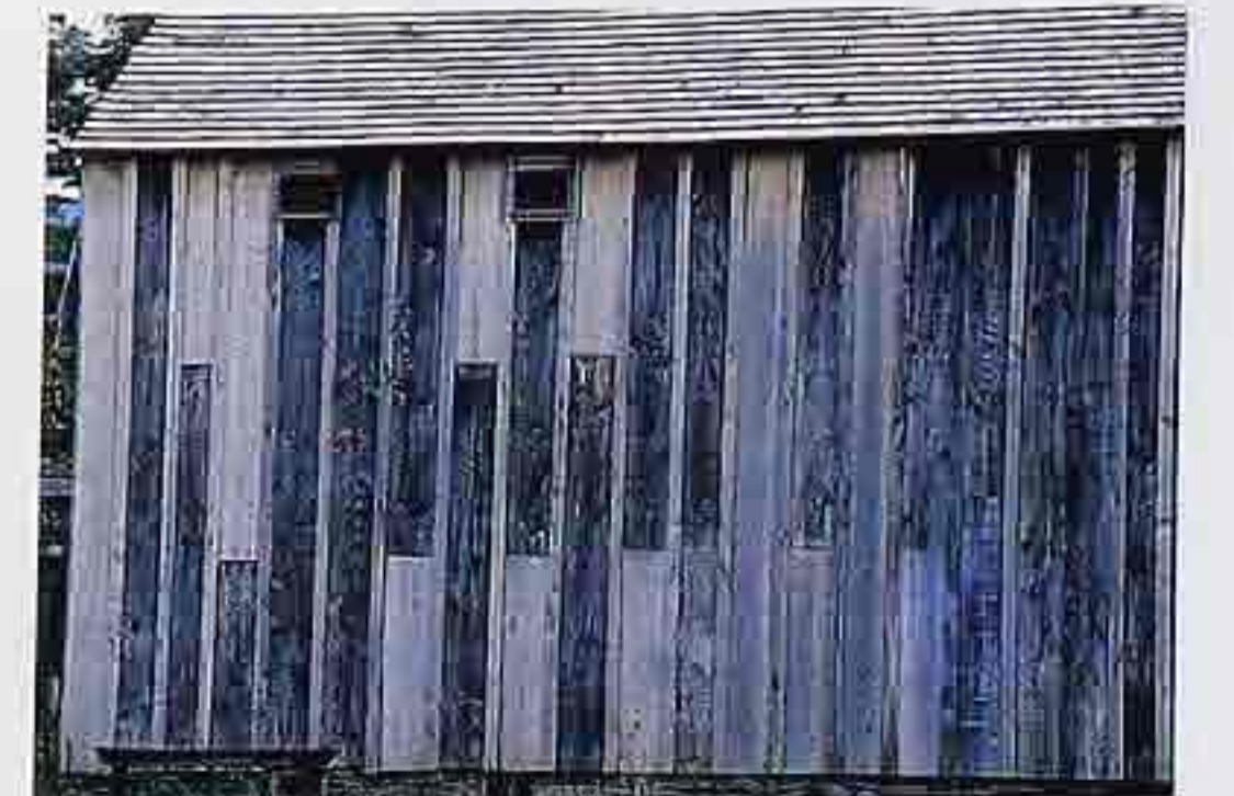
WA-27 Weathered board-and-batten siding on outbuilding
