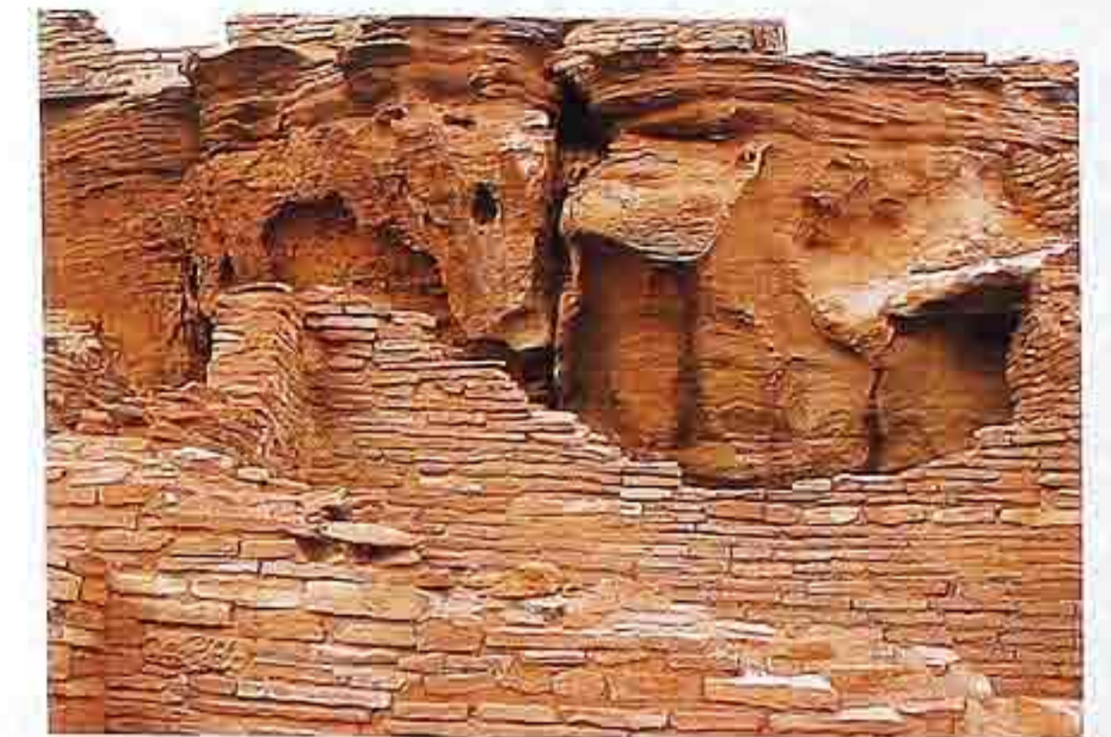
WA-77 Roughly squared sandstone in random ashlar attached to natural stone wall
