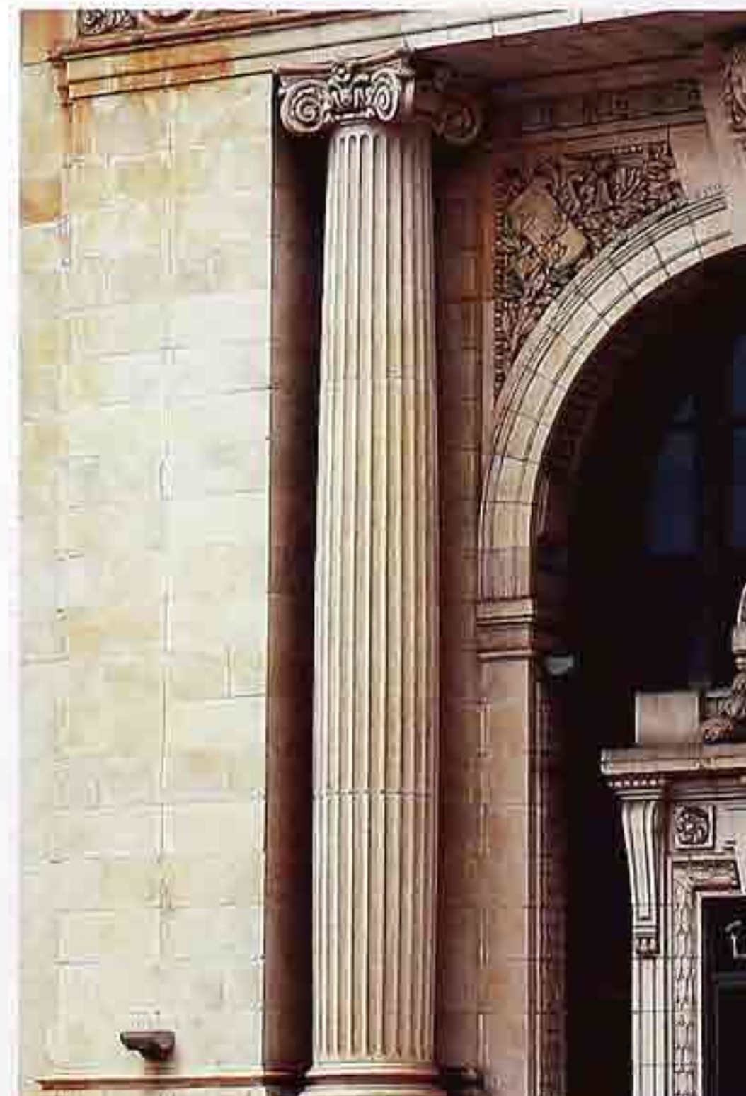
CP-78 Ionic fluted column with pronounced entasis
