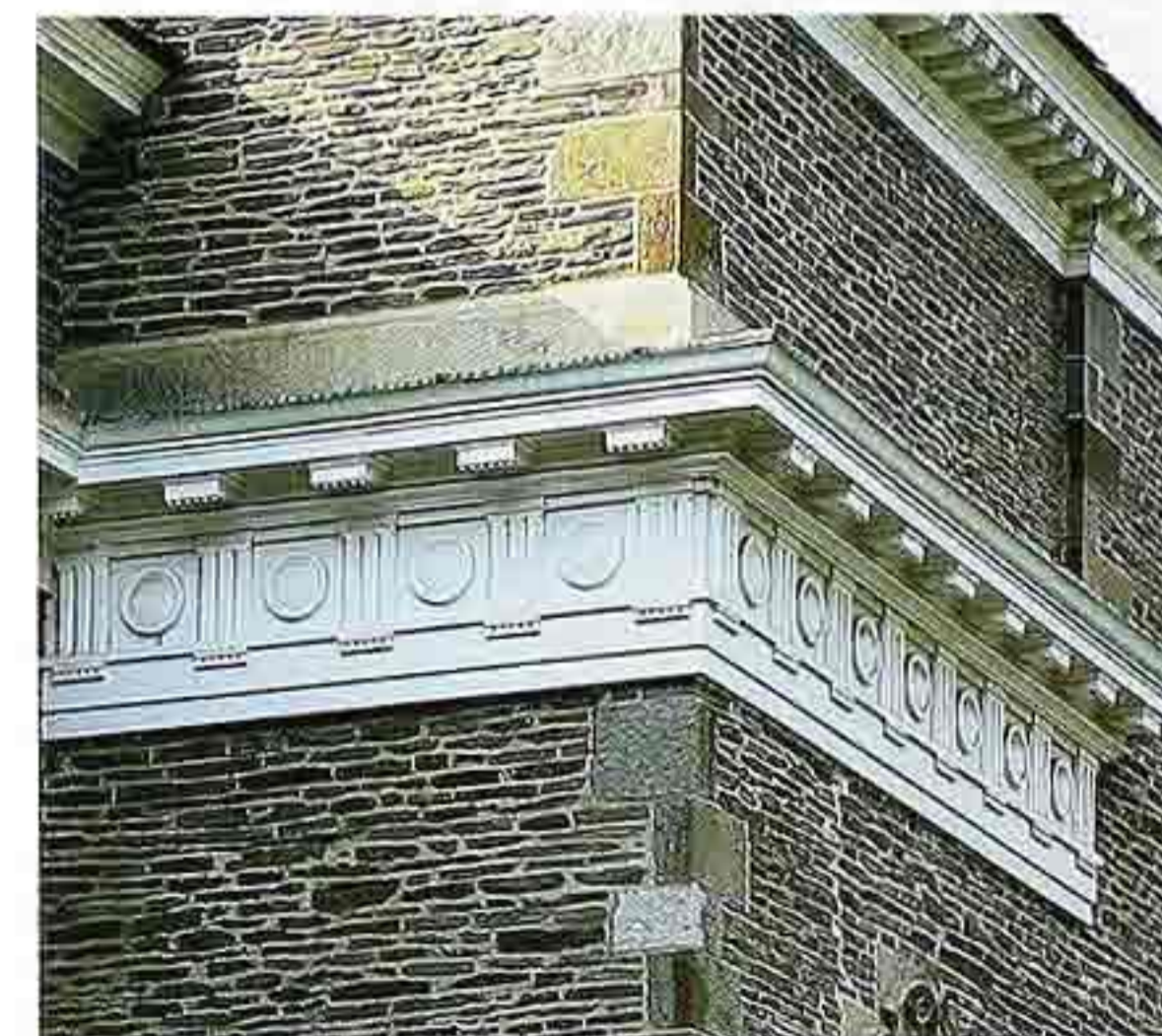
OM-84 Doric entablature with block modillion band and frieze with discs in metopes alternating with triglyphs
