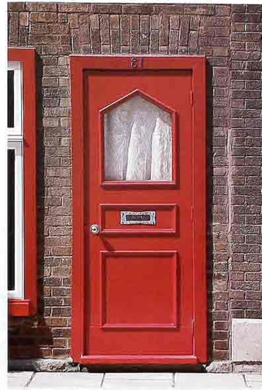
DW-41 Painted paneled door with pentagonal light in top panel, brass letter slot, in brick entry with jack arch
