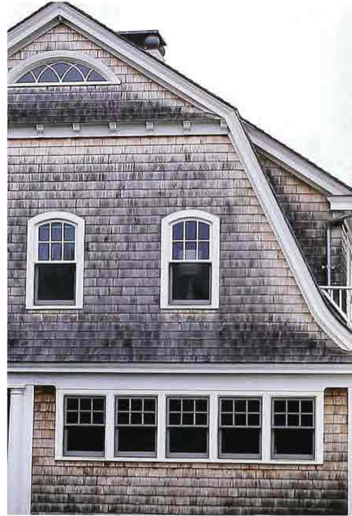
WI-49 Top to bottom: arched gable window; arched six-over-one double-hung windows; six-over-one double-hung windows, traditional shingle house
