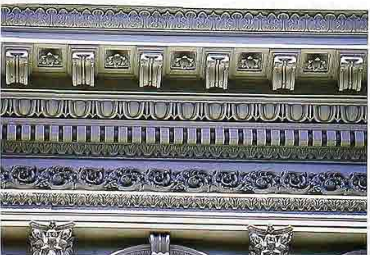
OM-71 Corinthian entablature. Top to bottom: cyma recta with anthemion, rosette-and-modillion cornice, egg-and-dart ovolo molding, dentil band, foliated frieze, tongue-and-dart cyma reversa
