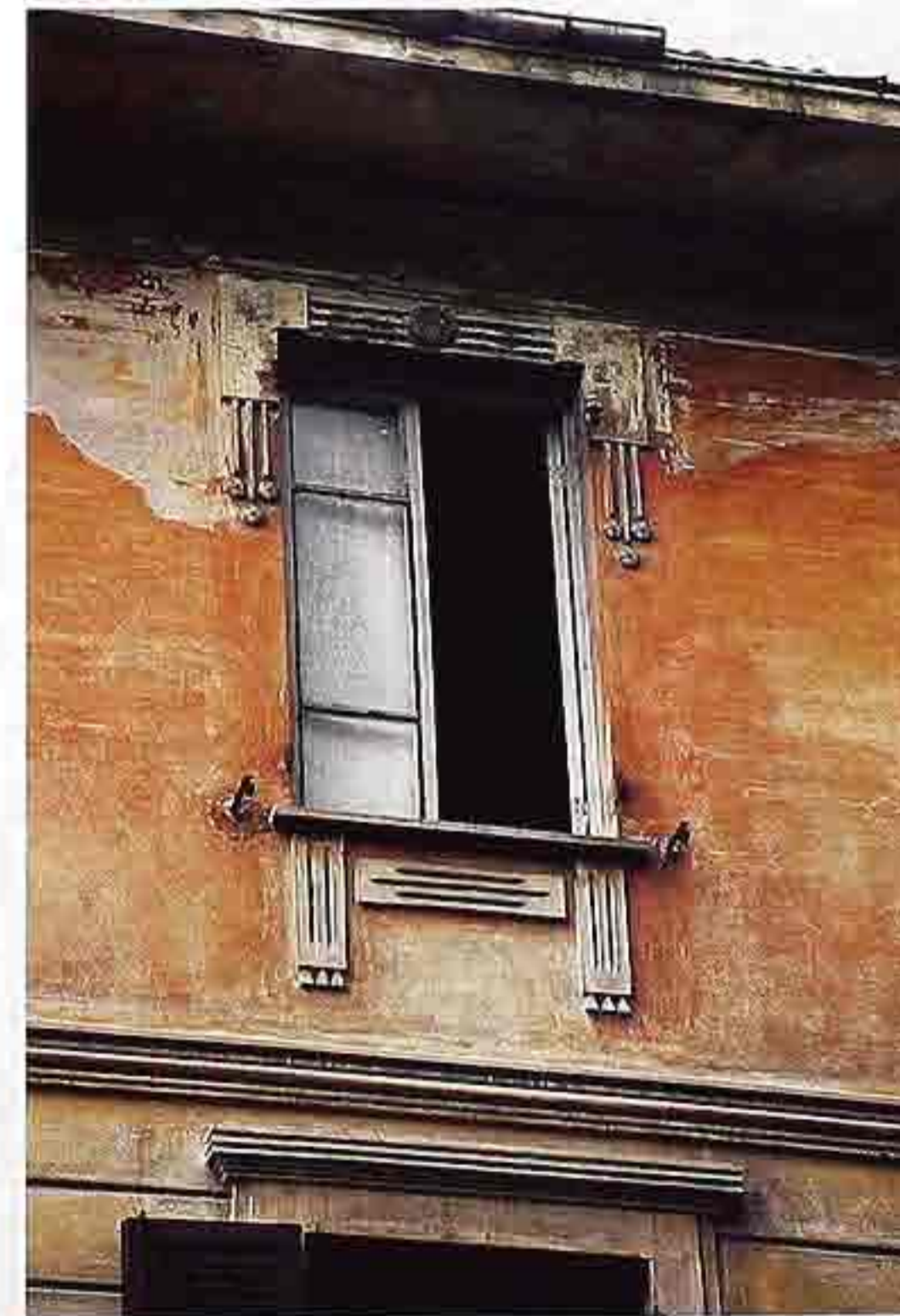
WI-36 Double-casement window in stucco wall
