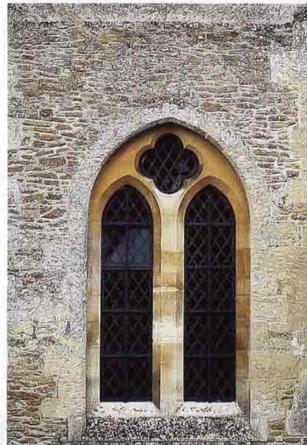
WI-135 Stone pointed segmental arch framing pair of leaded lancet windows with stone casings and leaded quatrefoil, 15th-c. English abbey
