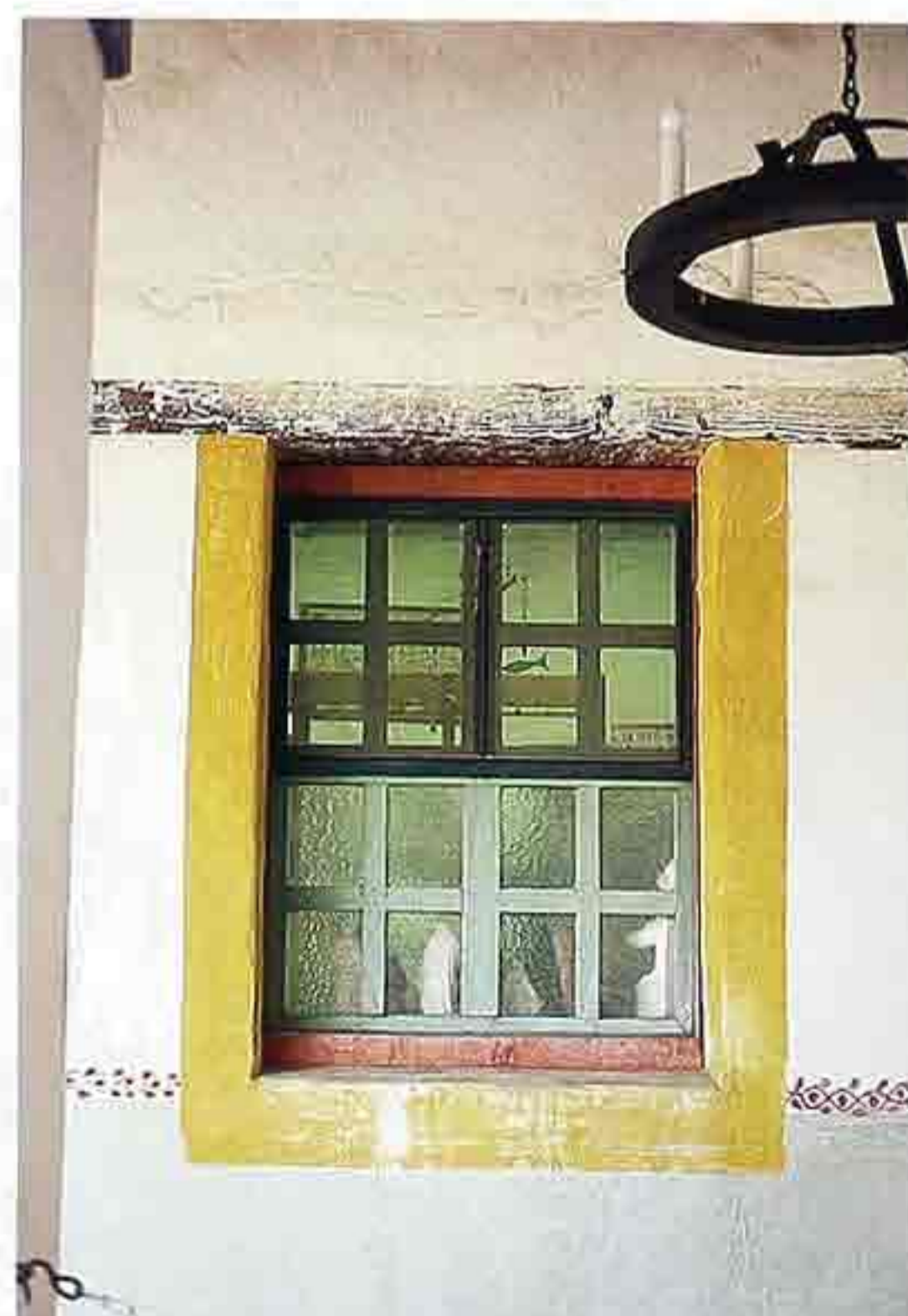
FA-78 Stucco-covered adobe painted with floral and ornamental bands on facade with window and exposed lintel, 18th-c. American Southwestern mission
