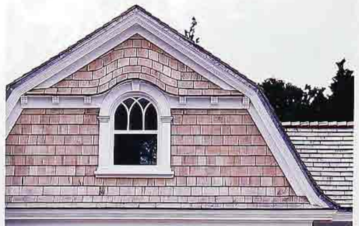
FA-52 New Alaskan yellow cedar shakes in common coursing, eyebrow window; gambrel roof
