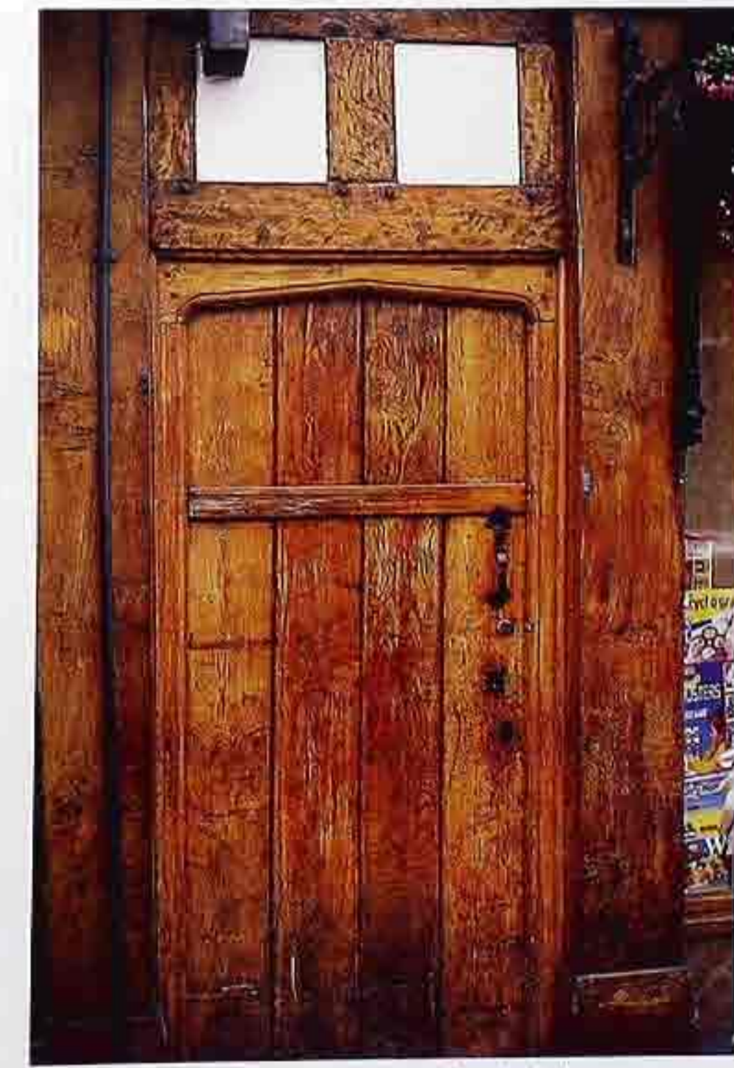
DW-36 Rustic wood-plank door with single brace, wrought-iron hardware, and two-paneled transom window; cambered arch; 16th- or 17th-c. England
