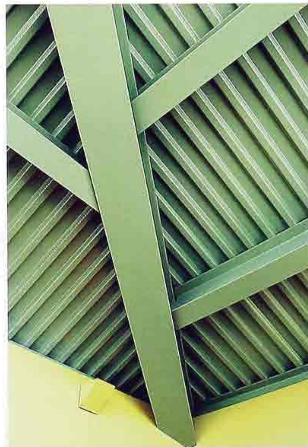
CR-4 Exposed ceiling beams: painted steel frame and corrugated steel decking, modern house
