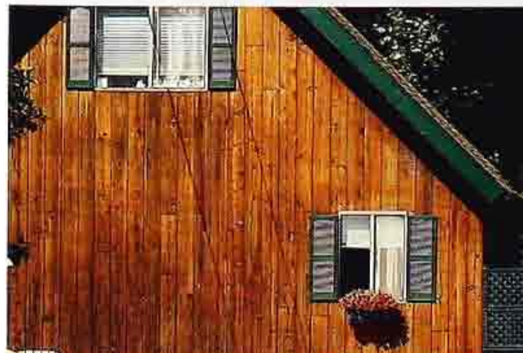
WA-26 Stained and sealed flush vertical board siding on traditional house
