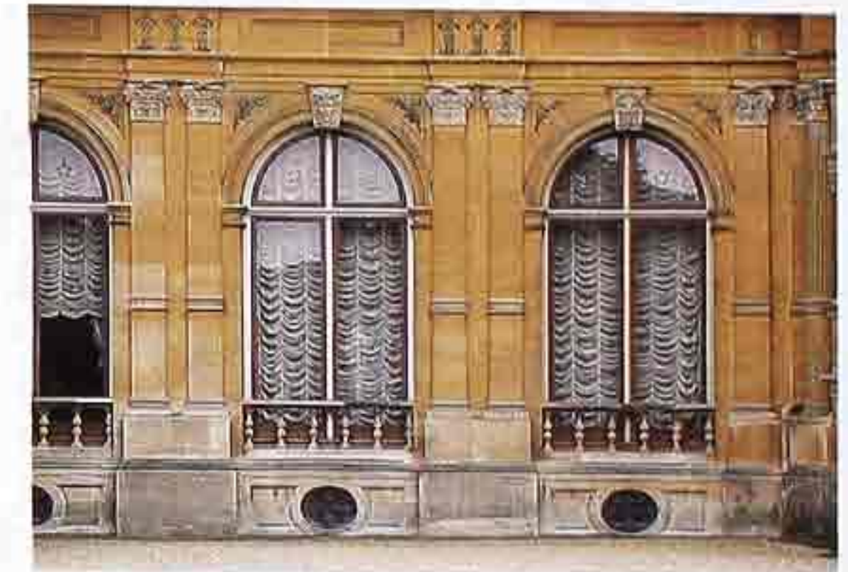
WI-99 Semicircular-arch transom lights over French doors in stone surround with keystones and pilasters, English house
