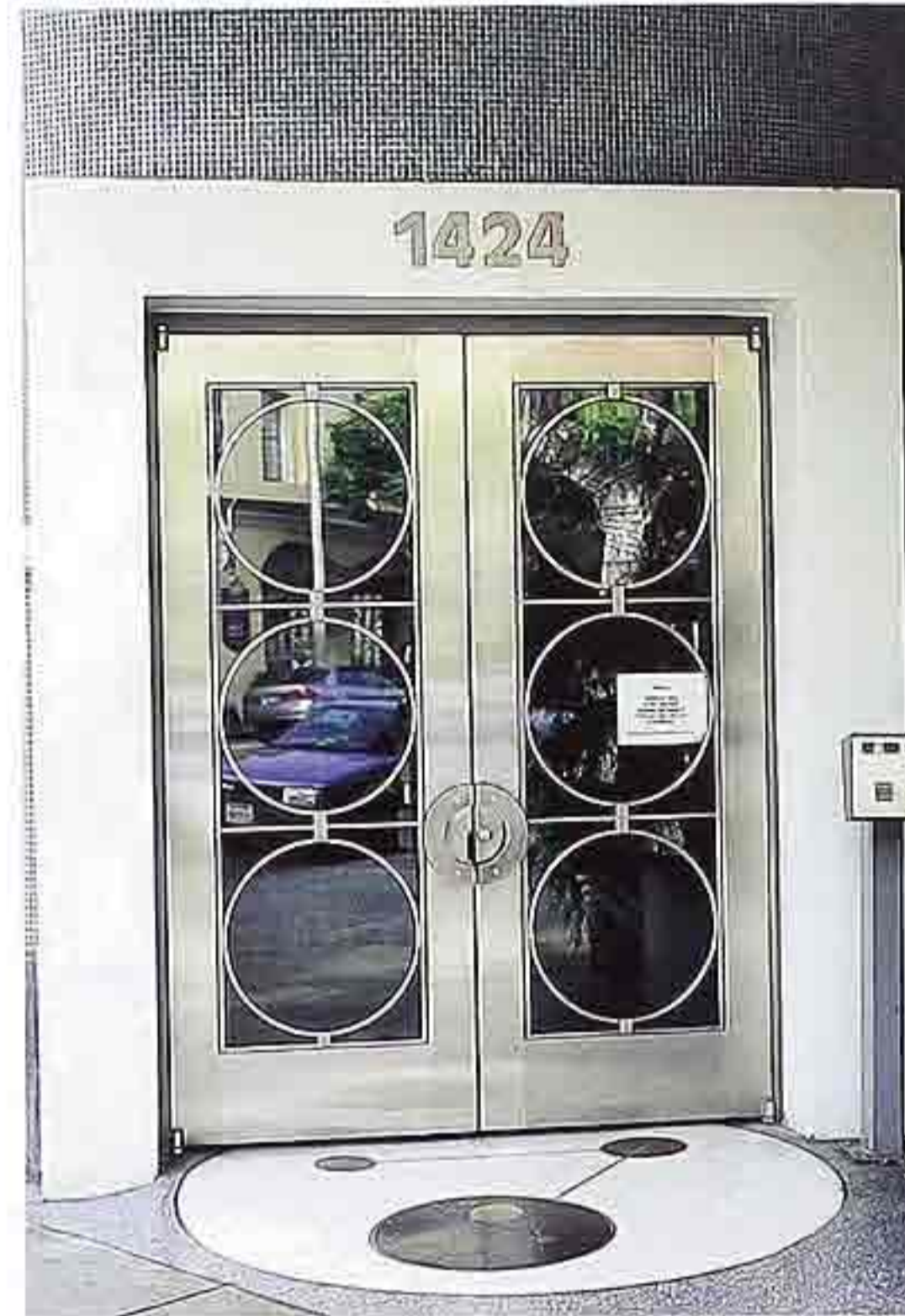
DW-46 Stainless steel double doors with full glass in circular muntins or grille
