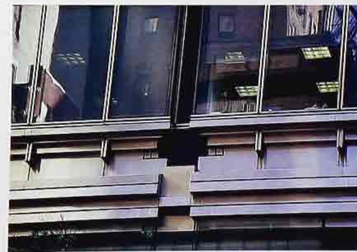
OM-78 Metal fascia bands suggesting a classical entablature, broken at the division between bays (detail of OM-75)
