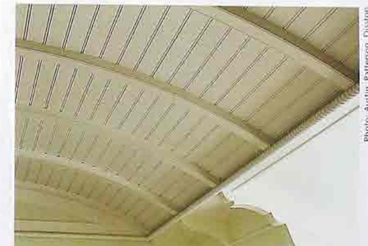
CR-8 Painted barrel ceiling with tongue-and-groove between exposed ribs, modern house
