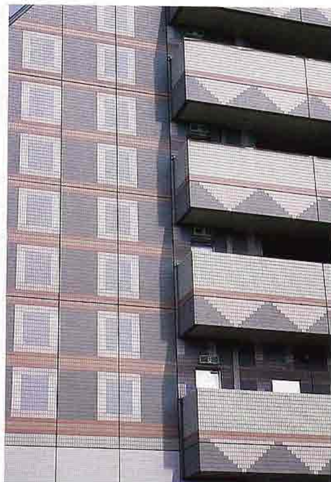
FA-71 Polychrome tiles in geometric patterns on walls and balconies of modern apartment house
