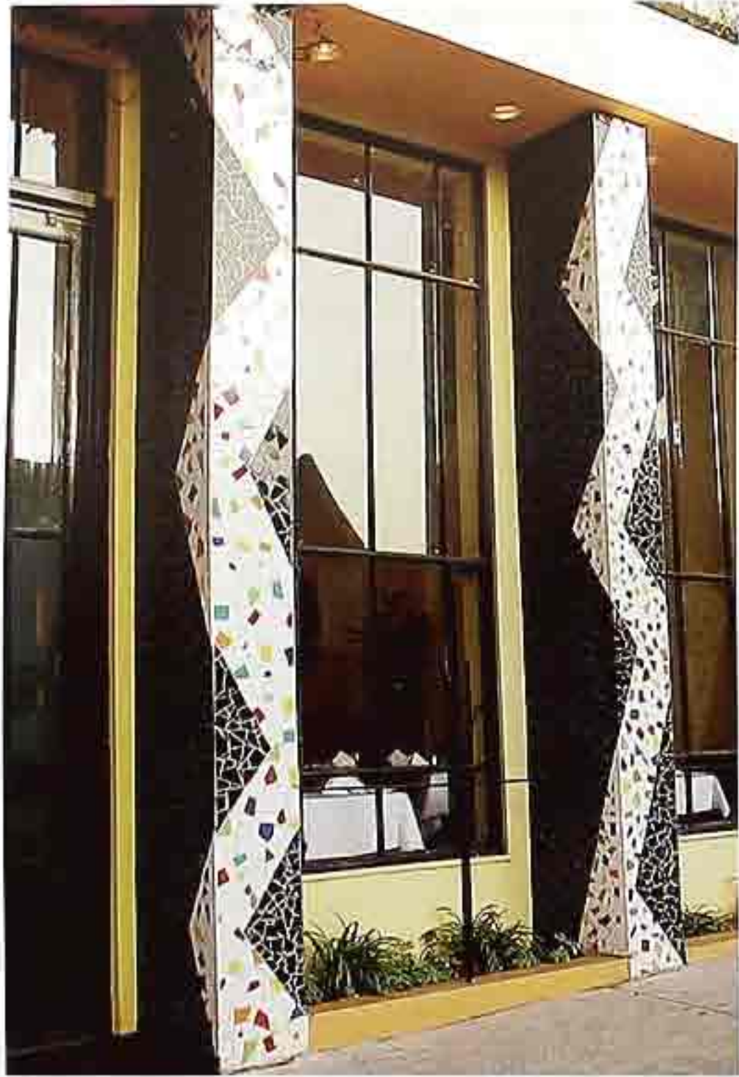
CP-80 Pilasters with a mosaic zigzag pattern, restaurant facade.
