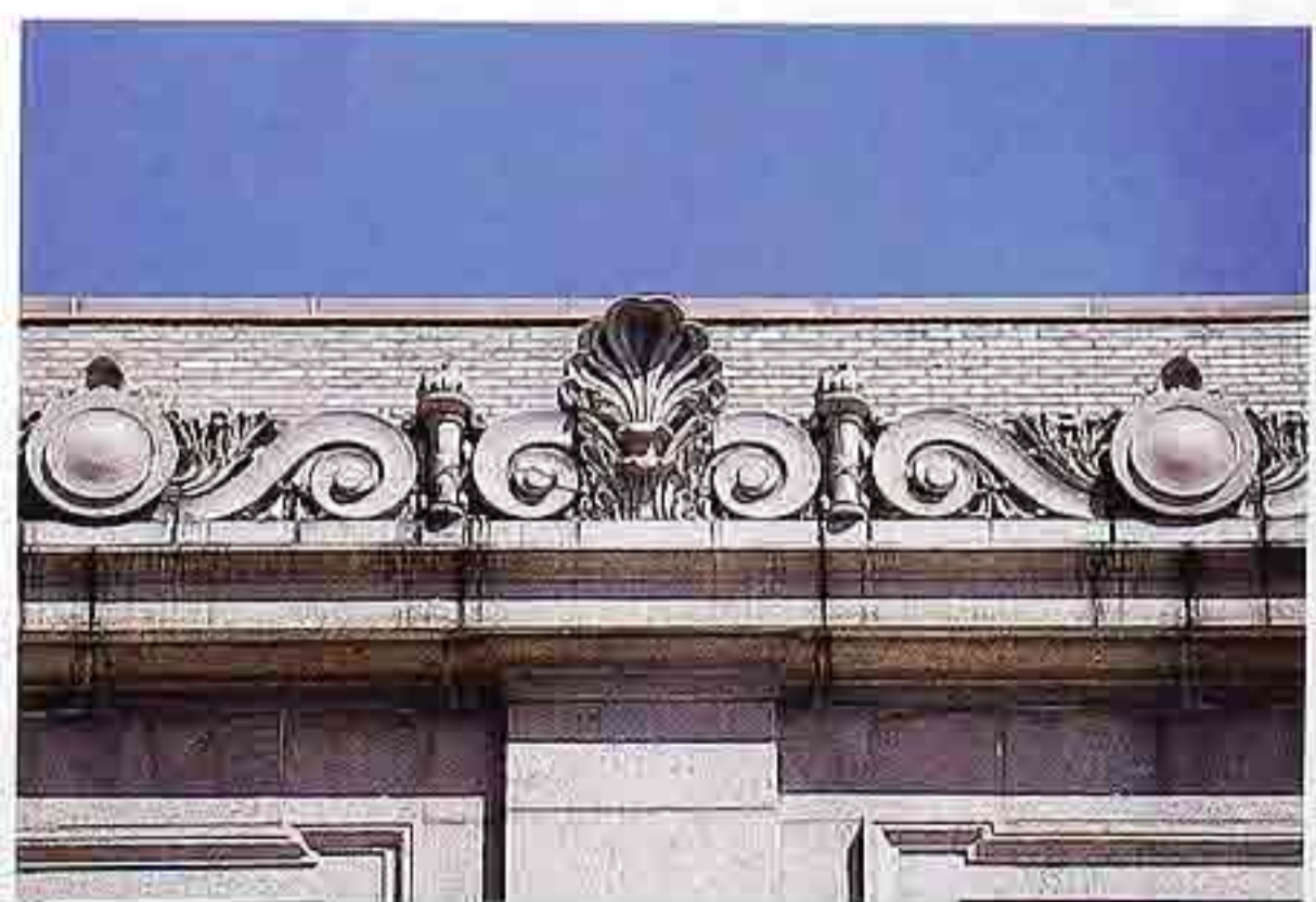
OM-62 Reverse and repeat running ornament above a cornice: from center out: anthemion, volute, torche, volute, foliated ornament, plain patera
