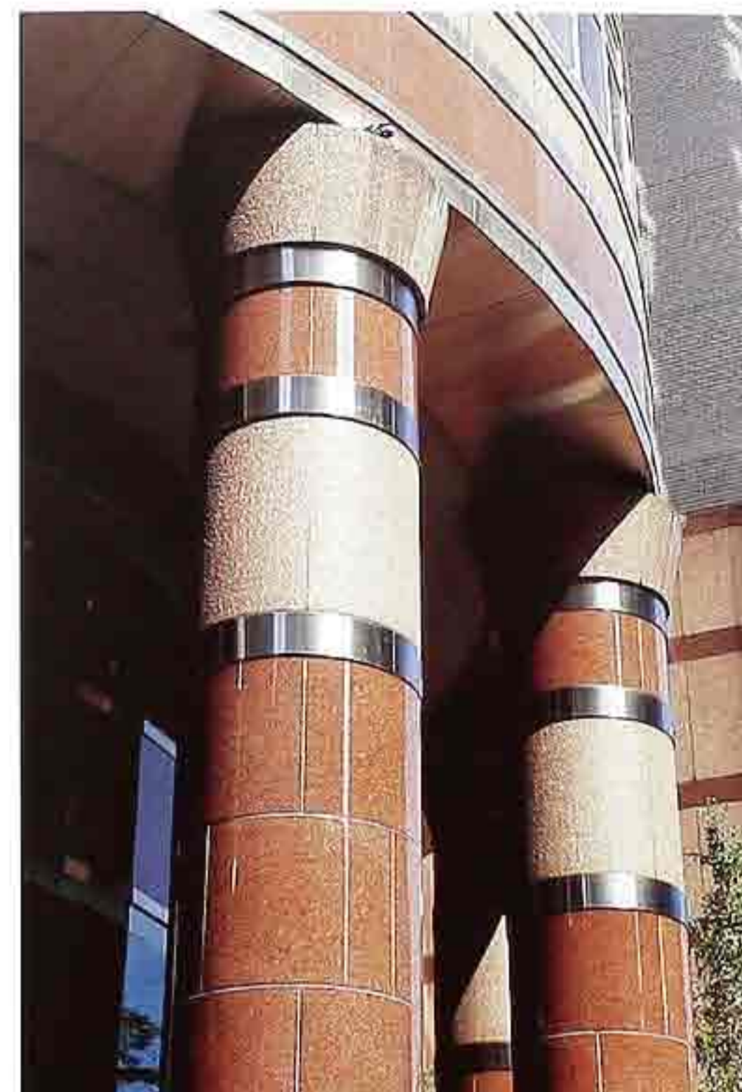
CP-126 Steel or concrete piers with polished stone and metal cladding, modern commercial building
