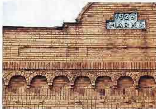
WA-161 Parapet wall in running bond with blind semi-circular arches and corbels below soldier course
