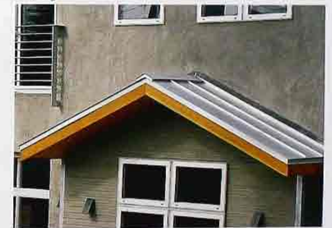
CR-112 Metal and wood gable with eave acting as door hood, modern beach house
