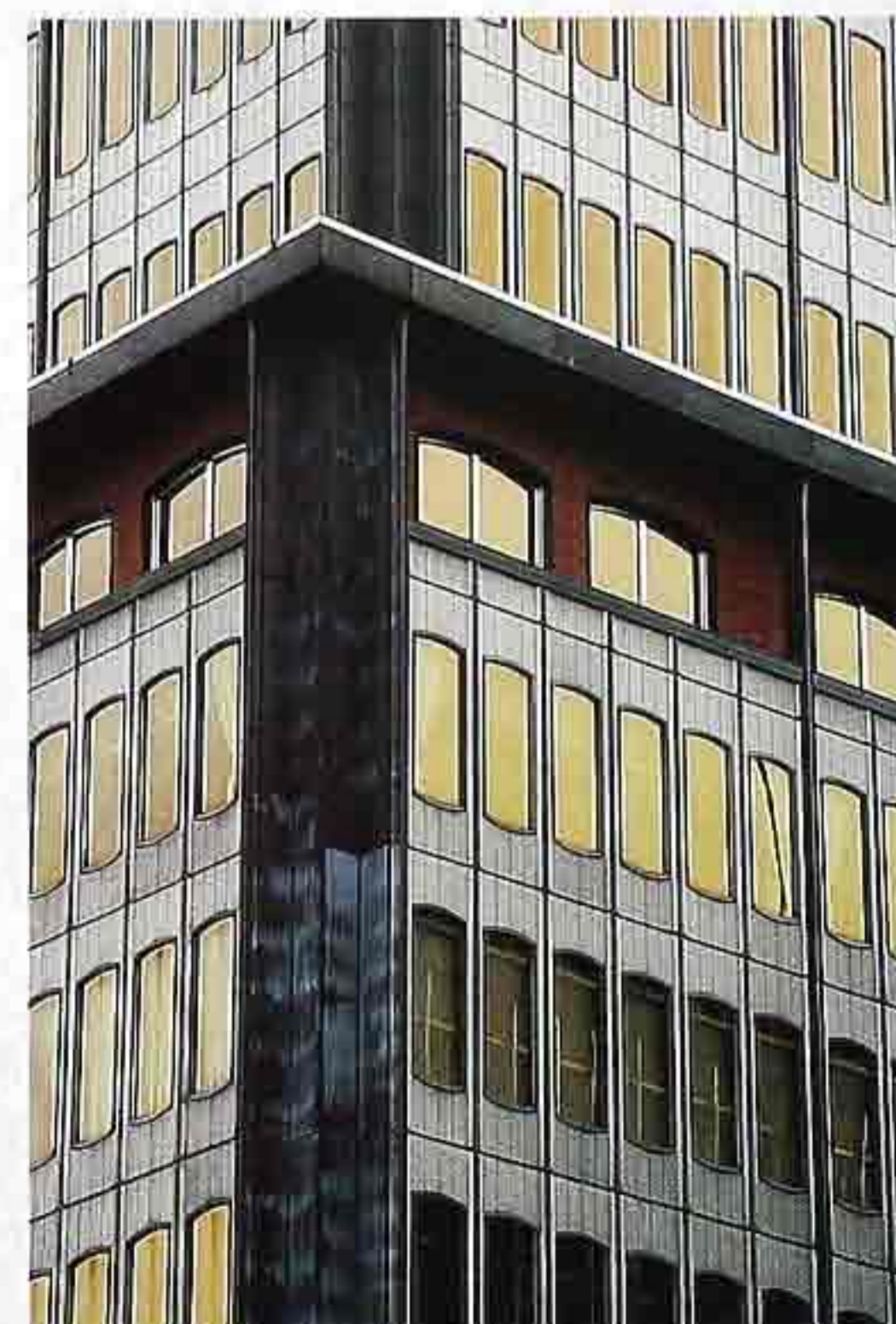
WI-17 Bronze mirror-glass windows in curtain wall, modern commercial building
