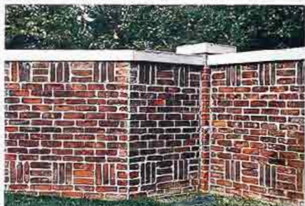
WA-156 Basket-weave borders around running-bond; concrete capstone, garden wall
