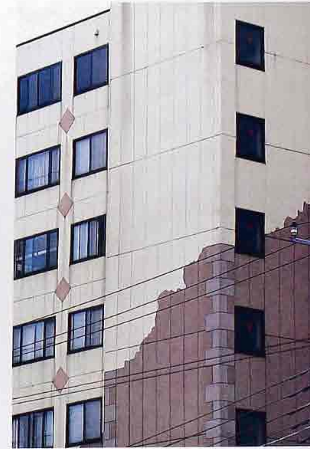
WA-247 Colored smooth stucco supergraphic with stucco quoins in lower section, modern apartment house
