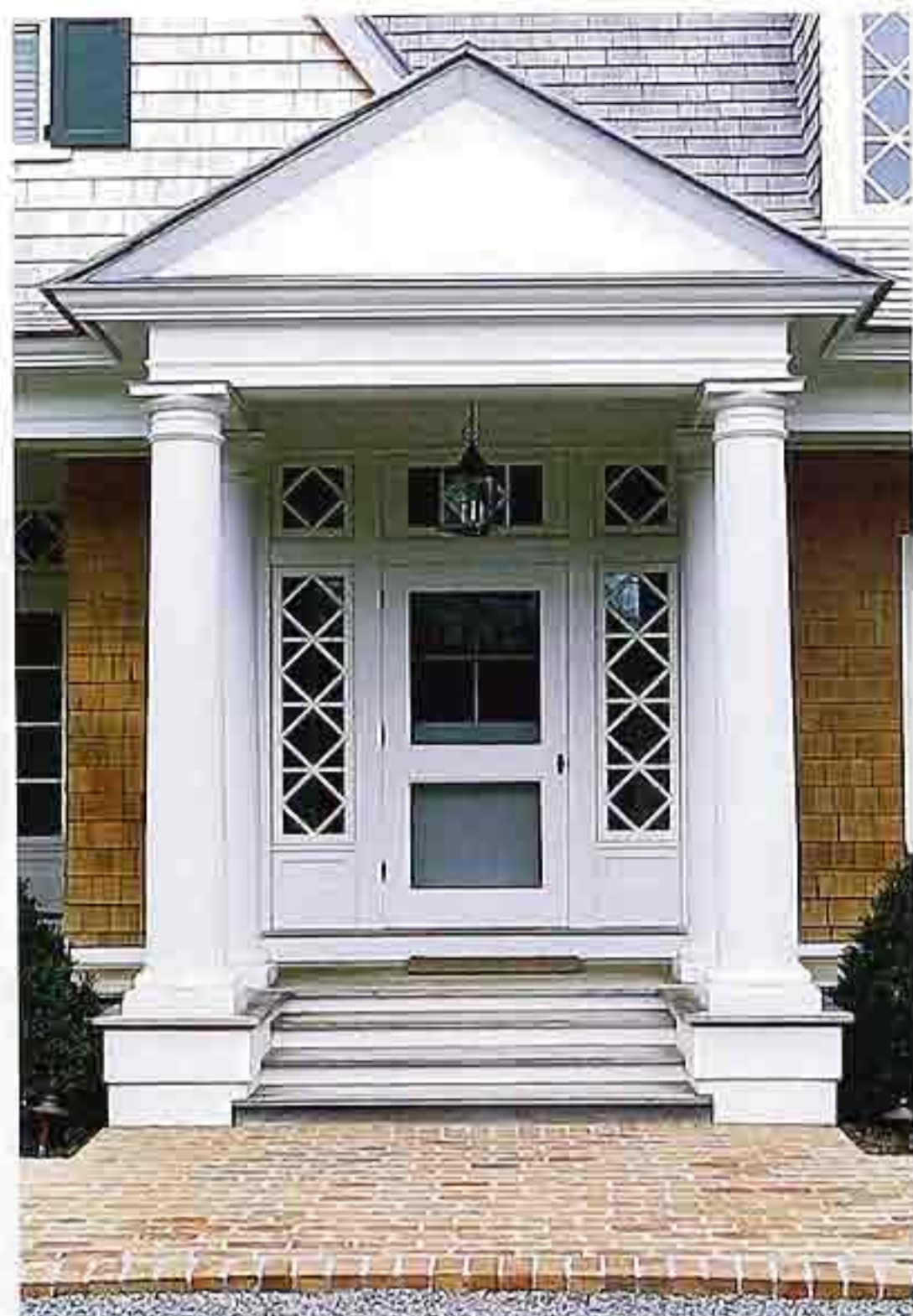
DW-81 Tuscan-style painted wood columns and entablature with pediment porch, paneled door, diamond side lights, traditional house
