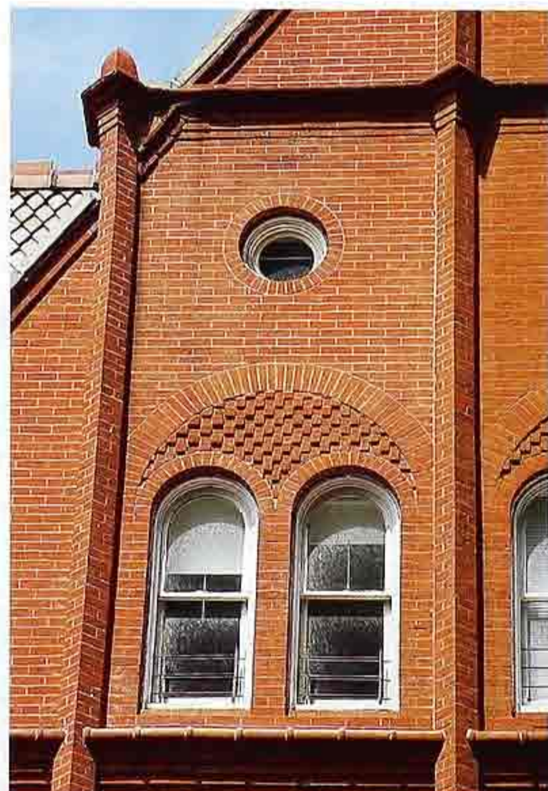
WI-58 One-over-one double-hung, arched top sashes with fixed lights; fixed bull's eye window above
