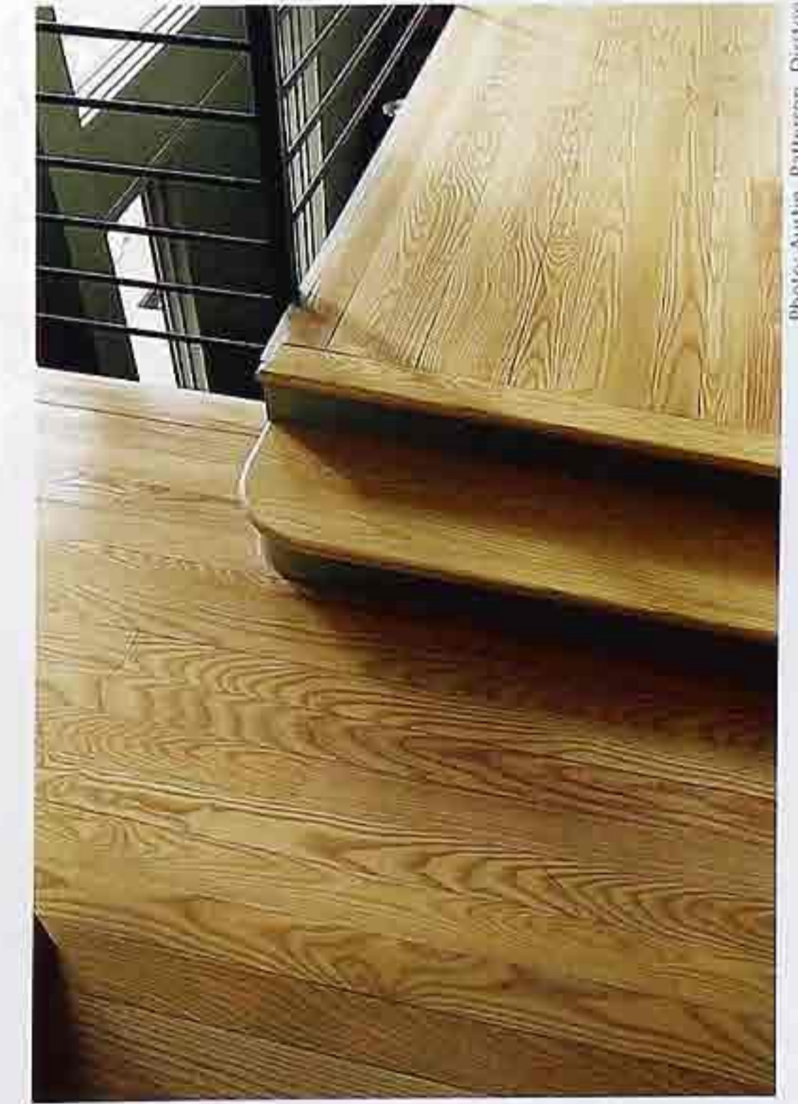
FP-7 Ash flooring and steps with rounded nosing in balcony hallway
