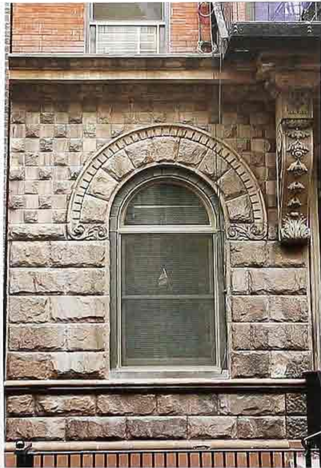
WI-140 Ornamented brownstone voussoirs around semi-circular-arch window
