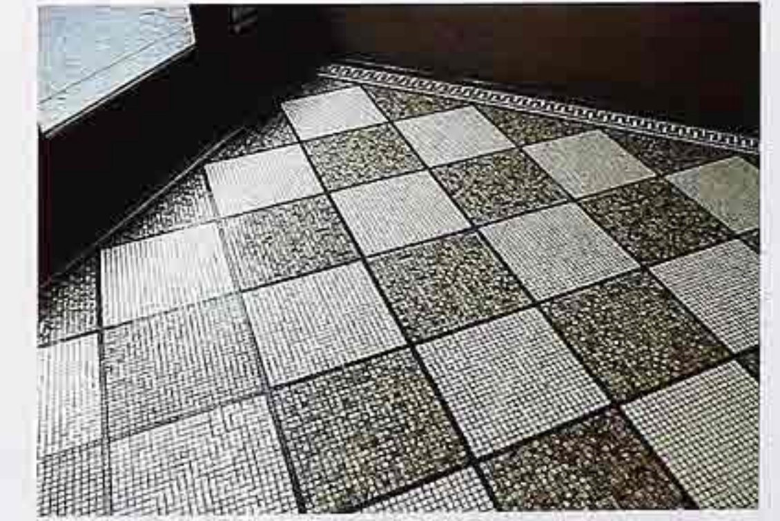
FP-100 Squares of pre-grouted stone mosaic tiles in checker design with dark mosaic grid outline squares, commercial entry
