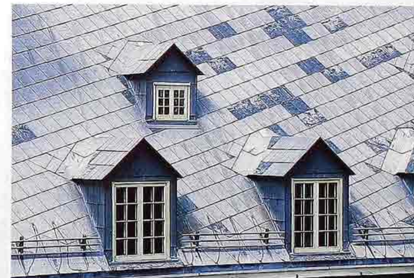
CR-28 Sheet-metal shingles with flat seams on roof and dormers; pipe-style snow guard on lower edge
