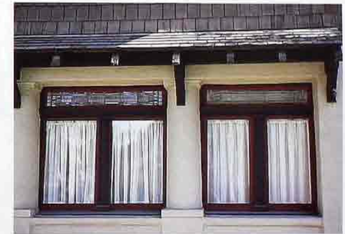
WI-101 Leaded rectangular transom lights over casement windows; hood supported by brackets, Arts and Crafts house
