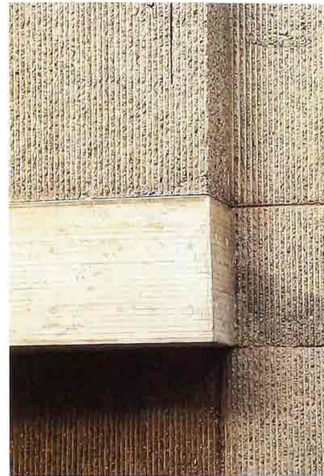
WA-217 Cast coarse-aggregate concrete, bush-hammered, with board-formed slab edge
