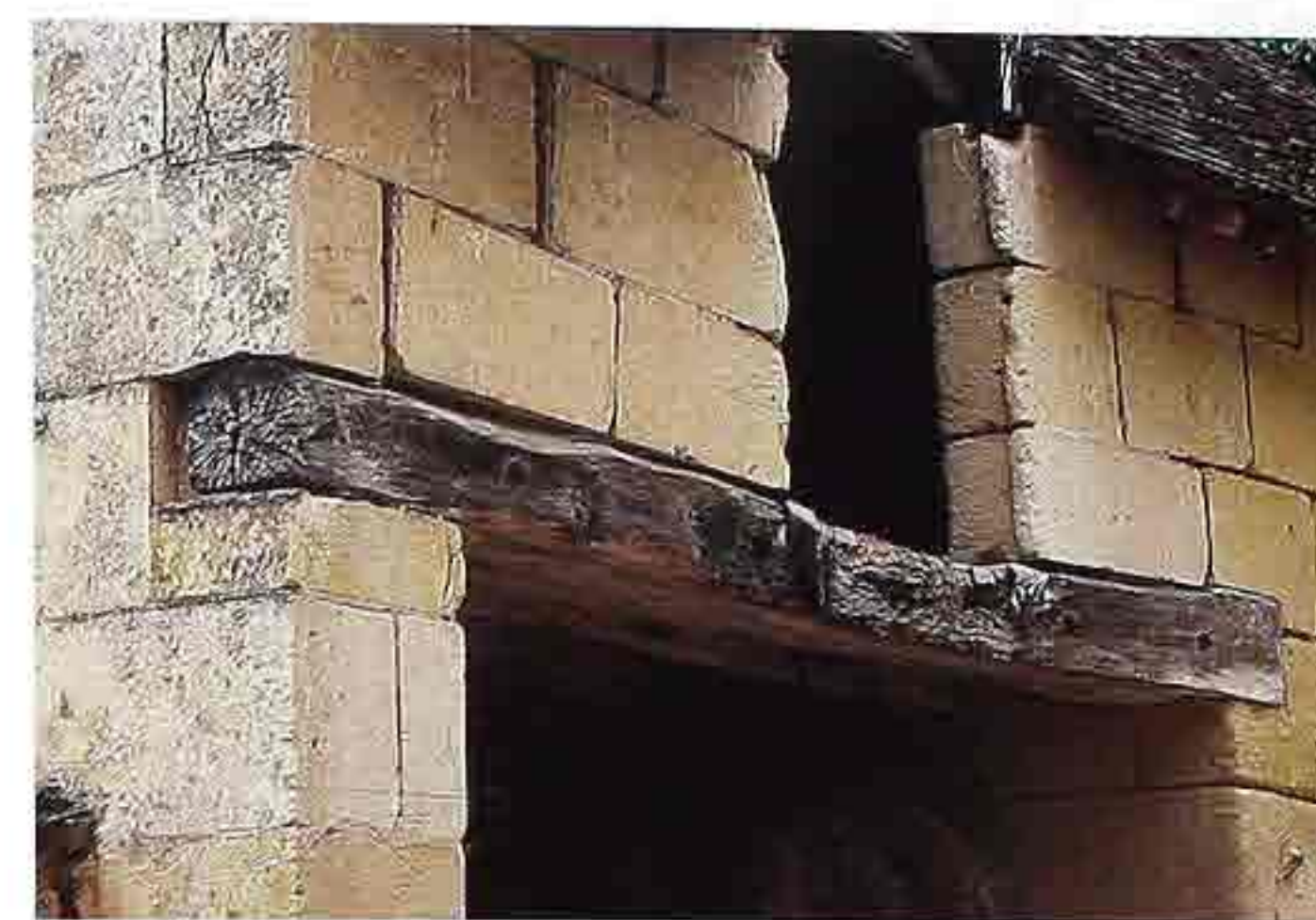
CP-109 Timber lintel in stone wall.
