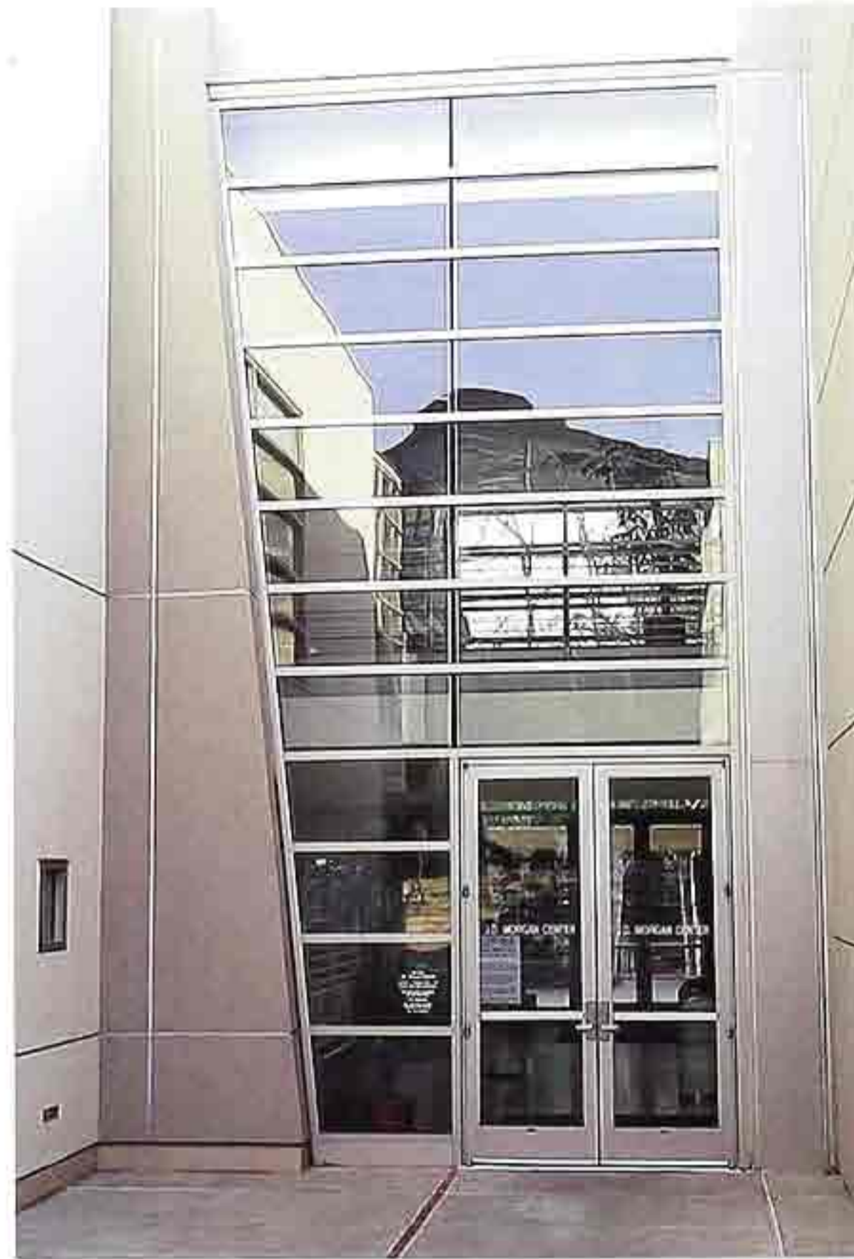
DW-102 Covered entryway: stainless steel double doors with full glass set in glass-paneled wall; masonry surround, modern commercial building
