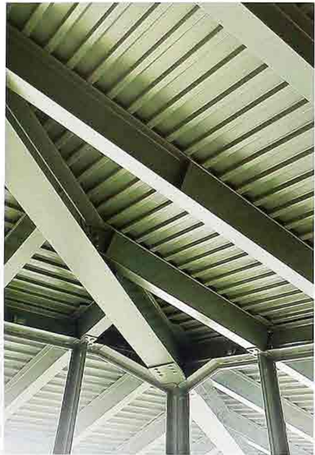
CP-122 Painted steel frame with wide-flange beams and riveted connections, supporting corrugated steel decking, ceiling of modern house
