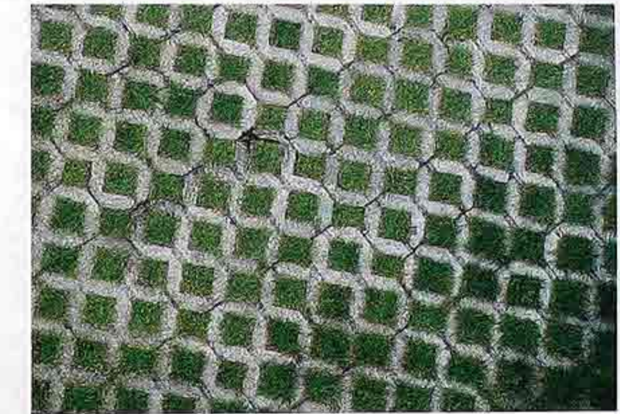
FP-88 Concrete screen-wall blocks set into the ground and planted with grass in patio
