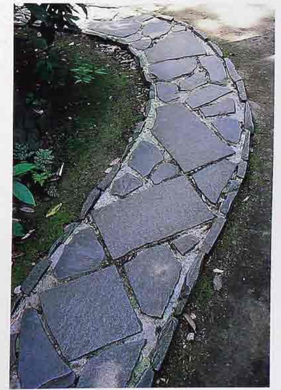
FP-50 Roughly squared paving stone in diamond pattern with border, garden path
