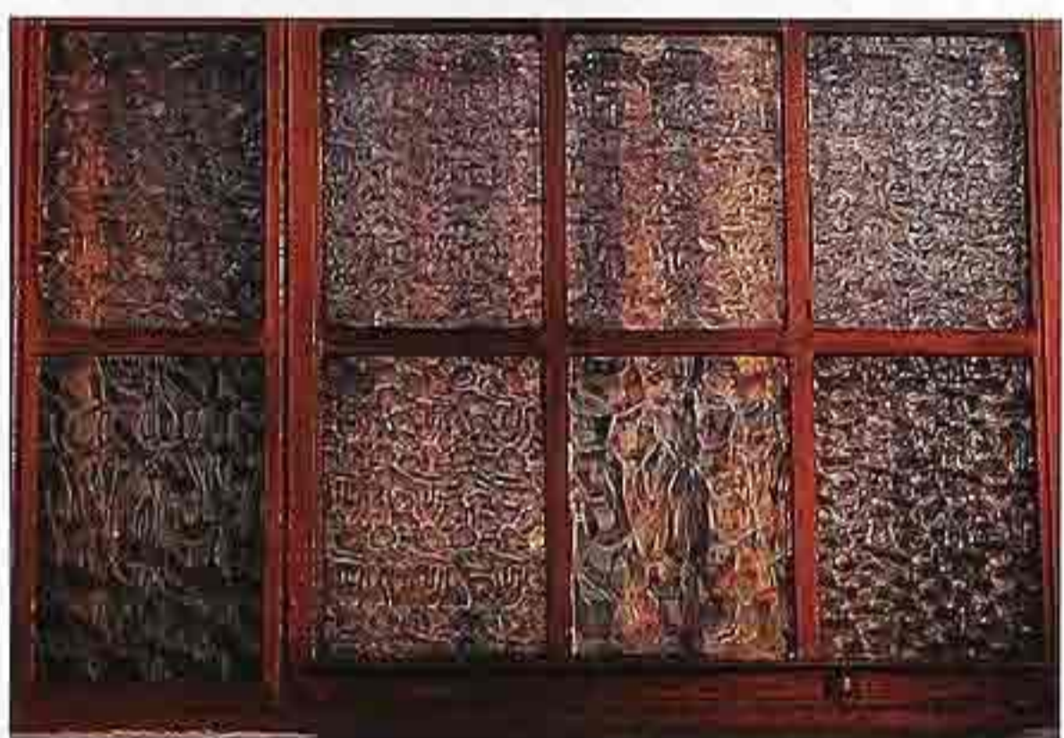
WI-11 Figured glass with flat metal muntins in a metal frame, industrial building
