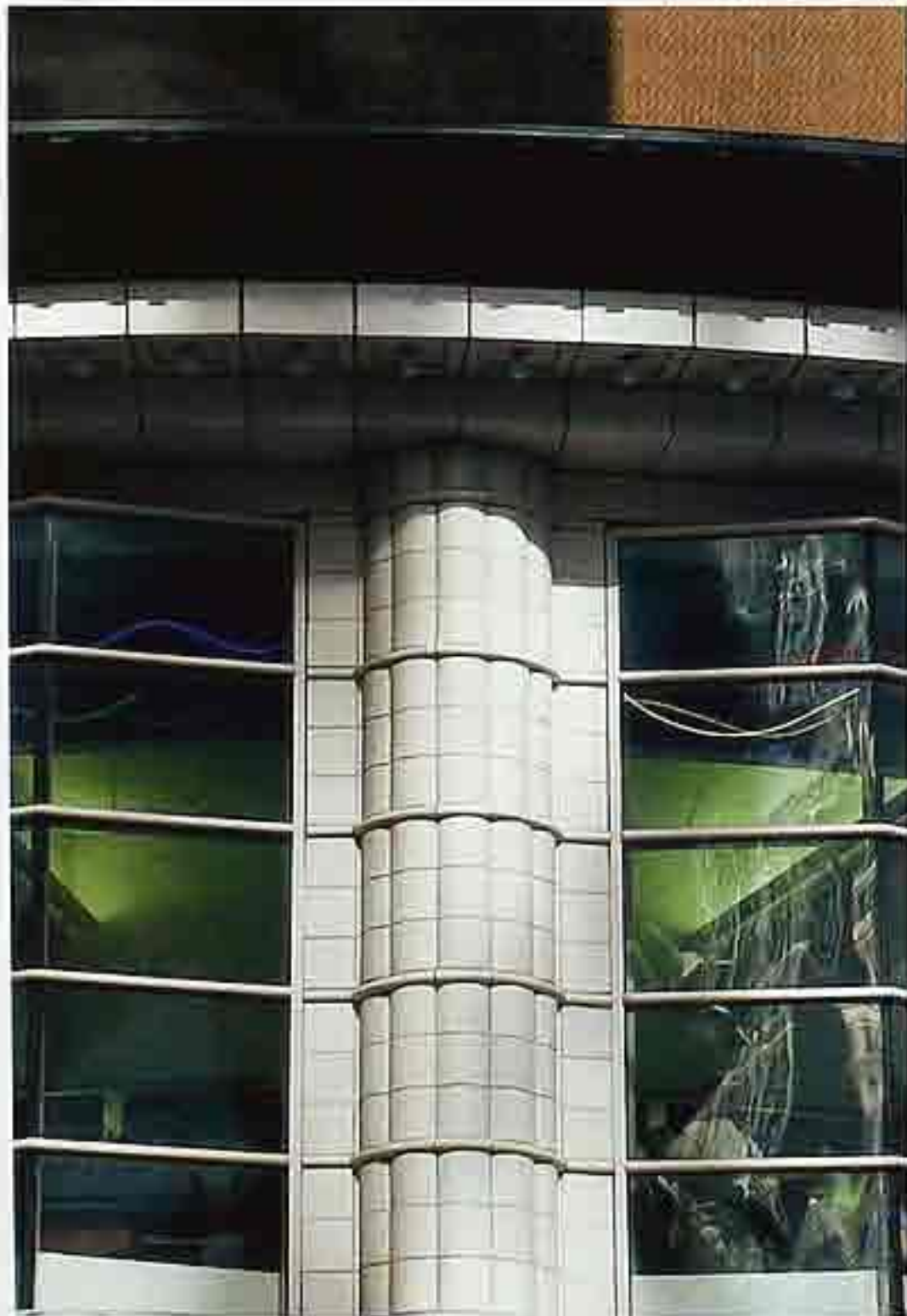
CP-98 Bundled pier on modern commercial building
