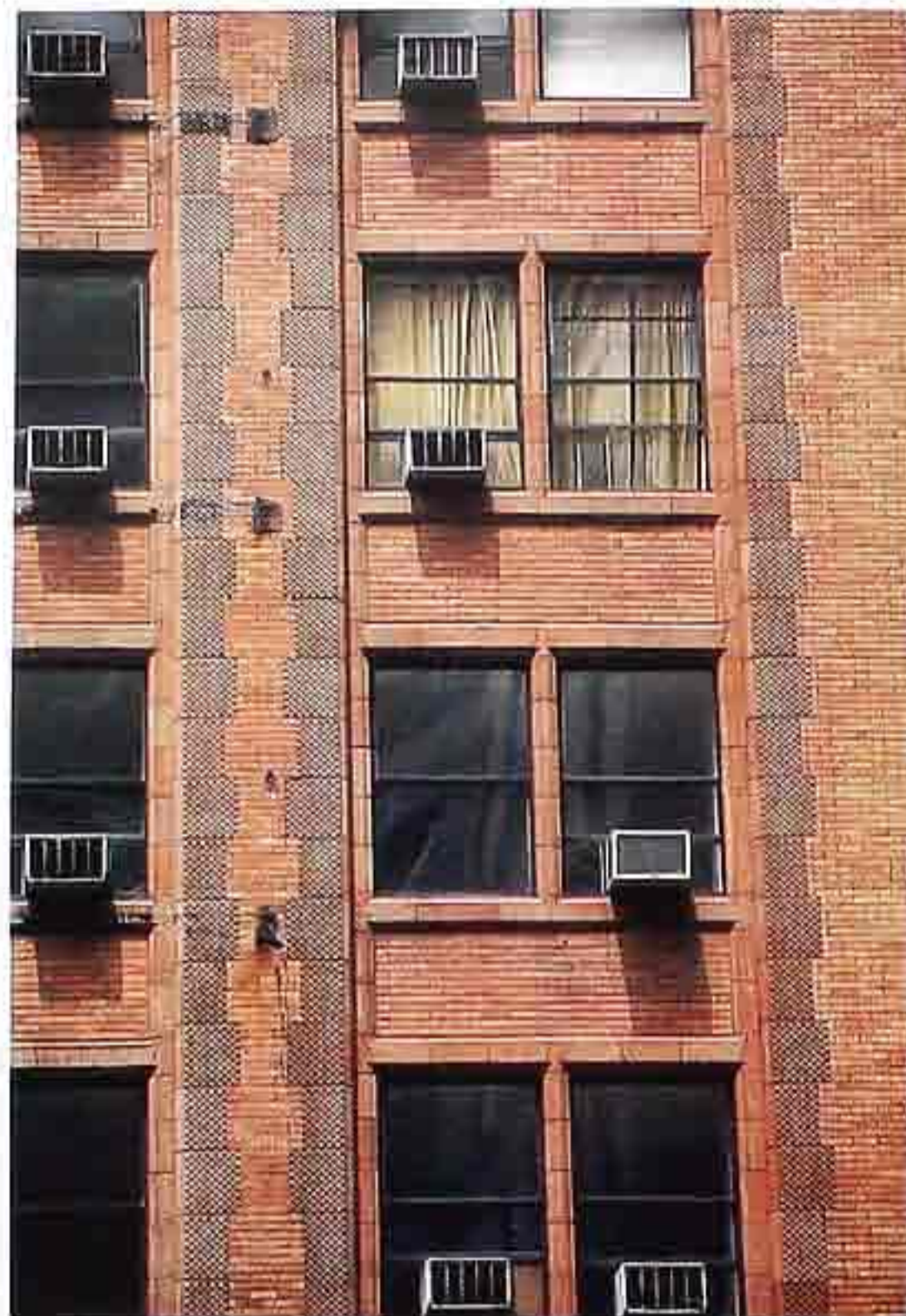
WA-197 Brick window-wall with recessed spandrels, brownstone window trim and quoins.
