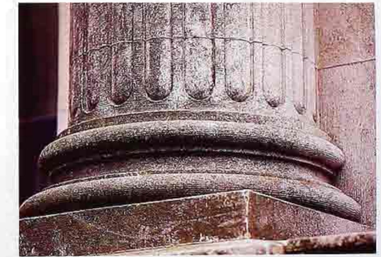
CP-38 Attic base on square plinth with detail of fluting
