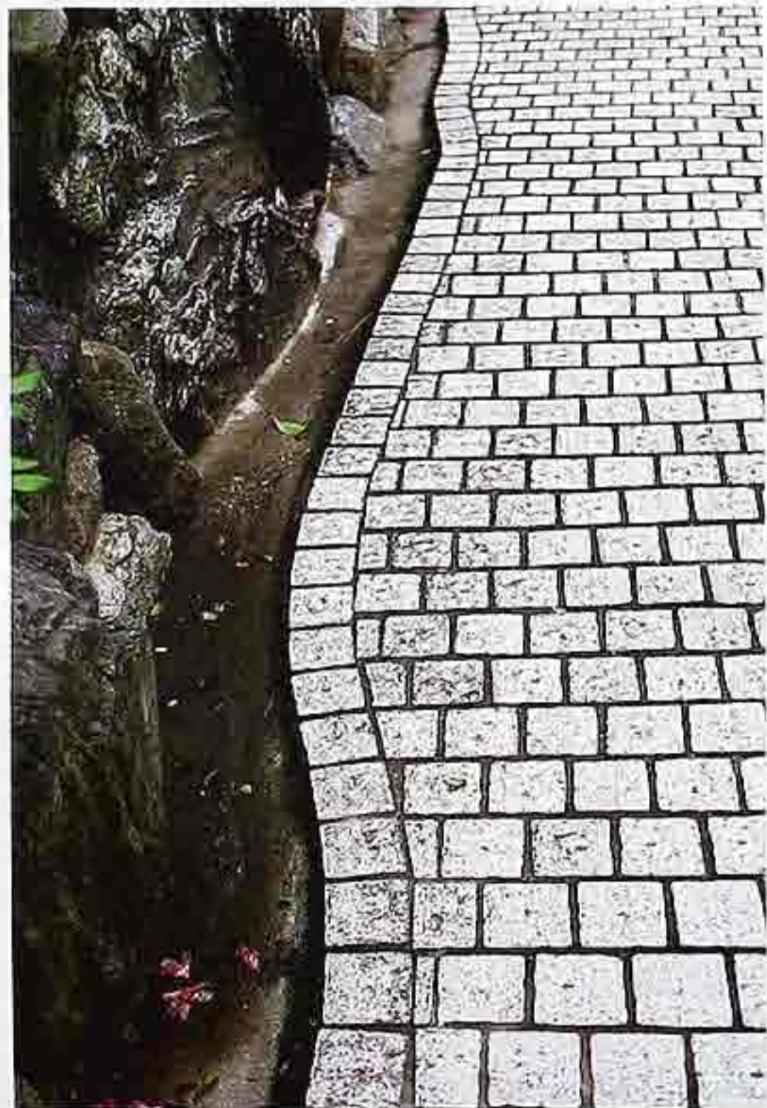
FP-21 Paving stones set in concrete in running bond with soldier-course border adjacent to natural rock wall, garden path
