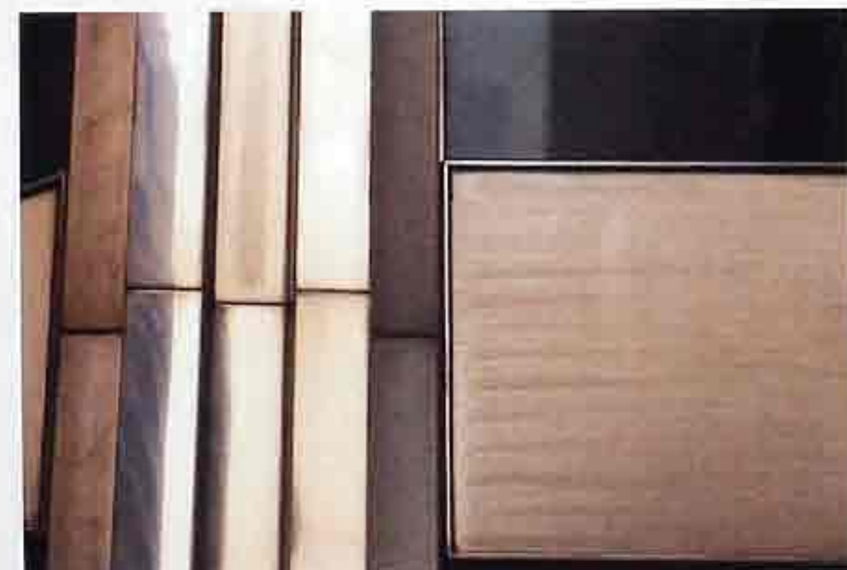
FA-5 Bronze over stainless steel spandrel panel with a raised edge and adjoining window (top right)
