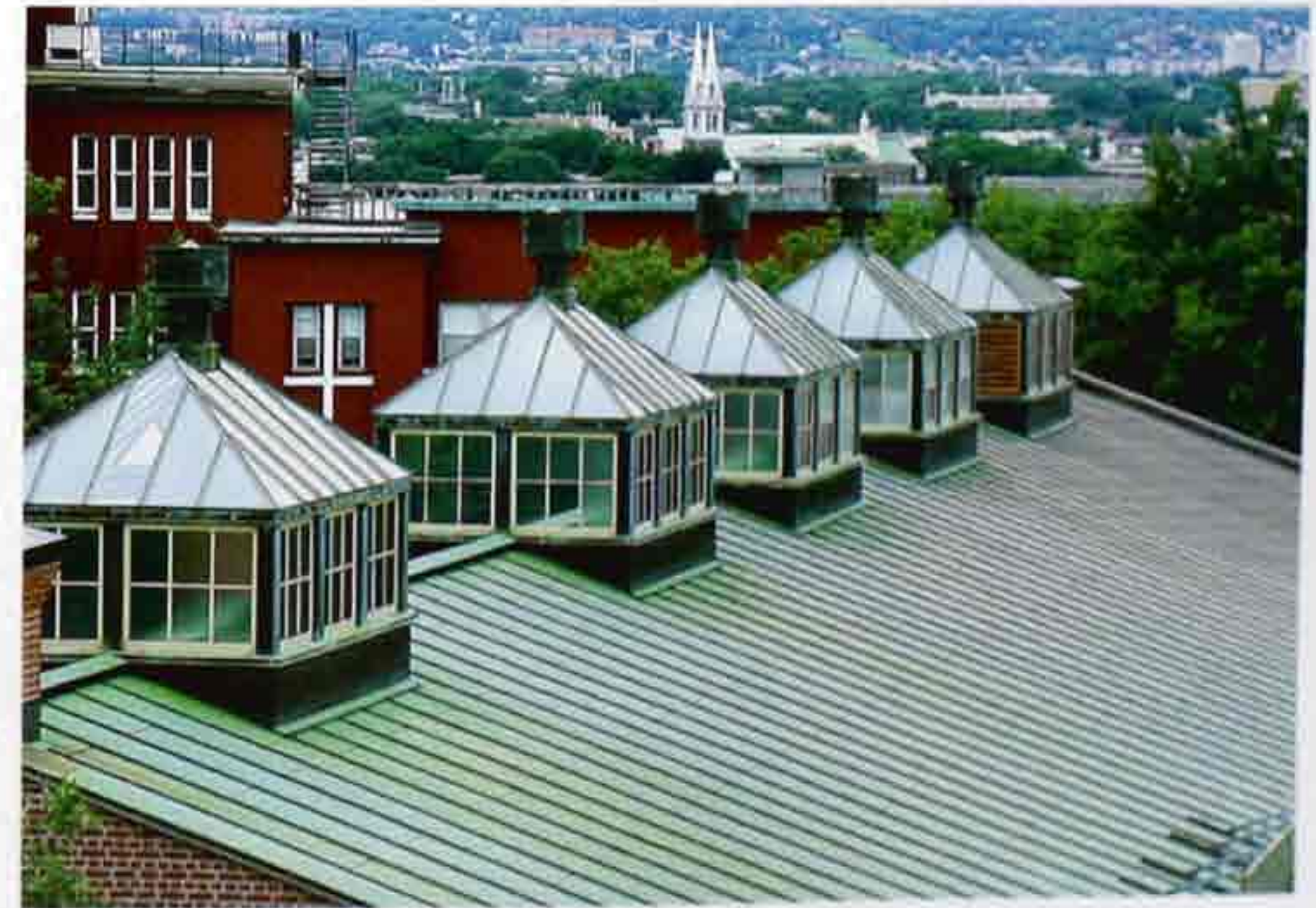
CR-36 Sheet metal with standing seams on gable roof and glassed monitors, modern commercial building
