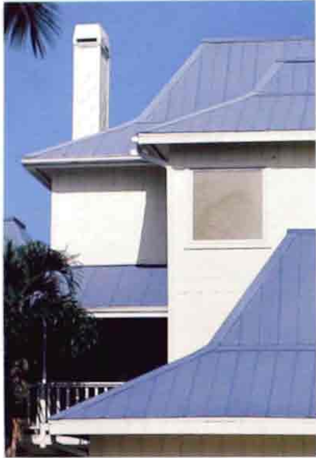
CR-30 Anodized aluminum or coated sheet steel with standing seams, variation of hipped roof, modern house
