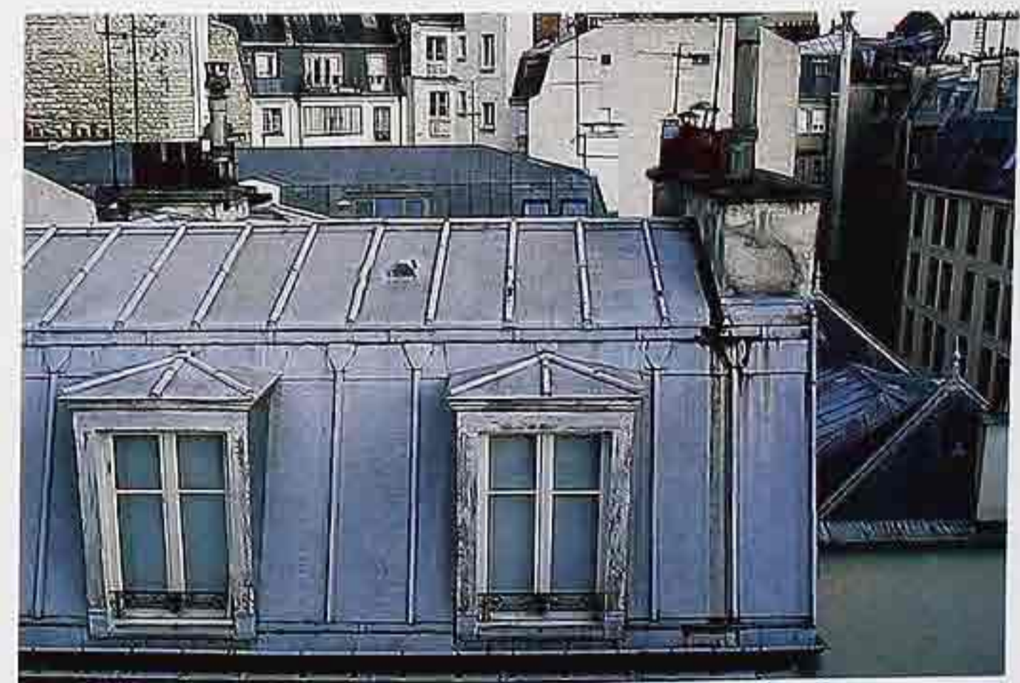
CR-29 Sheet metal with batten seams on gambrel roof and dormers, 19th-c. French apartment house
