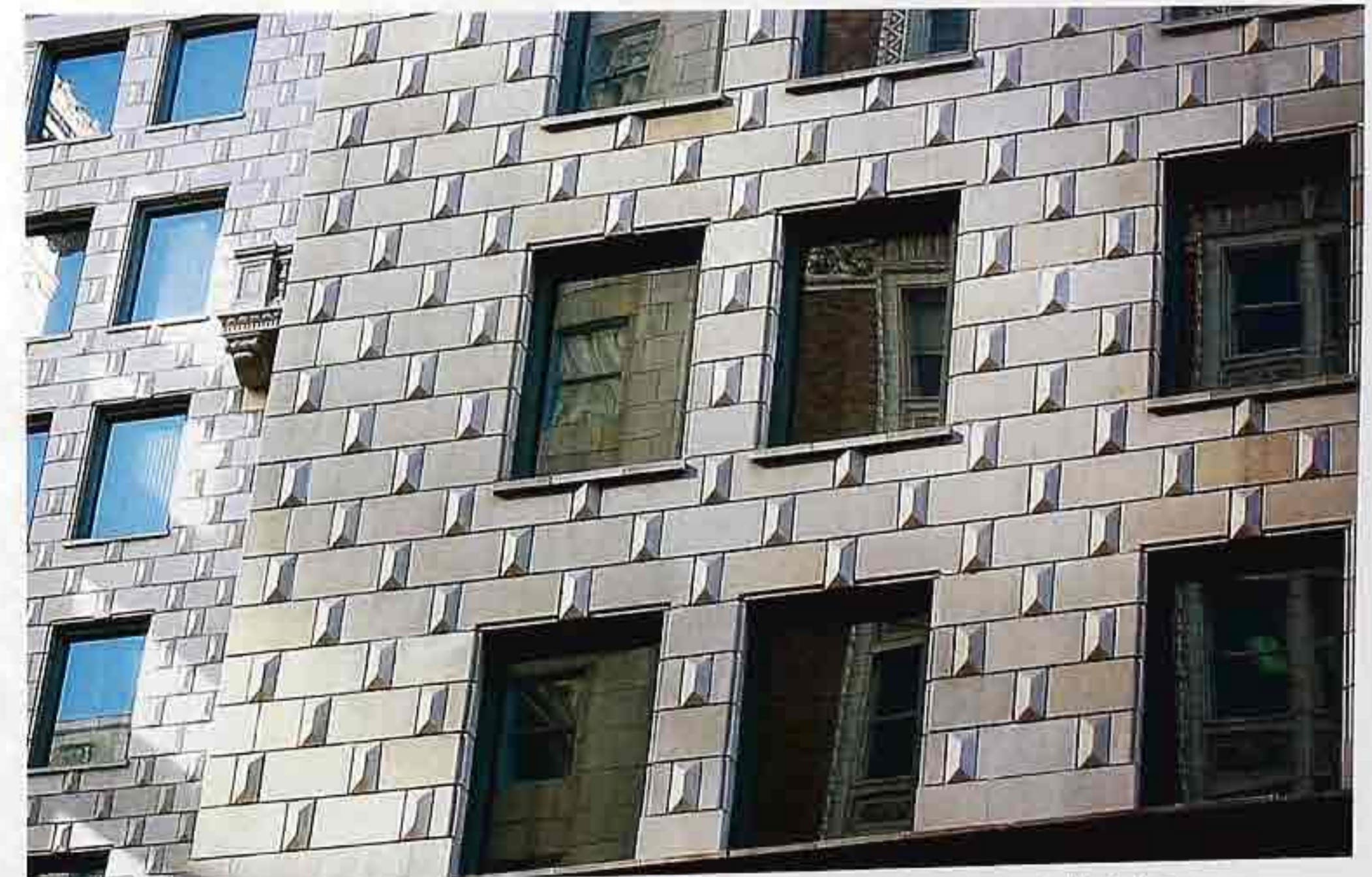
WA-144 Granite, with honed and gem-cut blocks in running bond, modern commercial building
