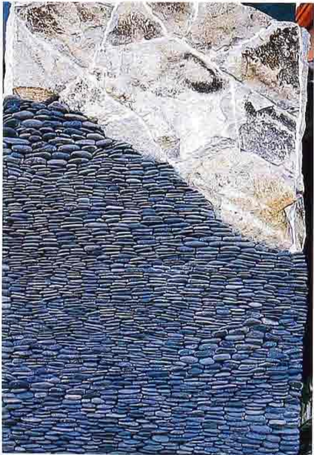
WA-74 Top: fieldstone rubble in mosaic bond; bottom: coursed rubble of beach pebbles
