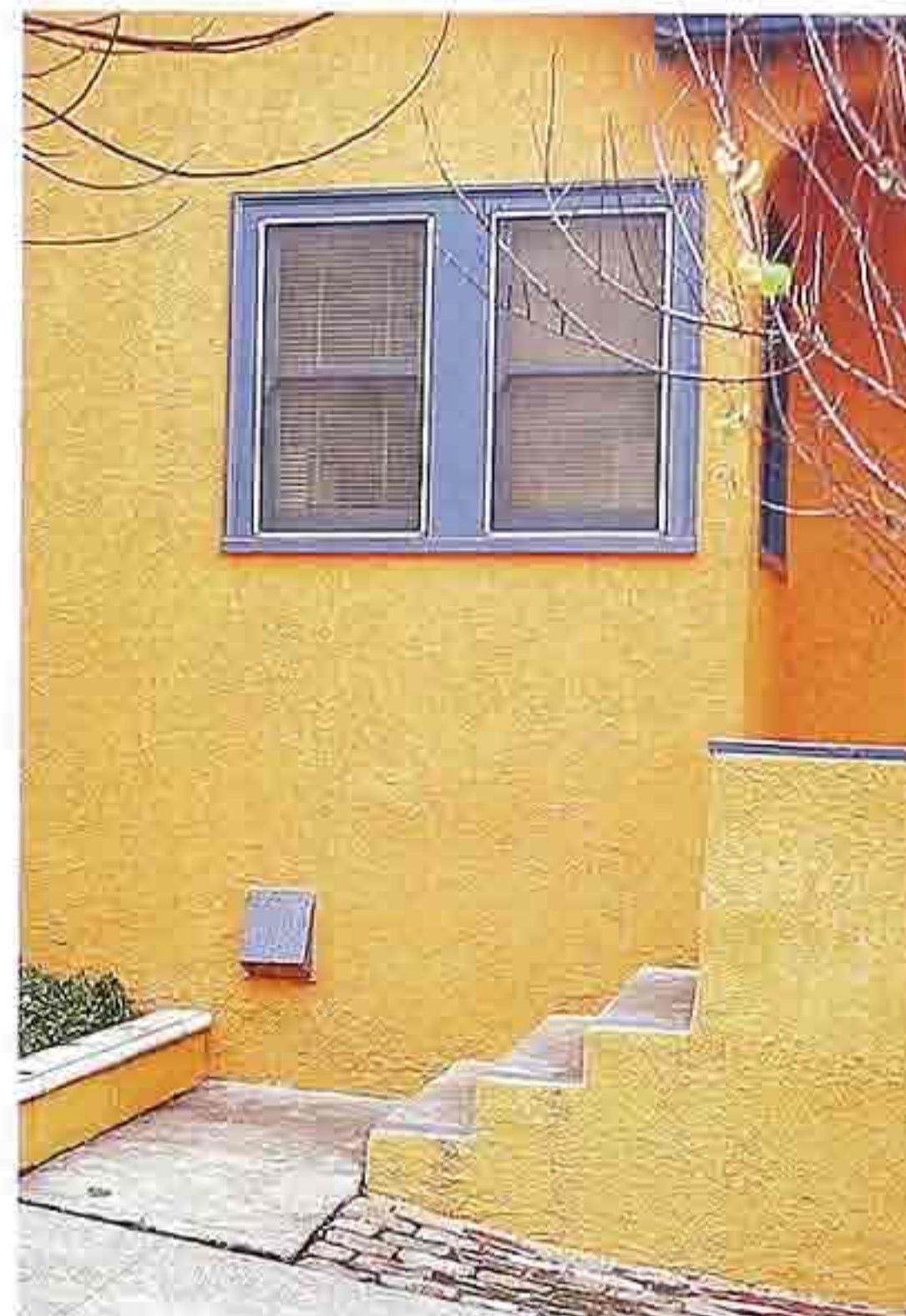
FA-76 Painted textured stucco with contrasting color around window, contemporary house
