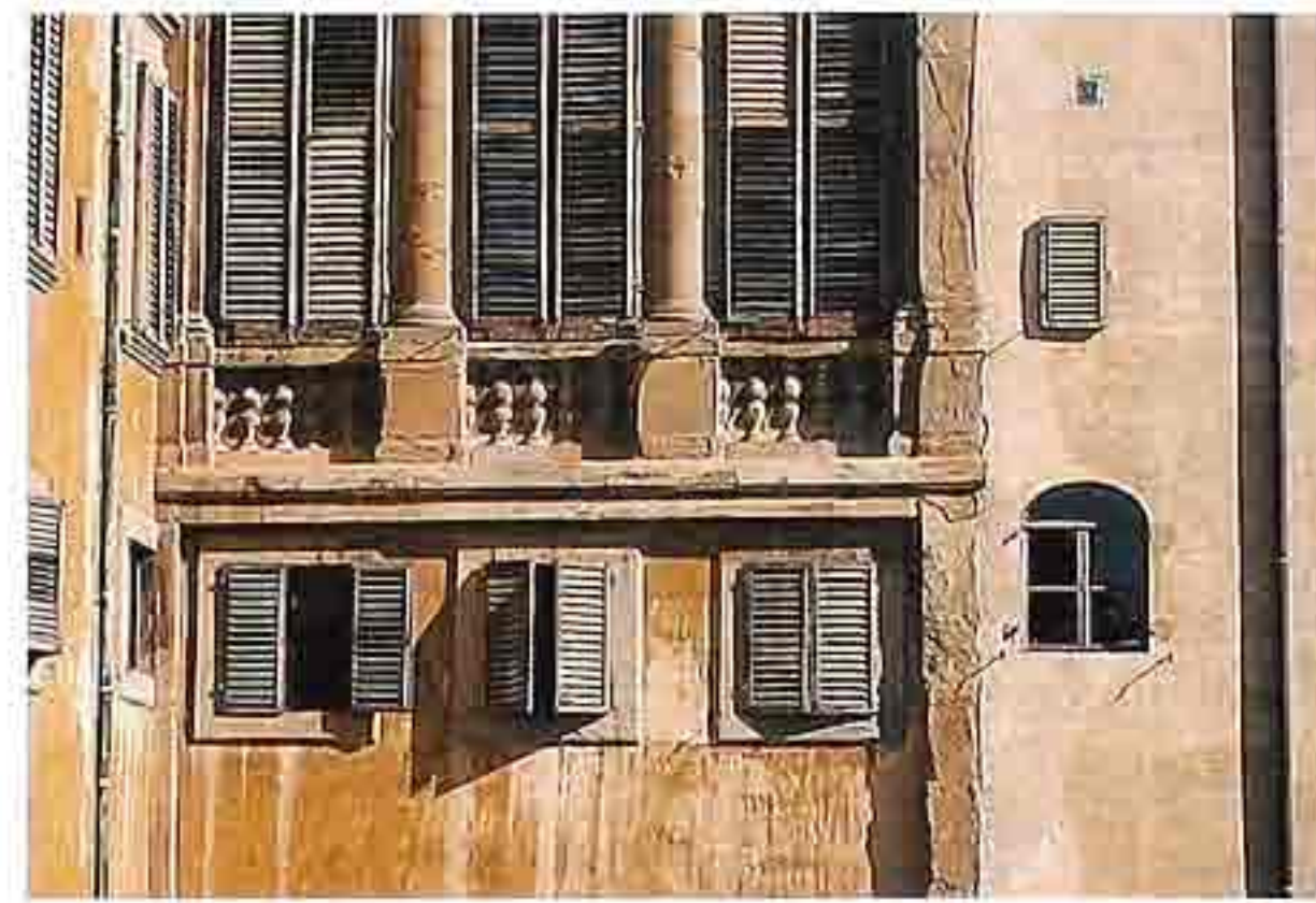
WA-255 Weathered colored smooth stucco on courtyard wall with balcony
