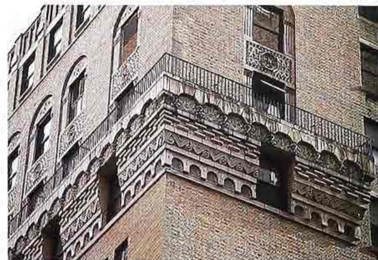
OM-87 Ornamented corbelled courses. Top to bottom: Gothic cornice, three rows of billet molding, zigzag band, Gothic cornice
