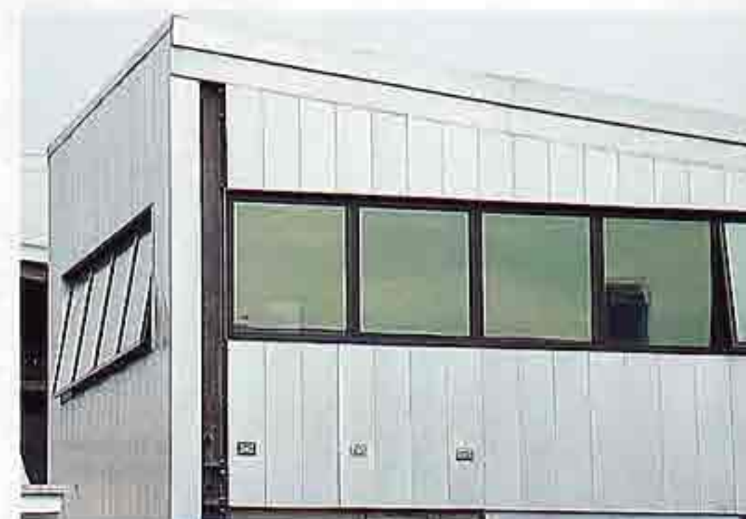
WI-43 Awning windows, modern metal-clad house
