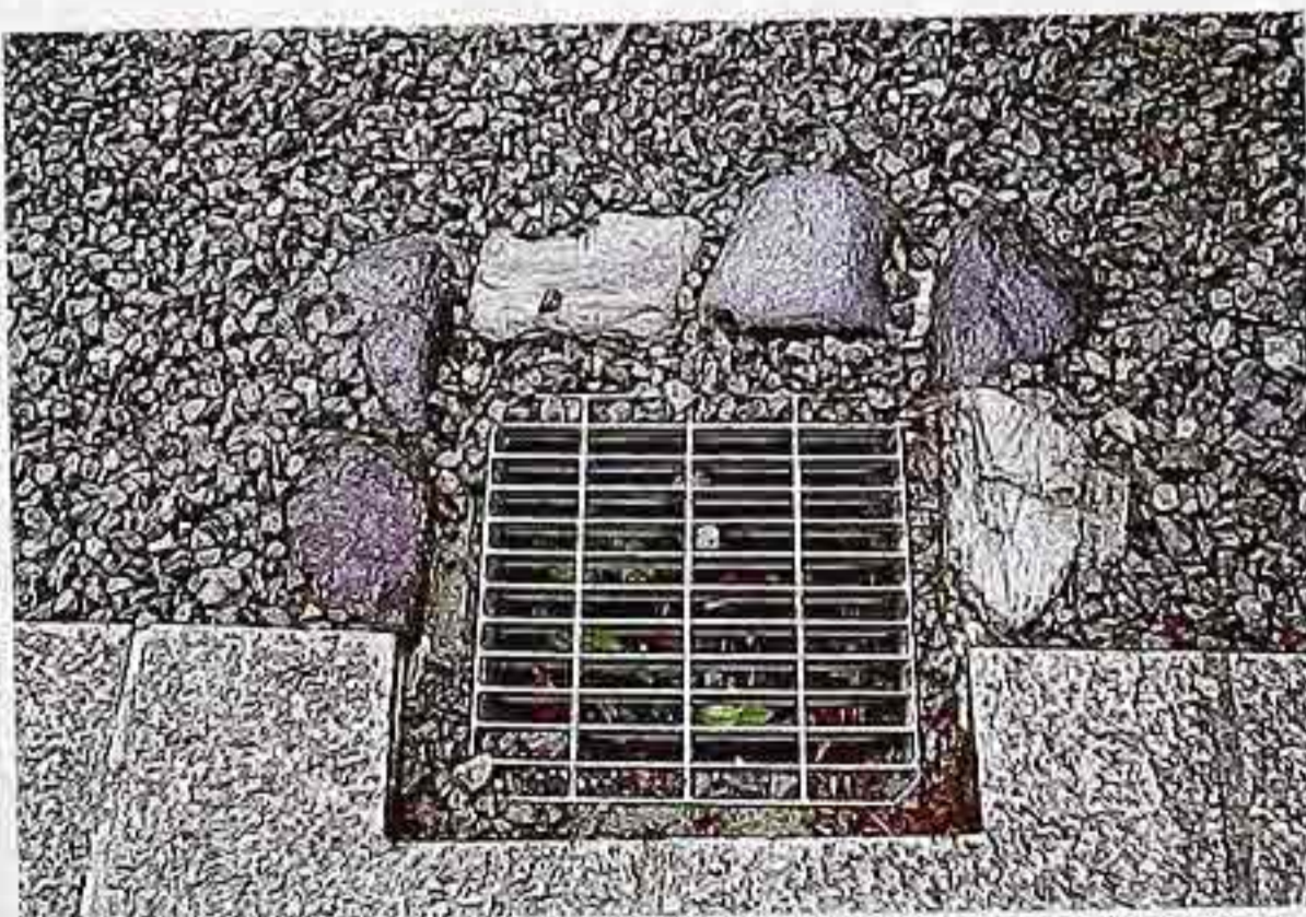
FP-117 Steel drain grate inset into dimension paving stone and gravel with natural rock border
