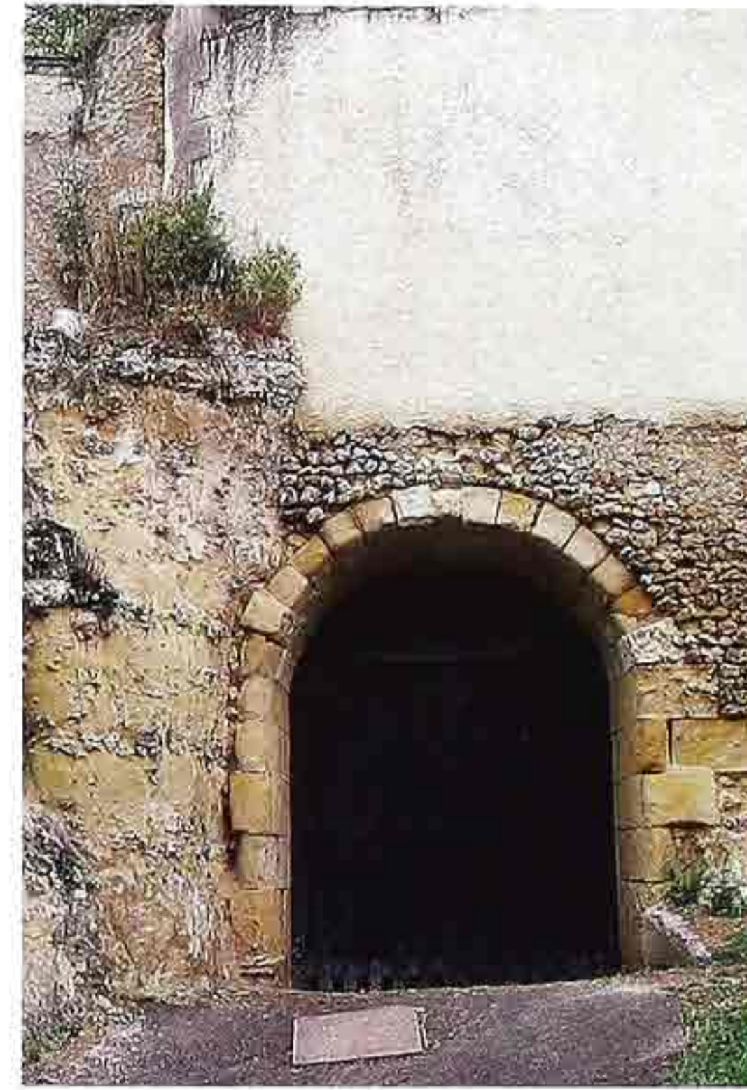
CP-150 Rustic semicircular masonry arch in rubble wall in natural rock formation
