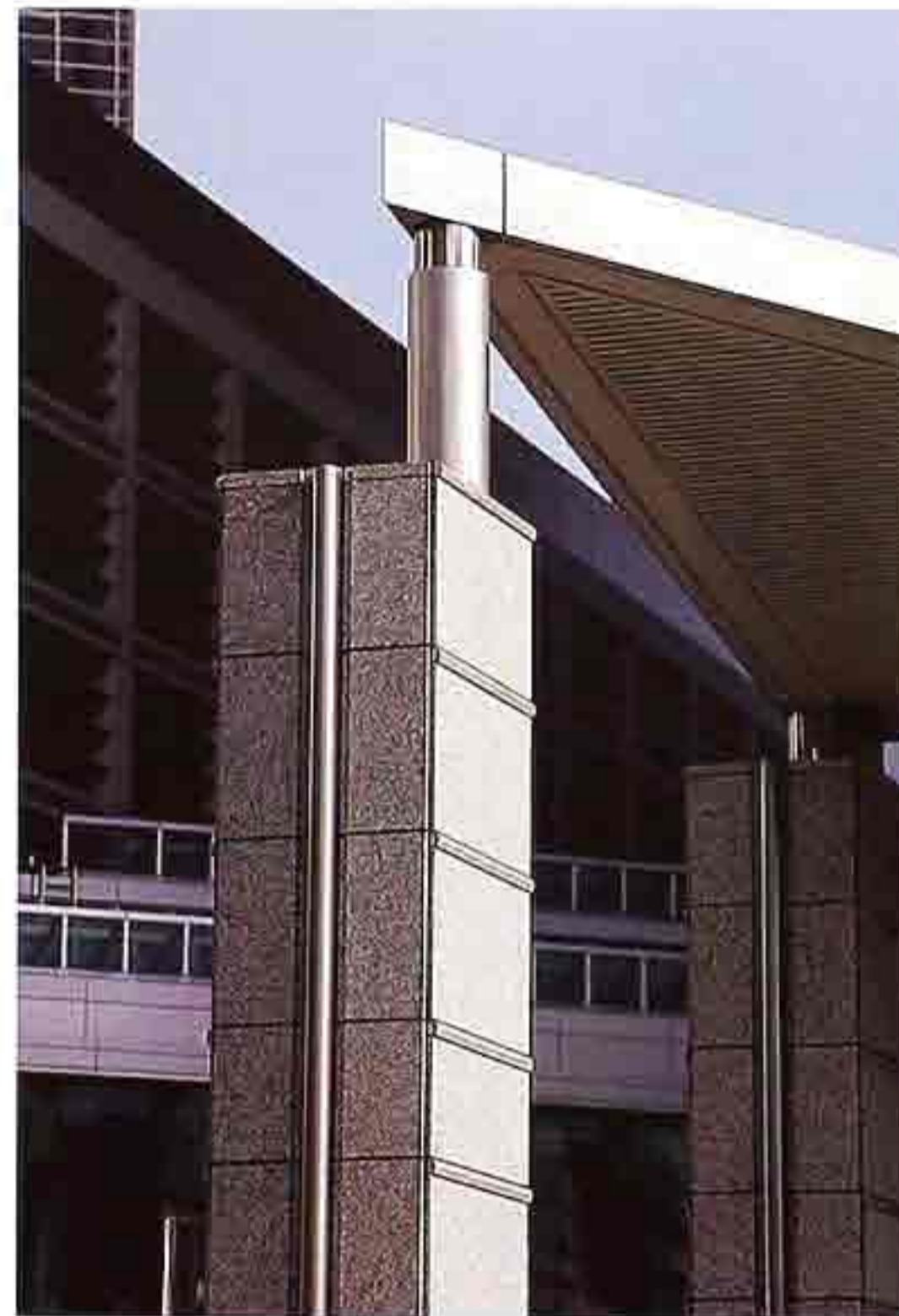
CP-131 Pier with metal post and stone cladding supporting entry canopy, modern commercial building
