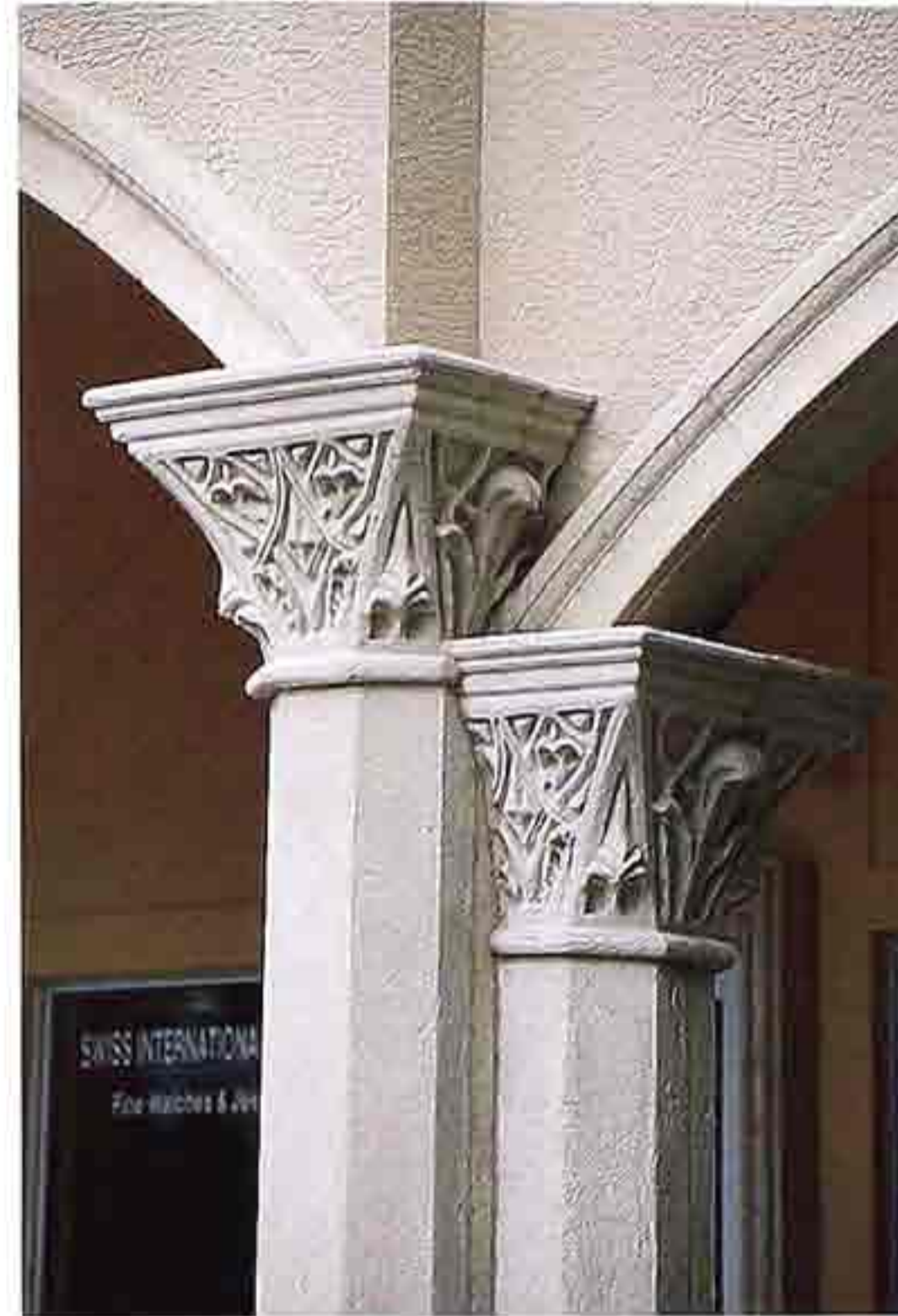
CP-14 Modern derivatives of Byzantine-style square capitals serving as imposts on octagonal shafts
