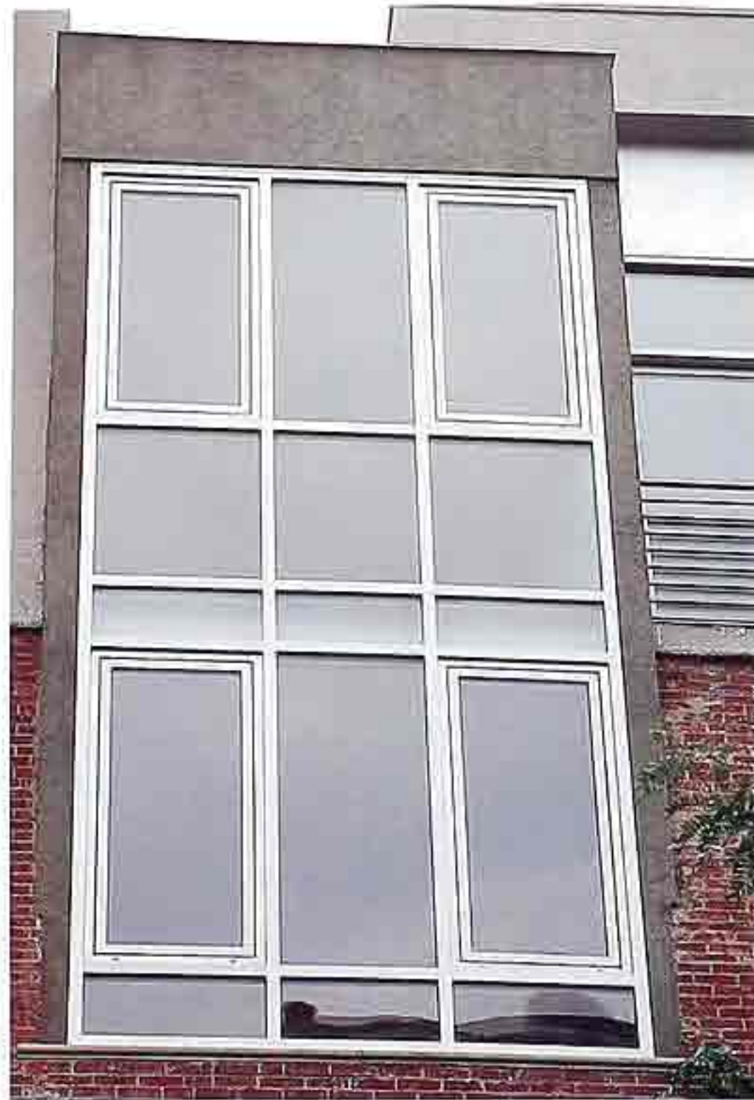
WI-38 Casement or awning windows set in fixed windows with probably extruded aluminum framing, modern townhouse
