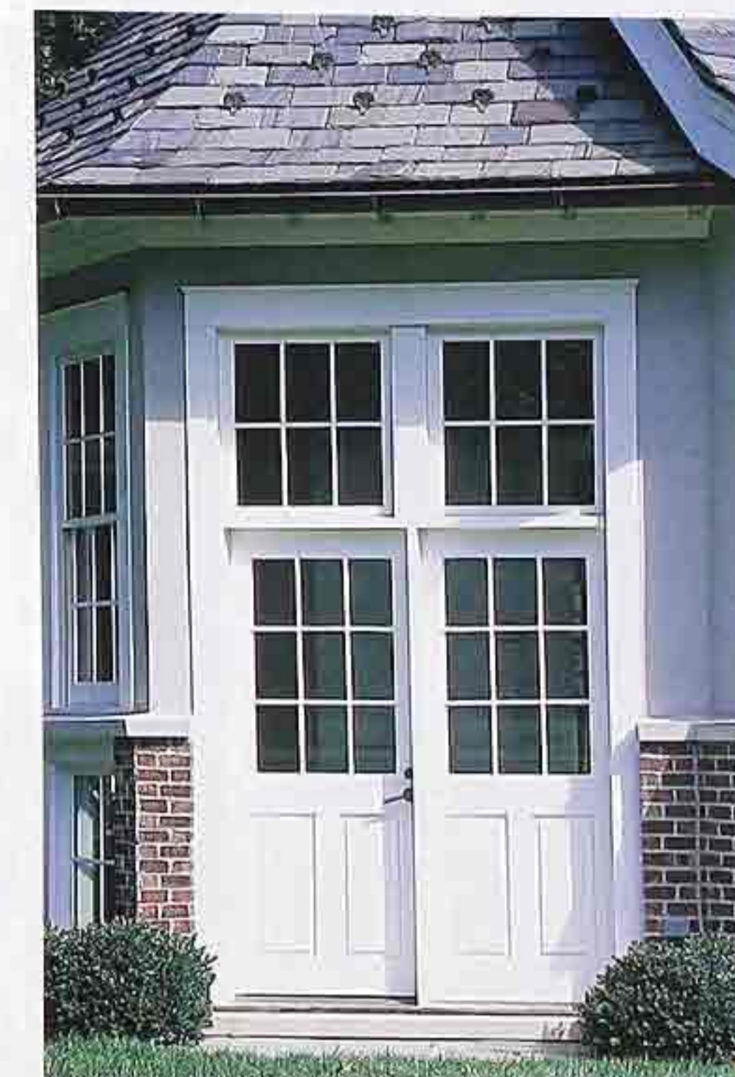
DW-63 Six-light double transom panels over nine-light painted wood double doors with center post, traditional house
