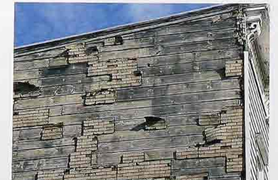
FA-56 Weathered bituminous shingles in faux brick pattern, exposed wood cladding
