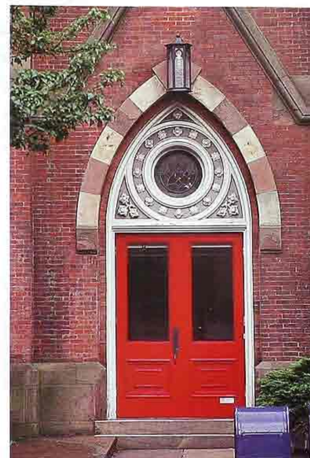
DW-76 Pointed arch in banded stone over carved stone transom panel with bull's eye window; two-paneled single-light double doors, brick church
