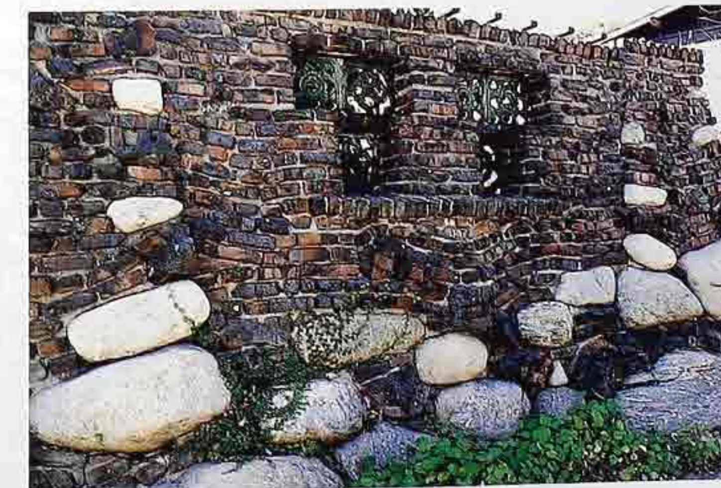
WA-272 Boulders and large cobbles randomly interspersed with custom-bond brick, openings filled with grillework or screen blocks, battered garden wall
