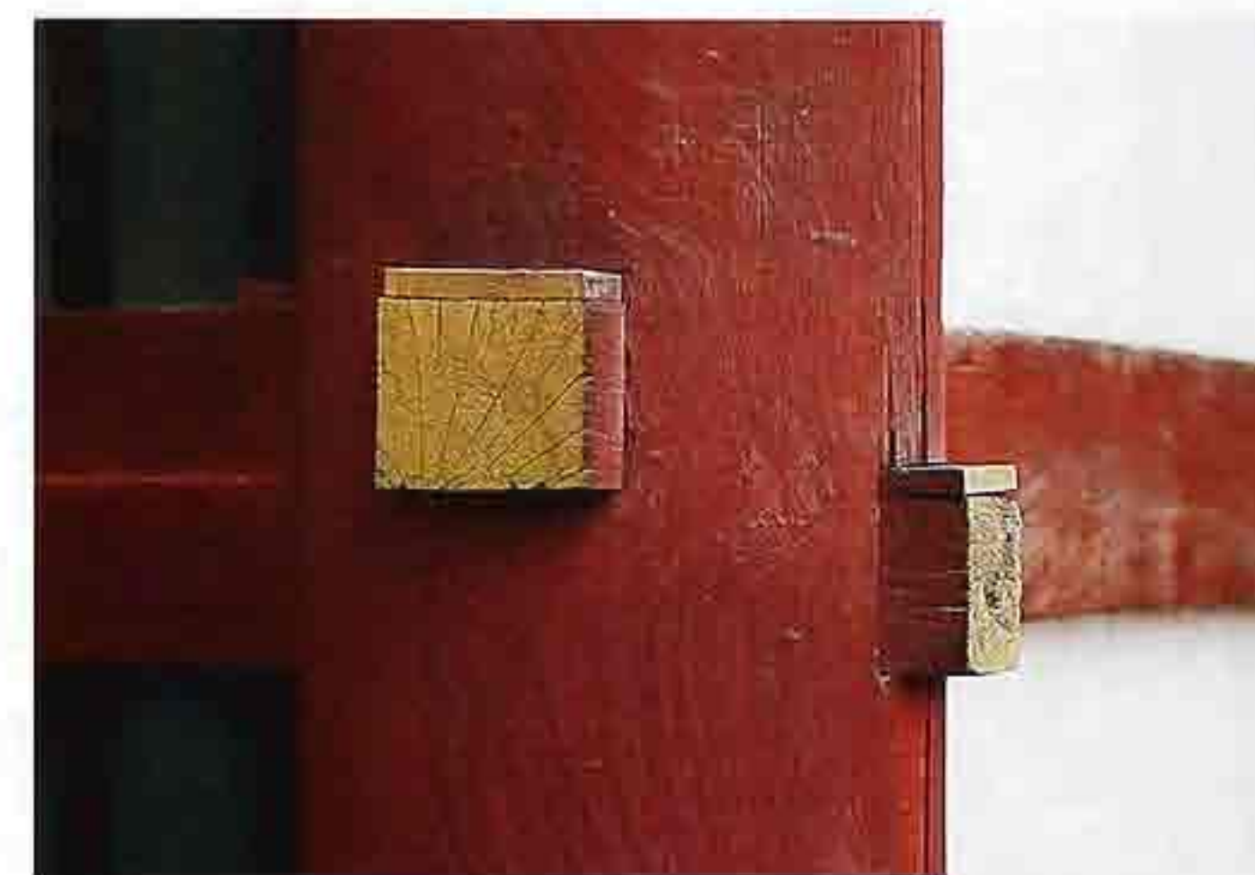
CP-110 Timber corner post with two offset mortise-and-tenon connections to beams.
