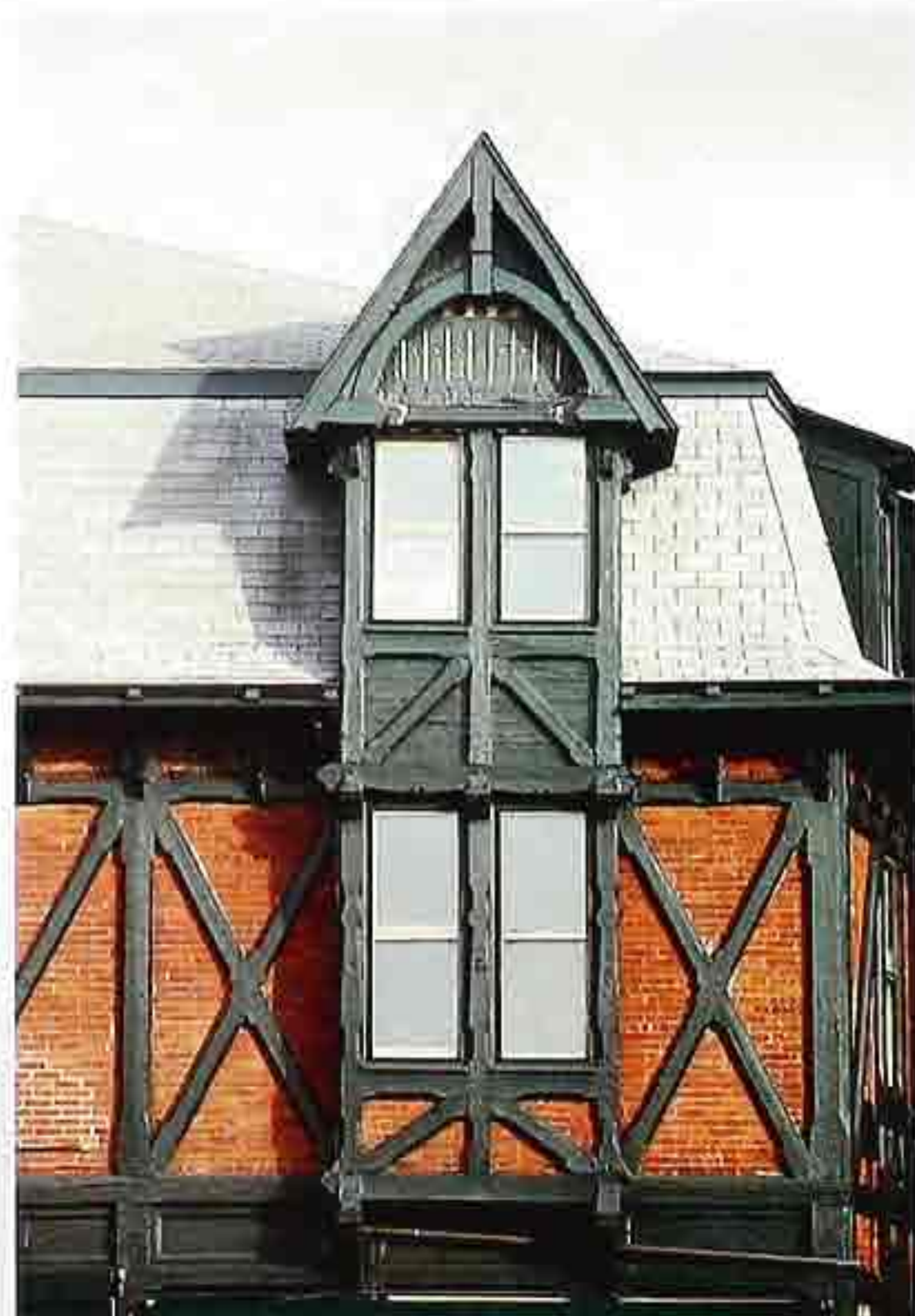
WA-285 Decorative half-timbered facade with flat wood "timbers," brick infill, and bay windows, 20th-c. house
