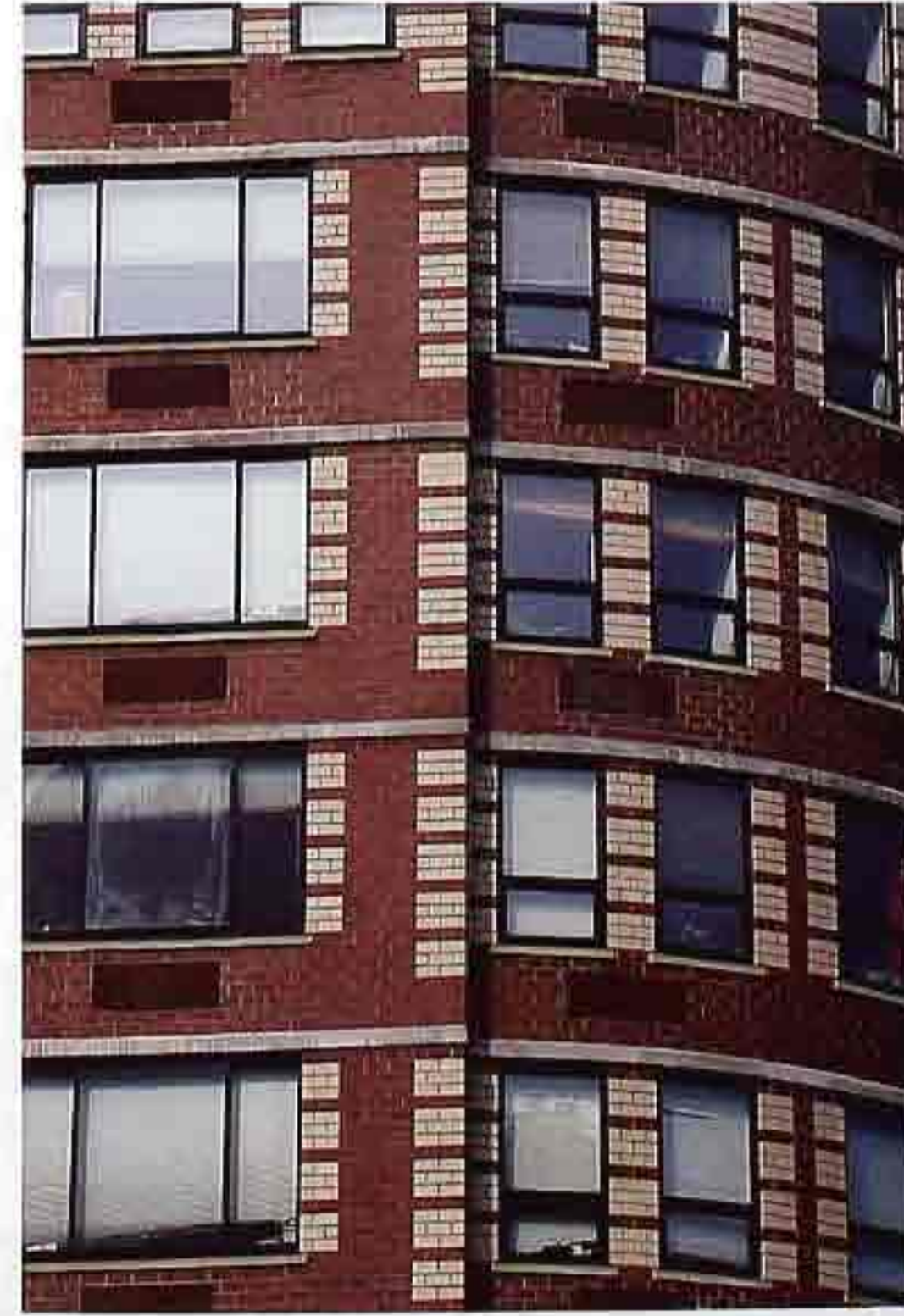
WI-156 Repetitive fenestration of picture windows with side lights and double-hung windows (right) with brick quoins, modern commercial building
