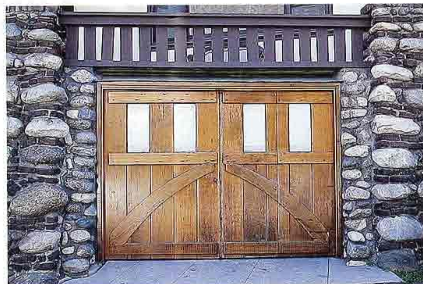
DW-31 Wood double garage doors with lights and curved Z-braces in fieldstone wall, Arts and Crafts house
