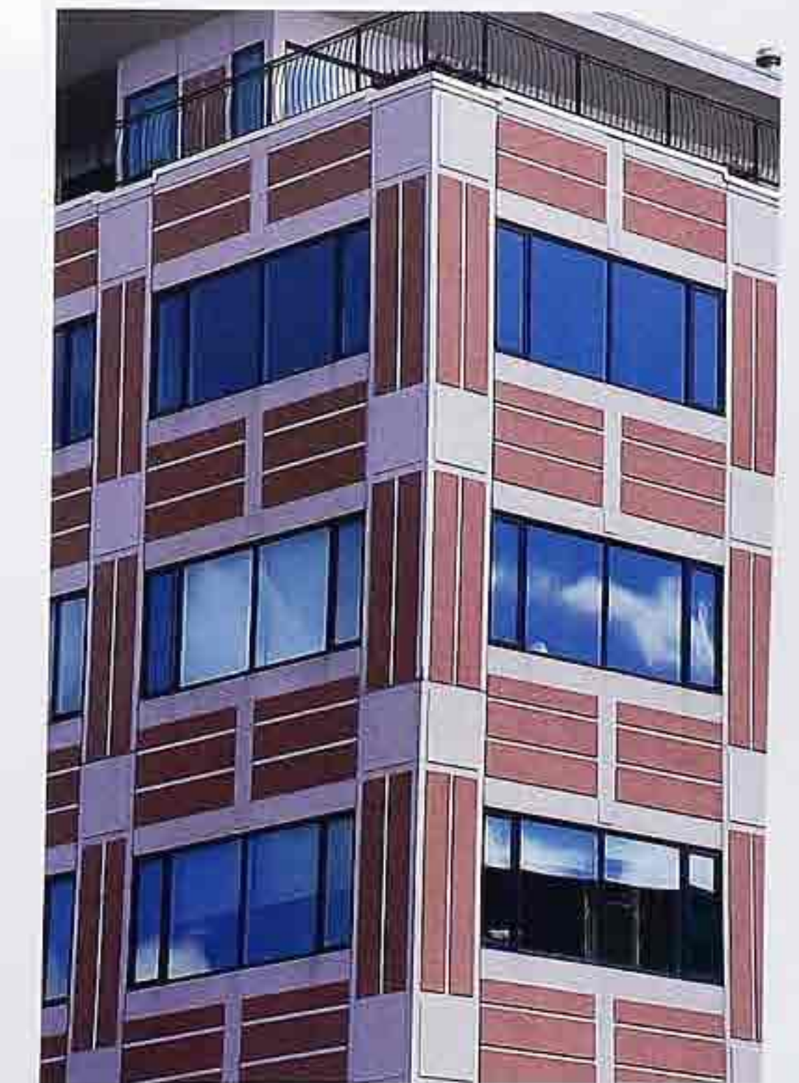
FA-127 Trabeated facade finished in colors suggesting post-and-lintel construction, modern mixed-use building
