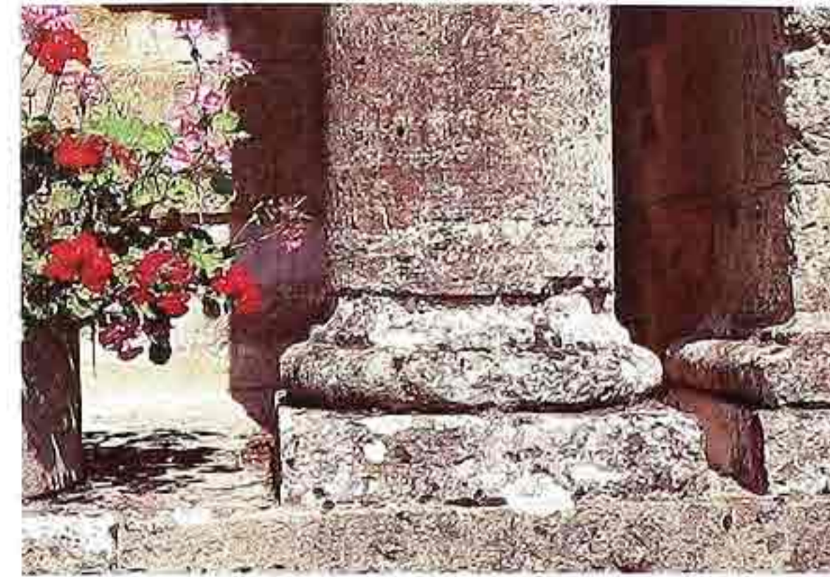
CP-35 Doric base of heavily weathered volcanic stone column on square plinth
