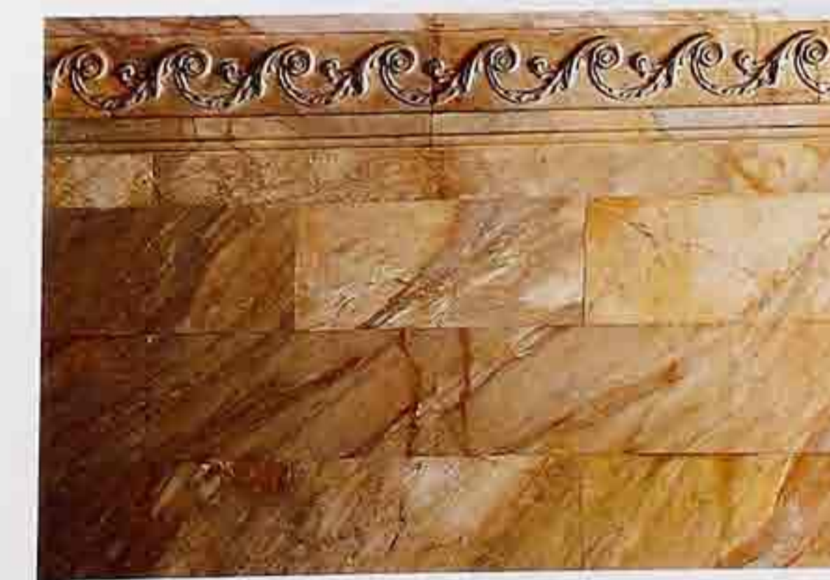
WA-71 Siena marble in running bond with Vitruvian scroll frieze on hallway wall
