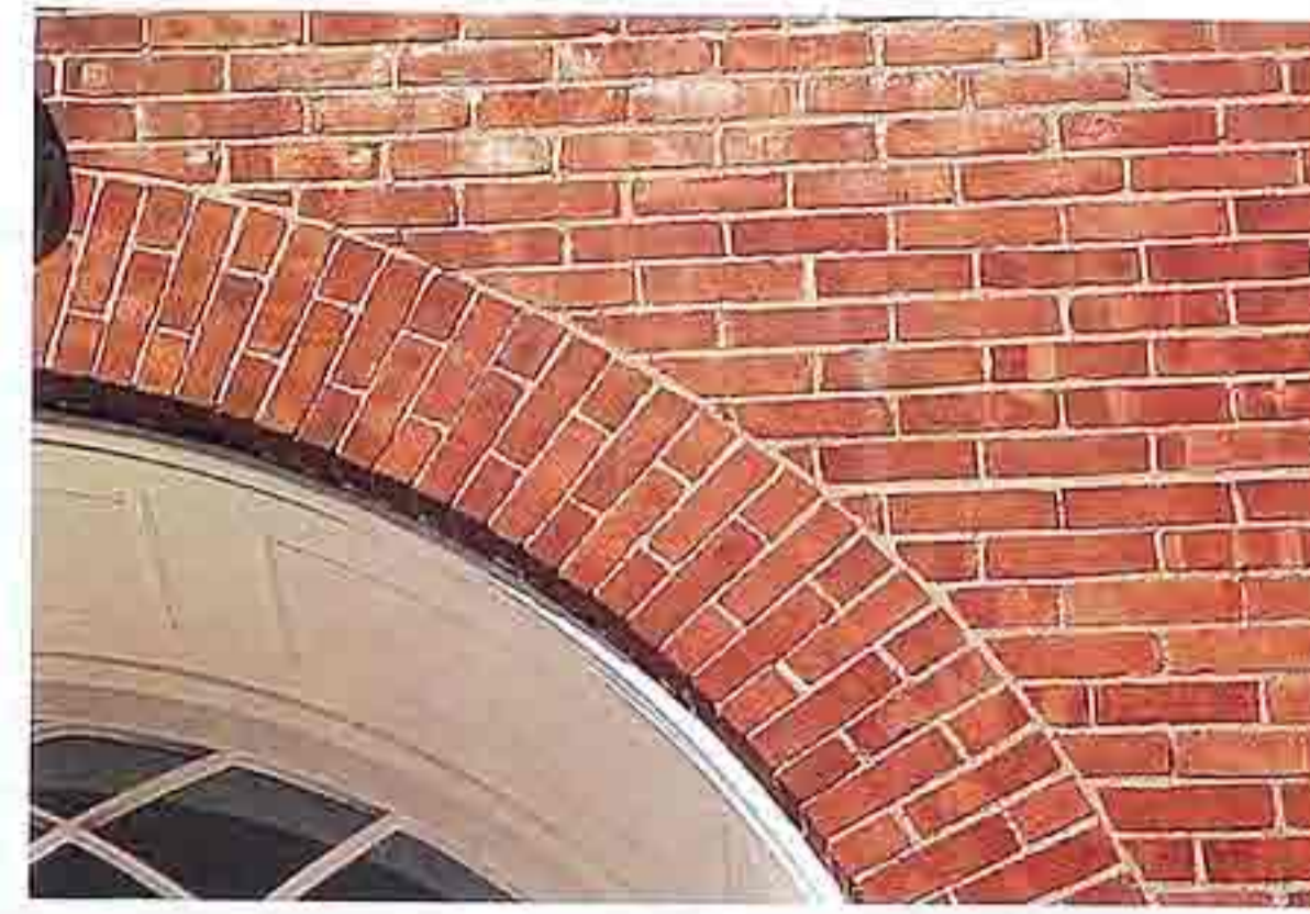
WA-169 Detail of gauged-brick arch surrounded by running bond
