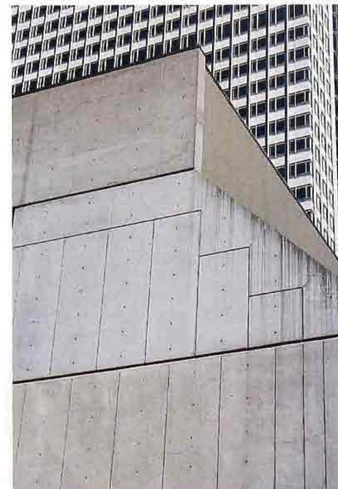
WA-210 Cast concrete with smooth finish, articulated formwork panels, and horizontal expansion joints
