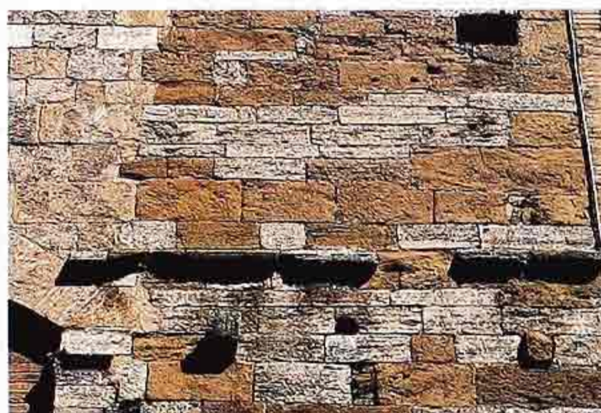
WA-62 Ancient Roman travertine wall in coursed ashlar with sandstone repairs
