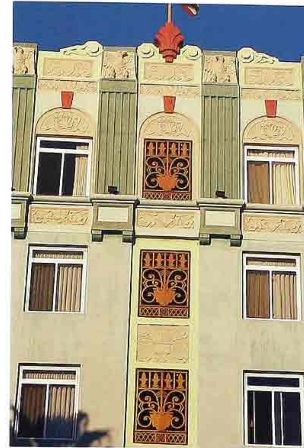
FA-124 Polychrome facade with low relief ornament in stucco and cast concrete, Art Deco hotel
