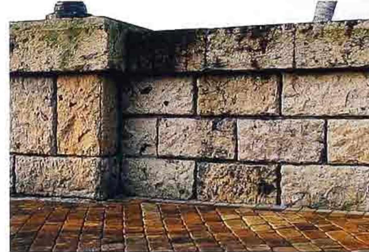
WA-78 Split-faced and rusticated Mexican volcanic stone in running bond, footbridge wall
