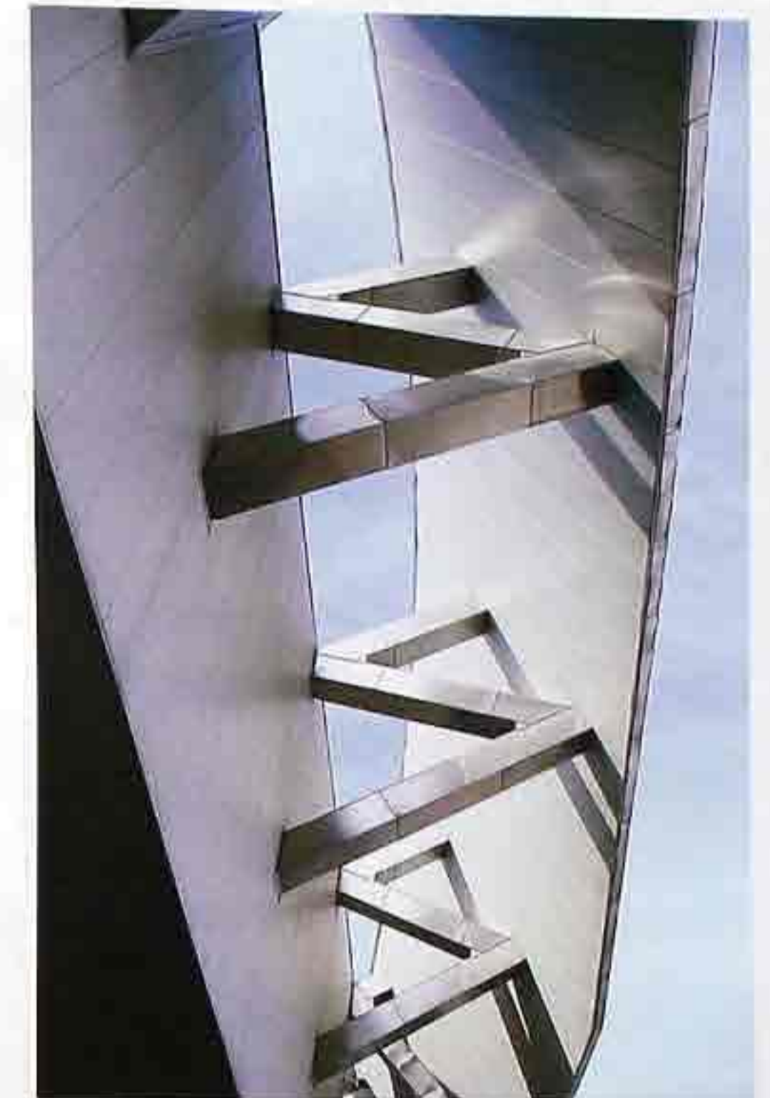
CR-110 Semidetached extension of metal roof connected to facade by Z-shaped brackets, modern commercial building
