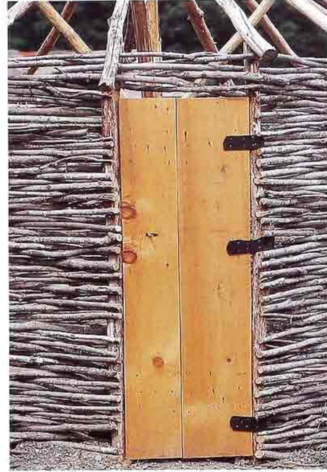
DW-24 Plain-sawn plank door with wrought-iron strap hinges; woven wood walls, 18th-c. corn crib
