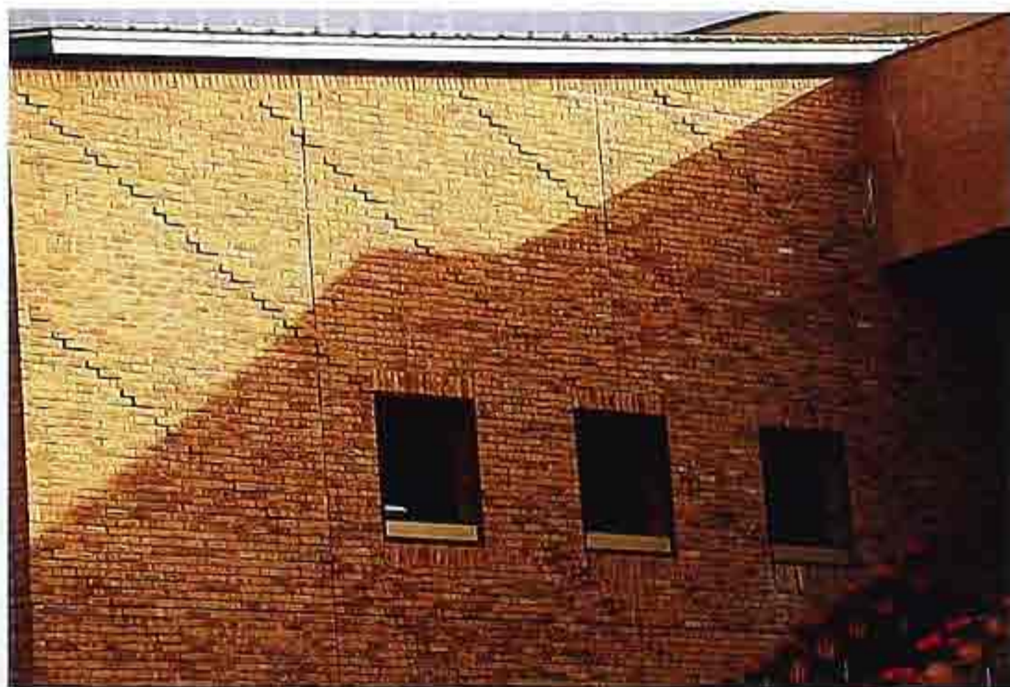
WA-206 Brick in random tones with projecting diagonal pattern and soldier courses above square windows, modern commercial building
