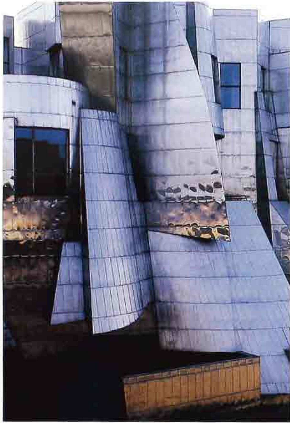
FA-26 Stainless steel shingle cladding with lapped seams, modern institutional building
