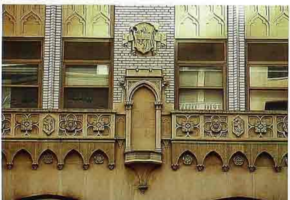
OM-61 Top to bottom: cartouche over a niche; alternating ornamental panels with quatrefoil devices with rosettes; Gothic molding
