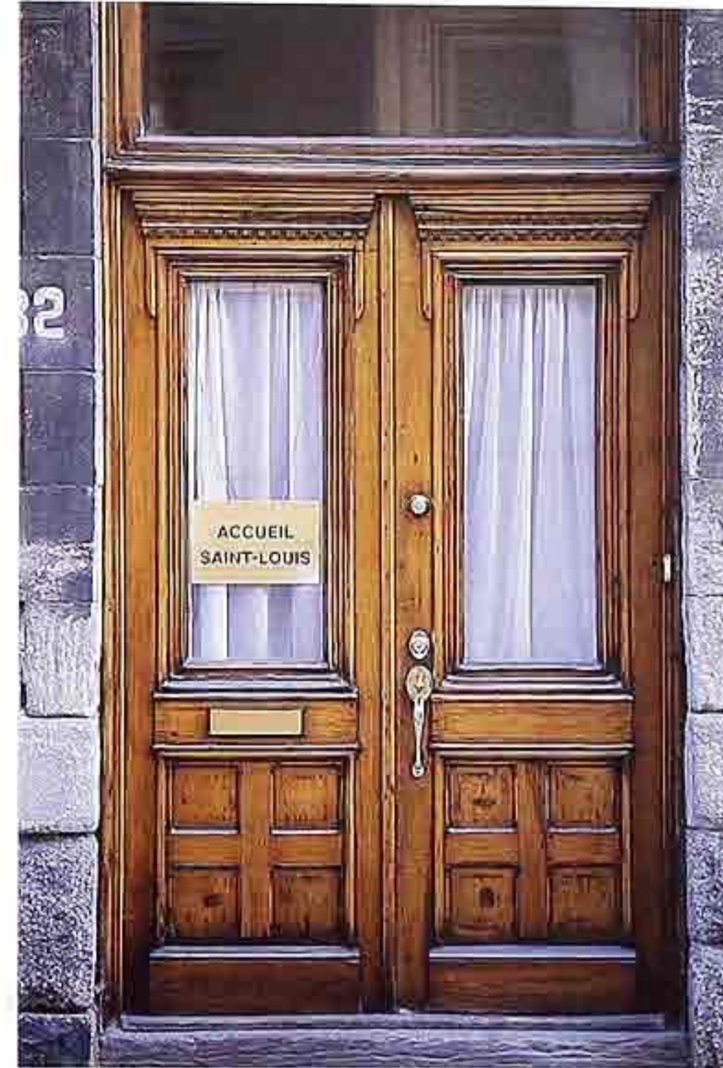
DW-19 Two-panel wood double doors with flush molding; upper panels glass, lower panels divided; letter slot in center stile; split transom light
