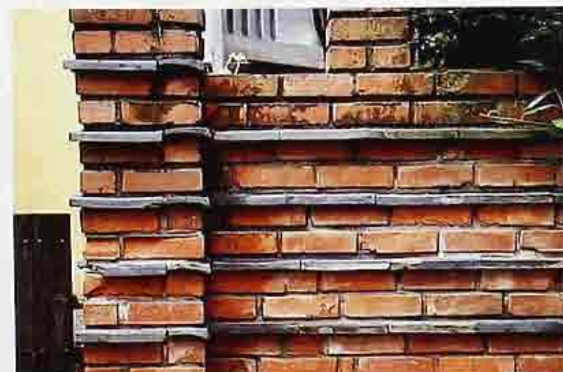
WA-268 Single courses of slate alternating with double courses of brick in running bond, garden wall
