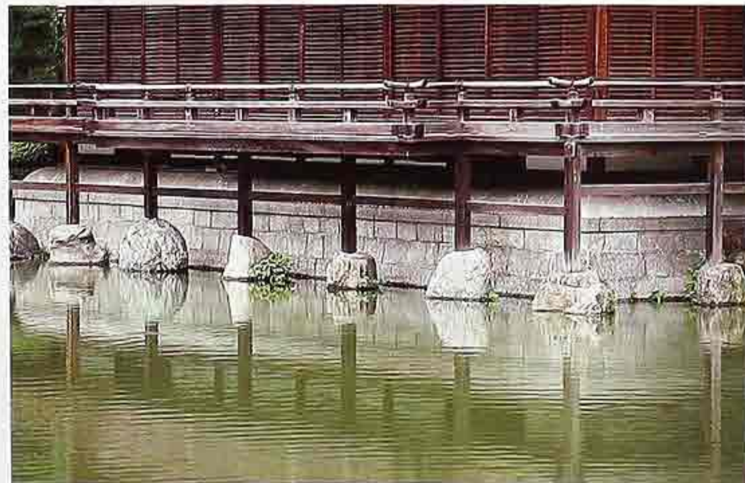
CP-53 Natural boulders supporting timber posts under deck of pavilion in Japanese garden pond
