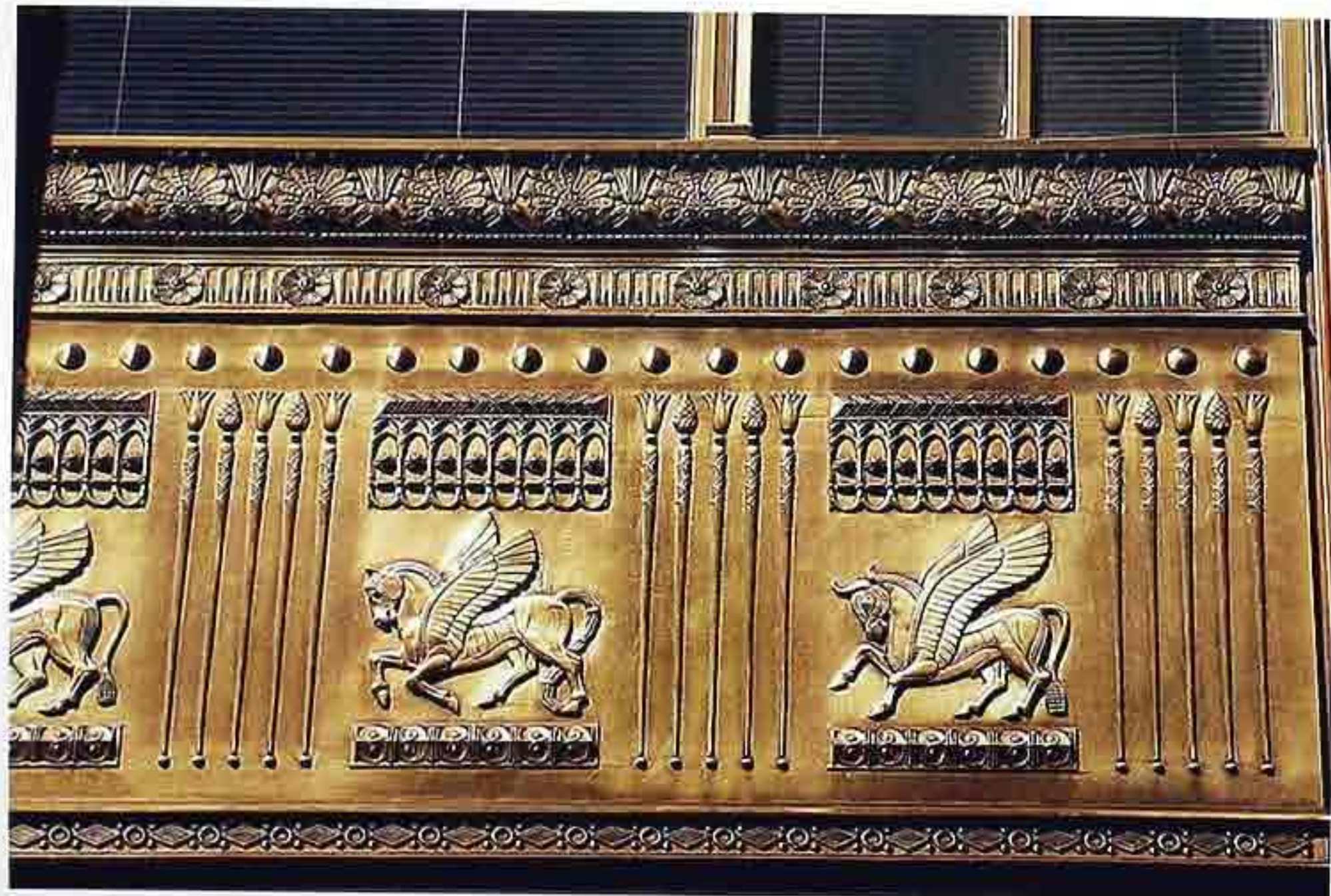
OM-3 Cast bronze frieze based on classical entablature: Pegasus figures ("metopes") alternating with "torch" ornaments ("triglyphs")
