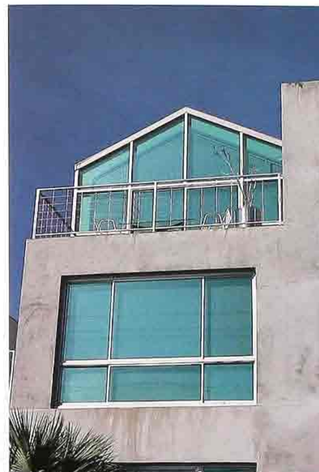
WI-15 Colored glass in stainless steel frame in lower window and gable wall, modern mixed-use building
