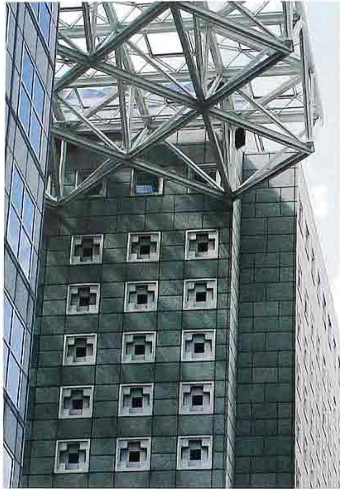
WA-138 Granite veneer with contrasting granite window inserts surmounted by space frame, modern commercial building
