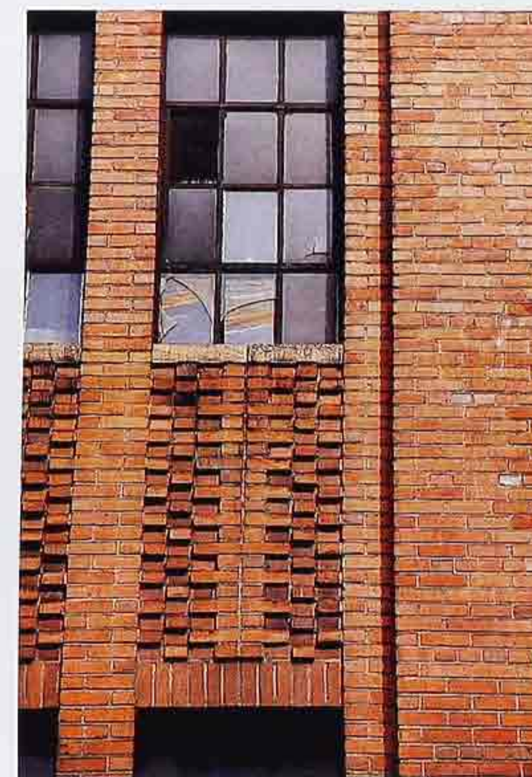
WA-182 Common bond with sixth-course headers; recessed spandrels with checker pattern; soldier course above windows
