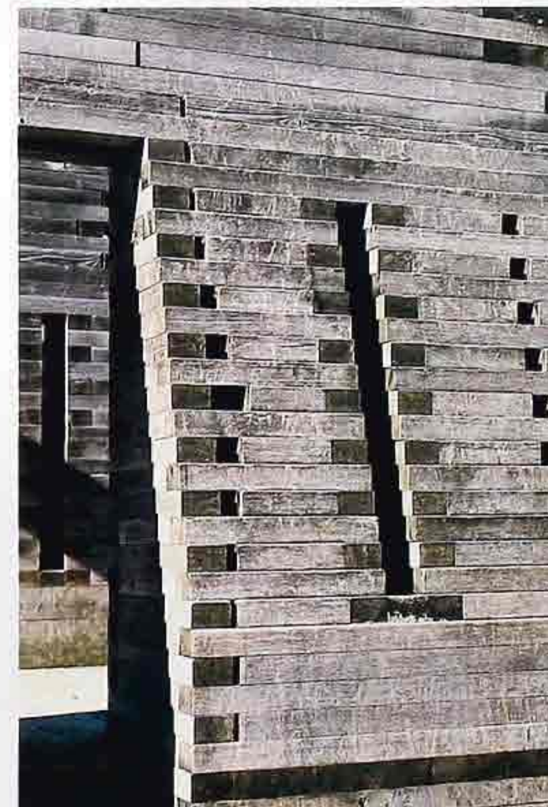
WA-49 Fortification-style battered wall with lapped-joint corners
