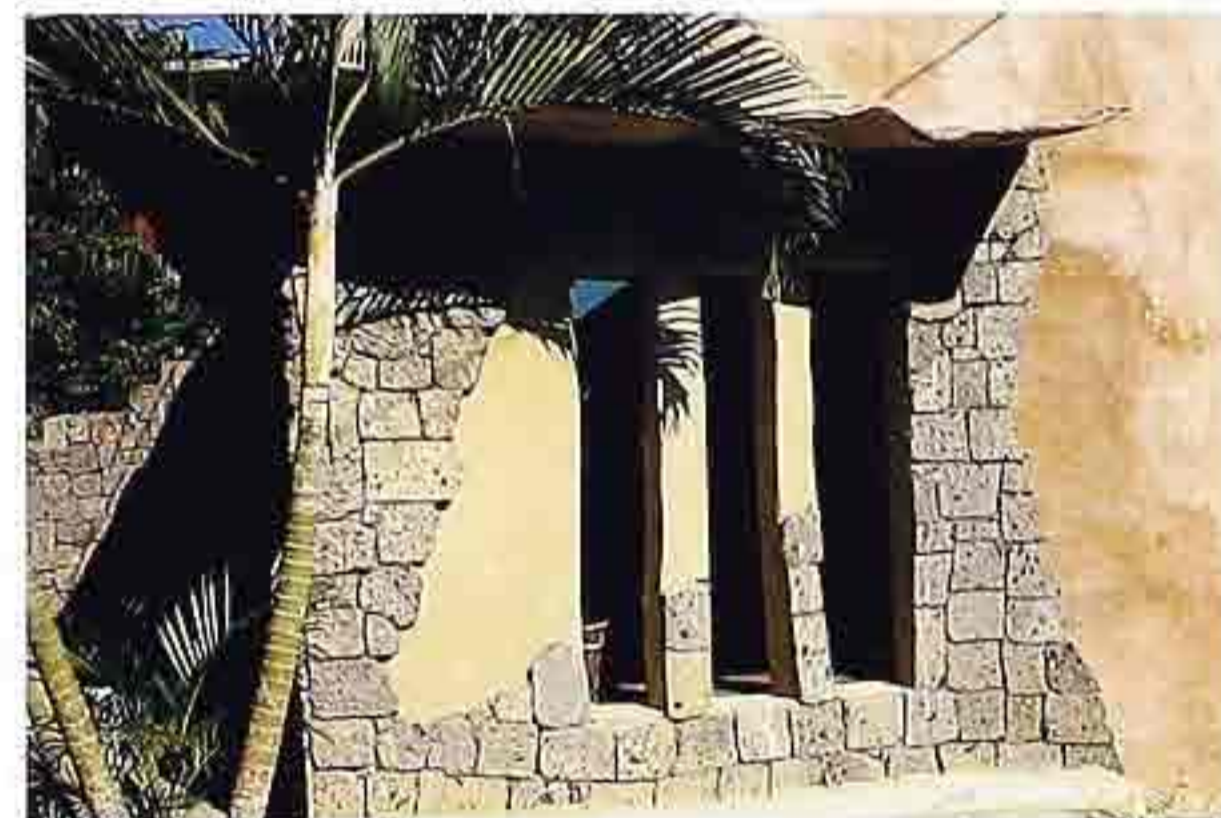
WA-241 Stucco over random ashlar stone
