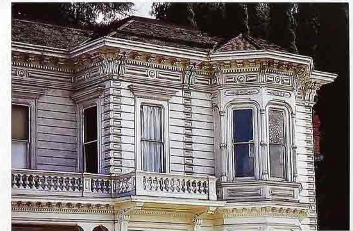
WI-116 Ornament, molding, and balustrade around double-hung windows in cant-bay and wall windows; 19th-c. American clapboard house
