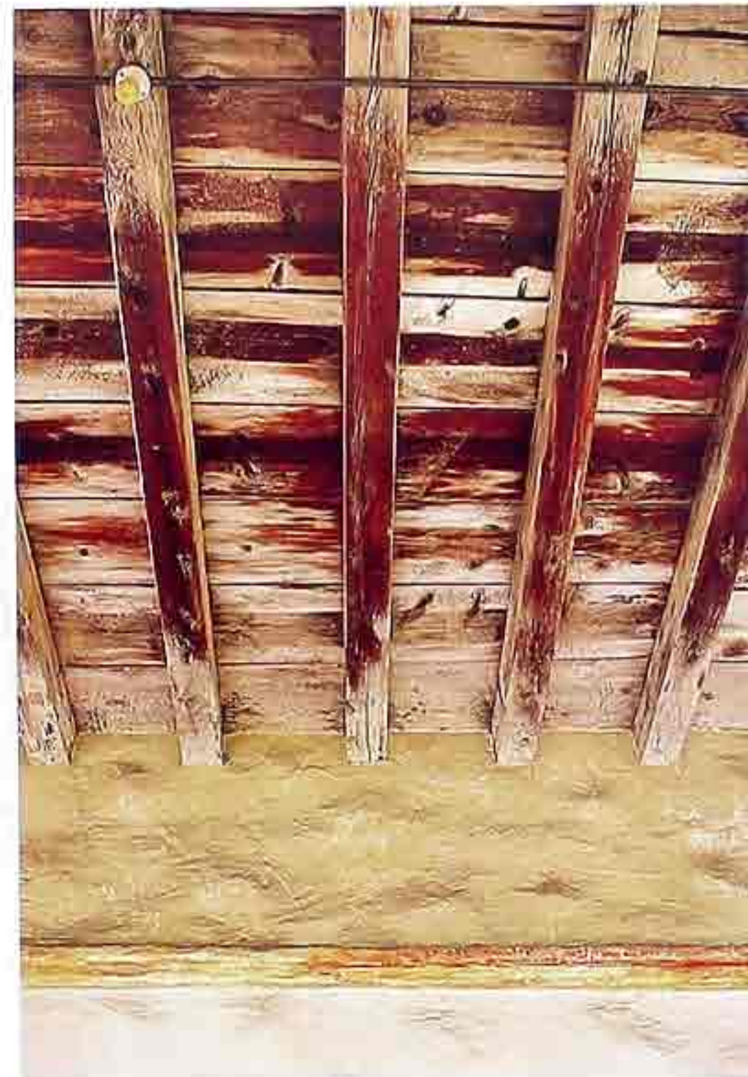
CR-2 Roughly hewn exposed rafters anchored in adobe wall and covered with rough-sawn planks; 18th-c. American Southwestern mission
