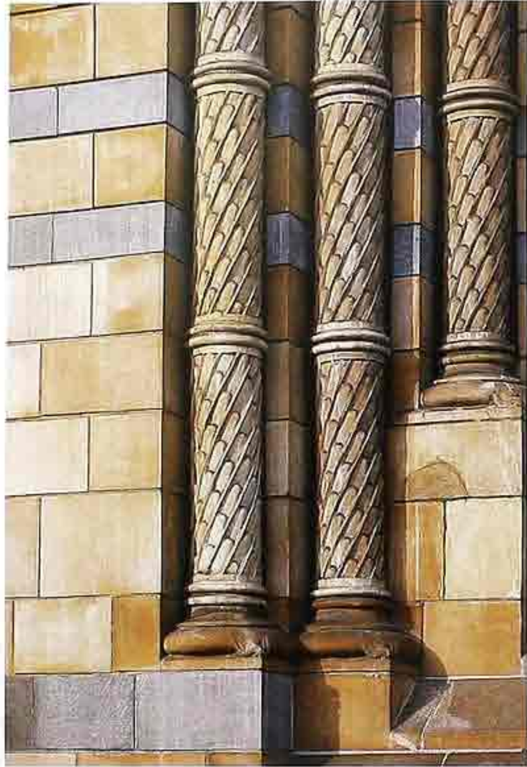
CP-96 Reticulated colonnettes (jamb-shafts) in a portal with annulets
