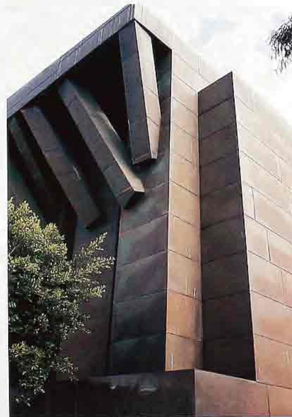
FA-13 Copper cladding, modern commercial building
