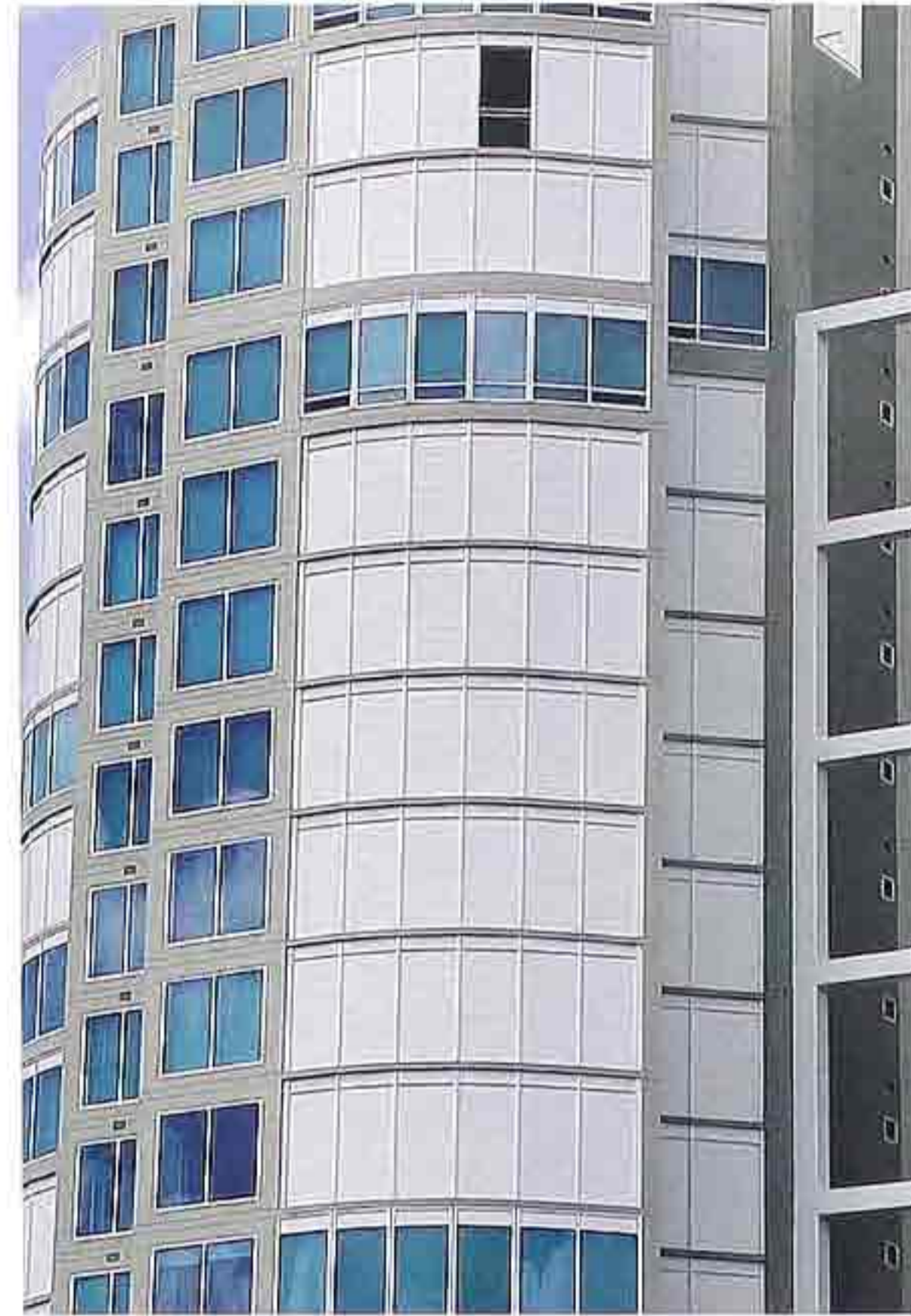
WI-203 Hurricane shutters, modern apartment house
