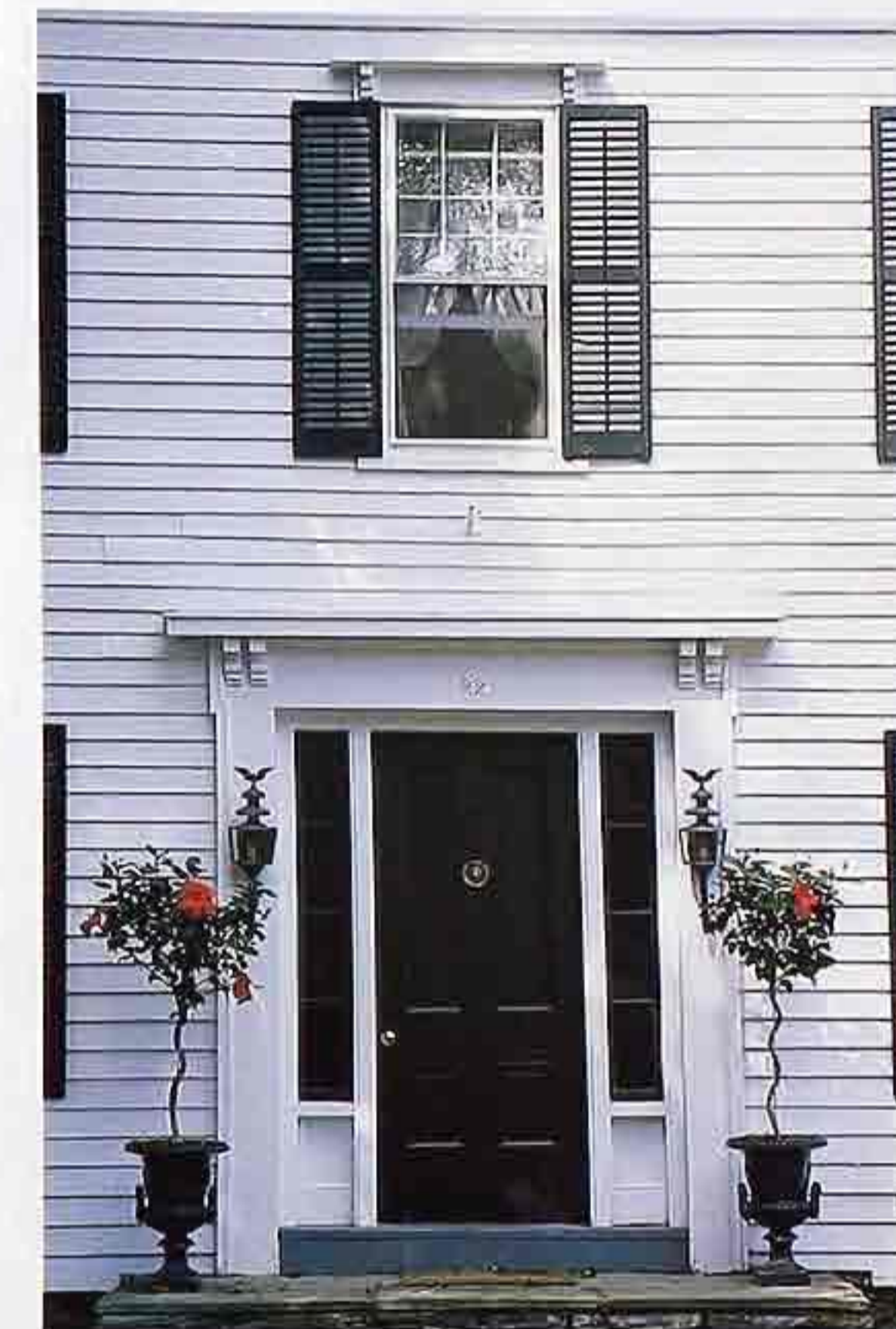
DW-85 Crown molding door hood on cut brackets over paneled door with side lights, 19th-c. American house
