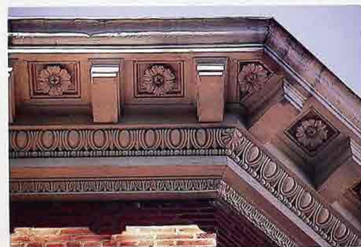
OM-90 Top to bottom: Corinthian cornice; block modillions between coffers with rosettes; egg- and leaf-and-dart moldings; simple fascia; bead-and-reel molding; tongue-and-dart molding
