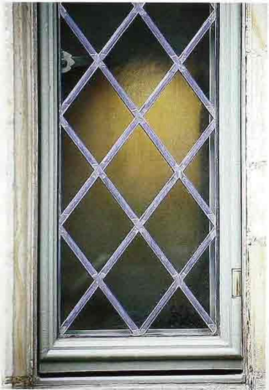
WI-3 Leaded casement window with came in diamond lattice pattern
