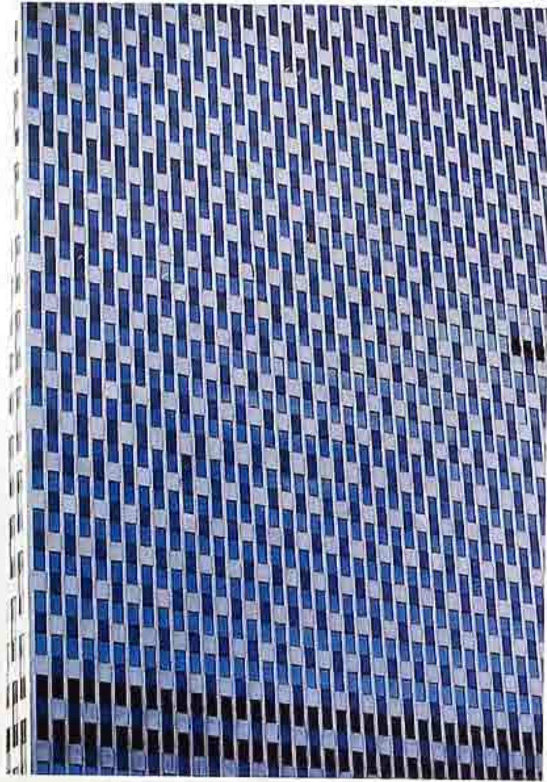
FA-32 Cladding system of staggered spandrel elements, probably pre-cast concrete and glass.
