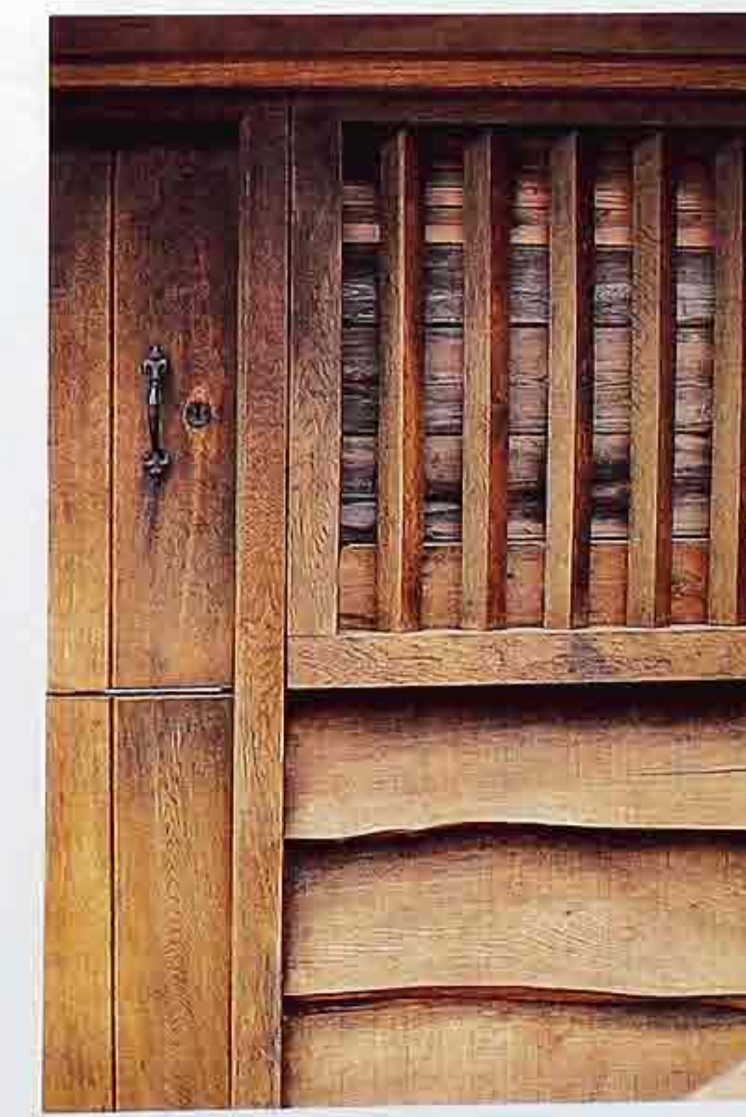
WA-8 Batten door (left); shutter behind diagonally split square-stock wood bars (upper right); elm waney-edged clapboard bottom (lower right) on an outbuilding
