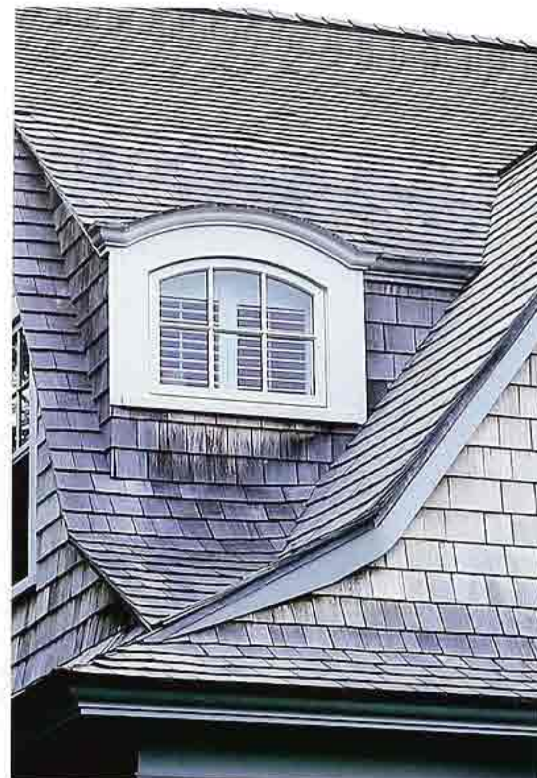
CR-65 Alaskan yellow cedar shingles; roof valley at intersection of gables; traditional American house.
