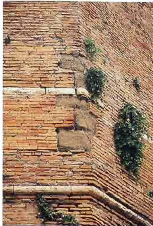
WA-159 Ancient Roman brick running-bond wall with stone quoins, banding course, and bead molding
