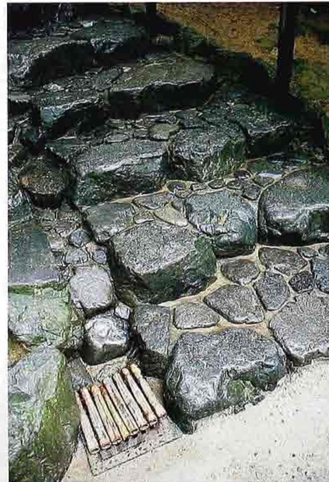
FP-46 Steps made from roughly squared split, polished fieldstone set in concrete. Bottom left: bamboo drain cover
