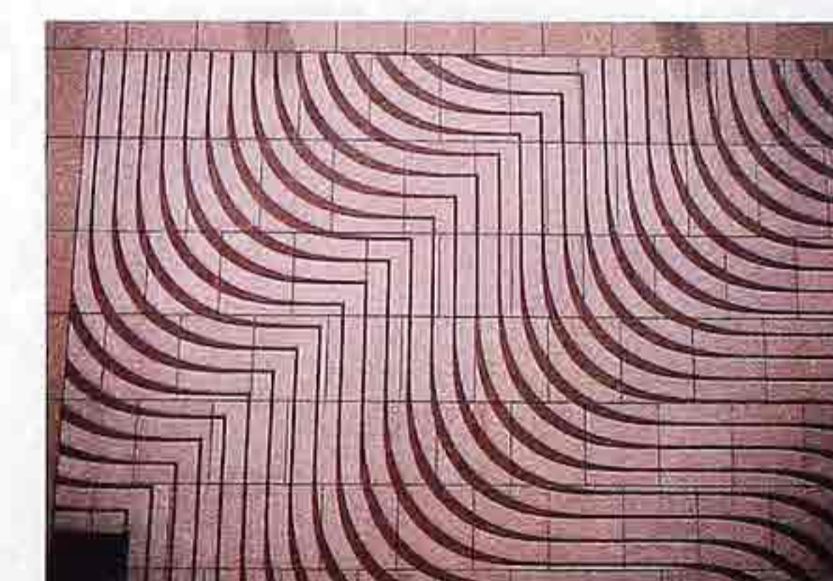
WA-69 Pink granite in running bond with polished and flamed finishes forming supergraphic, modern commercial building
