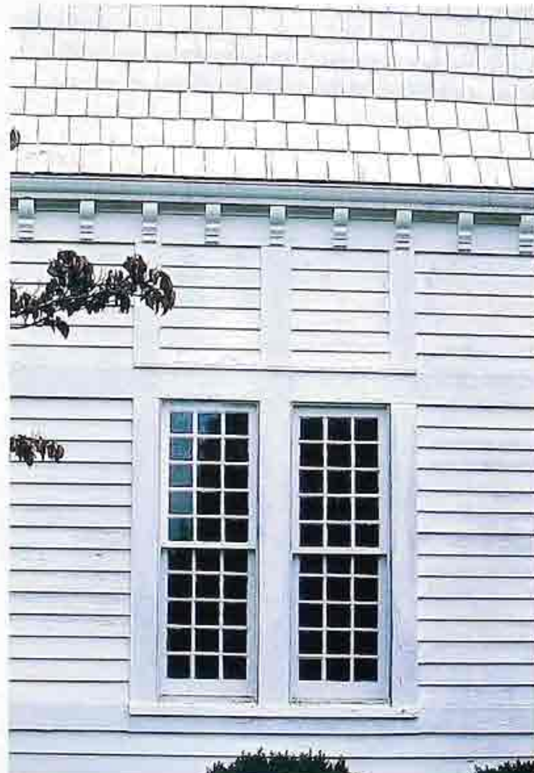
WA-39 Painted clapboard siding divided by wide trim, double-hung windows, modillion cornice, and painted shingled roof
