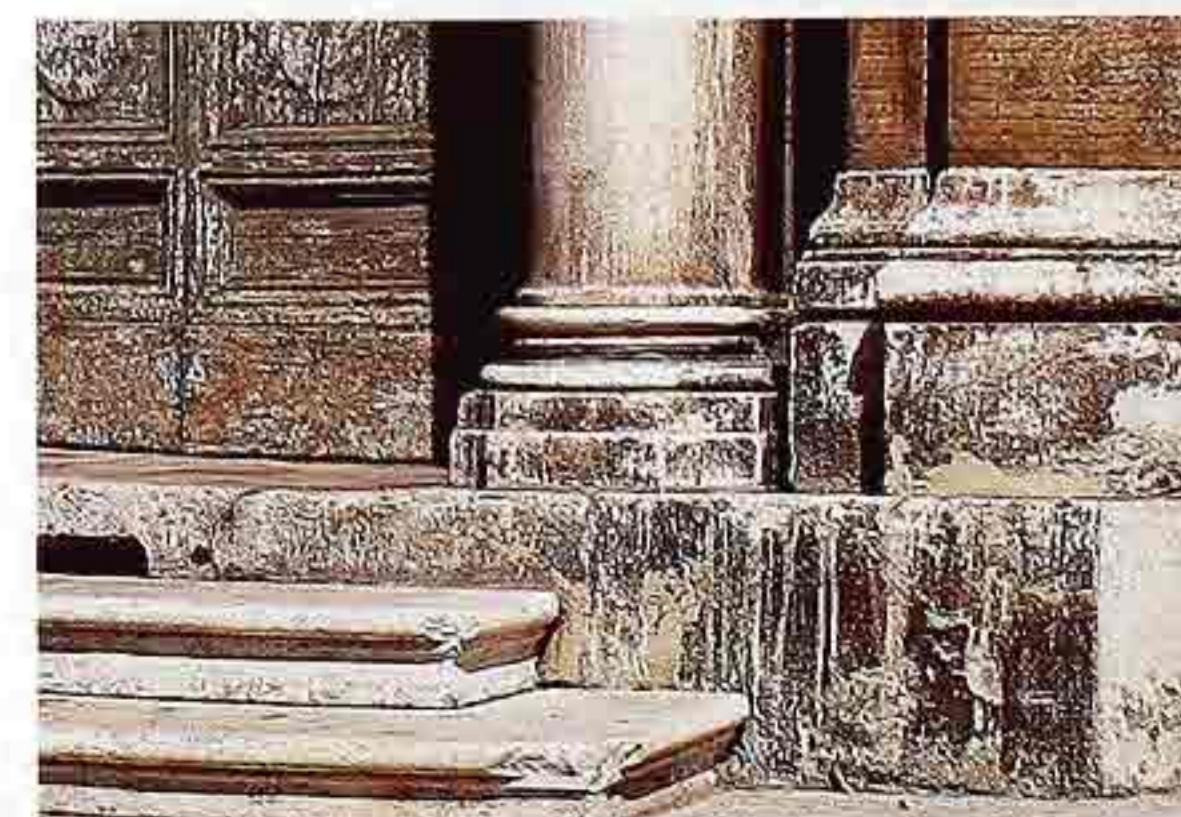
CP-39 Weathered marble column with Attic base on stepped octagonal plinth; right: brick pilaster on square marble base
