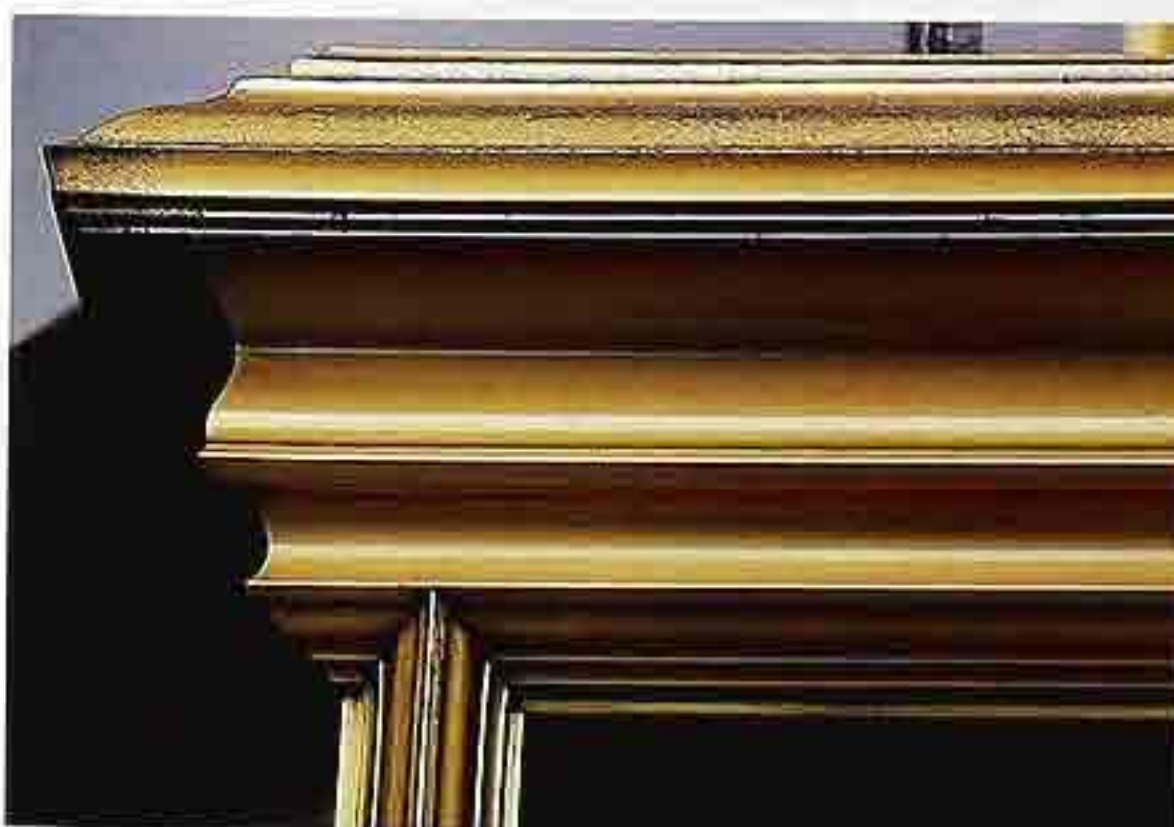
OM-77 Cast metal molding. Top to bottom: cyma recta, cove, stepped fillets, cavetto, cyma recta, cyma reversa
