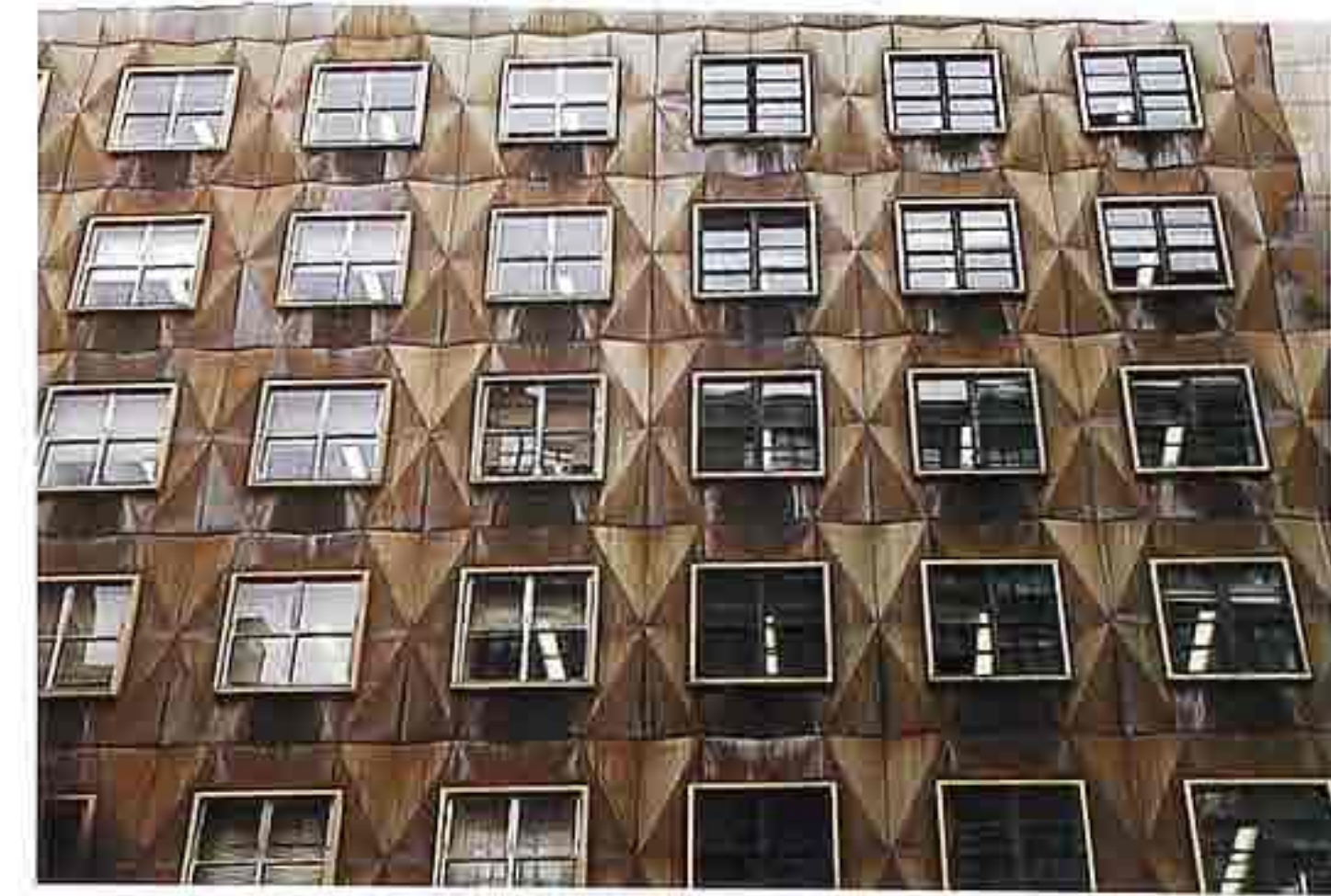
FA-23 Weathered panelized wall system with stamped diamond pattern, modern apartment house
