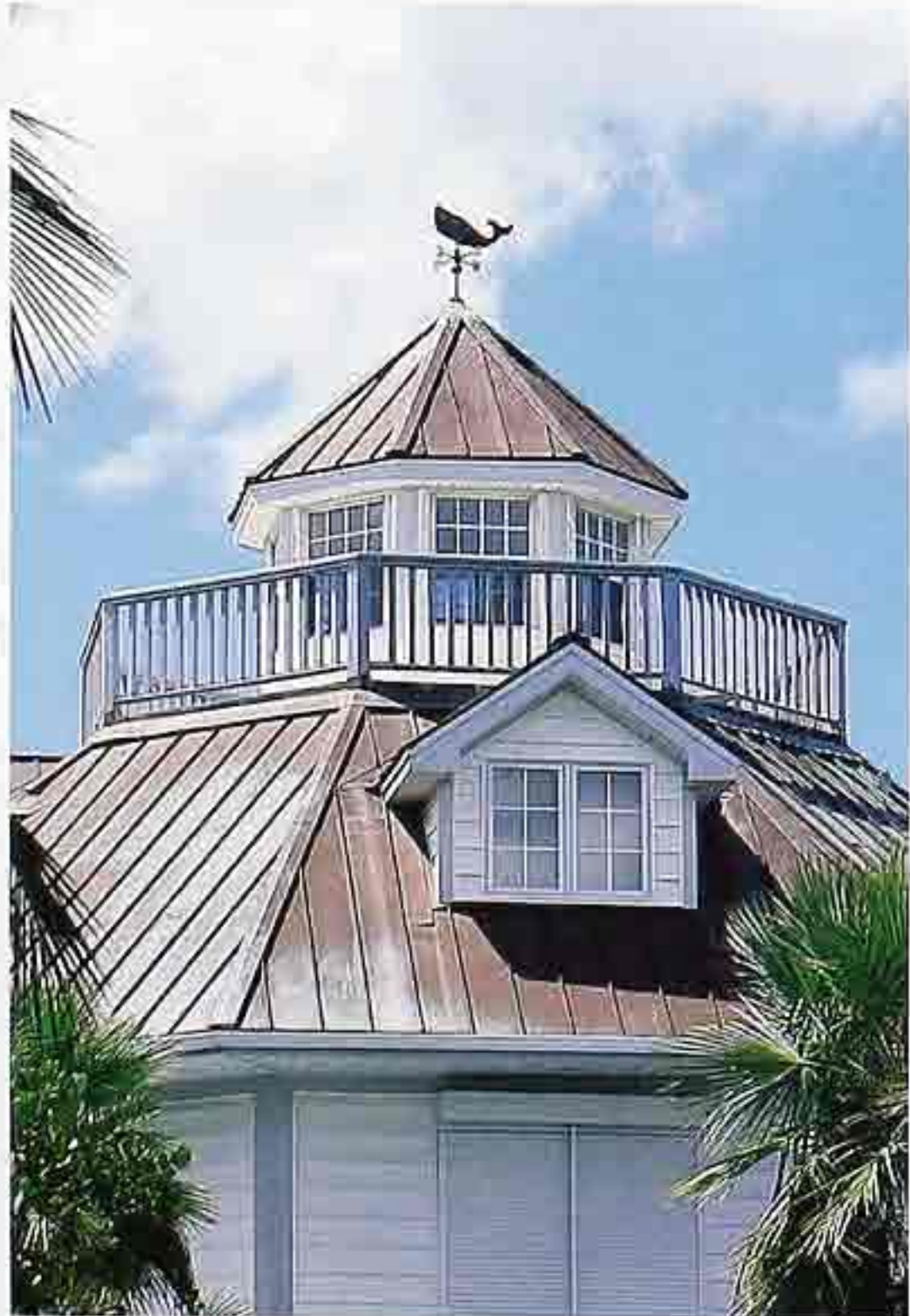
CR-128 Octagonal painted standing-seam metal roof with widow's walk and gabled roof dormer
