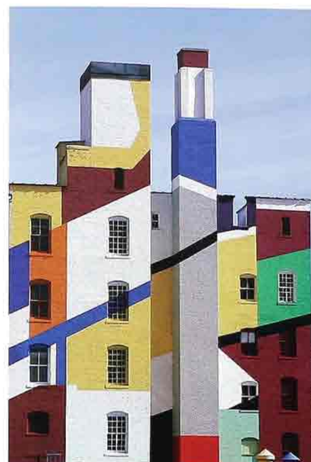
FA-88 Painted geometric pattern on brick facade of industrial building (paint manufacturer)
