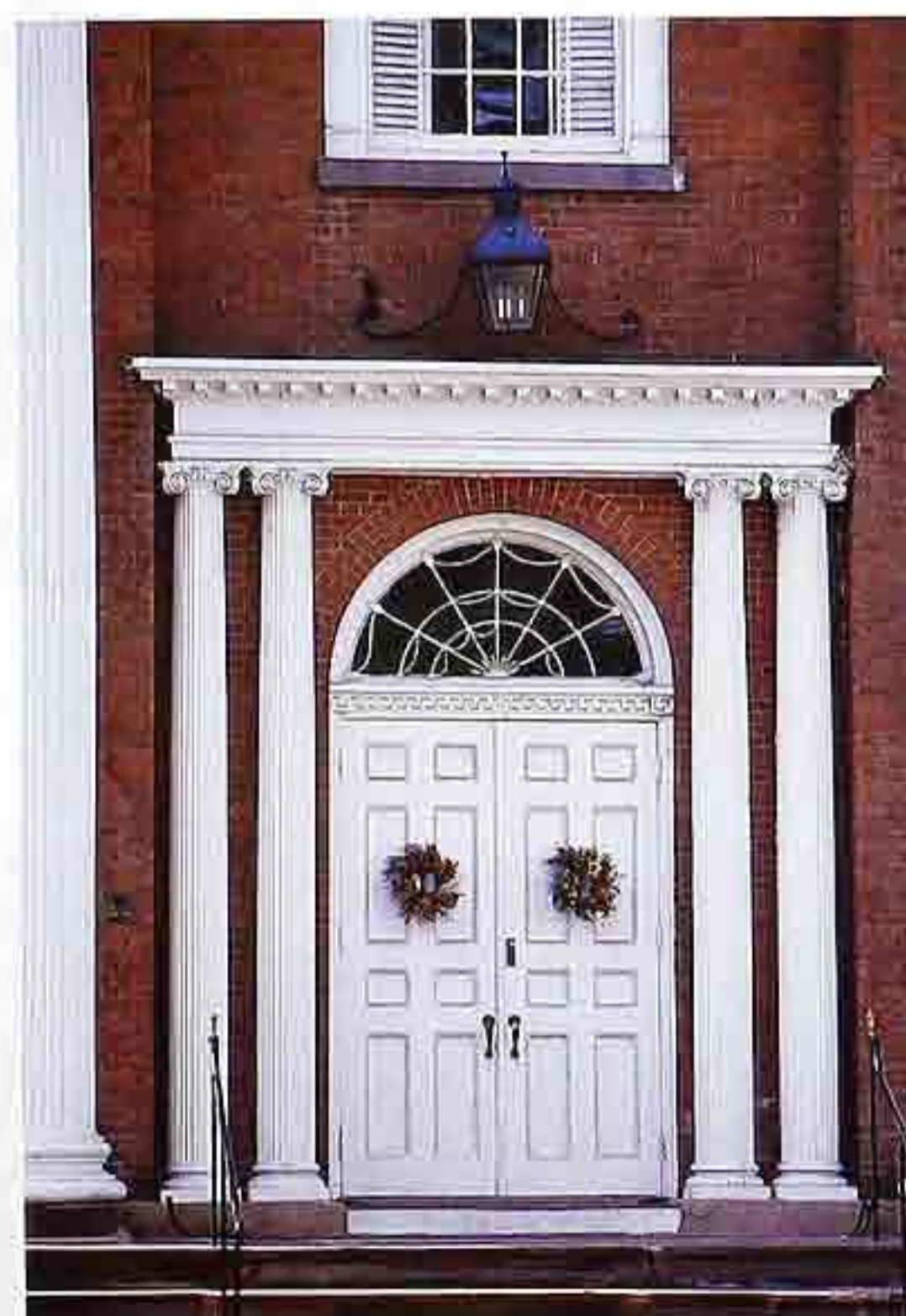
DW-74 Neoclassical entry with pairs of Ionic engaged columns supporting dentil entablature, eight-paneled double doors, bat-wing fanlight
