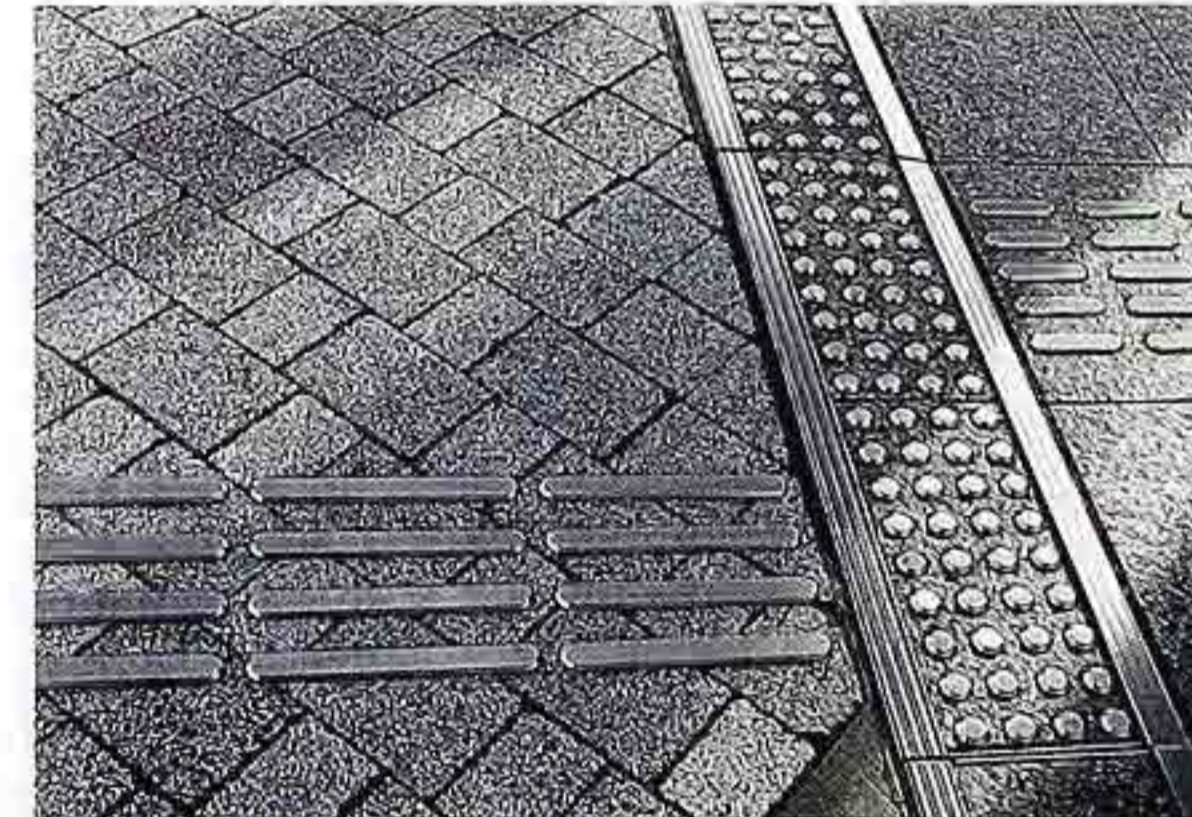
FP-109 Metal safety-paving brads and strips applied to granite pavers, urban public space
