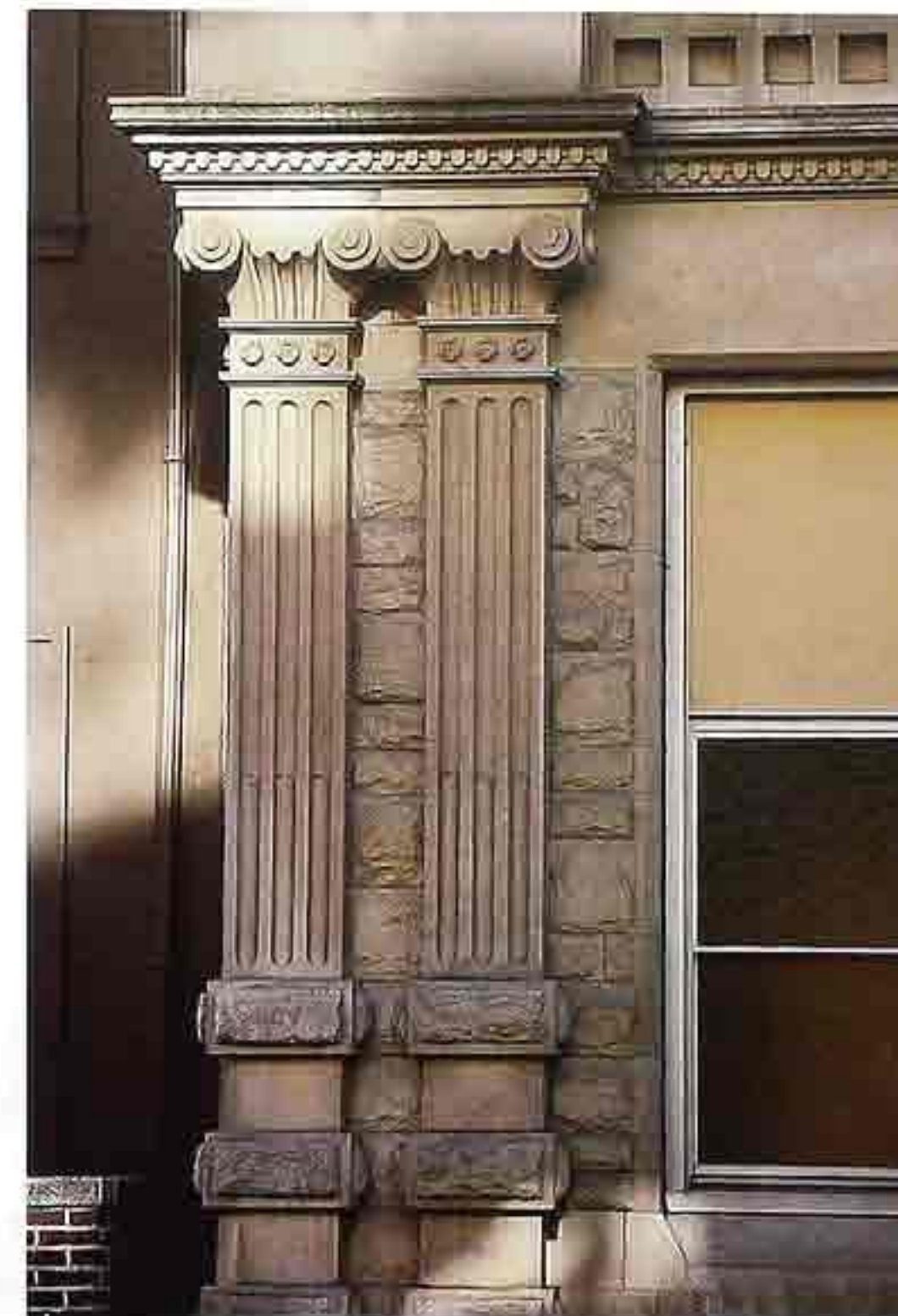
CP-84 Stone pilasters with flutes and banded rusticated bases
