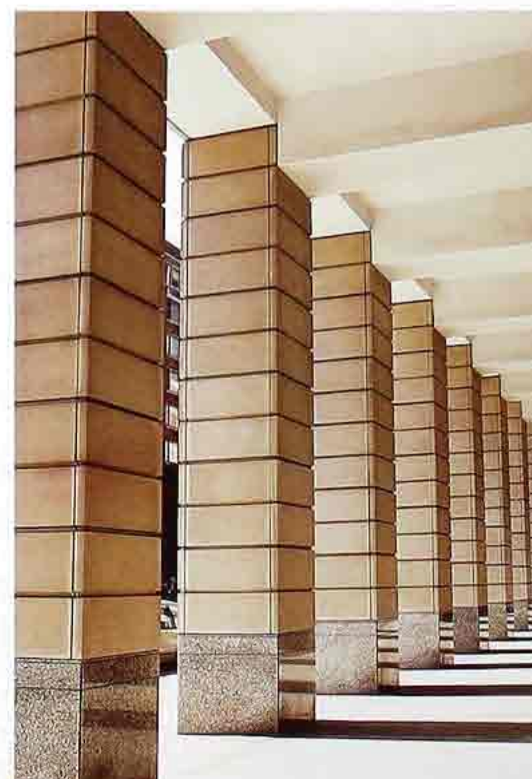
CP-136 Polished rusticated granite-veneer piers with adjoining boxed beams in arcade, modern commercial building
