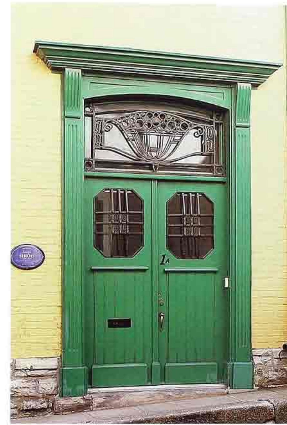
DW-69 Paneled double doors with octagonal lights with leaded glass transom in cambered arch; letter slot; fluted pilasters; crown molding
