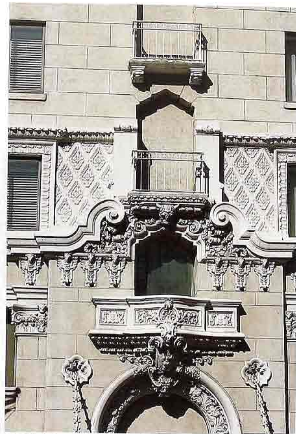
FA-113 Balconies over portal, broken pediment, and ornate details on multistory masonry facade
