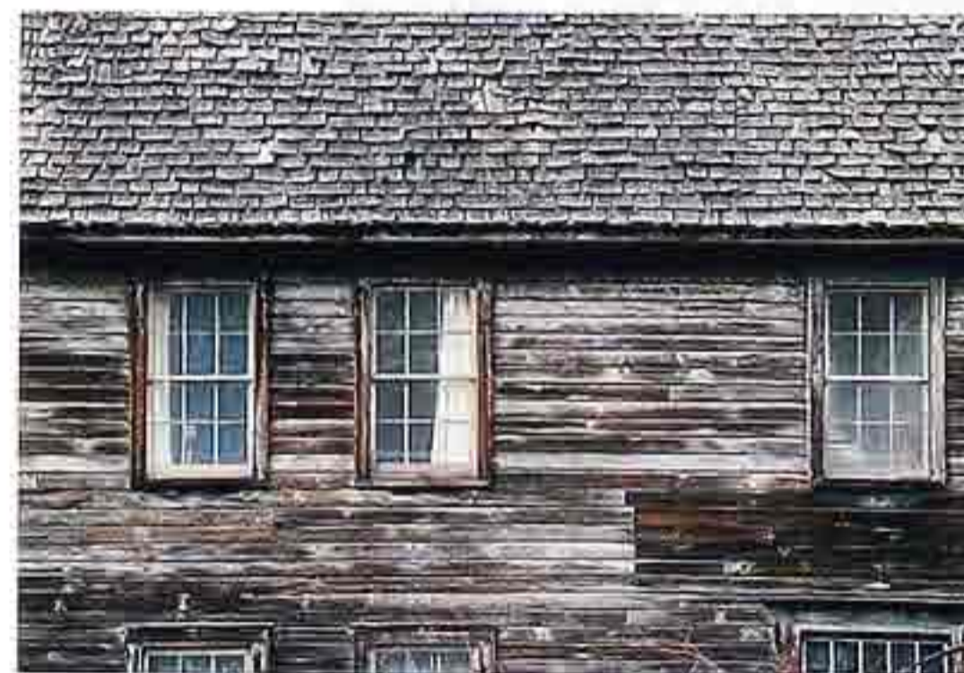
WA-24 Unpainted clapboard showing evidence of repair, with double-hung windows, American colonial house
