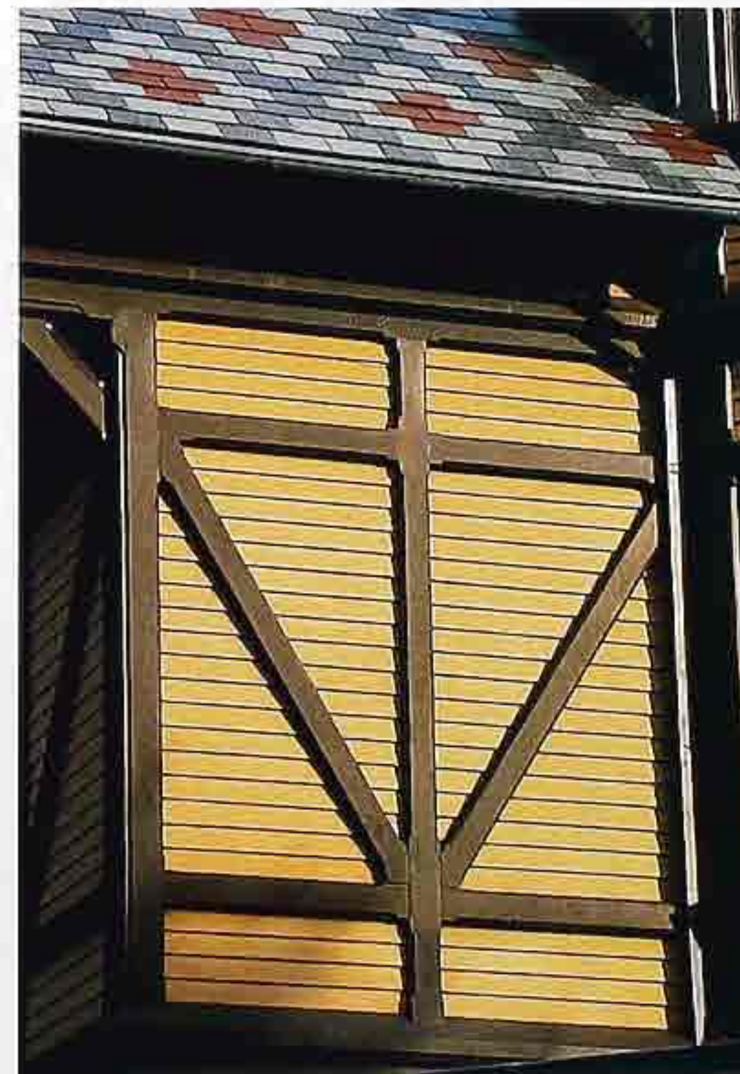
WA-42 Stylized half-timber wall with decorative framing over clapboard infill
