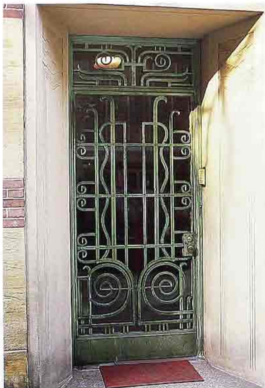
DW-114 Wrought-iron gate recessed in wall
