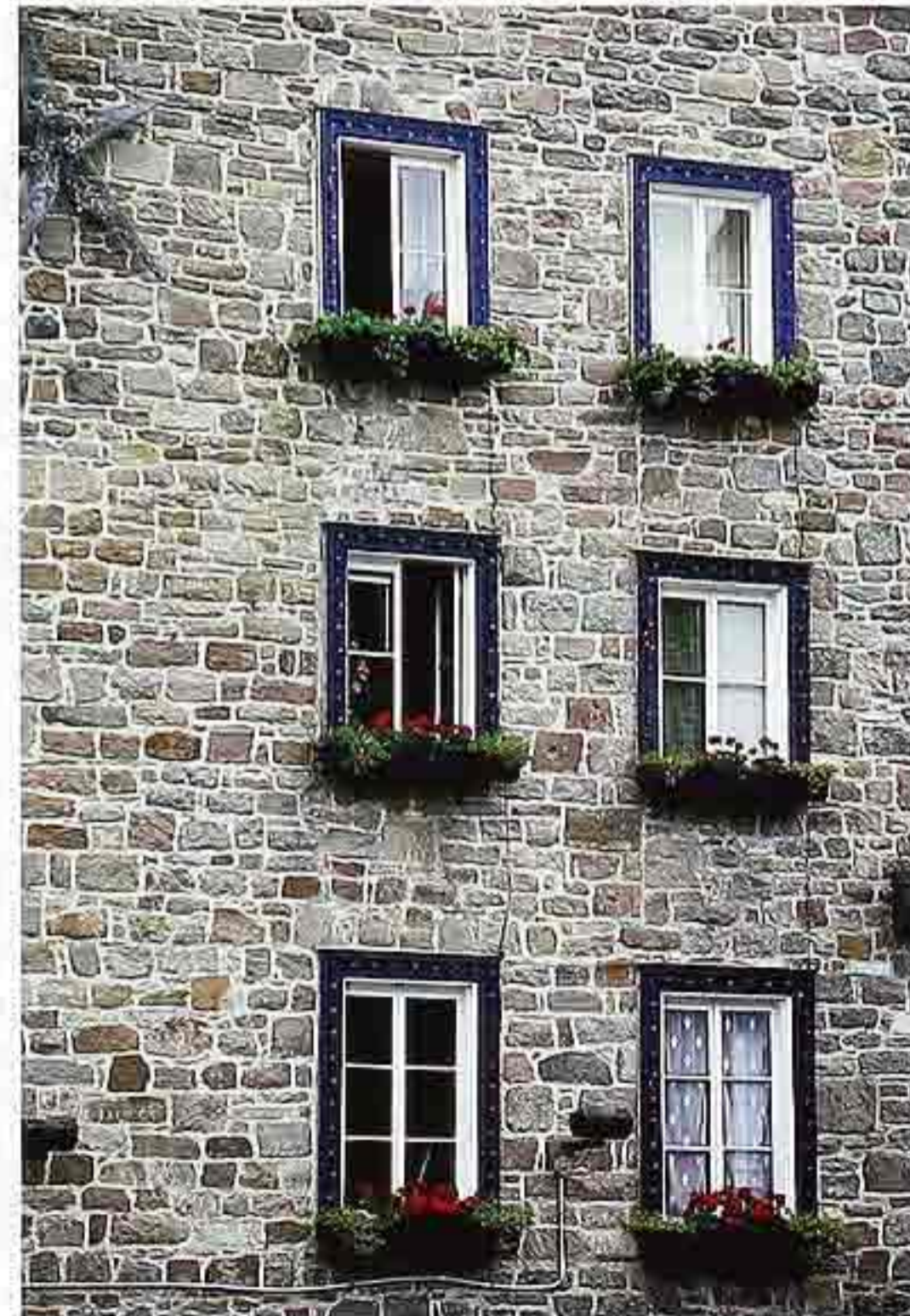
WI-33 Two- and three-light double-casement windows
