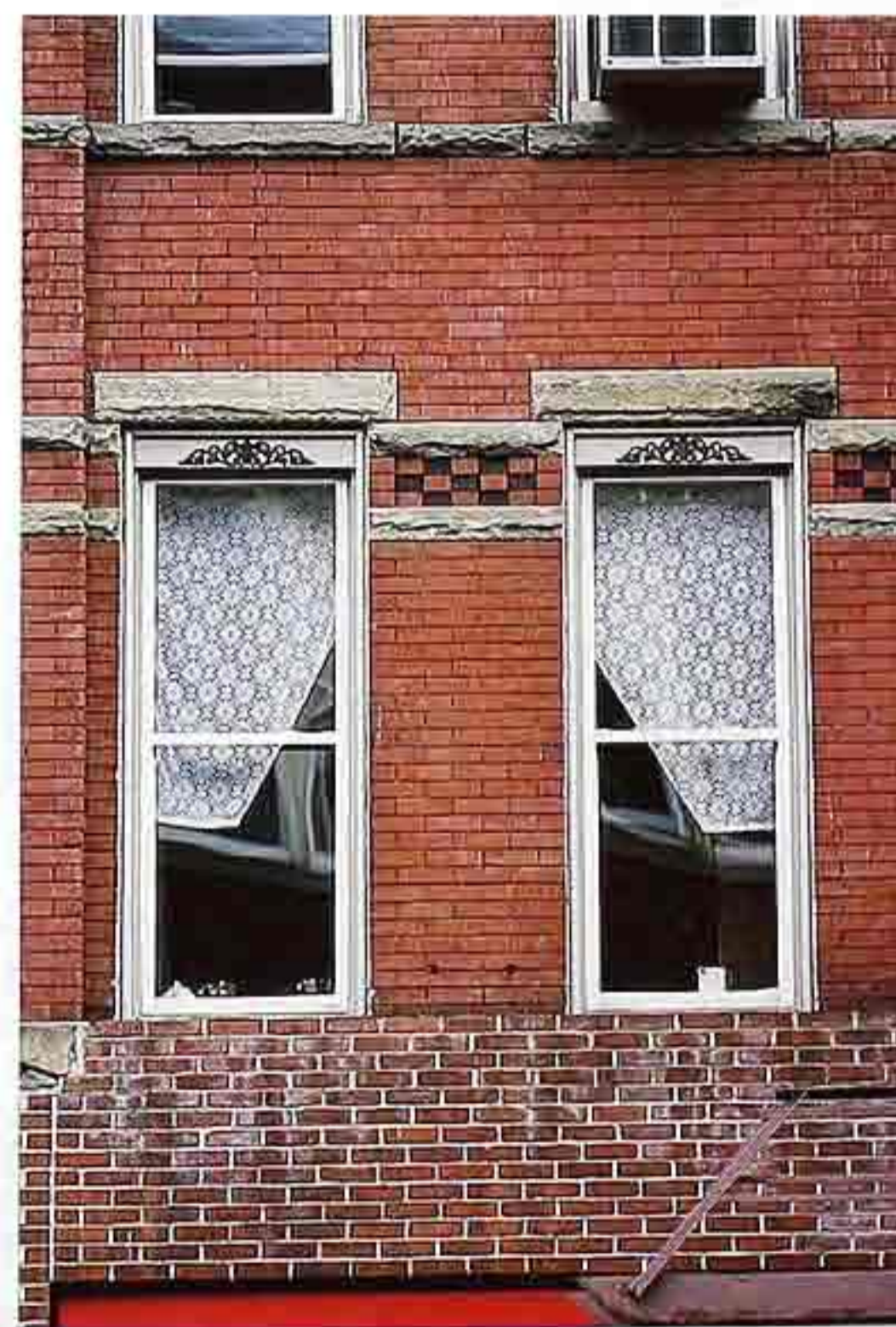
WI-124 Stone lintels and carved casing tops with stone and brickwork band around double-hung windows in brick wall
