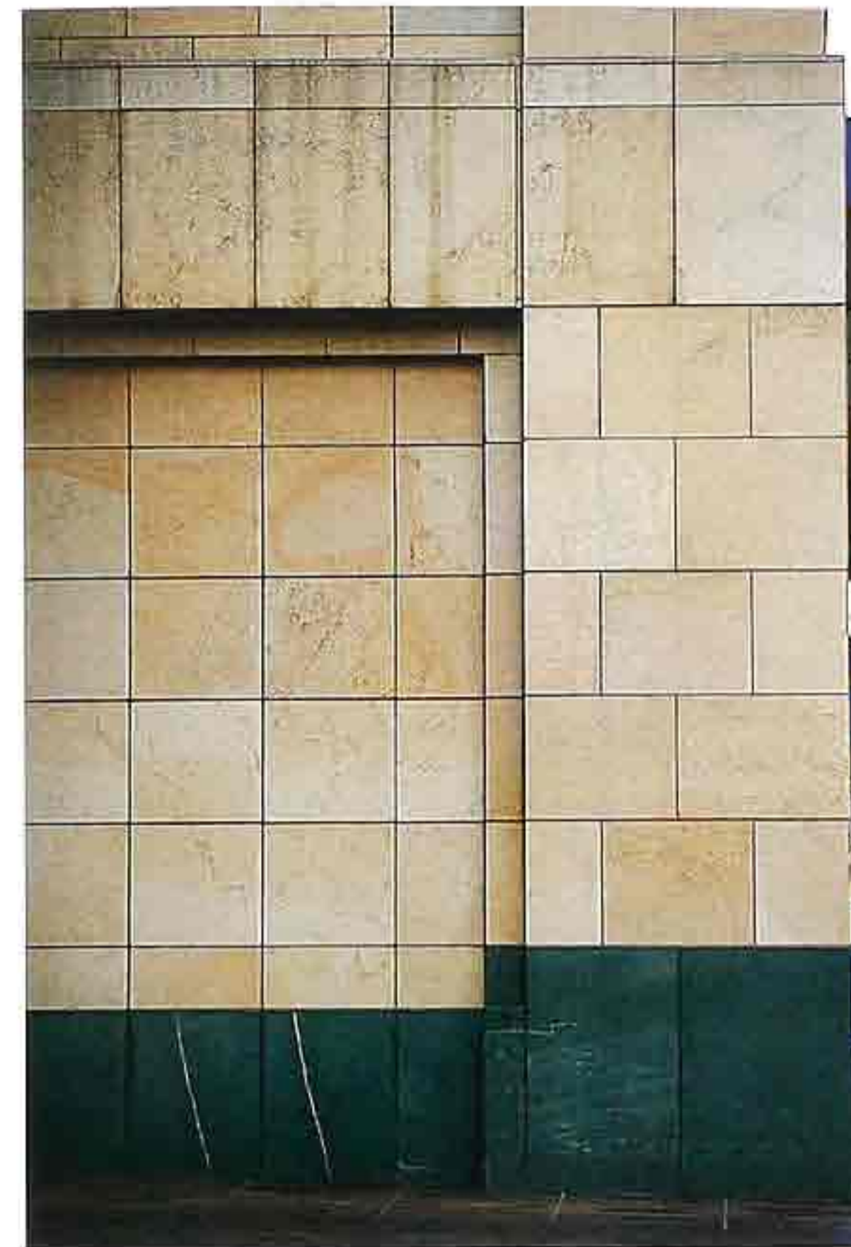
WA-142 Sandstone coursed-ashlar frame with stack-bond inset, flush marble-veneer base, modern commercial building
