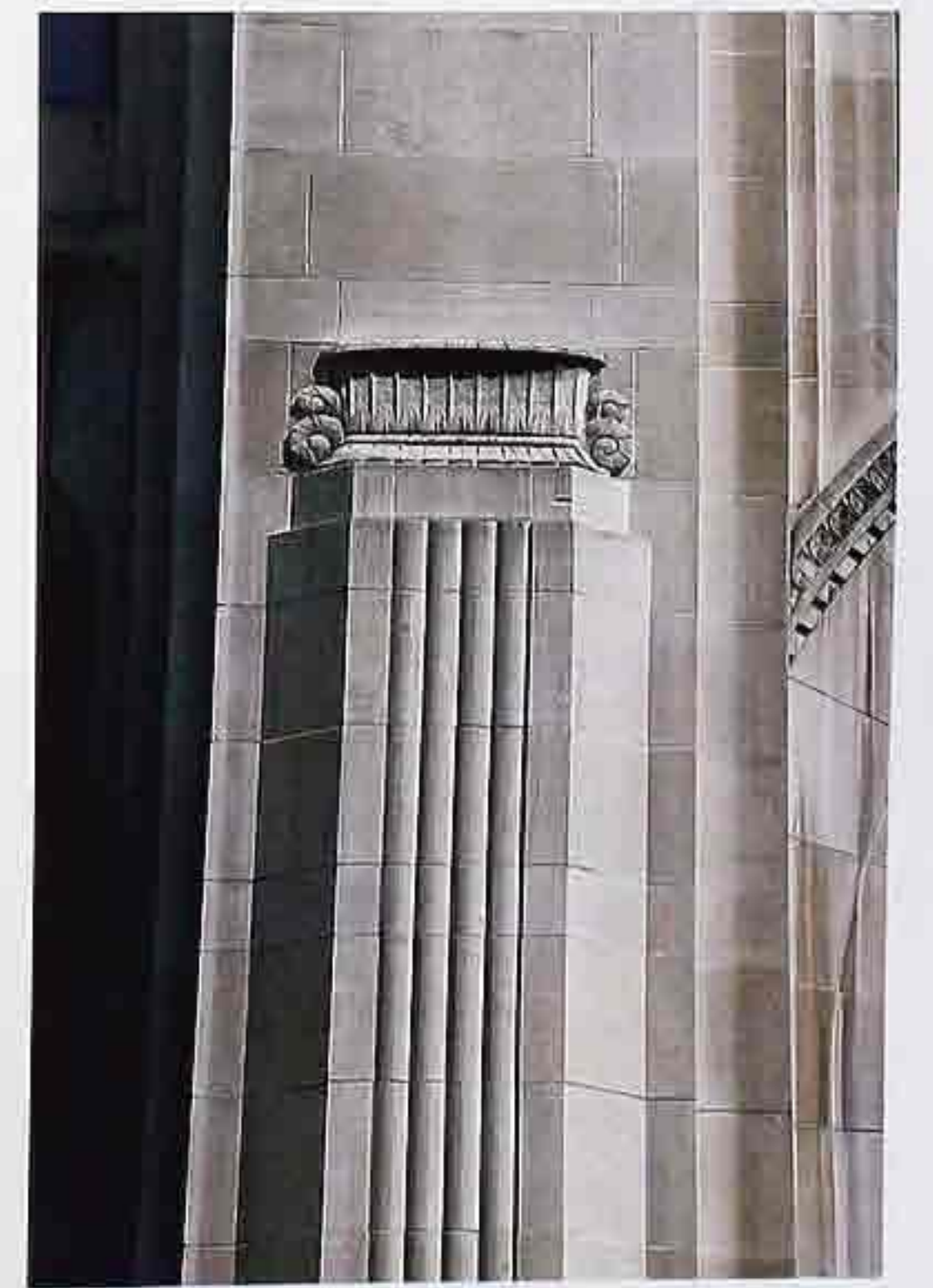
CP-87 Pilaster with trapezoidal profile, cabled, with a diminished capital resembling an Egyptian bell capital
