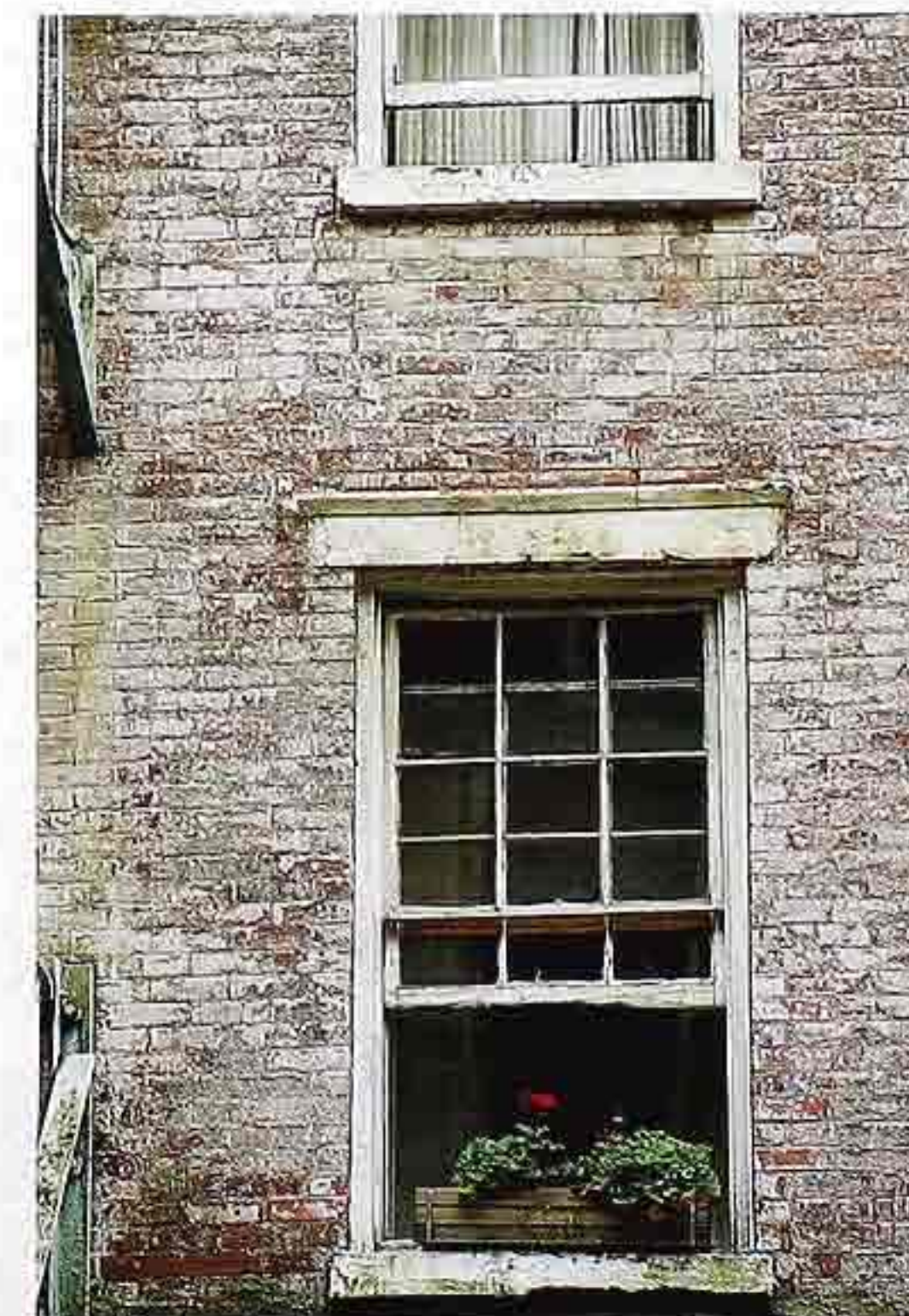
WI-46 Six-over-six double-hung window with stone lintel in weathered brick wall
