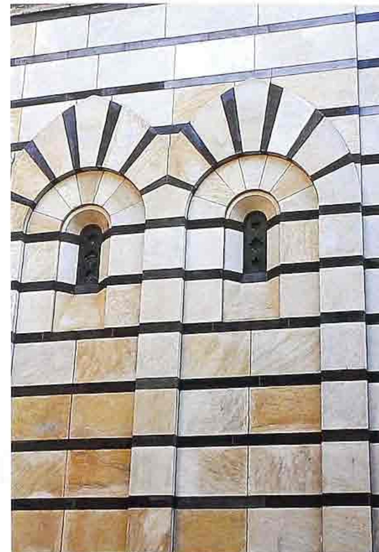
WA-120 Alternating polychrome bands of marble veneer in stack and running bonds with Moorish blind arches with recessed windows
