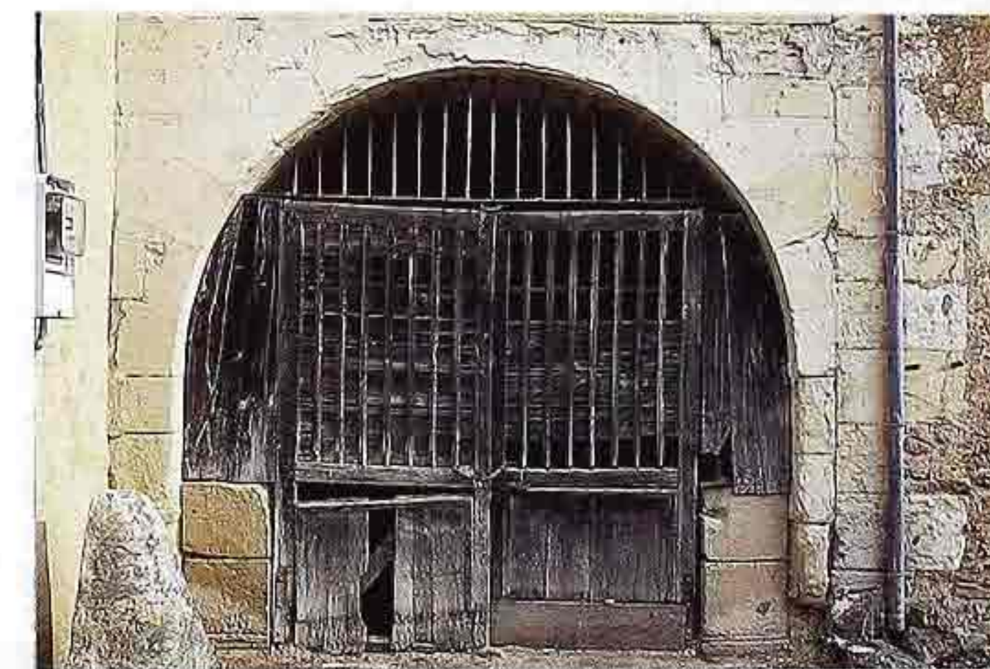
CP-160 Weathered stucco-covered stone semicircular arch with wood double doors, rustic courtyard
