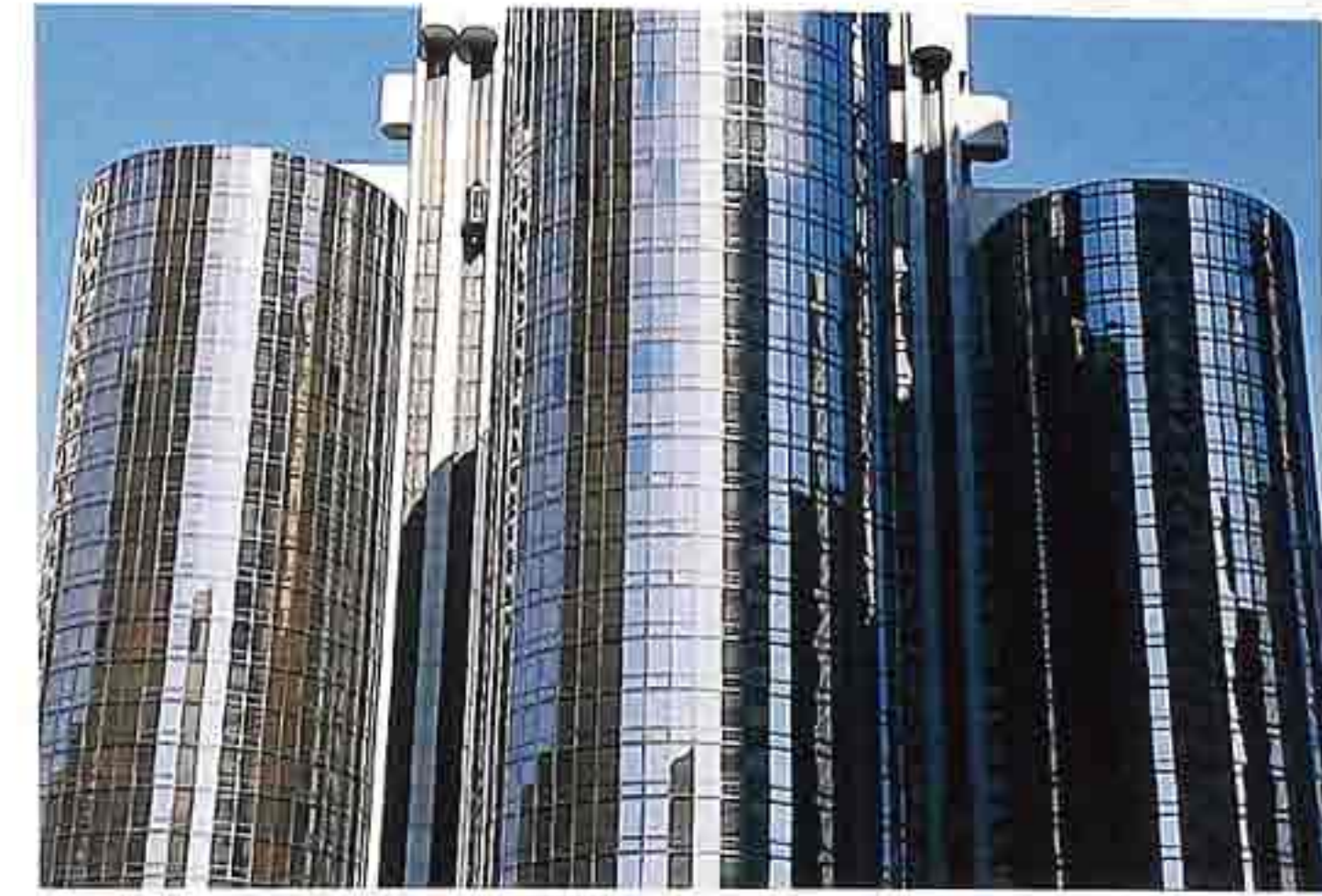
FA-29 Fully glazed curved curtain walls with mirror glass
