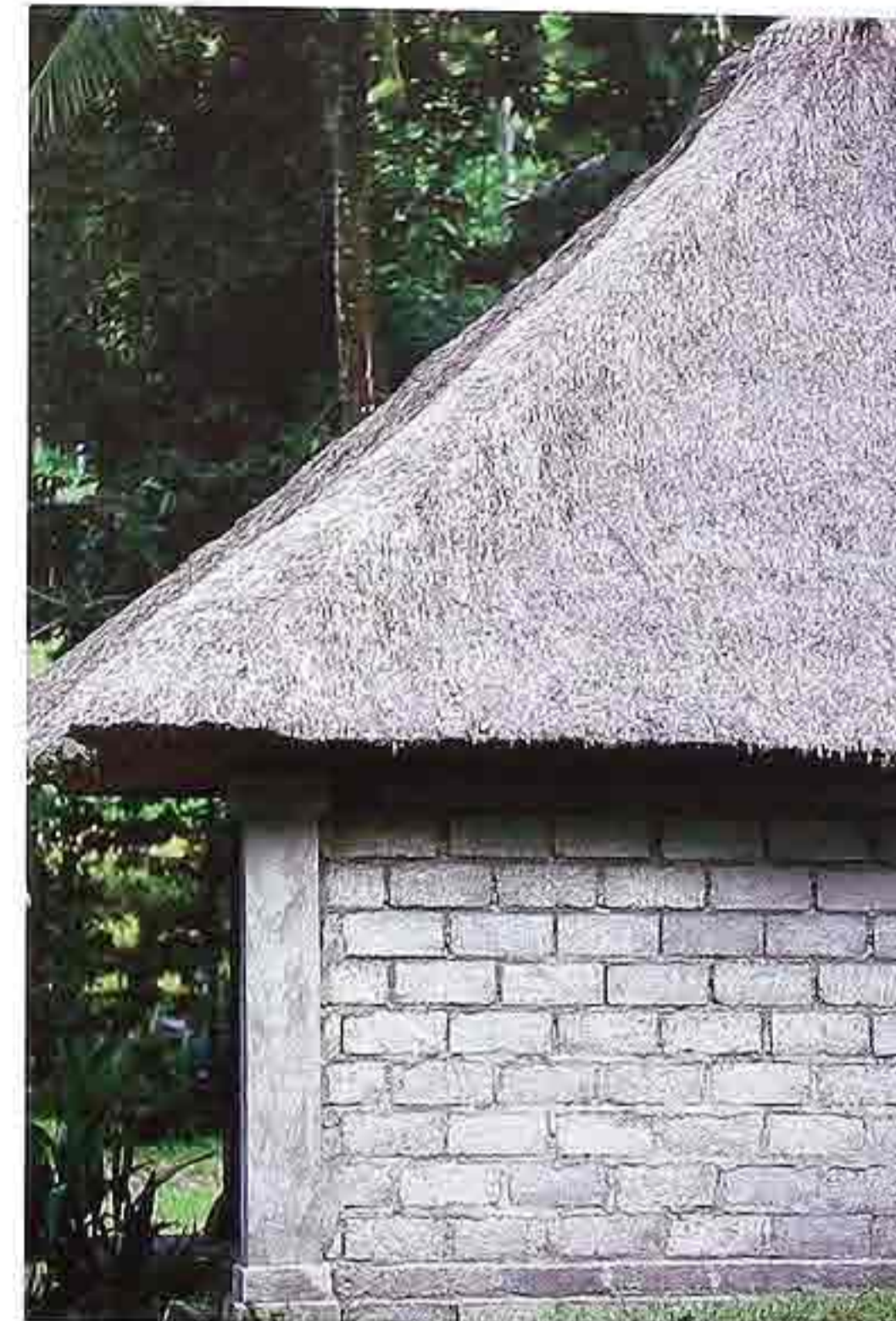
CR-70 Trimmed thatch on concrete-block building, Bali
