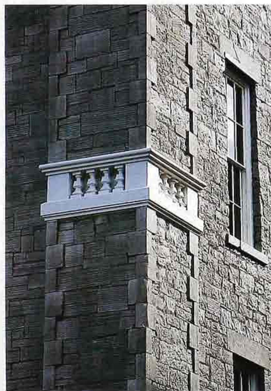
WA-99 Outside corner of split-faced, random ashlar with raised sand-finished quoins and engaged balustrade
