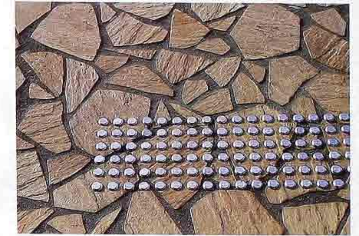
FP-108 Metal safety-paving brads on flagstone set in concrete, urban public space
