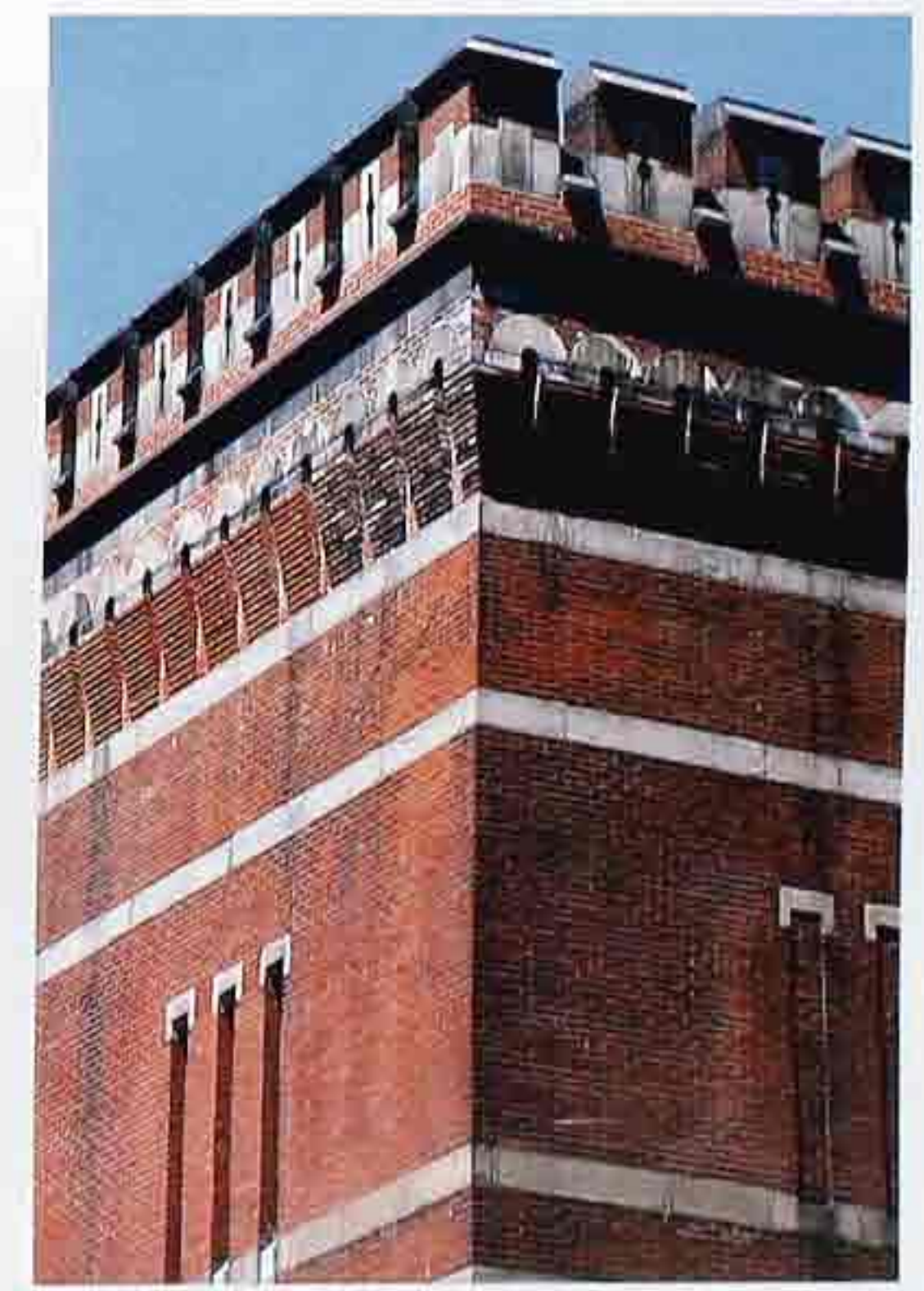
WA-196 Corner detail of Romanesque-style brick building with stone banding, parapet roof with crenellation
