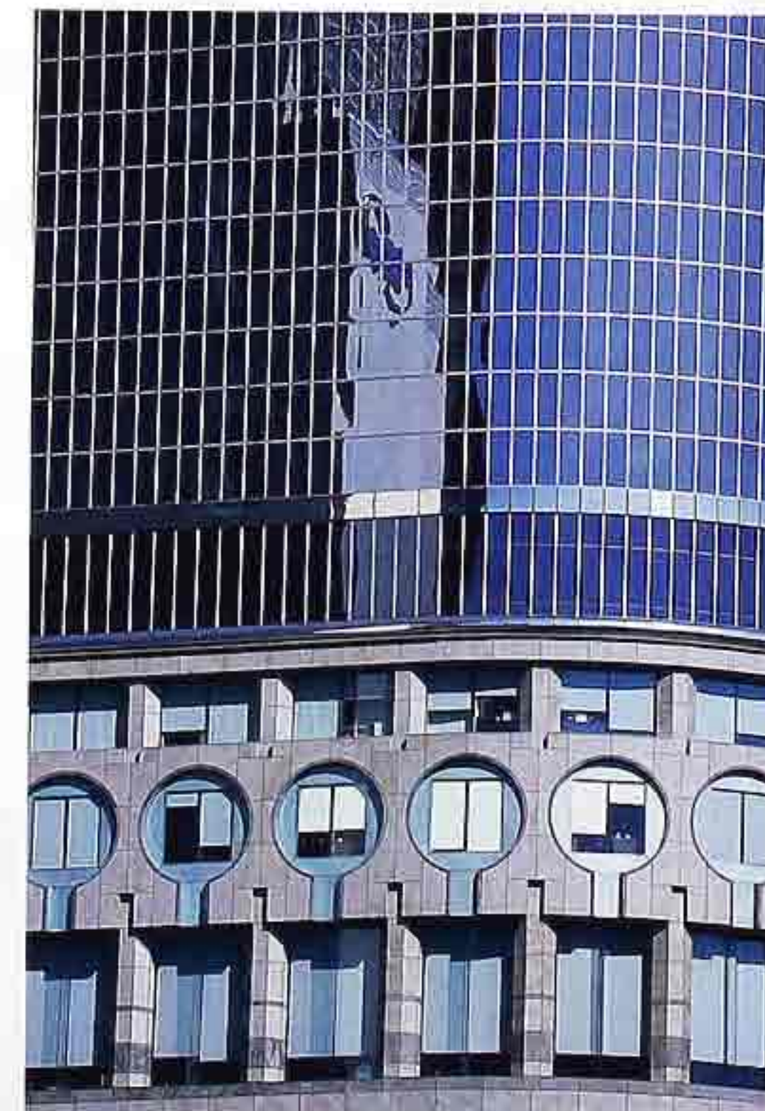
FA-126 Curving glass curtain wall above stone-veneer facade with expressed piers and keyhole window surrounds, modern commercial building
