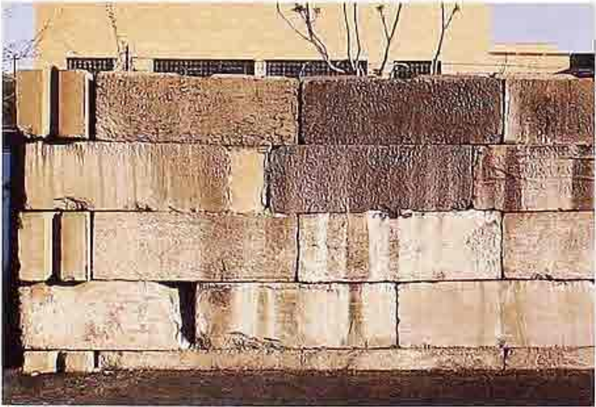
WA-223 Concrete-block dry wall in irregular running bond, industrial wall
