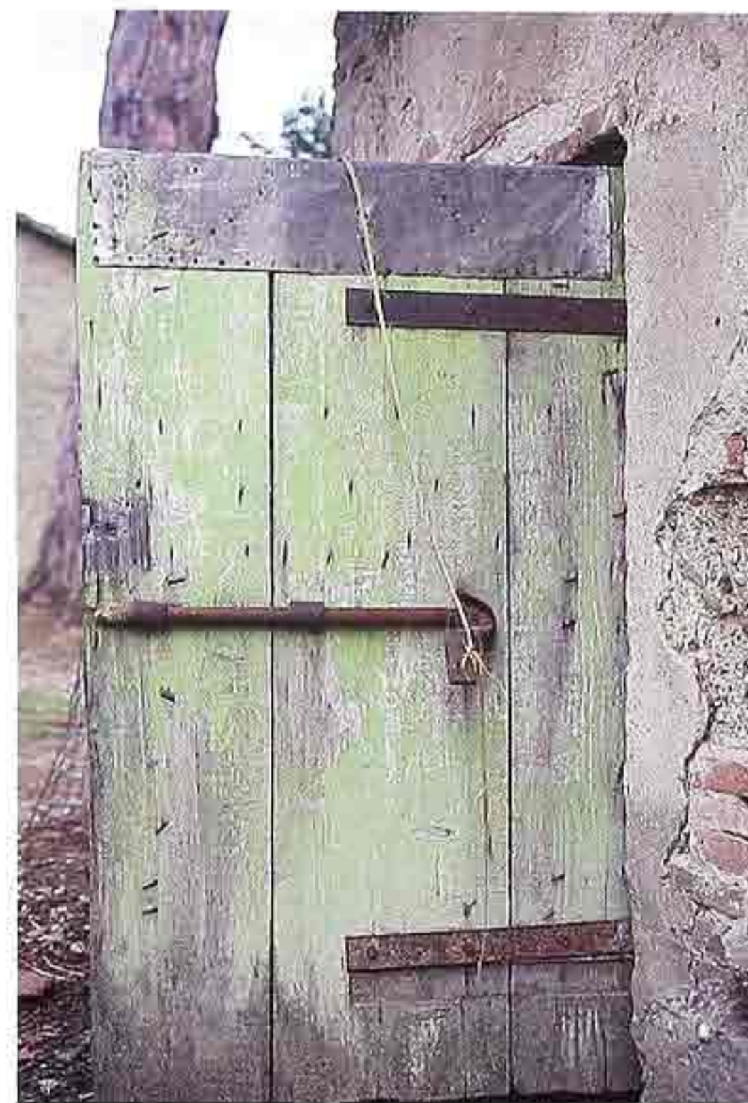
DW-33 Weathered painted wood-plank door with rustic iron strap hinges and latch, farm courtyard
