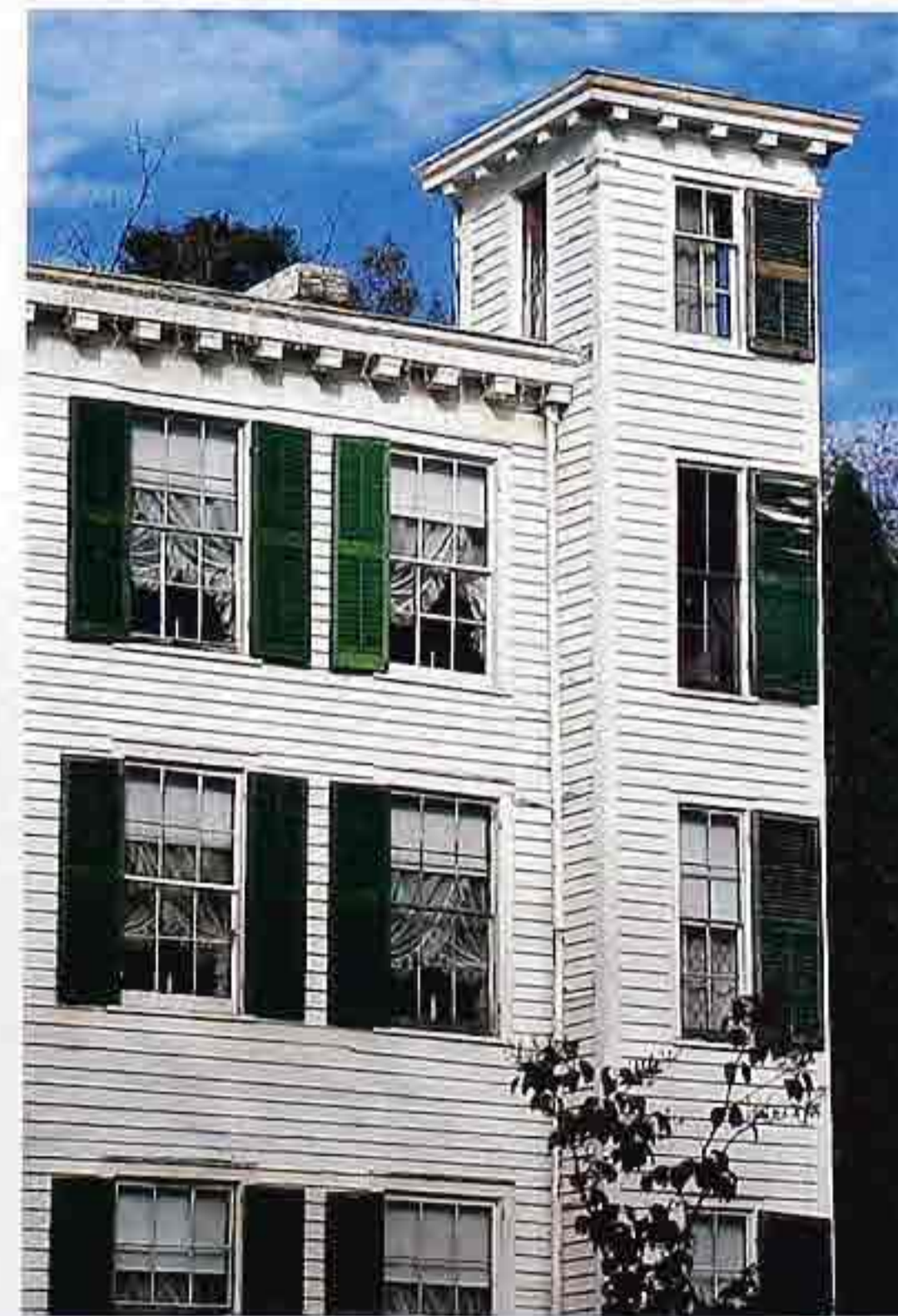
WA-34 Painted clapboard and block modillion cornice on corner tower, Italianate house
