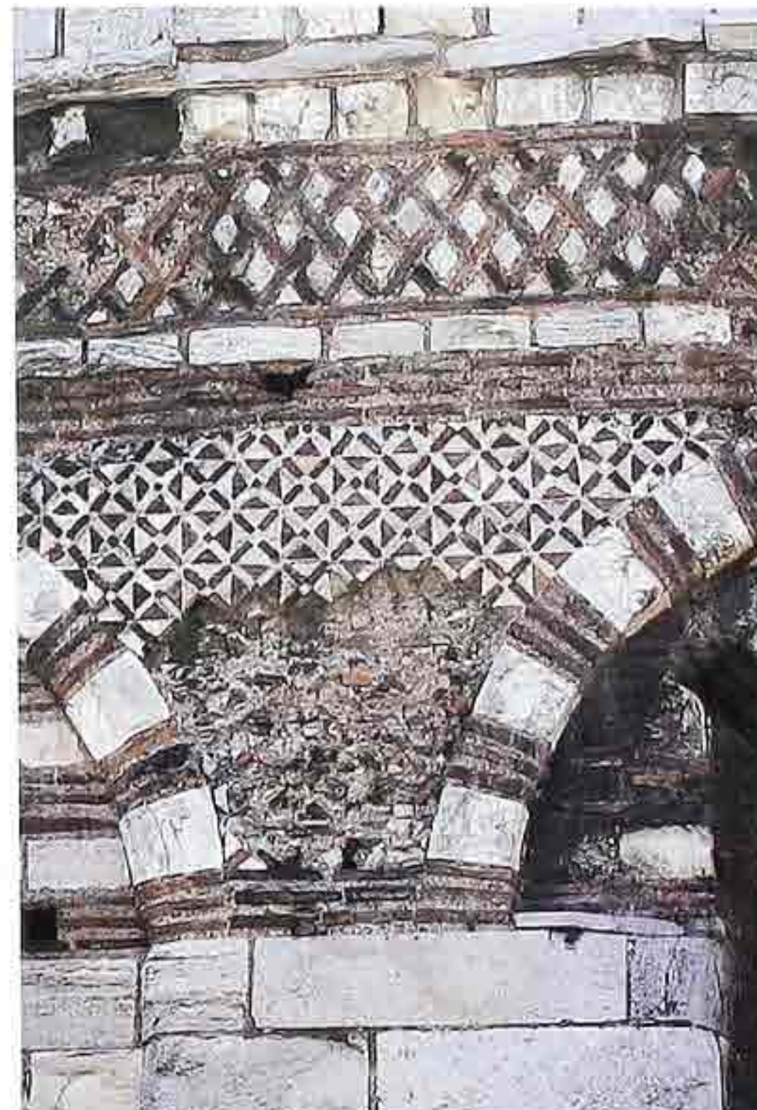
WA-286 Ancient arcade. Top to bottom: roughly squared stone; diaper brickwork; courses of stone and Roman brick, weathered tile with substructure, brick-and-stone arches; coursed-ashlar stone
