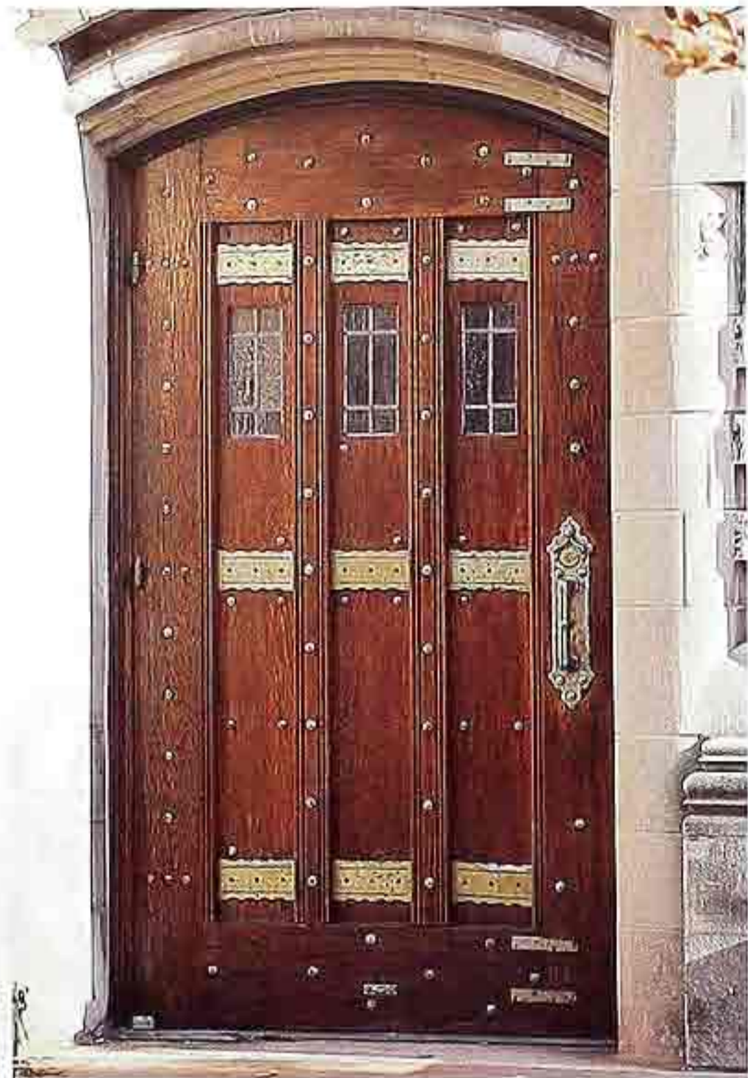
DW-1 Three narrow panels, wood, with leaded lights, brass handle, decorative plates and studs on stiles, panels, and rails; segmental-arch doorway
