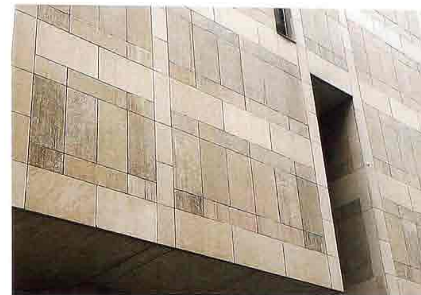
WA-135 Limestone-veer panels framed by contrasting stack-and-running-bond courses, modern commercial building
