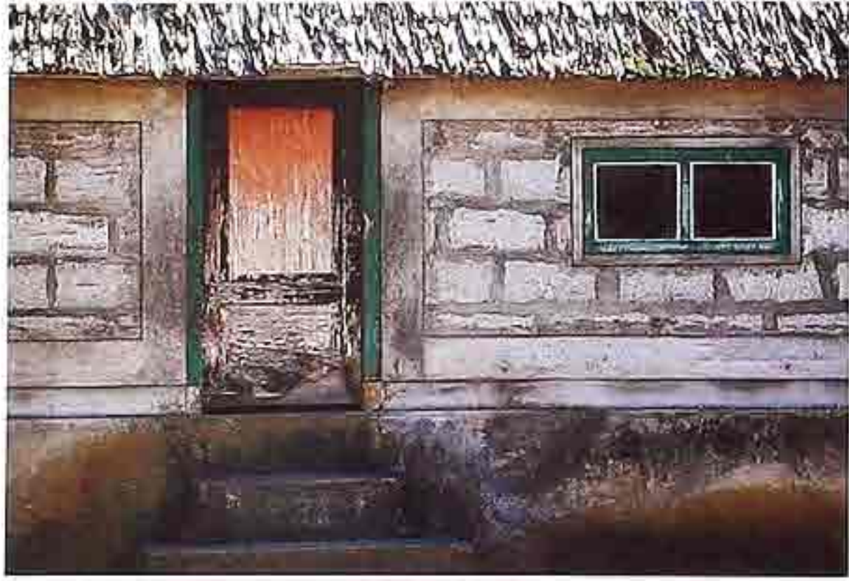
WA-221 Weathered handmade concrete block with mortar in irregular running bond on house
