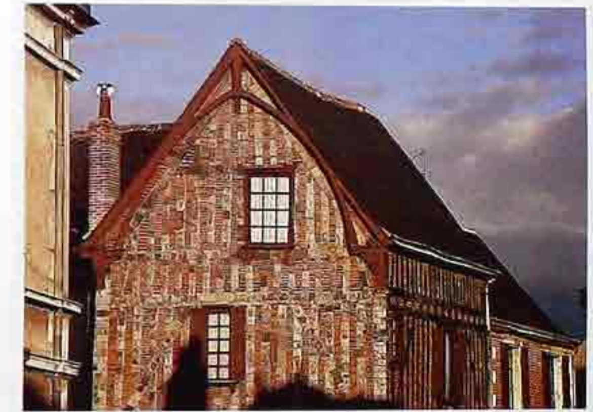
CR-123 Half-timbered gable, with surface arch
