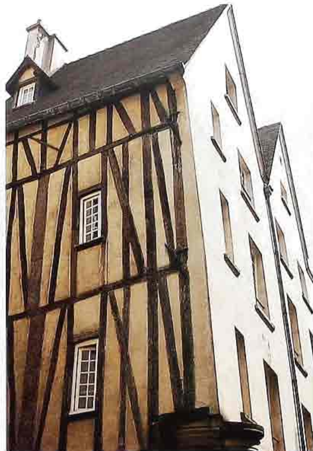
WA-283 Half-timber with stucco infill, 15th- or 16th-c. French house
