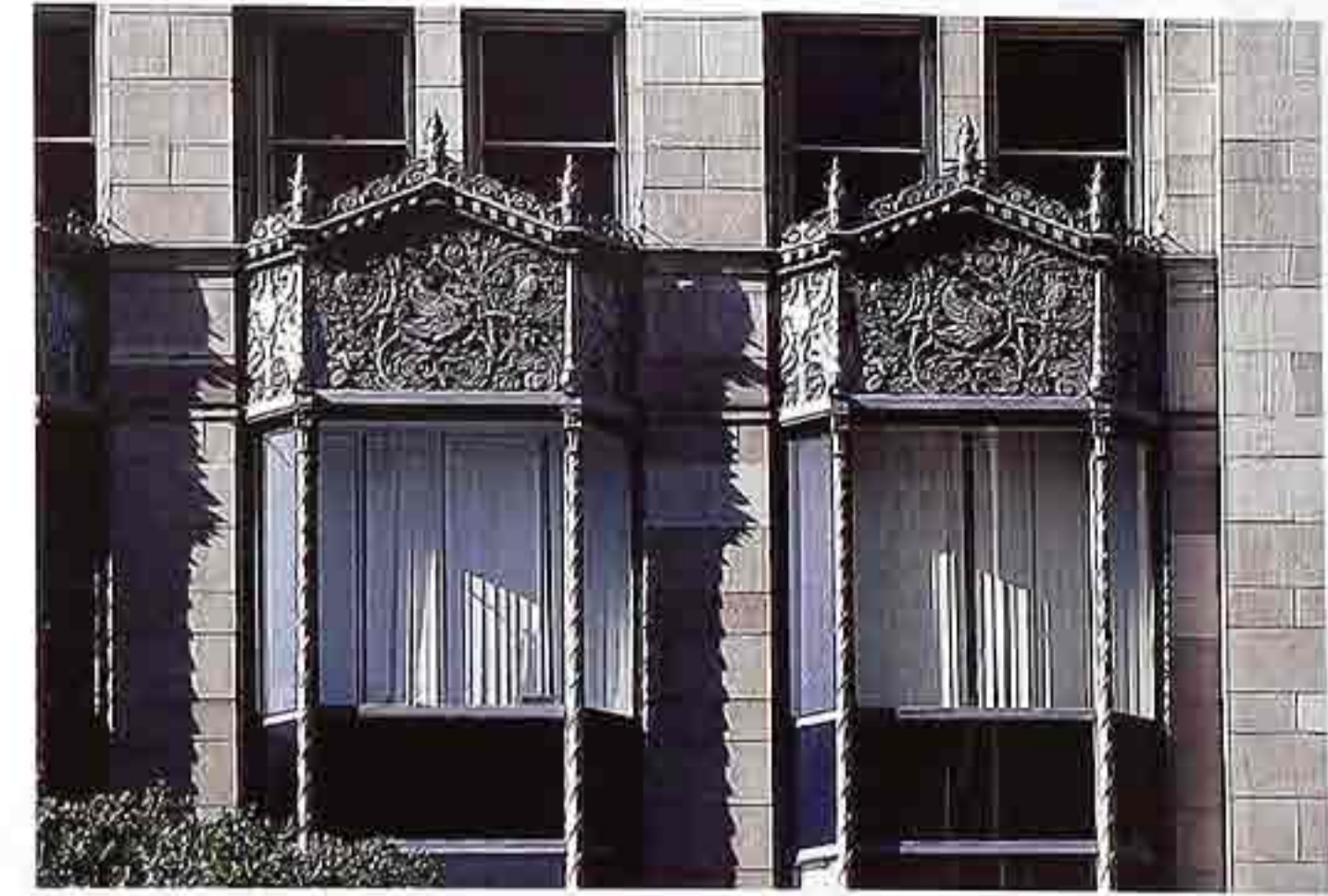
WI-83 Two-story cant-bay windows: fixed lights below ornamental cast or pressed metalwork, apartment house
