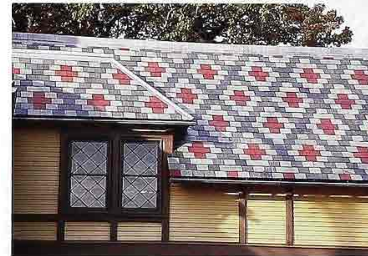
CR-60 Rectangular slate roofing in polychrome diaper pattern
