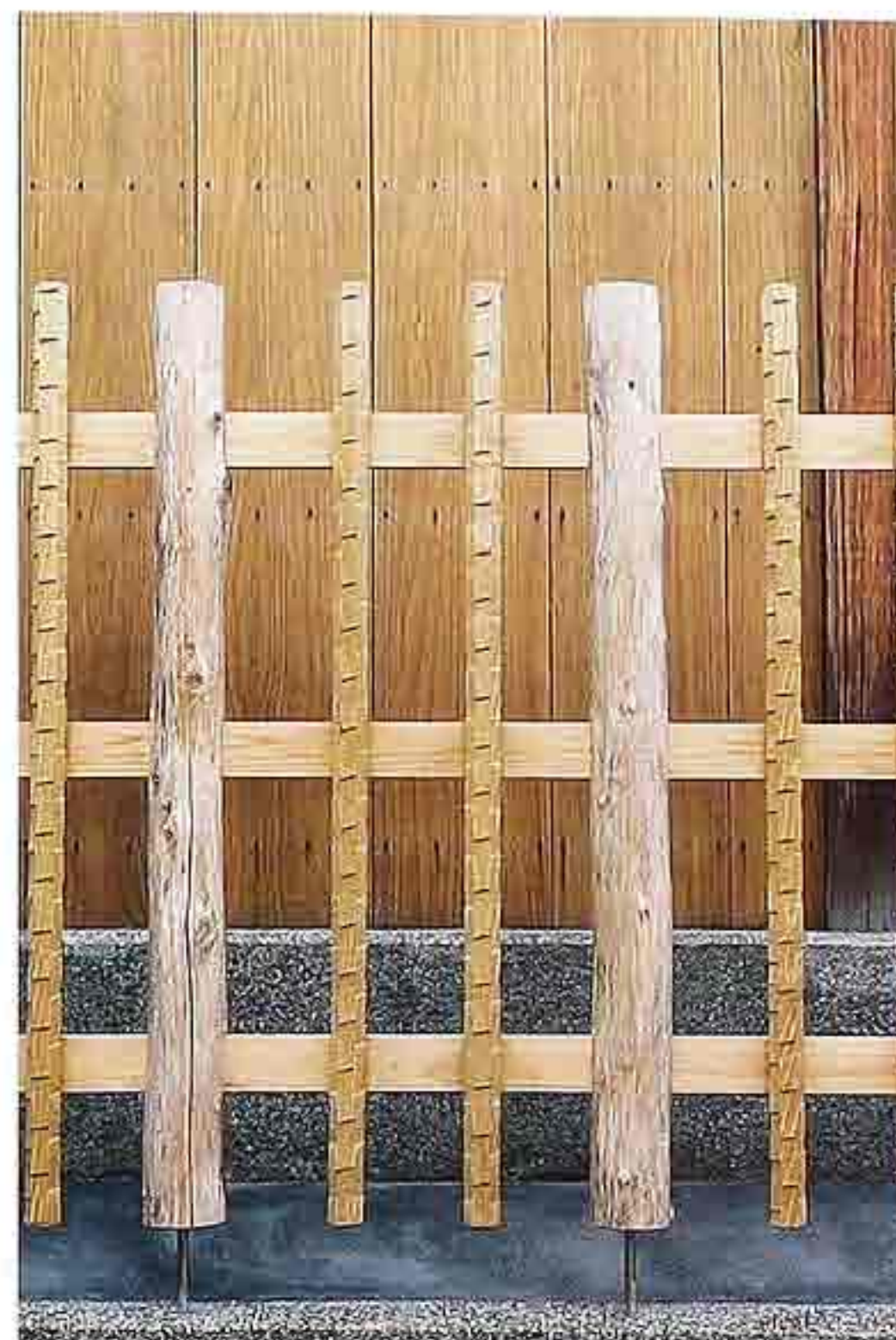
DW-110 Unfinished-wood entry gate of alternating notched square stock and roughly dressed timber posts attached to horizontal battens
