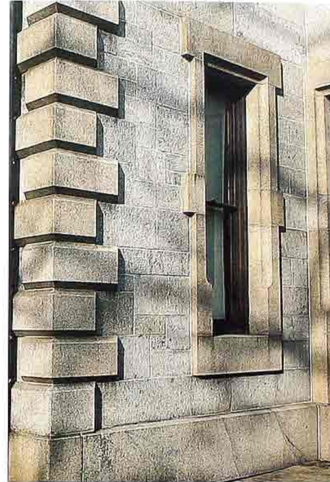
WA-93 Sawn granite in random ashlar with tooled quoins; flat granite window and base trim
