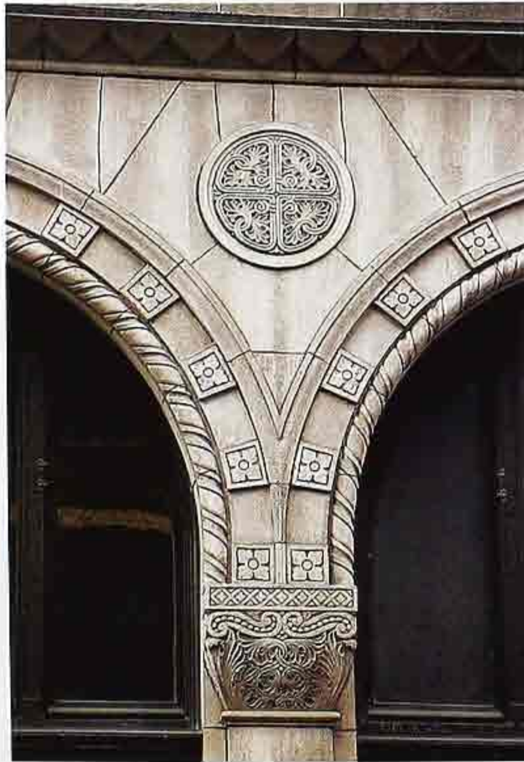
CP-148 Arcade of semicircular arches, rope molding in intrados, square panel rosettes, and quatrefoil medallion in spandrel
