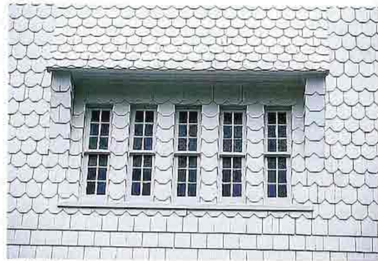
FA-48 Painted sawn shingles in fish-scale pattern on shed dormer
