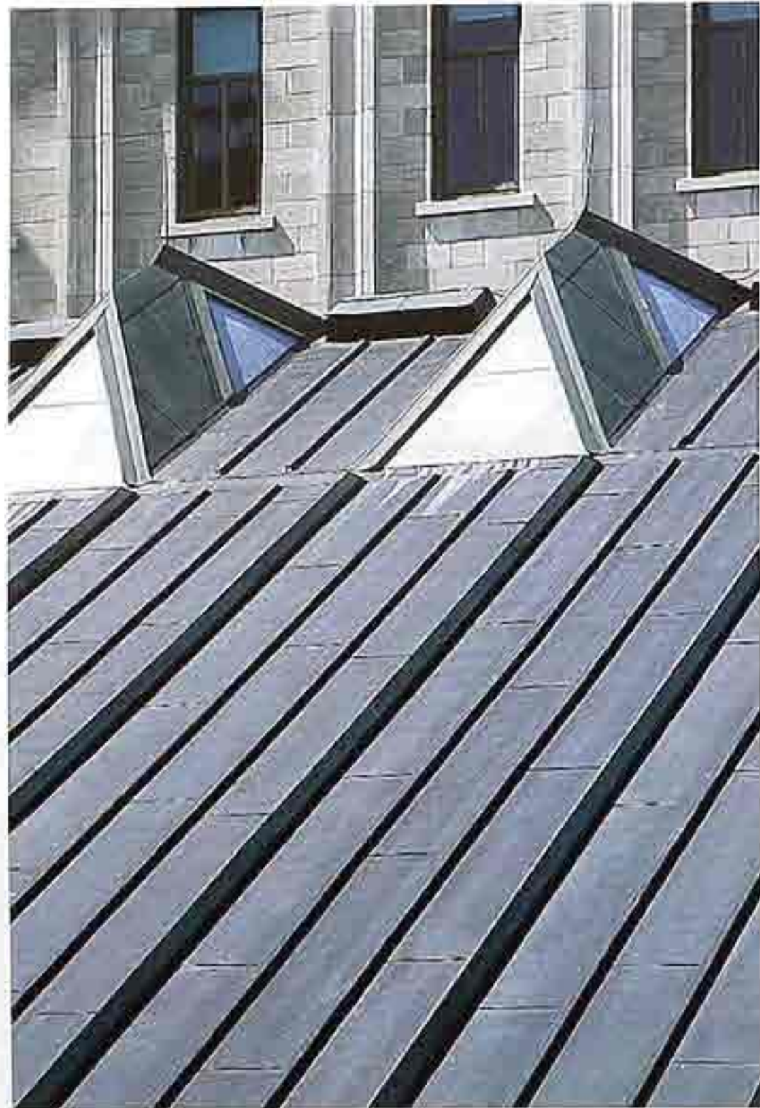
CR-21 Anodized aluminum or coated sheet steel with batten seams, modern commercial building
