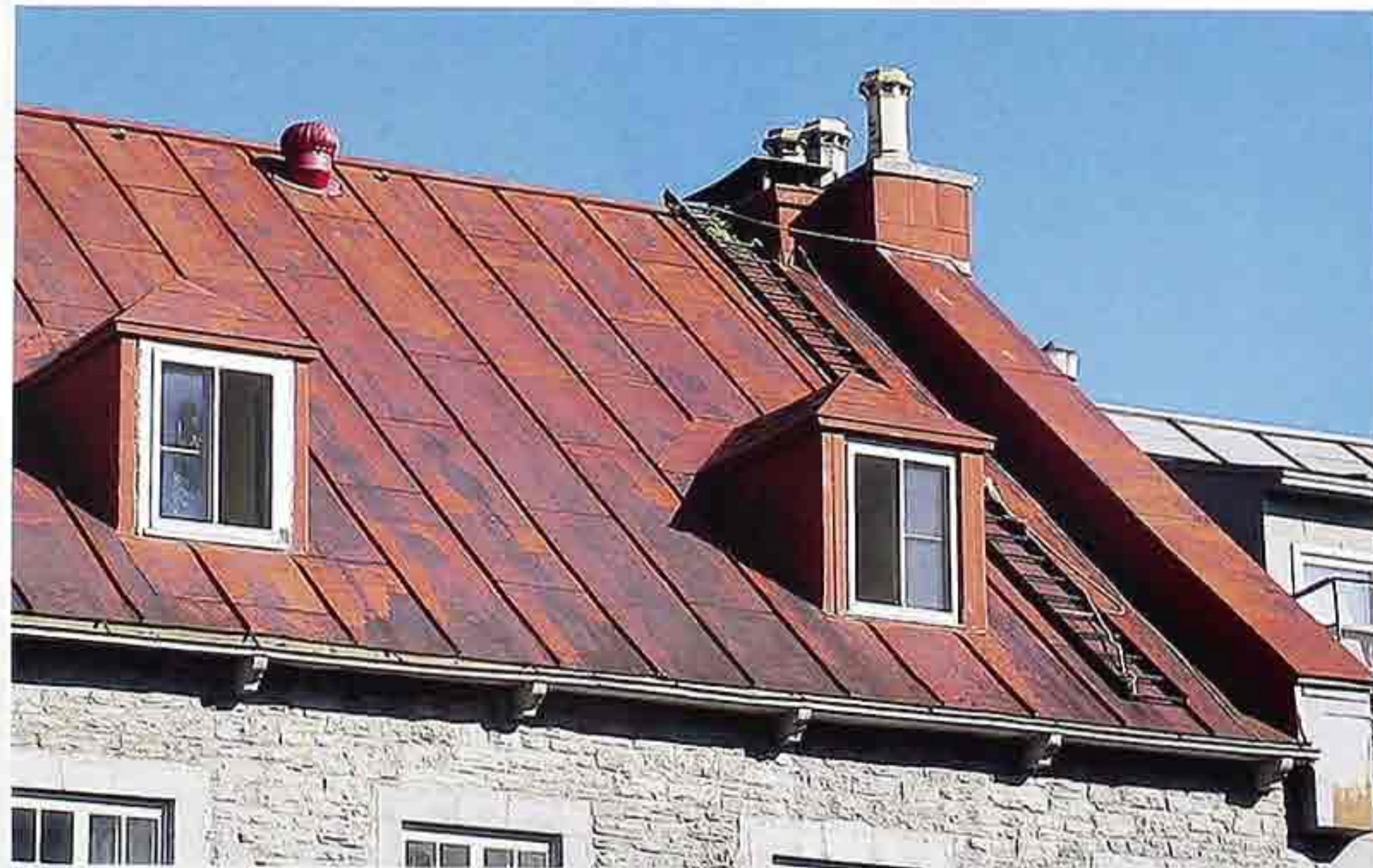
CR-39 Standing seams with hipped roof dormers
