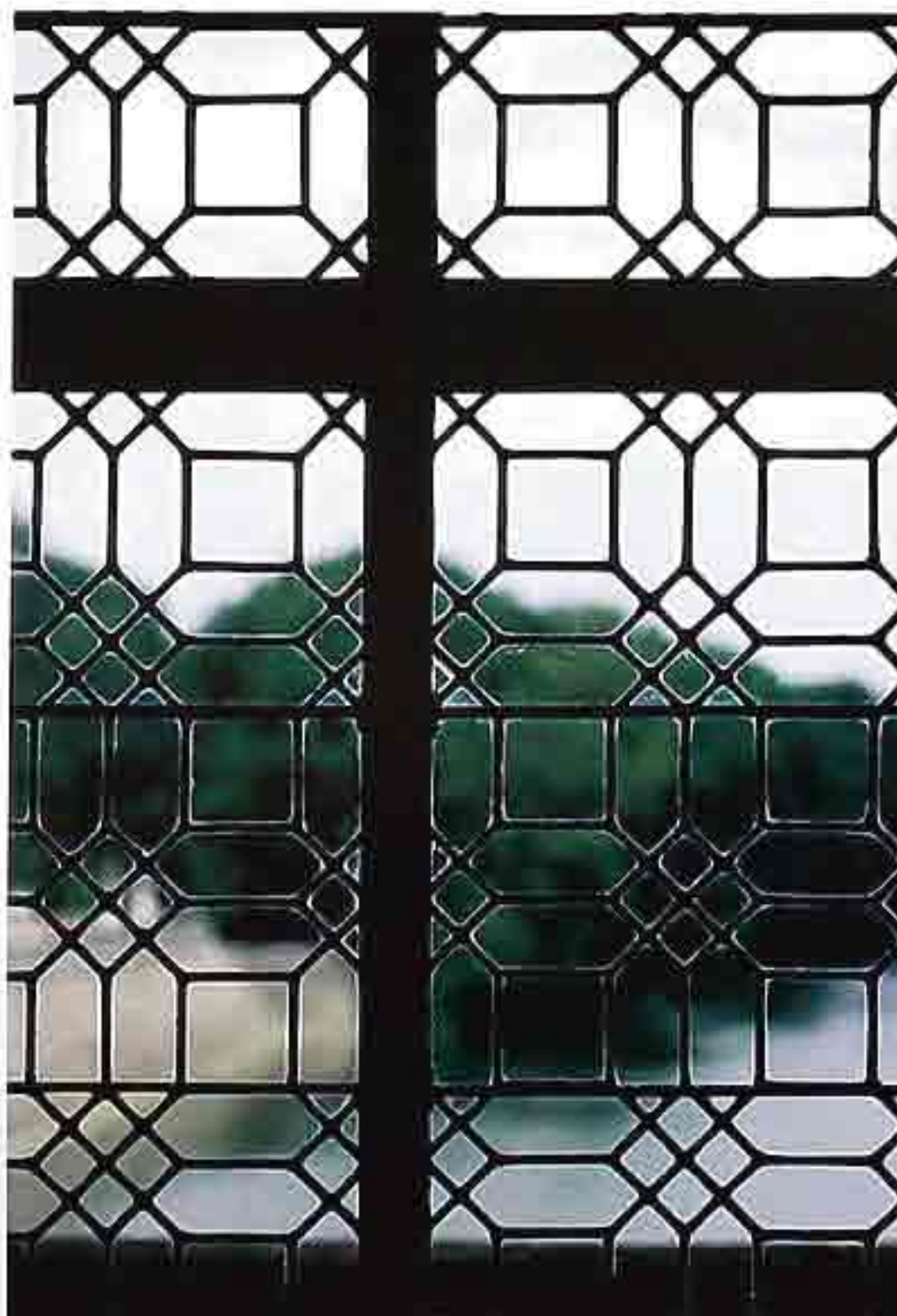
WI-4 Leaded glass with octagonal brass-muntins in interlocking pattern
