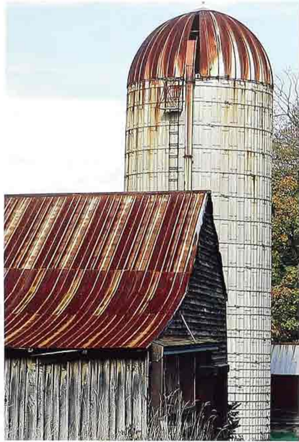
CR-37 Weathered corrugated metal roofs with flared gable on barn and domed roof on silo.
