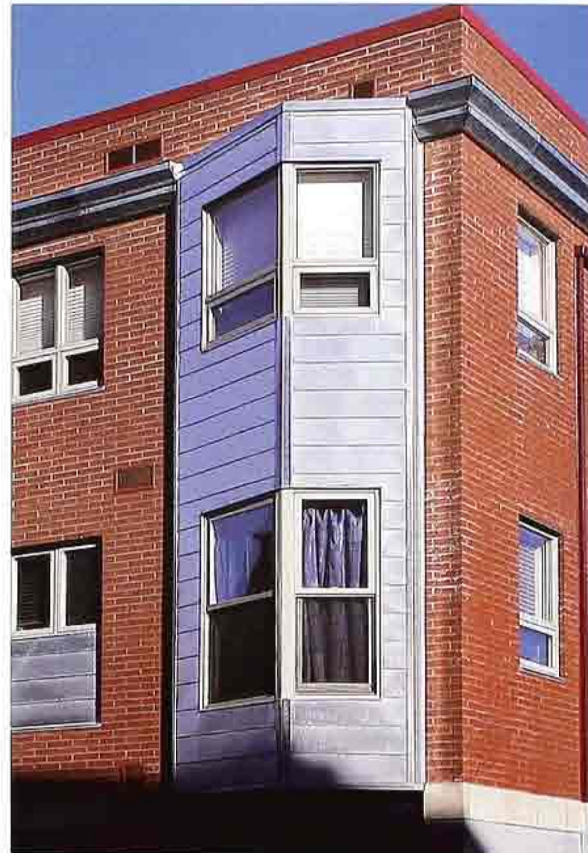
WI-81 Metal-clad two-story angled bay. Top: fixed windows with awning lights; bottom: one-over-one double-hung sashes, modern apartment house
