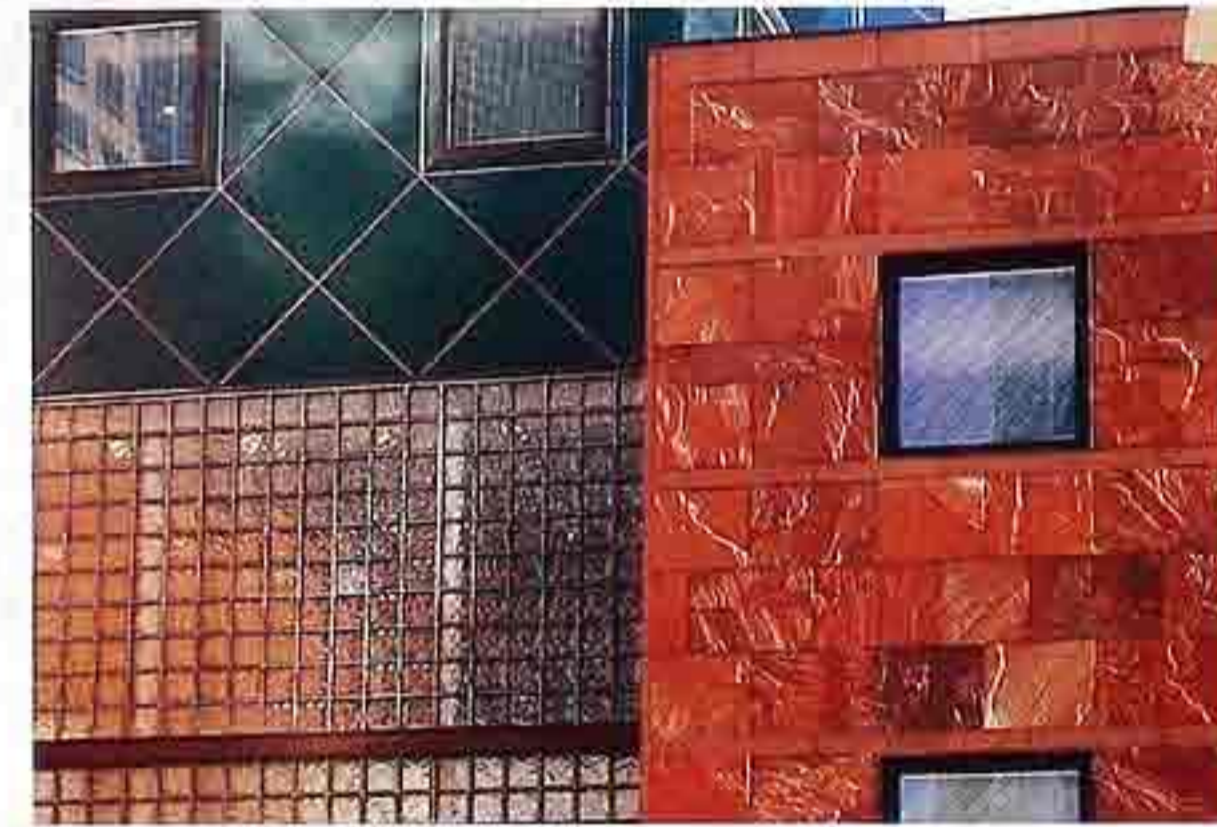
WA-300 Split-face sandstone with glass block and tile (top left), modern commercial building
