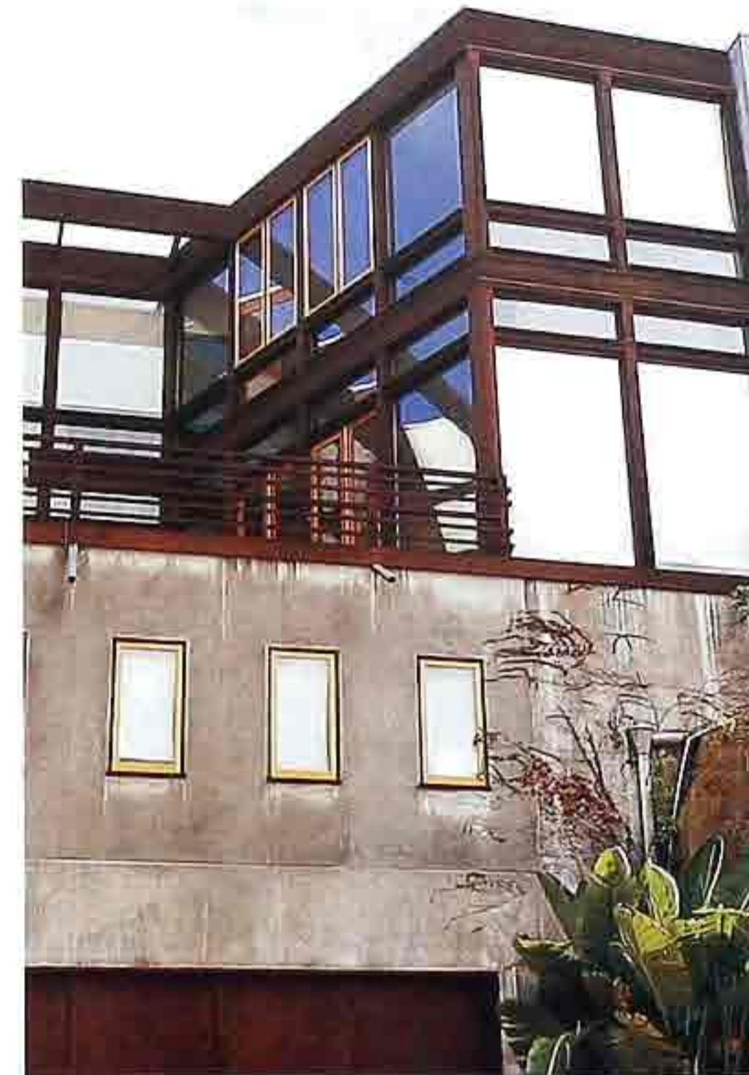
WA-208 Weathered cast-in-place concrete with smooth finish; metal and glass upper story, modern house
