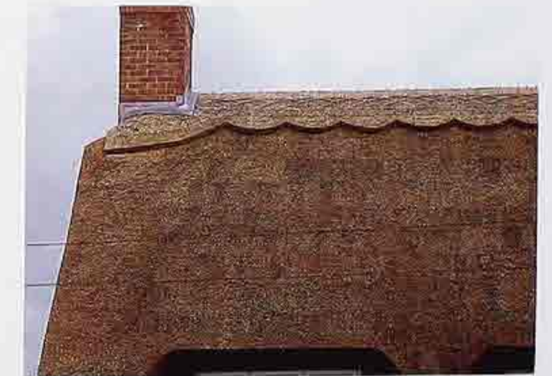
CR-73 Scalloped roof ridge on traditional English thatched house
