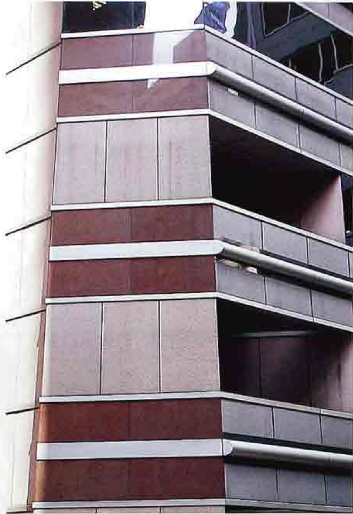
OM-79 Metal molding in a panelized wall system resembling an exaggerated bead molding flattened when it turns the corner
