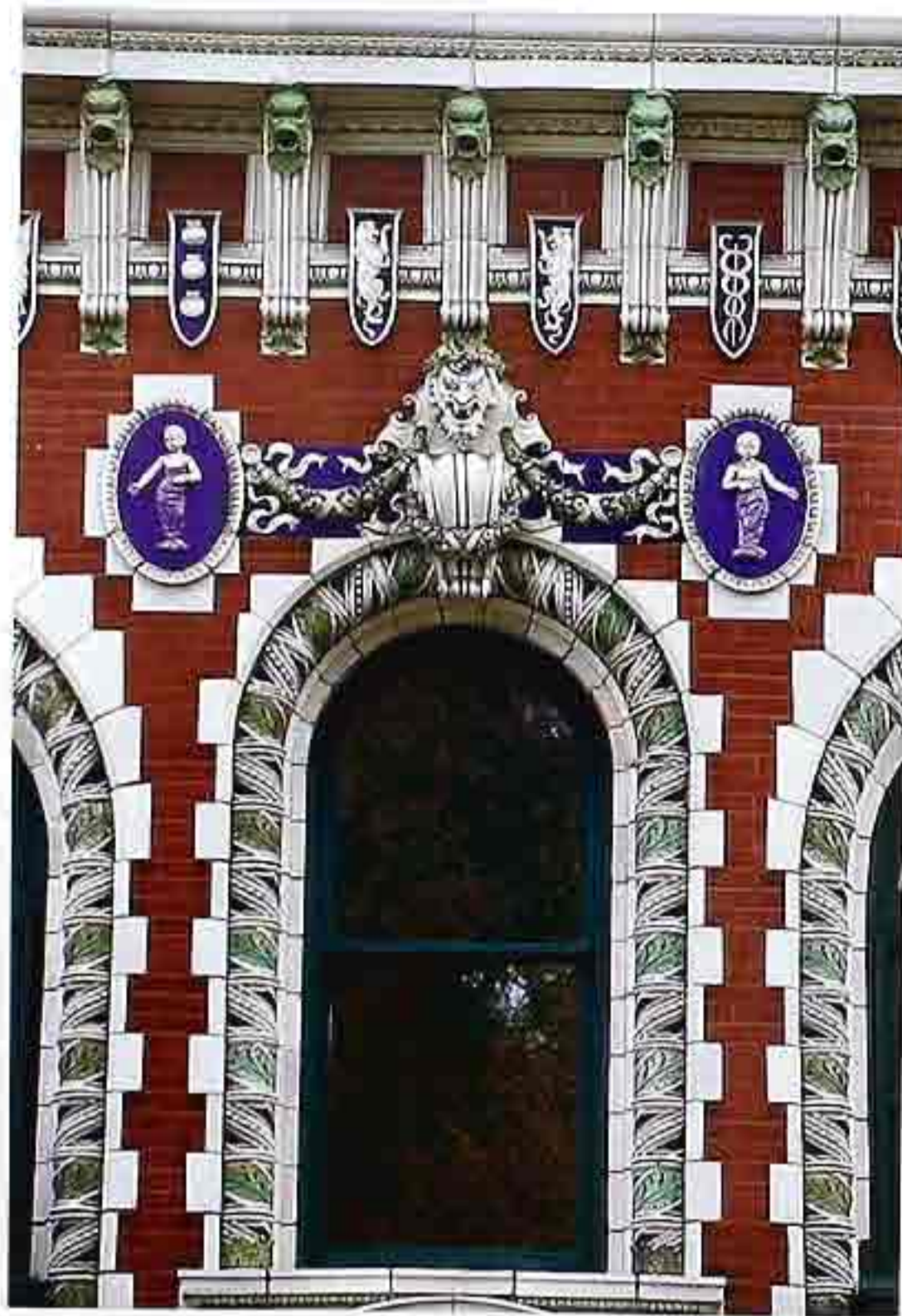
FA-59 Brick facade with polychrome glazed ornamental details: bracket cornice, cartouches, garlands, ancon, and rope molding around semicircular windows.
