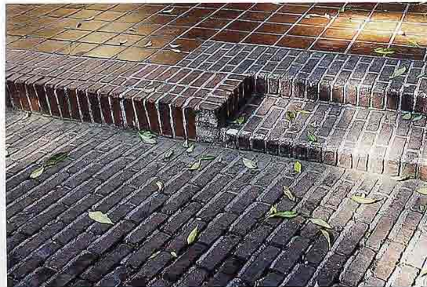
FP-60 Top to bottom: Mexican paving tile, straight-joint installation; mortared brick pavement and steps in running bond; soldier-course brick curb, residential entry
