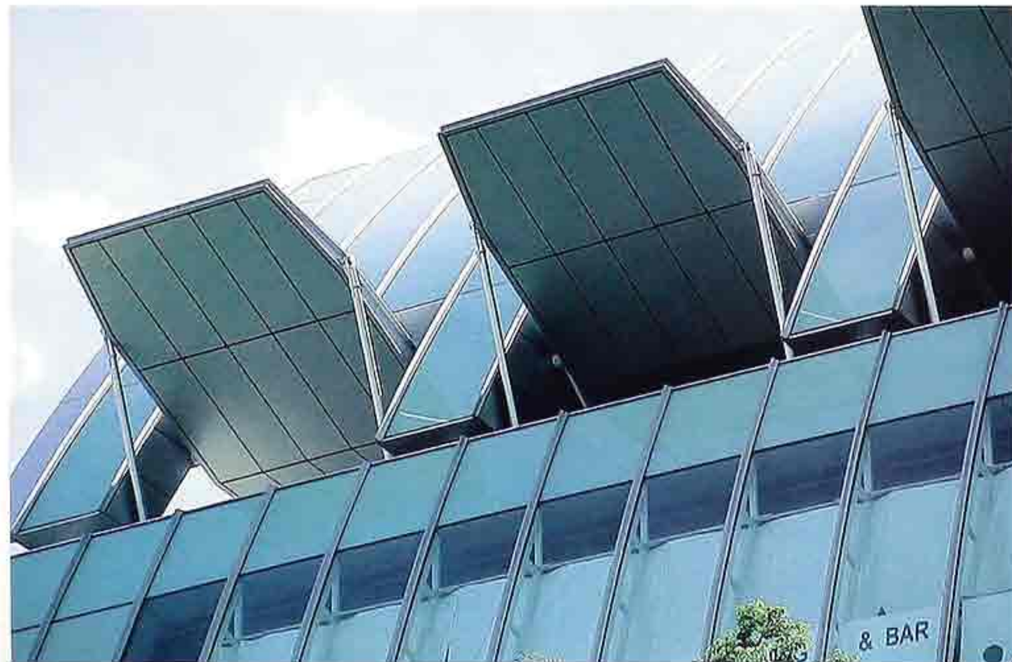
WI-204 Skylight shutters, modern commercial building
