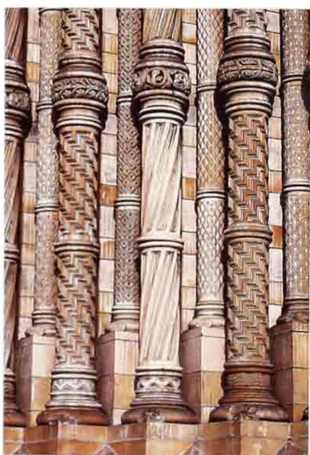
CP-68 Gothic-style jamb-shafts with annulets; varied shaft treatments: spiral fluting and stepped helical geometric pattern
