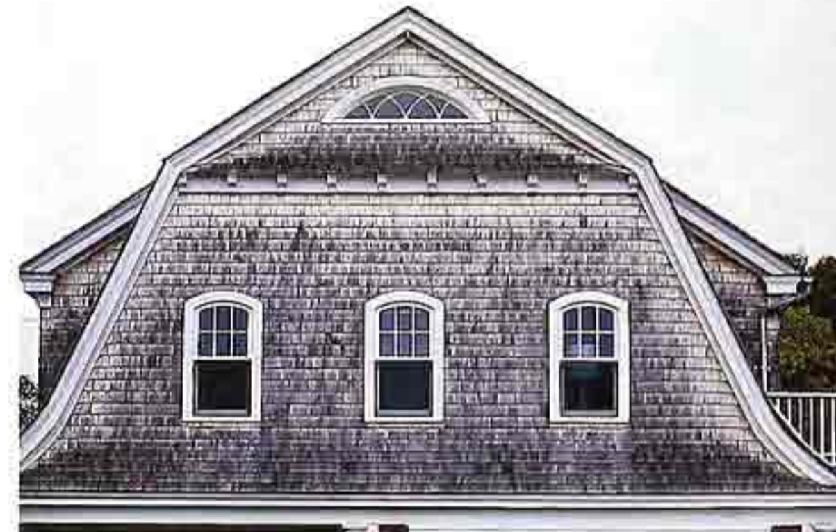
CR-96 Gable-end wall of flared gambrel roof with white cedar shingles; corbelled tie spanning gable
