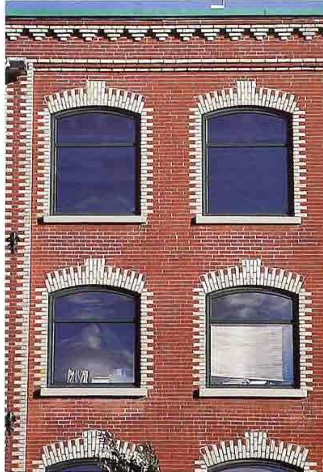
WI-119 Gauged-brick segmental-arch windows with brick quoins and "keystones" in contrasting color
