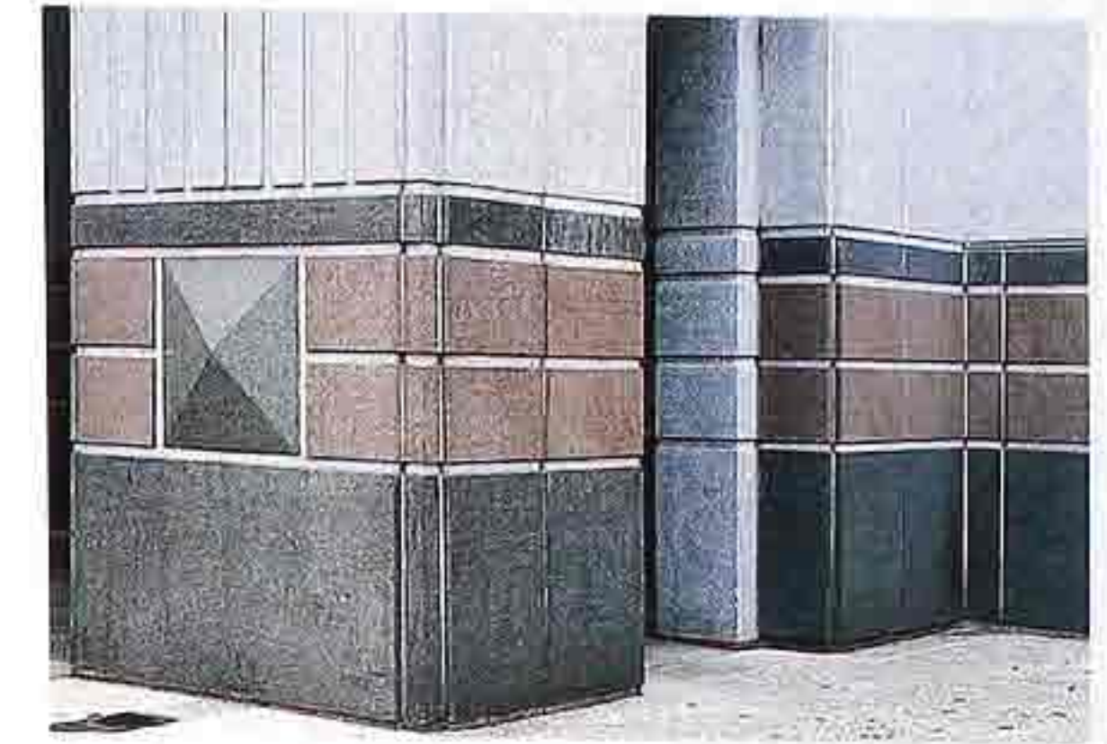
WA-127 Corner detail of polychrome banded granite veneer with gem-cut decorative block
