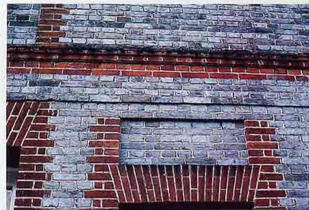
WA-173 Jack-arch window and dog-tooth course of contrasting brick in English bond wall with recessed panel
