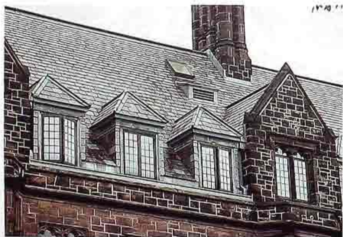
CR-97 Three hipped-roof dormers and a gabled wall dormer; slate cladding on roof dormers and roofs
