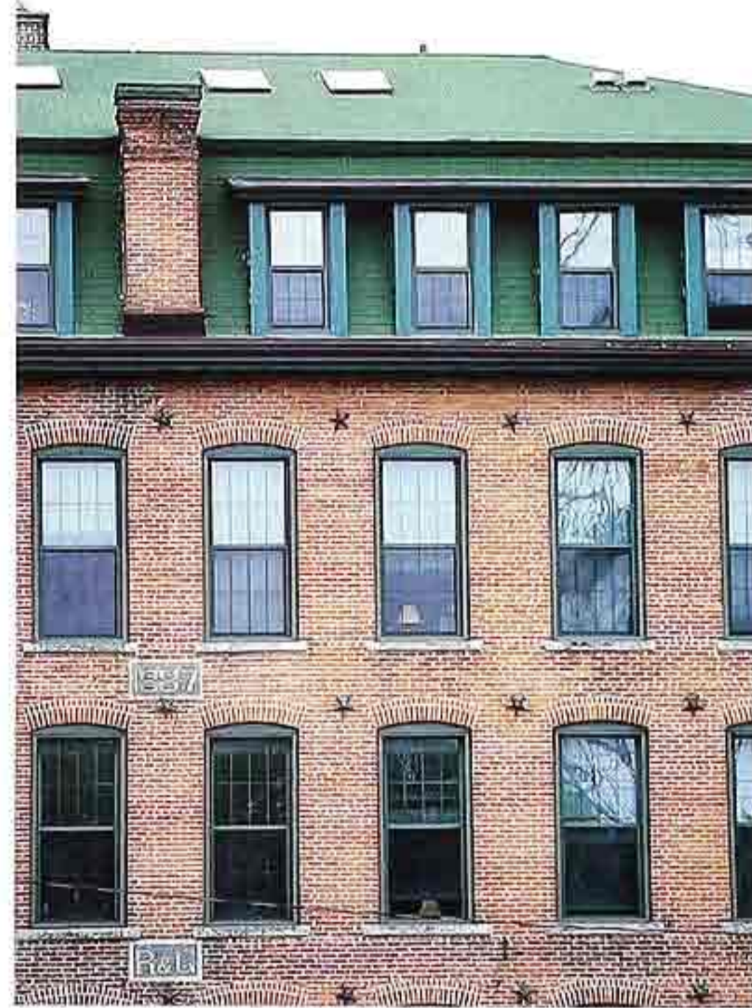
WI-56 Double-hung metal or vinyl replacement windows with internal muntins, 19th-c. brick industrial building
