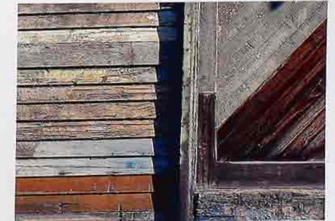
FA-101 Weathered painted clapboard and siding with diagonal board framed door
