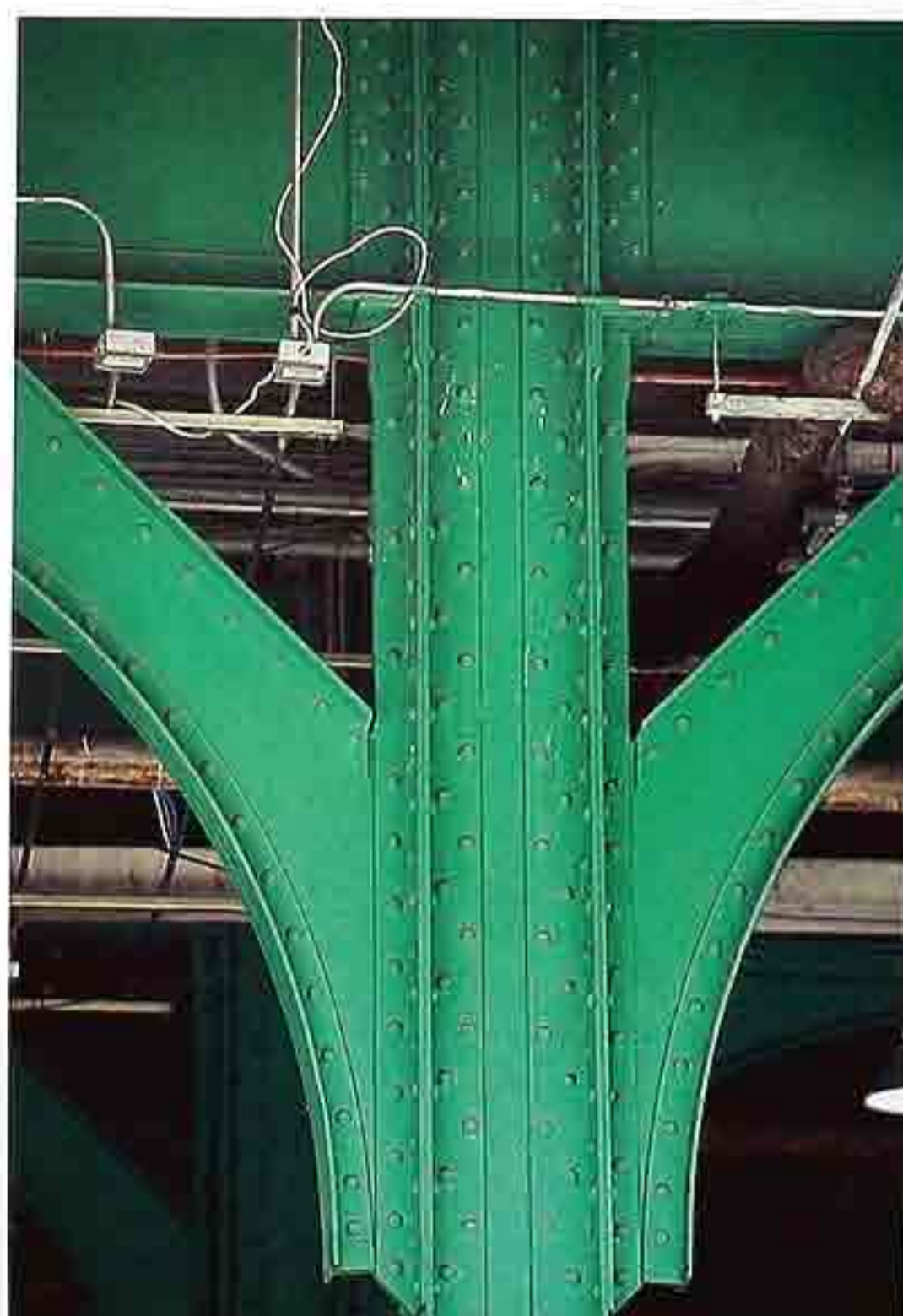
CP-125 Painted steel truss of riveted plates, industrial building
