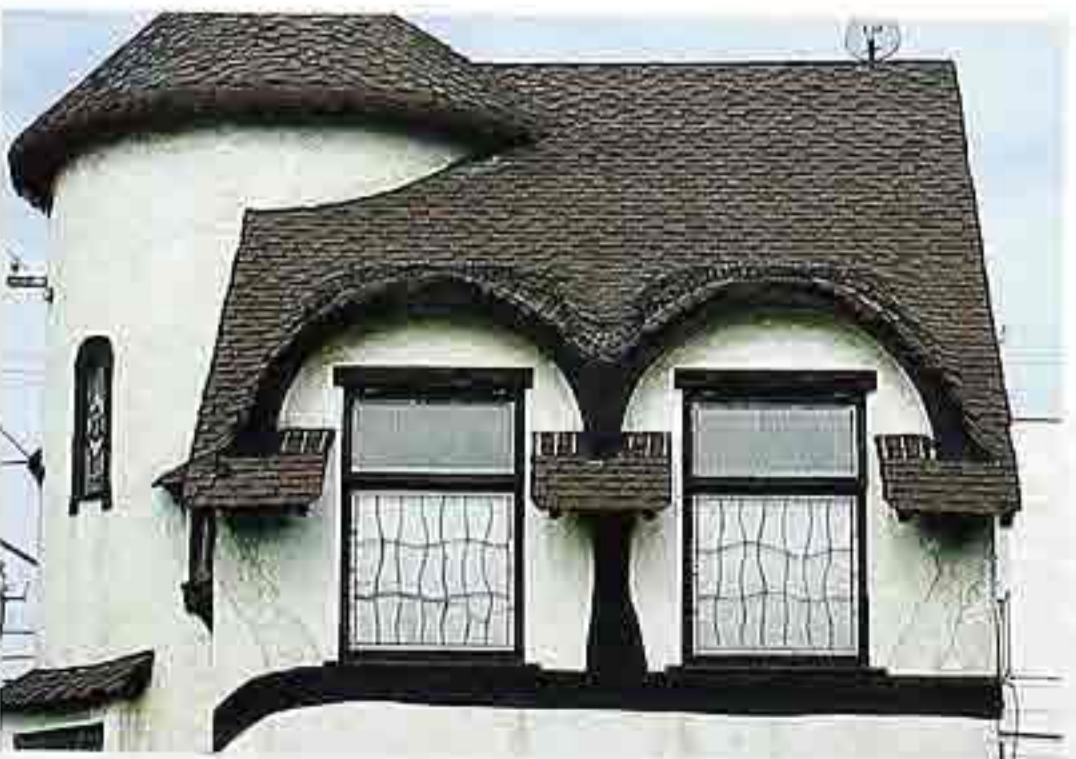
CR-68 Asphalt shingles on roof with arched wall dormers
