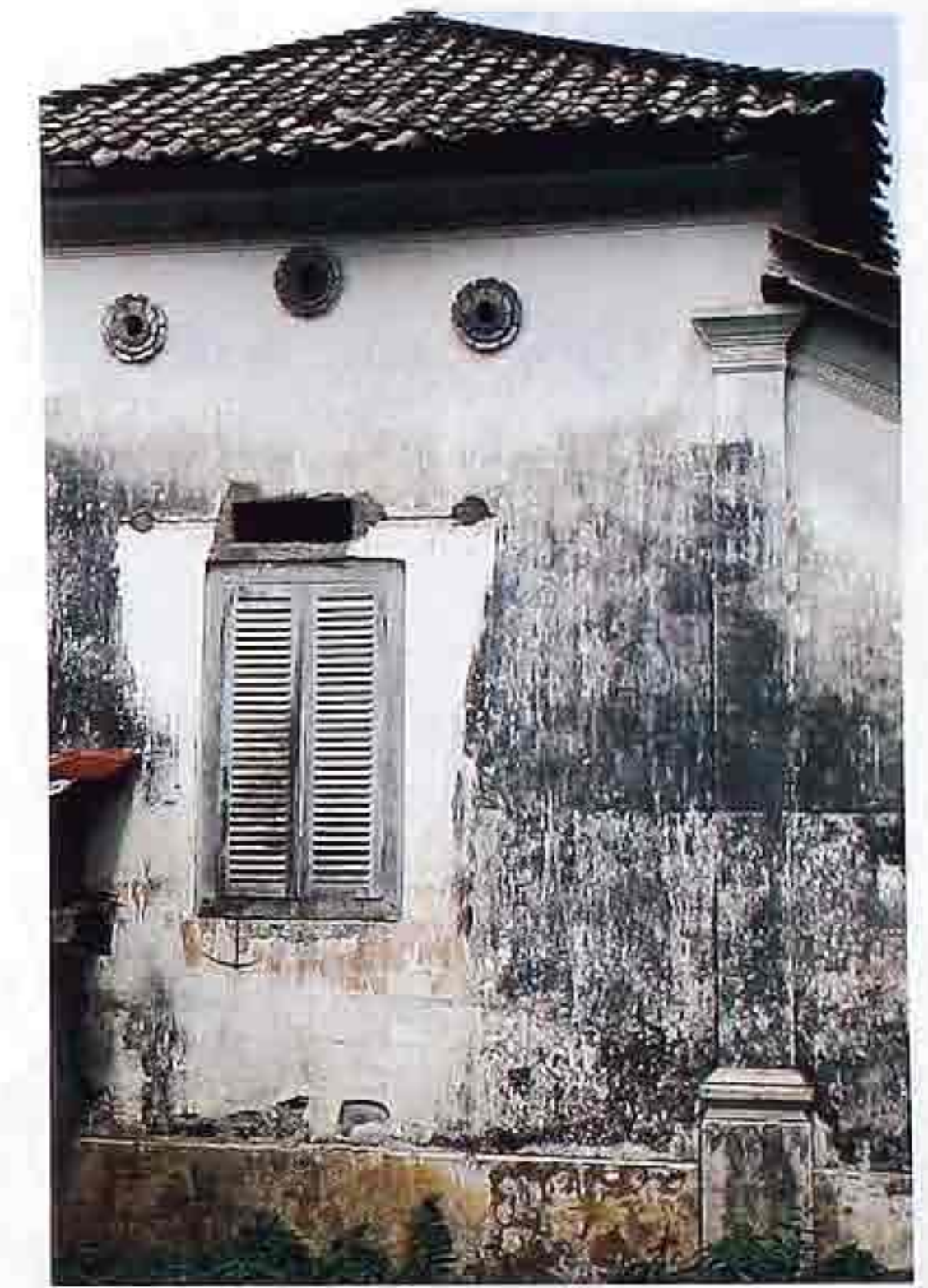
WA-261 Weathered stucco wall with pilaster
