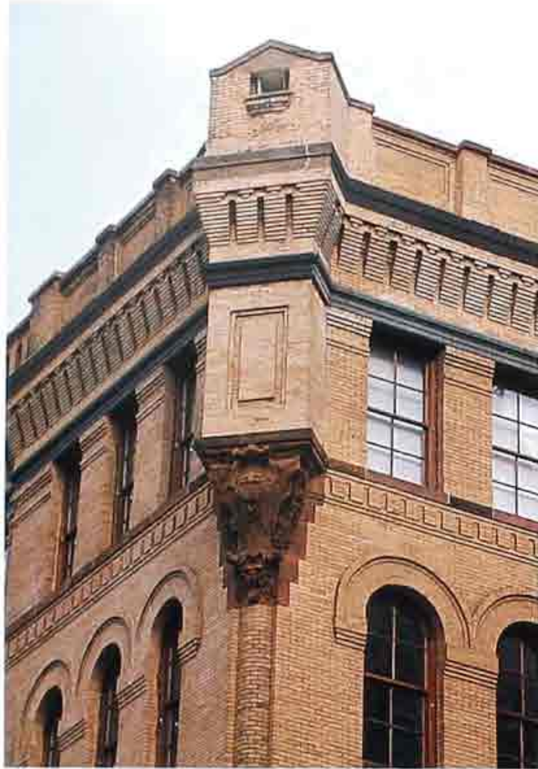
WA-189 Romanesque-style decorative brickwork with ornate corbel on corner below parapet roof
