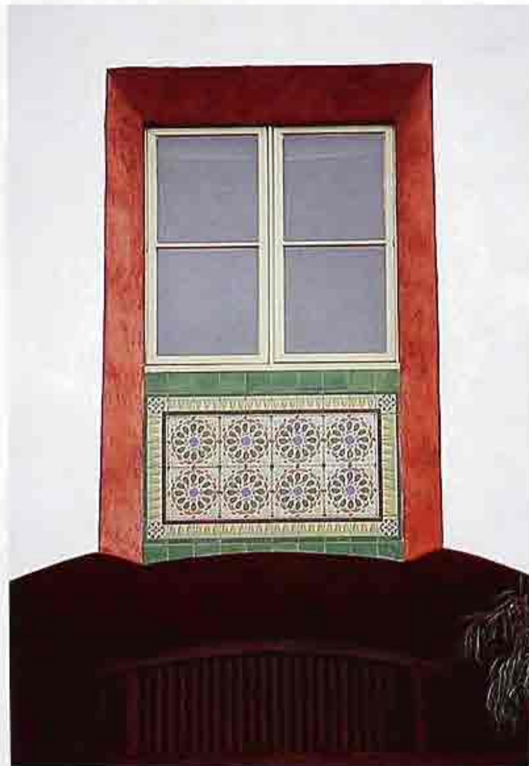
WI-152 Square casement window recessed in stucco wall above arch; painted Spanish-colonial-style motifs
