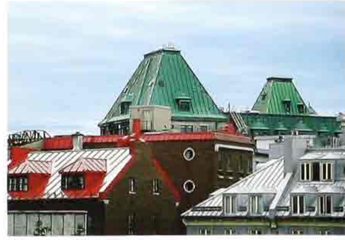
CR-116 Parapeted gable with hipped-roof dormers (left), hipped roof with hip dormers (right), and flared mansard with hip dormers (top), all sheet metal
