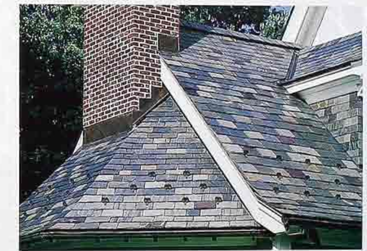
CR-61 Variegated Vermont slate roofing with snow guards
