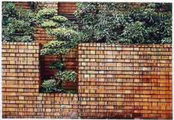
WA-157 Notched garden wall in Flemish bond with rowlock-course coping
