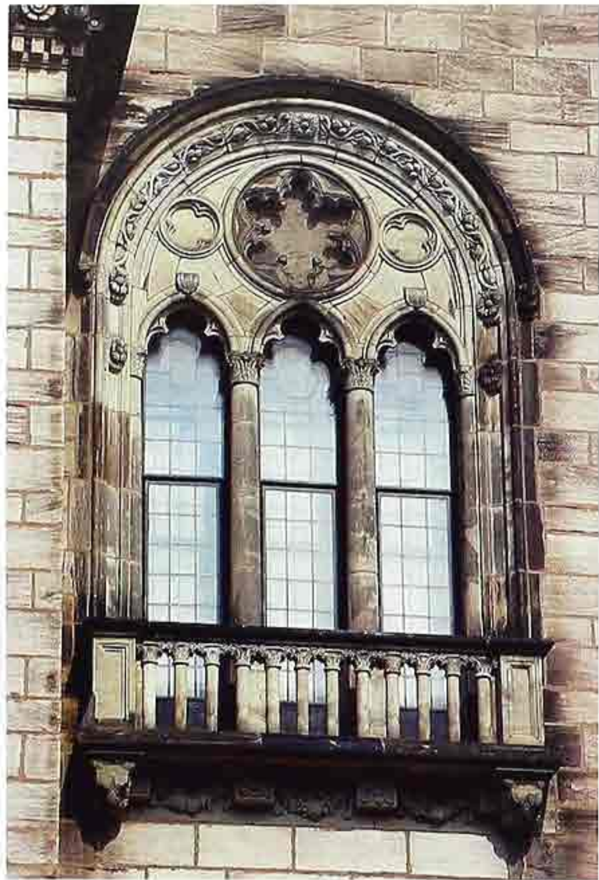
CP-170 Semicircular arch enclosing three compound pointed trefoil arched windows below sexfoil and two trefoil ornaments, with balustrade
