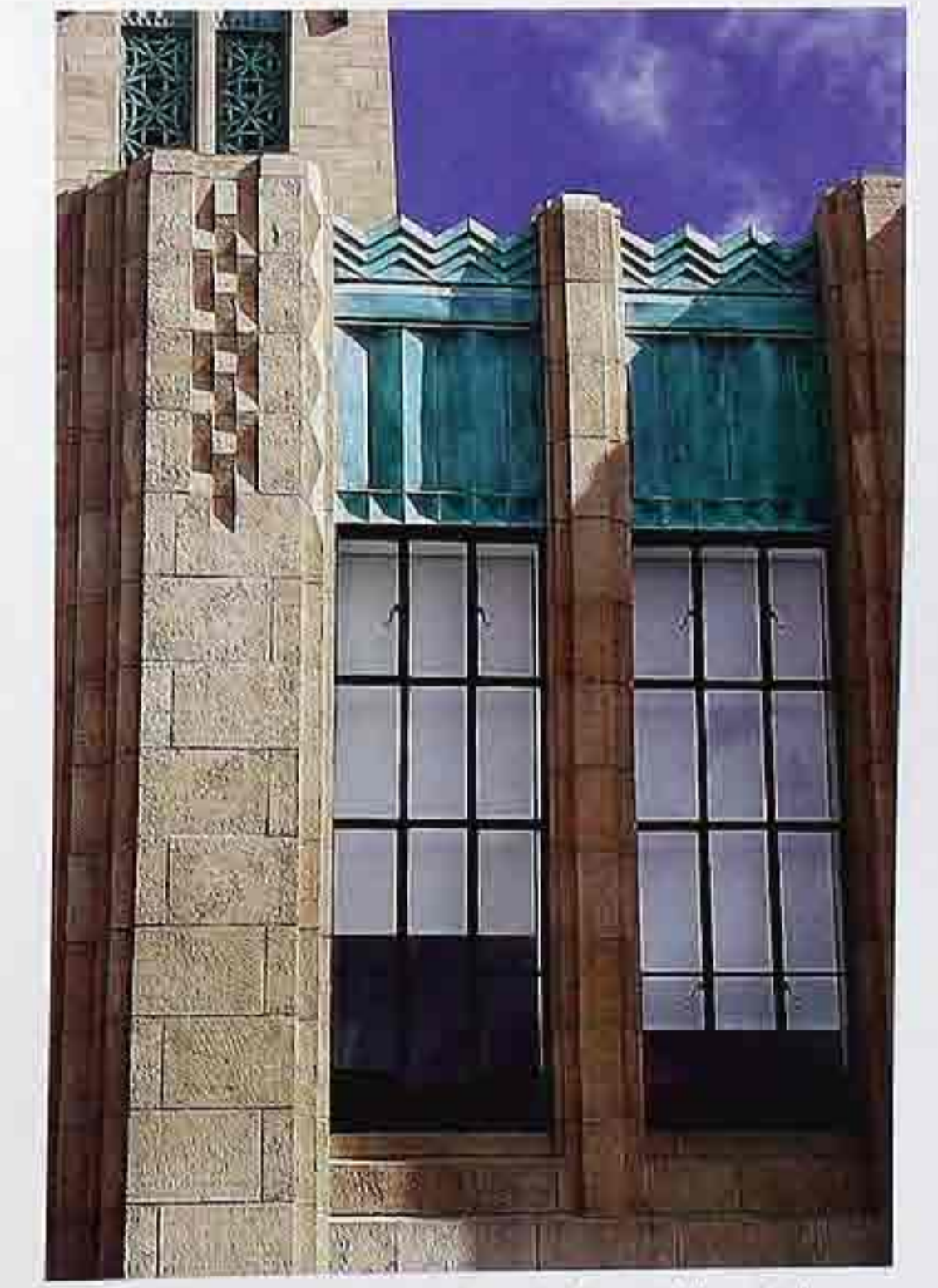
WI-149 Copper panels capping windows with metal sashes in recessed stone casings, 20th-c. commercial building
