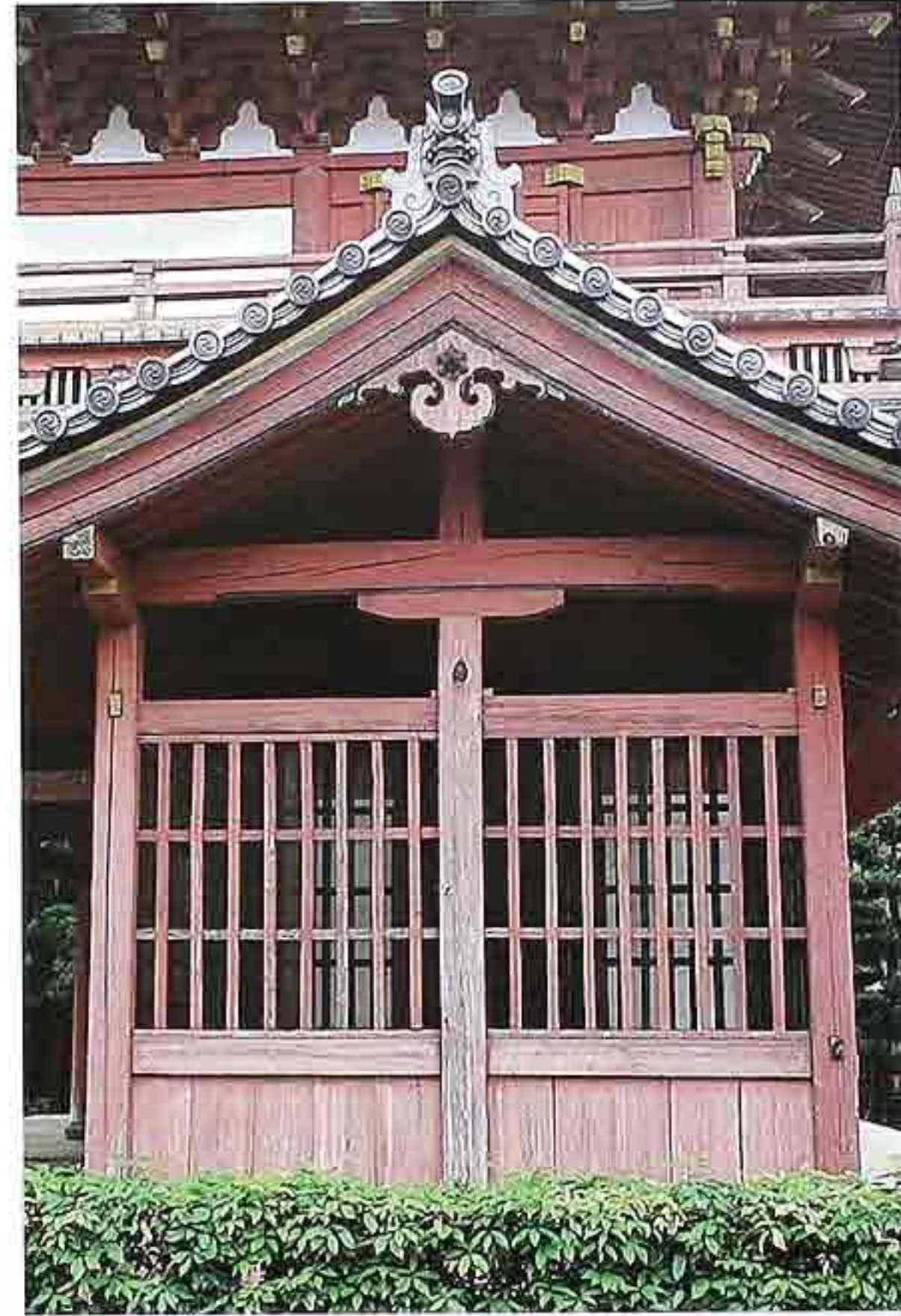
DW-88 Traditional Japanese entry with lattice screen under gable
