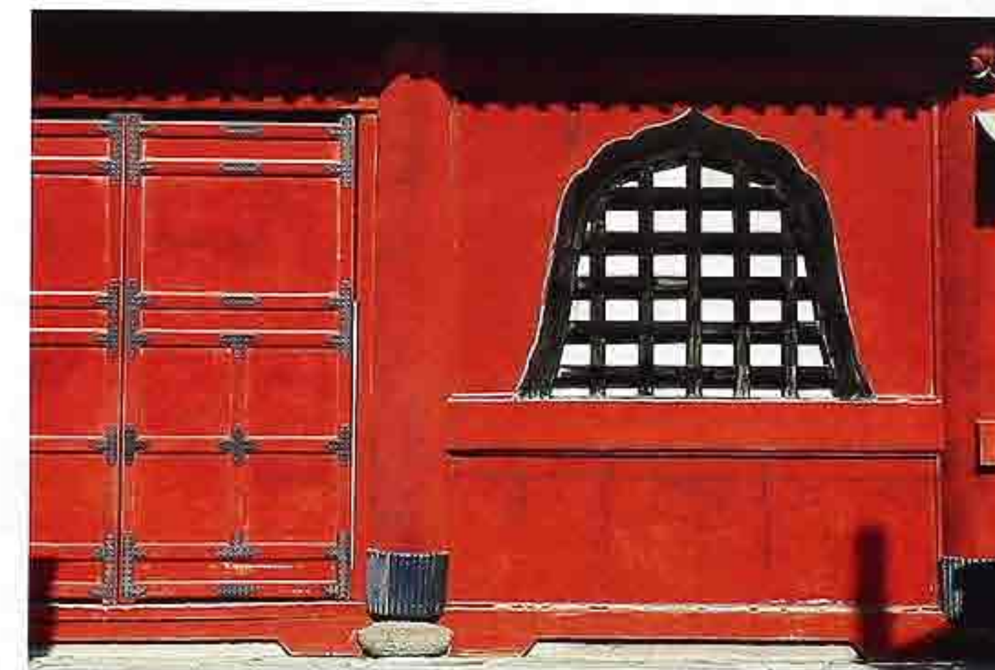
FA-73 Traditional red painted wood-infill post-and-beam facade and paneled door, Japanese entry gate
