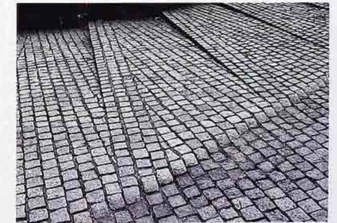
FP-34 Paving stone in ramp-like steps, entry of modern commercial building
