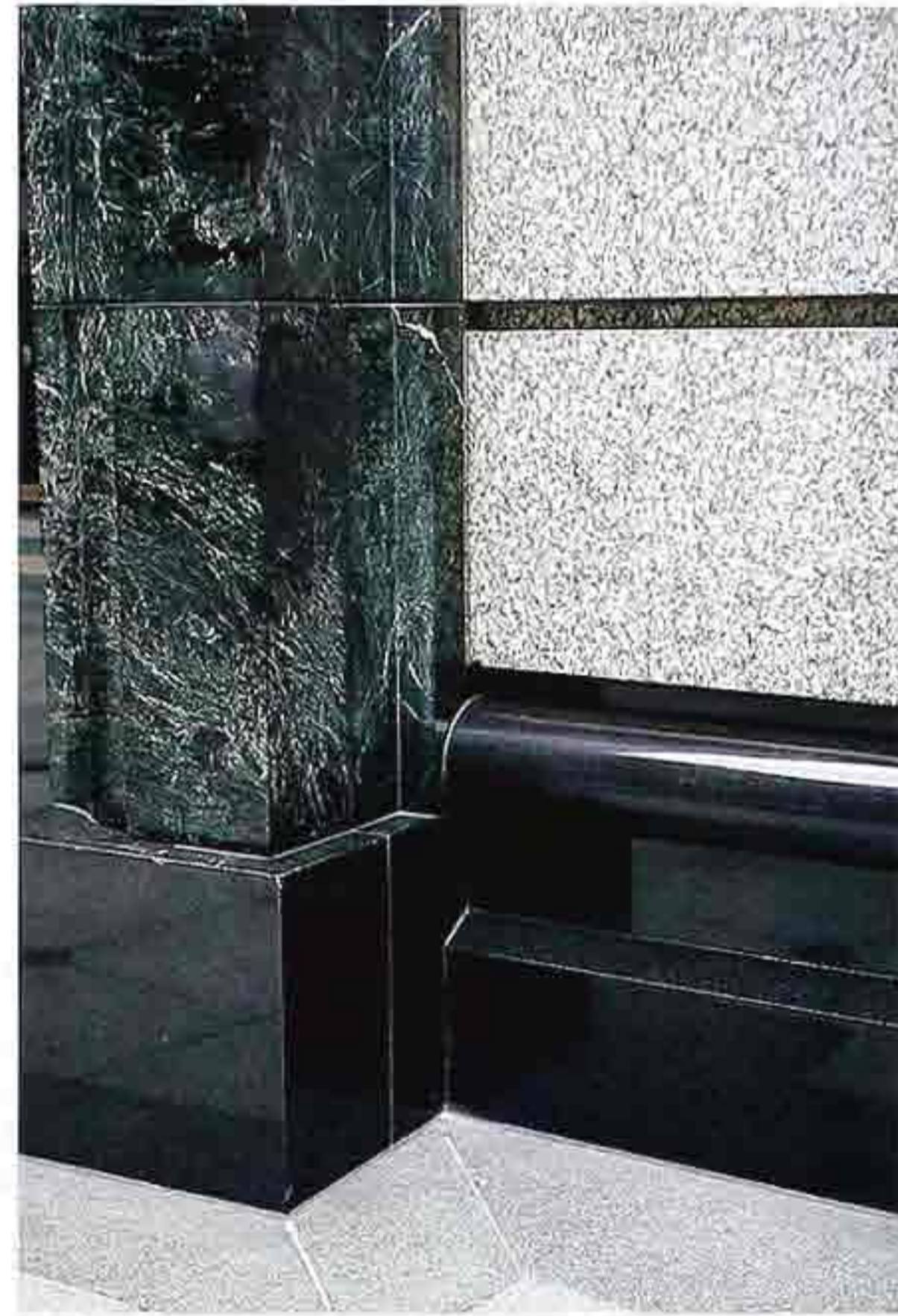
OM-80 Stone base molding with a large bead and plinth with a chamfered top edge
