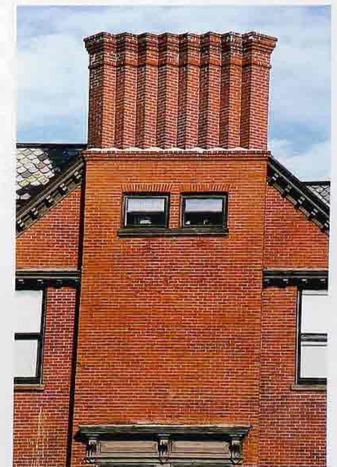
CR-146 Engaged rectangular chimney stack
