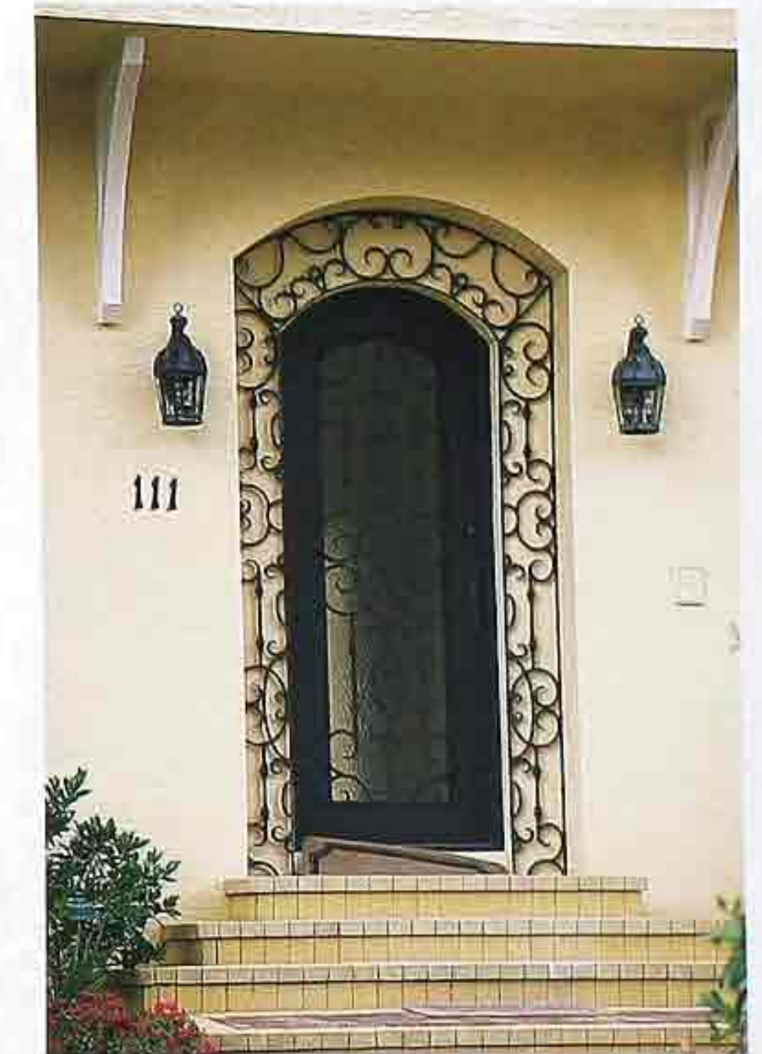
DW-91 Door hood over arched doorway framed with wrought-iron filigree band; metal door with grille over full glass, modern house
