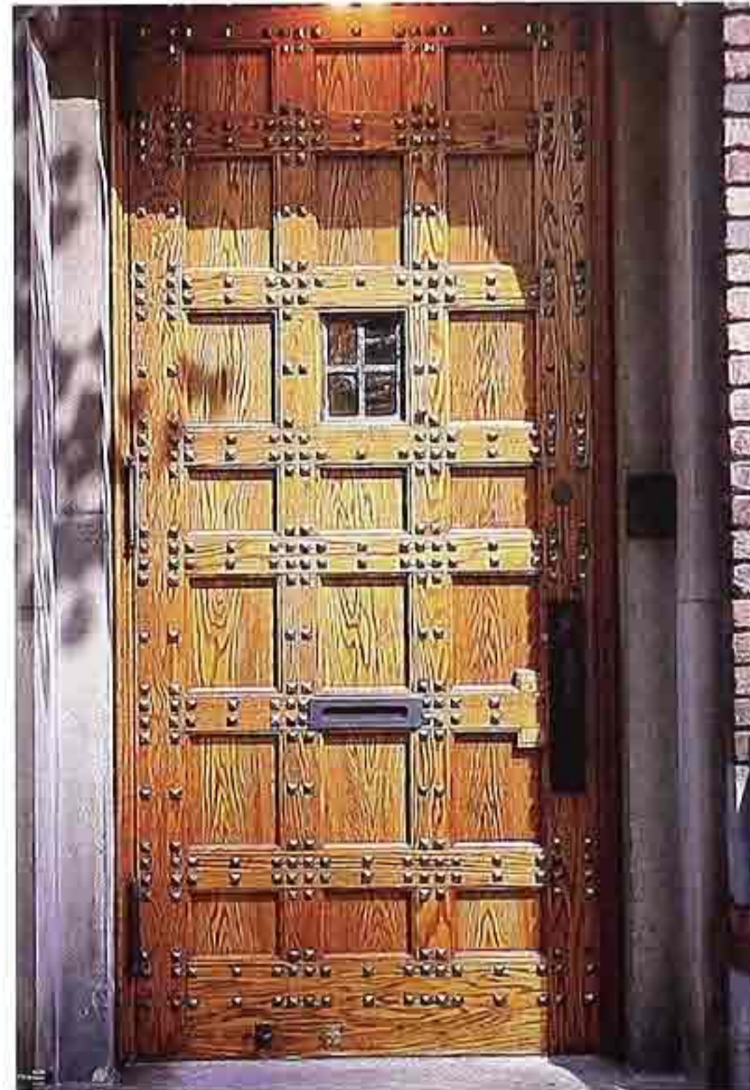
DW-2 Twenty-one panels, wood, with leaded light, mail slot, and decorative studs on rails and stiles
