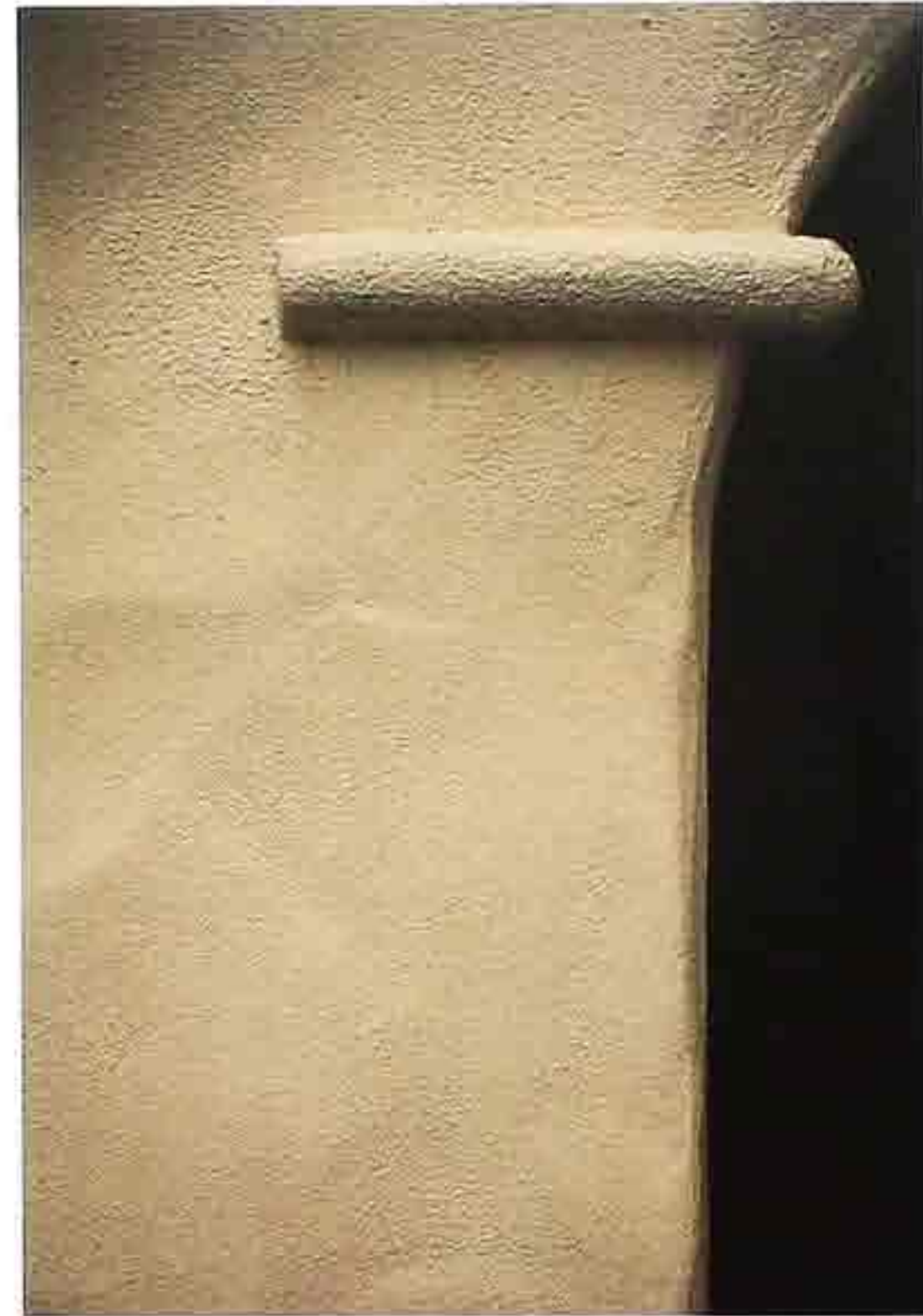
WA-231 Detail of arched opening with impost-like molding, stucco over adobe, American Southwestern mission
