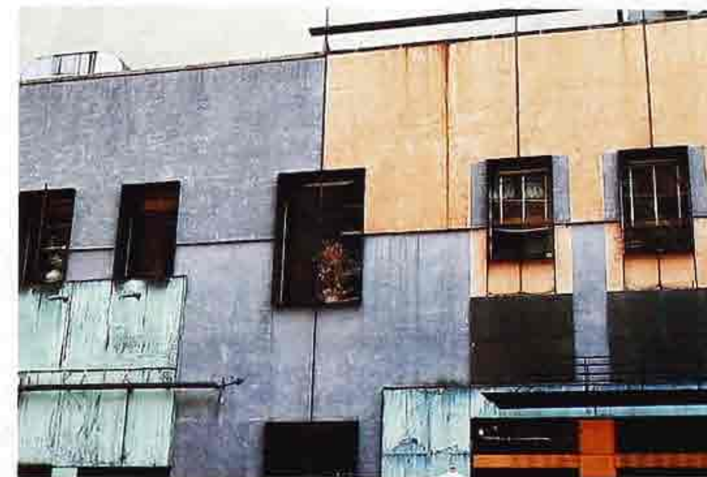
FA-24 Painted and patinated metal panels with lapped seams, modern commercial building
