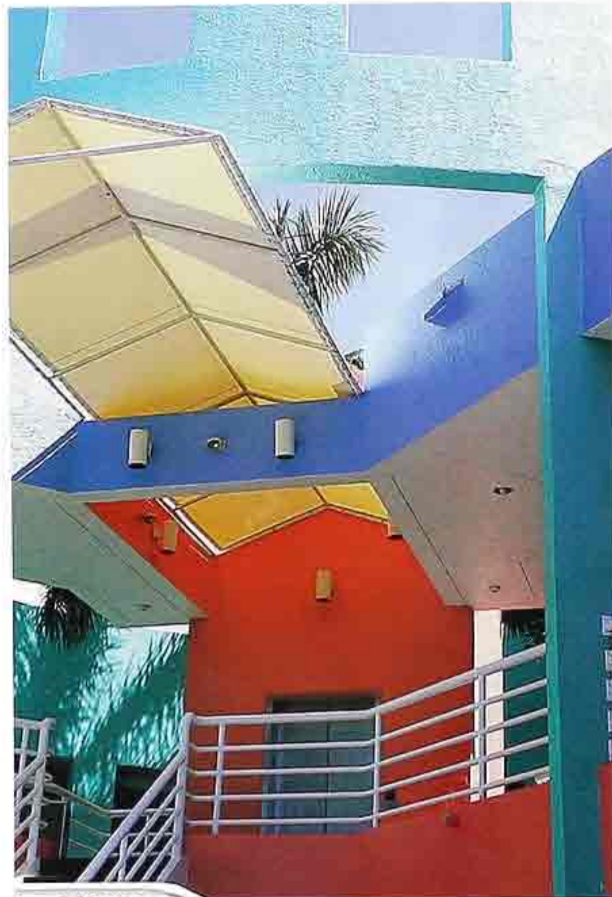
CR-141 Cantilevered fabric awning springing from freestanding stucco wall and ceiling, outdoor public space
