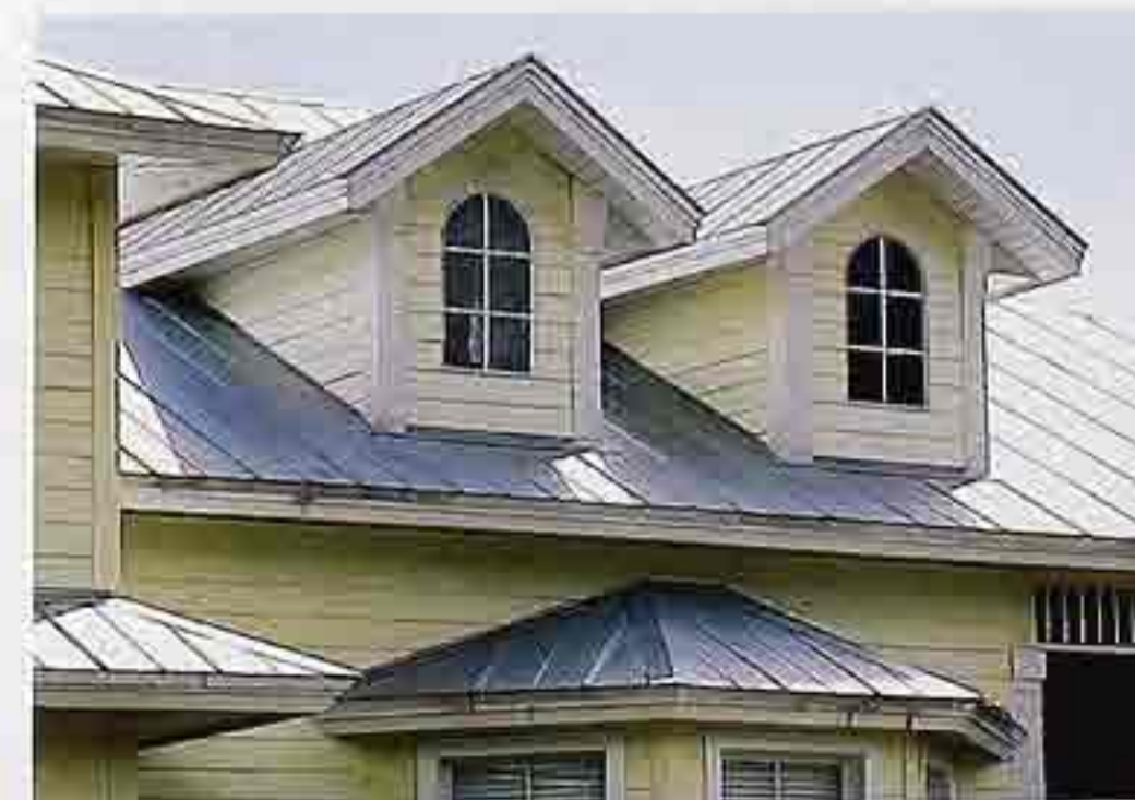
CR-103 Gable-roof dormers with deep eaves
