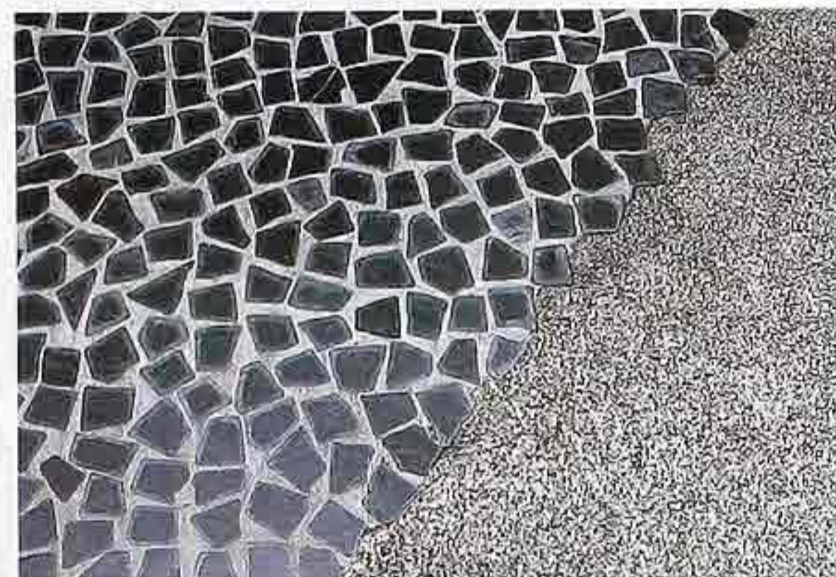
FP-74 Pea-sized gravel aggregate (right) next to randomly shaped and placed tile
