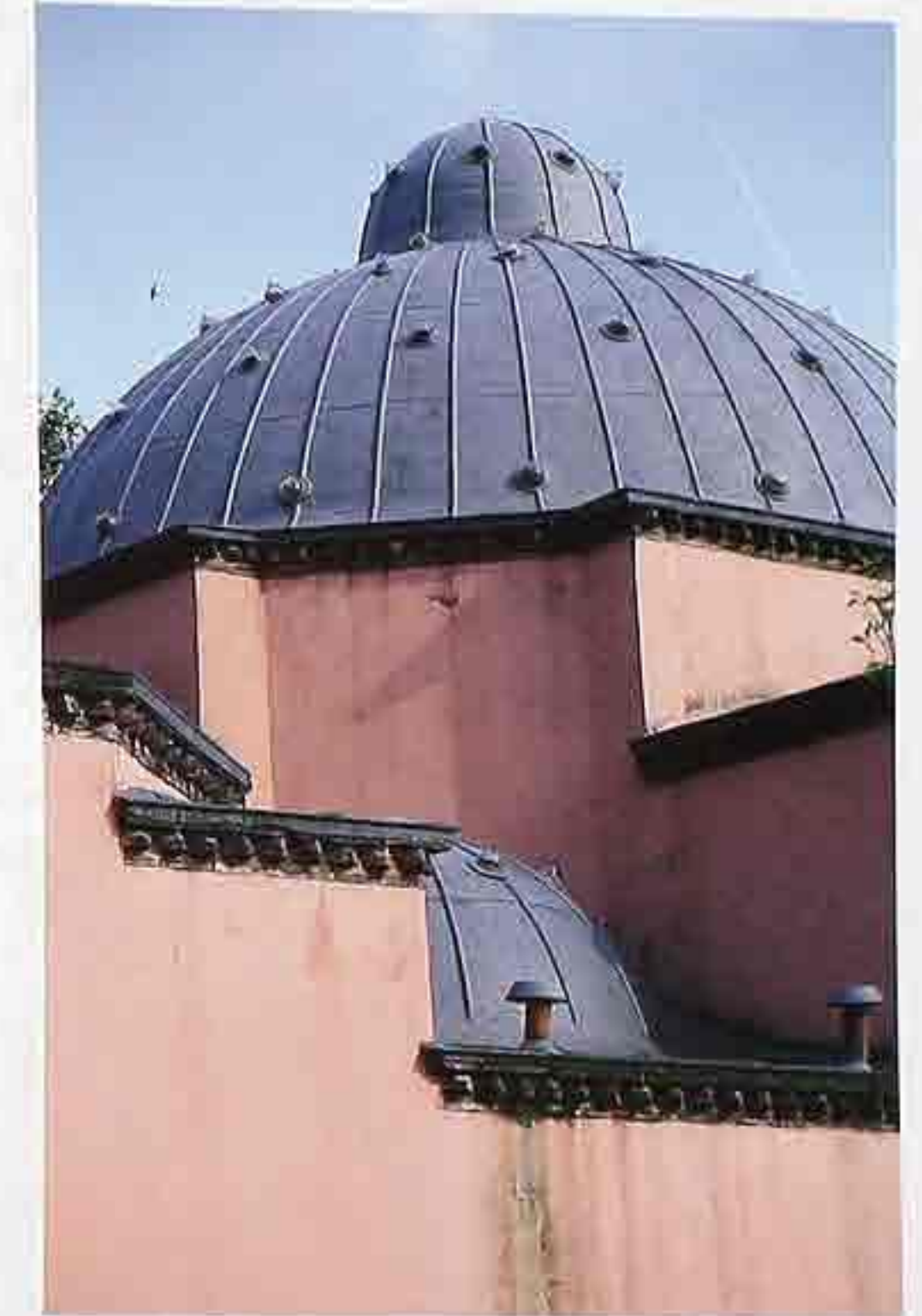
CR-131 Composite dome, metal with standing-seam
