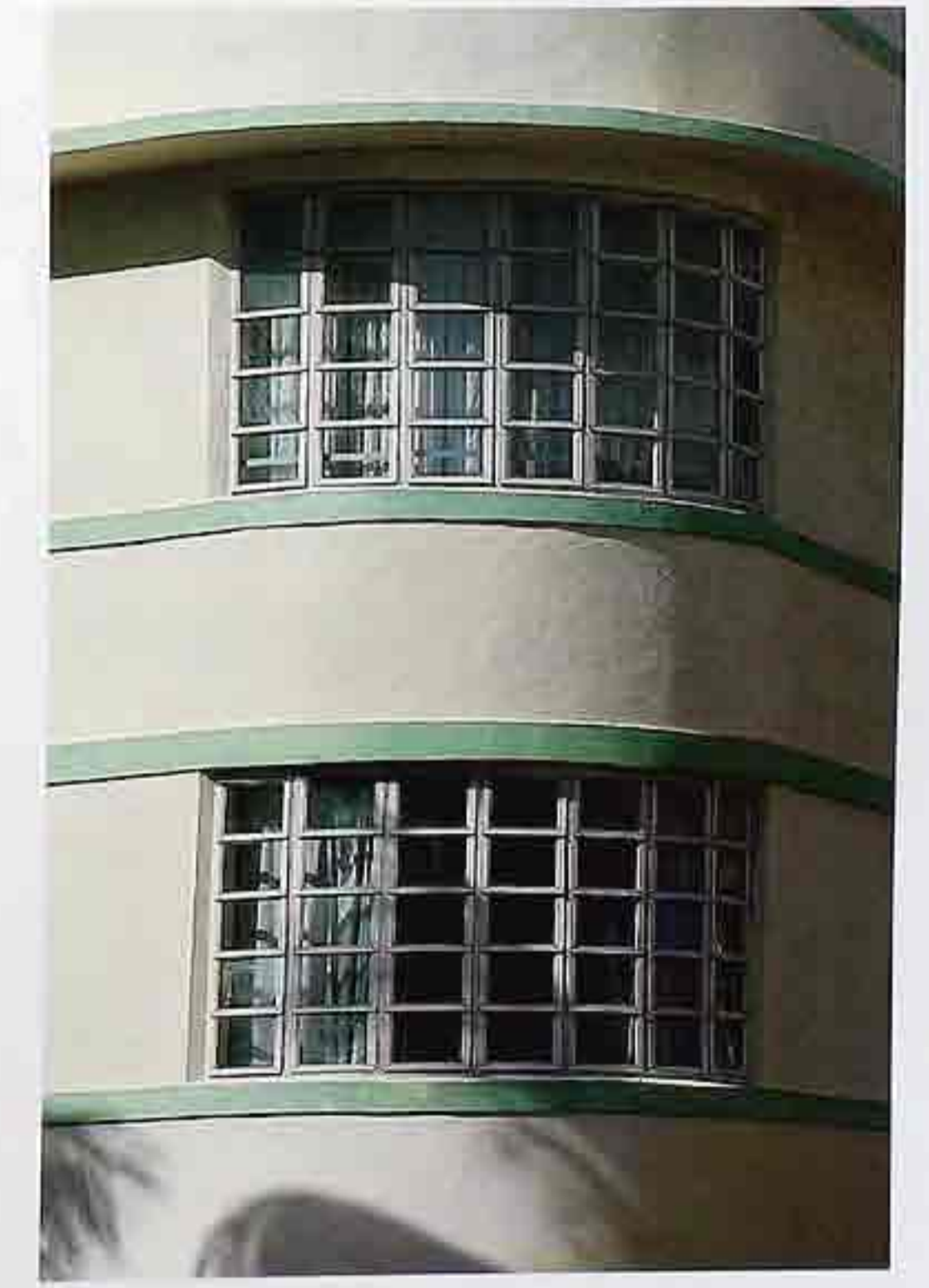
WI-37 Awning windows in curved corner, Art Deco apartment house
