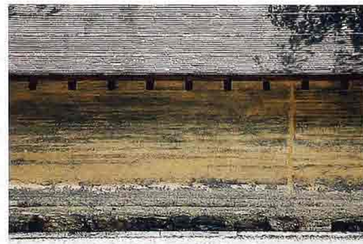
WA-243 Mud wall with layers of tinted mud stucco, courtyard wall
