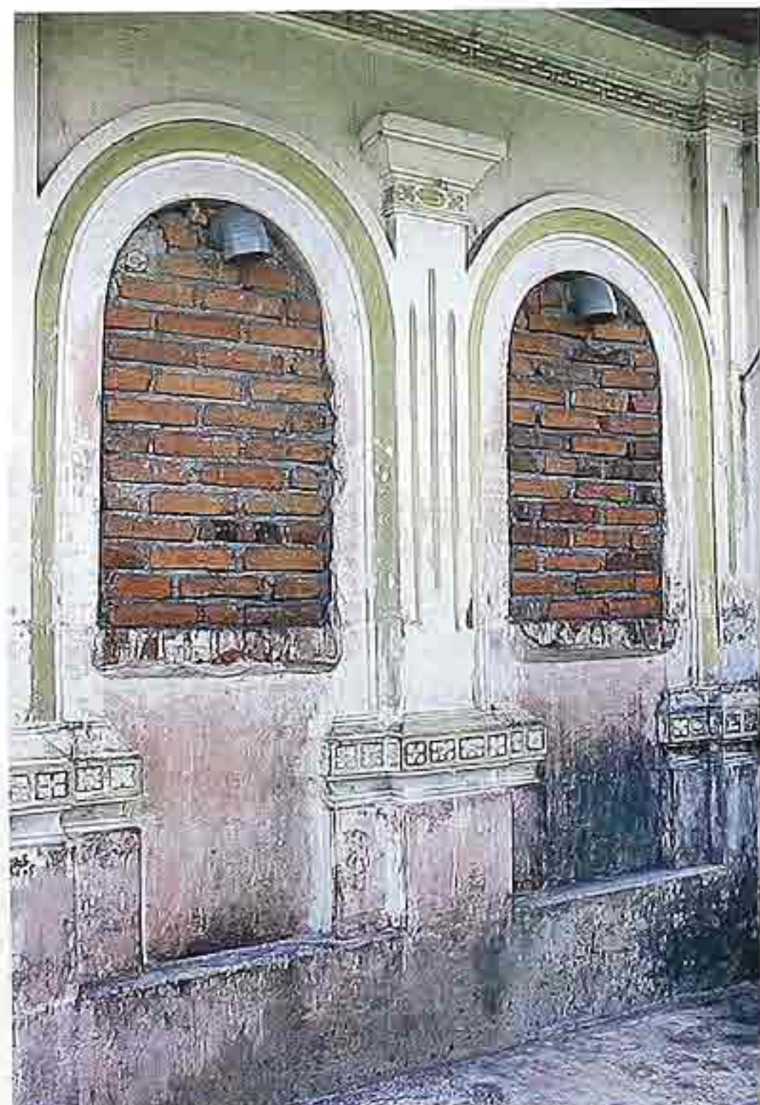
CP-88 Weathered painted pilasters in a blind arcade with semicircular arches
