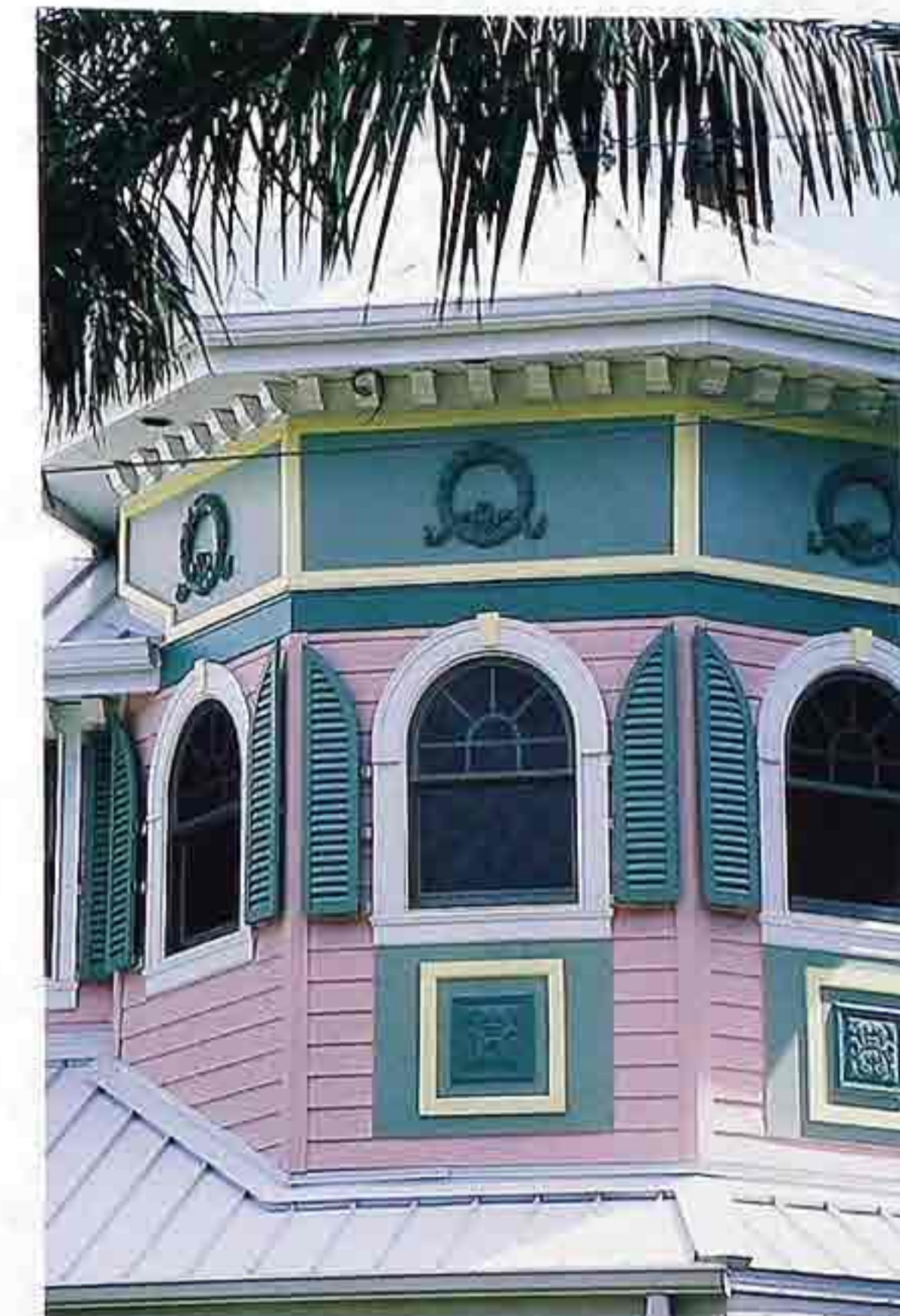
FA-80 Octagonal turret on contemporary polychrome house, modillion cornice, repeated ornament, and ornamental shutters around windows
