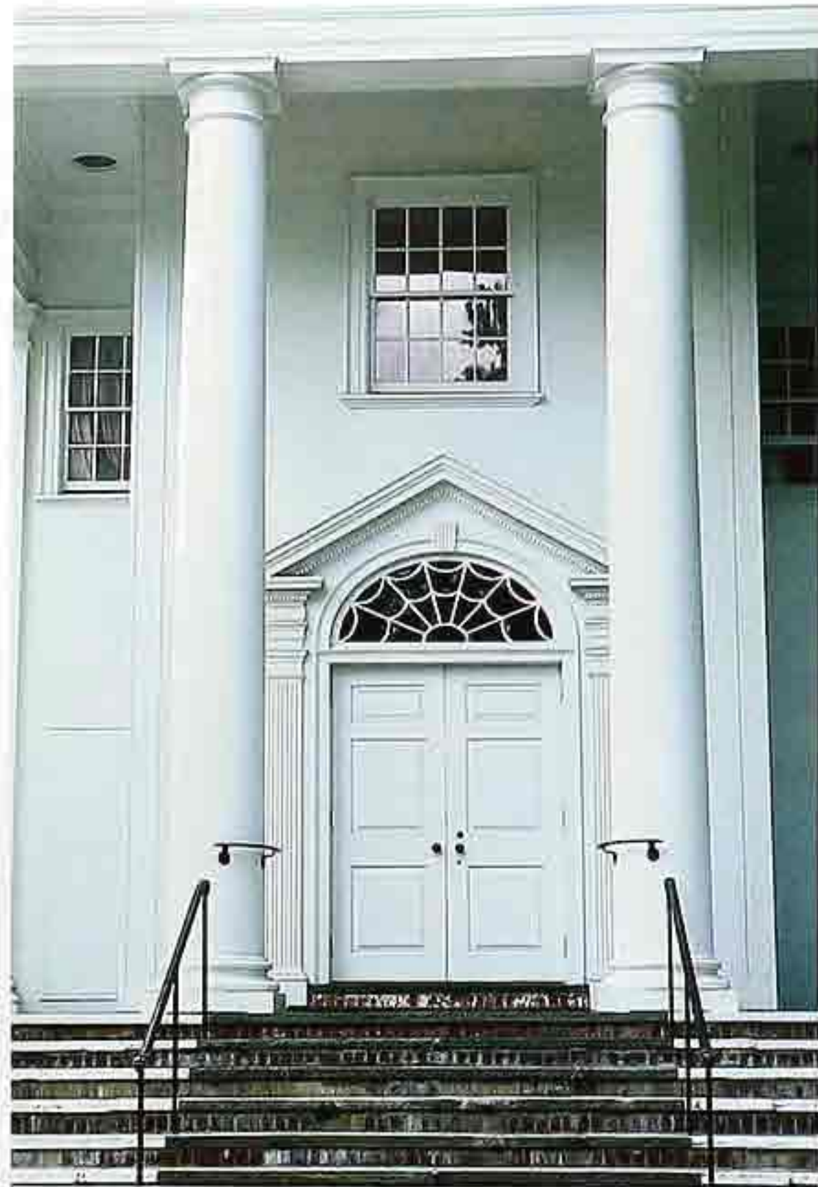
CP-73 Roman-style Doric columns with Attic base supporting portico; pedimented door
