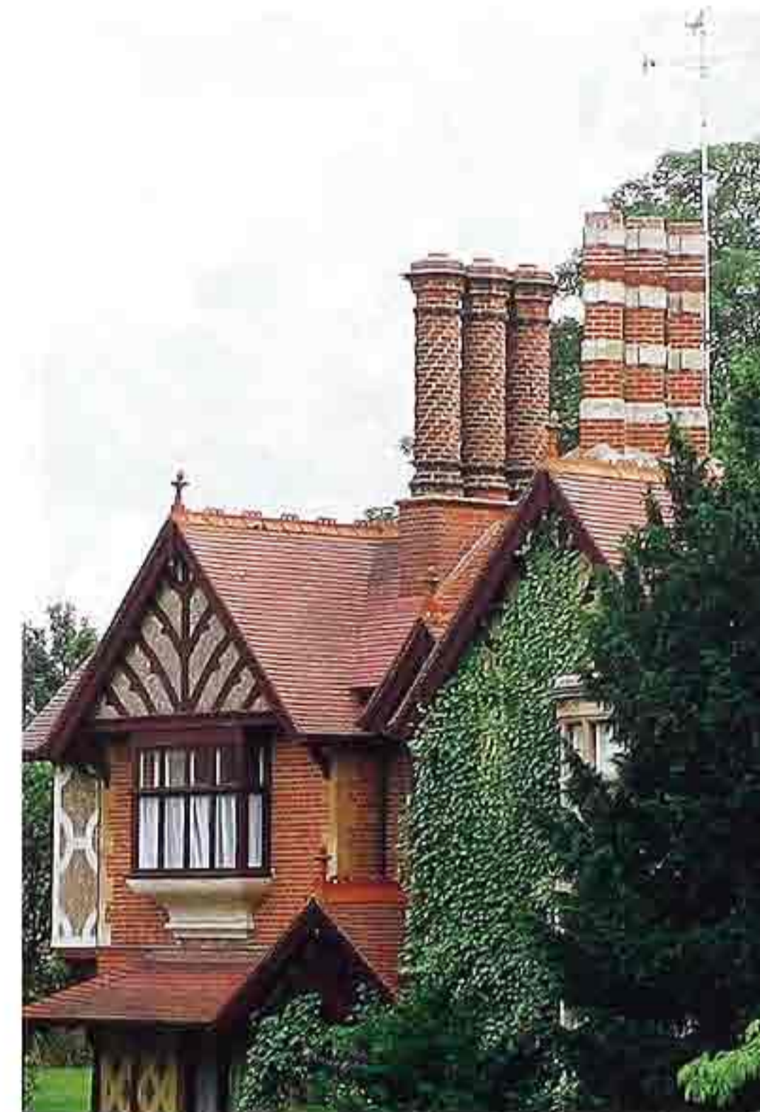
CR-143 Brick-pilaster chimneys: spiral (left); banded (right)
