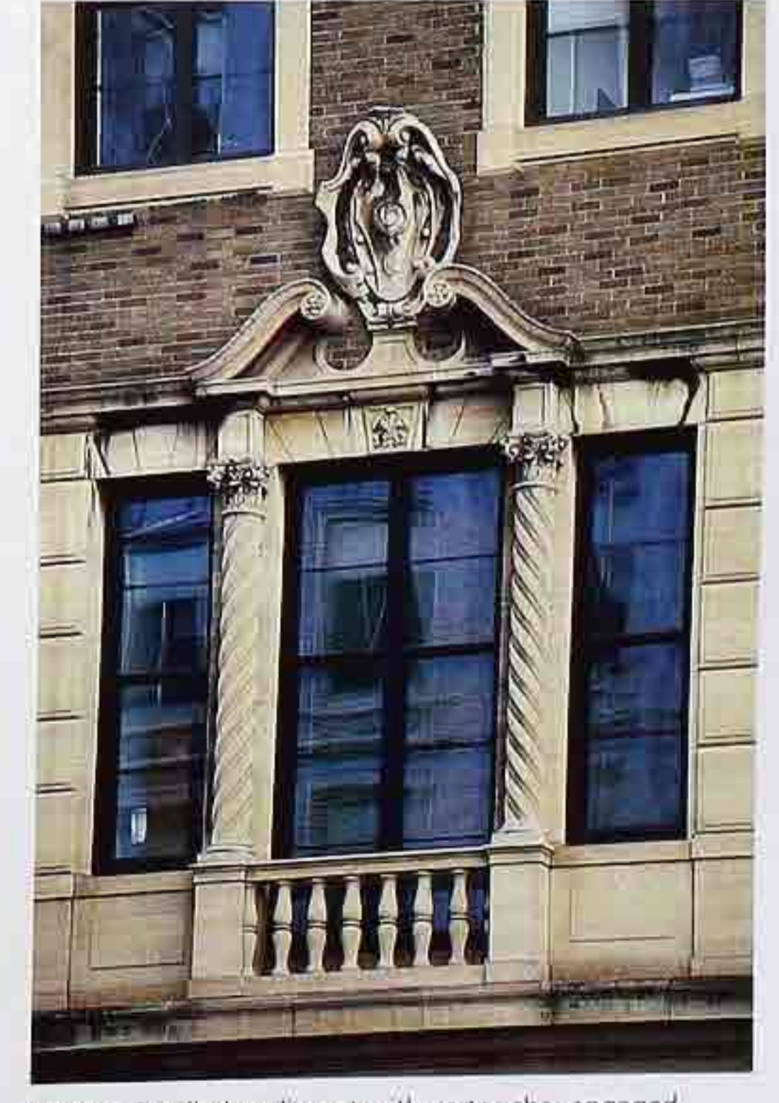
WI-139 Scrolled pediment with cartouche, engaged columns, and balustrade below window with side lights, apartment house
