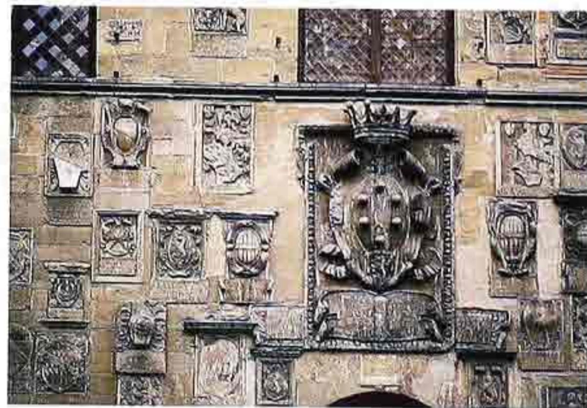
OM-31 Large cartouche surmounted by a crown, with molded frame with crossettes, surrounded by smaller cartouches of similar design
