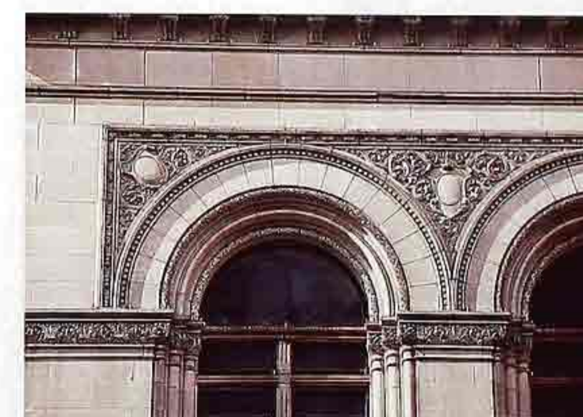
CP-144 Arcade of semicircular compound arches; spandrels with cartouches and foliated ornament
