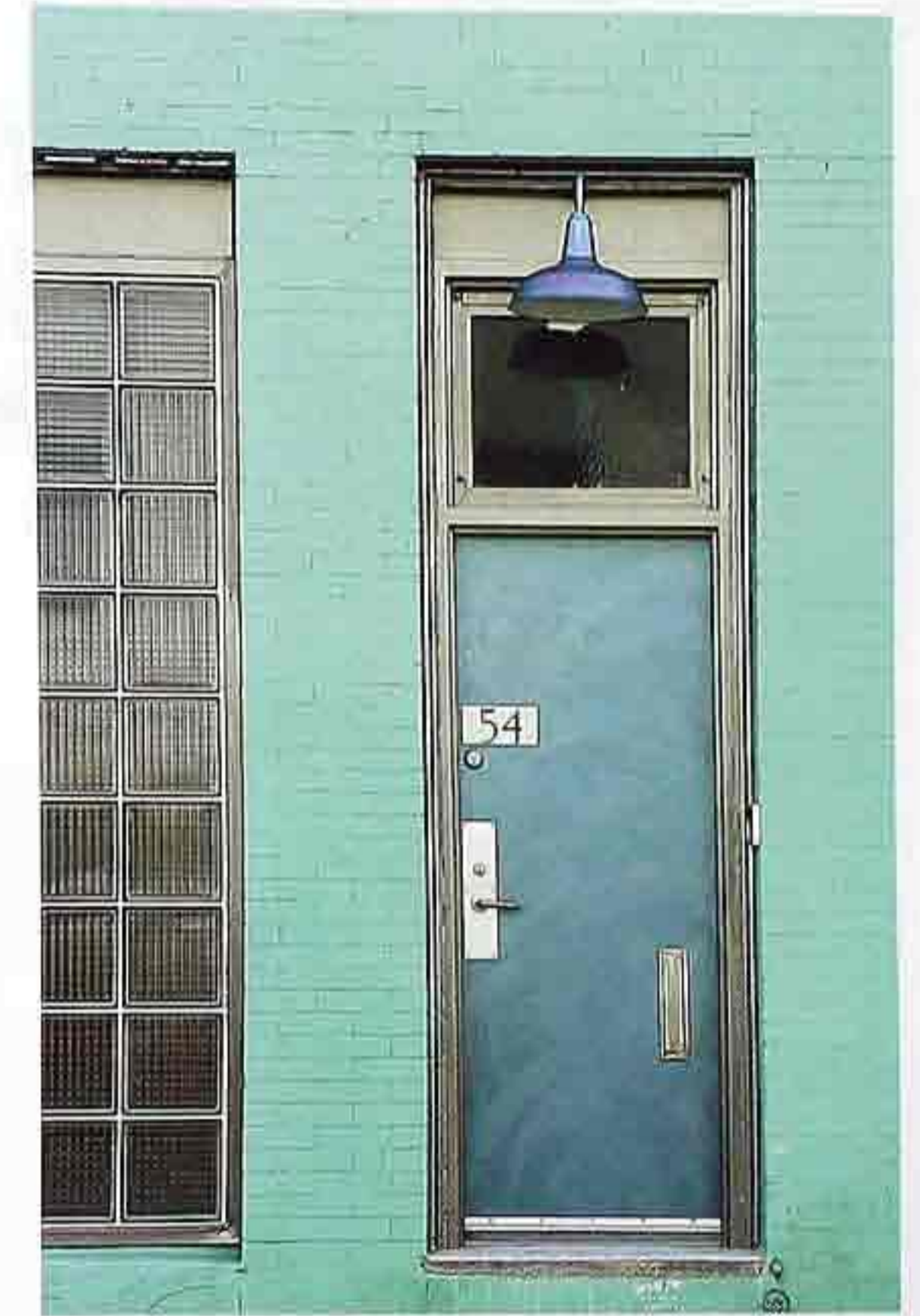
DW-56 Painted metal door with stainless steel hardware; brushed stainless steel doorframe with transom light
