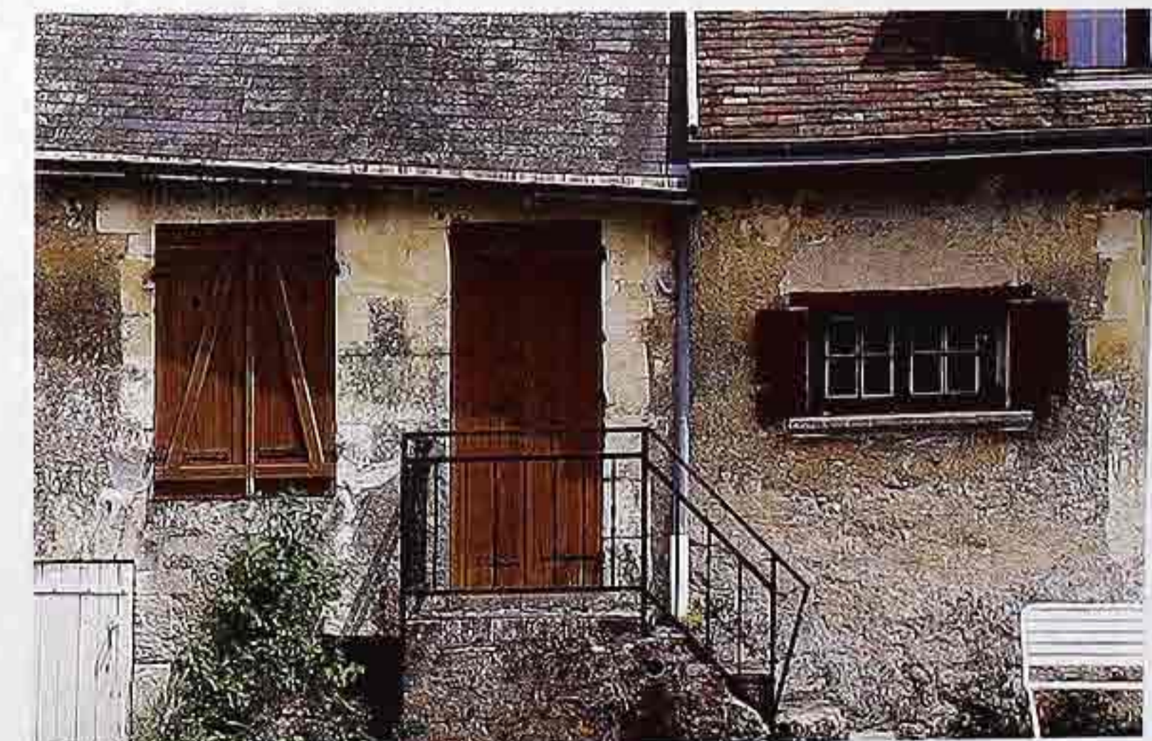
WI-193 Batted shutters and door
