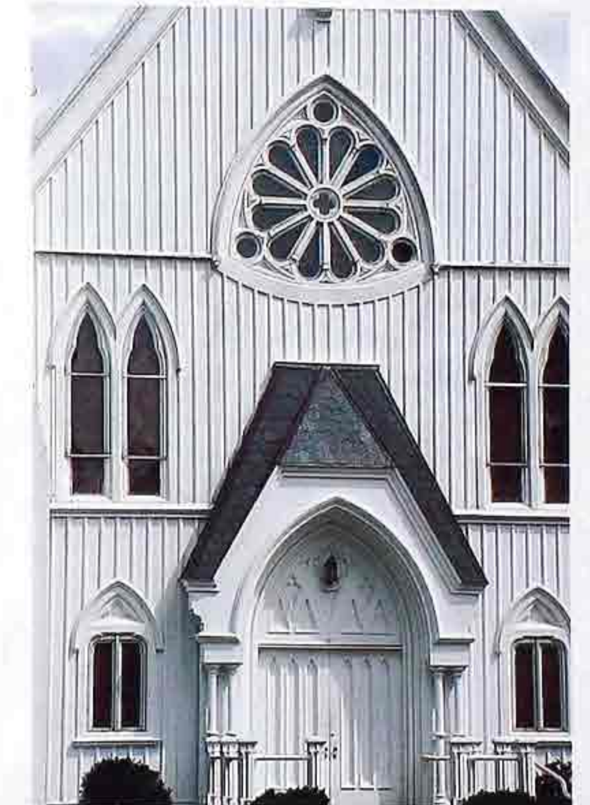
WA-33 Board-and-batten siding with rose window and lancet windows; jerkinhead-roofed entry, Carpenter Gothic church
