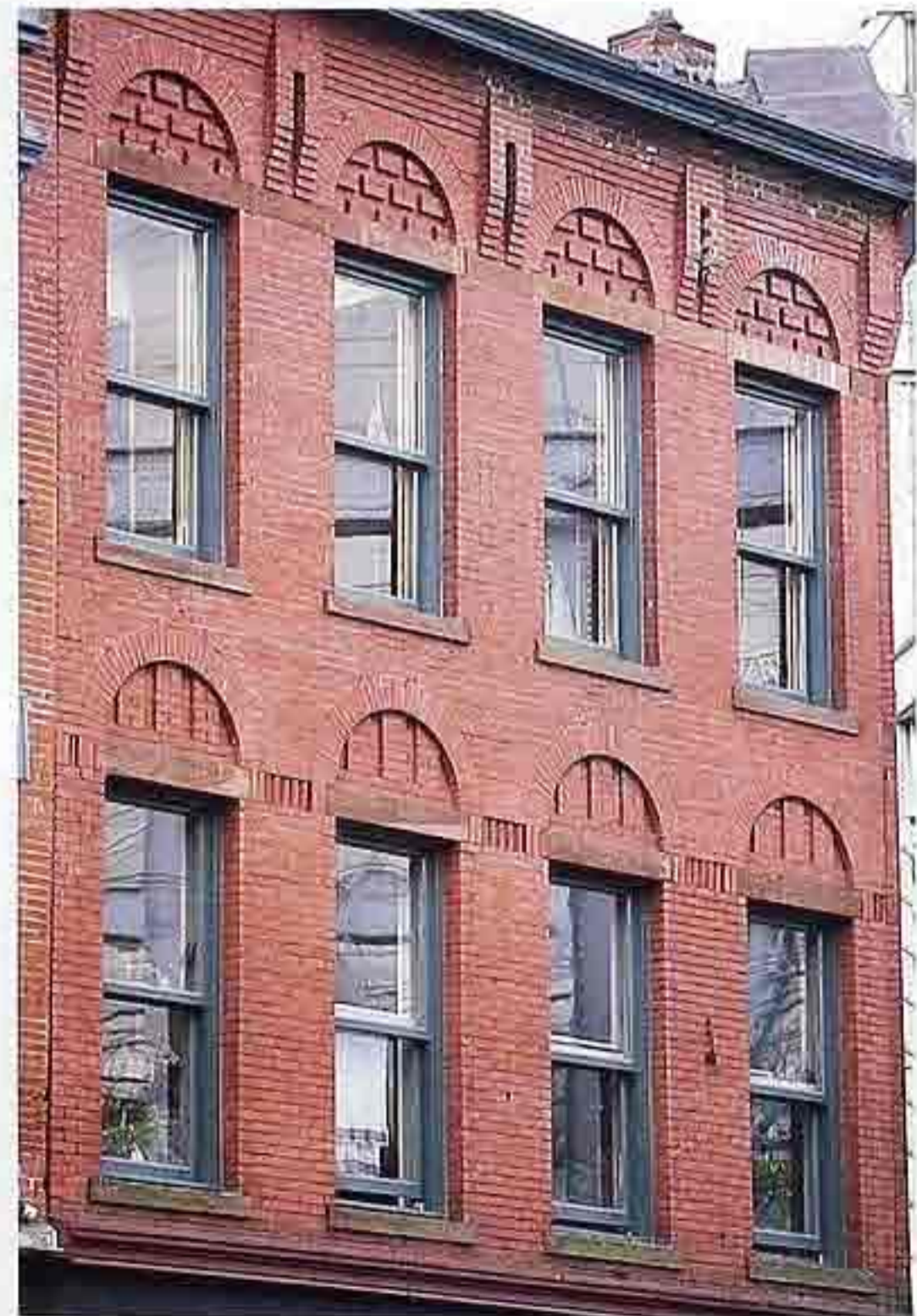
WI-57 One-over-one double-hung metal or vinyl replacement windows, 19th-c. brick apartment building
