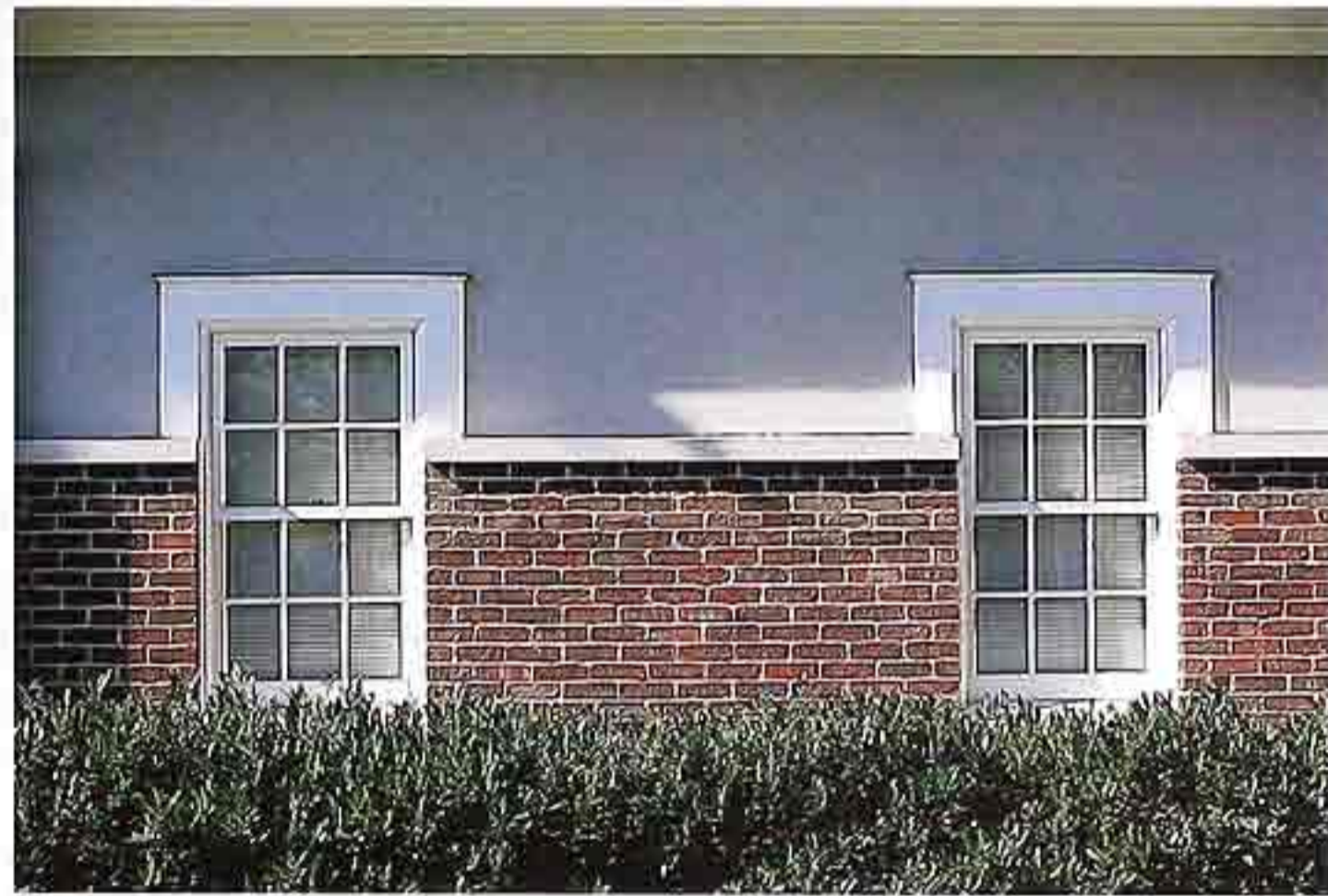
WI-105 Flat wood casing around double-hung windows in stucco and brick wall, traditional house
