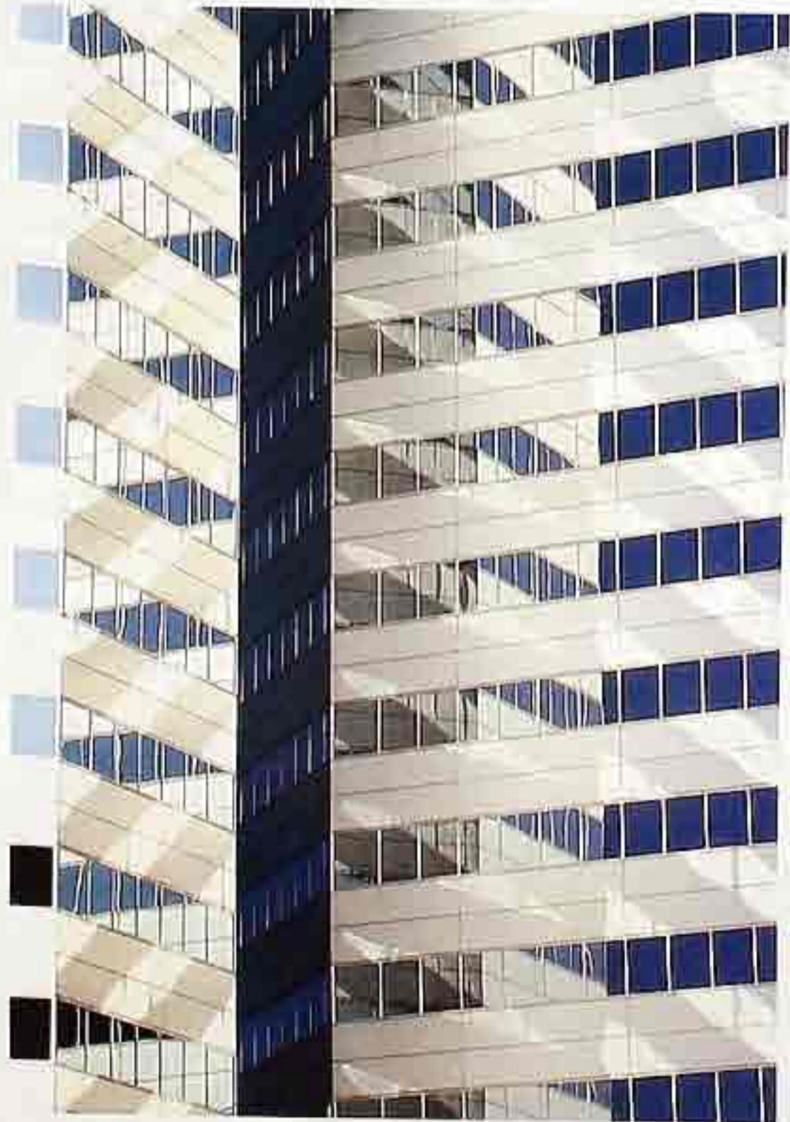
FA-34 Banded curtain wall, alternating mirror glass and solid spandrel panels
