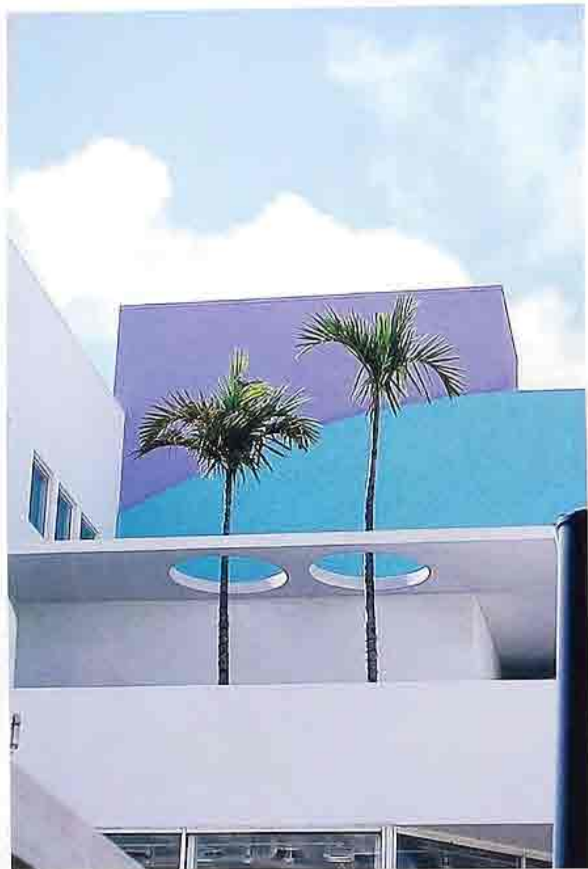
R-140 Flat, punctured roof with projecting eave and palm trees growing through concrete canopy
