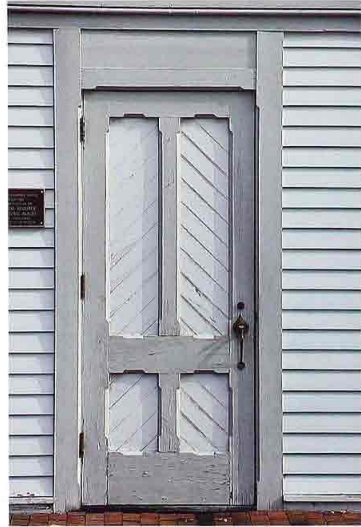
DW-10 Four diagonally planked panels, painted door with wrought-iron handle, clapboard house
