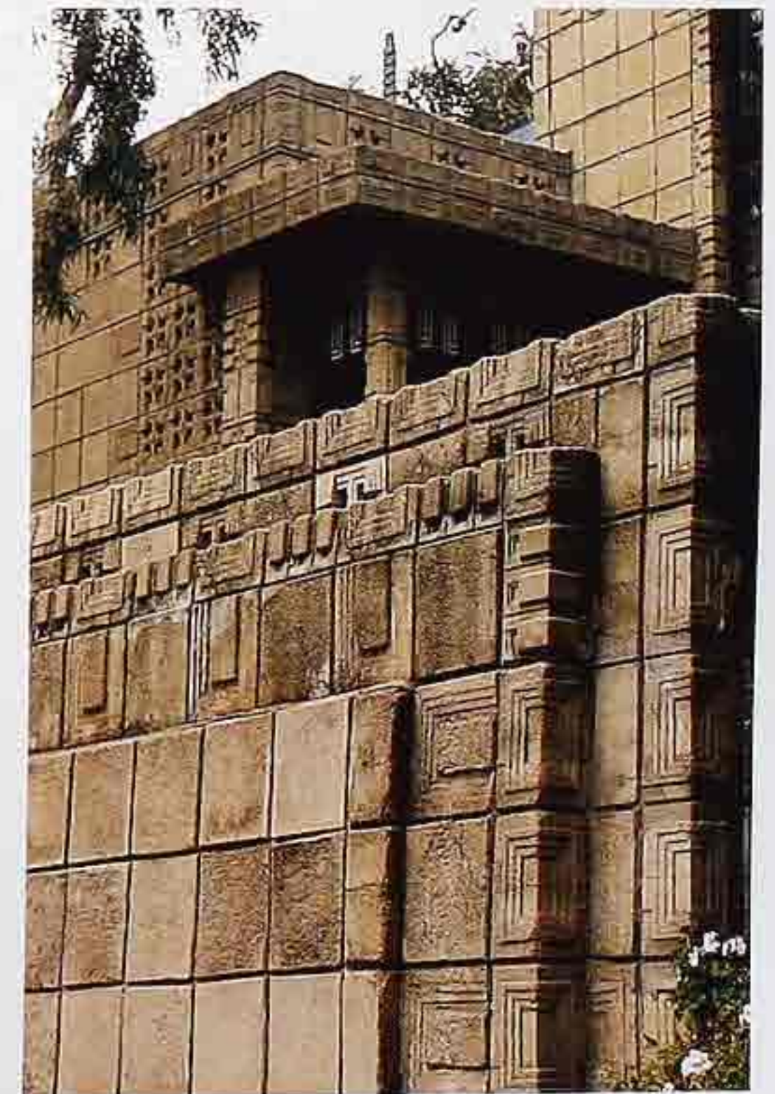
WA-229 Custom concrete blocks with screen wall (top), residential entryway
