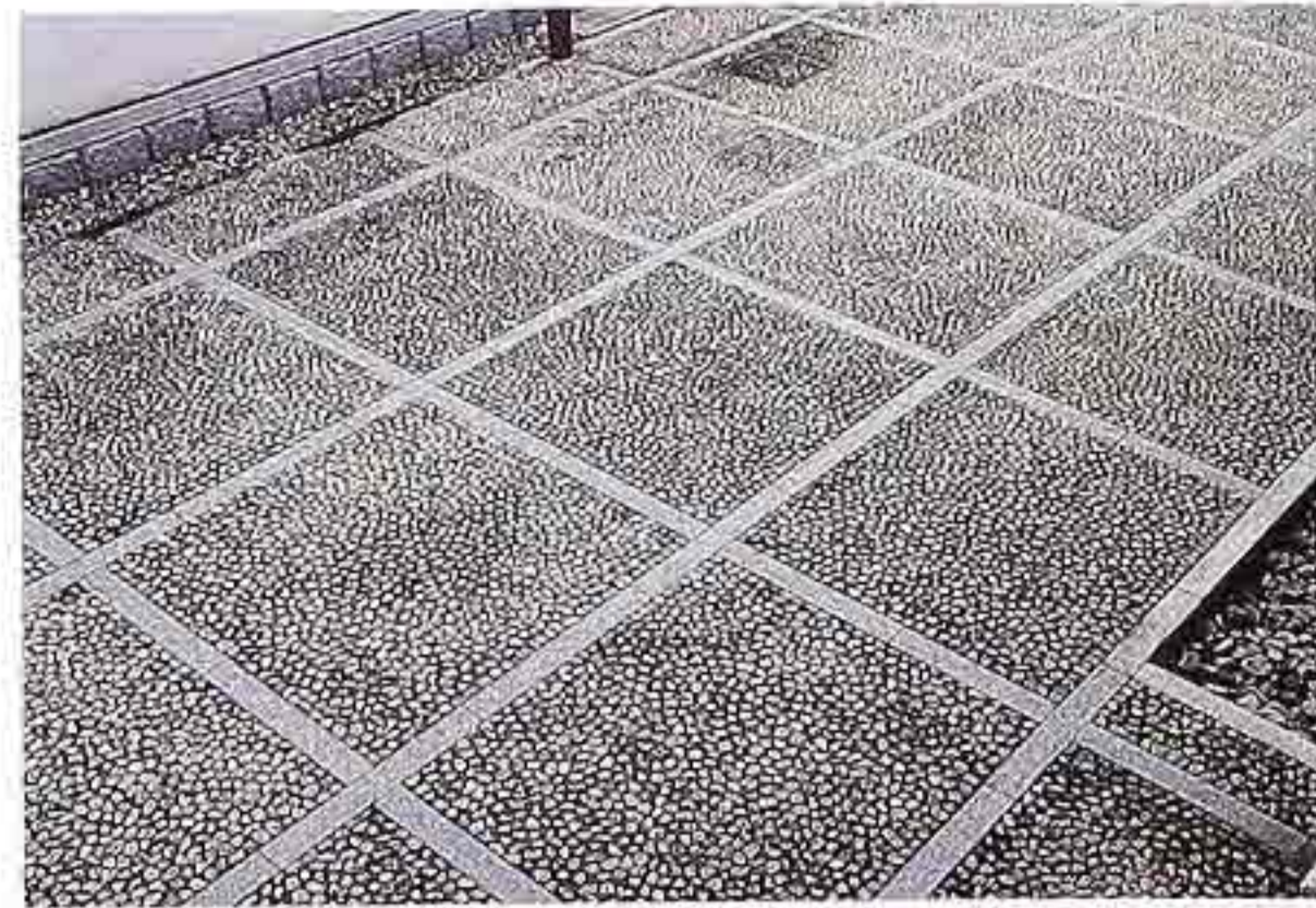
FP-73 Squares of exposed aggregate (possibly pre-cast) separated by metal or concrete grid in courtyard of modern commercial building
