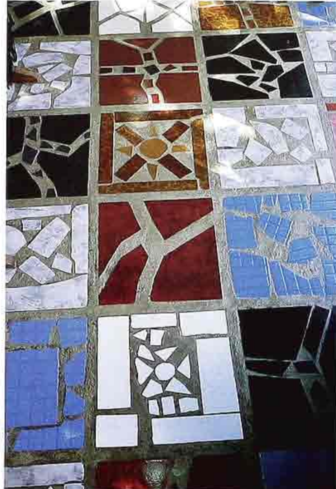
FP-104 Random-shaped tile pieces used as tesserae in mosaic grid design set in concrete
