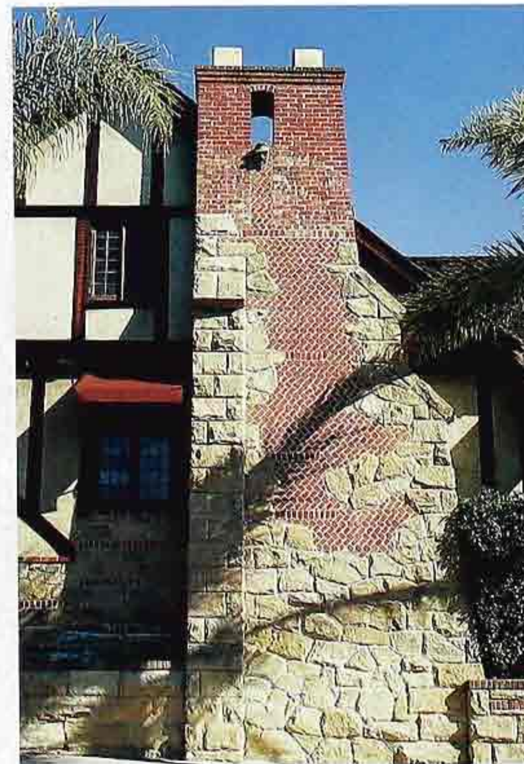
CR-150 Chimney: coursed-ashlar buttress and random ashlar stonework, herringbone brick
