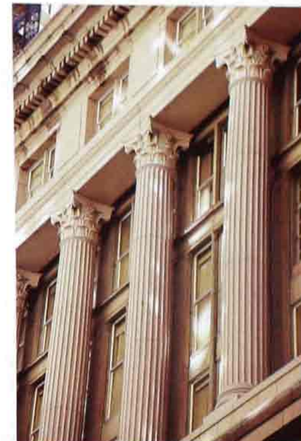
CP-70 Corinthian columns with fluted shafts
