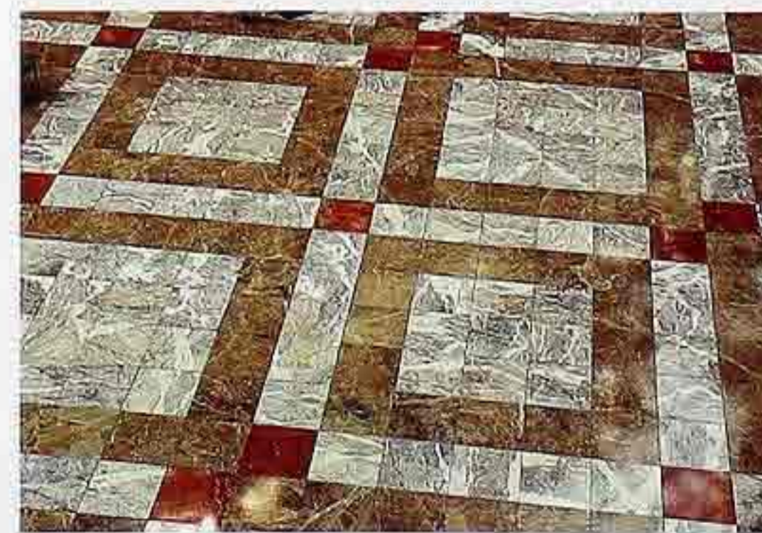
FP-17 Marble parquet in polychrome geometric pattern, interior of modern commercial building
