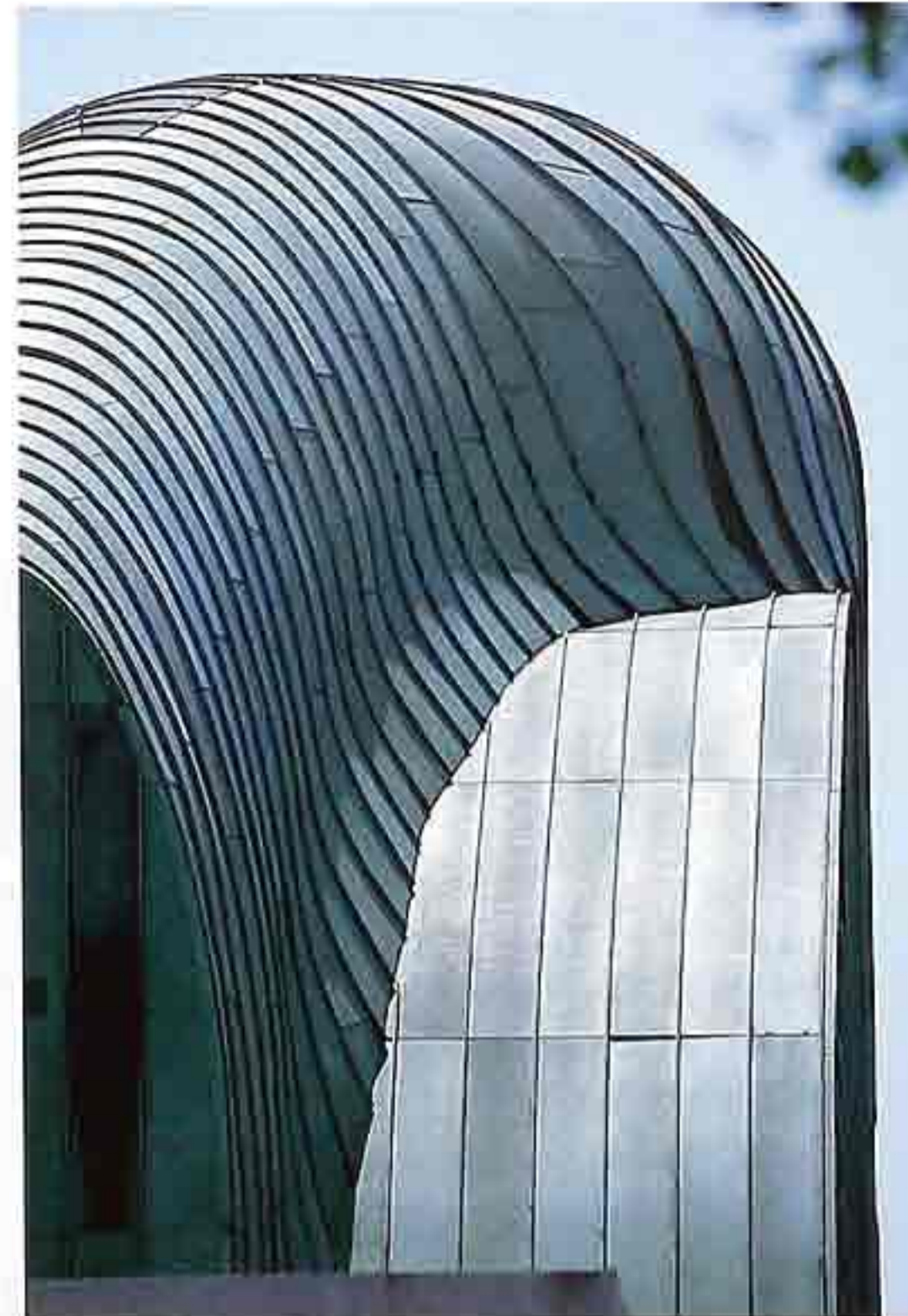
CR-22 Zinc or copper with flat seams, modern commercial building
