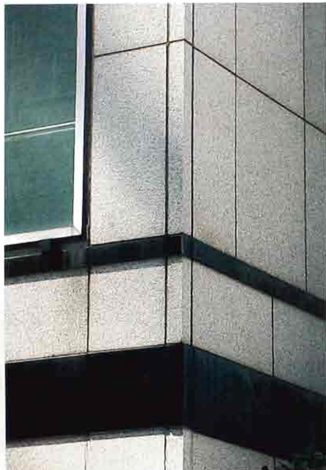
WA-131 Outside corner of granite veneer with raked joints; belt courses at window and jetty, modern commercial building
