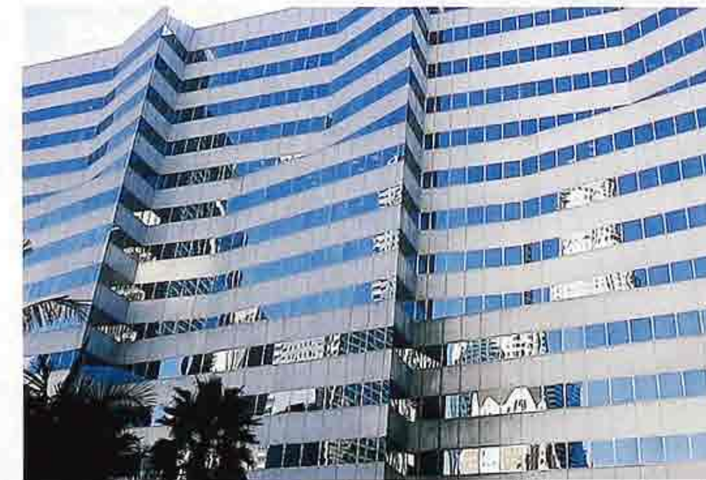
FA-30 Banded curtain wall, alternating mirror glass and solid spandrel panels
