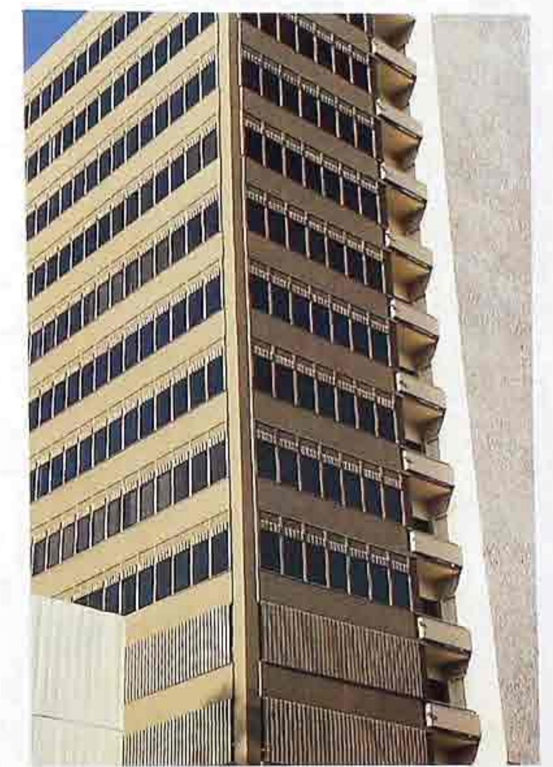
WA-303 Concrete building with metal trim
