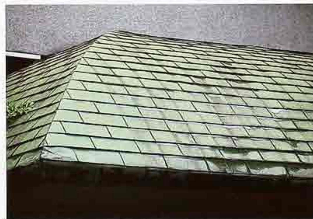
CR-23 Copper shingles on curved hipped roof
