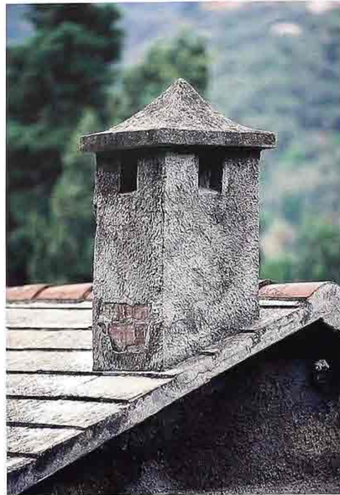
CR-148 Stucco-over-brick chimney with pyramidal hood
