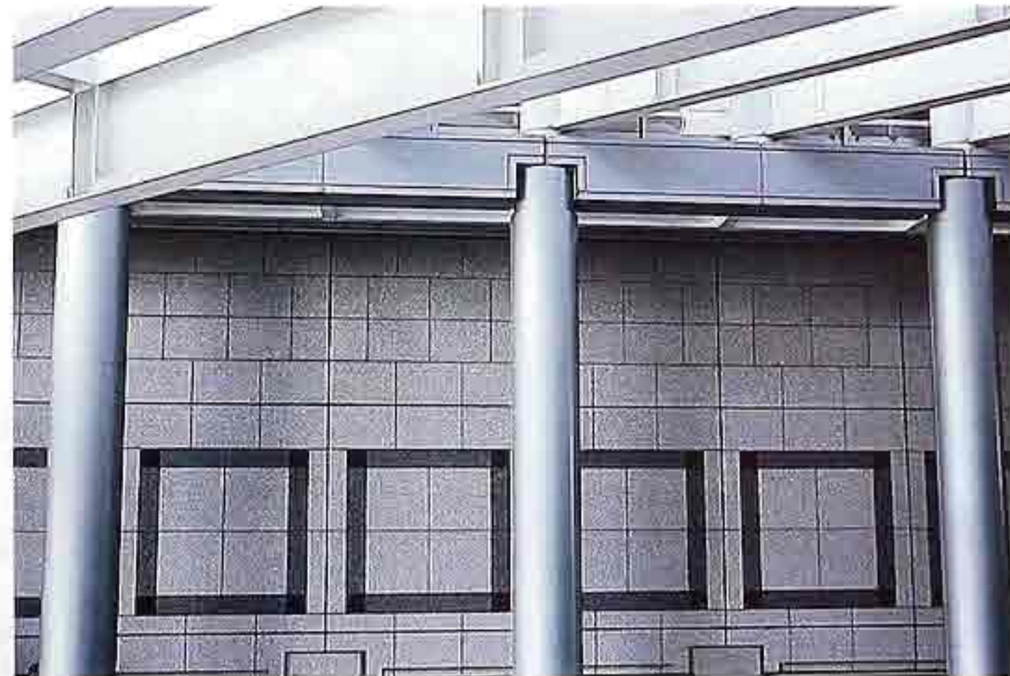
CP-138 Steel frame with metal-clad column and beam beneath exposed riveted plate girders, modern commercial building
