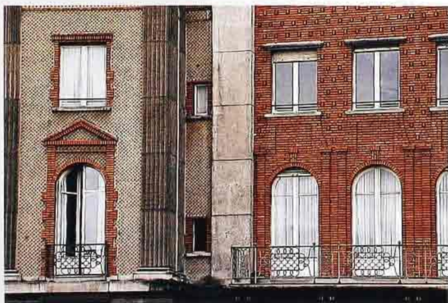
WA-207 Decorative brickwork. Left to right: square brick or tile in diagonal pattern with brick window ornament; projecting ornament over stacked bond pilasters, 19th-c. French apartment house
