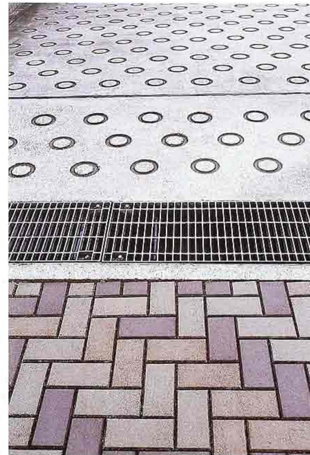
FP-78 Top to bottom: circle diaper pattern stamped in concrete; metal grate drain cover; pre-cast polychrome concrete pavers in herringbone pattern
