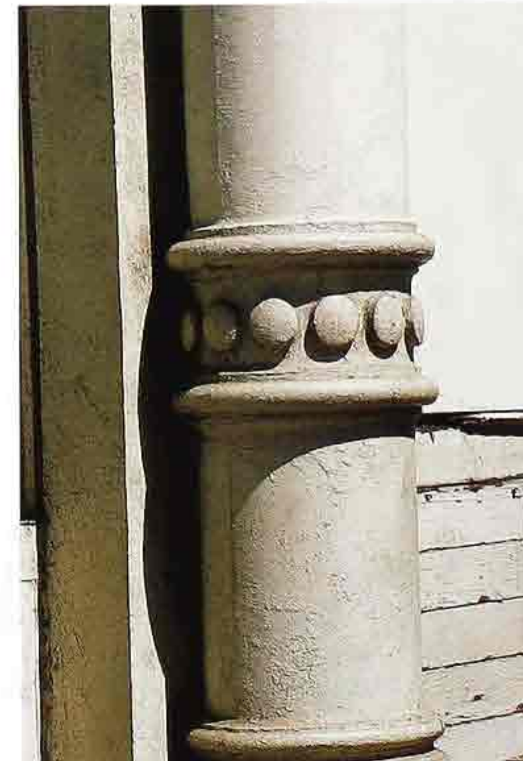
CP-63 Cast-iron column with Doric/Tuscan base and a band of round ornaments on round pedestal with Attic base
