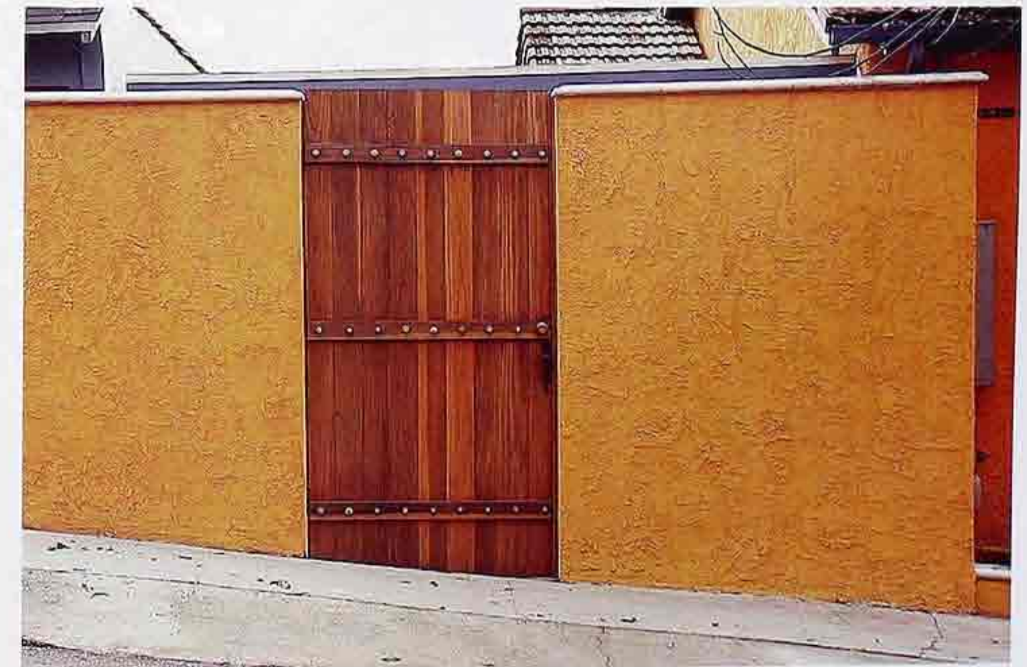
DW-29 Stained wood courtyard gate with horizontal braces, set in painted stucco wall
