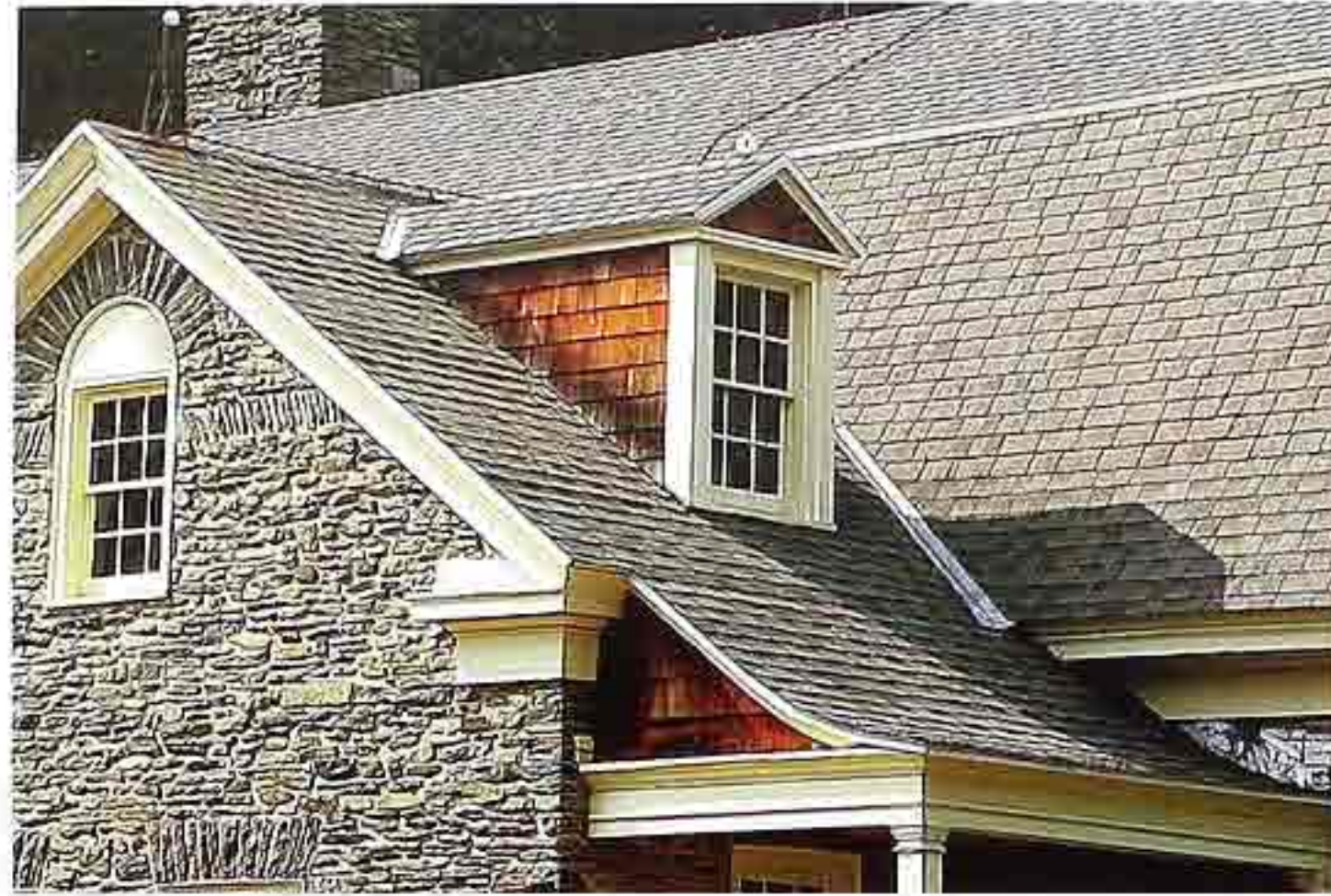
CR-86 Shingled roof dormer above flared eave covering porch; stone gable-end wall
