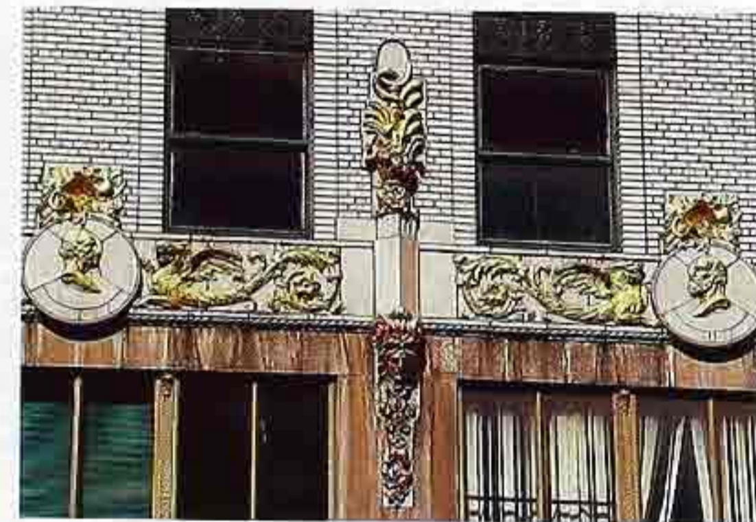
OM-49 Gilded ornament: large medallions, foliated band, bracket with a mascarons, and central finial
