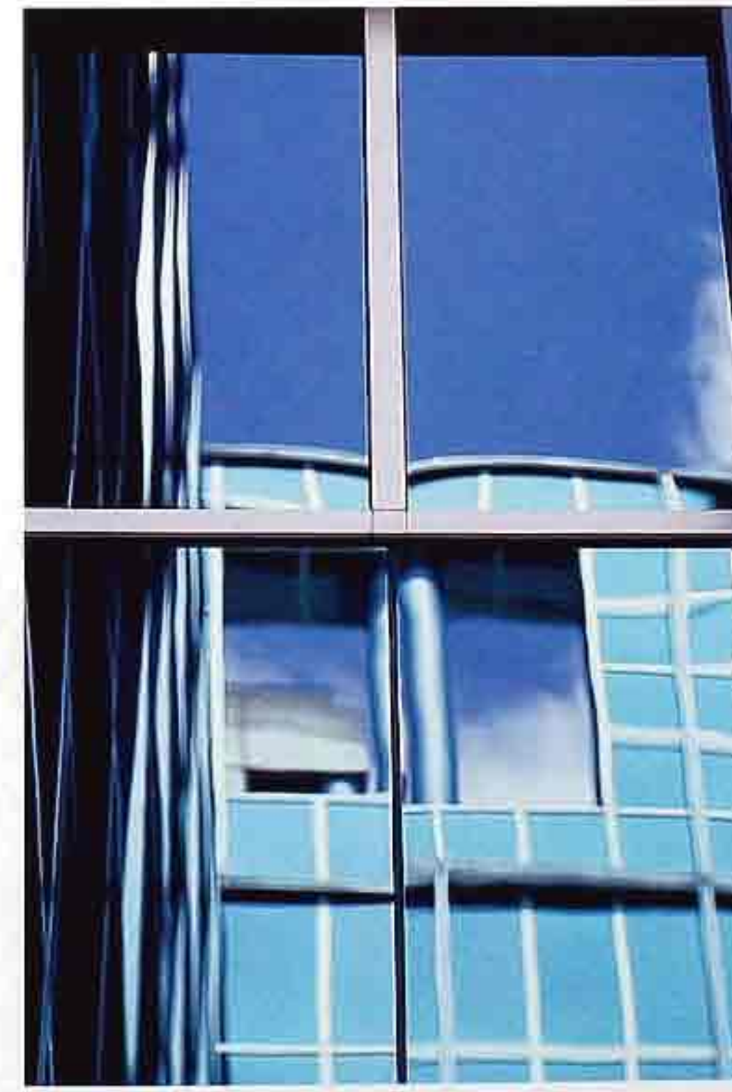
WI-7 Stainless steel muntins, modern commercial building
