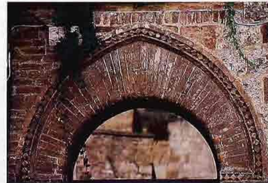
CP-154 Florentine arch (extrados and intrados not concentric), gauged brick. Extrados emphasized with a molding
