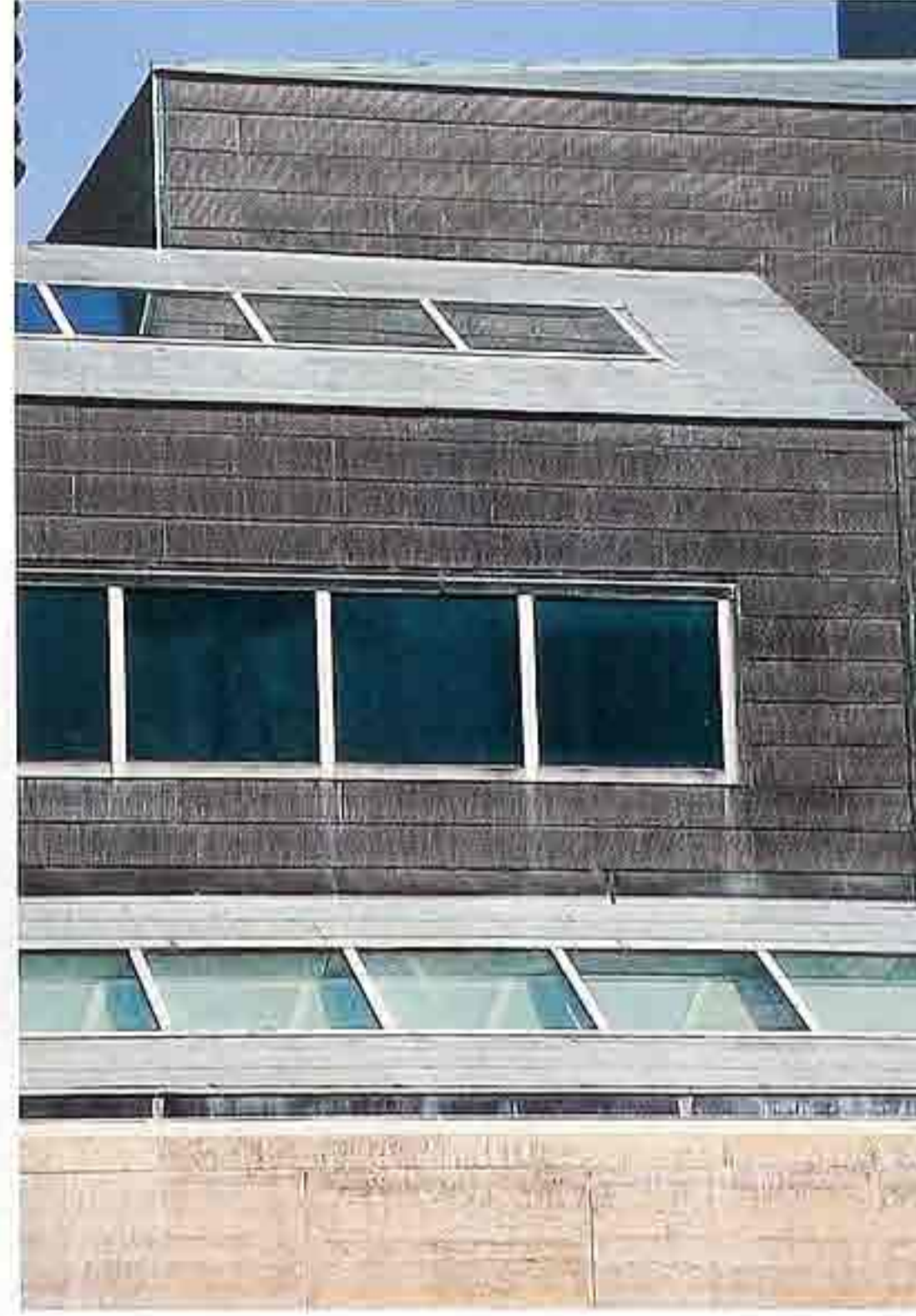
FA-12 Corrugated metal patinated shingles surrounding strip windows and skylights
