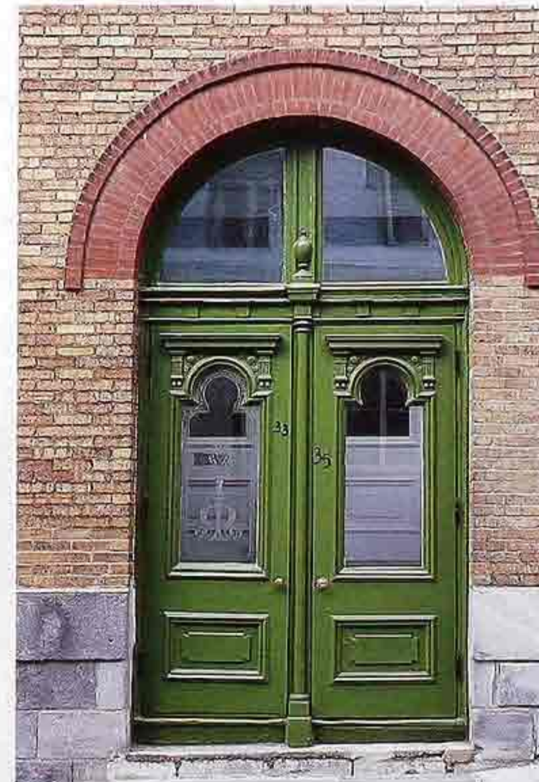
DW-21 Wood double doors with glass upper panels and flush-molded lower panels; split transom light in segment
