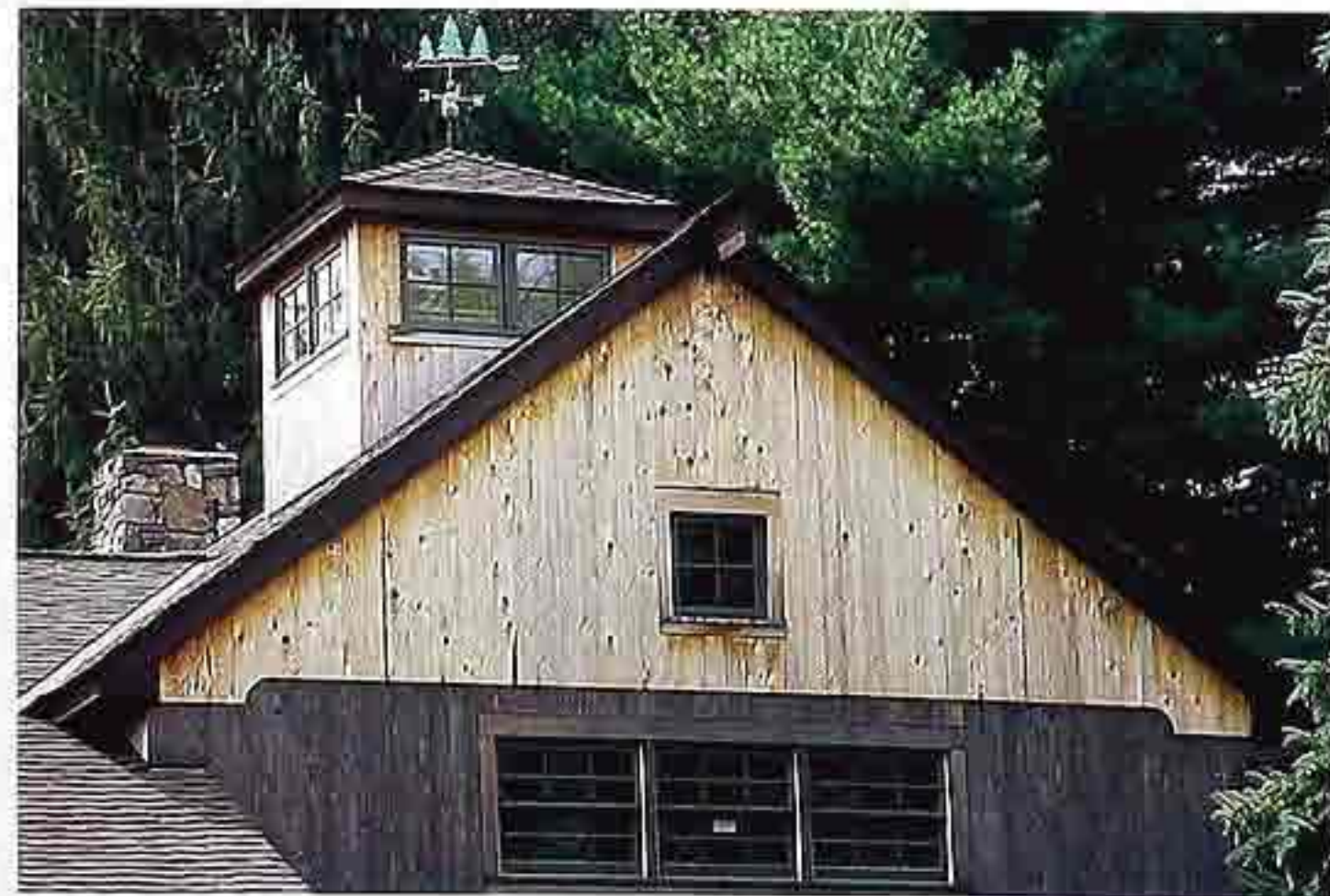
CR-88 Gable-end wall with new flush board siding above weathered siding; glazed monitor with pyramidal roof
