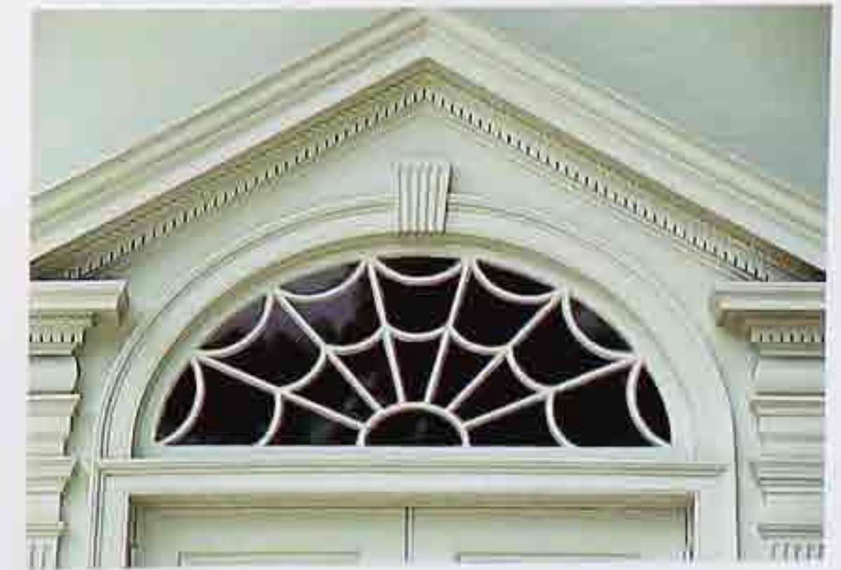
WI-103 Bat-wing fanlight under pediment
