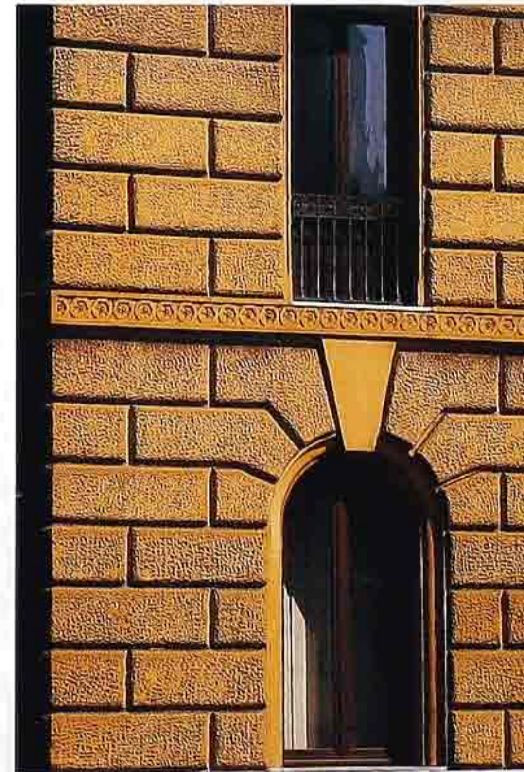
WA-112 Rusticated running bond with hand-tooled finish; sand-finish keystone; crossettes; carved ornamented belt course
