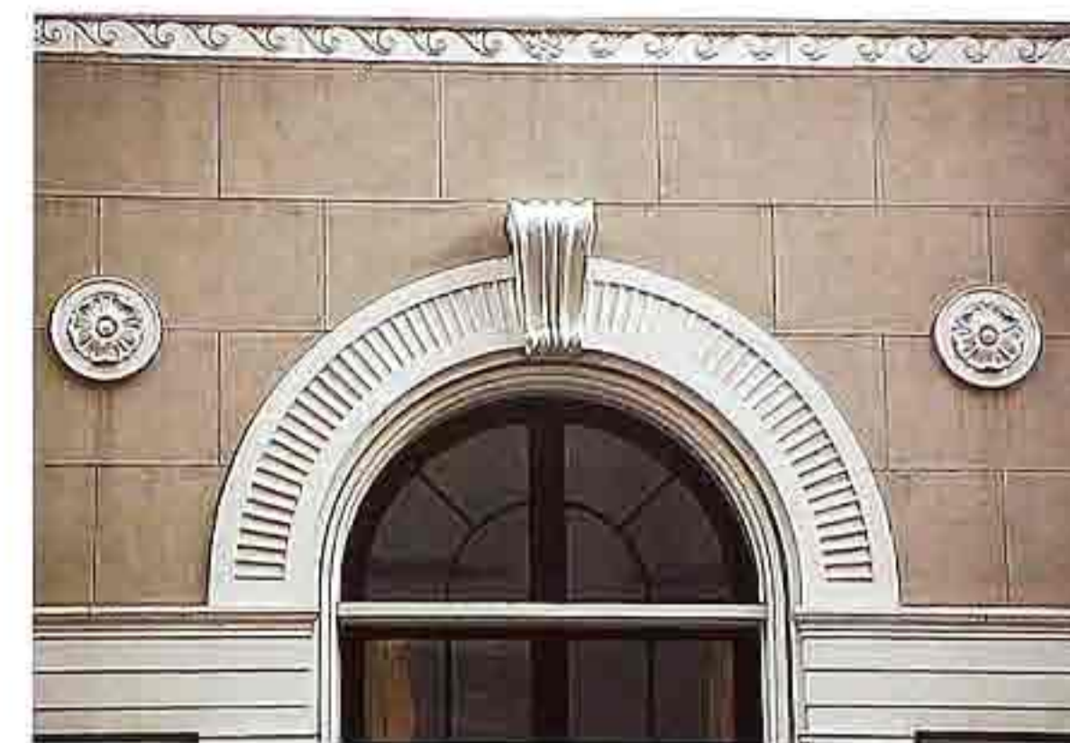
CP-141 Semicircular arch with an ancon keystone on masonry running-bond wall with Vitruvian scroll trim and rosette medallions
