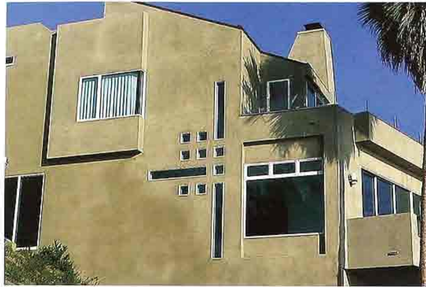
WI-73 Geometric fixed windows, modern house
