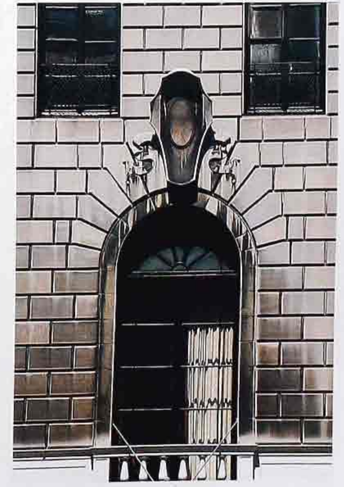
WA-113 Weathered sand-finish limestone in running bond, with cartouche keystone in stepped arch
