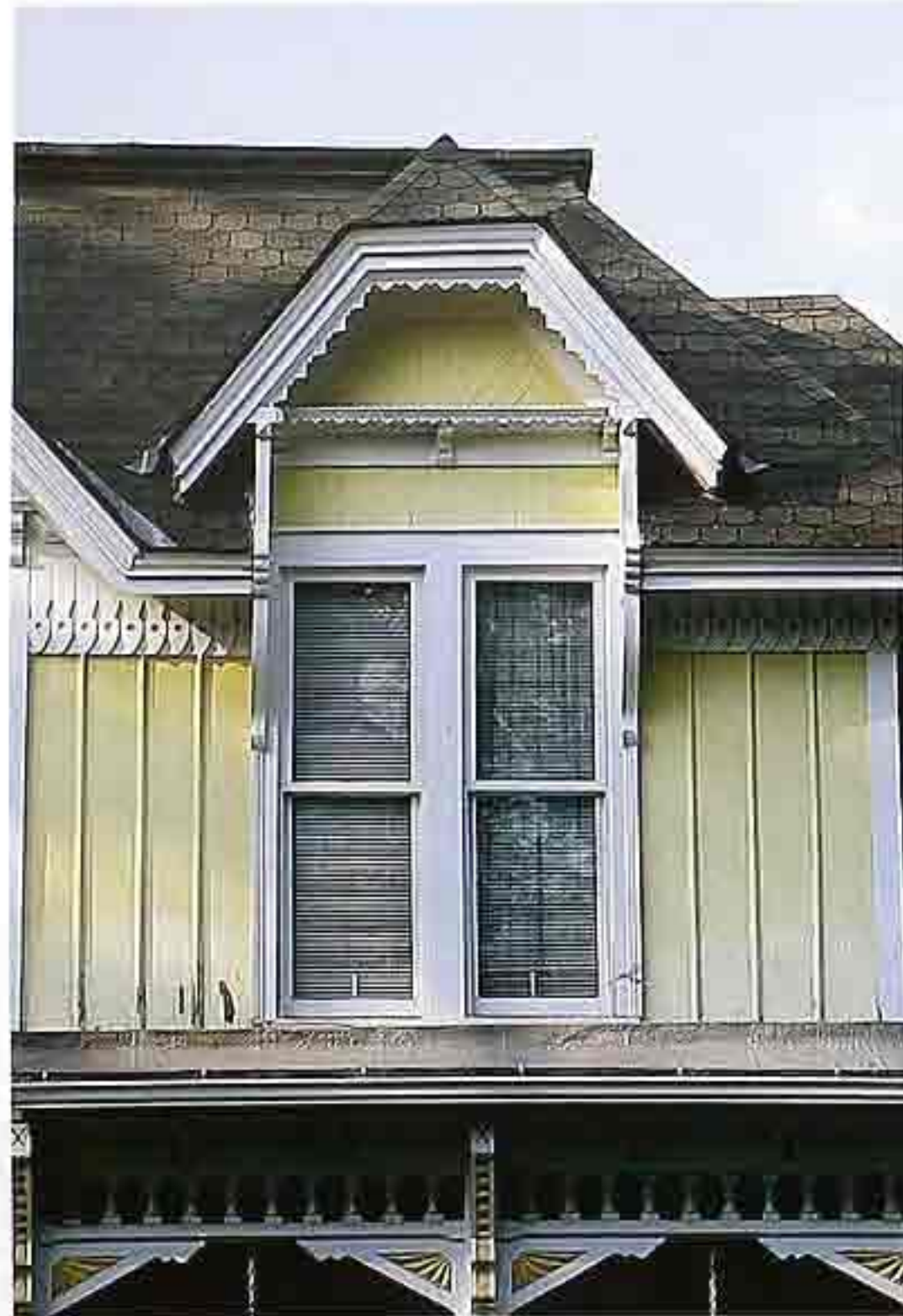
CR-76 Wall dormer with jerkinhead roof
