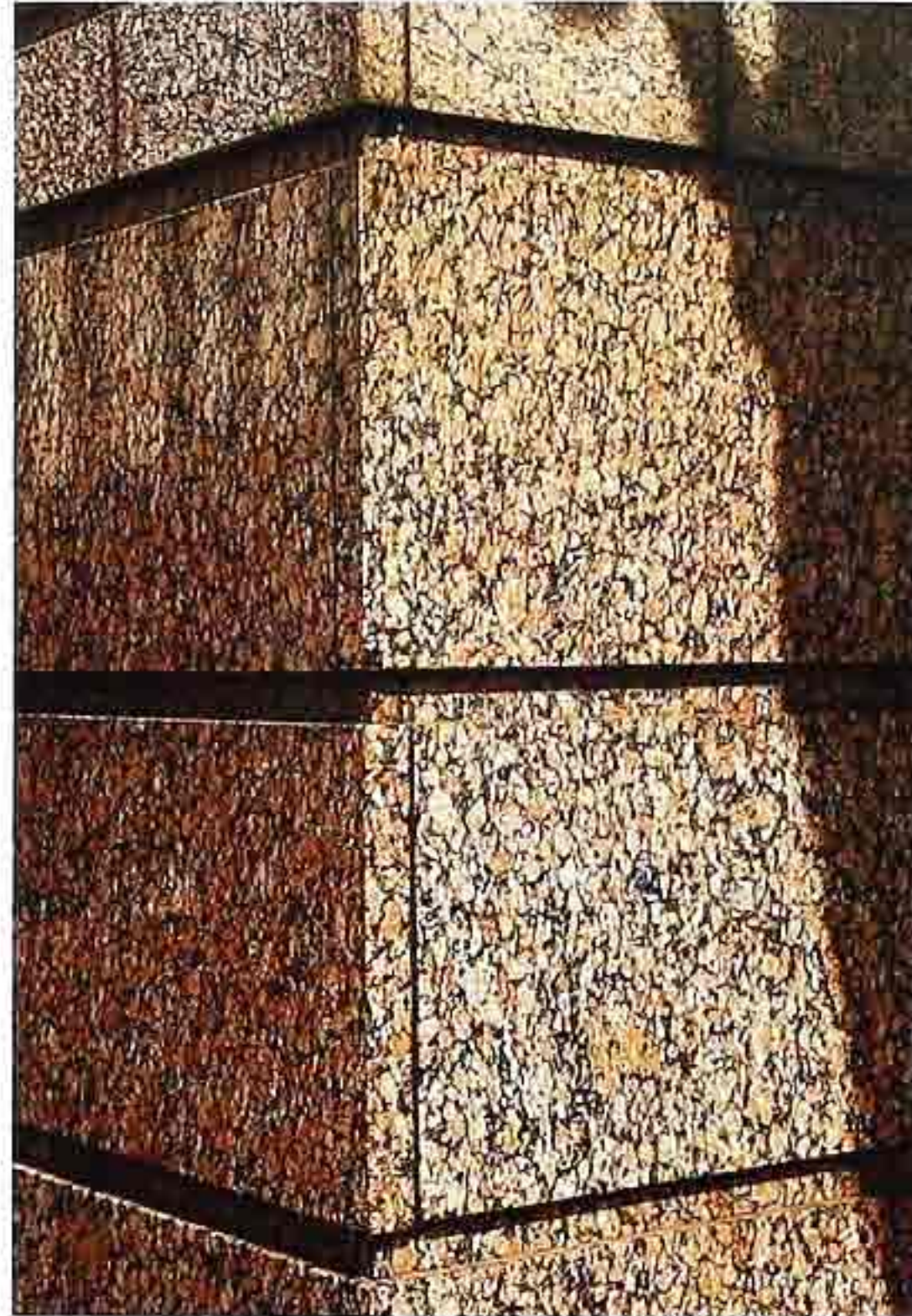
WA-83 Corner detail of polished granite veneer with lapped corner joints
