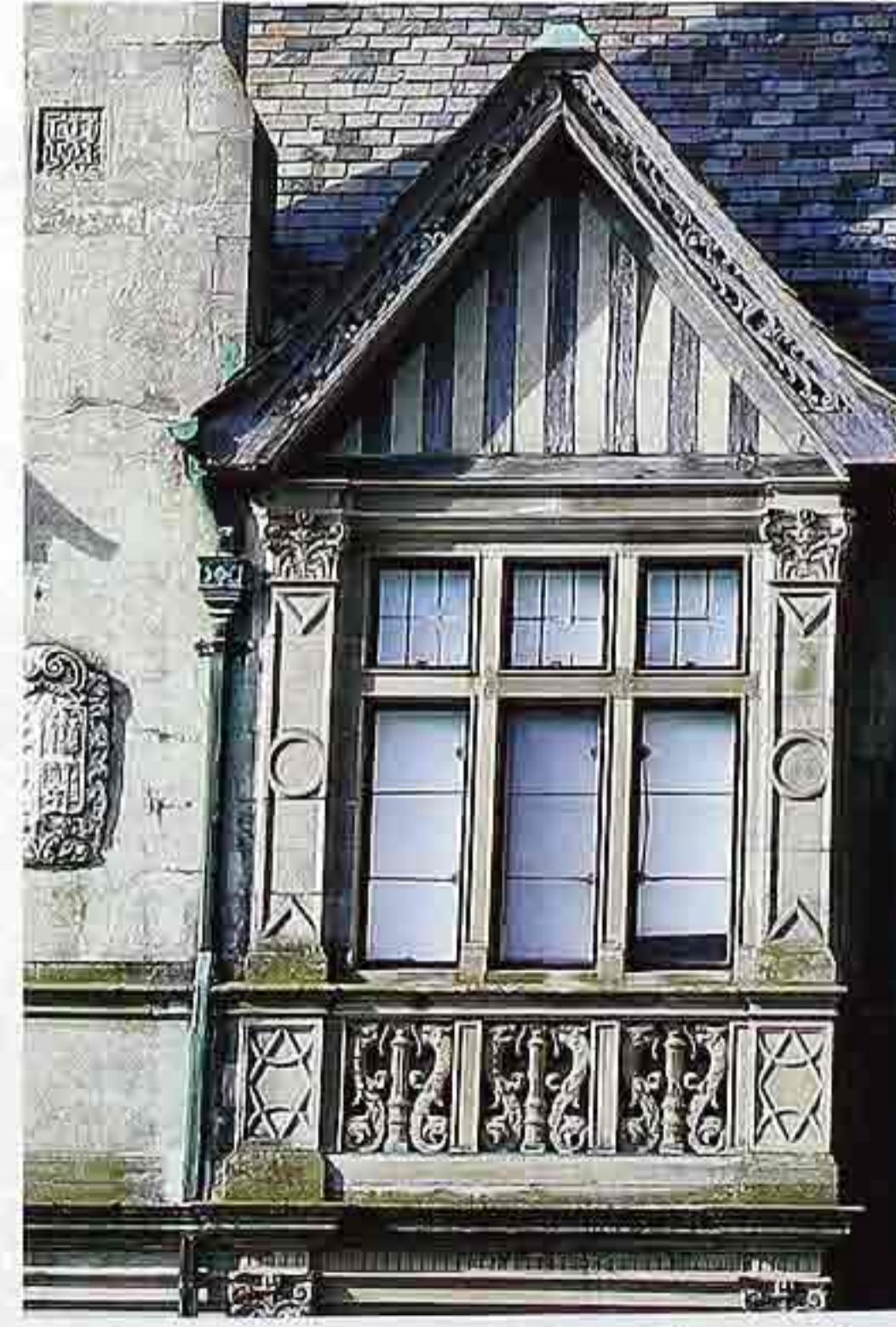
WI-138 Set of three dormer windows with stone casing flanked by pilasters in half-timber-style gable with engaged balustrade
