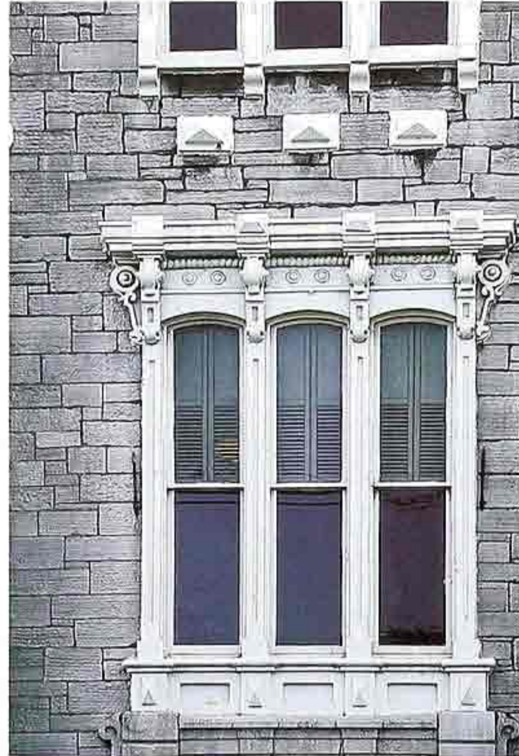
WI-112 Ornament and molding around group of three double-hung windows; consoles supporting cornice, 19th-c. American stone commercial building
