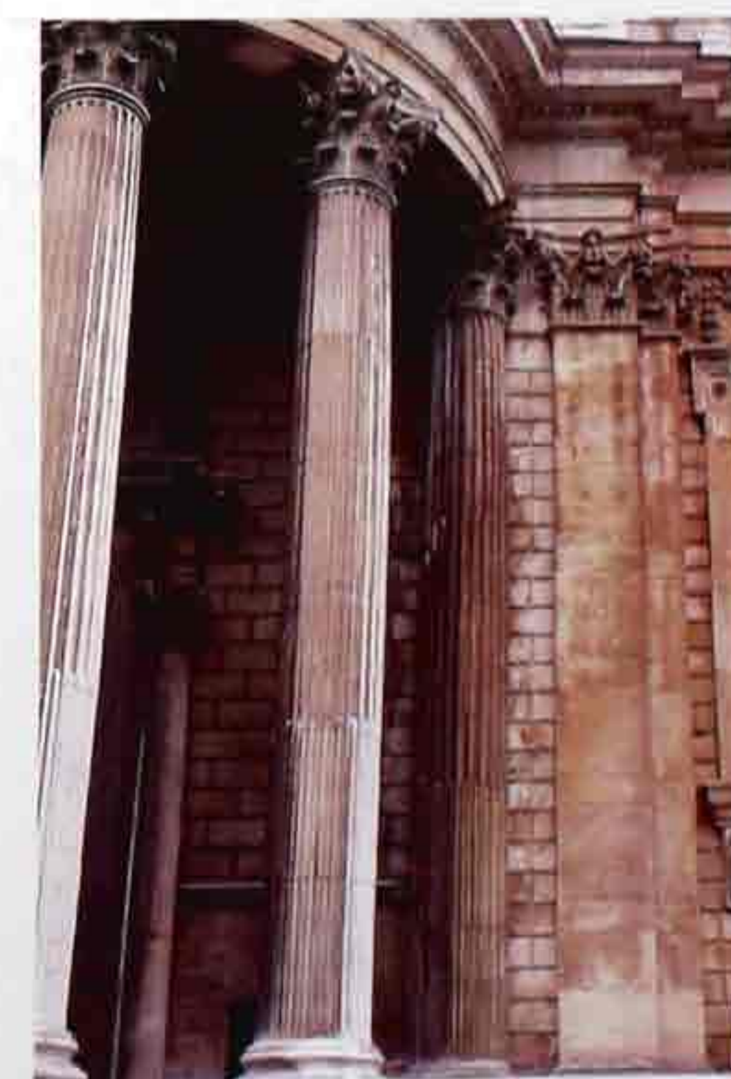
CP-72 Corinthian columns with partially fluted shafts next to flat pilasters
