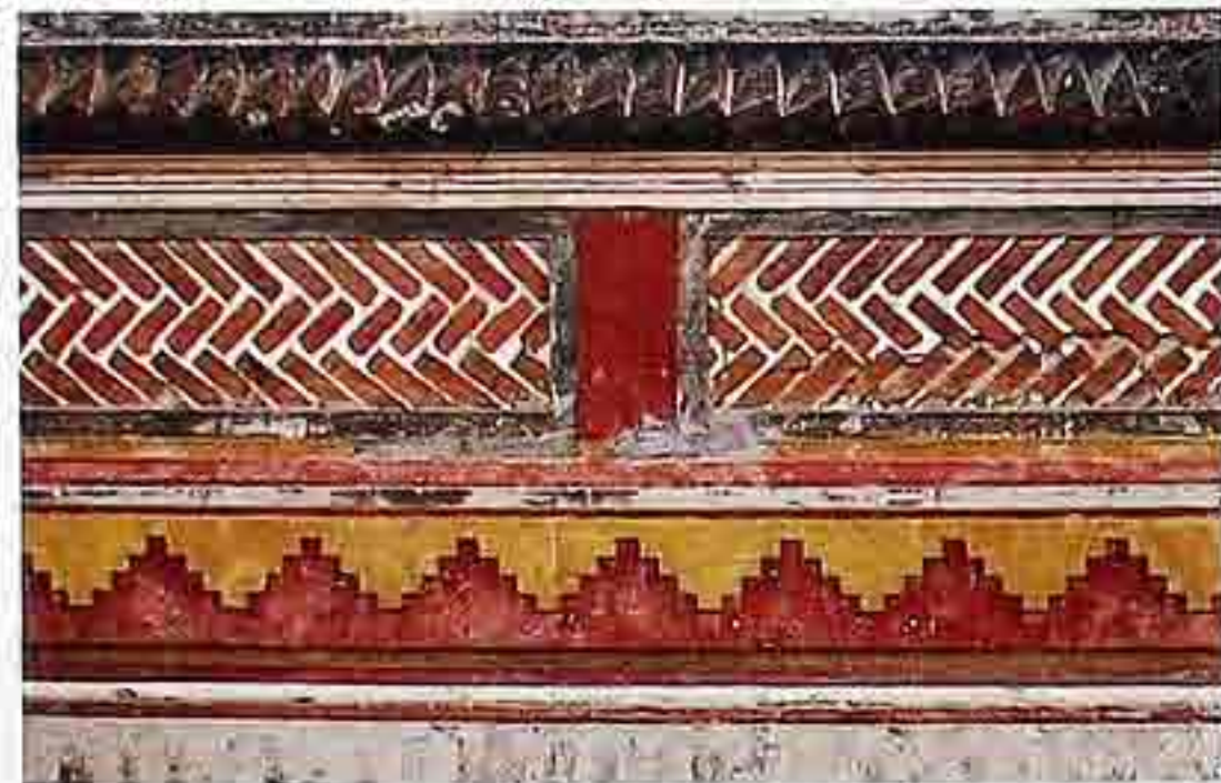
WA-266 Courtyard wall. Top to bottom: cast-concrete coping; saw-tooth brick course; light-colored stone, herringbone-bond brick in concrete frame; painted brick; stone base
