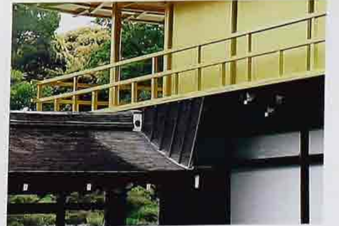
CR-114 Eave of shed roof connected to balcony to shelter courtyard walkway, traditional Japanese house
