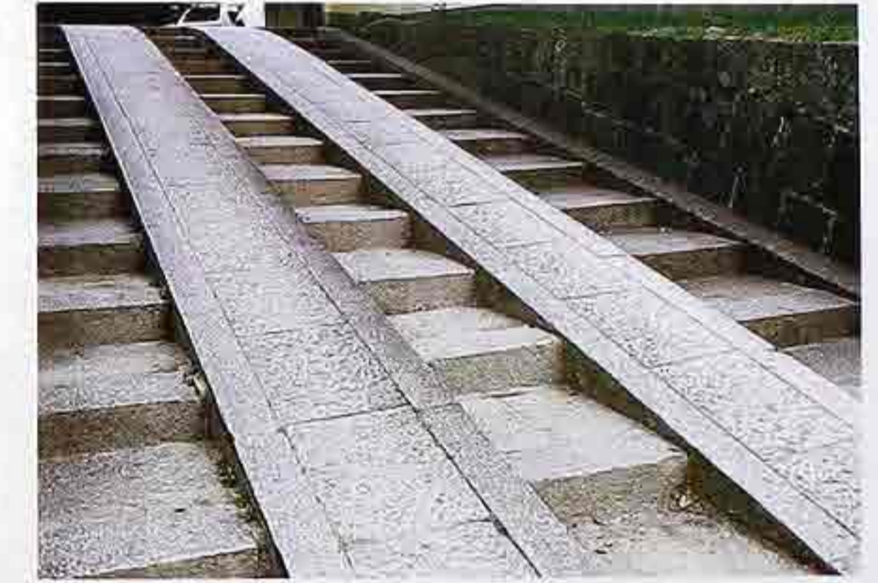
FP-26 Stone stairway divided by stone ramps, urban public space
