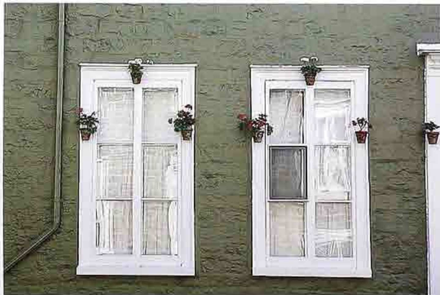
WI-106 Flat wood casing around double-casement windows
