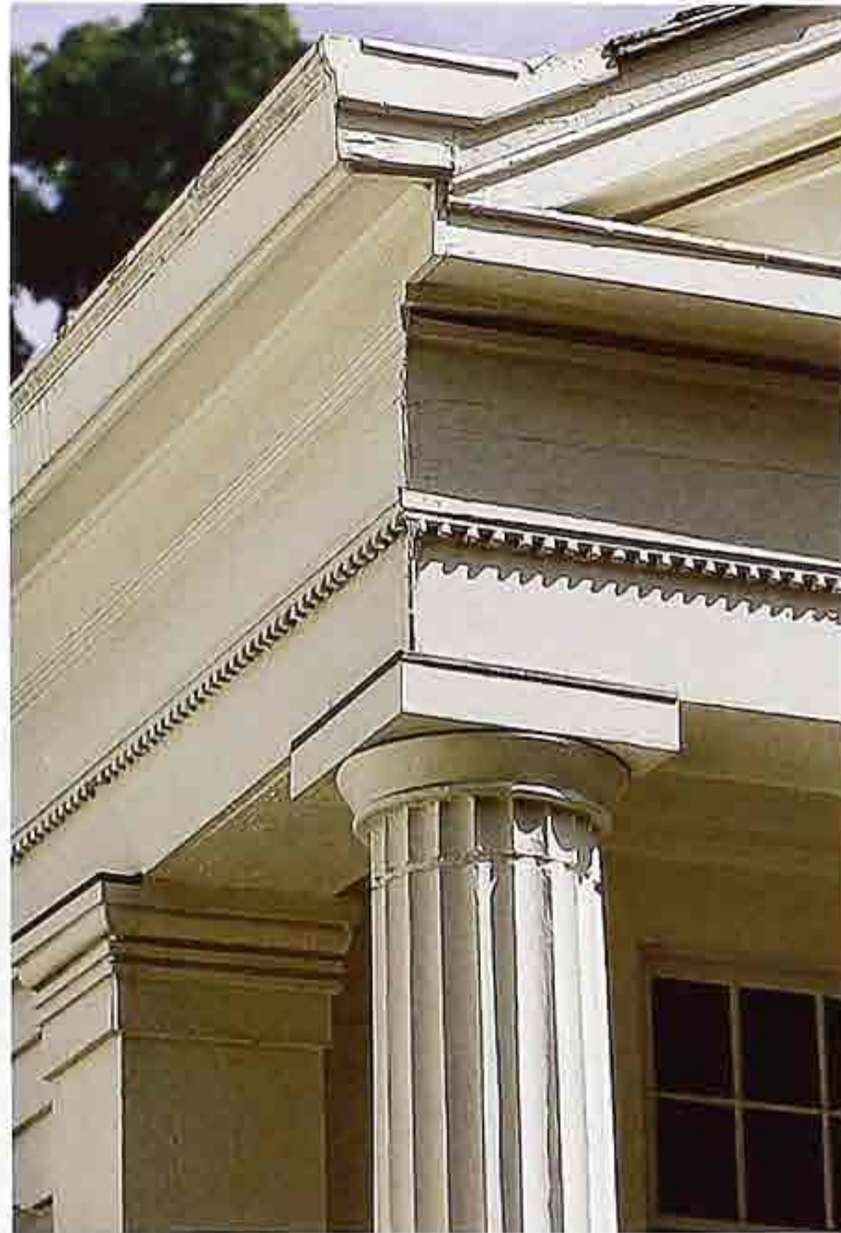
CP-11 Doric capital with Roman proportions; characteristic Greek groove replacing astragal molding
