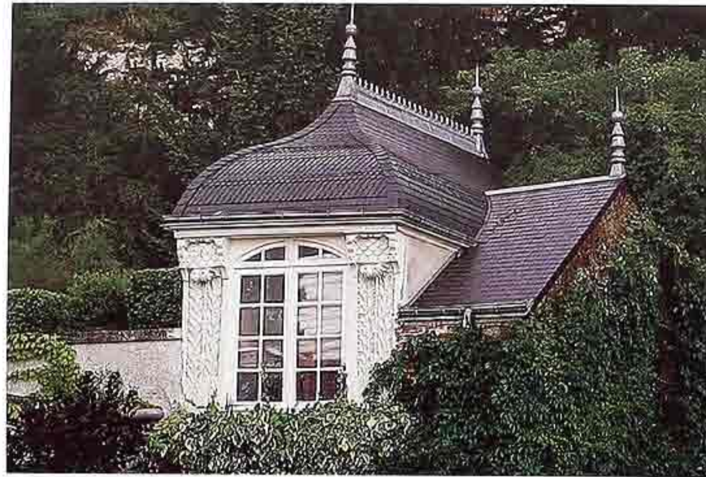
CR-134 Ogee slate roof adjacent to gable roof, both with metal ridge ornamentation
