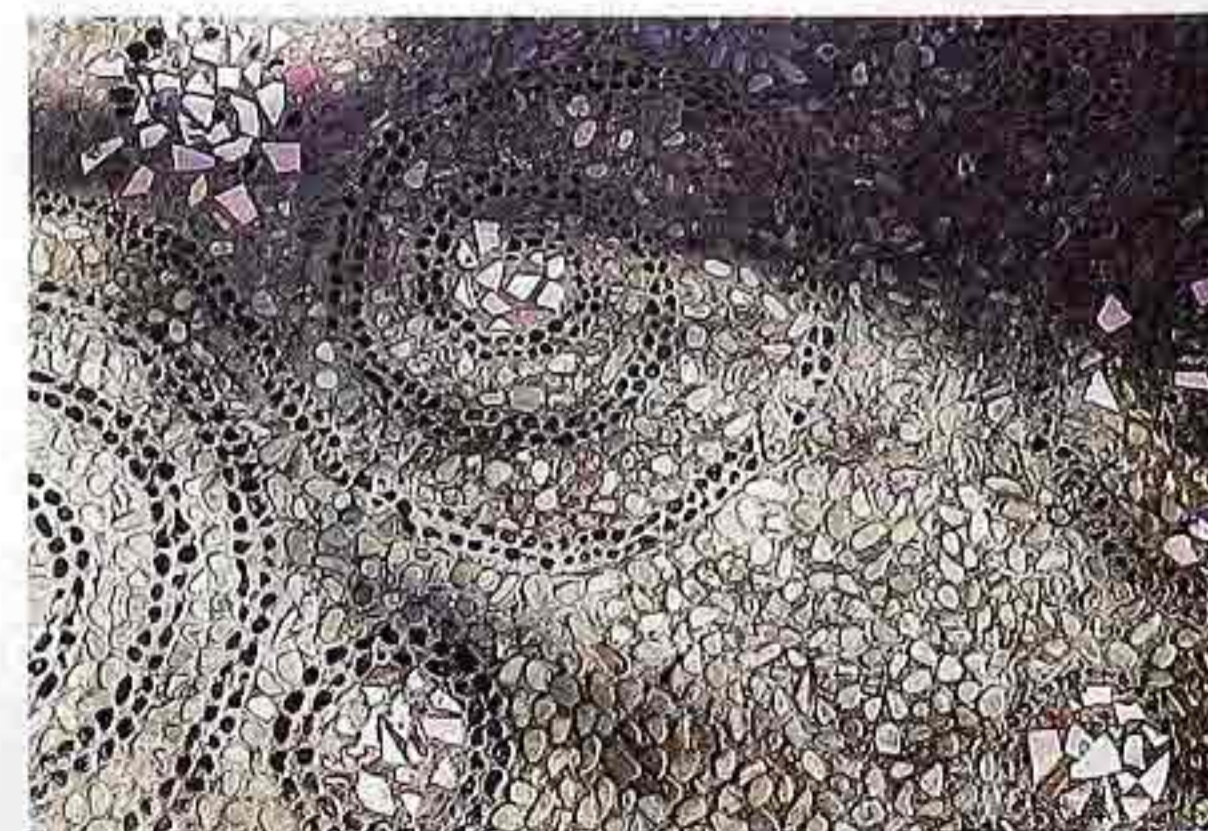
FP-77 Serpentine design of polychrome pebbles in exposed aggregate
