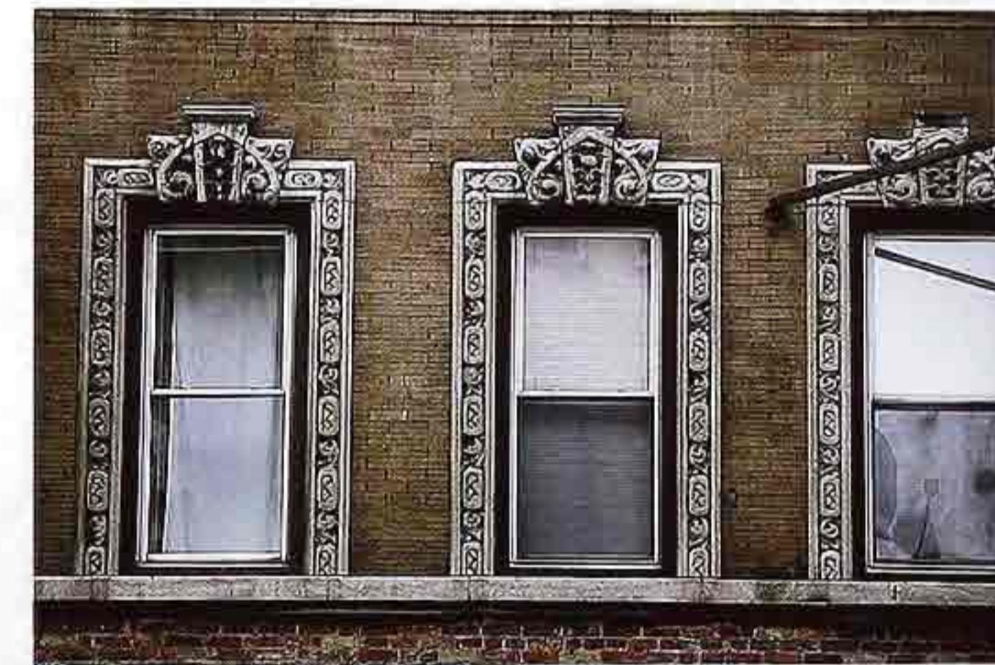
WI-130 Stone or cast concrete casings with relief ornament and ornated keystones, early 20th-c. apartment house
