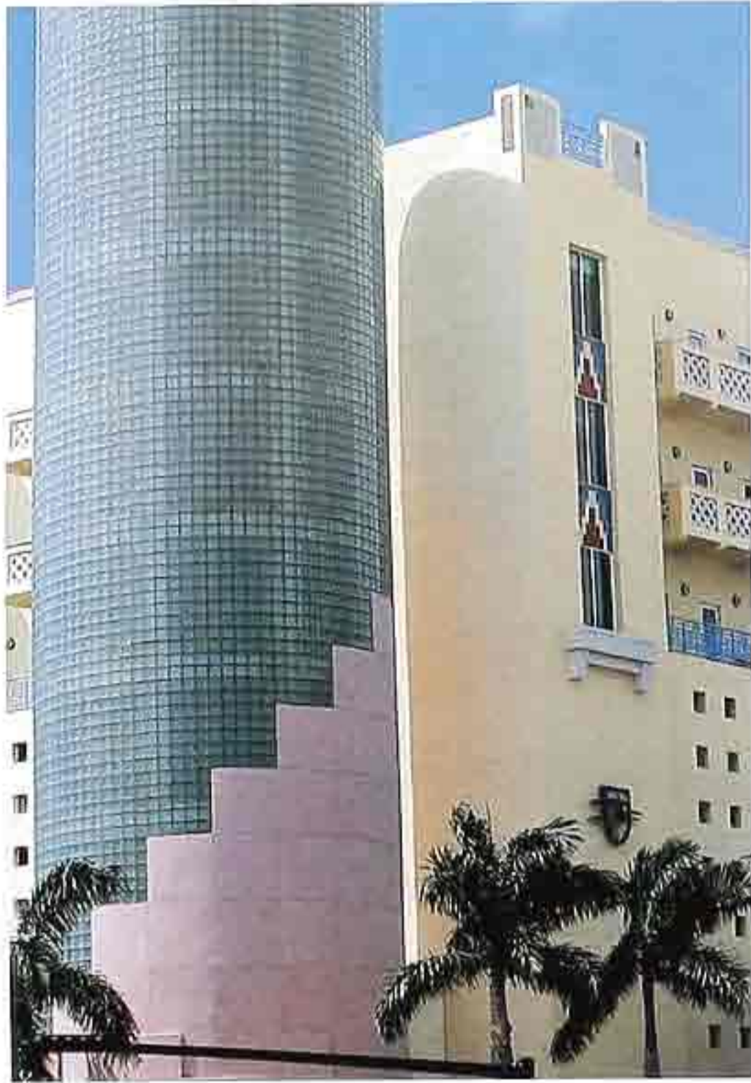
WA-306 Glass-block tower with stepped cast concrete at base next to cast-concrete Art Deco-style modern residential building
