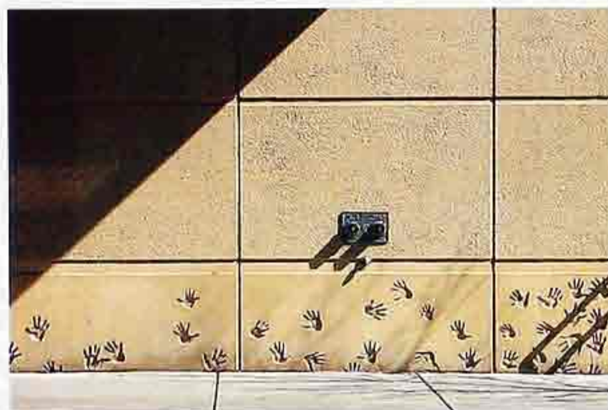
WA-240 Cast concrete walls imitating stack bond, base course decorated with imprints of children's hands, urban public space
