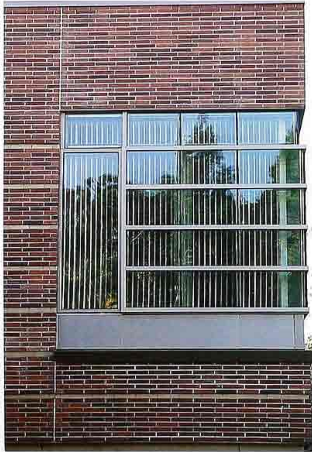
WI-86 Corner window: fixed lights with metal sashes, muntins, and mullions, modern commercial building
