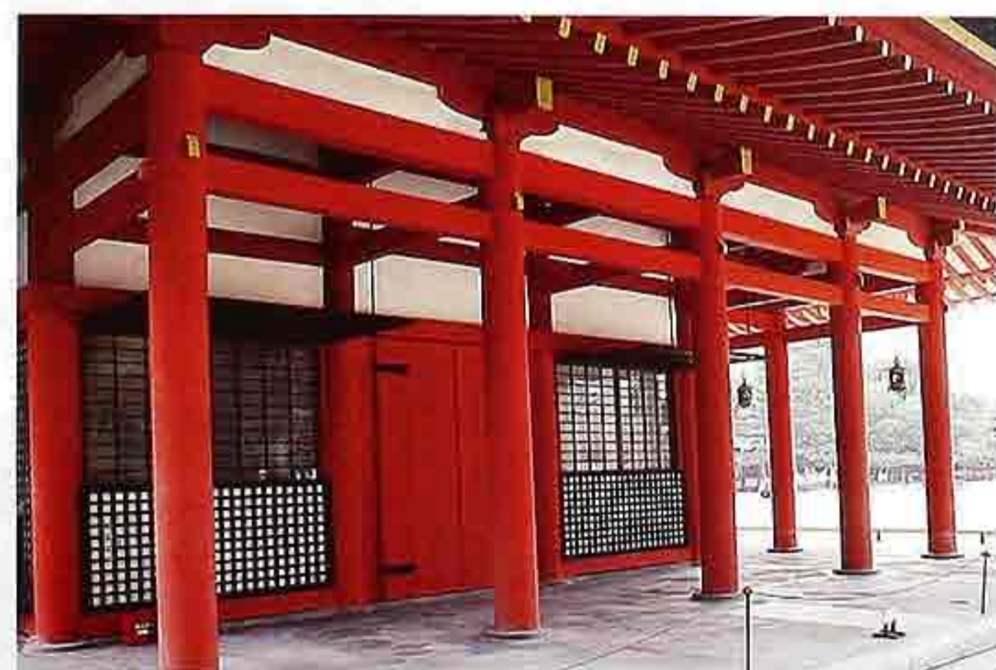
CP-140 Post-and-beam construction, Japanese temple
