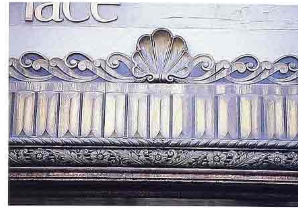
OM-4 Bands. Top to bottom; stylized Vitruvian scroll with shell antefix; vertical corrugated pattern; rope molding, and foliated ovolo molding with pattern reversed at center
