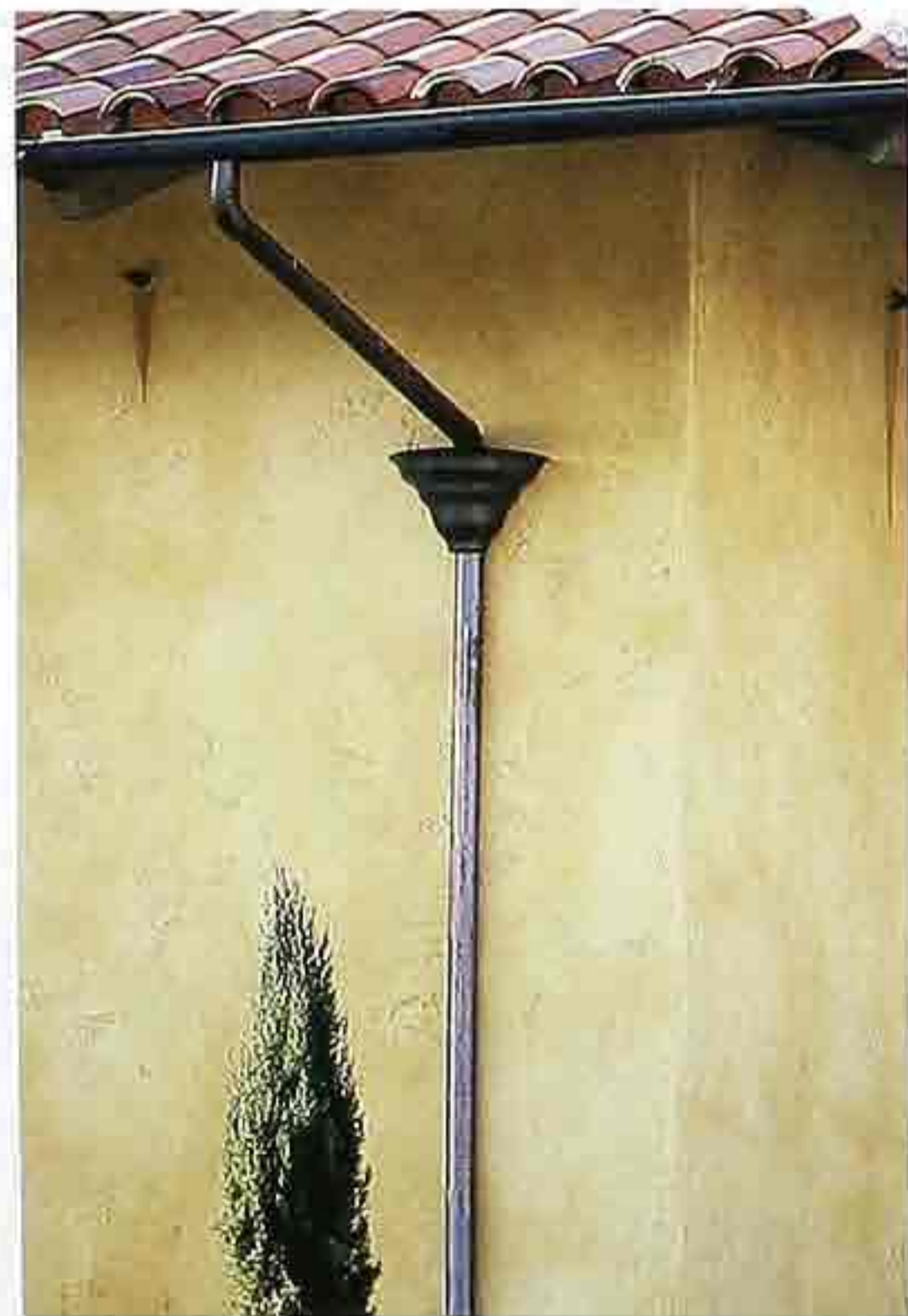
CR-157 Metal gutter, drainpipe, and rainwater head
