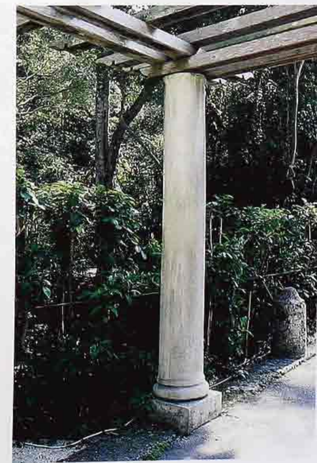
CP-137 Stone post with Attic base supporting wooden garden trellis
