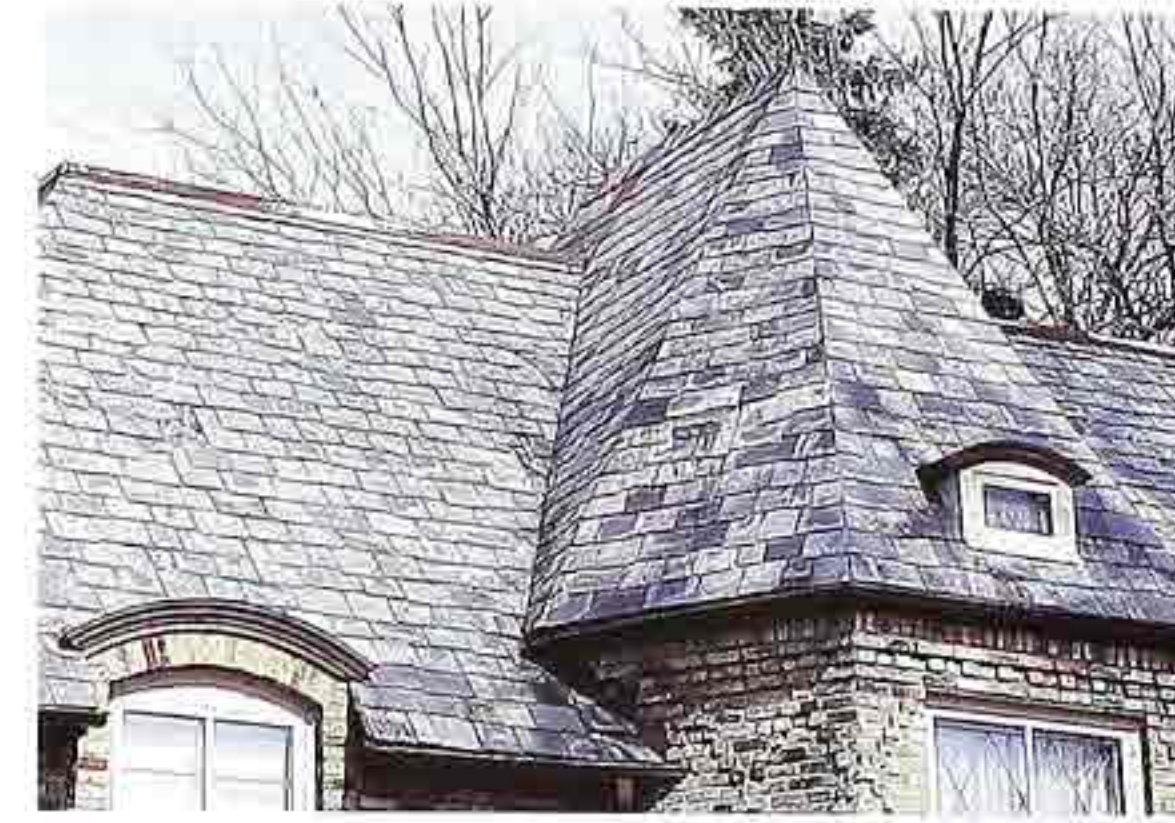
CR-58 Variegated slate roofing on hipped roof with pyramidal wall dormer, American house
