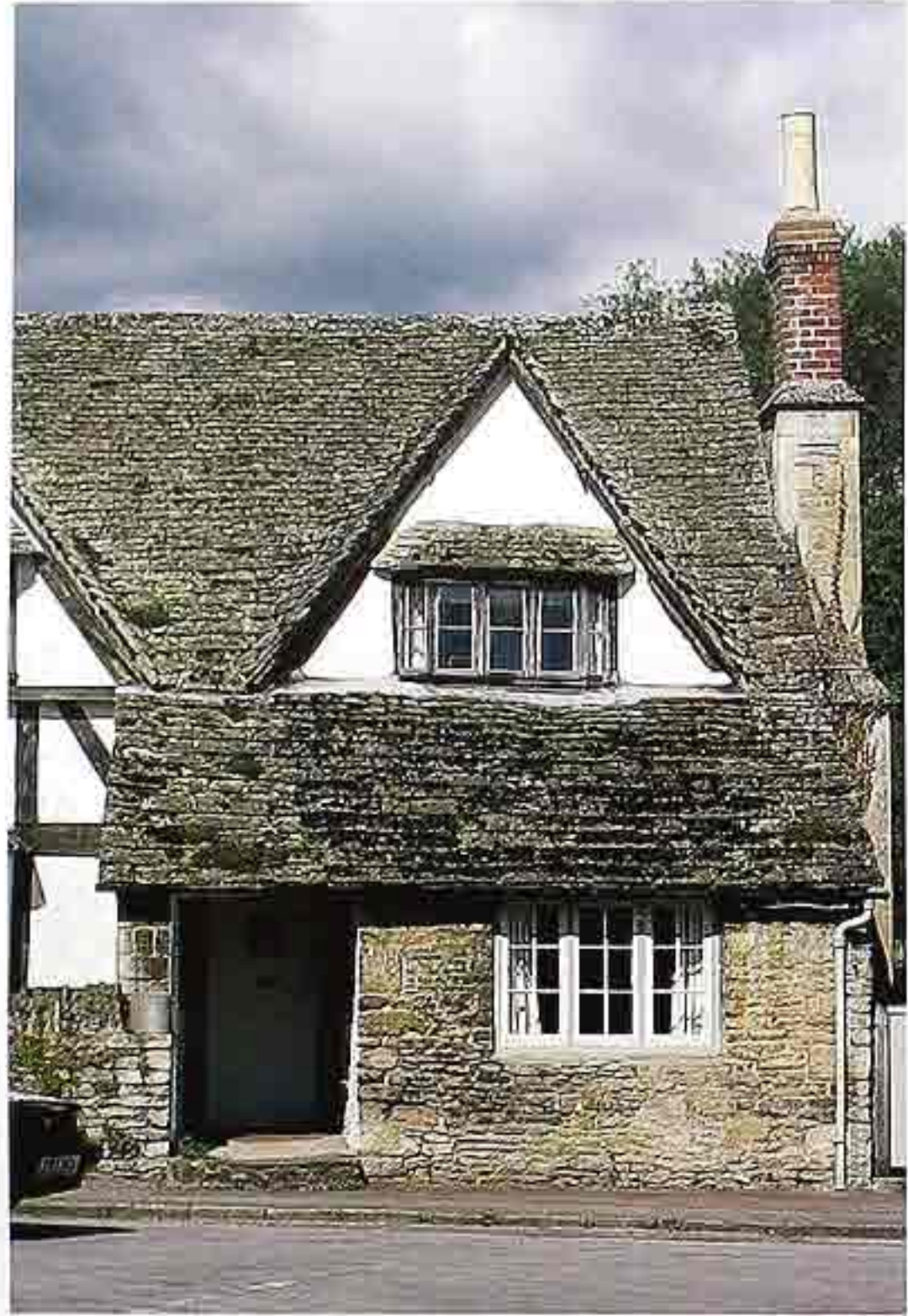
CR-126 Slate gable roof and gabled roof dormer with bay
