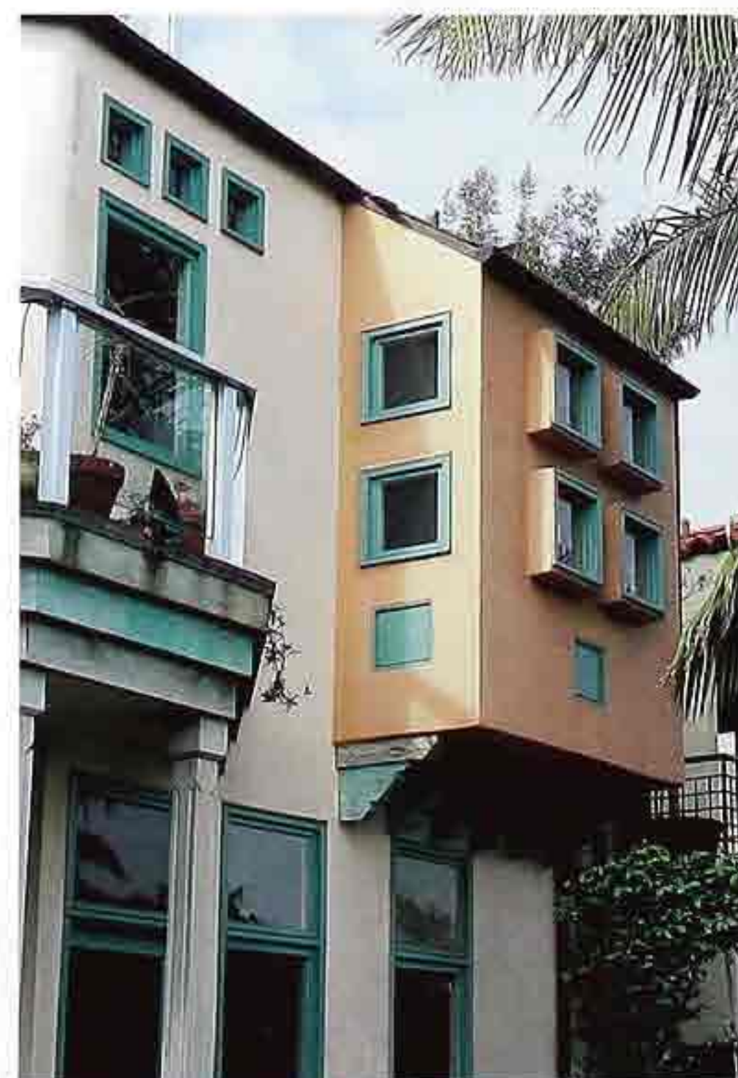
WI-92 Oriel with awning or fixed windows, shed roof, and corbels, modern apartment house
