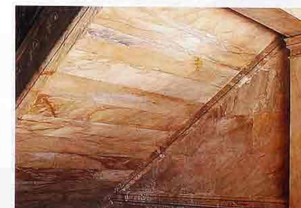
WA-104 Siena marble veneer on staircase soffit, molding and pilaster
