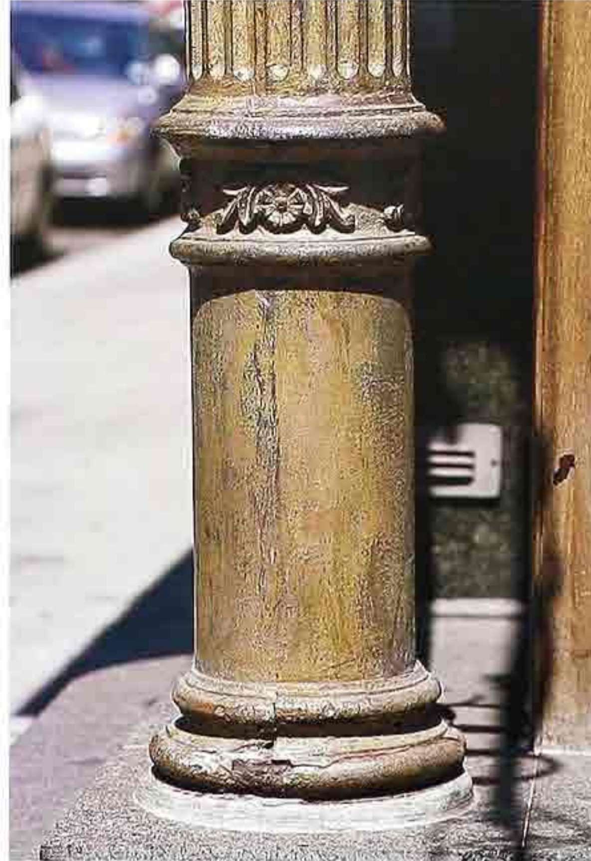
CP-59 Fluted column with Doric base on round pedestal with Attic base and floral ornament
