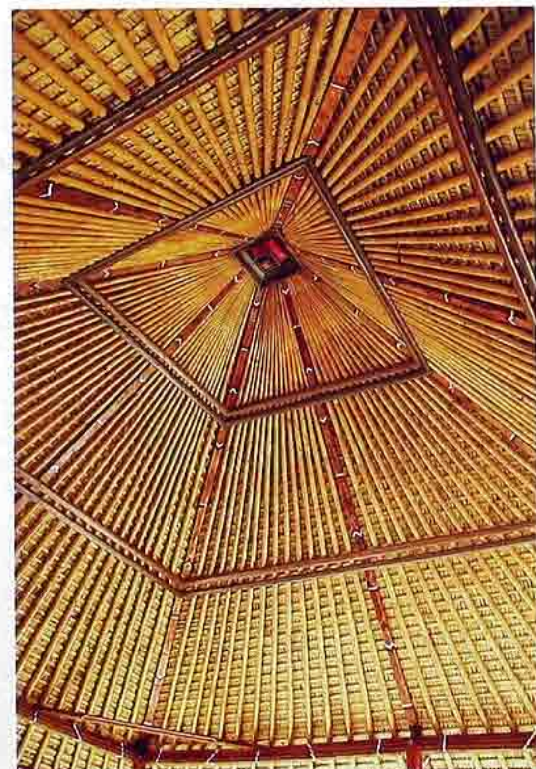
CR-3 Grass thatch roof showing connection between thatching and structure
