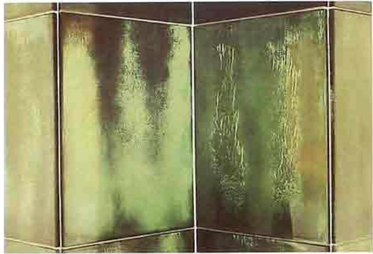
FA-1 Corner detail of clear-coated verdigris cladding, with grouted seams
