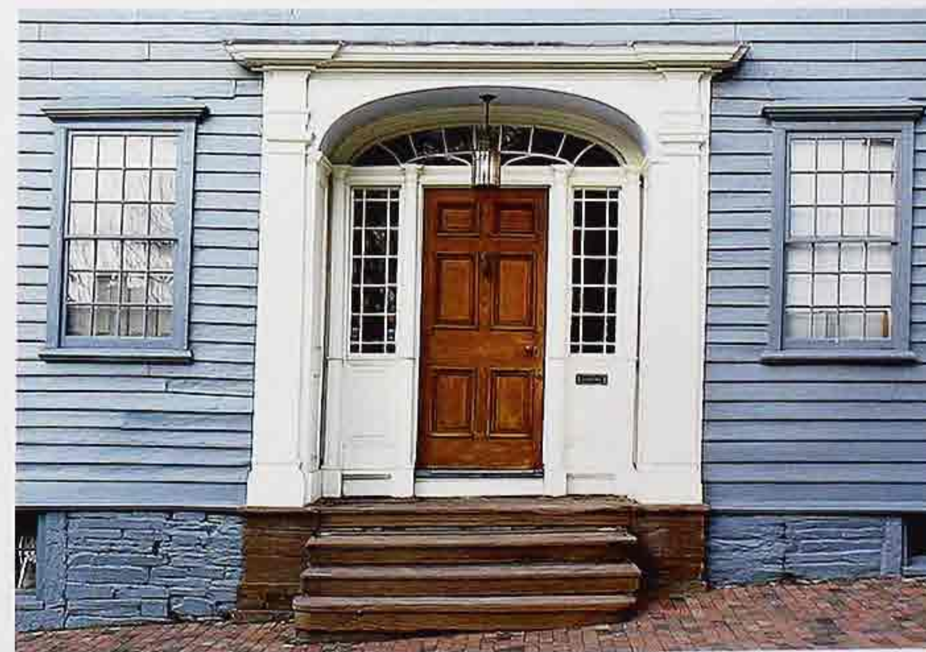
DW-86 Arched entry with crown molding and pilasters around paneled door, side lights, and fanlight, 18th-c. American house
