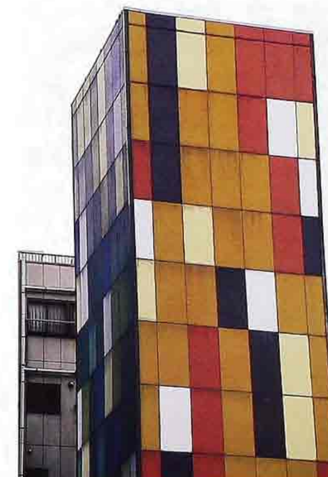
FA-89 Multicolored painted plywood cladding on building under renovation
