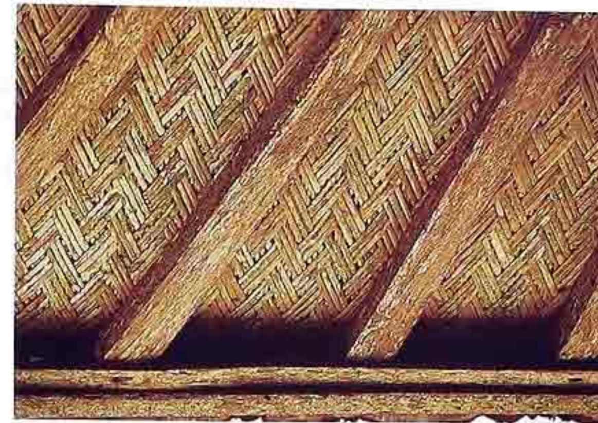
CR-5 Woven split bamboo behind roughly hewn rafters, Indonesian pavilion
