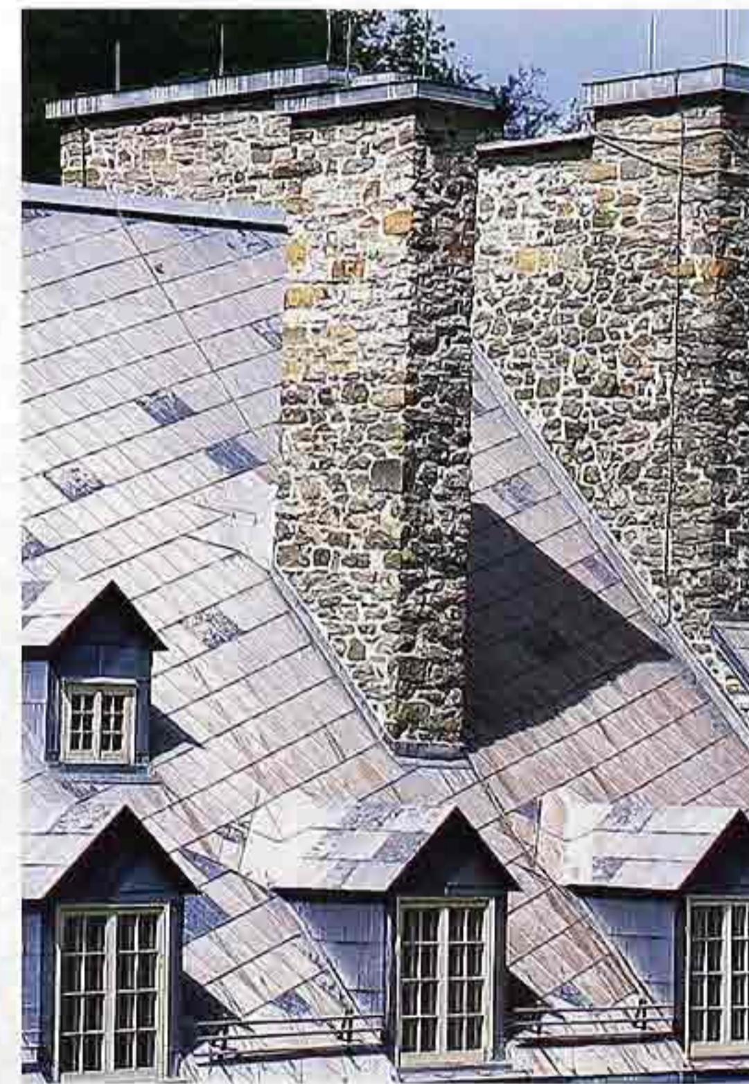
CR-153 Coursed-rubble chimney
