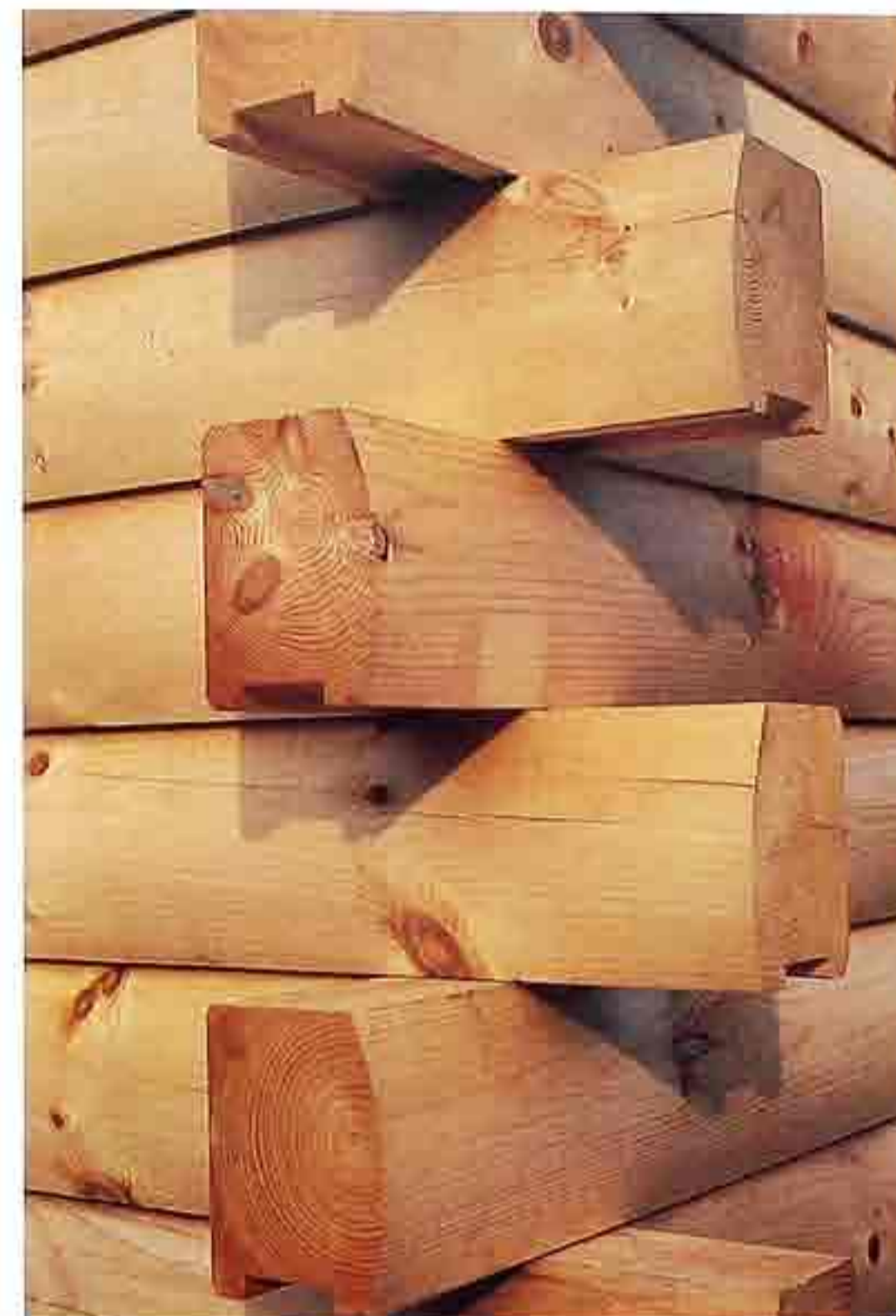
WA-5 Pine log house construction, corner detail
