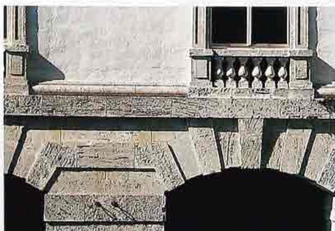
WA-116 Sawn fossil-stone in coursed ashlar with raised voussoirs; engaged balustrade with bead base molding above belt course
