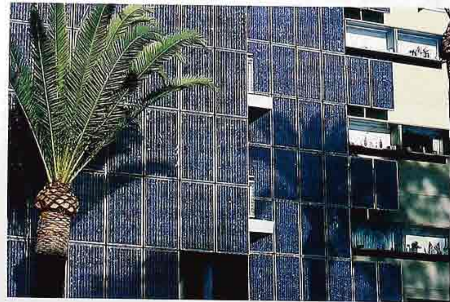
FA-42 Photovoltaic-panel cladding, modern commercial building
