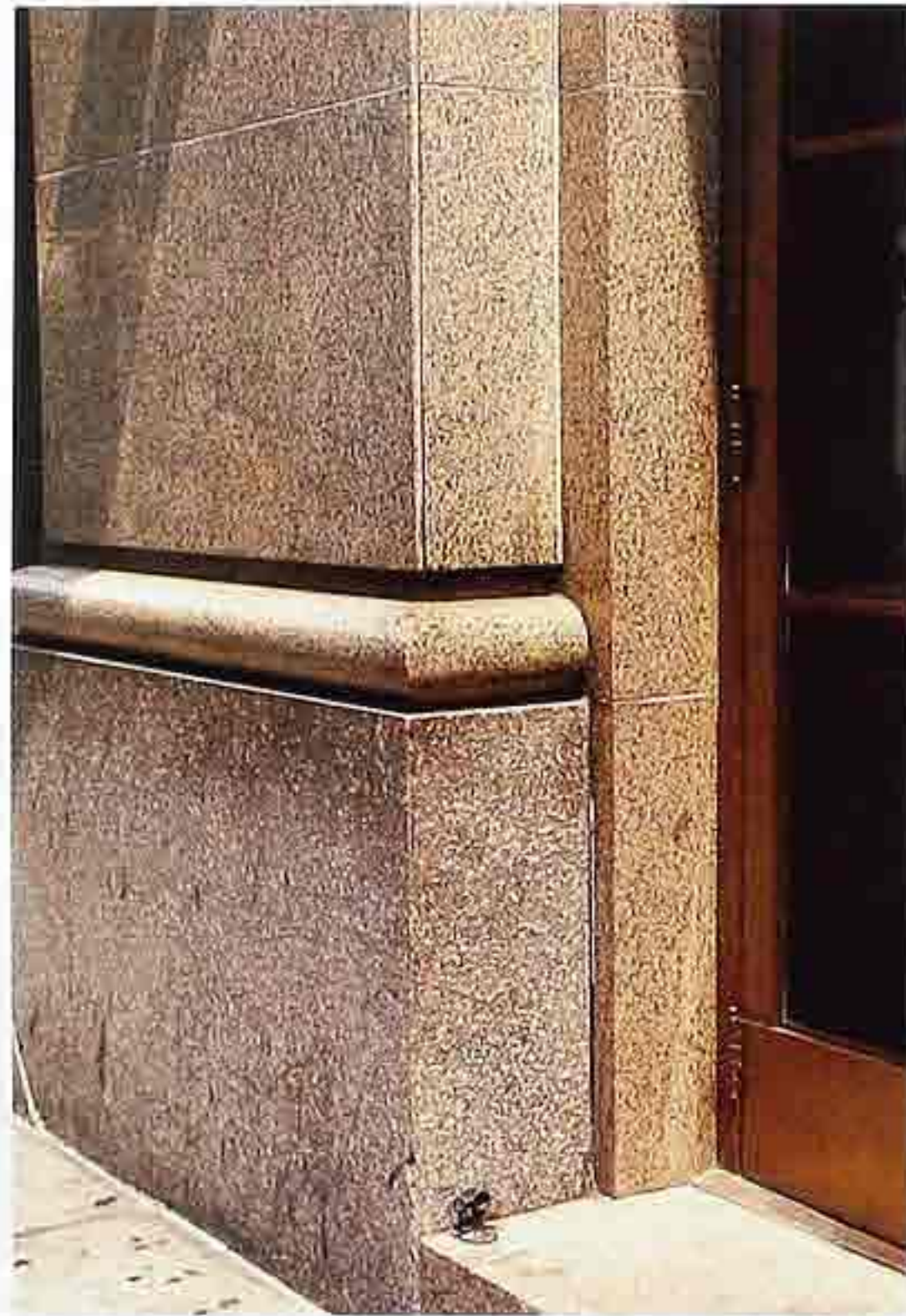
WA-89 Honed granite veneer with solid granite base and bead molding beside granite door casing
