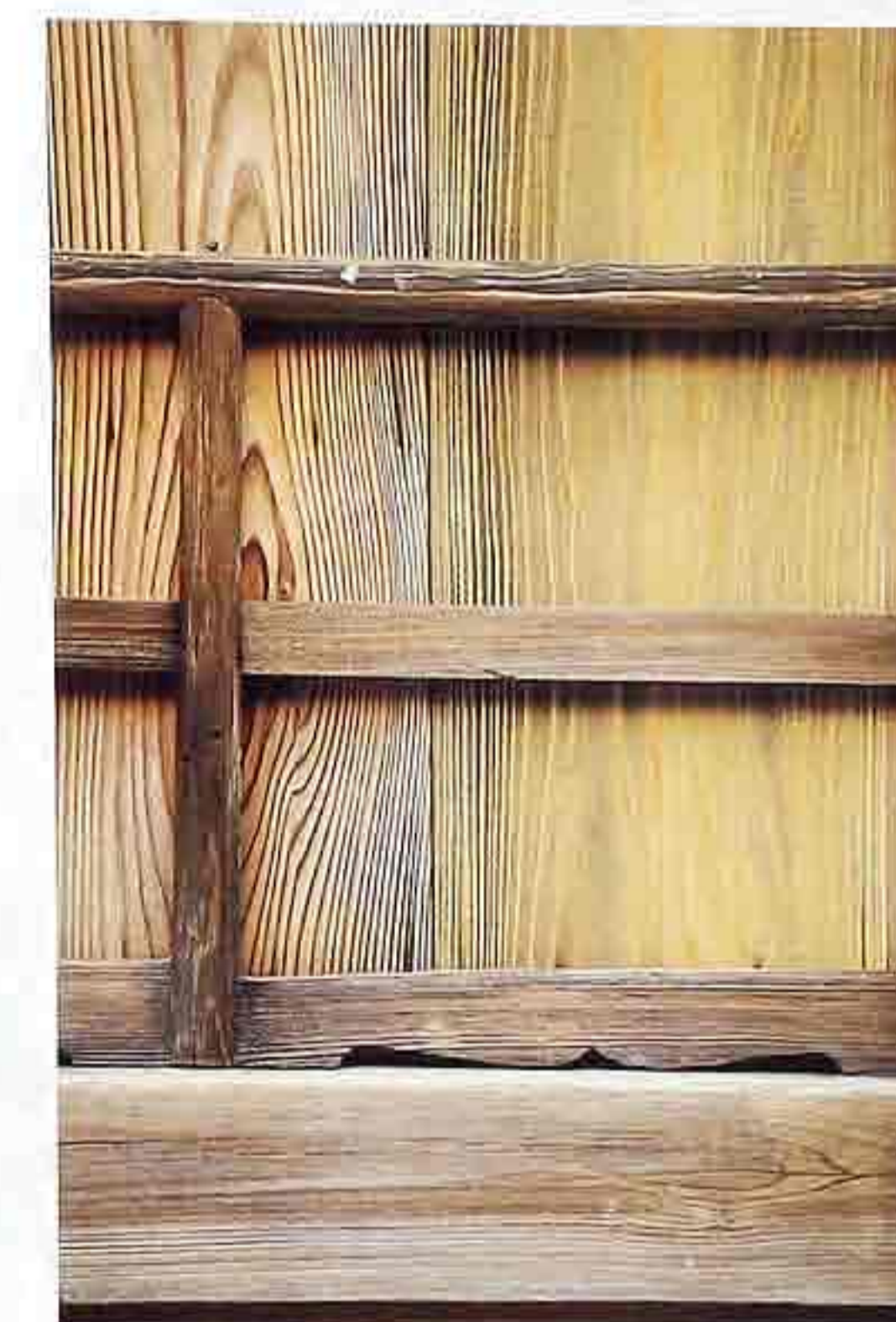
WA-6 Plain-sawn vertical planks with decorative battens
