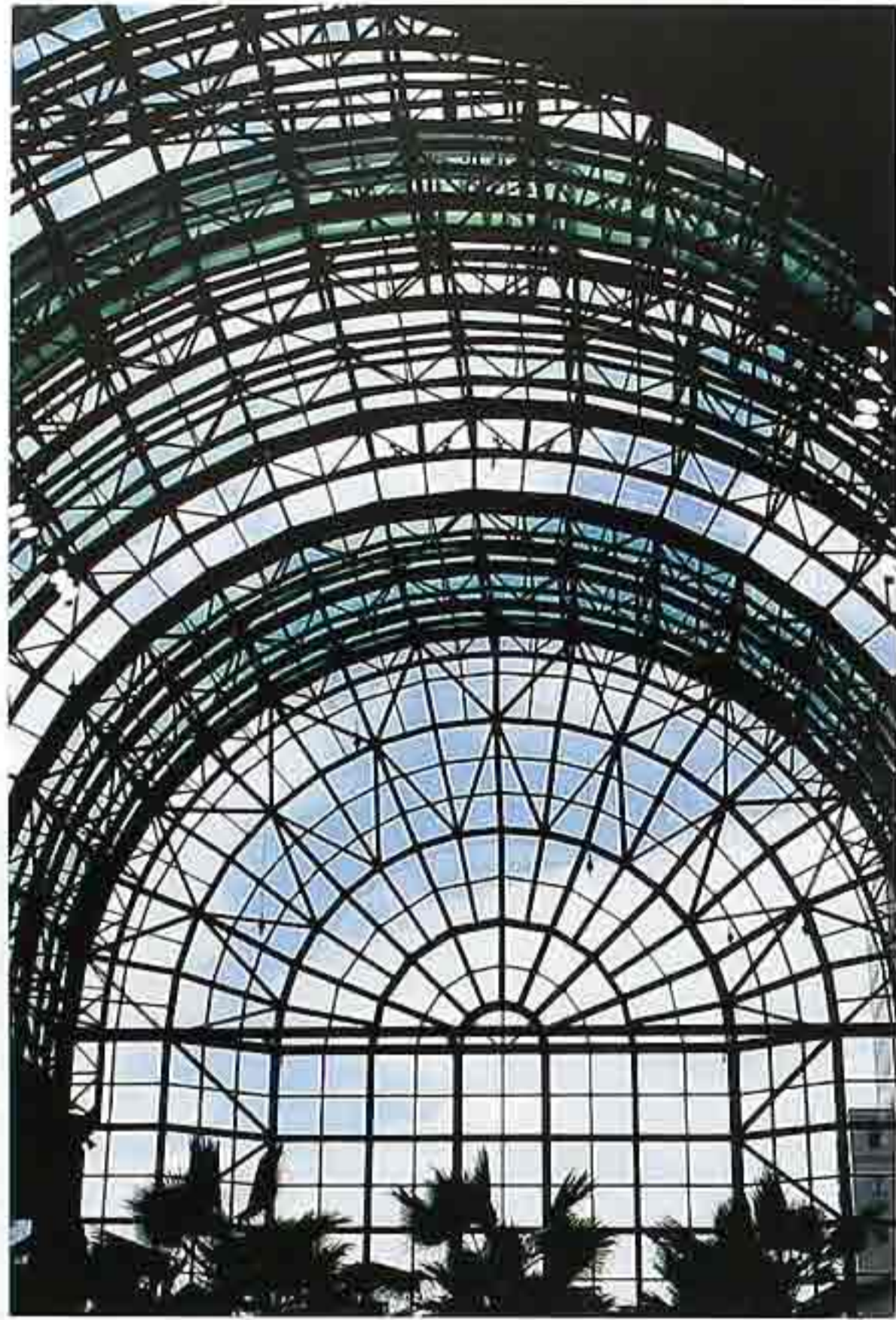
CP-176 Barrel-vaulted metal and glass modern greenhouse structure
