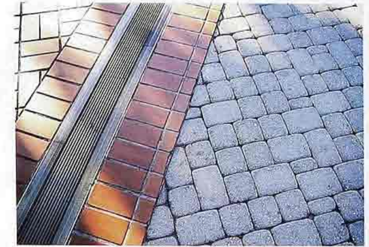
FP-86 Tumbled pre-cast concrete pavers in random-ashlar pattern; flexible paving (left) bordered by terracotta tile and drain grate, urban public space
