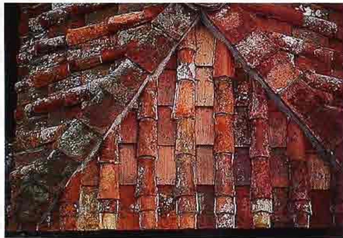
CR-46 Weathered terracotta tiles on pyramidal roof
