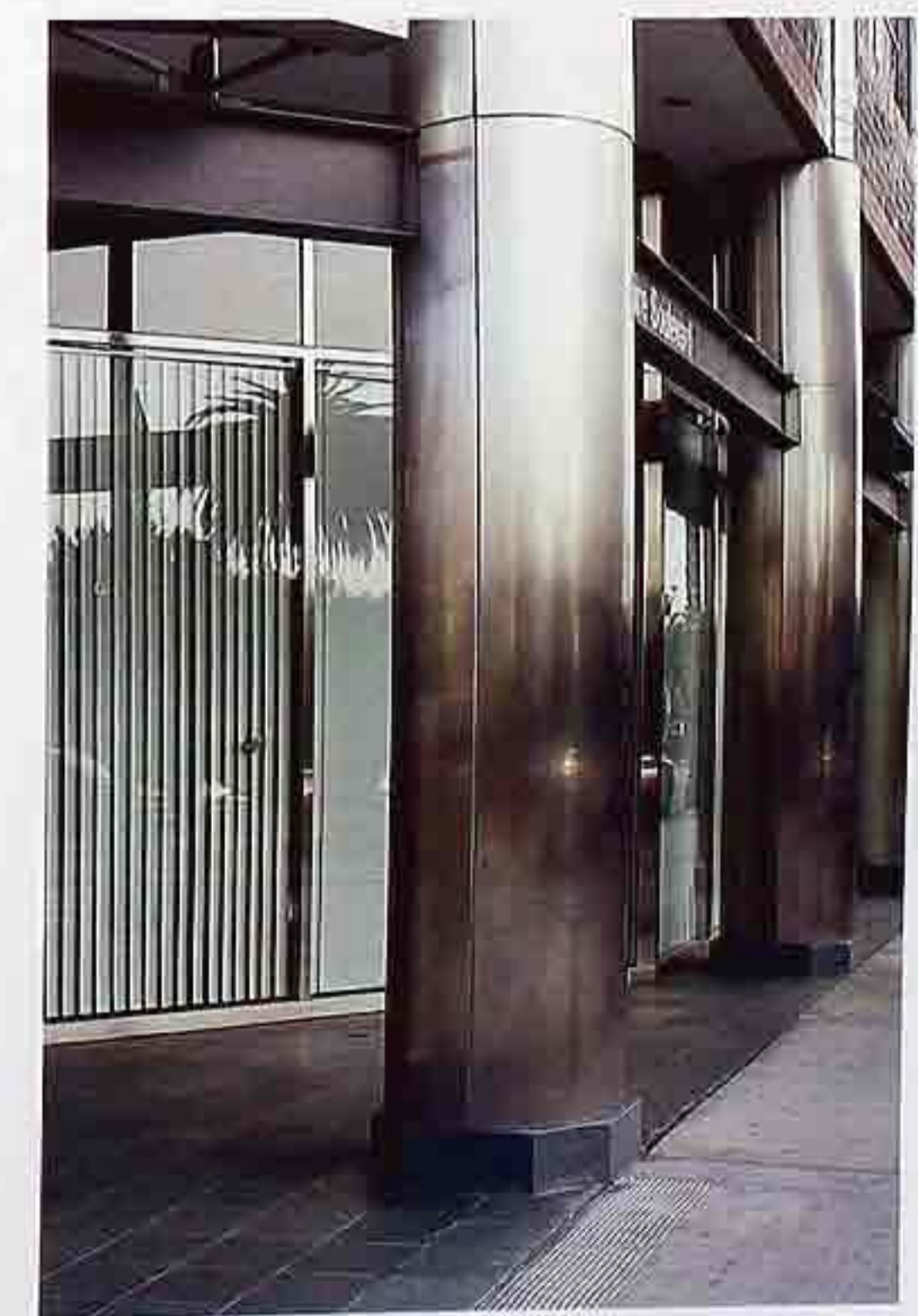
CP-129 Steel column with stainless-steel cladding supporting entry canopy, modern commercial building
