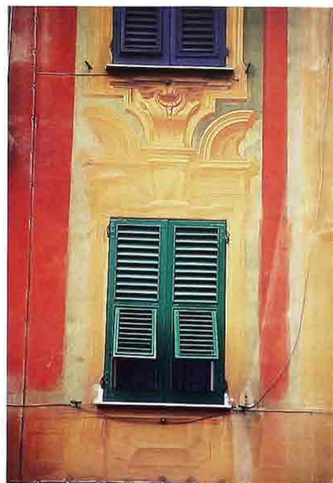
FA-83 Weathered trompe l'oeil moldings and pediment around shuttered windows on Tuscan wall
