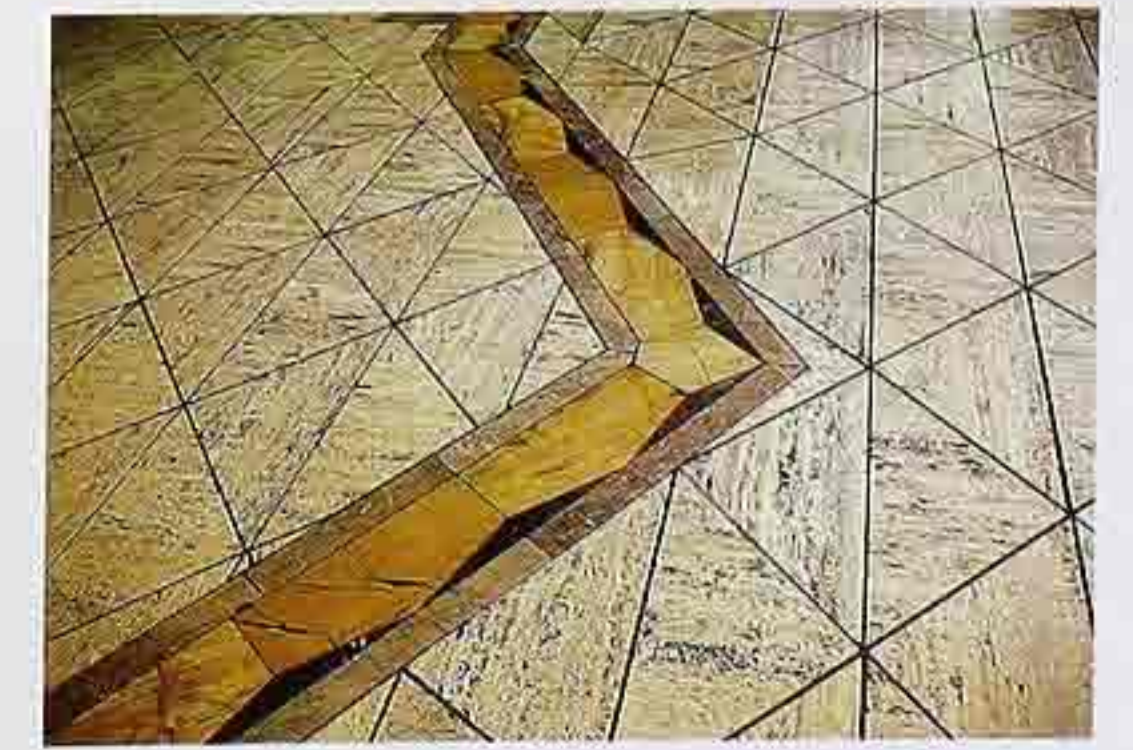
FP-18 Travertine and marble parquet in geometric pattern with marble polychrome band in foyer
