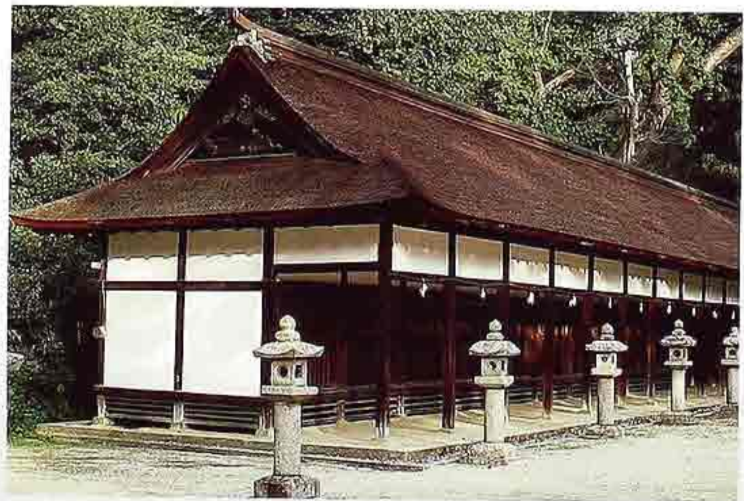
CR-136 Thatched gable on hipped roof, Japanese temple
