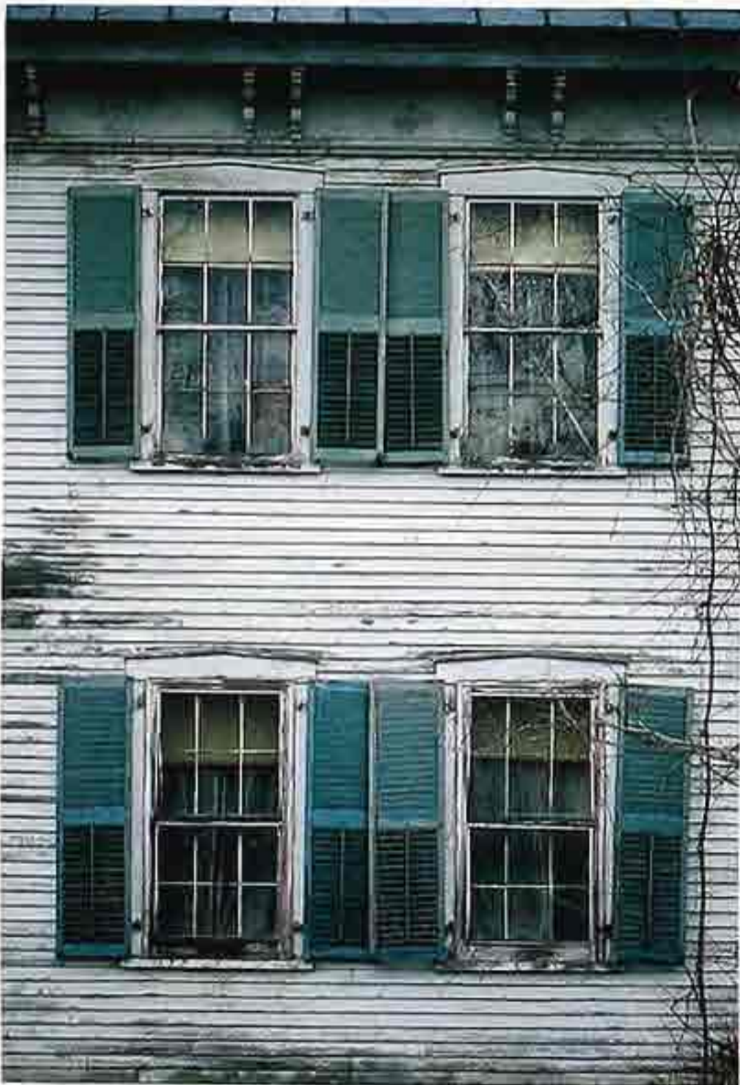
FA-94 Weathered painted clapboard facade
