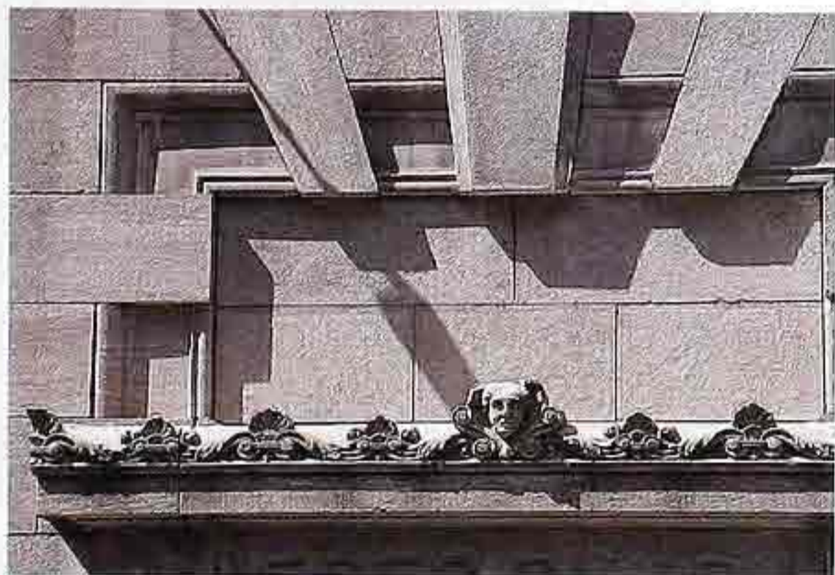
OM-59 Antefixes on cornice over a portal, the center one a mascaroon
