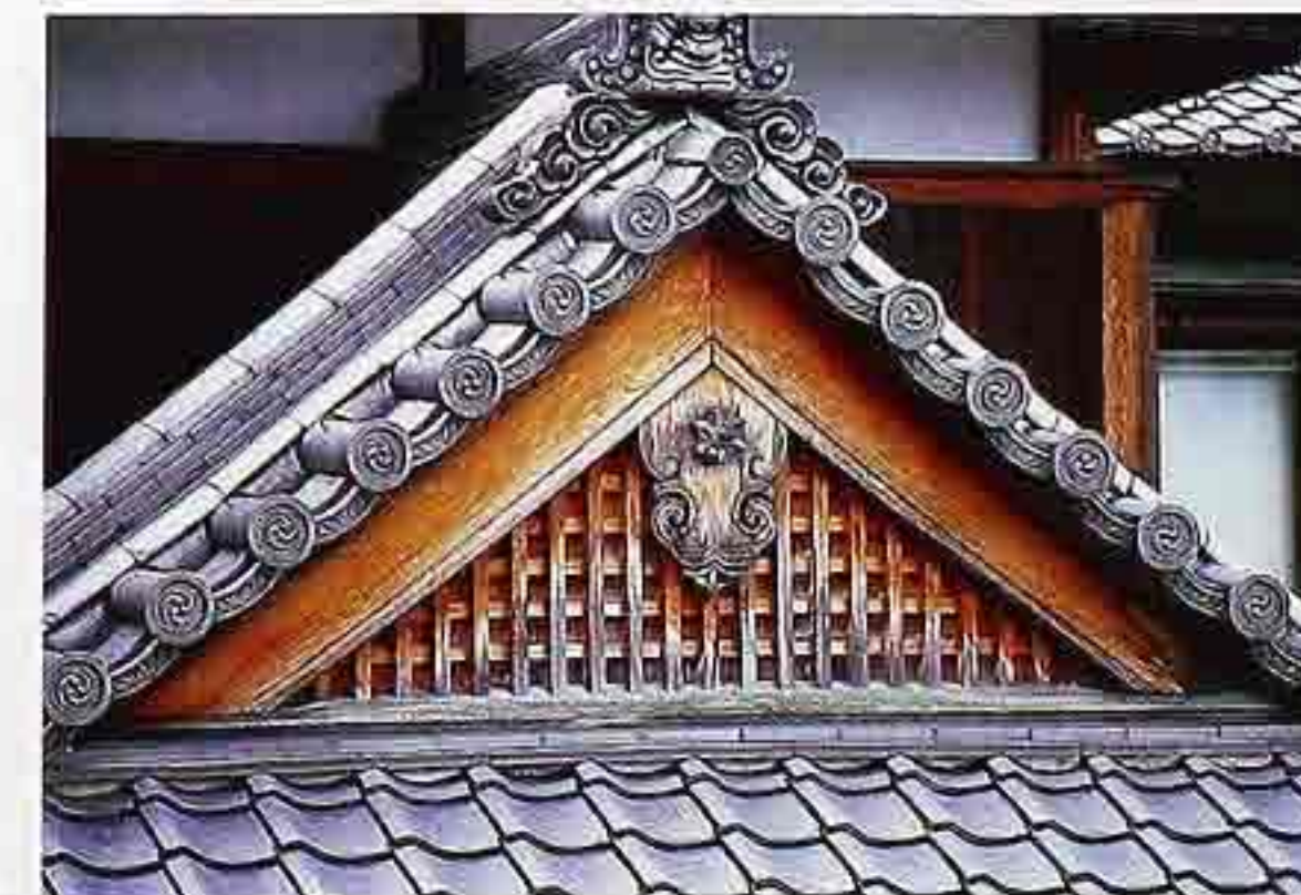
CR-84 Wood gable with lattice; ceramic tiles on gable roof and adjoining shed roof (bottom), Japanese temple
