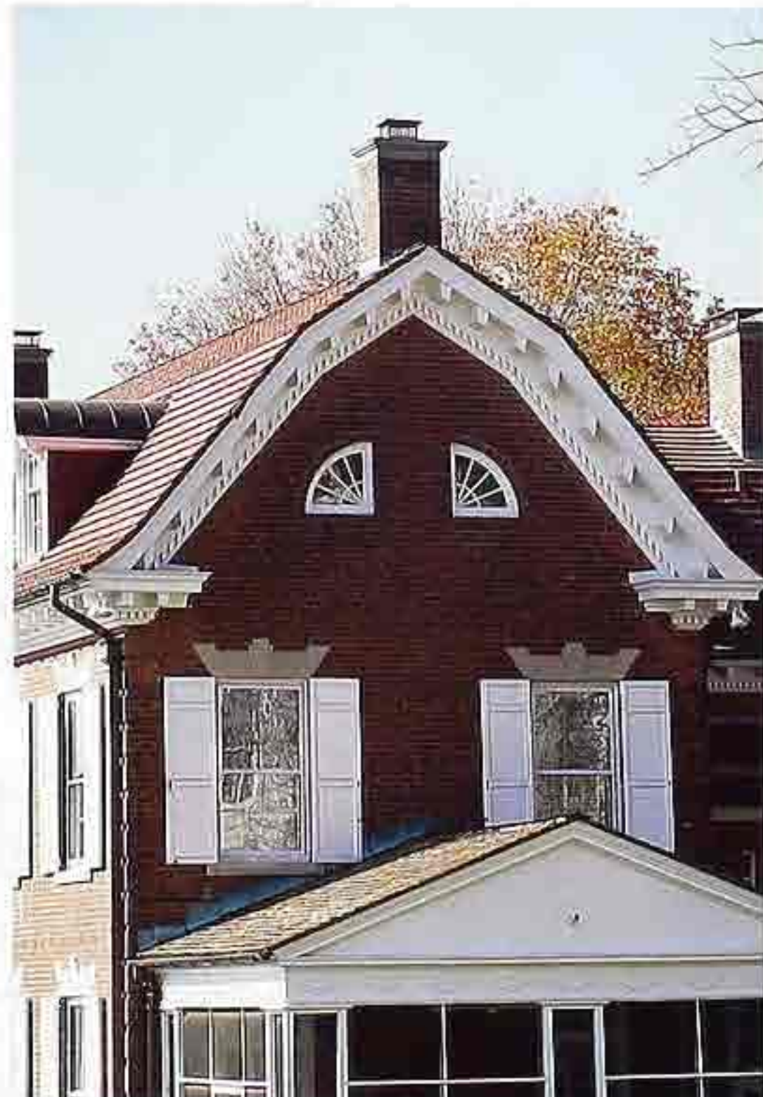
CR-129 Flared gambrel, soffit with modillions
