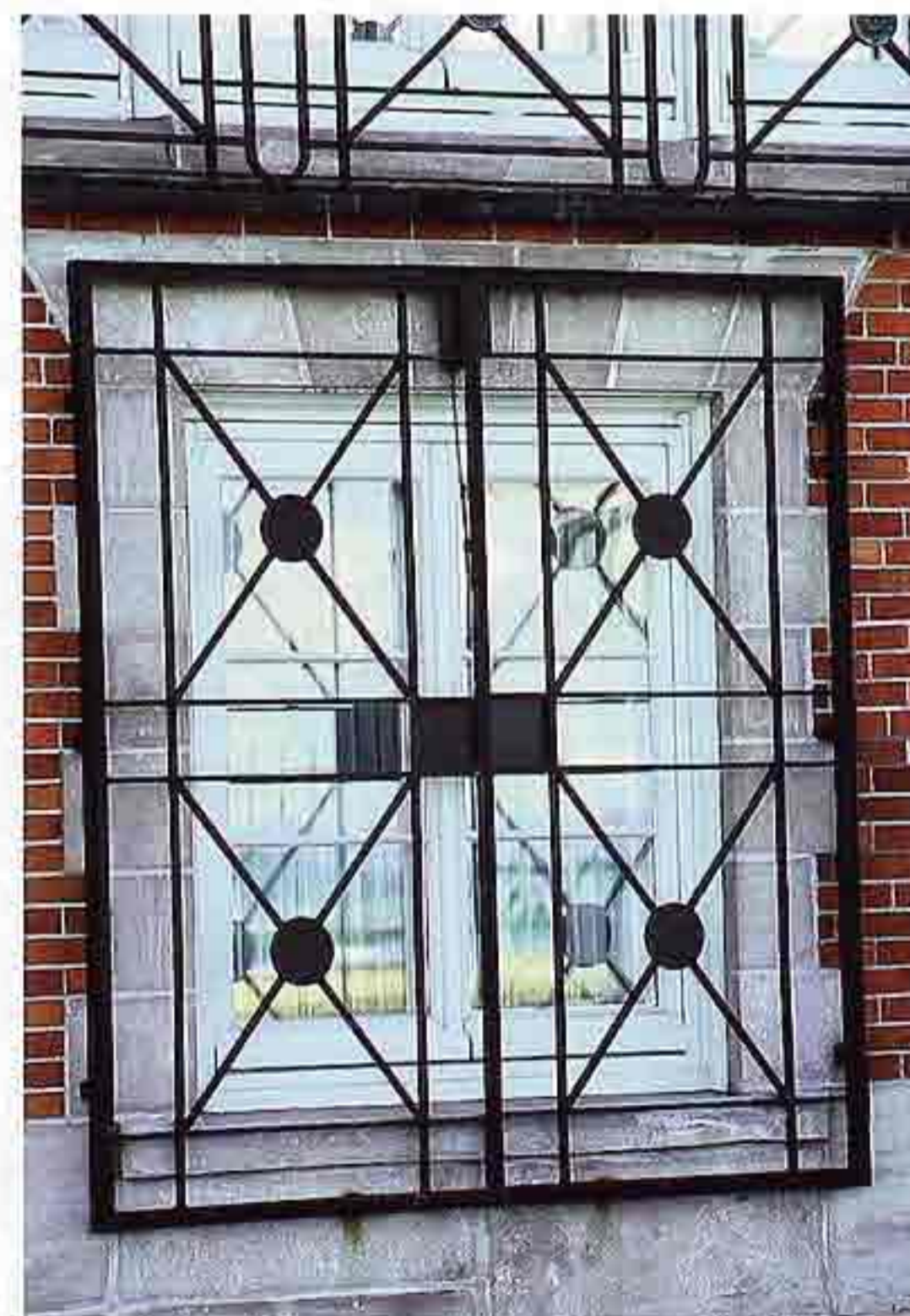
WI-170 Wrought-iron window gates with diaper pattern, modern apartment house
