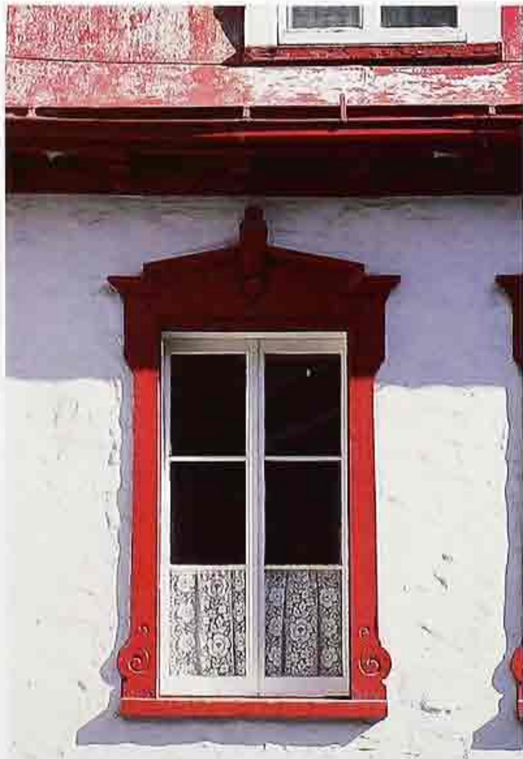
WI-113 Profiled flat casing around double-casement window
