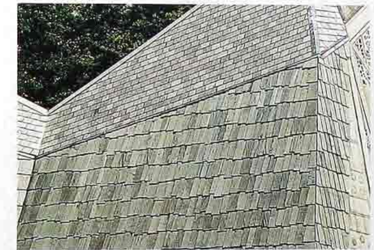
WA-129 Inside and outside corners of slate roof and cladding, modern commercial building
