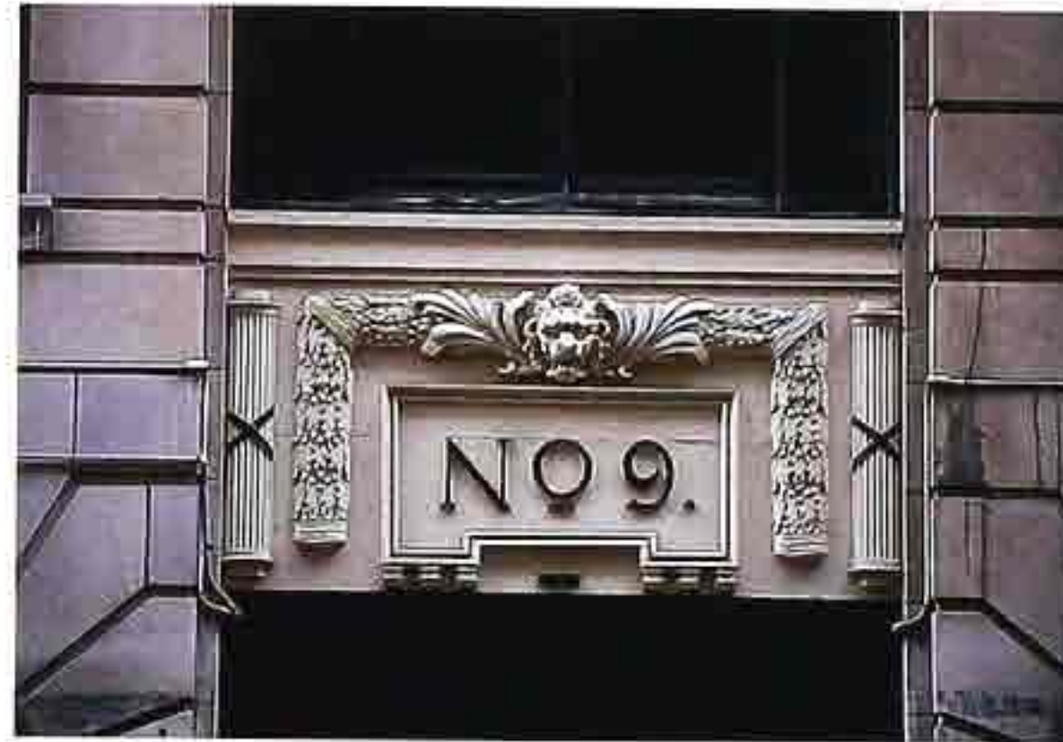
OM-24 Cartouche with building number above guttae, with festoon and center antic
