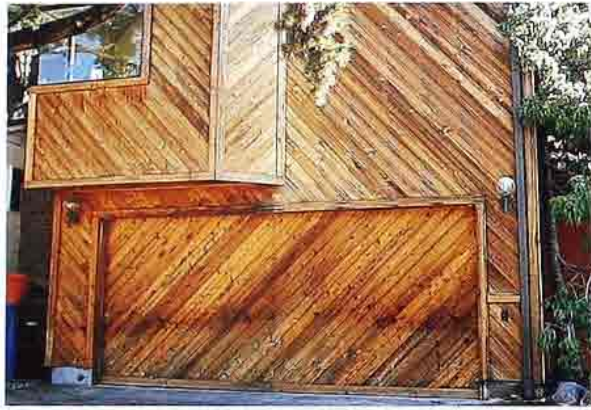
WA-51 Diagonal siding with flat edge trim and corner window, modern house
