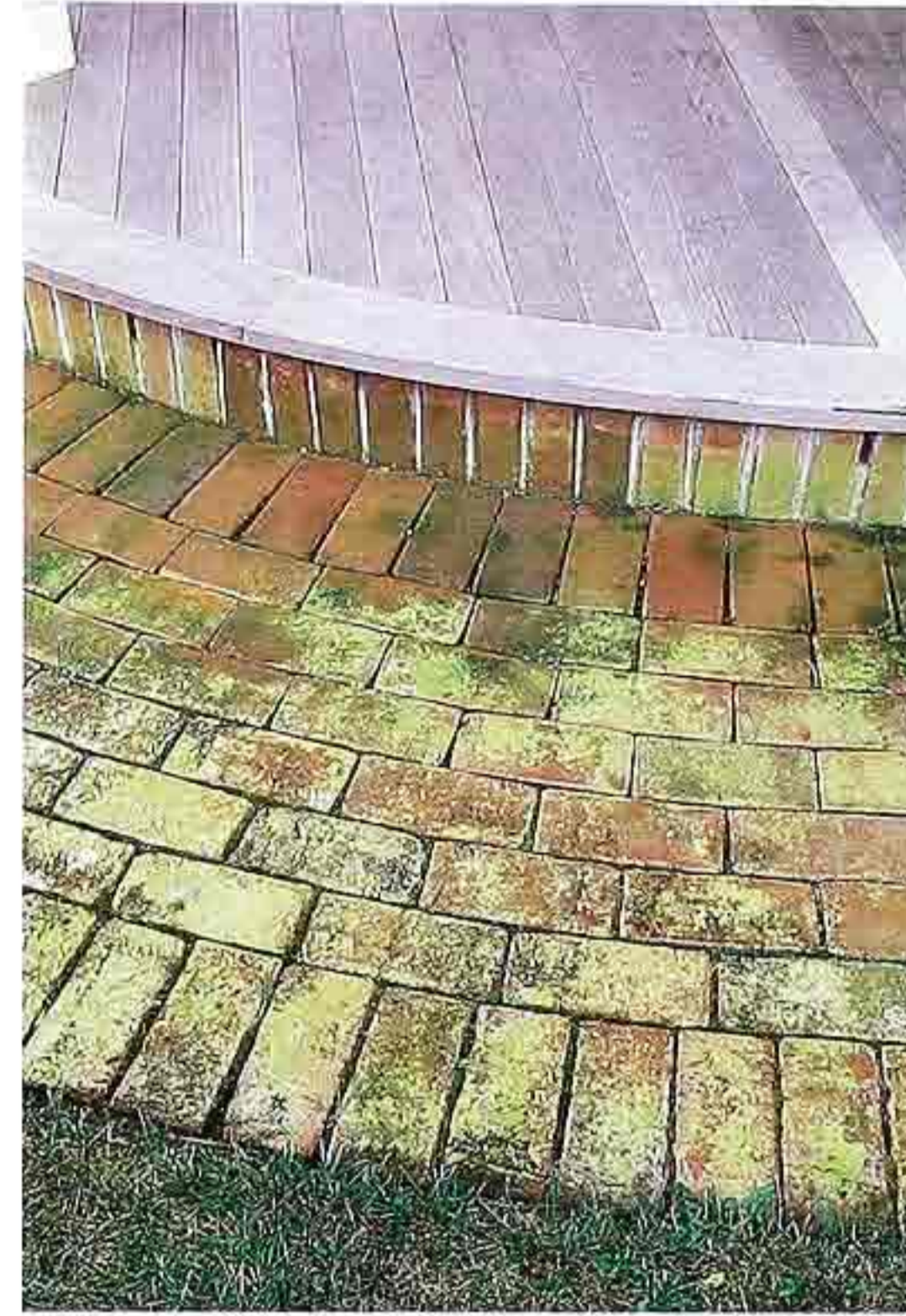
FP-61 Belgian-blend brick in running bond; soldier-course border and facing of mahogany decking, residential patio
