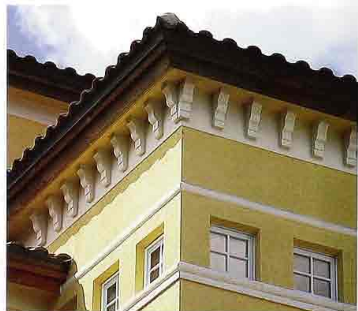
CR-108 Profiled eave brackets on modern Mediterranean-style house
