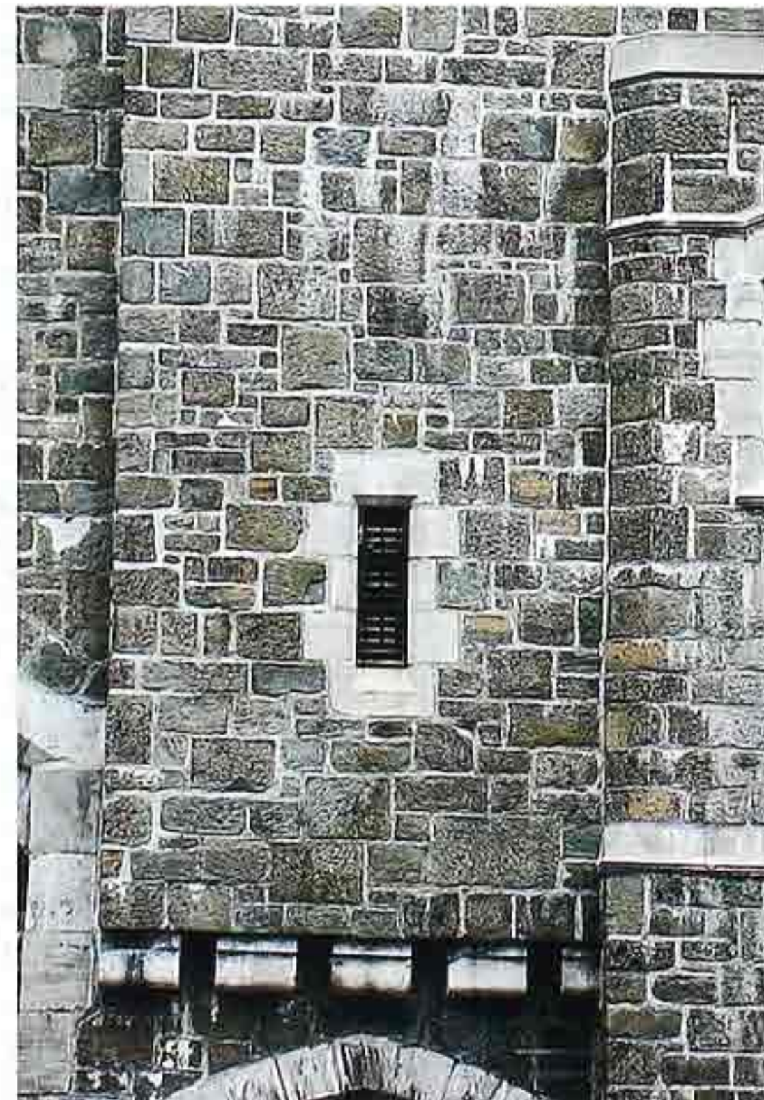
WA-109 Granite in random ashlar with corbelled jetty, dimension-stone window quoins
