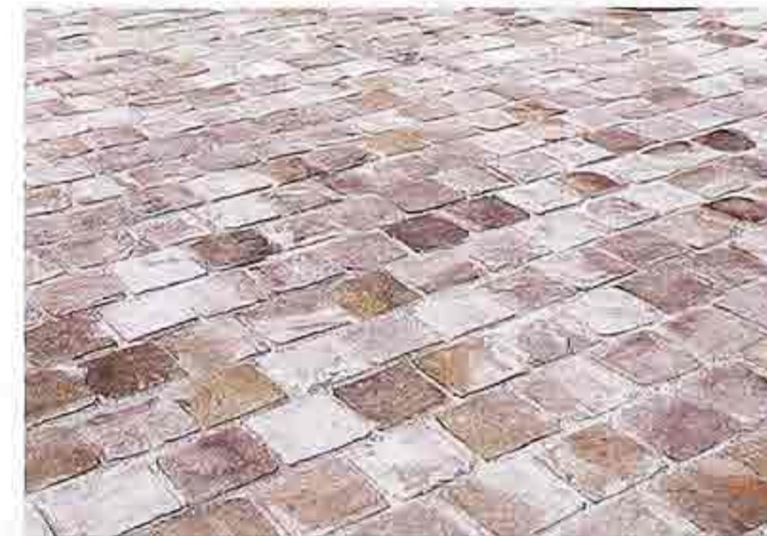
FP-33 Tumbled paving stone, courtyard of modern commercial building
