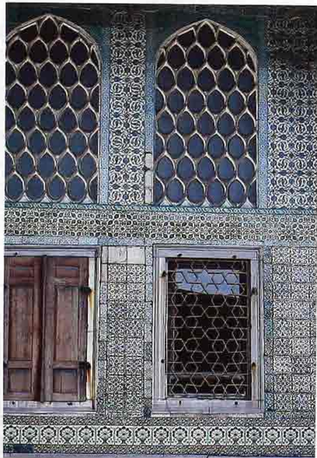
FA-70 Glazed patterned tiles around square windows with metal grille and wood shutter and ogee windows with grille, Turkey
