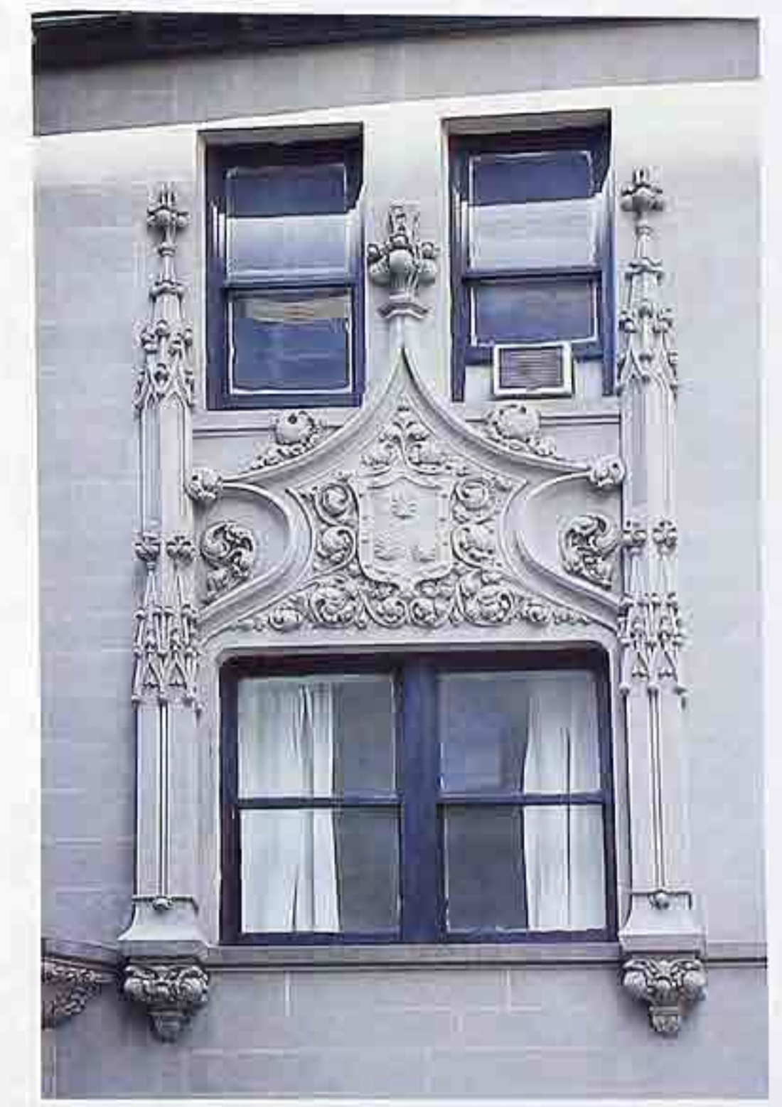
WI-137 Fanciful neo-Gothic spandrel with cartouche flanked by corbelled pilasters, apartment building
