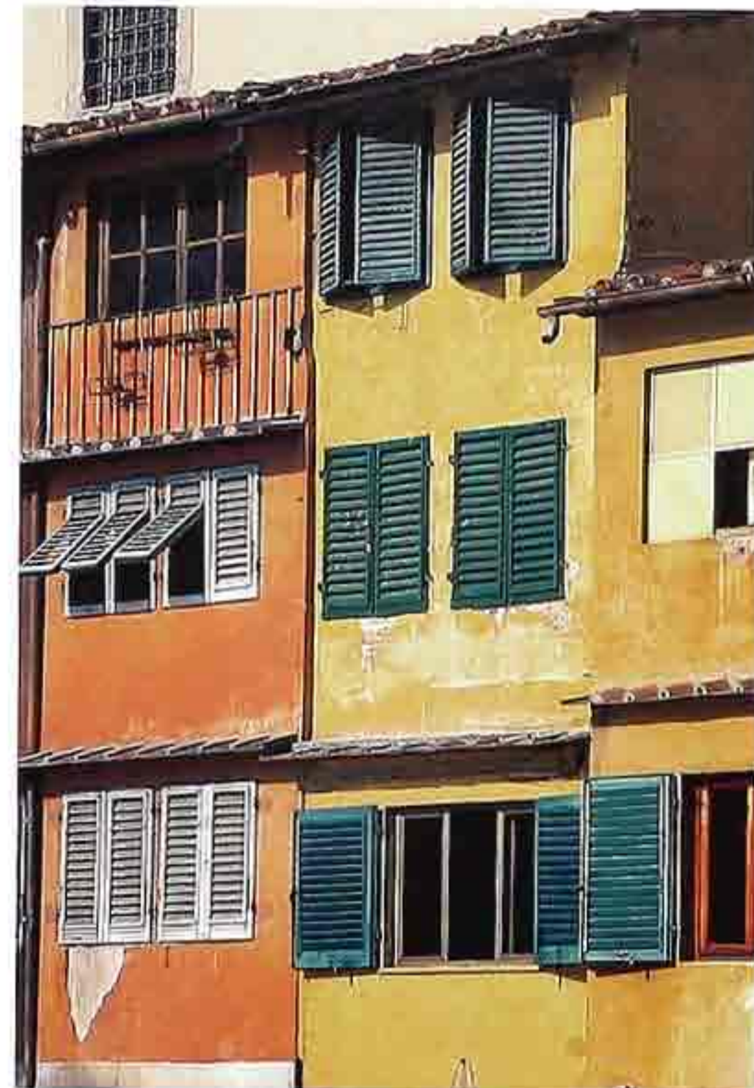
FA-93 Painted stucco facades, Italian riverfront buildings
