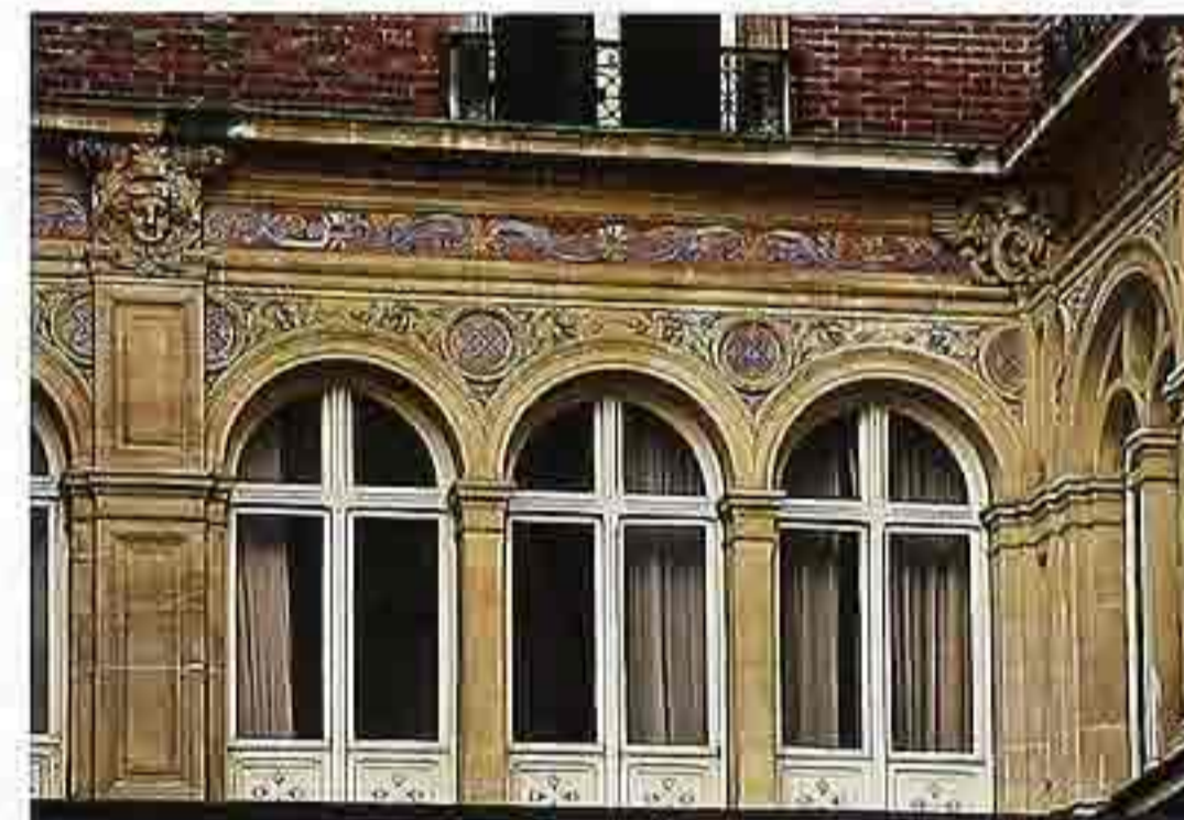
WI-143 Series of arches, pilasters, and polychrome terracotta or stone spandrels framing windows in stone casing, 19th-c. French mixed-use building
