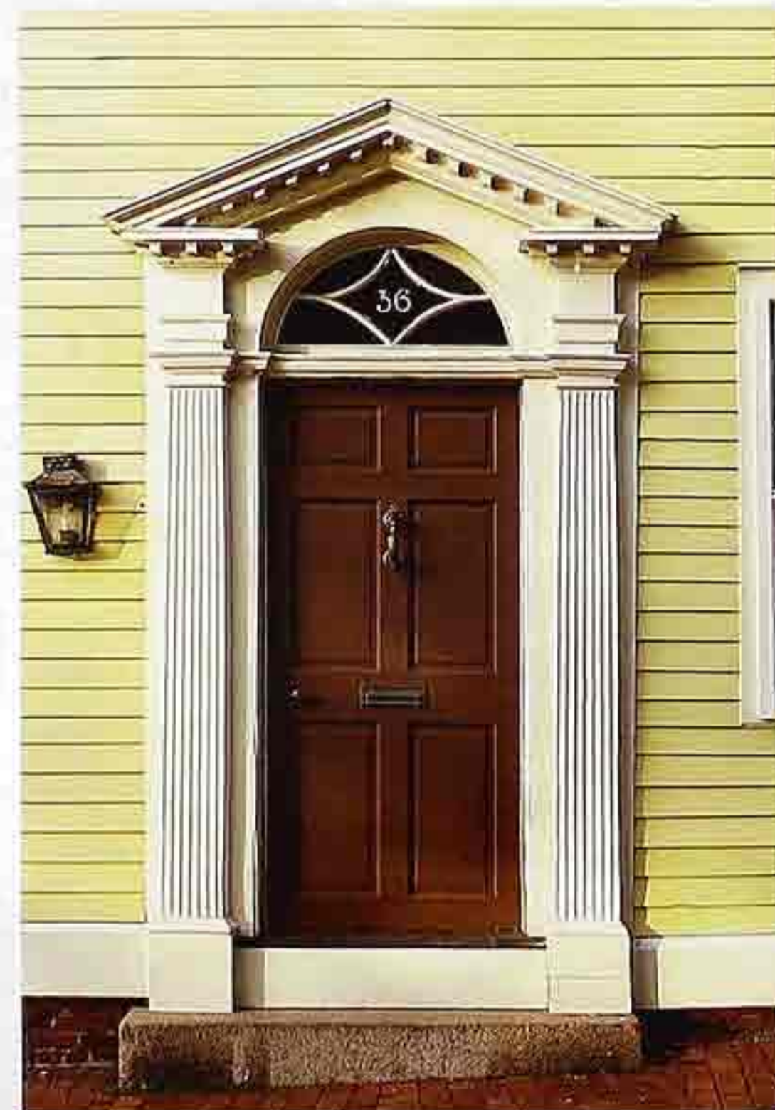
DW-83 Neoclassical pedimented door hood over pilasters and arched doorframe; wood panel door with fanlight
