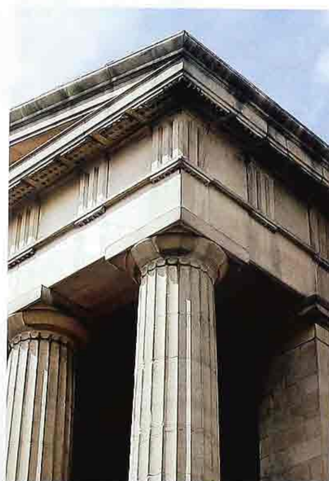
OM-108 Greek Doric-style entablature: plain architrave, triglyphs and plain metopes in the frieze, mutules with guttae in the soffit
