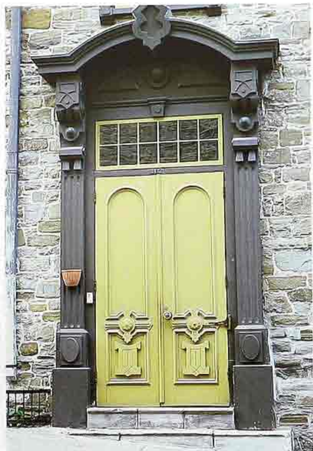
DW-80 Door hood: arch with ornate pilasters, carved paneled doors, twelve-light transom panel; 19th-c. building
