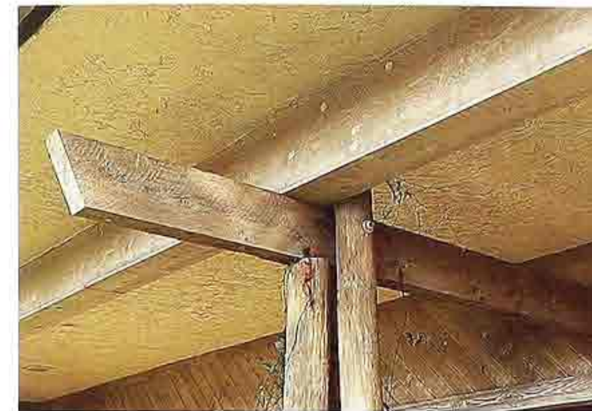
CP-116 Hammer-beam sitting on post supporting a beam above
