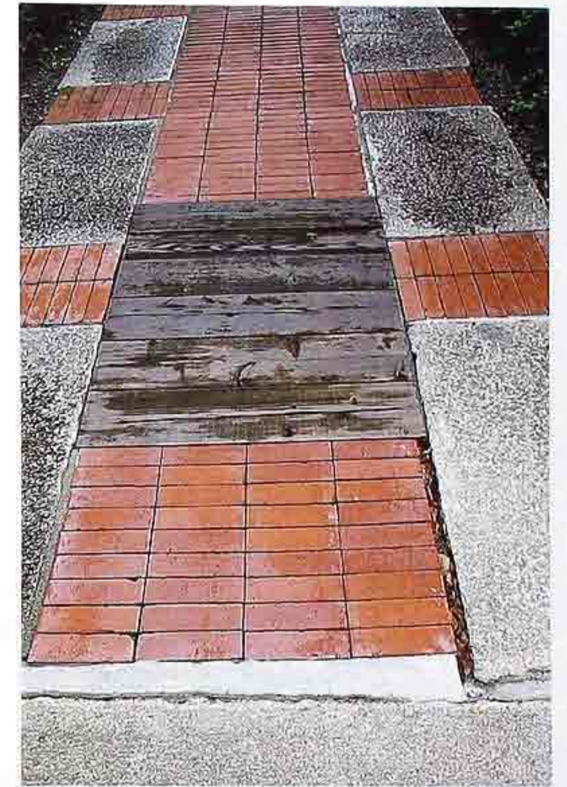
FP-62 Brick pavers in stack bond alternating with wood planks and large-aggregate concrete, urban public space
