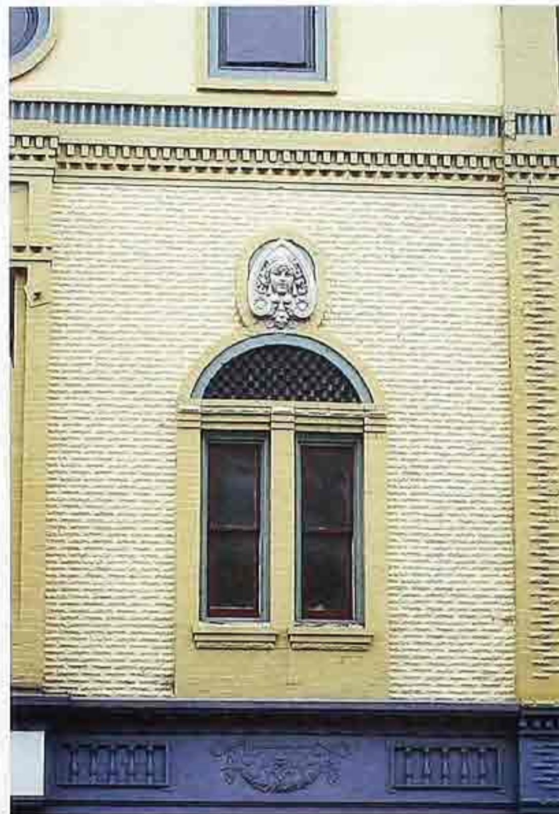
WA-176 Painted rock-face brick with dentil molding, pilasters, and double window under arch in recessed panel with cartouche
