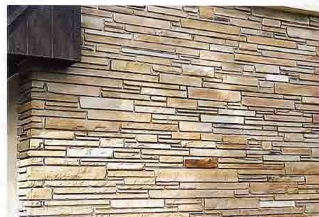
WA-65 Split- and rock-faced sandstone; shelf course, random ashlar with raked mortar
