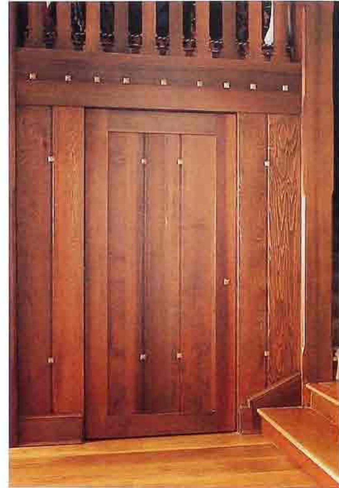
WA-19 Framed oiled cedar vertical board paneling, interior hallway
