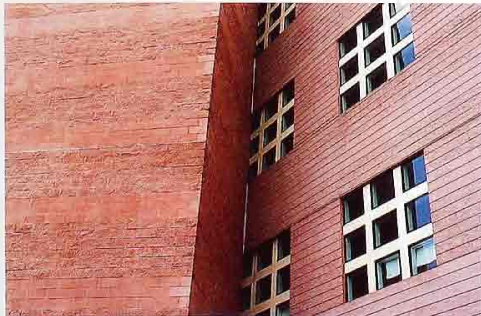
WA-225 Interior and exterior corners of split-face concrete walls with banding and smooth-faced and contrasting color block, modern commercial building
