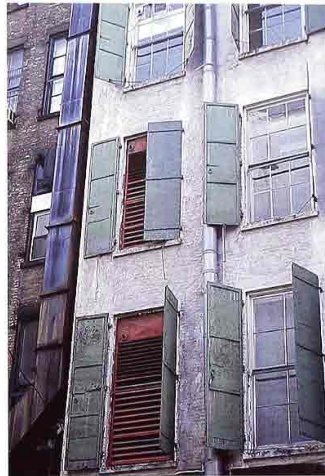
WI-179 Metal shutters, 19th-c. industrial building
