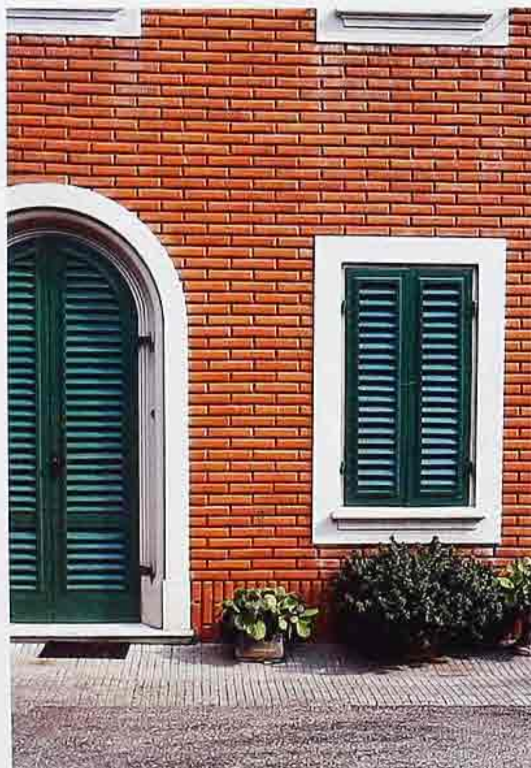
WA-177 Modern variation of Roman brick in running bond with tinted mortar and soldier base course; louvered shutters on door and window
