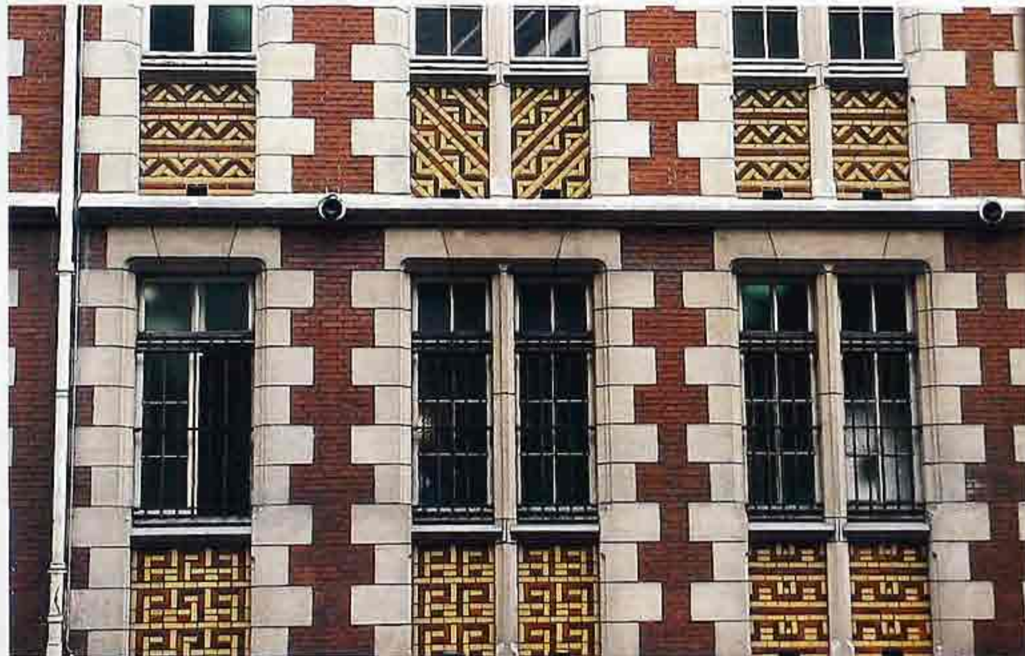
WA-292 Brick with stone quoins between spandrels with geometric tile patterns
