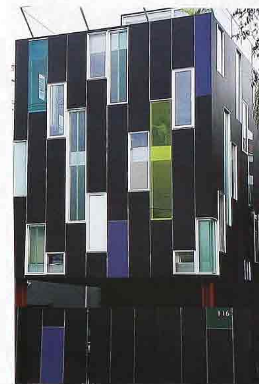
WI-16 Colored and clear fixed and casement windows (note floor plate behind the middle windows), modern house
