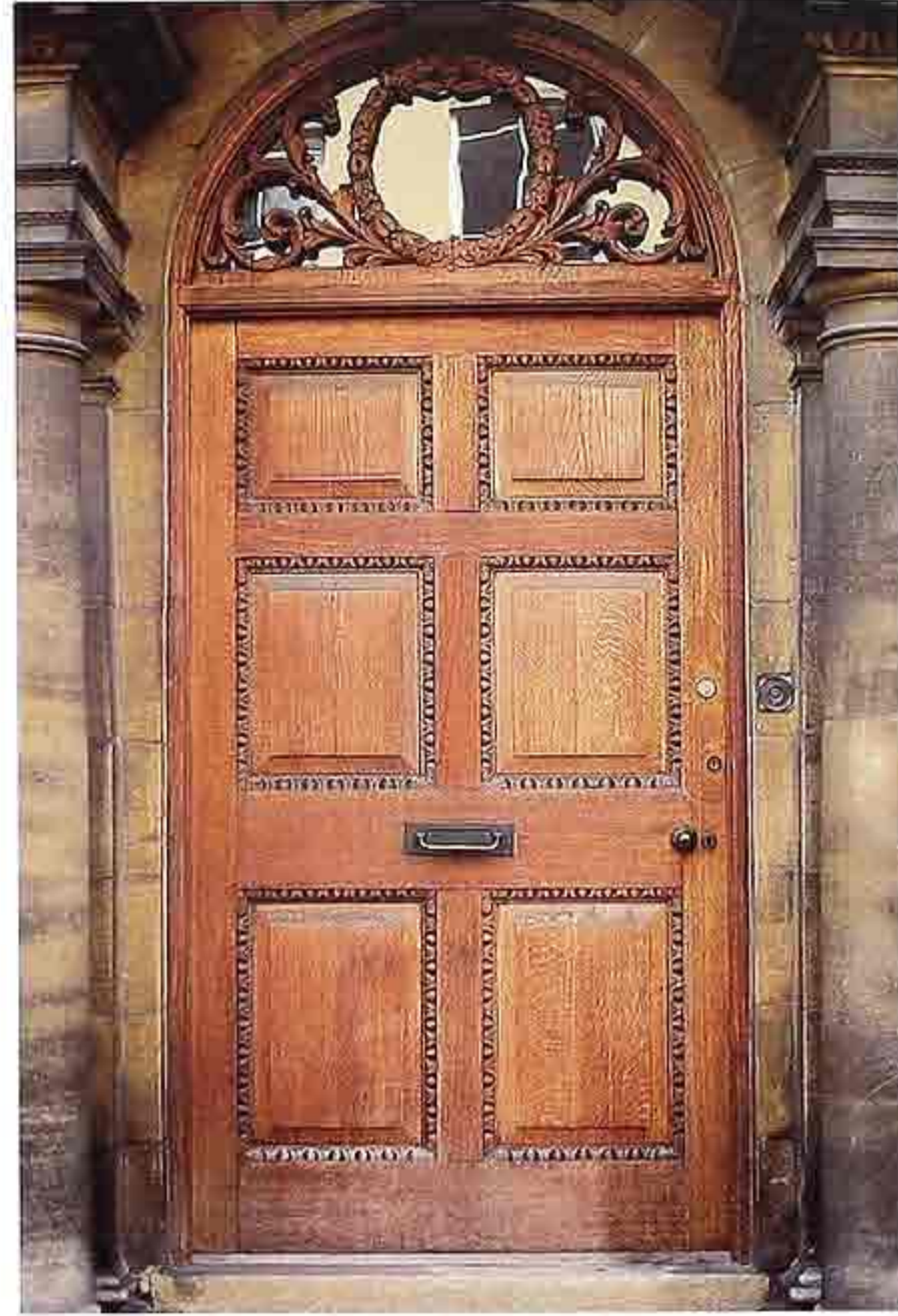
DW-17 Six-panel wood door with raised panels, carved molding, and half-round transom light
