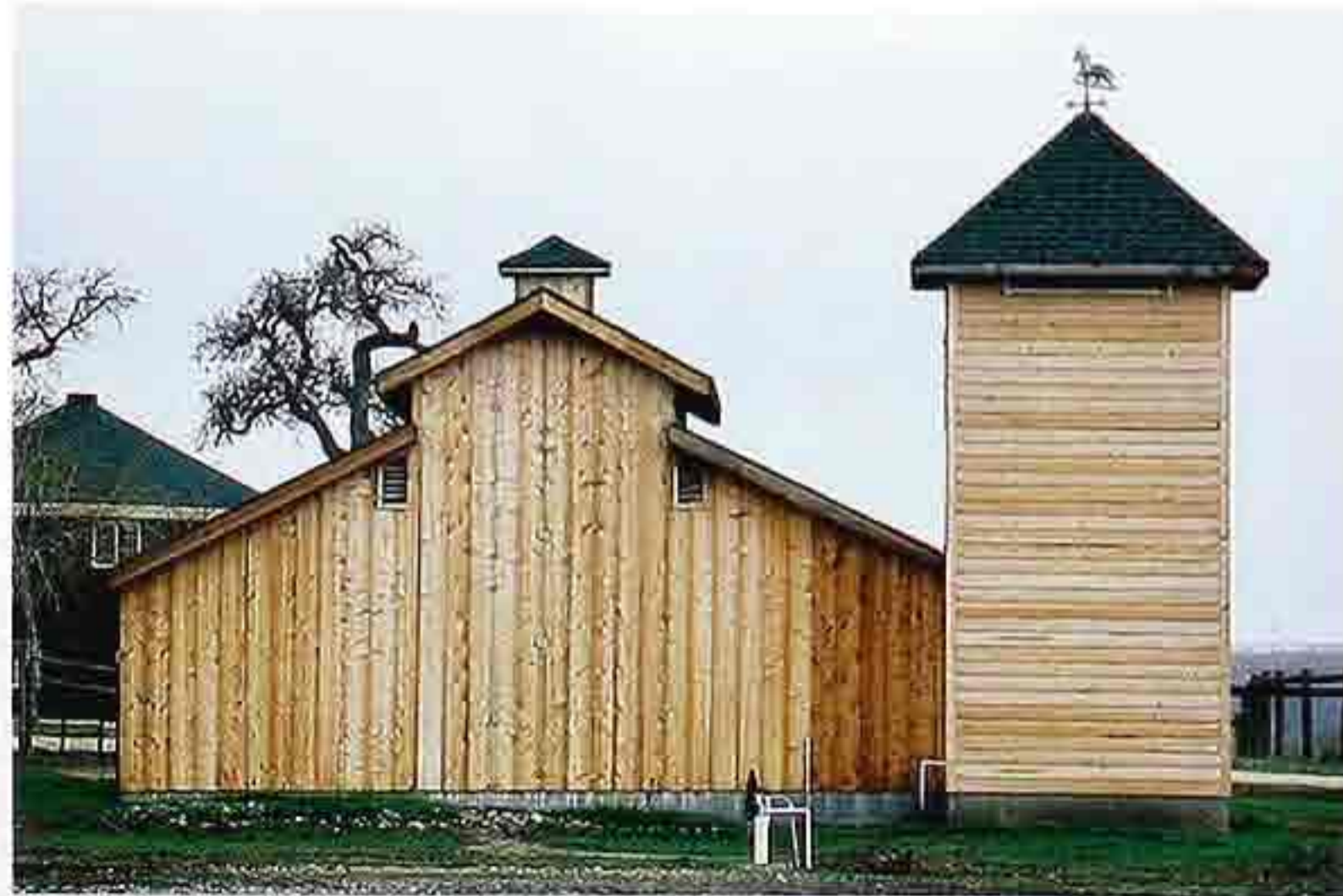
CR-119 Left: gable with gable monitor and cupola; right: pyramid roof with weather-vane
