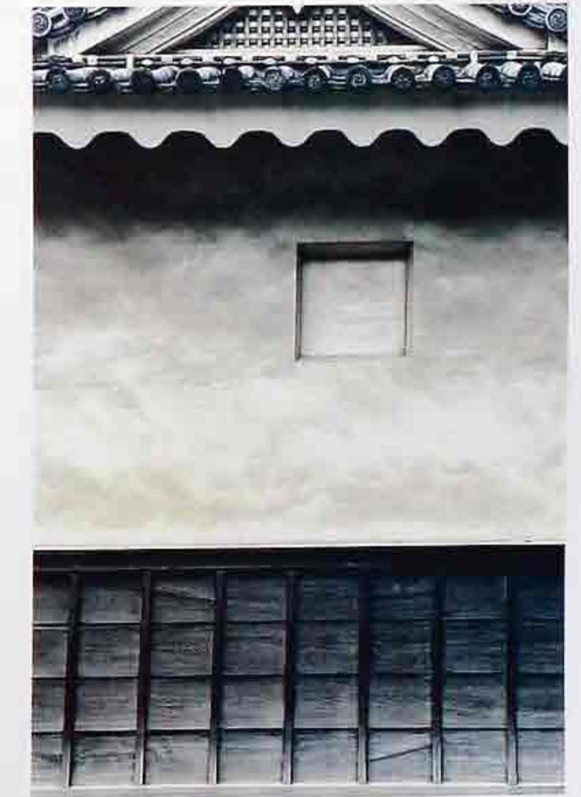
WA-281 Timber frame with infill of undulating stucco and framed planks, traditional Japanese building
