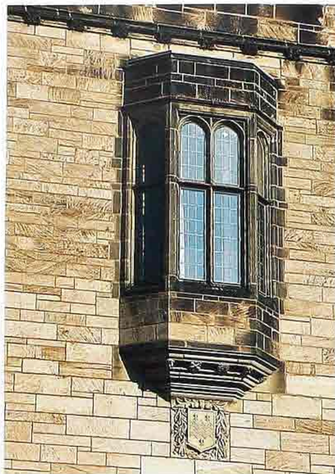
WA-114 Partially cleaned Indiana Birmingham buff limestone, sawn veneer, in random ashlar with oriel
