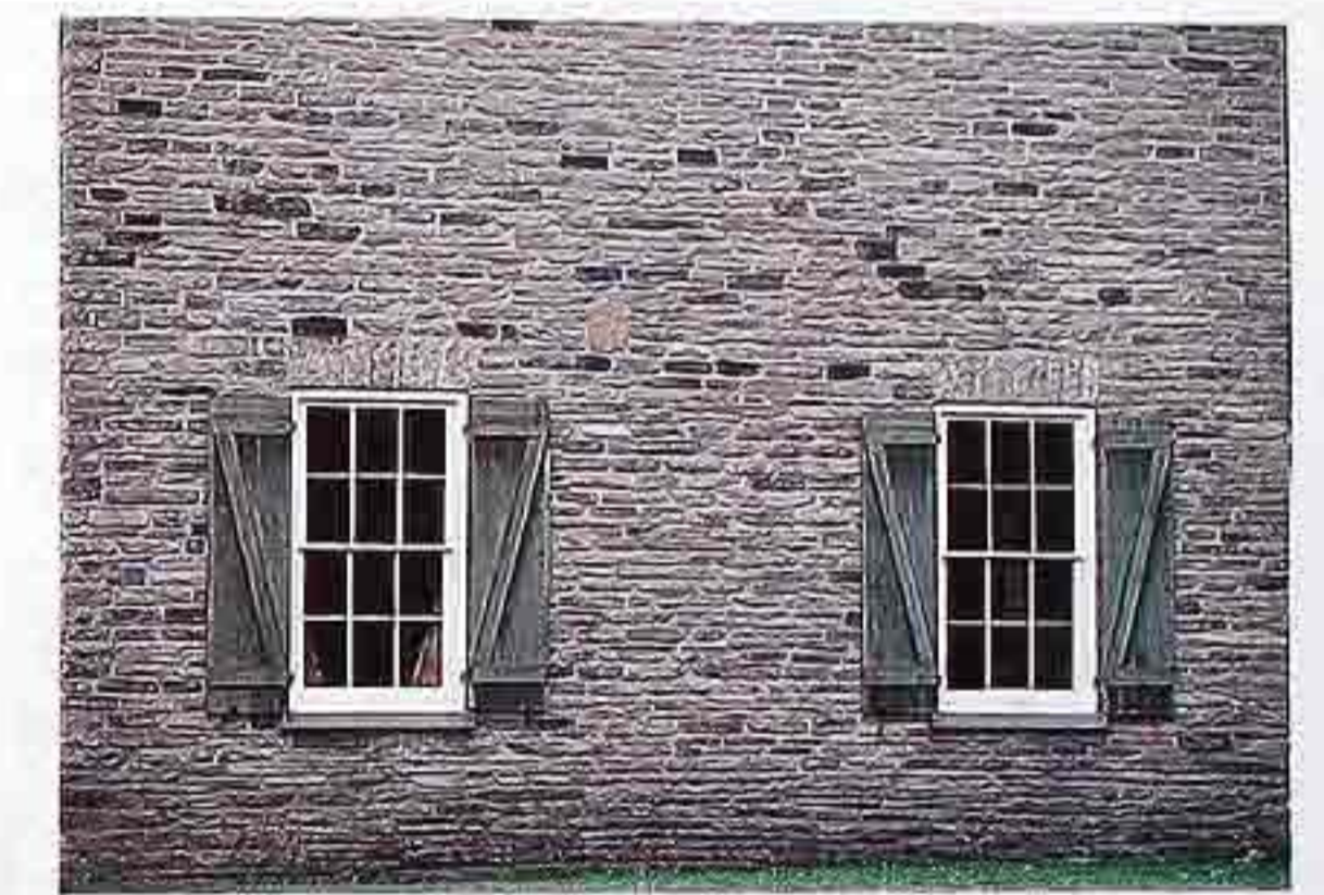
WI-192 Shutters with Z-battens
