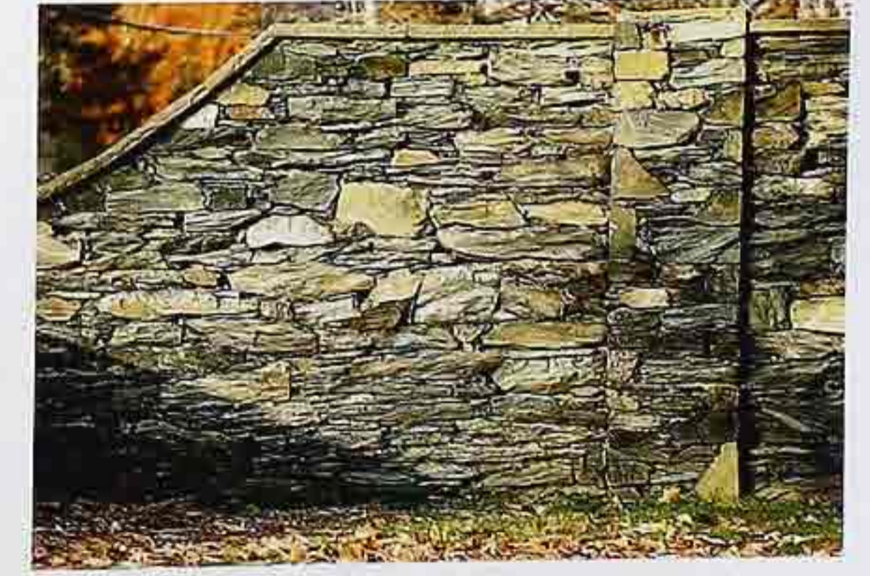
WA-81 Coursed rubble drywall with pilaster and flagstone coping
