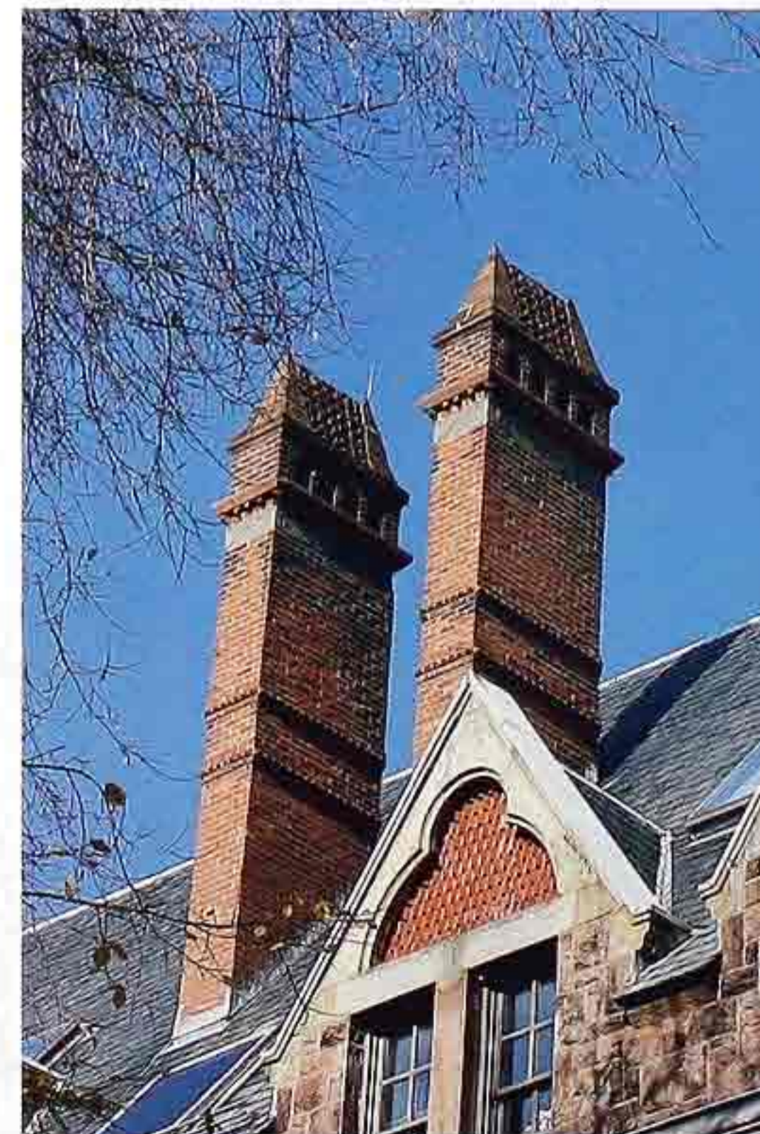
CR-145 Brick chimneys with hipped chimney hoods
