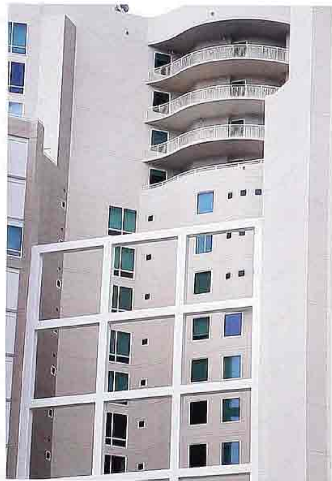
FA-130 Facade of simple punched windows, curvilinear balconies, and large-scale open grid, modern apartment house
