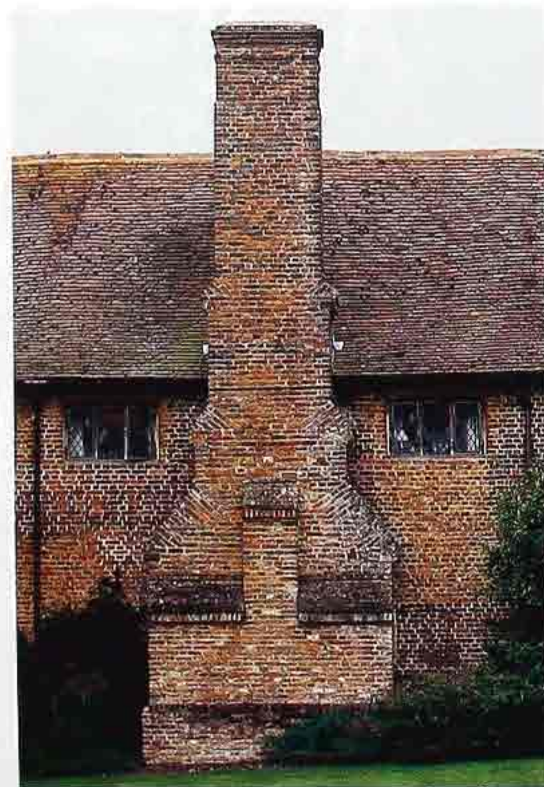
CR-149 Brick chimney
