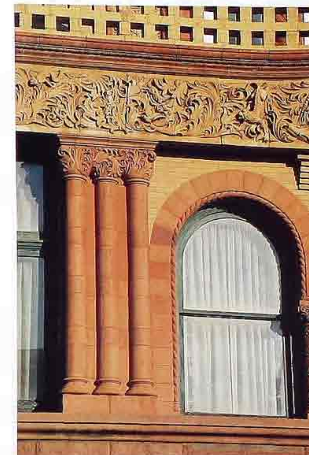
CP-93 Triplet of engaged Romanesque columns with foliated entablature
