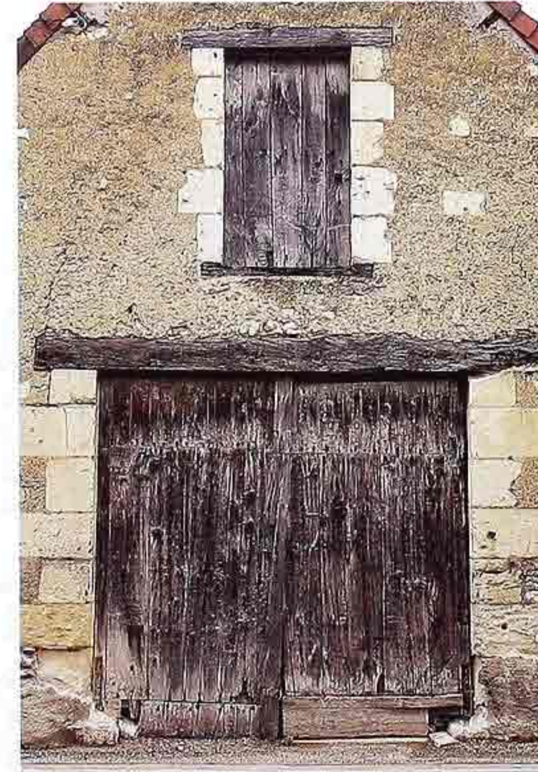
DW-26 Weathered plank doors under rough-hewn timber lintel; rustic stone and stucco gable wall of barn and hayloft
