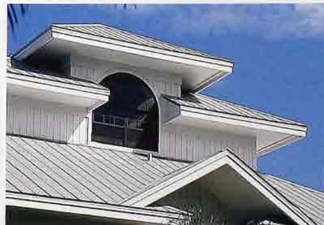
CR-113 Multiple eaves on hipped roof dormers and gable-wall dormers
