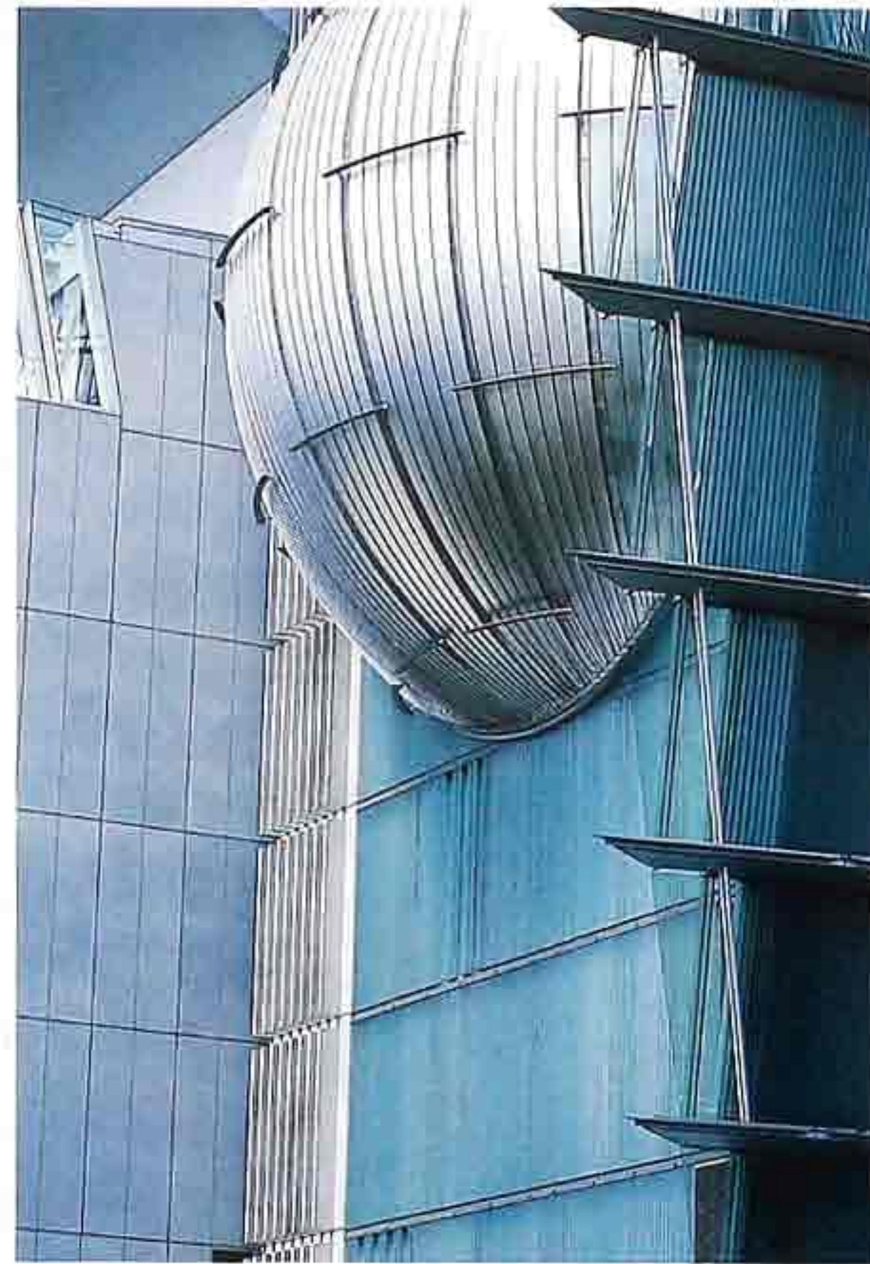
FA-27 Ovoid projection on facade made of custom fabricated metal panels, modern commercial building
