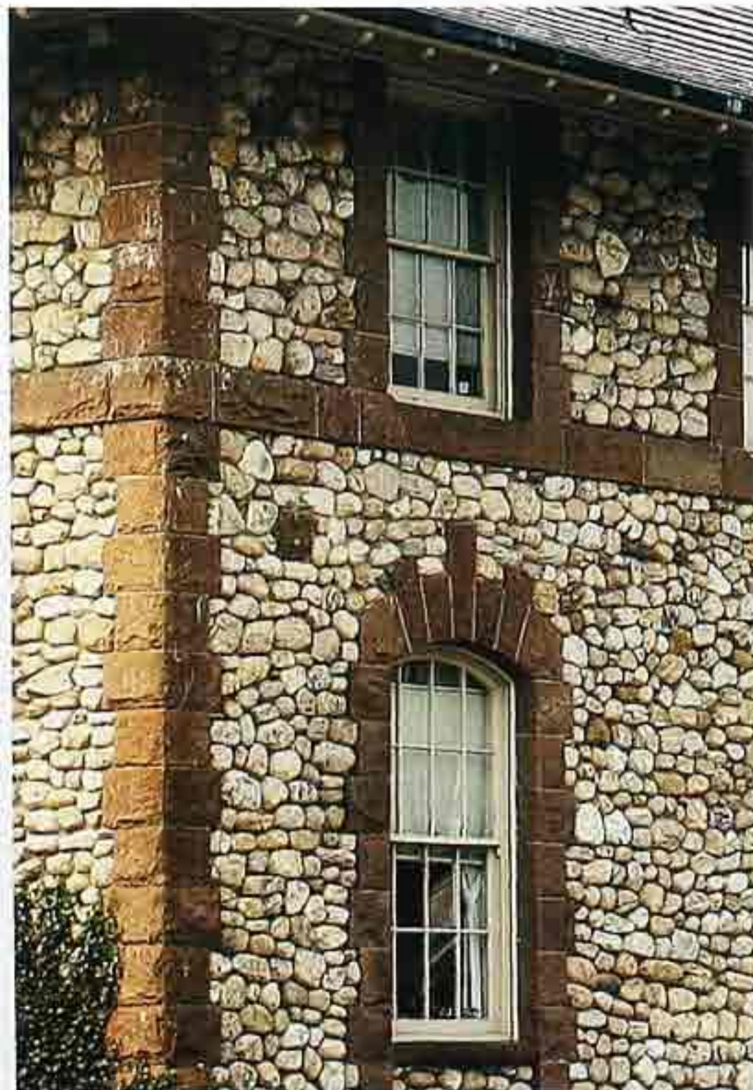
WA-108 Random rubble of cobbles with rusticated dimension-brownstone quoins, belt course, and voussoirs around arch window
