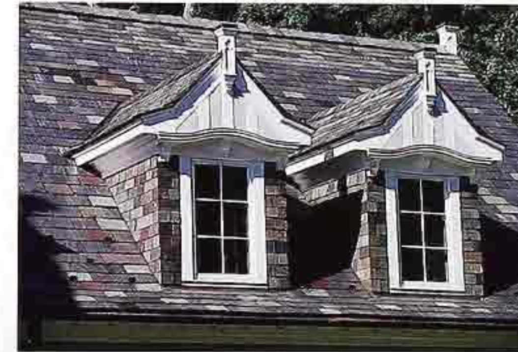
CR-82 Double roof dormers clad with slate shingles
