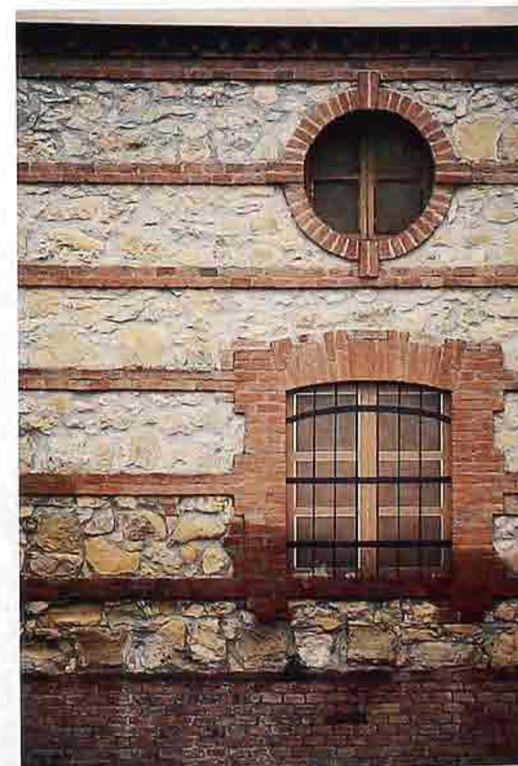
WA-288 Uncoursed rubble wall with brick-framed windows and brick belt courses; cambered arch window with trompe l'oeil grille and shutters
