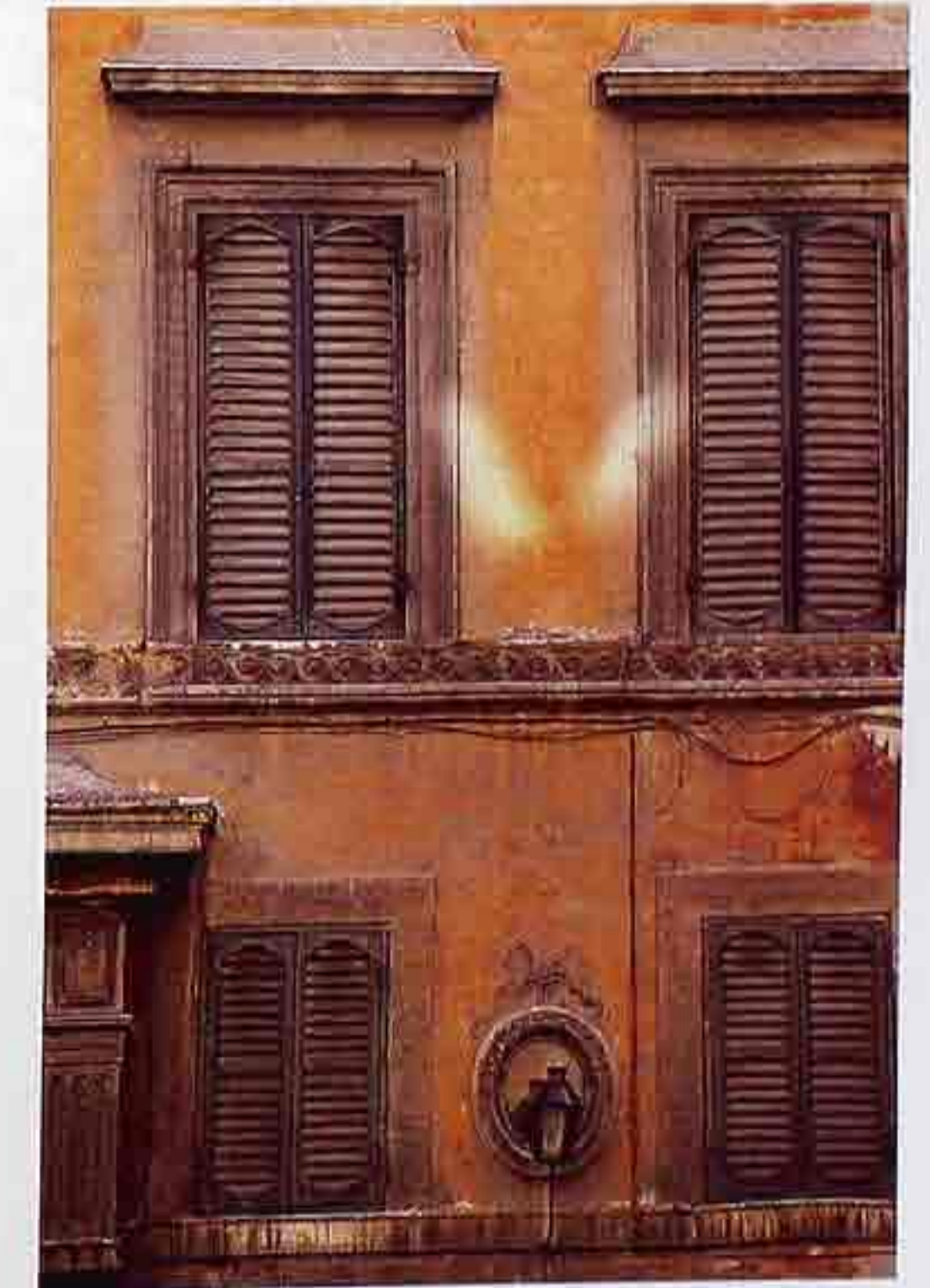
WI-182 Pairs of framed louvered shutters
