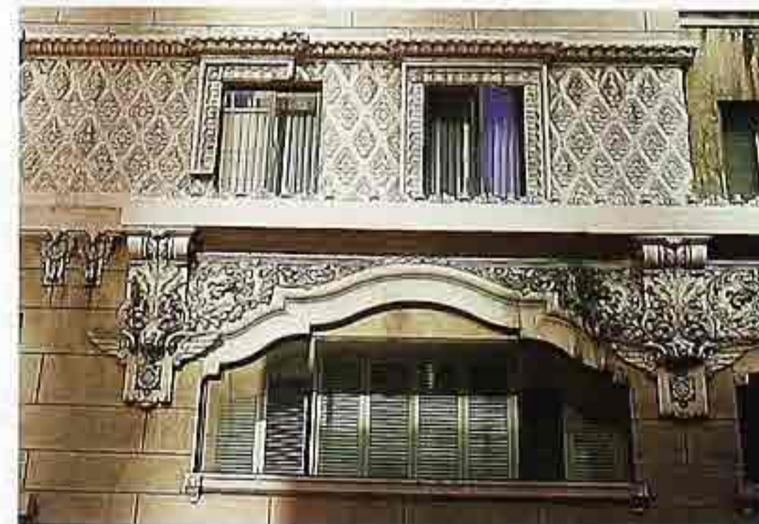
WI-145 Assortment of moldings and ornament around square casement windows over profiled fixed window
