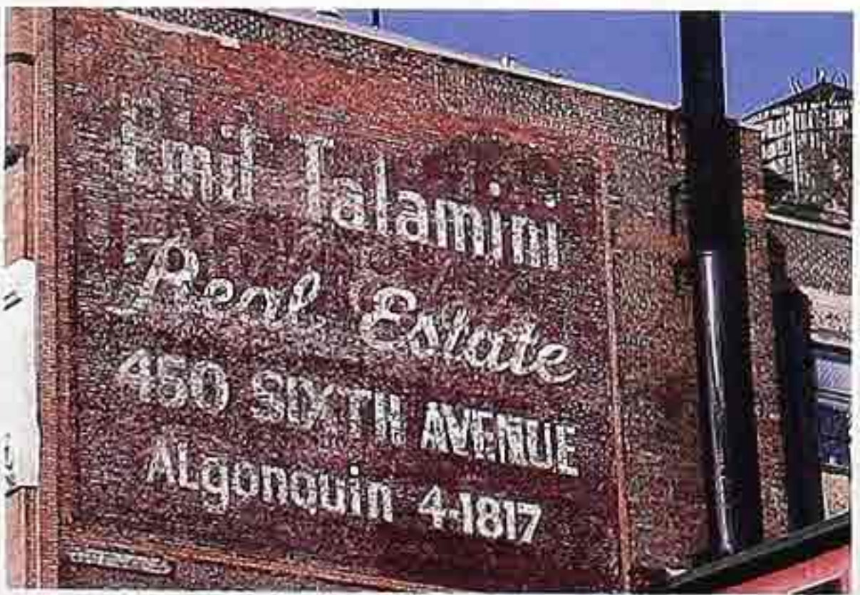
FA-106 Painted sign on blank brick facade
