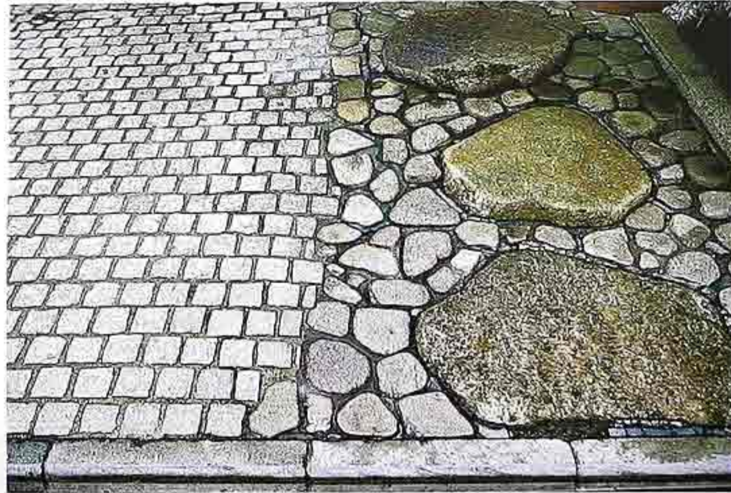
FP-37 Paving stone in running bond (left), with split fieldstones around split bolders; border of roughly squared paving stone
