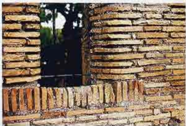
WA-158 Roman bricks with soldier course and shaped bricks forming crenel, ancient parapet wall
