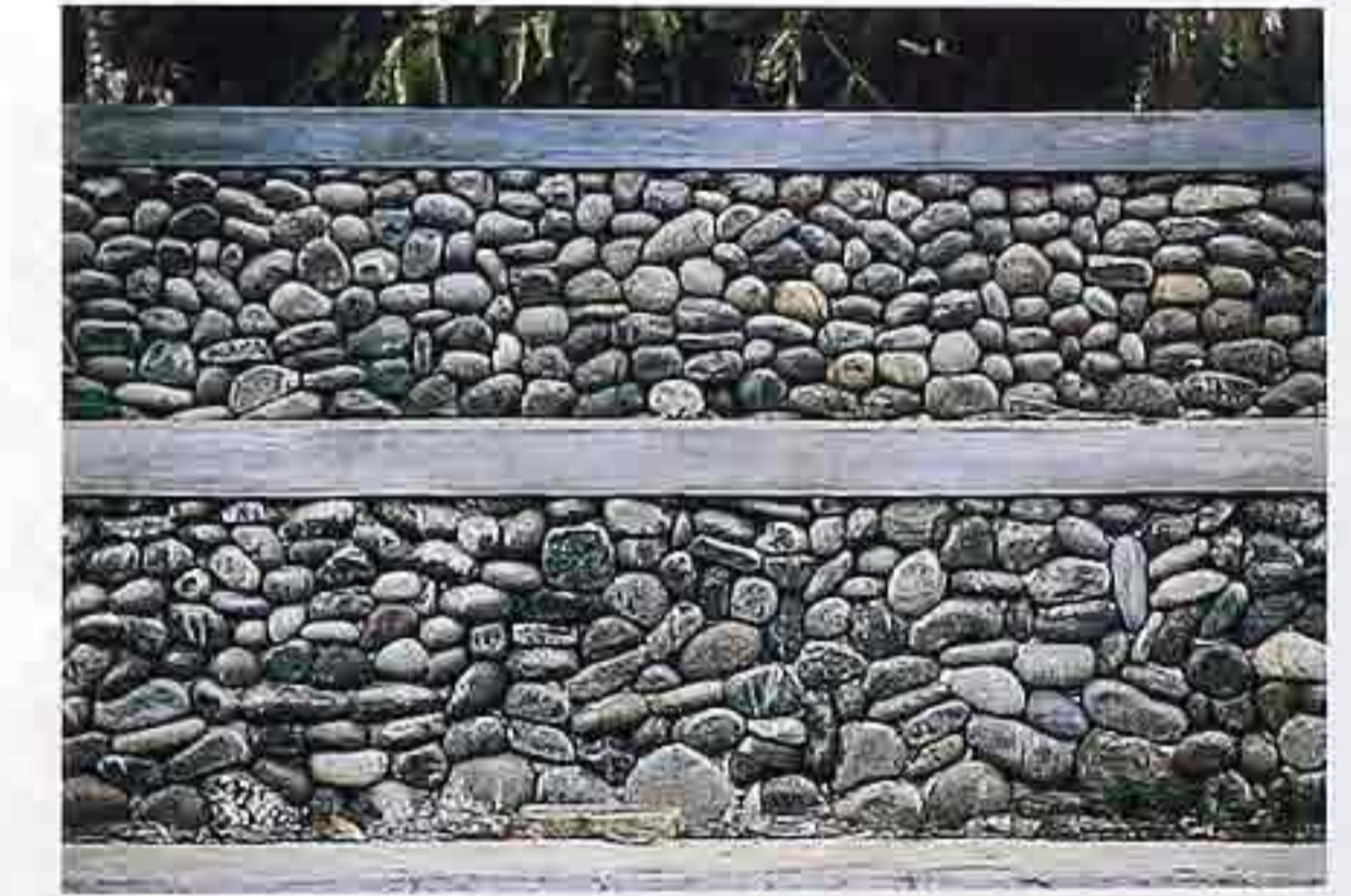
WA-79 Rubble walls of cobbles with wide squared stone step capping lower wall and coping on upper wall
