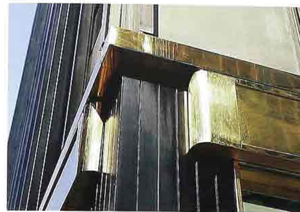
OM-73 Metal cladding suggesting a frieze and cornice, "entablature" broken at corner to reveal the soffit of the "cornice," modern building facade
