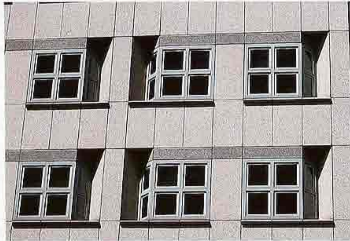
WI-160 Stone spandrels dividing recessed square metal fixed windows, modern commercial building
