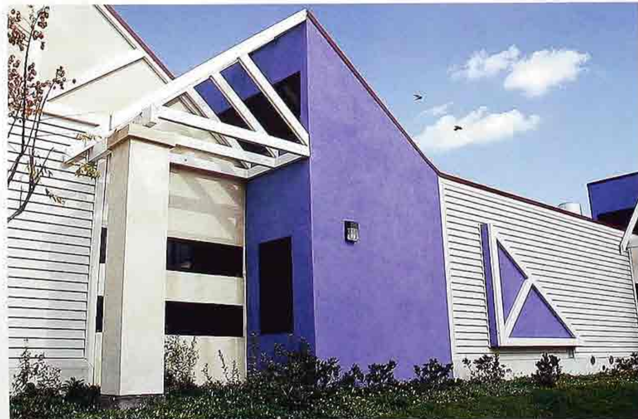
CR-142 Shed-roofed entry with revealed rafters, braces, and joists
