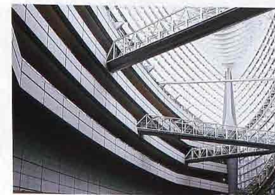
CR-17 Elliptical atrium of metal-framed glass with pedestrian bridges, modern commercial building
