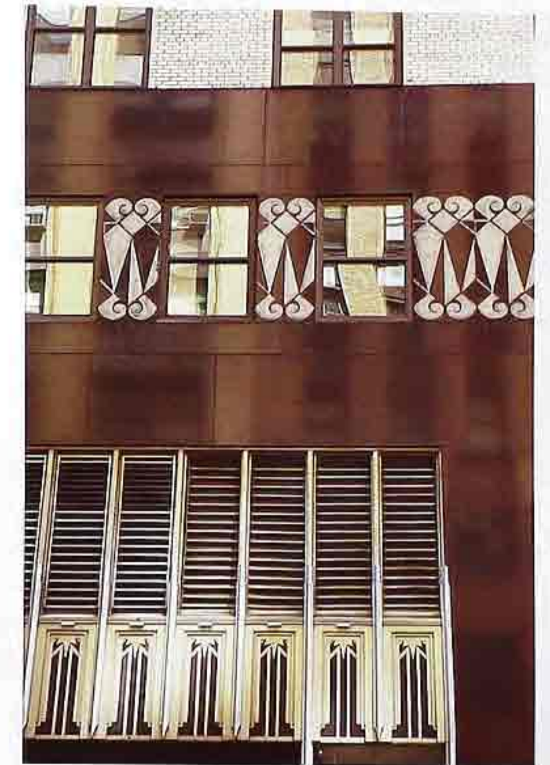
FA-116 Art Deco facade, highly polished stone cladding with geometric ornament below white glazed brick
