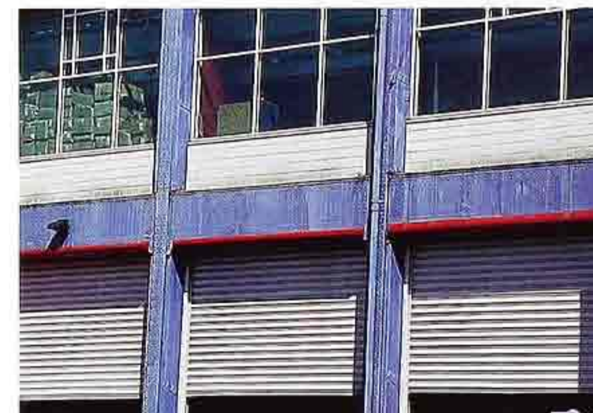
CP-118 Painted metal beam with welded and riveted connections; painted corrugated metal walls
