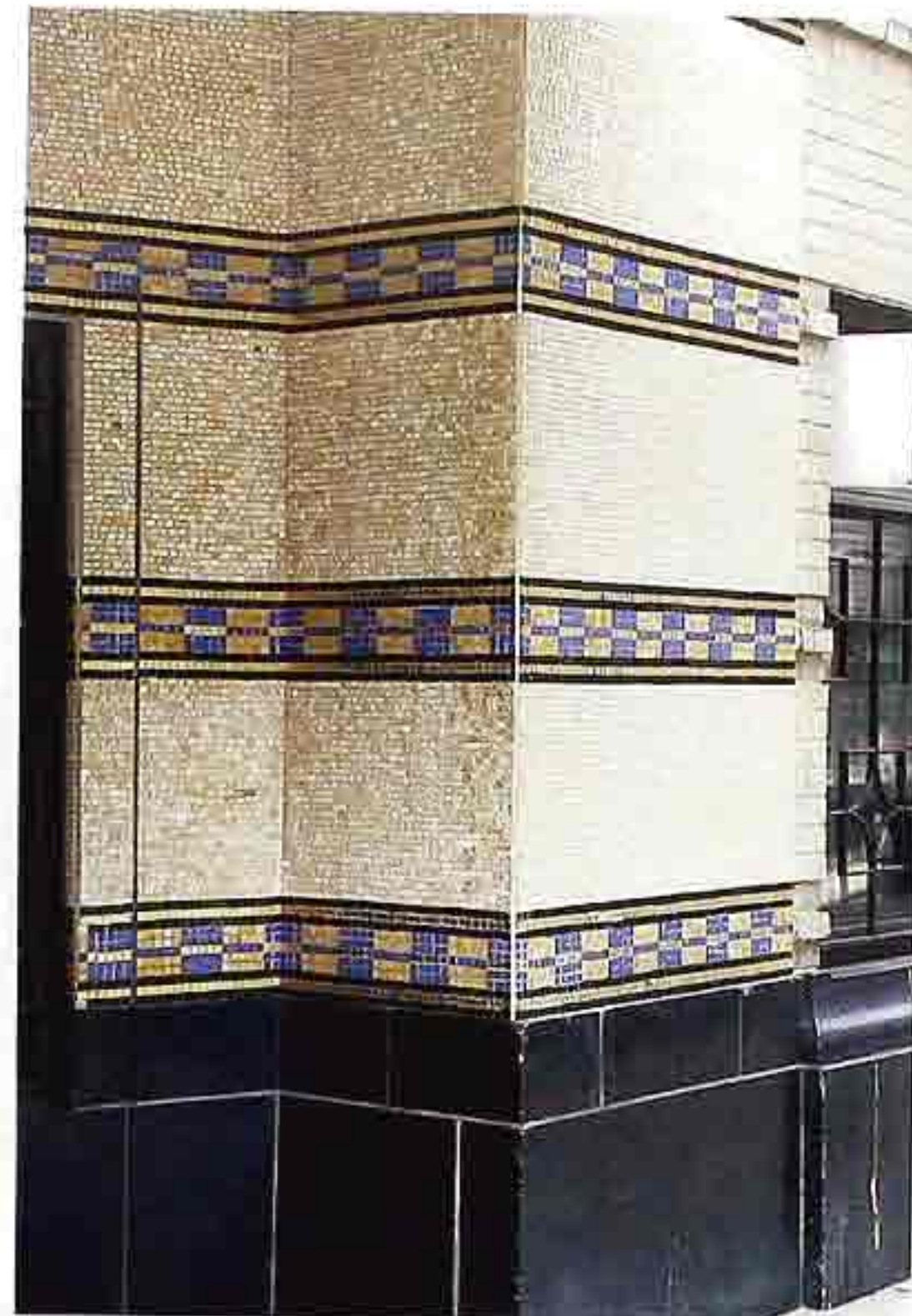
FA-69 Mosaic with horizontal bands of tiles in geometric pattern, entry of modern apartment house
