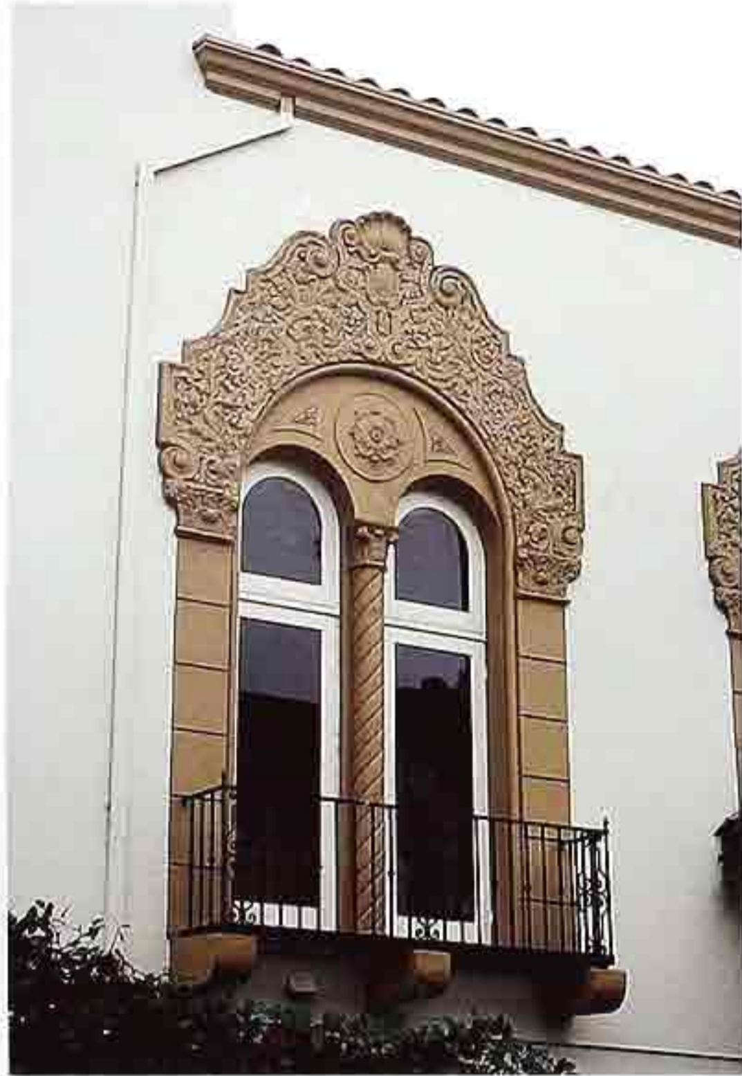
WI-150 Relief ornamental panel and pilasters around variation of Venetian-style window with balcony; 20th-c. apartment house
