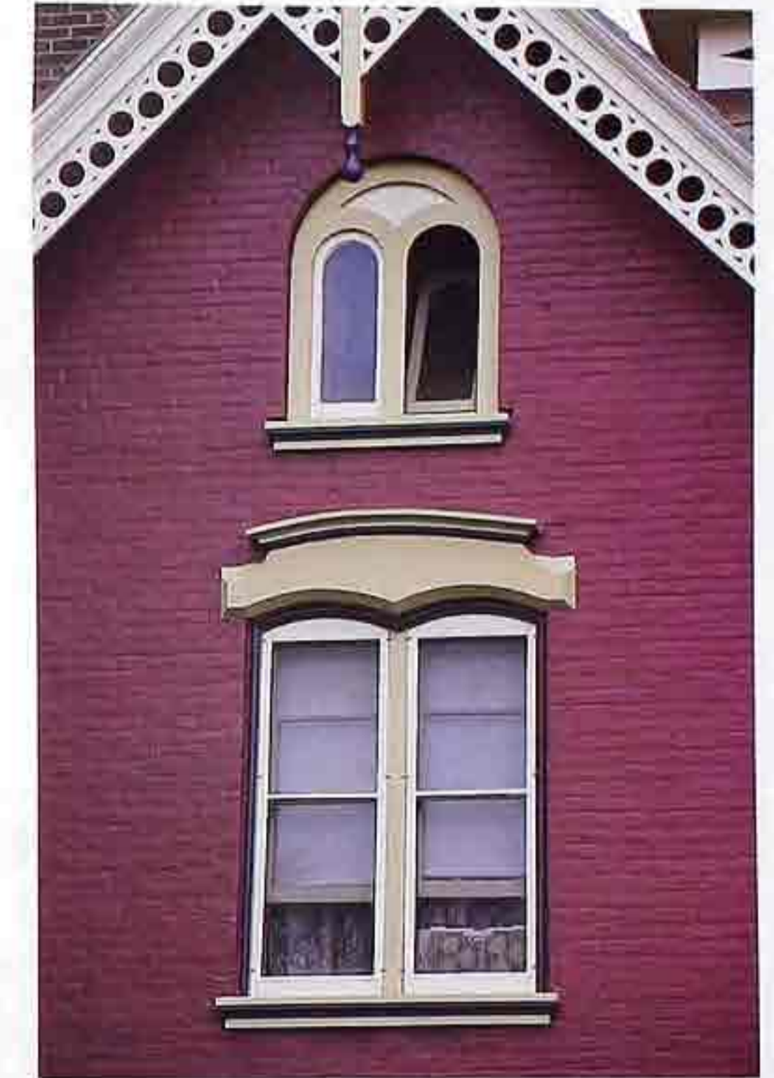
WI-108 Flat trim echoing arch profiles of window openings, American brick house
