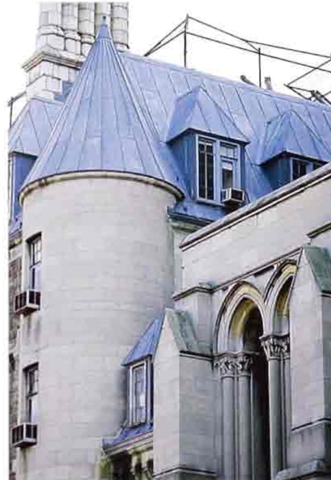
CR-33 Sheet metal with standing seams on conical turret roof; hipped roof and hipped roof dormer, 19th-c. chateau-style hotel
