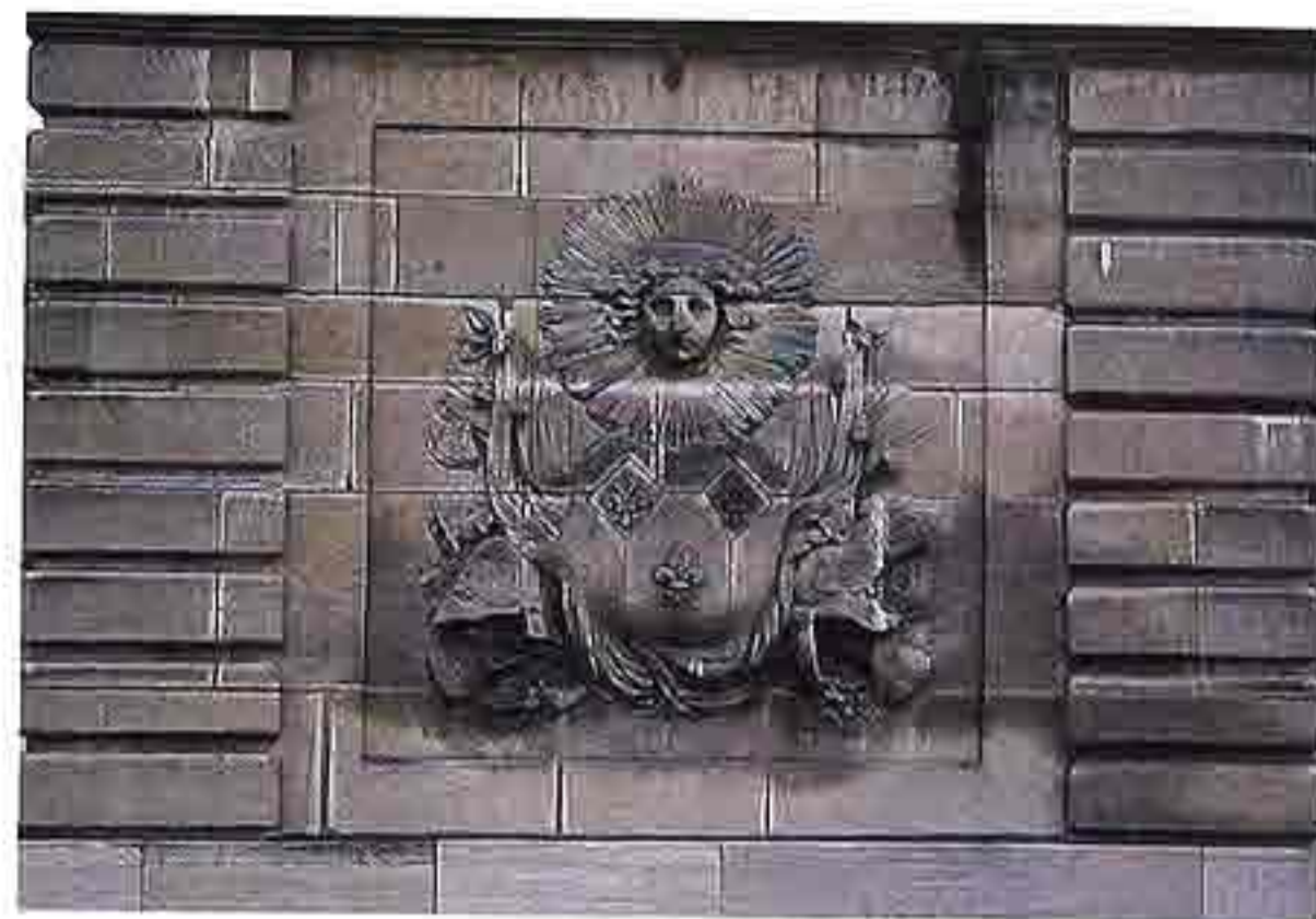
OM-29 Sandstone cartouche in square panel with a mascaron inside a sunburst
