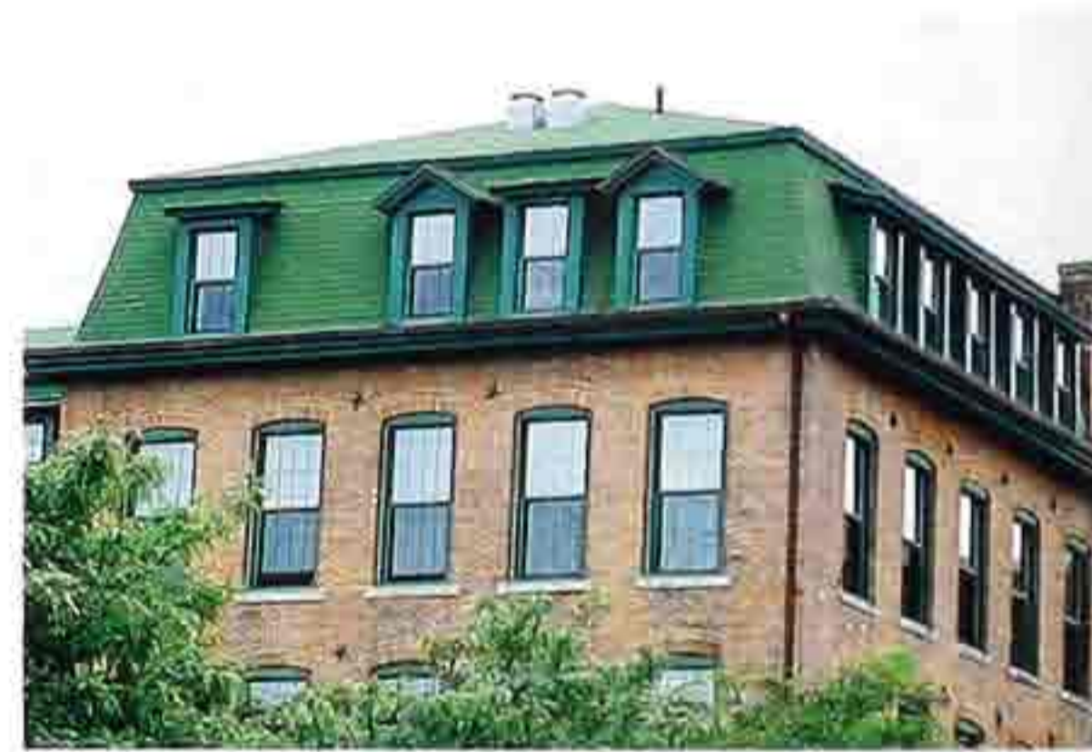
CR-118 Mansard with row of shed dormers (right) and alternating gable and shed dormers (left)
