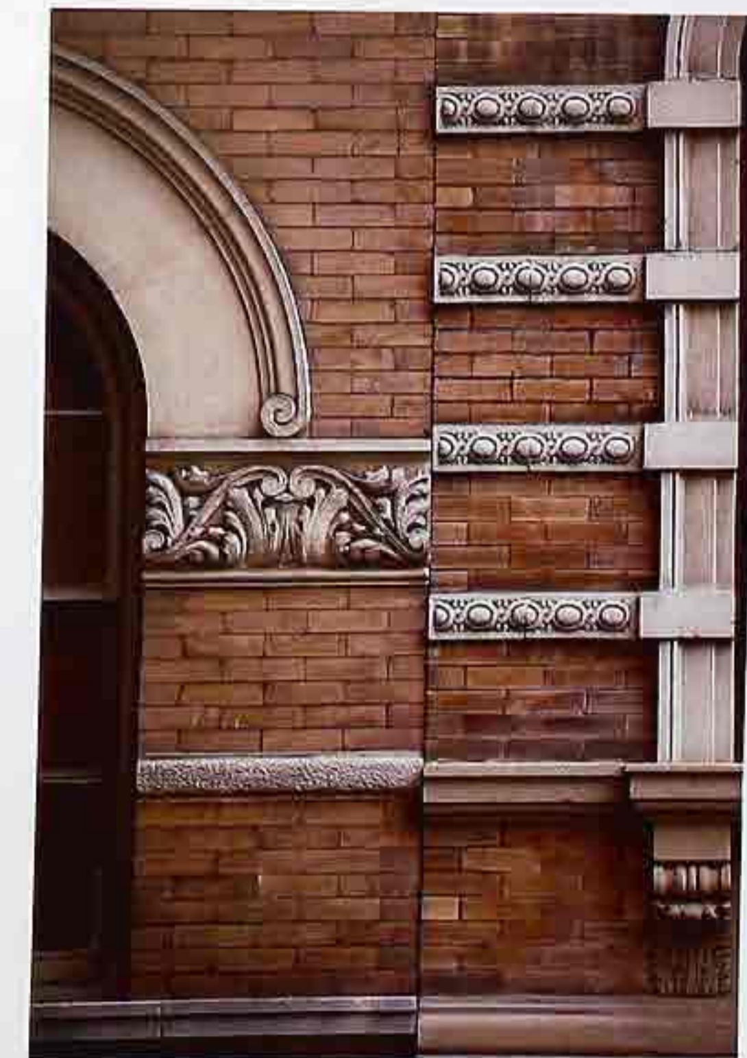
OM-56 Left: scrolled archivolt terminating at a foliated impost; right: banding with guilloche pattern
