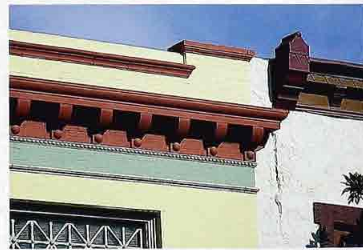
OM-91 Cornice with simple modillion
