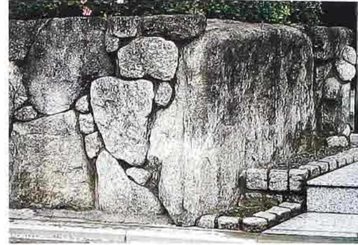
WA-76 Massive rubble with gallets, garden wall
