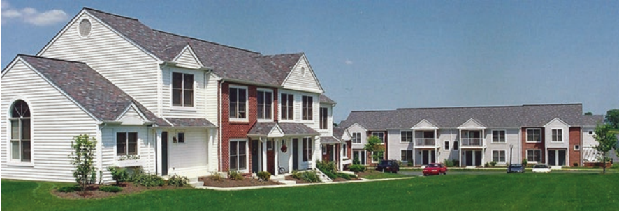
Fig. 8.15 Buildings at Bentley Ridge overlook common greens and sidewalks rather than parking lots
