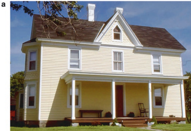
Fig. 5.17 (a) The narrow spans of the American Gothic farmhouse were an inspiration for this model house at Eirean Mohr in Salisbury, MD. (b) The floor plan had modules that were only 14’–16’ wide and had a two-story element facing the street with a one-story element in back. This is the very same practical-yet-livable floor plan of many historic farmhouses
