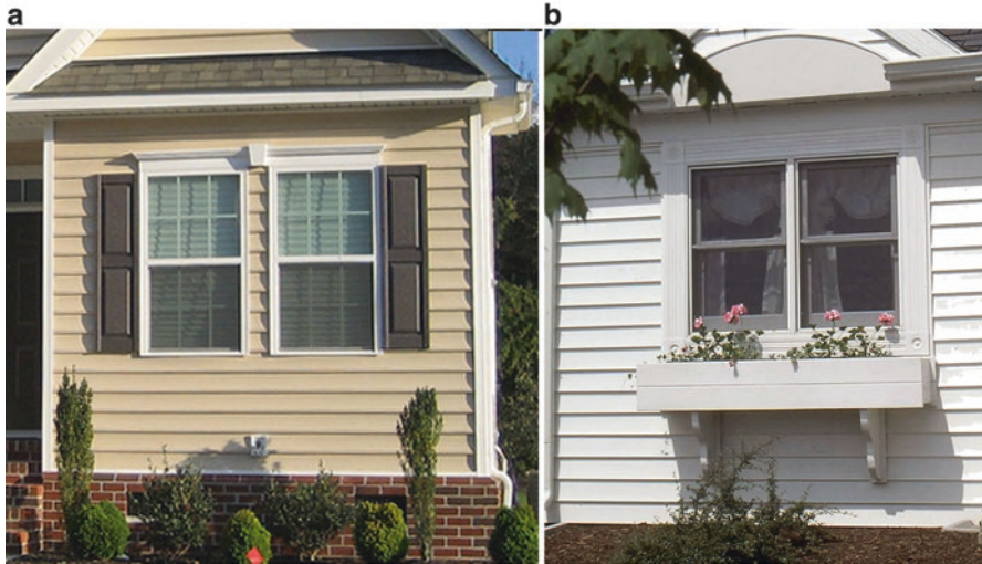
Fig. 7.15 Correct detailing of windows is critical to the success of a façade. (a) Shutters that are out-of-proportion to the window sizes are problematic. (b) Well-received window dressing techniques may include added headers and sills, trim, shutters, and flower boxes
