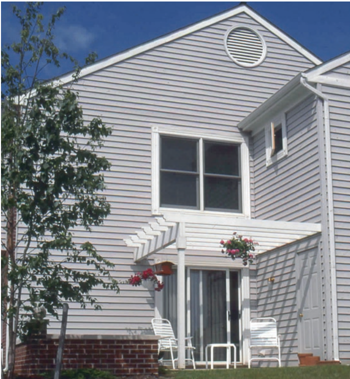
Fig. 8.13 The lower patios at Bentley Ridge in Lancaster, PA are open to the sky, thanks to the upper units' decks being located off of another room in the plan—giving both upper and lower units more privacy in their outdoor spaces
