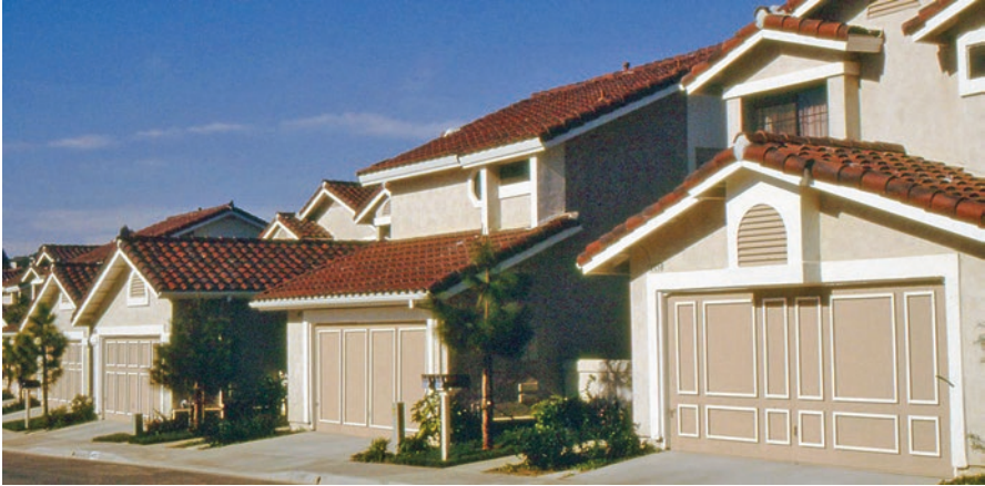
Fig. 2.2 In the Sunbelt and Western states, communities can look like this: tiny lots with narrow frontages, oversized houses dominated by garage doors, and little sign of habitation when viewed from the street
