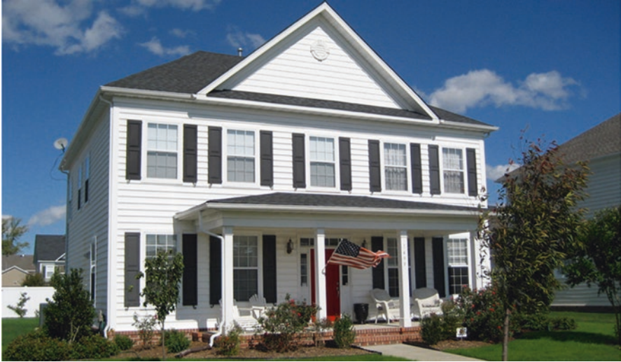
Fig. 7.18 Choosing appealing colors for the materials and other elements is tremendously important, and costs literally nothing to enhance the façade. Light color siding with dark accents and a red door works well
