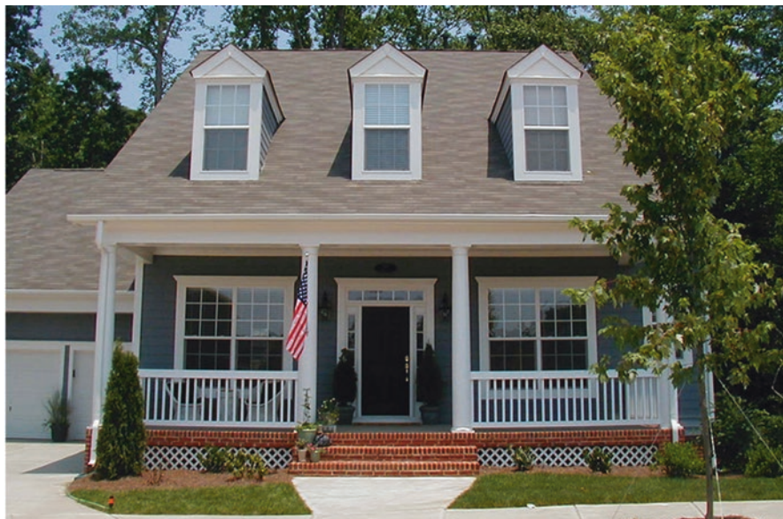
Fig. 7.17 Detailing the façade with appropriately scaled elements is critical. Beams, columns, railings, window trim, and other materials need to be sized to impart a sense of stability and permanence to the home
