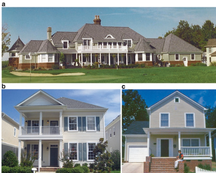
Fig. 5.9 (a) Larger houses tend to be more complex in plan shape, while simplicity is an ally of more affordable houses (b and c)
