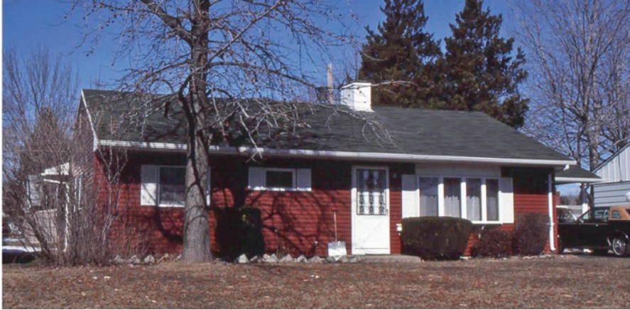
Fig. 7.7 Though a common cost-saving measure, a low roof pitch can often make a house look too cheap
