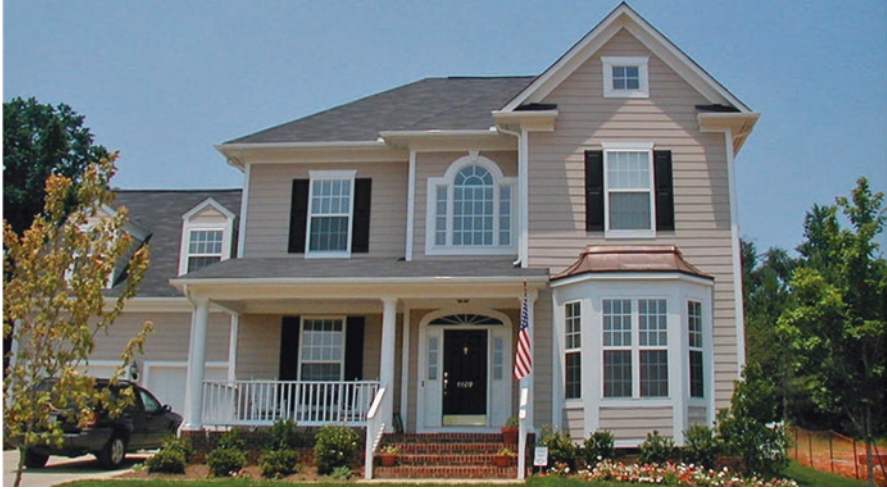
Fig 7.3 In this house, the focus of the front elevation is a large specialty window above the entry door
