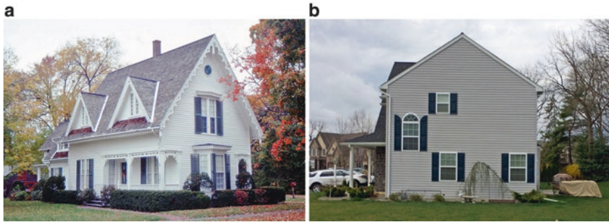
Fig. 5.10 (a) Historical designs generally had a sense of order on all elevations, as seen on this side view of an older house. (b) Today, random placement of windows or other elements on side elevations is common
