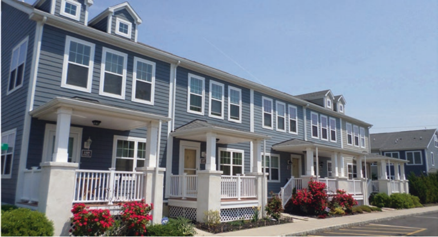
Fig. 9.6 At Schoolhouse Square , site-built front porches and well-ordered façades worked lent themselves to providing an attractive street view for these affordable modular townhouses
