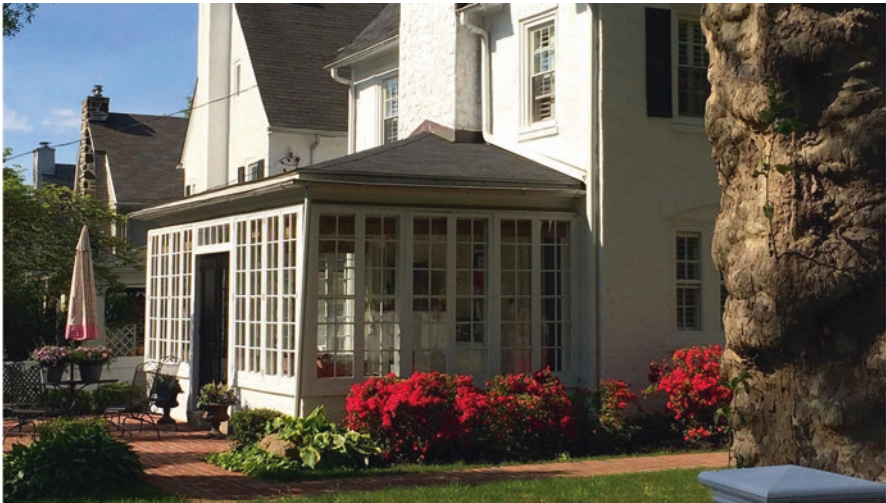
Fig. 5.28 The popularity of sunrooms can be attributed to their projected presence on the main house, and to their three exterior walls made primarily of glass, as seen in this historical example
