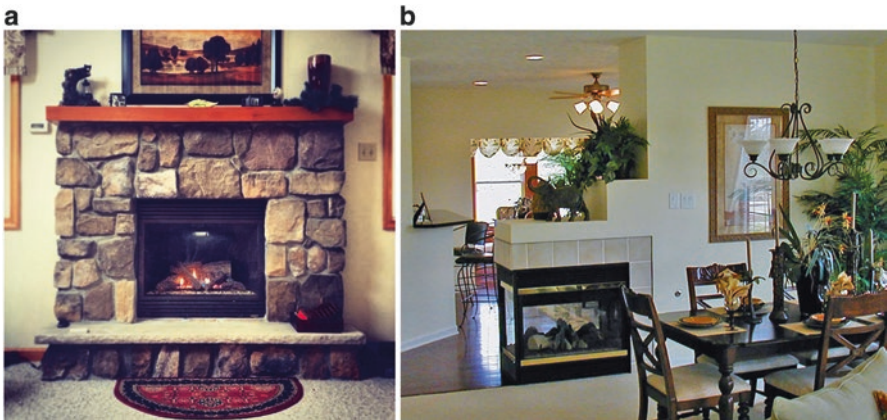
Fig. 6.1 (a) Traditionally, fireplaces have been heavy, site-built masonry structures, but with the introduction of (b) prefabricated assemblies, designers have the freedom to locate fireplaces in new roles
