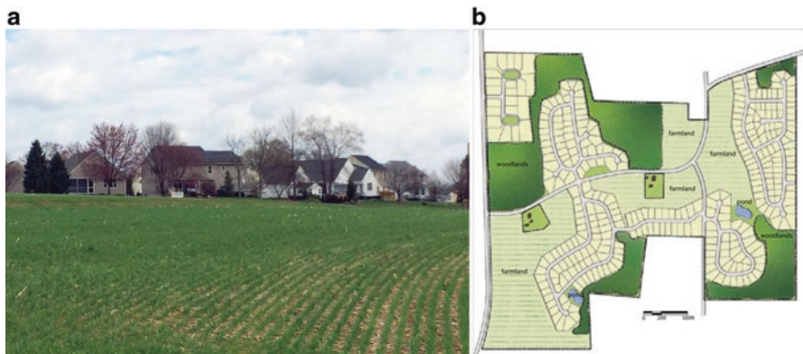
Fig. 3.19 (a) At Charter Homes' Wheatstone in Lancaster, PA, houses were clustered on smaller lots, which allows most homes to border farmland. (b) At Farmview in pastoral Bucks County, PA, Realen Homes clustered 334 homes on roughly half of a 500-acre farm tract, leaving over 180 acres under cultivation and 70 more acres as environmentally sensitive open space. (Figure (b) courtesy National Lands Trust)
